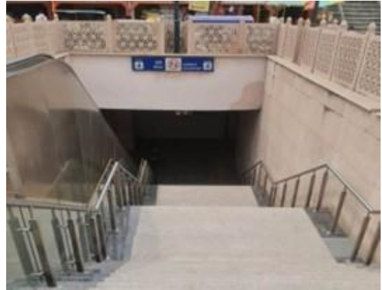
Station Entry to Concourse Level
