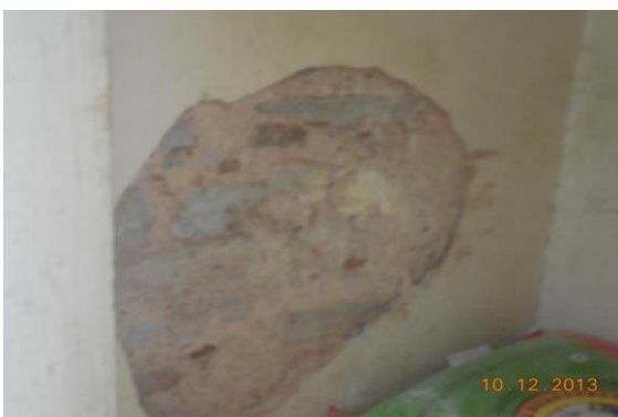
Photo 203 Peeling of Plaster on Wall No. 1 of Store No.1 of First Floor
