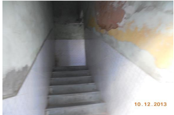
Photo 176 Peeling of Plaster on Wall No. 1 & 2 of Part B Staircase Ground Floor To First Floor of Ground Floor
