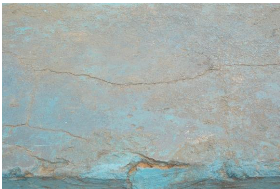
Photo 11 Plaster Crack on External Wall No. 3 of Boundary Wall B of Ground Floor
