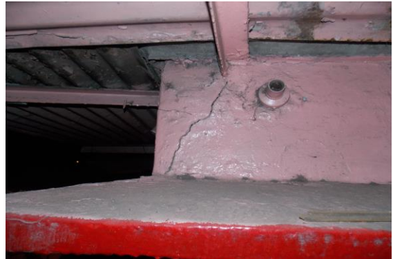
Photo 4 Plaster Crack on Wall No. Leftside Wall of Barahling Temple of Ground Floor
