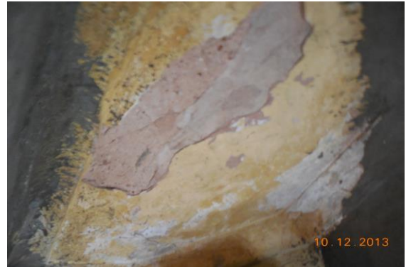
Photo 242 Peeling of Plaster on Roof of Toilet No. 1 of Second Floor
