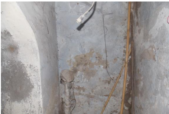
Photo 87 Dampness/Seepage on Wall No. 1, 2 & 4 of Passage No.1 of Ground Floor
