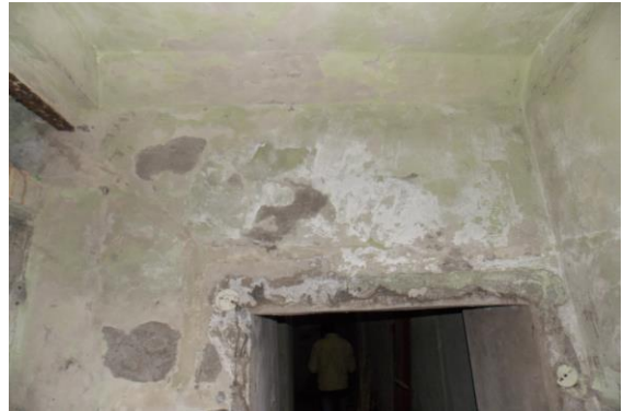
Photo 164 Dampness/Seepage on Wall No. 4 of Passage
