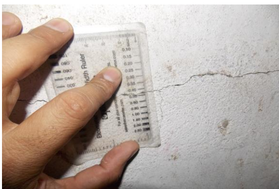
Photo 16A Horizontal Crack on Wall No. 1 of Part A of Shop No. 782, Ground Floor Approx. Width = 0.5mm, Approx. Length = 2.7m. Distance from Wall No. 3 = 0m, Height from Floor = 1.5m.
