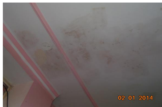
Photo 34 Dampness/Seepage on Roof of Store of First Floor
