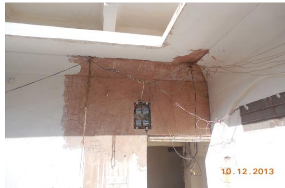
Photo 232 Peeling of Plaster on Wall No. 4 of Open Sky No.3 of First Floor
