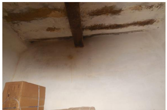
Photo 138 Dampness/Seepage on Wall No. 4 of Room No. 7 of Ground Floor
