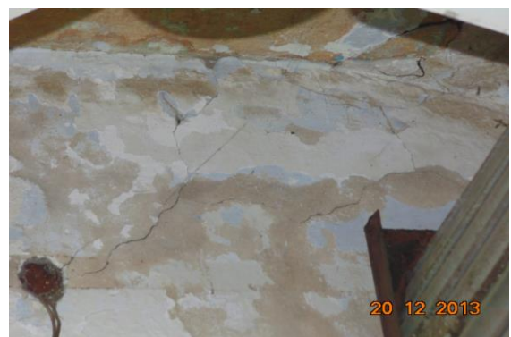
Photo 87 Plaster Crack on Wall No. 4 of Shop No.172 of Ground Floor
