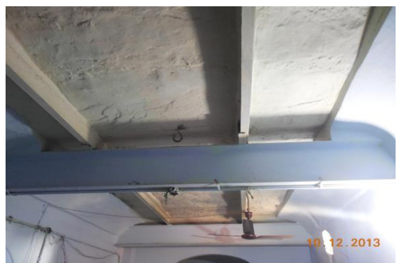
Photo 258 Dampness/Seepage on Roof of Room No. 6 of Second Floor
