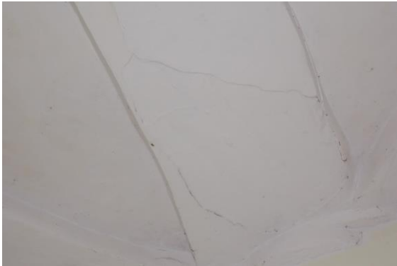
Photo 109 Peeling of Plaster on of Room No. 11 of Ground Floor
