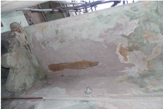
Photo 157 Damaged Portion on Roof of Open Sky area
