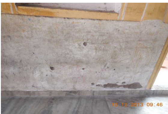
Photo 104 Peeling of Plaster on Wall No. 1 of Varanda 1 of College & Temple, First Floor
