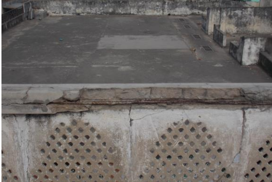
Photo 77 Dampness/Seepage on Wall No. 2, 4 & Roof of Toilet & Washroom of Terrace
