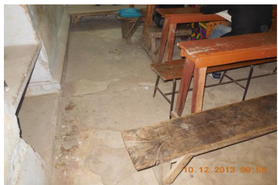
Photo 105 Peeling of Plaster on Floor of Hall No. 1(Part-I) of First Floor
