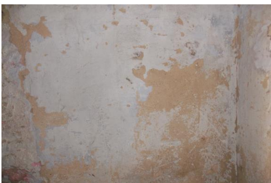
Photo 61 Peeling of Plaster on Wall No. 3 of Stair GF to FF of House No. 758, Stair Ground Floor to First Floor
