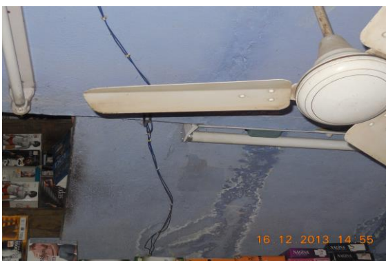
Photo 53 Dampness/Seepage on Roof of Shop Luxmi Agency of Ground Floor
