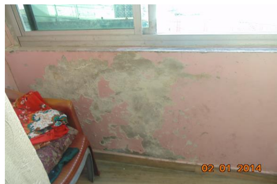
Photo 40 Dampness/Seepage on Wall No. 4 of First Floor
