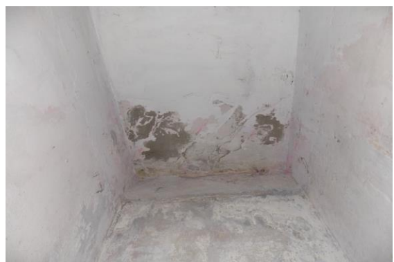
Photo 62 Dampness/Seepage on Roof of House No. 758, First Floor
