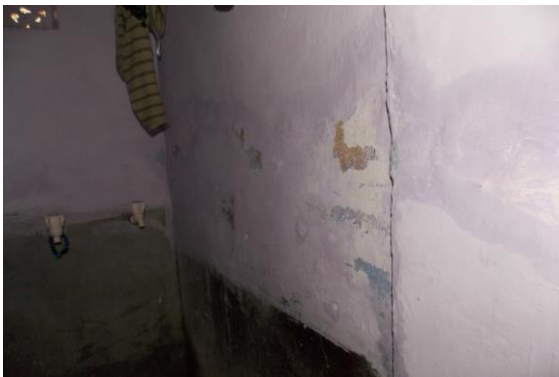
Photo 21 Peeling of Plaster on Wall No. 2 of Bathroom No. of First Floor
