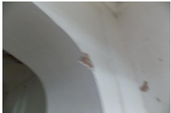
Photo 124 Peeling of Plaster on Wall No. 4 of Room No. 9 of
