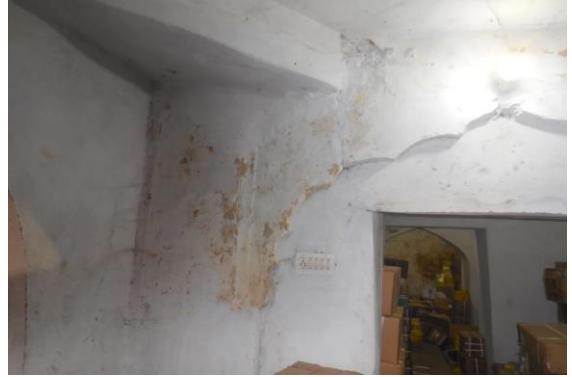
Photo 134 Peeling of Plaster on Wall No. 2 of Hall No. 1 of Ground Floor
