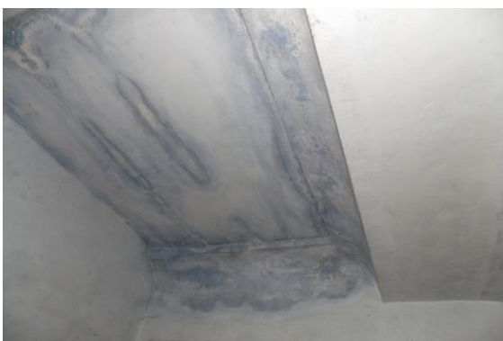
Photo 44 Dampness/Seepage on Wall No. 2 of Part C of Shop No.776 of Ground Floor
