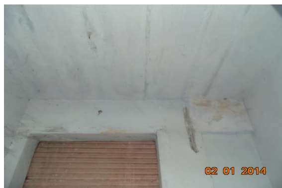
Photo 16 Dampness/Seepage on Wall No.1 & Roof of Shop No. 1 of Ground Floor
