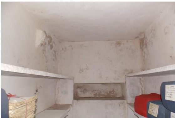
Photo 129 Dampness/Seepage on All Walls of Room No. 16(Part E)
