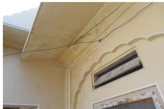
Photo 234 Dampness/Seepage on Wall No. 2 & Shade of Open Sky No.2 of First Floor
