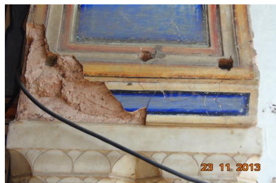
Photo 48 Peeling of Plaster on Column of Varanda No.1 of Ground Floor
