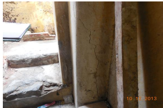
Photo 42 Inclined Crack on Wall No. 4 of Passage No. 1, First Floor, Approx. Width = 2.5mm, Approx. Length = 1.4m. Distance from Wall No. 2 = 0.1m, Height from Floor = 0m.
