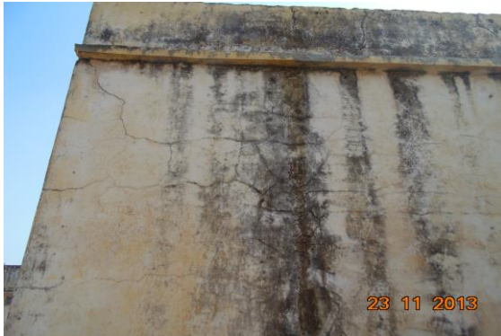
Photo 63 Peeling of Plaster on Wall No. 7 of Open area No.2 of First Floor
