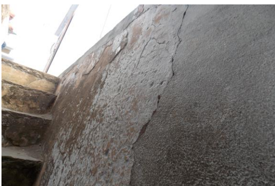
Photo 29 Peeling of Plaster on Wall No. 2 of Staircase FF to SF of First Floor
