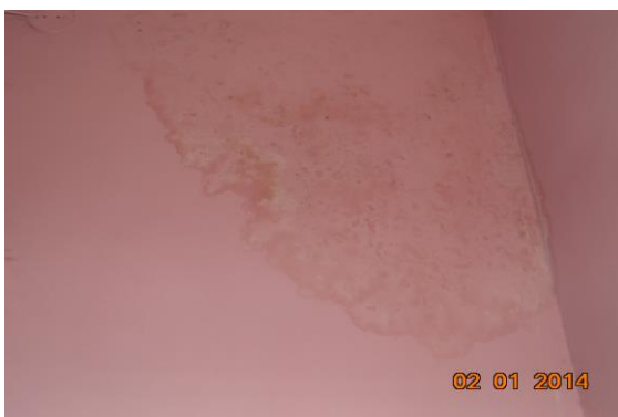
Photo 33 Dampness/Seepage on Wall No. 2 of Store of First Floor
