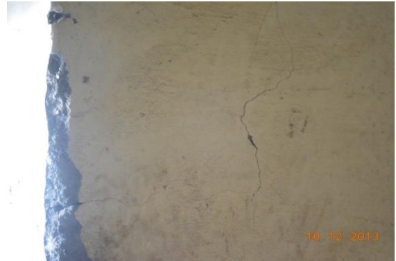
Photo 212 Peeling of Plaster on Wall No. 3 of Part B of Police Kotwali of First Floor
