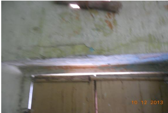
Photo 40 , Horizontal Crack on Wall No. 3 of Room No. 110, First Floor, Approx. Width = 1mm, Approx. Length = 1m. Distance from Wall No. 2 = 0.4m, Height from Floor = 1.9m.
