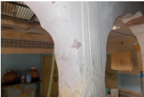
Photo 47 Peeling of Plaster on Wall No. 3 of Varanda of First Floor
