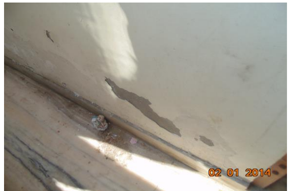
Photo 44 Peeling of Plaster on Wall No. 3 of First Floor
