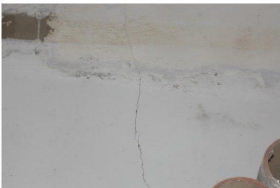
Photo 17 Horizontal Crack on Wall No. 3 of Part A, Shop No. 7, Ground Floor Approx. Width = 0.6mm, Approx. Length = 0.5m. Distance from Wall No. 2 = 2.3m, Height from Floor = 2.3m.
