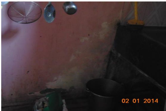
Photo 31 Peeling of Plaster on Wall No. 1 of Kitchen of First Floor
