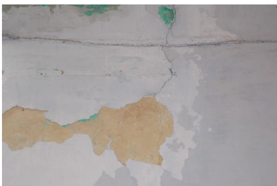
Photo 5 Inclined Crack on Wall No. 2 of Shop No.181, Ground Floor Approx. Width = 2mm, Approx. Length = 4m. Distance from Wall no.3 = 2.5m, Height from Floor = 0.8m.
