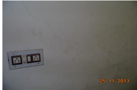
Photo 26 Inclined Crack on Wall No. 1 of Shop No. 16, Ground Floor, Approx. Width = 0.3mm, Approx. Length = 2.3m. Distance from Wall No.4 = 0m, Height from Floor = 0.3m.
