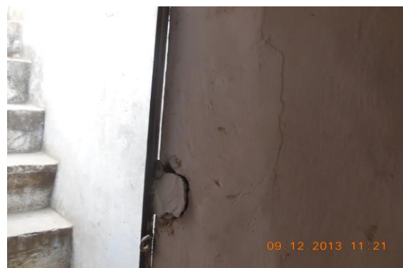
Photo 37 Peeling of Plaster on Wall No. 3 of Lobby of First Floor
