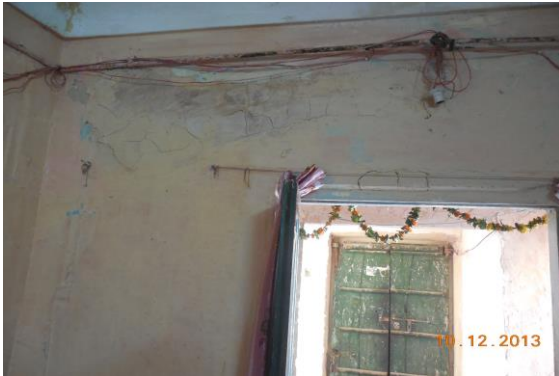
Photo 253 Plaster Crack on Wall No. 3 of Room No. 4 of Second Floor
