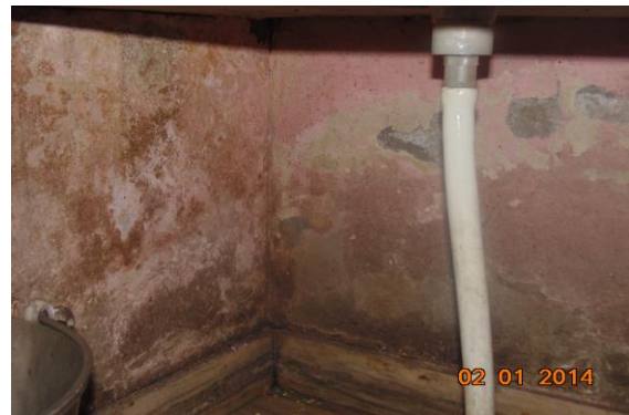
Photo 32 Peeling of Plaster on Wall No. 1 & 4 of Kitchen of First Floor
