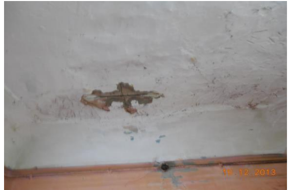
Photo 254 Peeling of Plaster on of Room No. 5 of Second Floor
