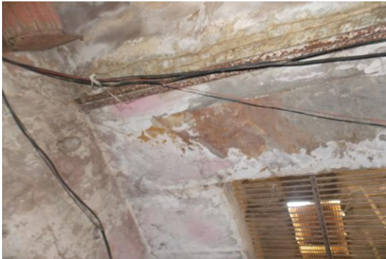
Photo 57 Peeling of Plaster on Roof of House No. 758, First Floor
