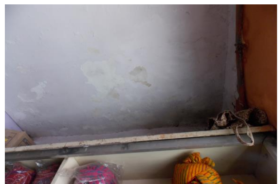
Photo 10 Horizontal Crack on Roof of Varanda of Shop No.791, Ground Floor Approx. Width = 0.1mm, Approx. Length = 2m. Distance from Rightside External Column = 0.5m, Height from Floor = 3m.
