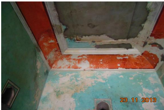
Photo 51 Dampness/Seepage on Wall No. 4 & Roof of Varanda No.3 of First Floor
