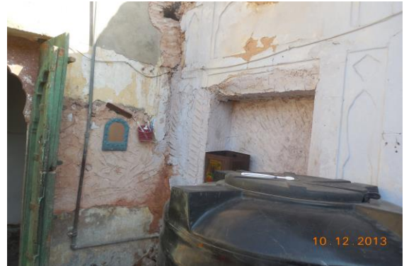
Photo 244 Peeling of Plaster on Wall No. 1 & 3 of Open Sky of Second Floor
