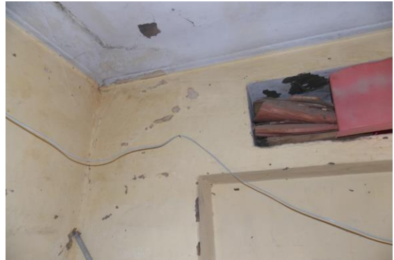
Photo 58 Peeling of Plaster on Wall No. 2 of Varanda of Second Floor
