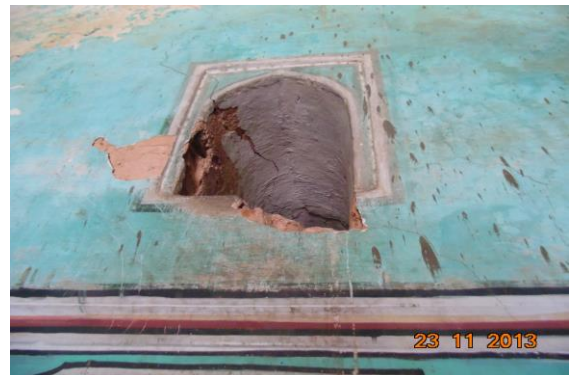
Photo 52 Peeling of Plaster on Wall No. 4 of Varanda No.3 of First Floor
