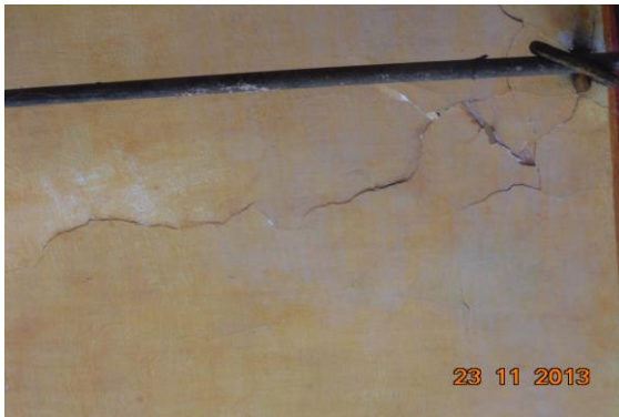
Photo 49 Peeling of Plaster on Roof of Varanda No.1 of Ground Floor
