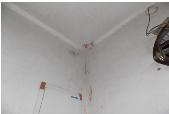
Photo 131 Peeling of Plaster on Wall No. 2 & 3 of Room No. 16(Part A)
