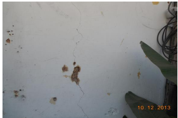
Photo 256 Peeling of Plaster on Wall No. 3 of Open Sky No.3 of Second Floor
