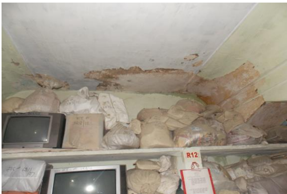
Photo 165 Peeling of Plaster on Roof of Part A of Store
