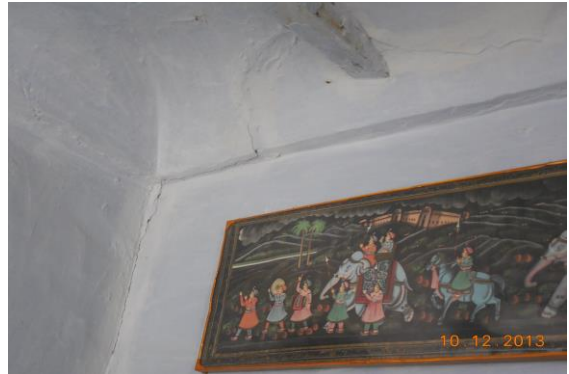
Photo 286 Dampness/Seepage on Wall No. 2, 4 & Roof of Kitchen of Second Floor
