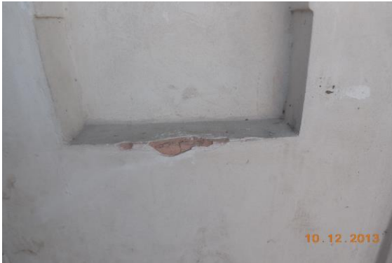
Photo 241 Peeling of Plaster on Wall No. 3 of Open Sky of Second Floor
