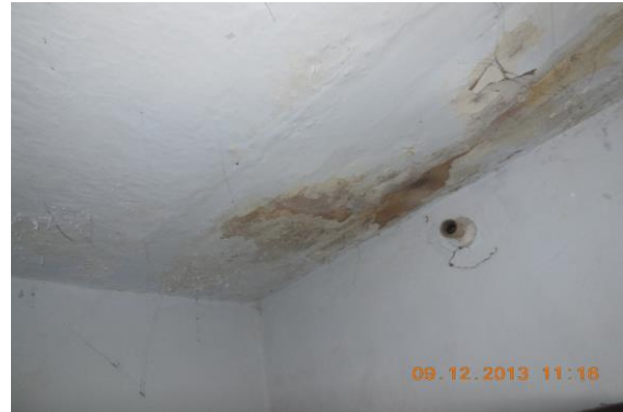
Photo 33 Dampness/Seepage on Roof of Store of First Floor
