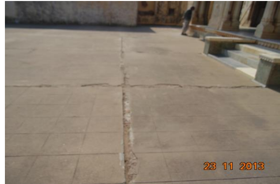
Photo 64 Peeling of Plaster on Floor of Open Area of First Floor
