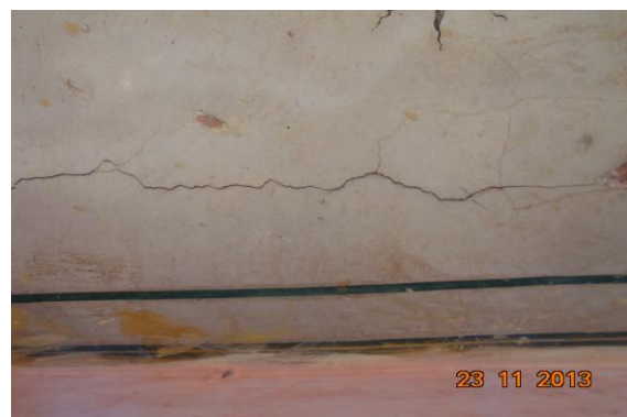
Photo 18 Inclined Crack on Outer wall of Maindoor, Ground Floor Approx. Width = 0.8mm, Approx. Length = 2m. Distance from Wall No.1 = 0m, Height from Floor = 2.25m.
