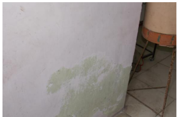
Photo 108 Peeling of Plaster on Wall No. 1 of Passage No.3 of Ground Floor
