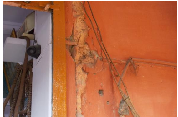
Photo 41 Damaged Portion on Rightside Outer Wall of Shop No.776 of Ground Floor
