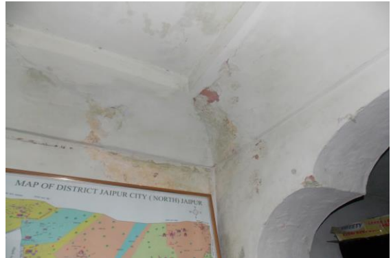
Photo 122 Dampness/Seepage on Wall No. 4 & Roof of Room No. 9 of
