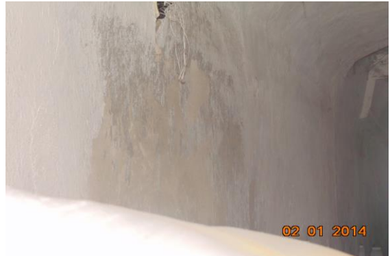
Photo 20 Peeling of Plaster on Wall No. 1 of Shop No. 3 of Ground Floor
