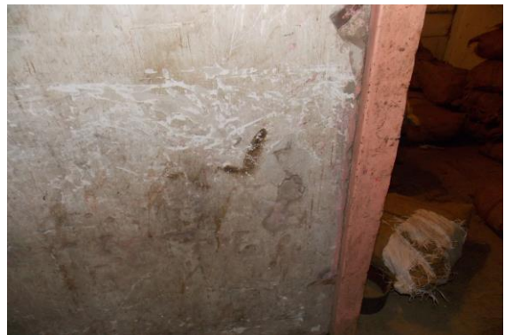
Photo 60 Peeling of Plaster on Wall No. 2 of House No. 758, First Floor
