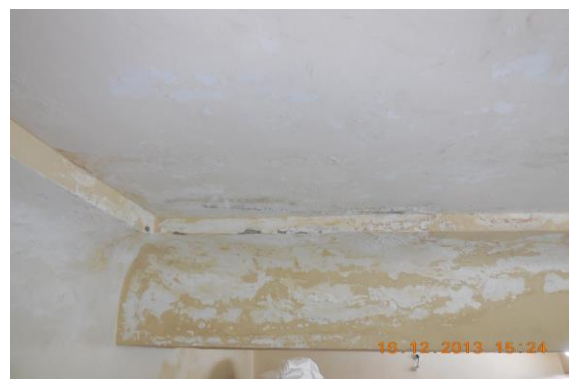
Photo 52 Horizontal Crack on Roof of Varanda of Shop No.767, Ground Floor Approx. Width = 2mm, Approx. Length = 1.5m. Distance from Rightside External Column = Backsidem, Height from Floor = 3m.
