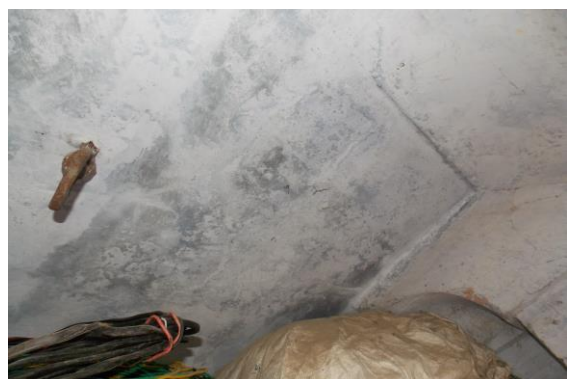
Photo 30 Dampness/Seepage on Roof of Store no.2 of First Floor
