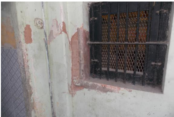
Photo 159 Peeling of Plaster on Wall No. 1 of Open Sky area
