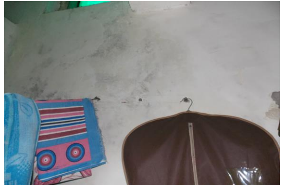
Photo 104 Dampness/Seepage on Wall No. 2 of Room No. 8 of Ground Floor
