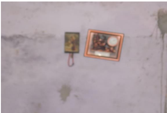
Photo 65 Dampness/Seepage on Wall No. 2 of Room No. 1 of House No. 758, First Floor
