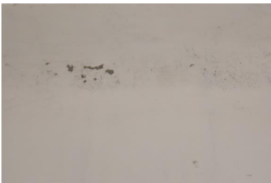
Photo 137 Peeling of Plaster on Wall No. 4 & Roof of Room No. 13
