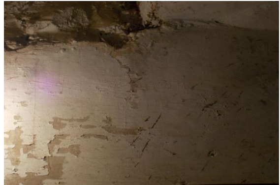
Photo 58 Peeling of Plaster on Wall No. 4 of House No. 758, First Floor
