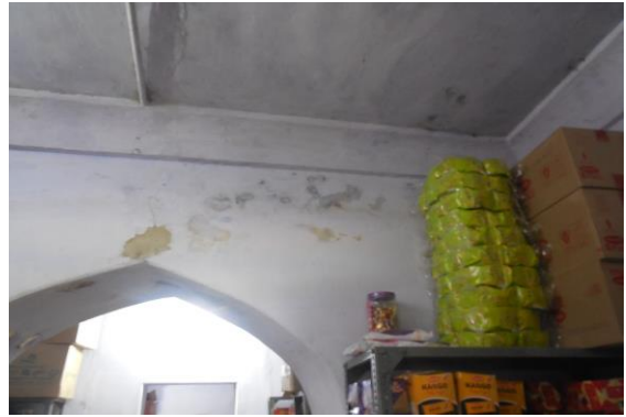
Photo 146 Dampness/Seepage on Wall No. 4 of Room No. 3 of Ground Floor
