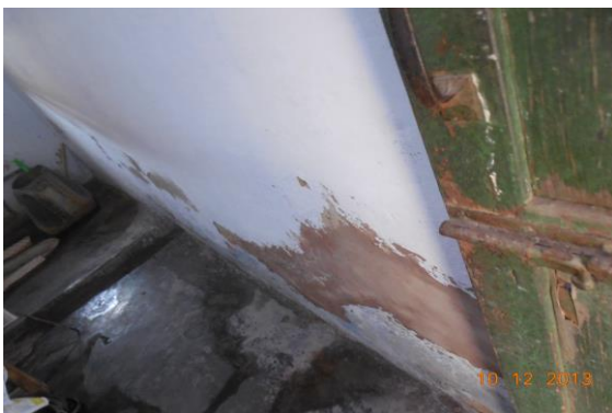
Photo 281 Dampness/Seepage on Wall No. 1 of Bathroom of Second Floor
