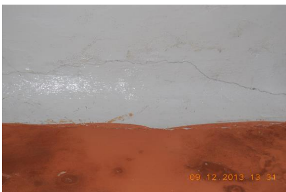
Photo 23 Horizontal Crack on Roof of Varanda, Shop No.21, Ground Floor Approx. Width = 0.4mm, Approx. Length = 1.5m. Distance from Left External Column = 0m, Height from Floor = 3m.
