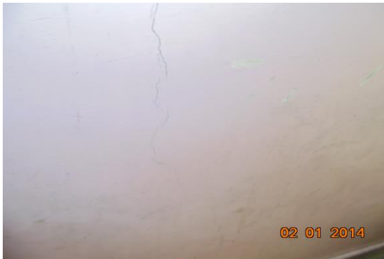
Photo 11 Inclined Crack on Wall No. 4 of , First Floor Approx. Width = 1mm, Approx. Length = 2m.
