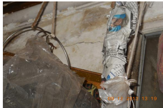
Photo 22 Horizontal Crack on of Part A, Shop no.15, Ground Floor Approx. Width = 1.5mm, Approx. Length = 0.5m. Distance from Wall No.1 = 0.15m, Height from Floor = 2.3m.
