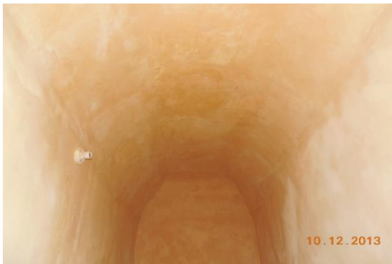
Photo 225 Dampness/Seepage on Wall No. 1 & Roof of Hall No. 1(Part C) of First Floor
