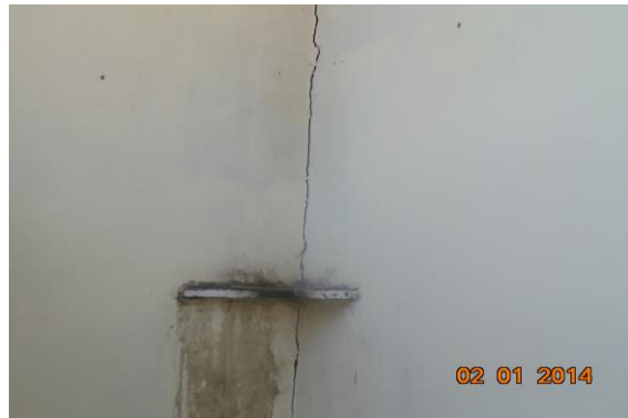
Photo 12 Vertical Crack on Wall No. 2 & 3 of Balcony, Second Floor Approx. Width = 2.5mm, Approx. Length = 2m.
