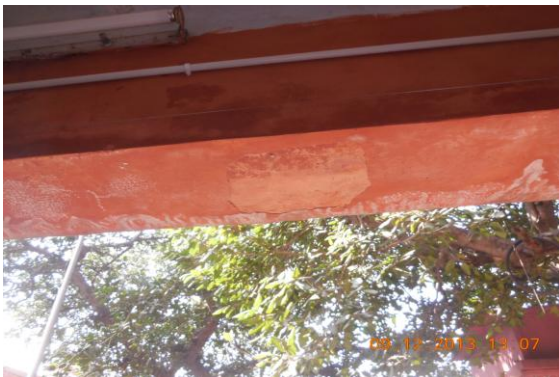
Photo 27 Dampness/Seepage on External Beam of Varanda of Shop No.8 of Ground Floor
