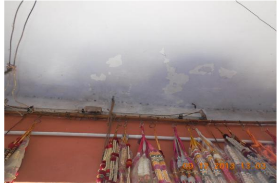
Photo 26 Peeling of Plaster on Roof of Varanda of Shop No.7 of Ground Floor
