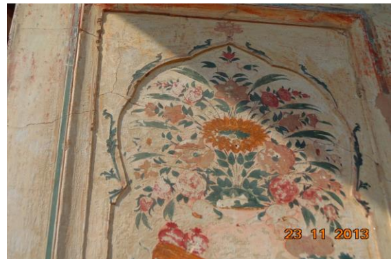
Photo 46 Peeling of Plaster on Column of Varanda No.1 of Ground Floor
