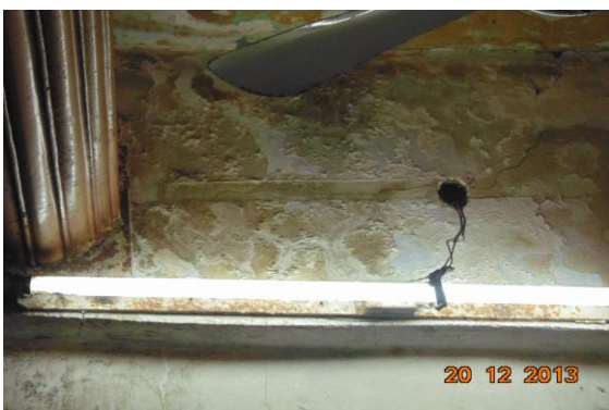
Photo 86 Dampness/Seepage on Wall No. 4 of Shop No.172 of Ground Floor
