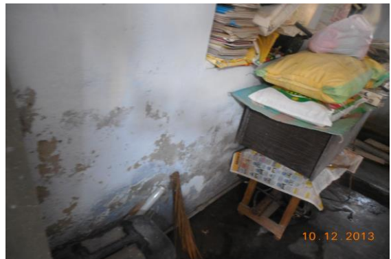
Photo 280 Dampness/Seepage on Wall No. 2 of Toilet No. 2 of Second Floor
