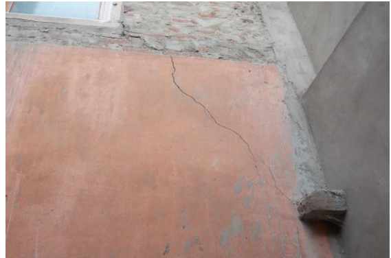
Photo 4 Inclined Crack on Wall No. 6 of Hall No. 2, First Floor Approx. Width = 3mm, Approx. Length = 2m. Distance from Wall No.4 = 0.15m, Height from Floor = 2.1m.
