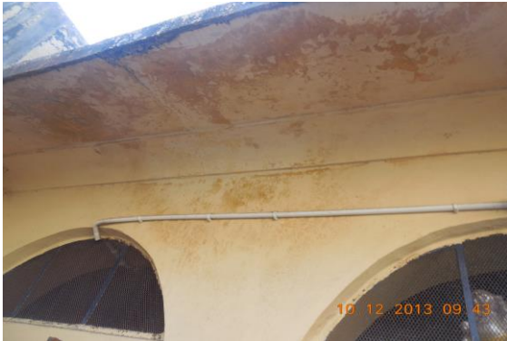
Photo 100 Dampness/Seepage on Roof Shade of Open Varanda of College & Temple, First Floor
