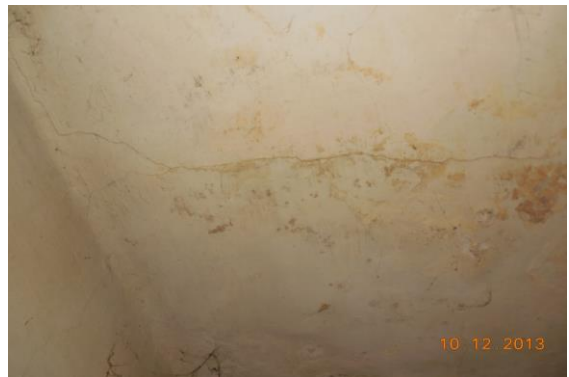
Photo 268 Peeling of Plaster on Roof of Bathroom of Second Floor
