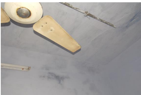
Photo 23 Dampness/Seepage on Wall No. 4 & Roof of Room No. 5 of First Floor
