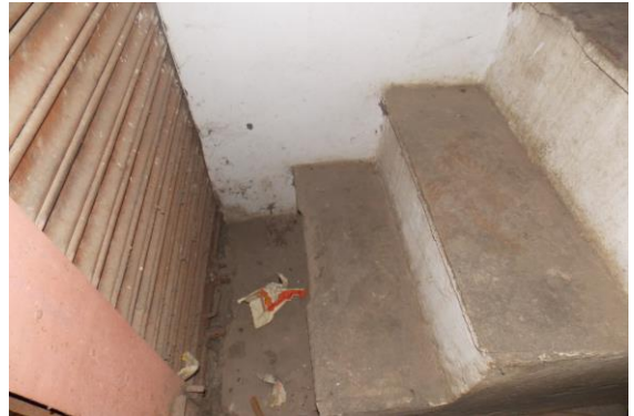
Photo 72 Damaged Portion of Stair Step GF to FF of
