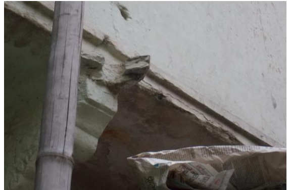
Photo 158 Damaged Portion on Roof of Open Sky area
