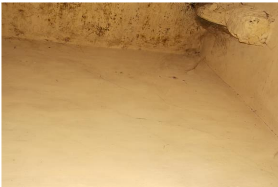
Photo 111 Peeling of Plaster on Wall No. 3 of Toilet No. 1(Part B) of Ground Floor
