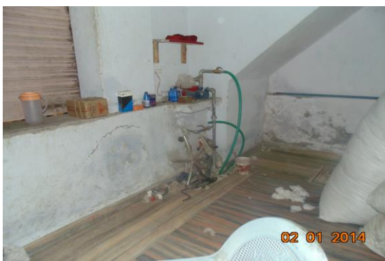
Photo 15 Dampness/Seepage on Wall No. 1 & 4 of Shop No. 1 of Ground Floor
