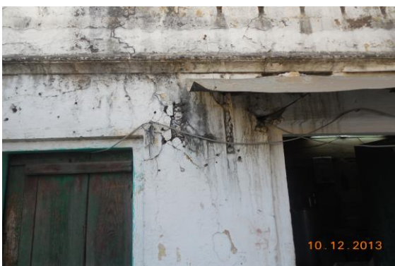
Photo 257 Peeling of Plaster on Wall No. 2 of Open Sky No.3 of Second Floor
