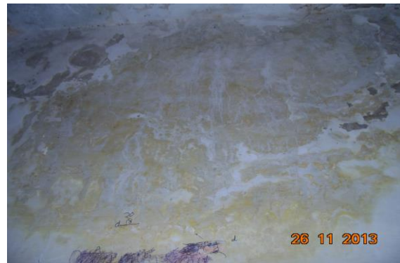
Photo 43 Dampness/Seepage on Passage 3 of Shop No. 221 of Ground Floor
