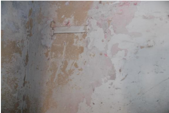
Photo 63 Peeling of Plaster on Wall No. 1 of House No. 758, First Floor
