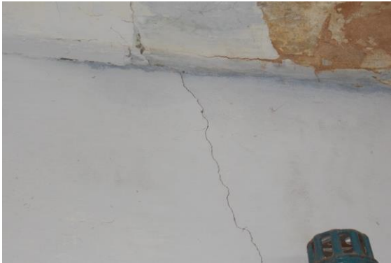
Photo 15 Inclined Crack on Wall No. 4 of Part A, Shop No. 7, Ground Floor Approx. Width = 0.6mm, Approx. Length = 0.6m. Distance from Wall No. 2 = 0.9m, Height from Floor = 2.2m.
