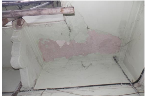
Photo 154 Damaged Portion on Roof of Open Sky area
