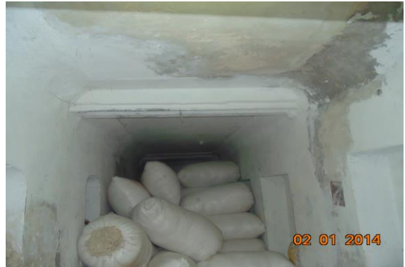
Photo 18 Dampness/Seepage on Wall No. 1&2&Roof, Shop No. 3 of Ground Floor
