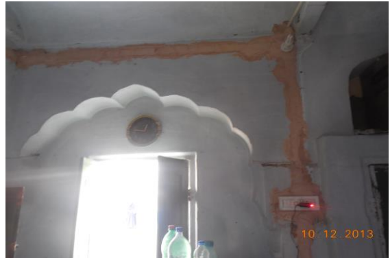
Photo 284 Peeling of Plaster on Roof of Room No. 14 of Second Floor
