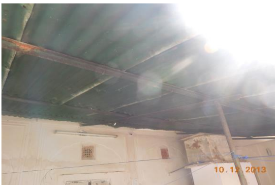
Photo 287 Dampness/Seepage on Roof of Balcony of Second Floor
