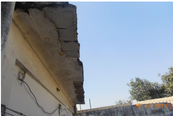
Photo 255 Damaged Portion on Wall No. 3 & Shade of Open Sky No.3 of Second Floor
