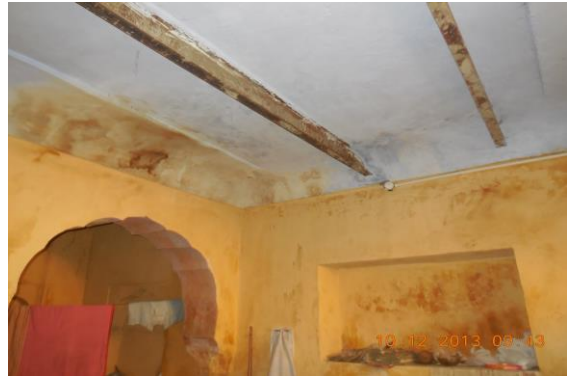
Photo 101 Dampness/Seepage on Wall No. 2 & 4 of Room No. 3 (Part-I) of First Floor
