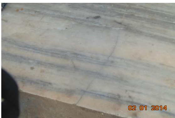
Photo 5 Inclined Crack on of Main Entry, Shop No. 1, Ground Floor, Approx. Width = 0.2mm, Approx. Length = 2m.
