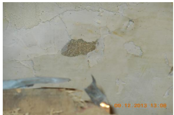
Photo 30 Peeling of Plaster on Roof of Shop No.8 of Ground Floor
