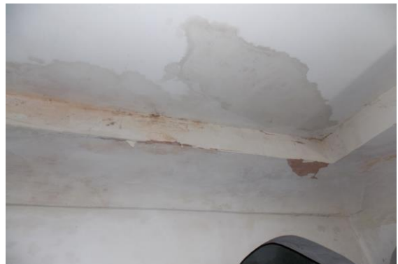
Photo 172 Peeling of Plaster on Roof of Store No.2
