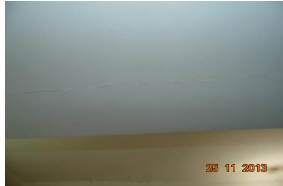
Photo 27 Horizontal Crack on of Shop No. 16, Ground Floor, Approx. Width = 0.3mm, Approx. Length = 3m. Distance from Wall No.4 = 0m, Height from Floor = 2m.
