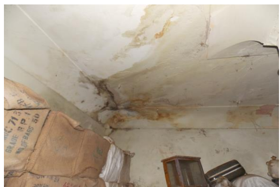
Photo 174 Dampness/Seepage on Roof of Store No.2
