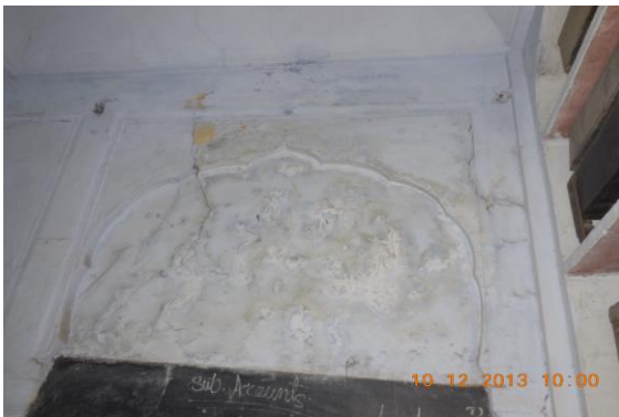
Photo 108 Dampness/Seepage on Wall No. 1 of Hall No. 1 (Part-II) of First Floor
