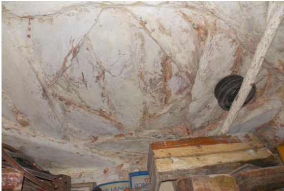
Photo 40 Peeling of Plaster on Roof of Part B of Shop No.777 of Ground Floor
