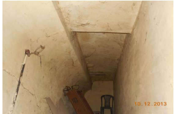
Photo 208 Damaged Portion on Roof of Store of First Floor
