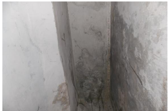
Photo 88 Dampness/Seepage on Roof of Passage No.1 of Ground Floor
