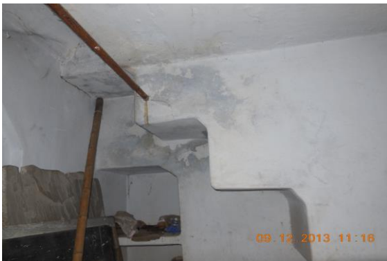
Photo 34 Dampness/Seepage on Wall No. 4 of Store of First Floor
