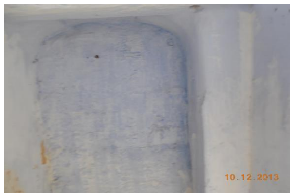
Photo 282 Peeling of Plaster on Roof of Room No. 15 of Second Floor
