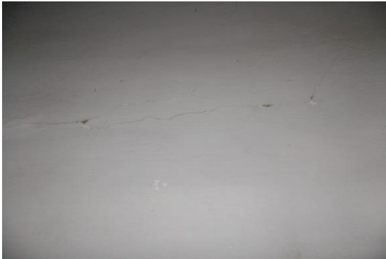
Photo 45 Peeling of Plaster on Wall No. 1 of Lobby of First Floor
