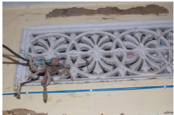
Photo 60 Peeling of Plaster on Wall No. 1 of Varanda of Second Floor
