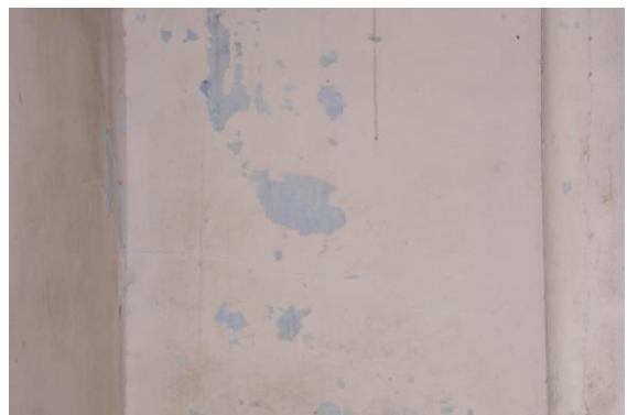
Photo 62 Peeling of Plaster on Wall No. 4 of Toilet No. 2 of Second Floor
