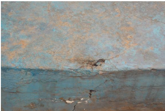
Photo 9 Peeling of Plaster on Wall No. 1 & Floor of Boundary Wall B of Ground Floor
