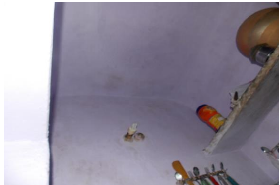
Photo 22 Dampness/Seepage on Wall No. 2 & Roof of Kitchen No.2 of First Floor
