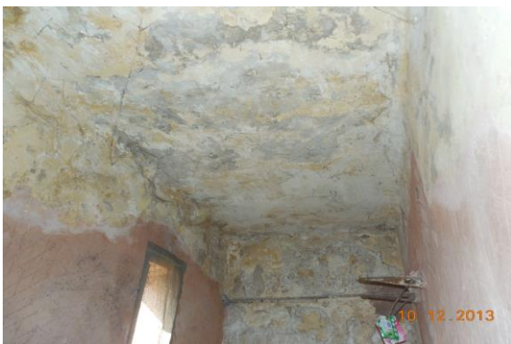
Photo 269 Dampness/Seepage on Wall No. 3, 4, Roof & 2 of Toilet No. 1 of Second Floor
