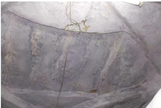
Photo 42 Dampness/Seepage on Roof of Part B of Shop No.776 of Ground Floor
