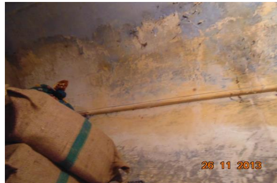
Photo 41 Peeling of Plaster on Wall No. 3 of Shop No. 47 of Ground Floor
