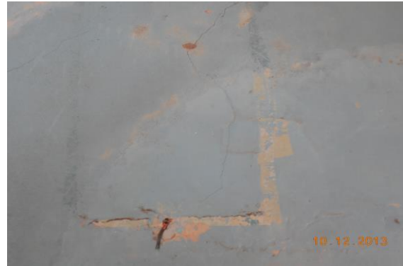
Photo 230 Plaster Crack on Wall No. 4 of S.D. Anubhag Room of First Floor
