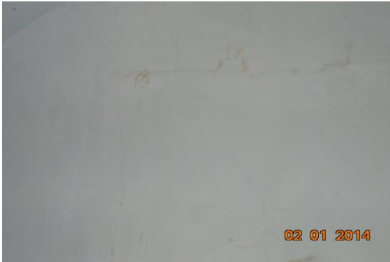
Photo 17 Plaster Crack on Wall No. 4 of Shop No. 1 of Ground Floor
