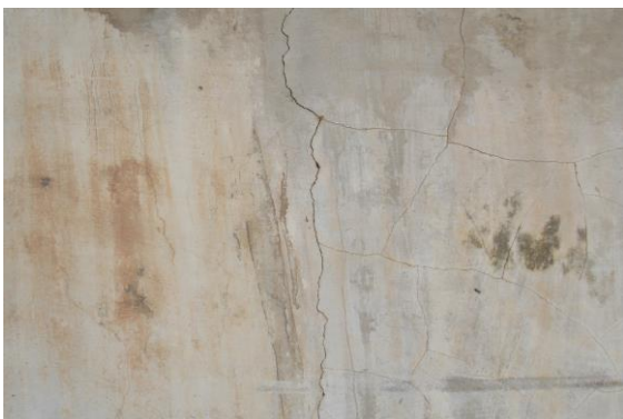
Photo 5 Inclined Crack on Wall No. 2 of Open Sky No.1, First Floor Approx. Width = 4mm, Approx. Length = 4m. Distance from Wall No.4 = 1.8m, Height from Floor = 0m.
