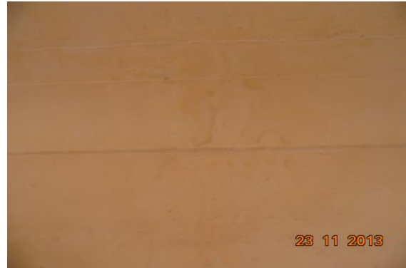
Photo 62 Dampness/Seepage on Wall No. 1 & Roof of Passage of First Floor
