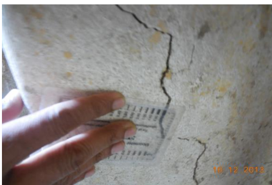
Photo 42A Inclined Crack on Wall No. 4 of Passage No. 1, First Floor, Approx. Width = 2.5mm, Approx. Length = 1.4m. Distance from Wall No. 2 = 0.1m, Height from Floor = 0m.
