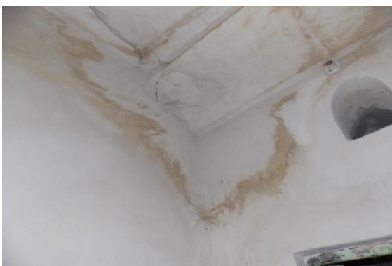
Photo 125 Dampness/Seepage on Wall No. 1, 4 & Roof of Room No. 3(Lobby) of
