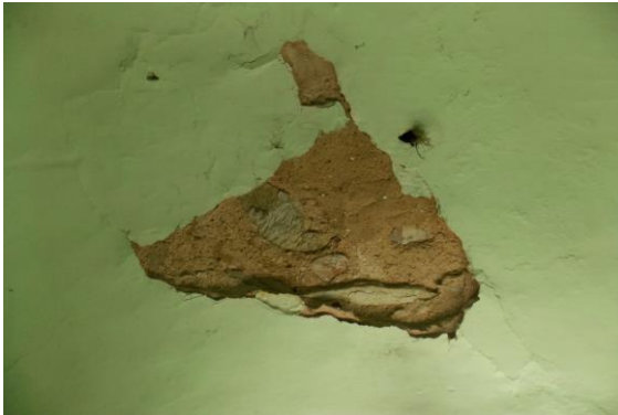
Photo 139 Peeling of Plaster on Roof of Room No. 13
