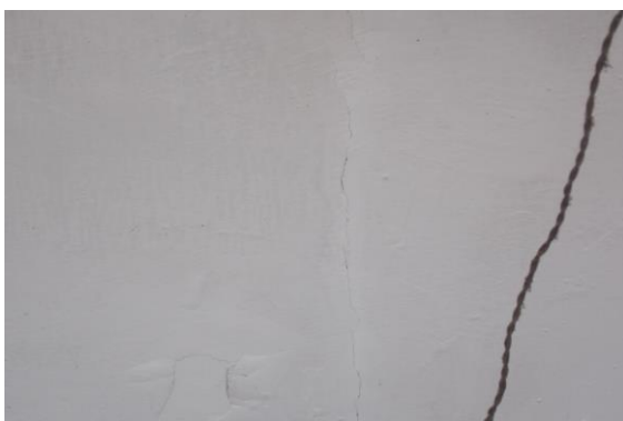
Photo 11 Horizontal Crack on Roof of Varanda of Shop No.791, Ground Floor Approx. Width = 0.1mm, Approx. Length = 1.2m. Distance from Leftside External Column = 1.4m, Height from Floor = 3m.
