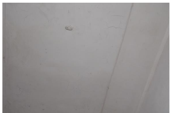
Photo 126 Peeling of Plaster on Roof of Pantry of
