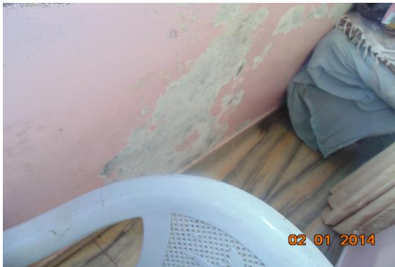
Photo 41 Peeling of Plaster on Wall No. 4 of First Floor
