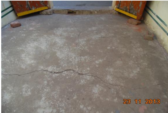
Photo 61 Peeling of Plaster on Floor of Passage of First Floor
