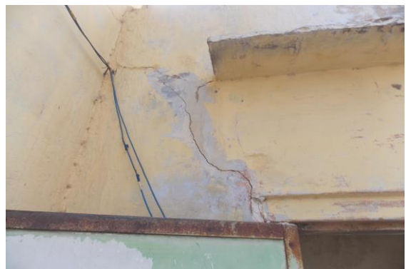
Photo 80 Peeling of Plaster on Wall No. 1 of Parapet of Terrace
