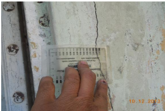
Photo 41A Inclined Crack on Wall No. 1 of Room No. 110, First Floor, Approx. Width = 2mm, Approx. Length = 4m. Distance from Wall No. 4 = 4.5m, Height from Floor = 0m.
