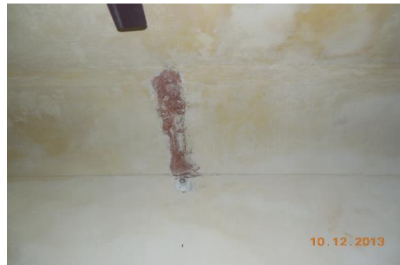
Photo 226 Peeling of Plaster on Roof of Hall No. 1(Part B) of First Floor
