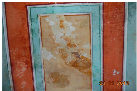
Photo 54 Peeling of Plaster on Roof of Varanda No.4 of First Floor
