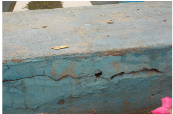
Photo 10 Plaster Crack on Boundary Wall B of Ground Floor
