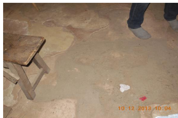
Photo 111 Peeling of Plaster on Floor of Hall No. 1 (Part-II) of First Floor
