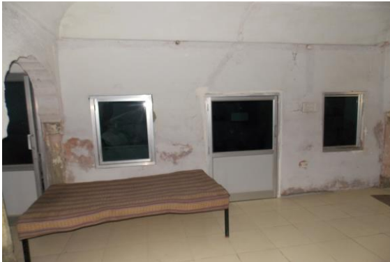
Photo 169 Dampness/Seepage on Wall No. 2 of Hall No. 1
