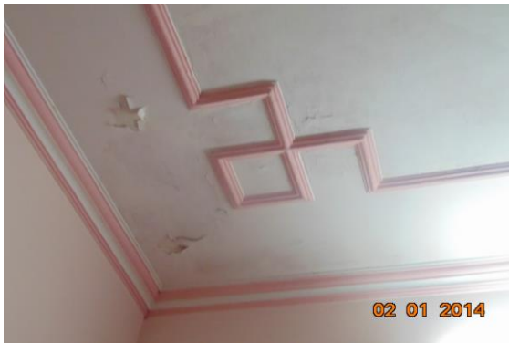
Photo 29 Peeling of Plaster of Varandah Roof of First Floor
