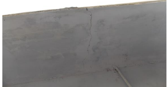
Photo 5 Horizontal Crack on Wall No. 2 of Shade Roof, First Floor Approx. Width = 2mm, Approx. Length = 1m. Distance from Wall No.4 = 1.7m, Height from Floor = 3m.
