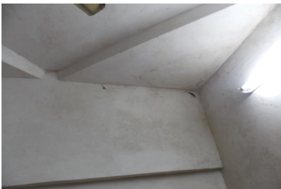
Photo 113 Peeling of Plaster on Wall No. 4 of Room No. 10 of Ground Floor
