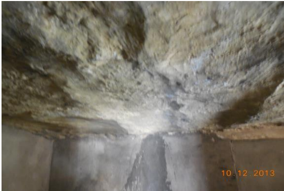
Photo 277 Dampness/Seepage on Roof of Bathroom of Second Floor
