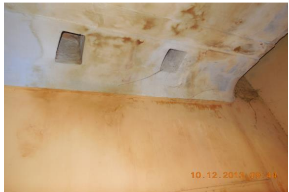
Photo 103 Dampness/Seepage on Wall No. 4 of Room No. 3 (Part-II) of First Floor
