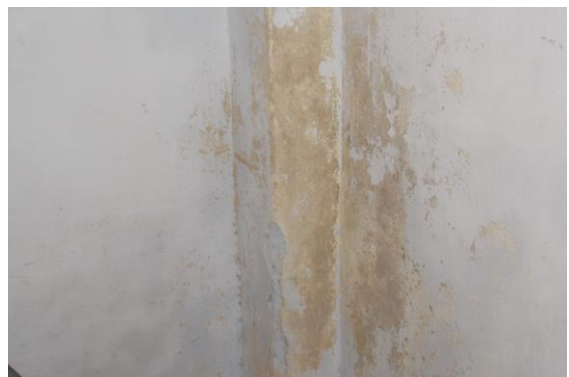
Photo 68 Peeling of Plaster on Wall No. 2 & 3 of Room No. 12 of House No. 758, First Floor
