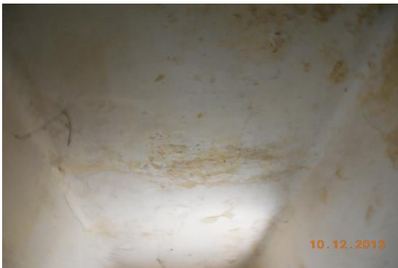
Photo 267 Dampness/Seepage on Roof of Bathroom of Second Floor
