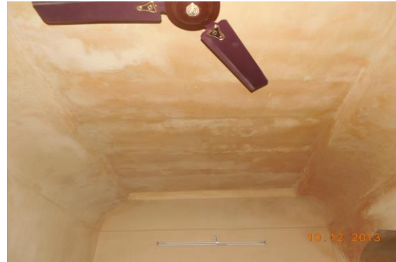
Photo 224 Dampness/Seepage on Roof of Hall No. 1(Part B) of First Floor
