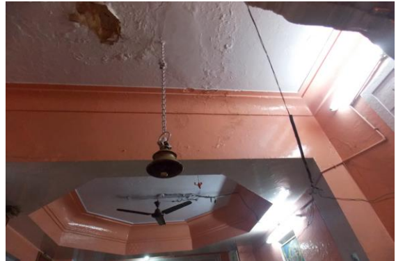
Photo 4 Peeling of Plaster on Roof of Shri Rojgareshwar Mandir of Ground Floor
