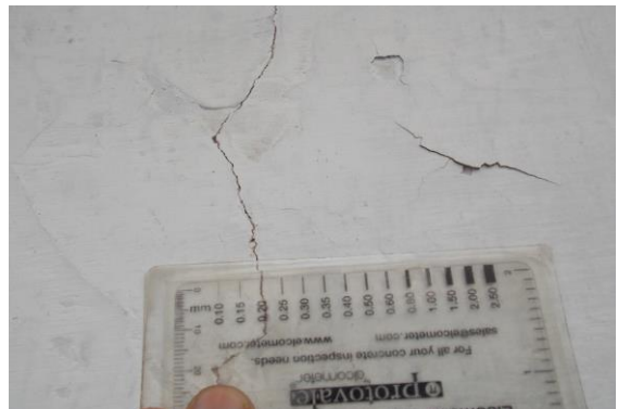
Photo 3A Inclined Crack on Wall No. 3 of Open Sky No.1, First Floor Approx. Width = 0.2mm, Approx. Length = 1.2m. Distance from Wall No.2 = 1.7m, Height from Floor = 2m.
