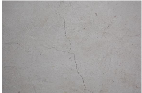
Photo 36 Plaster Crack on Wall No. 2 of Shop No. 5 of Ground Floor
