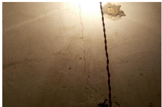
Photo 18 Inclined Crack on Wall No. 1 of Shop No. 5, Ground Floor Approx. Width = 0.6mm, Approx. Length = 0.7m. Distance from Wall No. 3 = 0.3m, Height from Floor = 1.5m.
