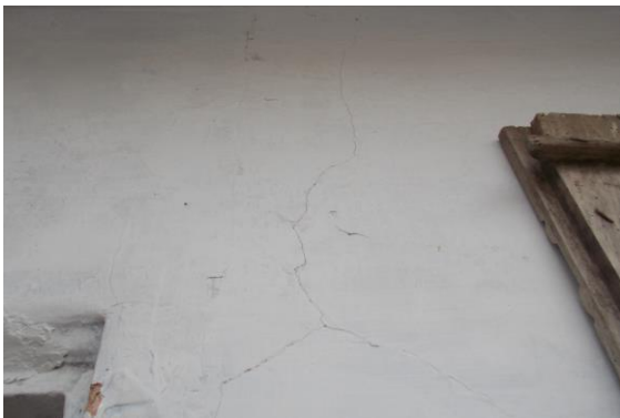
Photo 3 Inclined Crack on Wall No. 3 of Open Sky No.1, First Floor Approx. Width = 0.2mm, Approx. Length = 1.2m. Distance from Wall No.2 = 1.7m, Height from Floor = 2m.
