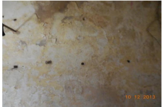
Photo 266 Dampness/Seepage on Wall No. 4 of Bathroom of Second Floor
