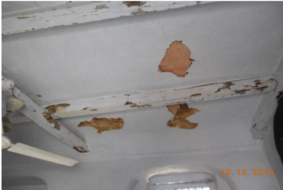
Photo 283 Peeling of Plaster on Wall No. 3 of Room No. 15 of Second Floor
