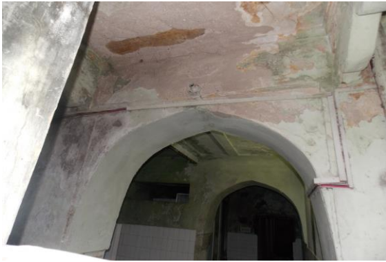
Photo 151 Peeling of Plaster on Wall No. 4 of Open Sky area
