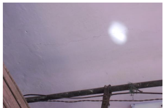
Photo 17 Horizontal Crack on Roof of Varanda of Shop No. 777, Ground Floor Approx. Width = 0.2mm, Approx. Length = 2m. Distance from Leftside External Column = 1.2m, Height from Floor = 3m.
