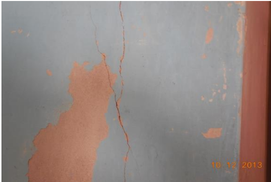
Photo 229 Plaster Crack on Wall No. 2 of S.D. Anubhag Room of First Floor
