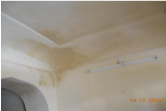
Photo 223 Dampness/Seepage on Roof of Hall No. 1(Part B) of First Floor
