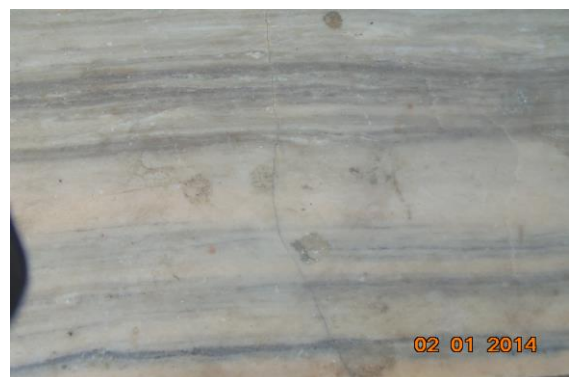
Photo 5A Inclined Crack on of Main Entry, Shop No. 1, Ground Floor, Approx. Width = 0.2mm, Approx. Length = 2m.
