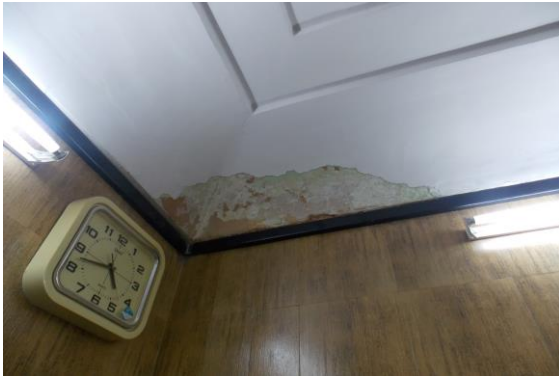
Photo 127 Peeling of Plaster on Wall No. 2, 4 & Roof of Room No. 1 (office) of
