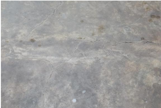
Photo 19 Peeling of Plaster on Floor of Open sky No.2 of First Floor
