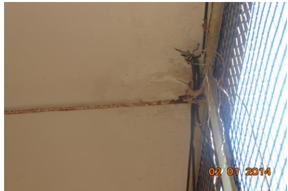
Photo 42 Dampness/Seepage on Roof of Balcony 2 of First Floor
