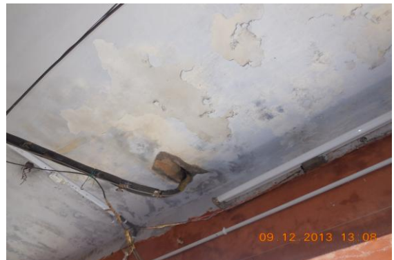
Photo 28 Dampness/Seepage on Roof of Varanda of Shop No.8 of Ground Floor
