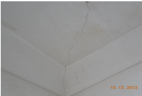
Photo 231 Plaster Crack on Wall No. 3 of Open Sky No.3 Shaft of First Floor
