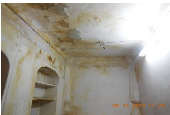
Photo 36 Dampness/Seepage on All Walls & Roof of Room No. 4 of Lohia Institute, First Floor
