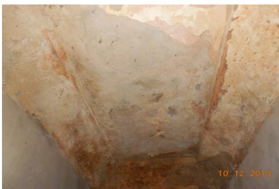
Photo 227 Dampness/Seepage on Roof of Room Dark Room of First Floor
