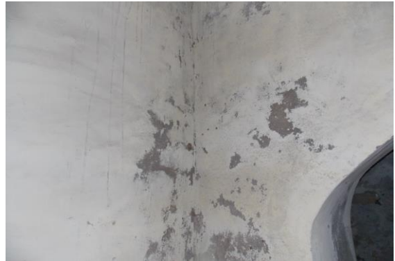
Photo 86 Dampness/Seepage on Wall No. 2 & 3 of Varanda No.1 of Ground Floor
