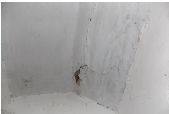
Photo 107 Peeling of Plaster on Roof of Passage No.3 of Ground Floor
