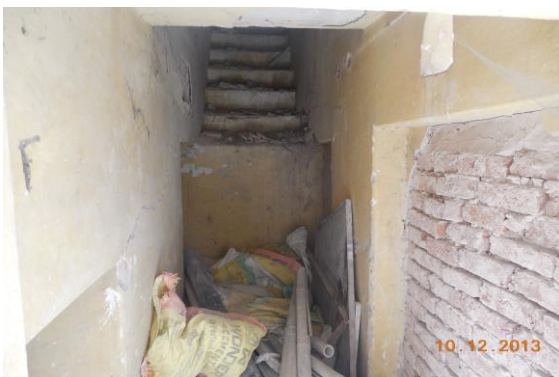
Photo 233 Damaged Portion of Staircase Near Open Sky No.3 of First Floor
