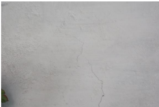
Photo 13 Inclined Crack on Wall No. 1 of Room No. 1, Second Floor Approx. Width = 0.5mm, Approx. Length = 2m.
