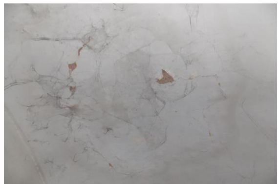
Photo 132 Peeling of Plaster on Roof of Room No. 15(PartA)
