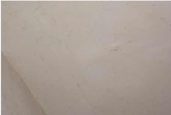
Photo 33 Plaster Crack on Roof of Shop No. 8 of Ground Floor
