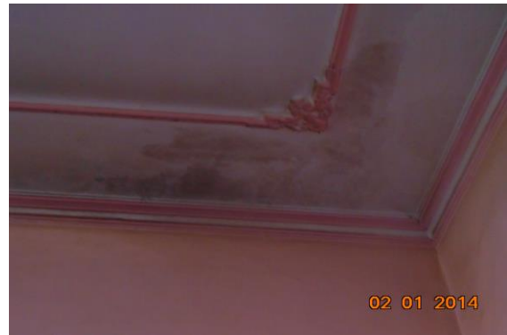
Photo 30 Dampness/Seepage on Roof of Kitchen of First Floor
