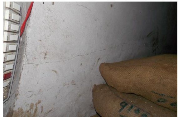
Photo 16 Horizontal Crack on Wall No. 1 of Part A of Shop No. 782, Ground Floor Approx. Width = 0.5mm, Approx. Length = 2.7m. Distance from Wall No. 3 = 0m, Height from Floor = 1.5m.
