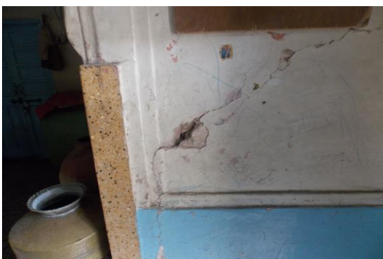
Photo 49 Peeling of Plaster on Wall No. 2 & Roof of Open Sky No.2 of First Floor
