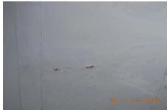
Photo 109 Peeling of Plaster on Roof of Hall No. 1 (Part-II) of First Floor
