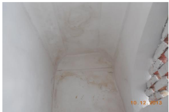
Photo 270 Dampness/Seepage on Roof & 4 of Bathroom No. of Second Floor
