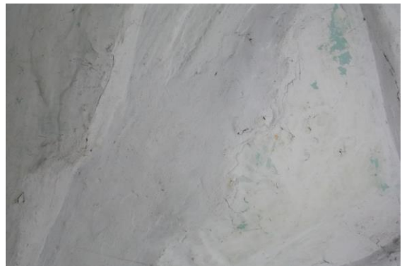
Photo 106 Dampness/Seepage on Roof of Passage No.3 of Ground Floor
