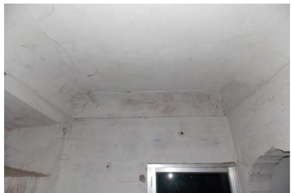
Photo 168 Dampness/Seepage on Roof of Hall No. 1
