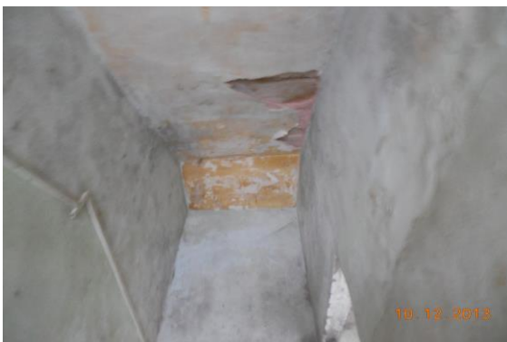
Photo 179 Peeling of Plaster on Roof of Part B Staircase Ground Floor To First Floor of Ground Floor
