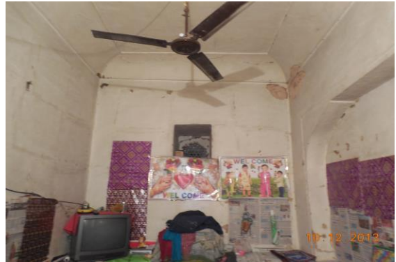
Photo 206 Peeling of Plaster on Wall No. 2 & 4 of Room of First Floor
