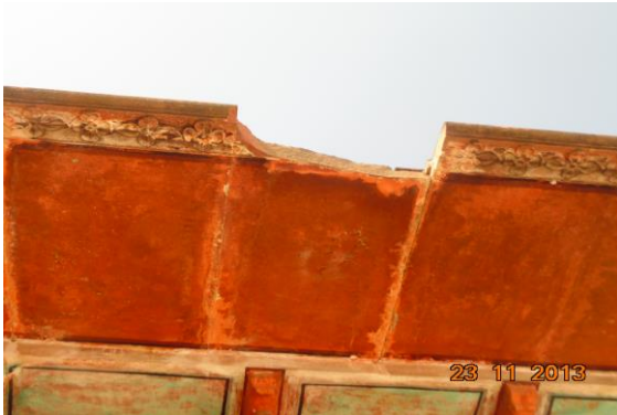
Photo 43 Peeling of Plaster on External wall of Temple of Ground Floor
