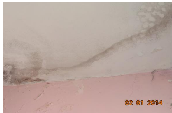
Photo 38 Dampness/Seepage on Roof of First Floor
