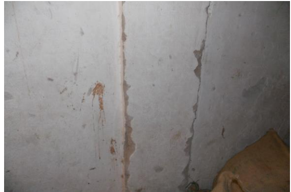
Photo 34 Peeling of Plaster on Wall No. 1 of Shop No. 5 of Ground Floor
