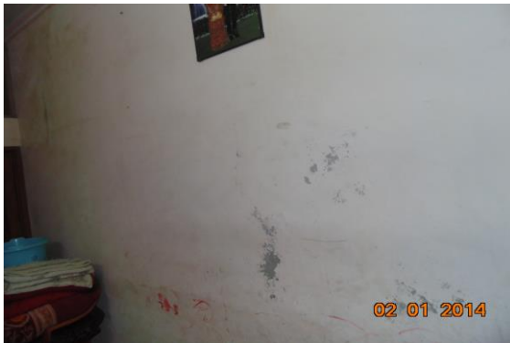
Photo 35 Dampness/Seepage on Wall No. 2 of Room No. 1 of First Floor
