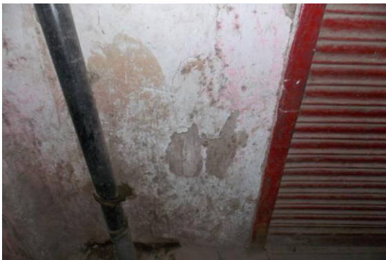
Photo 59 Peeling of Plaster on Wall No. 1 of House No. 758, First Floor
