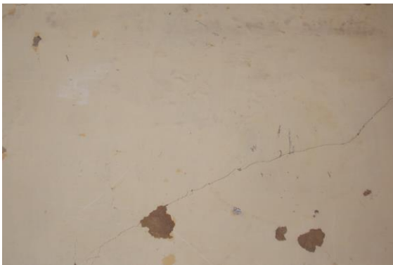
Photo 59 Peeling of Plaster on Wall No. 4 of Varanda of Second Floor
