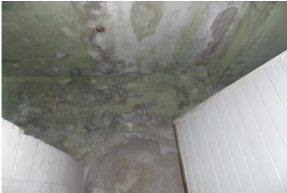
Photo 163 Dampness/Seepage on Wall No. 4 & Roof of Toilet No. 2+3+4
