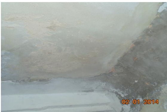
Photo 21 Peeling of Plaster on Roof of Shop No. 3 of Ground Floor
