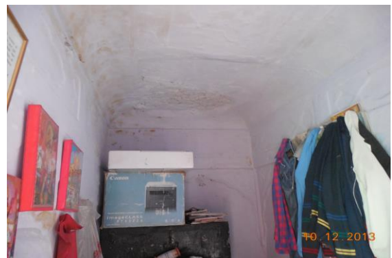
Photo 246 Dampness/Seepage on Wall No. 1 & Roof of Room of Second Floor
