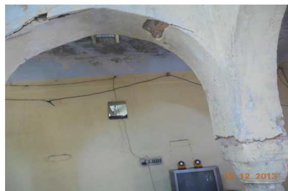
Photo 204 Damaged Portion on Roof & Column of Room Mess Room of First Floor
