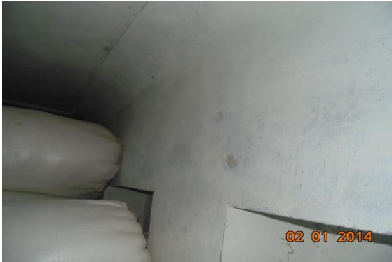
Photo 19 Dampness/Seepage on Wall No. 2 of Shop No. 3 of Ground Floor
