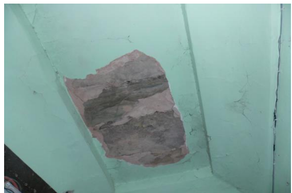
Photo 138 Peeling of Plaster on Roof of Room No. 13
