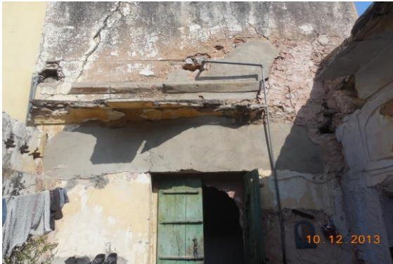
Photo 243 Damaged Portion on Wall No. 1, 3 & Shade of Open Sky of Second Floor
