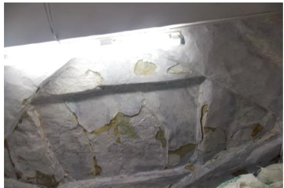
Photo 43 Dampness/Seepage on Roof of Part C of Shop No.776 of Ground Floor
