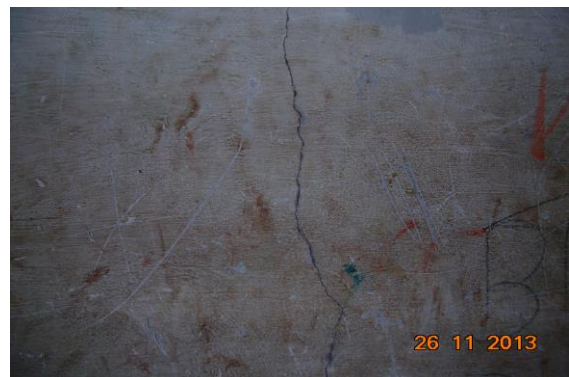
Photo 29 Vertical Crack on of Passage 3 of Shop No. 221, Ground Floor, Approx. Width = 0.8mm, Approx. Length = 2m. Distance from Wall No. 4 = 3.5m, Height from Floor = 2m.
