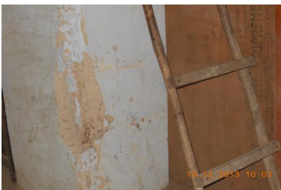
Photo 110 Peeling of Plaster on Wall No. 3 of Hall No. 1 (Part-II) of First Floor
