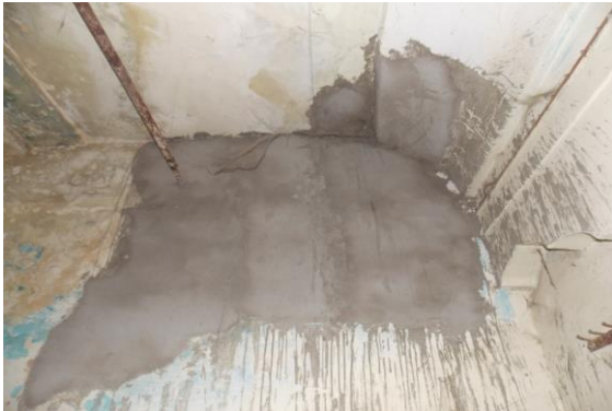
Photo 135 Peeling of Plaster on Wall No. 2 & Roof of Room No. 16(Part B)
