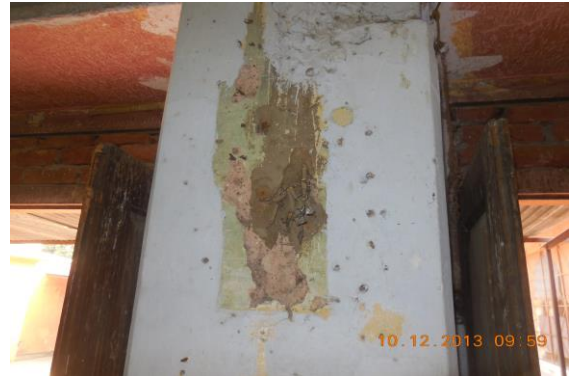
Photo 107 Peeling of Plaster on Wall No. 3 of Hall No. 1(Part-I) of First Floor
