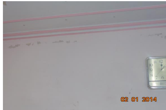
Photo 36 Peeling of Plaster on Wall No. 3 of Hall No. 1 of First Floor
