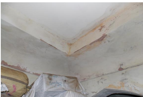
Photo 173 Peeling of Plaster on Roof of Store No.2
