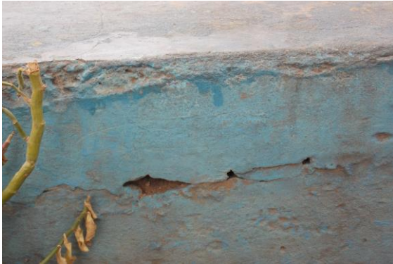
Photo 7 Peeling of Plaster on Boundary Wall B of Ground Floor
