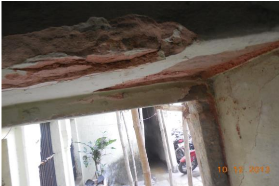
Photo 177 Peeling of Plaster on Roof of Part B Staircase Ground Floor To First Floor of Ground Floor
