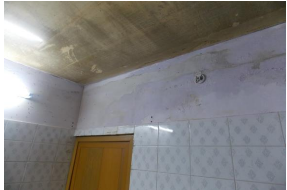
Photo 128 Dampness/Seepage on Wall No. 2 of Room No. 1
