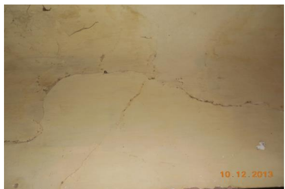
Photo 210 Plaster Crack on Wall No. 4 of Kitchen of First Floor
