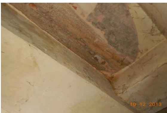
Photo 209 Damaged Portion on Roof of Store of First Floor
