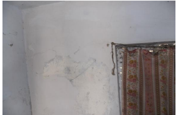
Photo 74 Peeling of Plaster on Wall No. 2 of Toilet No. 1 of First Floor
