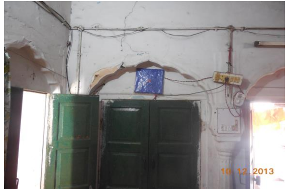
Photo 278 Peeling of Plaster on Wall No. 1 of Room No. 12 of Second Floor
