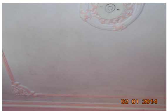
Photo 46 Peeling of Plaster on Roof of Hall No. 2 of Second Floor
