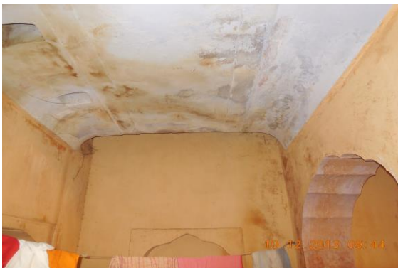
Photo 102 Dampness/Seepage on Wall No. 2, 3 & Roof of Room No. 3 (Part-II) of First Floor
