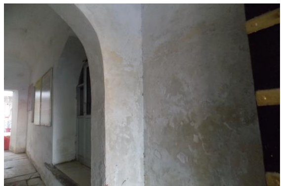
Photo 90 Dampness/Seepage on Wall No. 2 & 4 of Gate No.4 of Ground Floor
