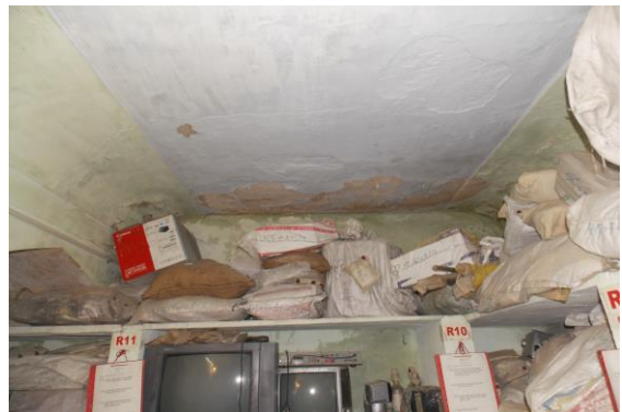
Photo 166 Peeling of Plaster on Roof of Part B of Store
