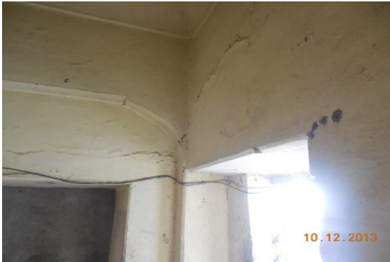
Photo 205 Peeling of Plaster of Kitchen of First Floor
