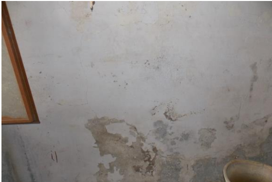
Photo 73 Peeling of Plaster on Wall No. 4 of Toilet No. 1 of First Floor
