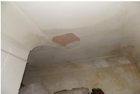
Photo 171 Peeling of Plaster on Roof of Store No.2
