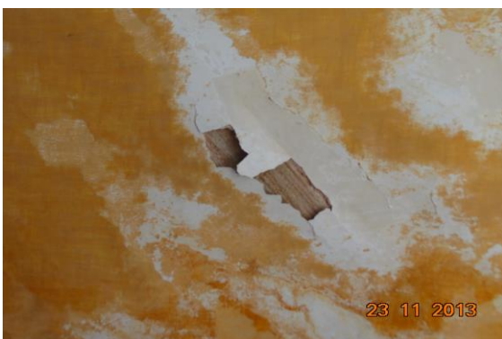
Photo 47 Peeling of Plaster on Roof of Varanda No.1 of Ground Floor
