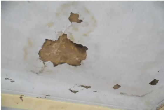
Photo 57 Peeling of Plaster on Roof of Varanda of Second Floor
