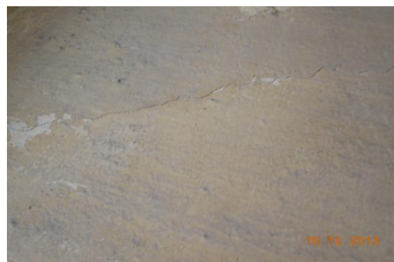
Photo 43 Inclined Crack on Wall No. 2 of Passage No. 1, First Floor, Approx. Width = 0.6mm, Approx. Length = 1m. Distance from Wall No. 4 = 0m, Height from Floor = 1.3m.
