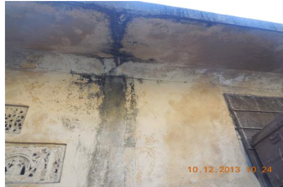
Photo 119 Dampness/Seepage on Wall No. 1 of Open Area 3 of College & Temple, First Floor
