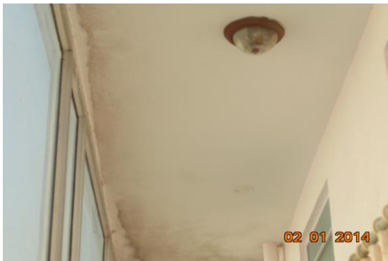
Photo 37 Dampness/Seepage on Roof of First Floor
