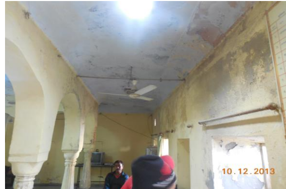
Photo 200 Dampness/Seepage on Roof of Room Mess Room of First Floor
