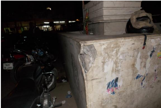
Photo 3 Damaged Portion on Backside Perapet Wall No.1 of Shiv Ji Ka Temple of Ground Floor
