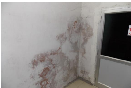
Photo 167 Dampness/Seepage on Wall No. 1 & 3 of Hall No. 1
