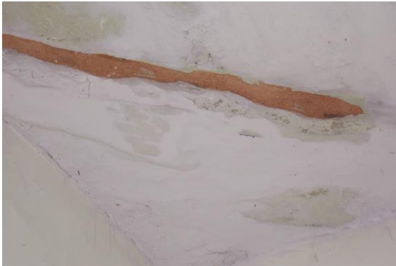
Photo 103 Peeling of Plaster on wall of Room No. 8 of Ground Floor
