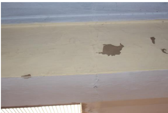
Photo 61 Peeling of Plaster on Wall No. 3 of Varanda of Second Floor
