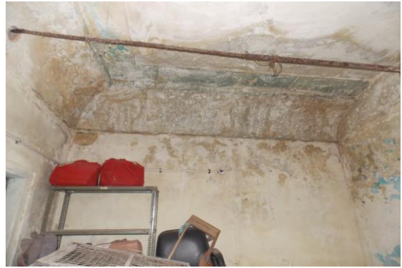
Photo 134 Peeling of Plaster on All Walls & Roof of Room No. 16(Part B)
