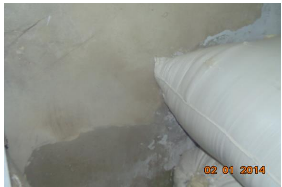
Photo 22 Dampness/Seepage on Wall No. 1 of Shop No. 4 of Ground Floor
