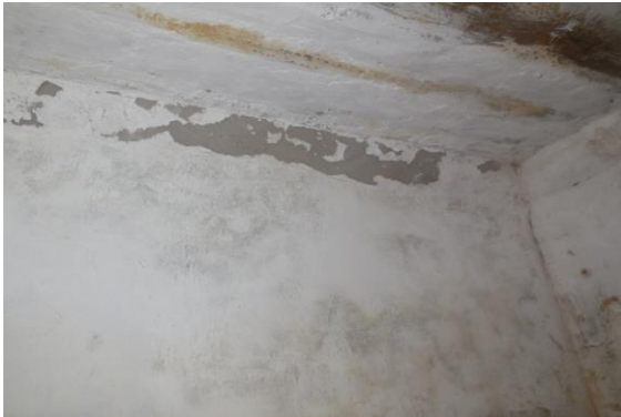
Photo 135 Peeling of Plaster on Wall No. 1 of Room No. 4 of Ground Floor
