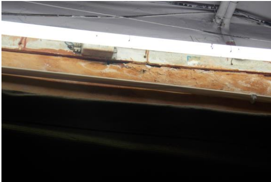
Photo 82 Peeling of Plaster on External Beam of Varanda of Shop No.178, Ground Floor
