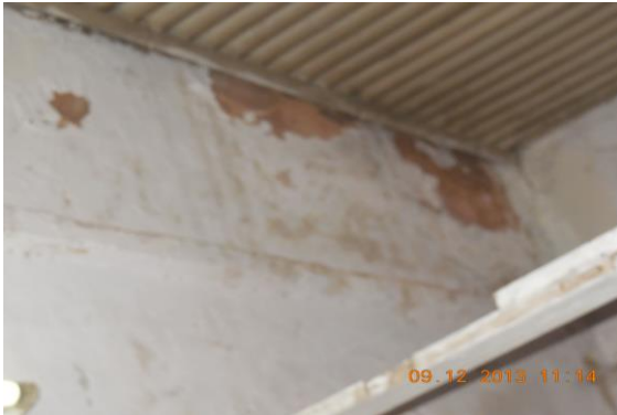
Photo 32 Peeling of Plaster on Wall No. 4 of Lobby of First Floor
