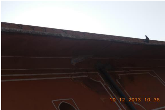
Photo 124 Peeling of Plaster on Shade of College + Temple of First Floor
