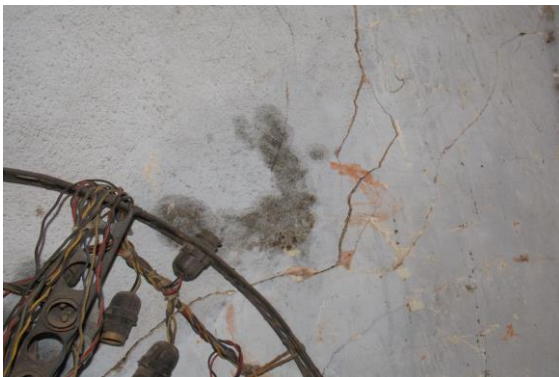
Photo 27 Peeling of Plaster on Wall No. 4 of Store No.2 of First Floor
