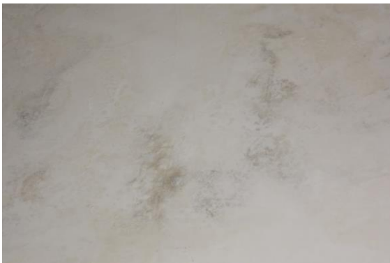
Photo 105 Dampness/Seepage on Wall No. 4 of Room No. 8 of Ground Floor
