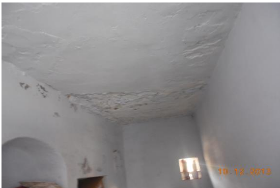
Photo 279 Peeling of Plaster on Roof of Toilet No. 2 of Second Floor
