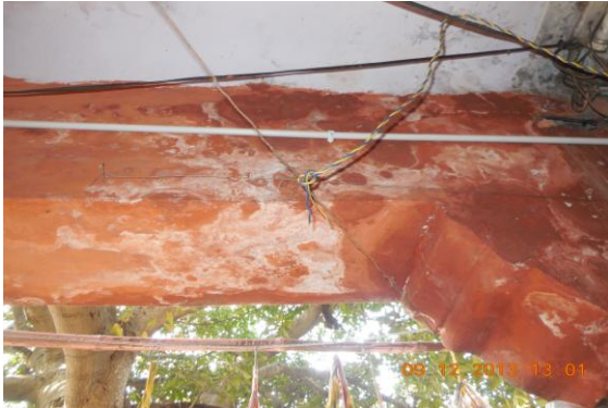
Photo 25 Dampness/Seepage on External Beam of Varanda of shop no.6A of Ground Floor
