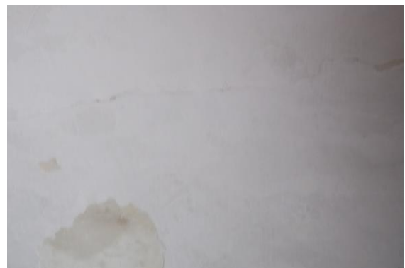
Photo 10 Horizontal Crack on Roof of Varanda of Shop No.791, Ground Floor Approx. Width = 0.1mm, Approx. Length = 2m. Distance from Rightside External Column = 0.5m, Height from Floor = 3m.
