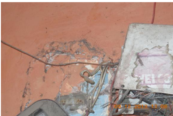
Photo 29 Damaged Portion on Leftside External Column of Varanda of Shop No.8 of Ground Floor
