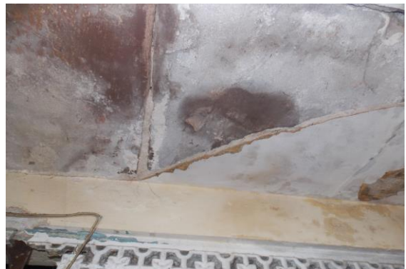
Photo 48 Peeling of Plaster on Wall No. 1 of Open Sky No.2 of First Floor
