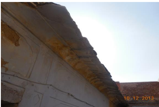
Photo 245 Damaged Portion on Wall No. 1 & Shade of Open Sky No.2 of Second Floor
