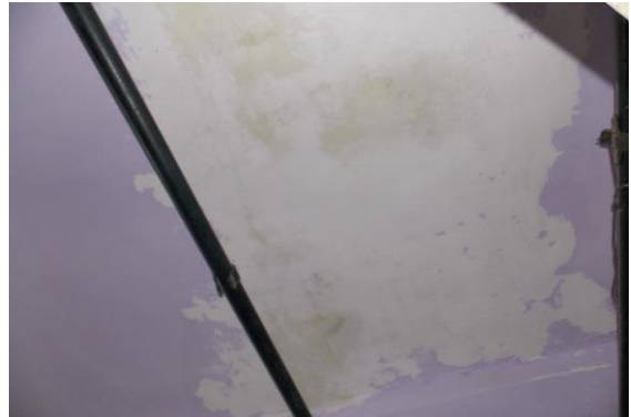
Photo 136 Dampness/Seepage on Roof of Room No. 14(Part B)
