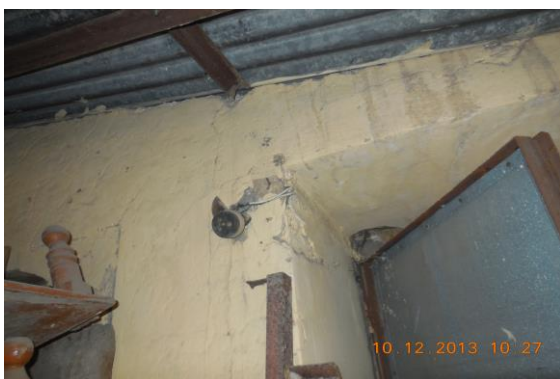
Photo 122 Peeling of Plaster on Wall No. 3 of Open Area 3 of College & Temple, First Floor
