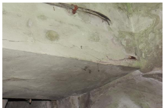
Photo 162 Peeling of Plaster on Wall No. 1 of Toilet No. 1
