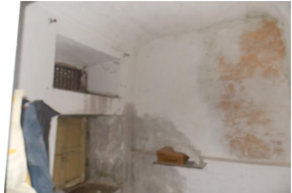
Photo 170 Dampness/Seepage on Wall No. 4 & 1 of Room No. 9
