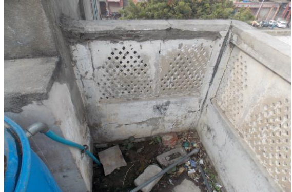
Photo 78 Dampness/Seepage on Wall No. 1, 4 & Roof of Hall No. 1 of Terrace
