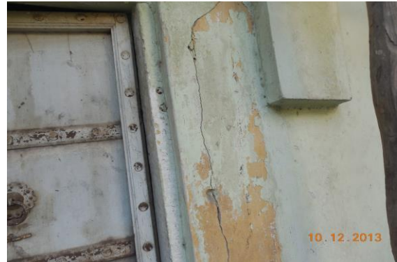
Photo 41 Inclined Crack on Wall No. 1 of Room No. 110, First Floor, Approx. Width = 2mm, Approx. Length = 4m. Distance from Wall No. 4 = 4.5m, Height from Floor = 0m.
