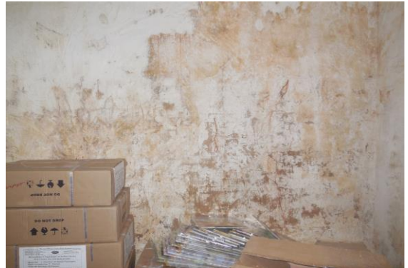
Photo 136 Dampness/Seepage on Wall No. 4 of Room No. 4 of Ground Floor
