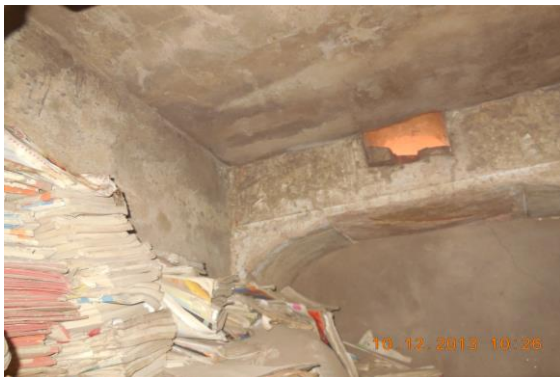
Photo 120 Dampness/Seepage on All Wall of Room No. 5 of First Floor
