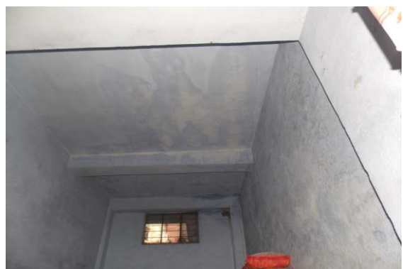
Photo 45 Dampness/Seepage on Wall No. 1, 2 & Roof of Part C of Shop No.776 of Ground Floor
