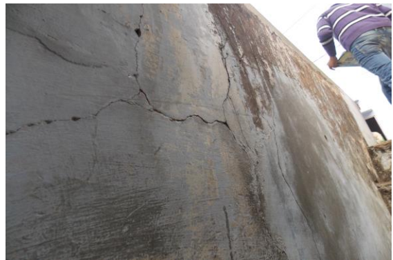
Photo 28 Peeling of Plaster on Wall No. 4 of Staircase FF to SF of First Floor
