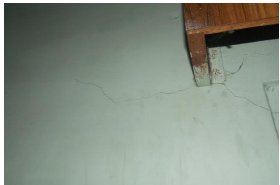
Photo 6 Inclined Crack on Wall No. 3 of Hall No. 5, First Floor Approx. Width = 0.4mm, Approx. Length = 1.1m. Distance from Wall no.2 = 1m, Height from Floor = 2m.
