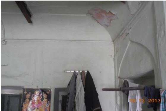
Photo 199 Peeling of Plaster on Roof of Room No. 107(Part A) of First Floor
