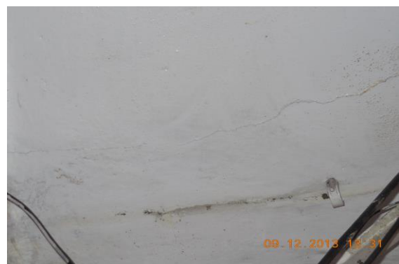
Photo 24 Horizontal Crack on Roof of Varanda, Shop No.21, Ground Floor Approx. Width = 0.5mm, Approx. Length = 0.6m. Height from Floor = 3m.
