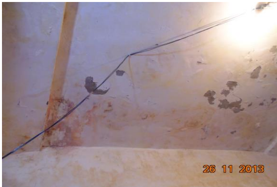
Photo 40 Peeling of Plaster on Roof of Shop No. 47 of Ground Floor
