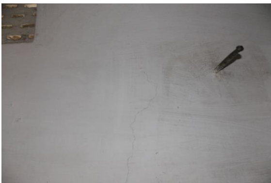
Photo 75 Plaster Crack on Wall No. 2 of Toilet No. 1 of First Floor
