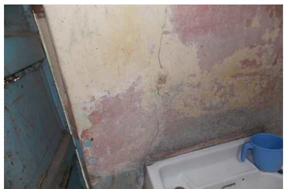
Photo 50 Peeling of Plaster on Wall No. 3 of Open Sky No.2 of First Floor
