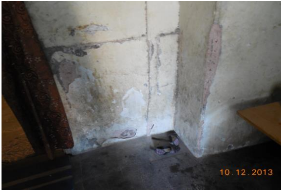
Photo 211 Peeling of Plaster on Wall No. 4 of Kitchen of First Floor
