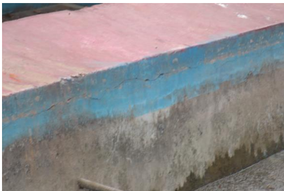
Photo 5 Horizontal Crack on Wall No. 2 of Boundary Wall B, Ground Floor Approx. Width = 0.5mm, Approx. Length = 3m. Distance from Wall No. 4 = 2m, Height from Floor = 0.4m.
