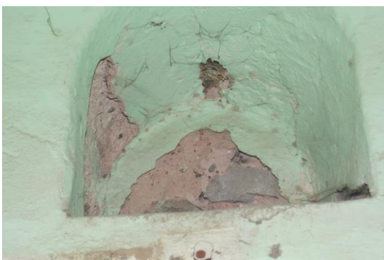
Photo 143 Peeling of Plaster on Wall No. 4 of Passage
