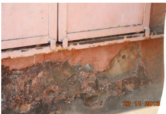
Photo 65 Peeling of Plaster on Left Side outer Wall Main gate of Temple of First Floor
