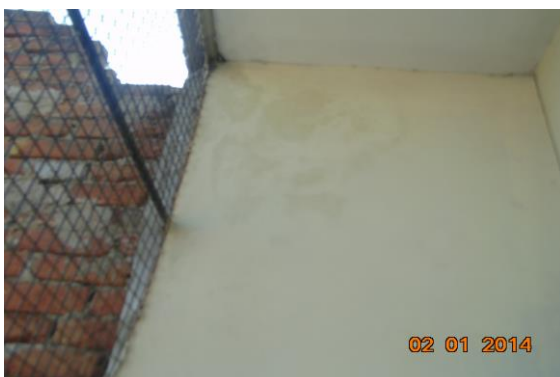
Photo 45 Peeling of Plaster on Roof of Hall No. 2 of Second Floor
