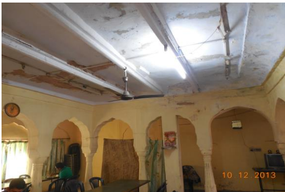
Photo 201 Dampness/Seepage on Roof of Room Mess Room of First Floor
