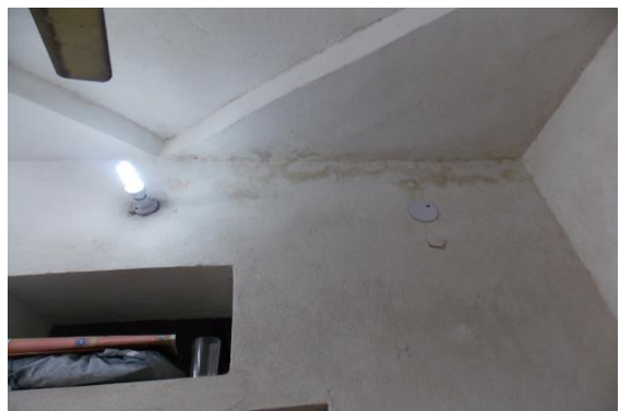
Photo 114 Dampness/Seepage on Wall No. 3 of Room No. 10 of Ground Floor
