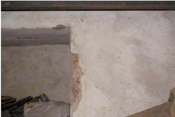
Photo 35 Peeling of Plaster on Wall No. 4 of Shop No. 5 of Ground Floor
