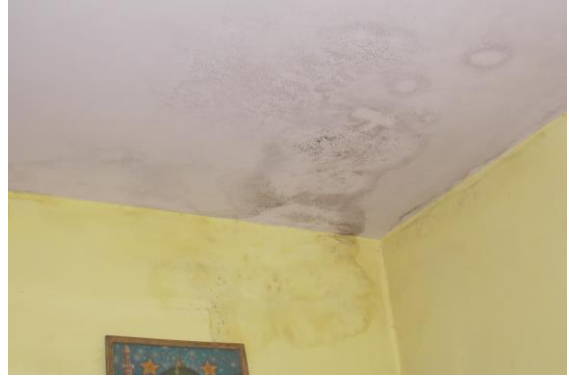
Photo 76 Dampness/Seepage on Floor of Terrace
