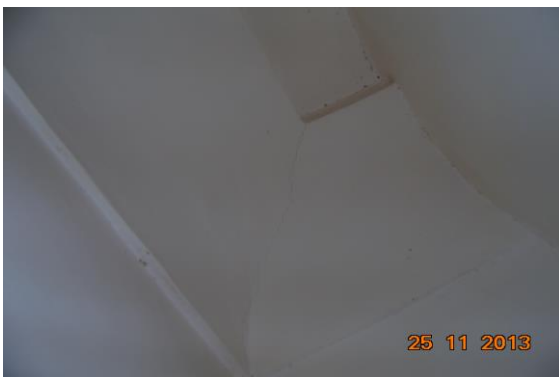
Photo 28 Inclined Crack on of Shop No. 16, Ground Floor, Approx. Width = 0.2mm, Approx. Length = 1.5m. Distance from Wall No.1 = 0.25m, Height from Floor = 2.1m.
