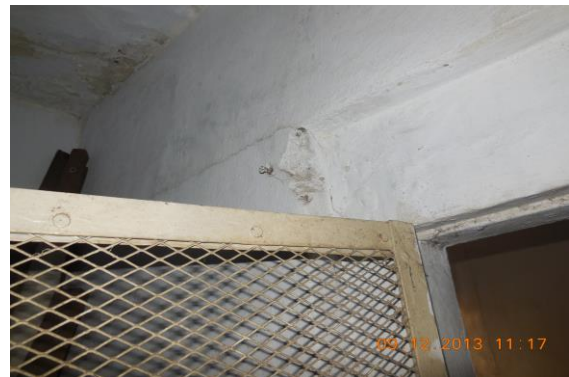
Photo 35 Peeling of Plaster on Wall No. 3 of Store of First Floor
