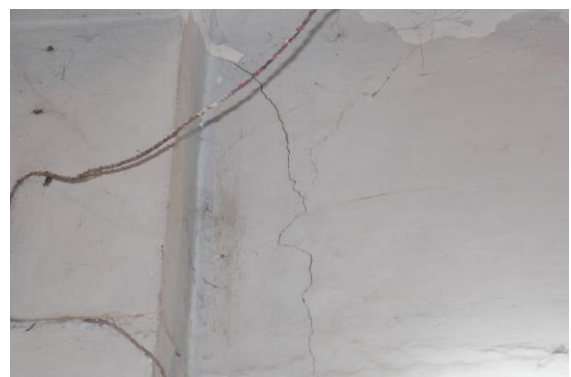
Photo 6 Inclined Crack on Wall No. 2 of Shop No.181, Ground Floor Approx. Width = 2mm, Approx. Length = 1.3m. Distance from Wall no.3 = 1.7m, Height from Floor = 2.6m.
