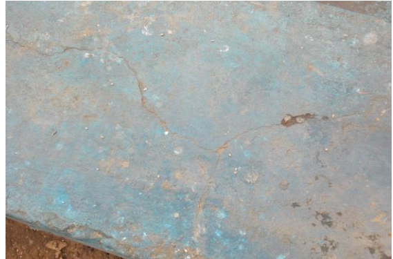
Photo 8 Peeling of Plaster on Floor of Boundary Wall B of Ground Floor
