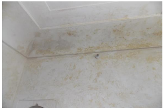
Photo 130 Dampness/Seepage on Wall No. 4, 2 & Roof of Room No. 16(part D)
