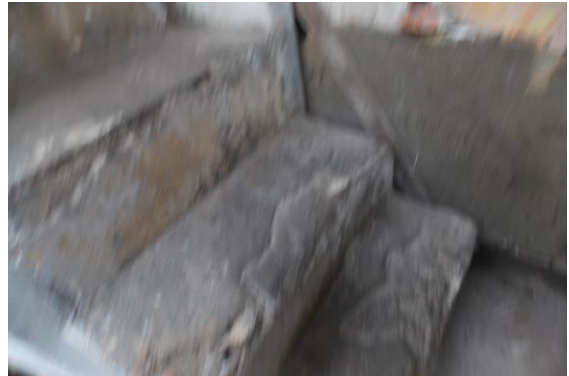
Photo 26 Peeling of Plaster on Staircase Steps of First Floor
