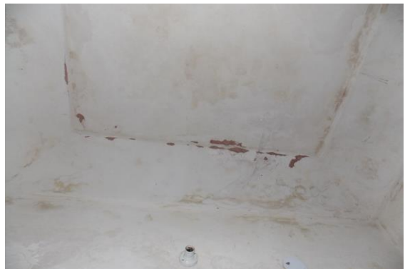
Photo 112 Dampness/Seepage on Roof of Room No. 10 of Ground Floor
