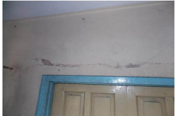
Photo 46 Peeling of Plaster on Wall No. 1 of Varanda of First Floor
