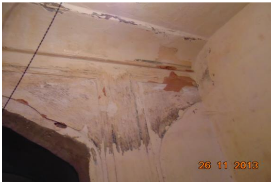
Photo 42 Peeling of Plaster on Wall No. 4 of Shop No. 47 of Ground Floor
