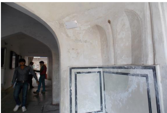
Photo 89 Dampness/Seepage on Wall No. 2 & 4 of Gate No.3 of Ground Floor
