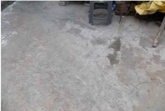
Photo 25 Peeling of Plaster on Floor of Open Sky No.1 of First Floor
