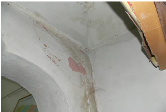
Photo 123 Dampness/Seepage on Wall No. 4 & Roof of Room No. 9 of
