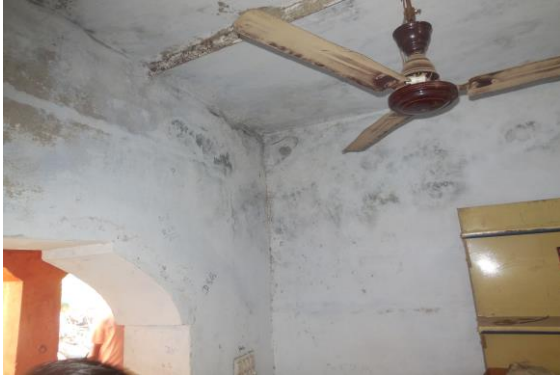
Photo 133 Dampness/Seepage on Wall No. 1 & 3 of Hall No. 1 of Ground Floor
