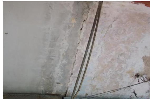
Photo 52 Horizontal Crack on Roof of Varanda of Shop No.767, Ground Floor Approx. Width = 2mm, Approx. Length = 1.5m. Distance from Rightside External Column = Backsidem, Height from Floor = 3m.
