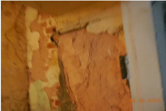
Photo 265 Peeling of Plaster on Wall No. 2 of Bathroom of Second Floor
