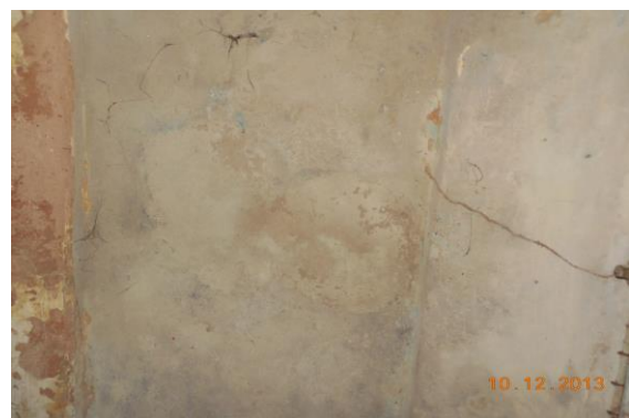
Photo 228 Dampness/Seepage on Roof of Room Dark Room of First Floor
