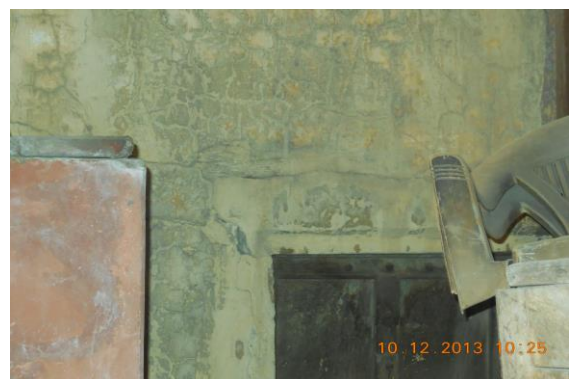
Photo 123 Peeling of Plaster on Outer Wall Right Side of Room No. 5 of First Floor
