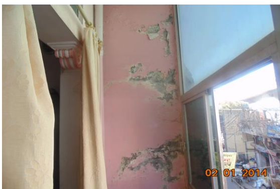
Photo 39 Dampness/Seepage on Wall No. 1 of First Floor
