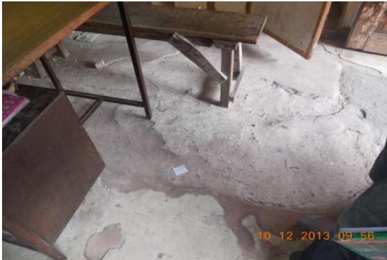
Photo 106 Peeling of Plaster on Floor of Hall No. 1(Part-I) of First Floor
