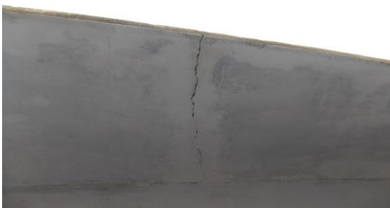
Photo 4 Horizontal Crack on Wall No. 2 of Shade Roof, First Floor Approx. Width = 3mm, Approx. Length = 1m. Distance from Wall No.3 = 1.7m, Height from Floor = 3m.
