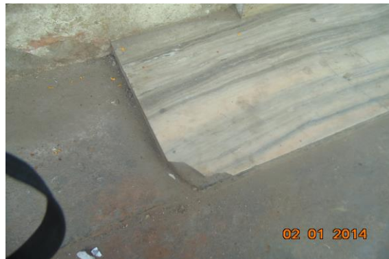
Photo 14 Damaged Portion on of Main Entry Marble Slab of Shop No. 1, Ground Floor
