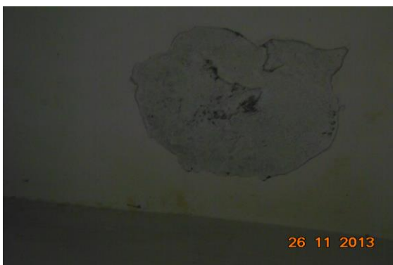
Photo 44 Peeling of Plaster on Wall No. 2 of Passage 3 of Shop No. 221 of Ground Floor
