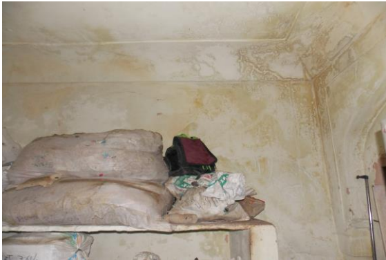
Photo 175 Dampness/Seepage on Wall No. 2 of Store No.2
