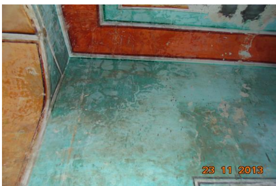
Photo 53 Dampness/Seepage on Wall No. 1 of Varanda No.4 of First Floor
