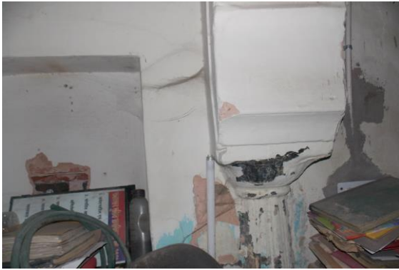
Photo 133 Peeling of Plaster on Wall No. 1 of Room No. 15(PartA)
