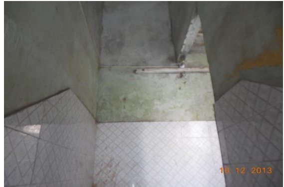
Photo 178 Dampness/Seepage on Wall No. 4 of Part B Staircase Ground Floor To First Floor of Ground Floor
