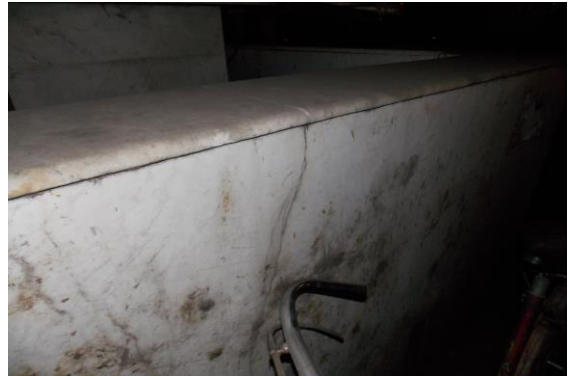
Photo 4 Damaged Portion on Rightside Perapet Wall of Shiv Ji Ka Temple of Ground Floor
