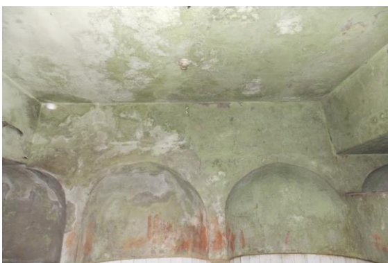
Photo 161 Dampness/Seepage on Wall No. 2, 4 & Roof of Toilet No. 1
