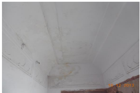
Photo 288 Damaged Portion on Roof of Balcony Gate of Second Floor
