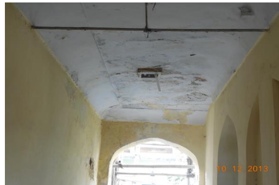
Photo 202 Dampness/Seepage on Wall No. 2, 3 & Roof of Room Mess Room of First Floor
