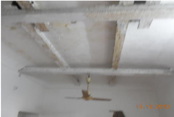
Photo 213 Dampness/Seepage on Roof of Room No. 111 of First Floor
