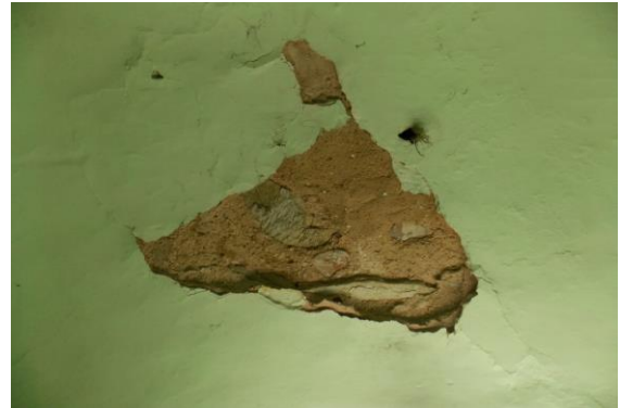
Photo 146 Damaged Portion on Roof of Passage
