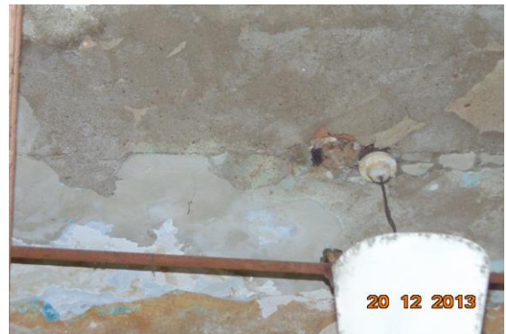
Photo 85 Peeling of Plaster on Roof of Shop No.172 of Ground Floor
