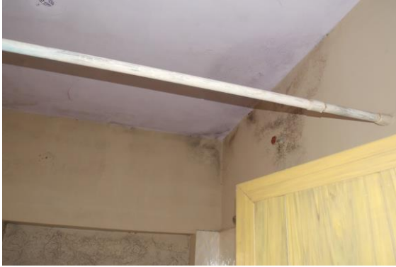
Photo 75 Dampness/Seepage on Wall No. 4 of Terrace
