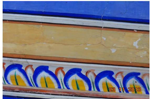
Photo 50 Peeling of Plaster on Roof of Varanda No.2 of Ground Floor
