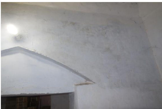
Photo 137 Dampness/Seepage on Wall No. 3 of Room No. 6 of Ground Floor
