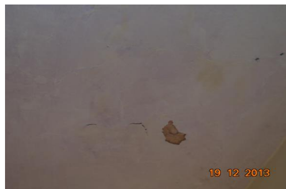
Photo 53 Dampness/Seepage on Roof of Bathroom of First Floor
