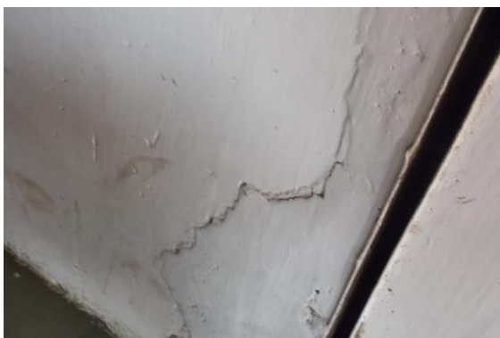
Photo 99 Plaster Crack on Roof of Shop No. 364A of Ground Floor
