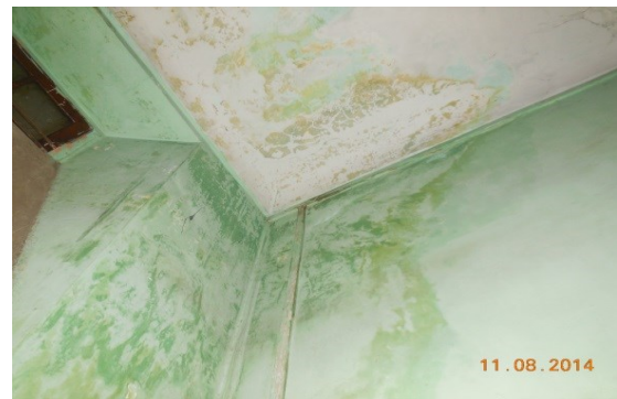
Photo 125 Seepage on Wall No. 1 & Roof of Room No. 2 of Hind Hotel, First Floor
