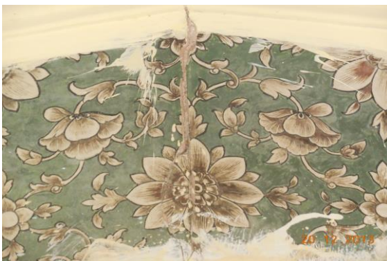
Photo 86 Peeling of Plaster on Wall No. 2 of Lobby No.1 of Ground Floor
