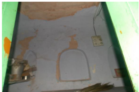
Photo 30 Peeling of Plaster on Wall No.4 & Roof of Room No. 3 of House No. 483, First Floor
