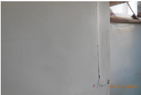
Photo 65 Peeling of Plaster of Room No. 1 of Second Floor
