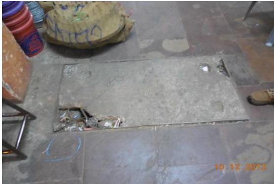
Photo 66 Damaged Portion on Floor of Varanda of Shop No. 307, Ground Floor
