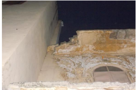
Photo 83 Peeling of Plaster on Front Side Wall of External Façade
