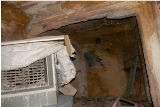
Photo 34 Peeling of Plaster on Roof of Hall No. 1 of First Floor
