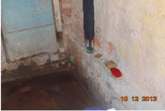
Photo 155 Peeling of Plaster on Wall No. 1, 2 & 4 of Second Floor
