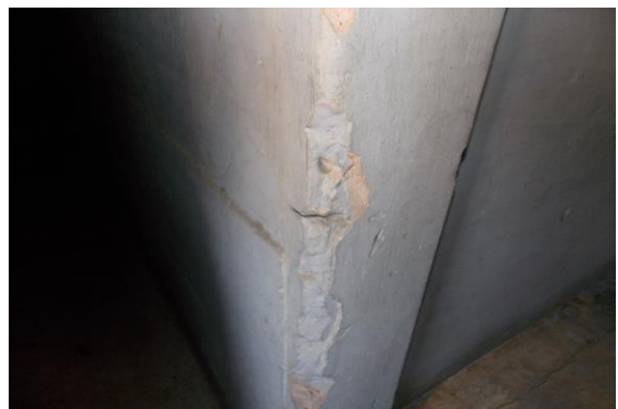
Photo 51 Peeling of Plaster on Wall No. 2 of Passage No.8 of First Floor
