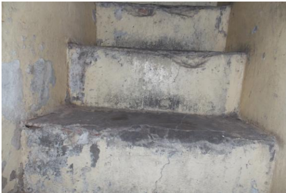
Photo 29 Damaged Portion on Steps of Staircase of
