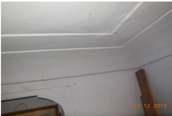
Photo 22 Inclined Crack on Wall No. 2 & Roof of Hall No. 2, Basement Approx. Width = 0.25mm, Approx. Length = 1.6m. Distance from Wall no.4 = 0.4m, Height from Floor = 1.5m.
