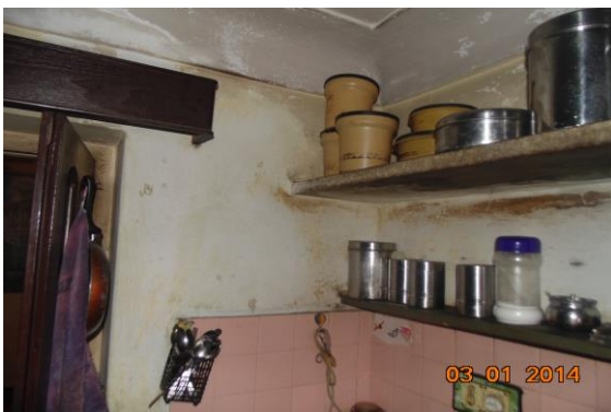
Photo 84 Dampness/Seepage on Wall No. 4 of Kitchen of Second Floor - Part B
