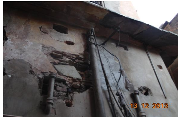
Photo 92 Dampness/Seepage on Right Side wall of External Façade of House No. 635, First Floor
