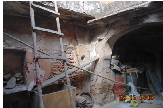
Photo 8 Peeling of Plaster on All Walls of Open Sky Area No.2 of First Floor
