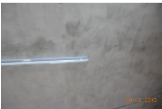
Photo 22 Horizontal Crack on Roof of Varanda, Shop No. 304, Ground Floor, Approx. Width = 0.8mm, Approx. Length = 3m. Distance from Left Side External Column = 0m, Height from Floor = 3m.
