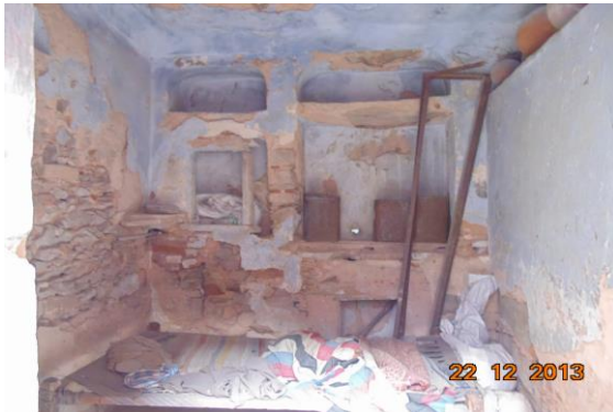
Photo 7 Peeling of Plaster on Room No. 2 of First Floor
