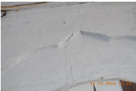
Photo 5 Inclined Crack on of Open Sky, House No. 483, First Floor Approx. Width = 0.4mm, Approx. Length = 0.9m. Distance from W1 = 1m, Height from Floor = 2.2m.
