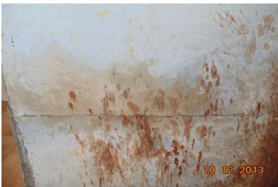
Photo 159 Peeling of Plaster on Wall No. 4 of Staircase SF to TF of Second Floor
