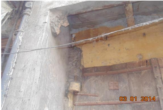
Photo 98 Peeling of Plaster on Shop 1 of External façade
