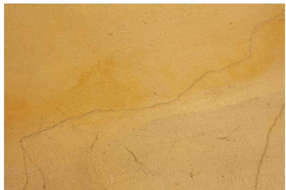
Photo 23 Inclined Crack on Wall No. 2 & Roof of Part B of Shop No.377, Ground Floor Approx. Width = 1mm, Approx. Length = 2m. Distance from Wall No.2 = 0m, Height from Floor = 2.4m.
