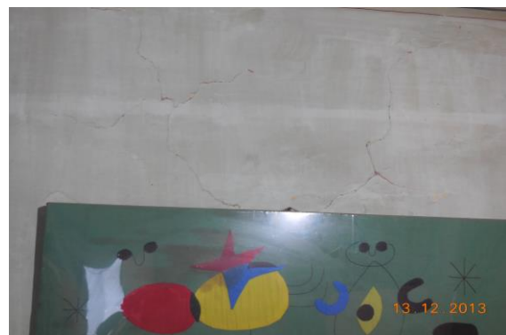
Photo 148 Plaster Crack on of Room No. 3 of Second Floor
