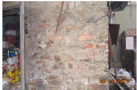
Photo 4 Peeling of Plaster on External Façade of Building
