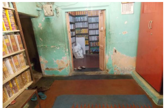
Photo 4 Inclined Crack on Wall No. 2 of Staircase, Ground Floor, Approx. Width = 2.5mm, Approx. Length = 1.8m. Distance from Wall no.3 = 2.3m, Height from Floor = 0m.
