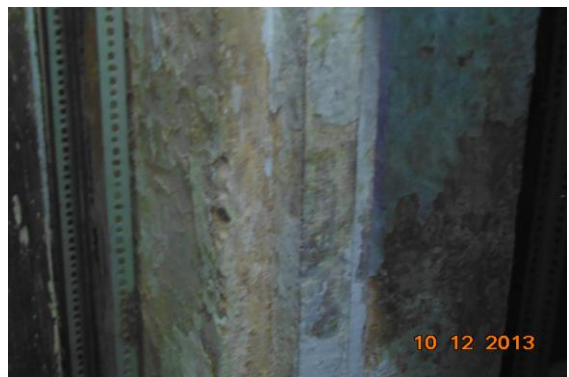
Photo 18 Peeling of Plaster on Wall No. 3 of Part-IV of Shop No.115 of First Floor
