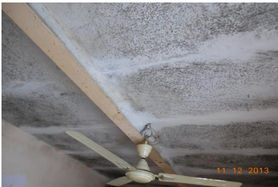
Photo 57 Dampness/Seepage on Roof of Room No. 14 of First Floor
