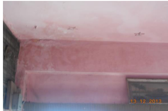
Photo 144 Dampness/Seepage on Wall No.4 & Roof of Room No. 4 of Second Floor
