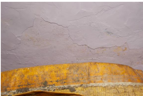
Photo 5 Peeling of Plaster on Roof of Shop No. 474 Part B of Ground Floor
