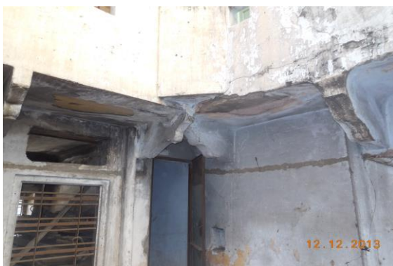
Photo 43 Peeling of Plaster on Sunshade of Open Area of House No. 424 Part A, Ground Floor
