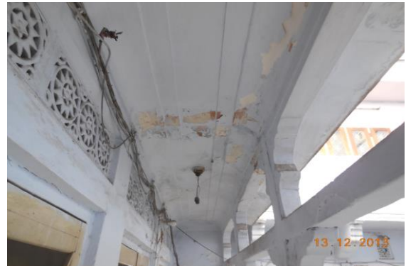
Photo 114 Peeling of Plaster on Roof of Balcony-4 of House No. 635, First Floor
