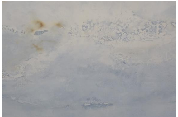
Photo 170 Peeling of Plaster on Roof of Lobby No.1 of Shri Krishna Chandra Ji Temple, First Floor
