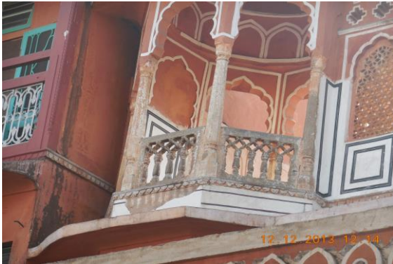
Photo 150 Peeling of Plaster on Front of Building portion of House No. 651, Second Floor
