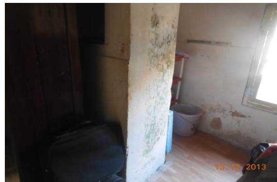
Photo 134 Peeling of Plaster on Floor of Store-1 of House No. 635, Second Floor
