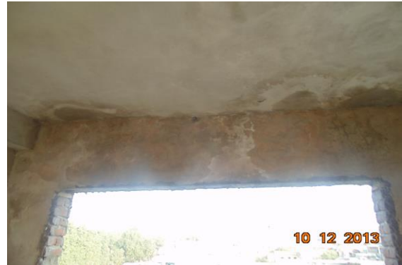
Photo 162 Dampness/Seepage on Wall No. 4 of Shop No.305 of Third Floor
