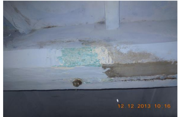
Photo 43 Dampness/Seepage on Roof of Shop No. 2 of Ground Floor
