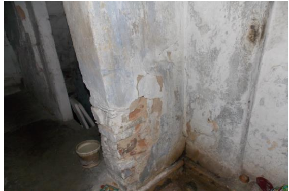
Photo 29 Peeling of Plaster on Wall No. 3 & 1 of Passage No.2 of First Floor
