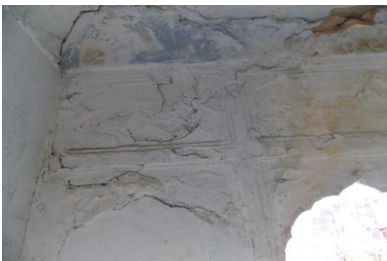
Photo 44 Peeling of Plaster on Wall No. 1 of Lobby No.1 of First Floor
