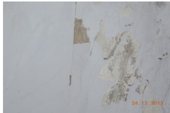
Photo 66 Peeling of Plaster on Roof of Lobby of House No.843,844 of Second Floor
