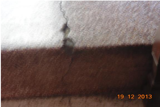
Photo 26 Damaged Portion on Floor of Passage No.1 of First Floor
