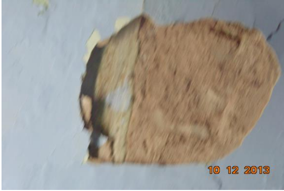
Photo 13 Peeling of Plaster on Roof of Part-II of Shop no.115 of First Floor
