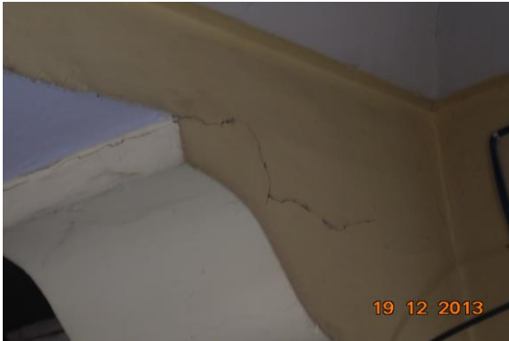
Photo 9 Inclined Crack on Wall No. 3 of Passage No. 1, First Floor, Approx. Width = 5mm, Approx. Length = 2m.
