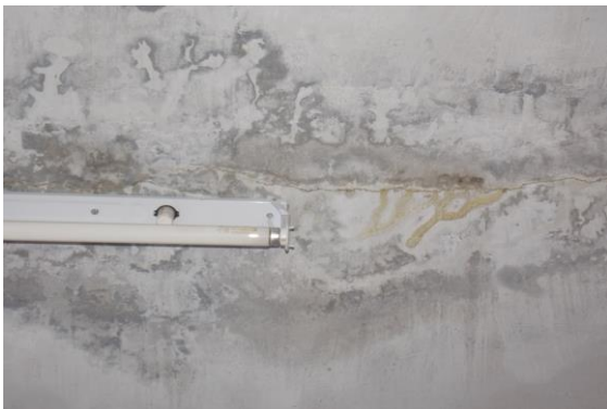
Photo 27 Horizontal Crack on Roof of Varanda of Shop No.205, G/F Approx. Width = 0.35mm, Approx. Length = 2.5m. Distance from Leftside External Column = Backsidem, Height from Floor = 3m.
