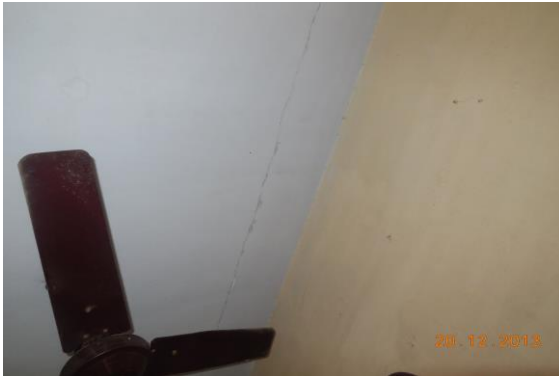
Photo 55 Inclined Crack on Roof of Room No. 7, First Floor Approx. Width = 0.5mm, Approx. Length = 3m.
