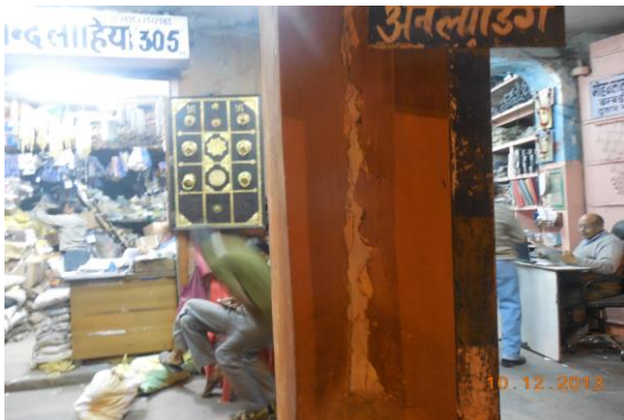
Photo 62 Damaged Portion on Right side External Beam of Shop No. 305 of Ground Floor
