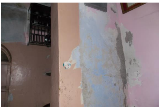
Photo 38 Peeling of Plaster on Roof of Room No. 6 of First Floor
