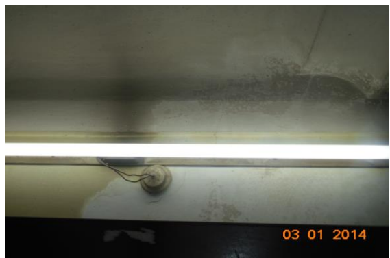
Photo 85 Dampness/Seepage on Wall No. 4 of Kitchen of Second Floor - Part B
