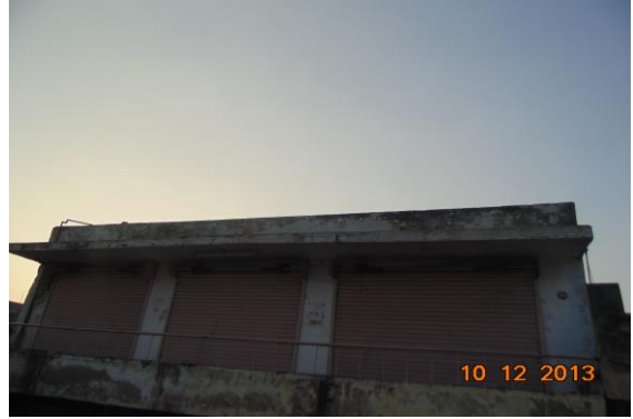
Photo 14 Dampness/Seepage on Outer wall Shade Roof of Shop no.312 to 314 of Third Floor
