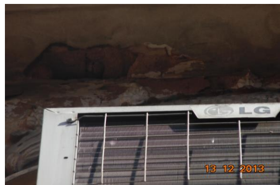
Photo 94 Damaged Portion on Front Side Wall & Shade of External Façade of House No. 635, First Floor
