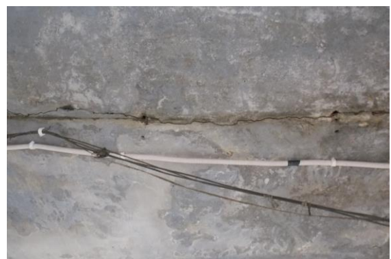
Photo 12 Horizontal Crack on Roof of Varanda of Shop No.274 A, Ground Floor, Approx. Width = 3mm, Approx. Length = 2.2m. Distance from Back of Left External Column = 0m, Height from Floor = 3m.
