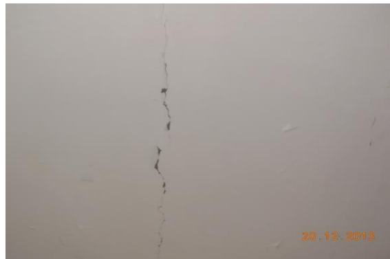
Photo 23 Inclined Crack on Room No. 1, First Floor Approx. Width = 1mm, Approx. Length = 2m.
