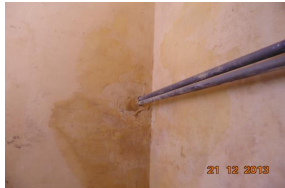
Photo 133 Dampness/Seepage on Wall No. 4 of Staircase of Ground Floor
