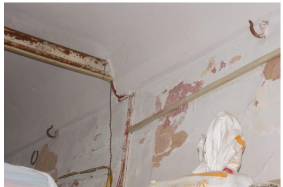
Photo 111 Peeling of Plaster on Wall No. 3 of Shop No.6 of Ground Floor
