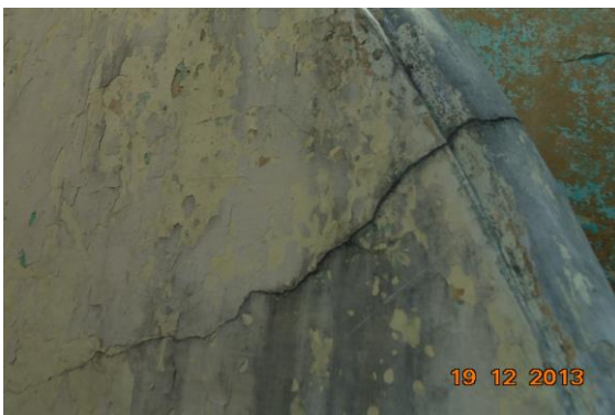
Photo 11 Inclined Crack on Wall No. 2 of Staircase First Floor to Second Floor, First Floor, Approx. Width = 1.5mm, Approx. Length = 1.5m. Distance from Wall No. 2 = 2m, Height from Floor = 1m.
