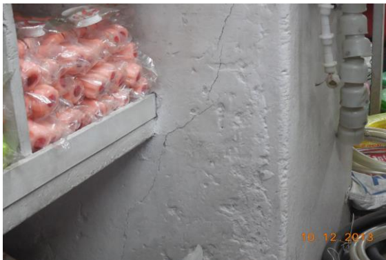
Photo 21 Inclined Crack on Wall No. 1 & Beam Portion of Shop No. 298, Ground Floor, Approx. Width = 1mm, Approx. Length = 1.5m. Distance from Wall No. 3 = 2m, Height from Floor = 0m.
