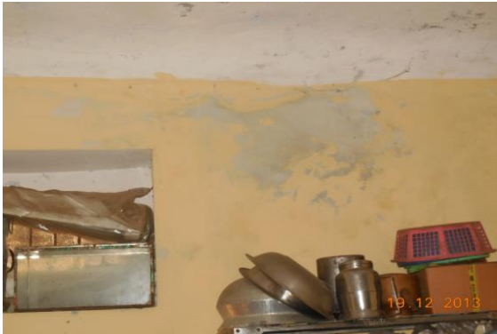
Photo 33 Peeling of Plaster on Wall No. 4 of Kitchen of First Floor
