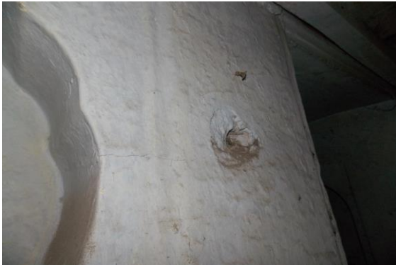
Photo 48 Peeling of Plaster on Wall No. 2 of Passage No.5 of First Floor
