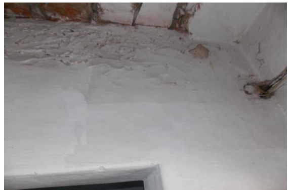
Photo 25 Peeling of Plaster on Wall No. 2 of Passage No.1 of First Floor
