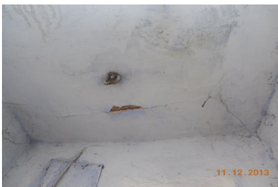
Photo 51 Peeling of Plaster on Wall No. 2 & Roof of Open Sky of First Floor
