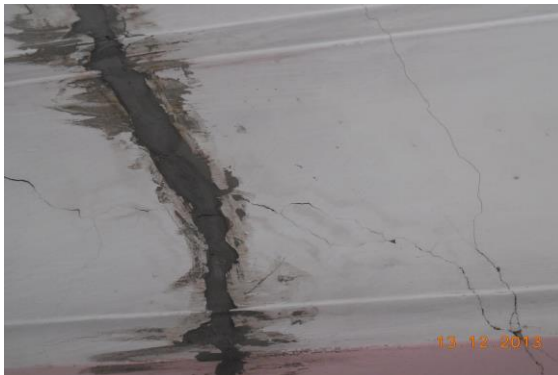
Photo 181 Plaster Crack on Wall No.2 & Roof of Room No. 5 of Second Floor
