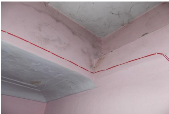
Photo 3 Inclined Crack on Wall No. 3 of Room No. 1, Second Floor, Approx. Width = 0.2mm, Approx. Length = 1.2m. Distance from Wall no.1 = 0m, Height from Floor = 3m.
