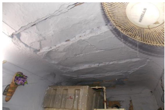
Photo 25 Dampness/Seepage on Roof of Room No. 1 of First Floor
