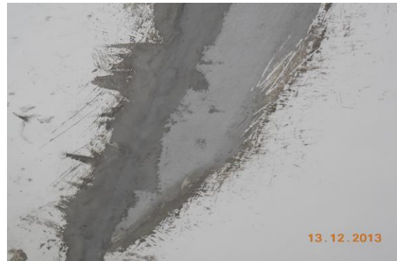
Photo 182 Peeling of Plaster on Roof of Room No. 5 of Second Floor
