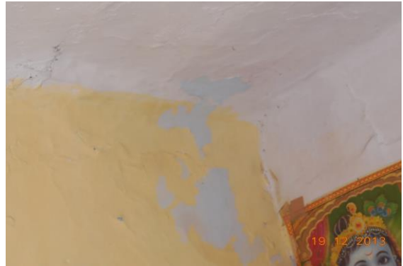
Photo 34 Peeling of Plaster on Wall No. 1 & Roof of Bilding Udey Singh Ji Ki Haveli of First Floor
