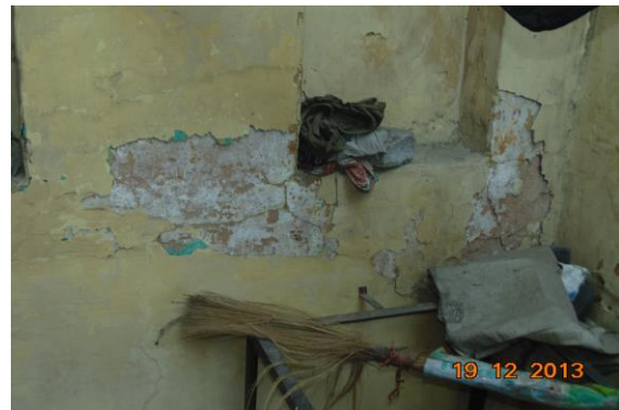
Photo 57 Peeling of Plaster on Wall No. 3 of Open Sky Area of First Floor
