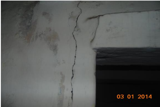
Photo 9 Inclined Crack on Wall No. 3 of Balcony 3, Second Floor - Part A Approx. Width = 3mm, Approx. Length = 1.3m. Distance from w2 = 1.5m, Height from Floor = 1.05m.
