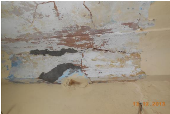
Photo 143 Peeling of Plaster on Roof of Temple of House No. 635, Second Floor
