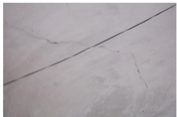
Photo 12 Inclined Crack on Roof of Varanda of Shop No. 380, Ground Floor Approx. Width = 0.6mm, Approx. Length = 1.8m. Distance from = Leftside External Column Backsidem, Height from Floor = 3.3m
