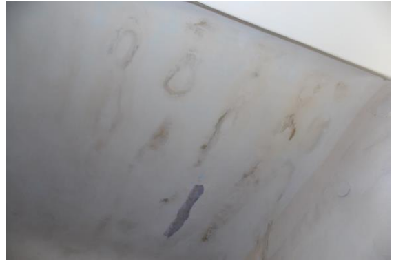
Photo 137 Peeling of Plaster on Roof of Hall No. 8 of Library, First Floor
