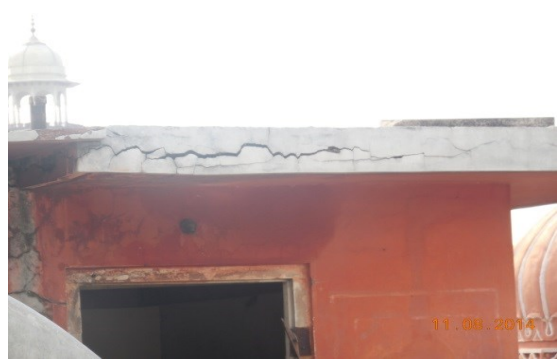
Photo 121 Damage on Shade of Room No. 1 of Hind Hotel, Terrace
