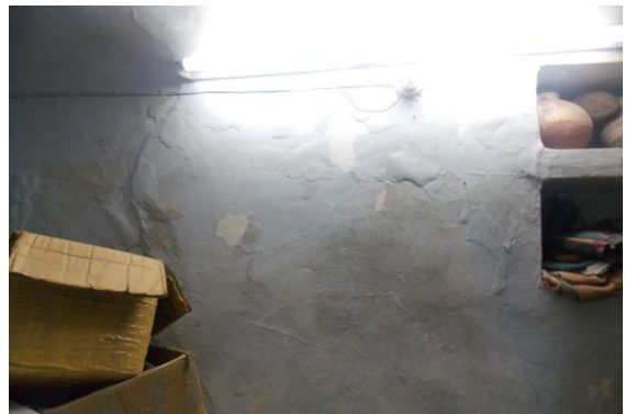
Photo 33 Peeling of Plaster on Wall No. 4 of Room No. 2 of First floor
