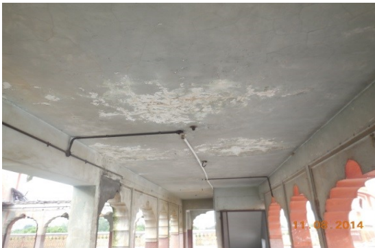
Photo 114 Seepage on Roof of Varanda No. 1 of Hind Hotel, Third Floor
