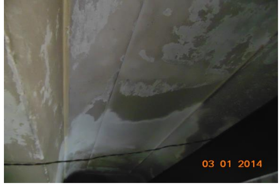
Photo 81 Peeling of Plaster on Wall No. 1 of Room No. 1 of Second Floor - Part B
