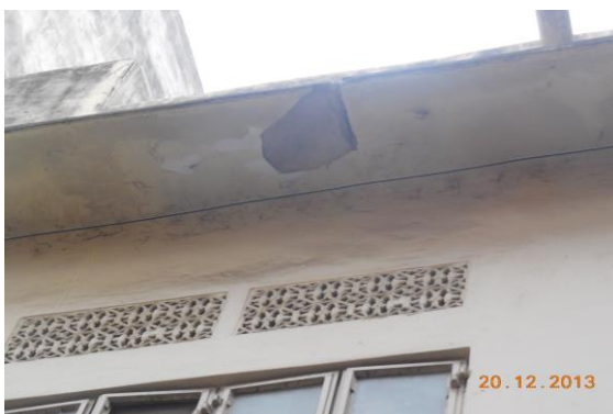
Photo 152 Damaged Portion on Outside Front Wall no.3 of Building of Second Floor
