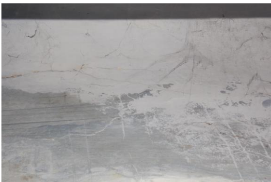
Photo 10 Inclined Crack on Wall No. 1 of Passage No.2, First Floor, Approx. Width = 2mm, Approx. Length = 2.1m. Distance from Wall No.3 = 2m, Height from Floor = 2.6m.
