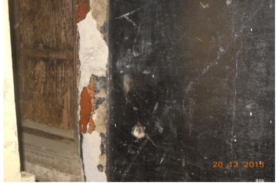
Photo 101 Damaged Portion on Frontside Wall No.3 of Temple of Ground Floor
