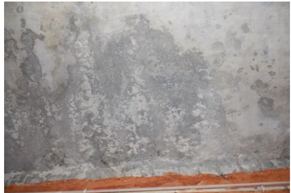
Photo 8 Dampness/Seepage on Roof of Varanda of Shop No.235 of Ground Floor
