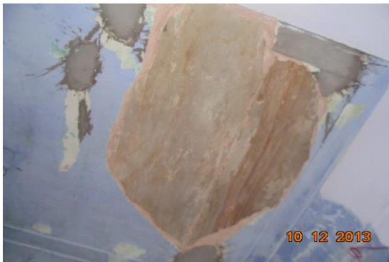
Photo 9 Peeling of Plaster on Roof & Front of Lobby of shop no.115 of First Floor
