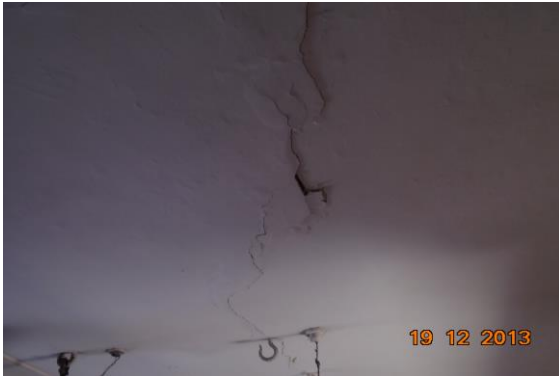
Photo 24 Damaged Portion on Roof of Room No. 1 of First Floor
