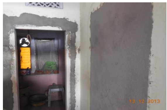
Photo 172 Peeling of Plaster on All Wall of Passage of House No. 635, Second Floor
