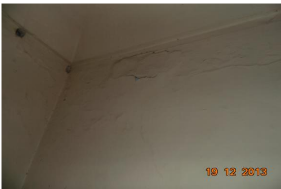
Photo 28 Peeling of Plaster on Wall No. 4 of Store No.1 of First Floor
