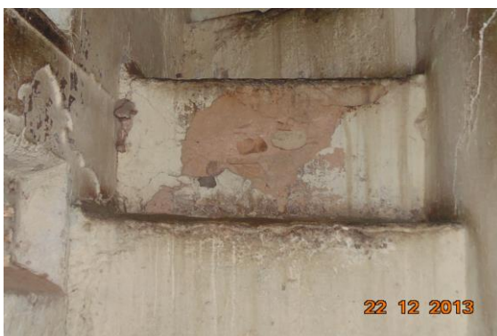
Photo 16 Peeling of Plaster on Steps of Staircase FF to SF of First Floor
