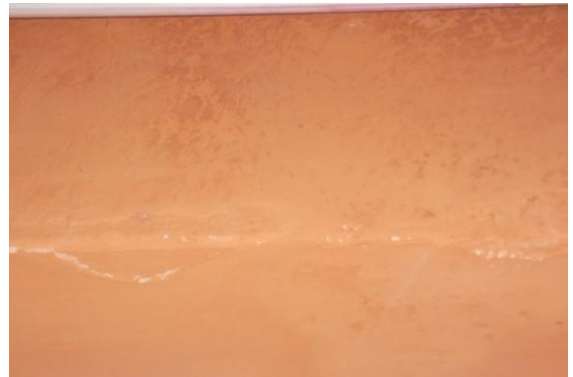
Photo 30 Peeling of Plaster on External Beam of Varanda of H.No.70 of
