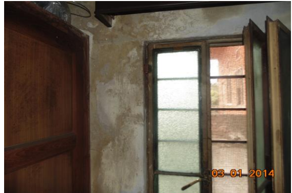
Photo 83 Peeling of Plaster on Roof of Kitchen of Second Floor - Part B
