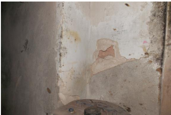
Photo 114 Peeling of Plaster on Frontside Wall of Shop No.6 of Ground Floor
