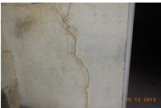
Photo 59 Inclined Crack on Wall No. 3 of Open Sky, Second Floor Approx. Width = 2.5mm, Approx. Length = 2m. Distance from Wall no.2 = 2.5m, Height from Floor = 0m.
