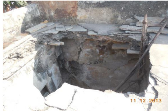
Photo 48 Dampness/Seepage on Roof of Room No. 7 of First Floor
