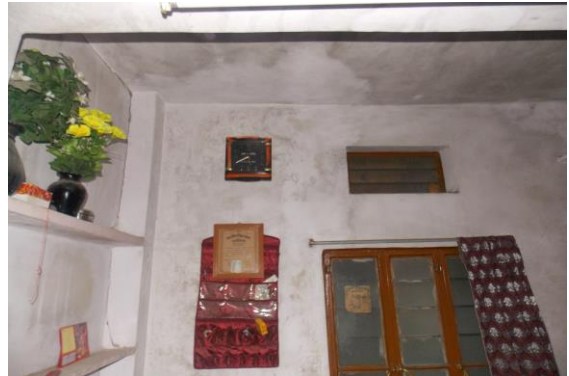
Photo 35 Dampness/Seepage on Roof & Wall No. 4 of Room No. 4 of First Floor
