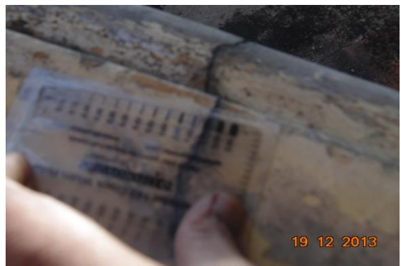
Photo 11A Inclined Crack on Wall No. 2 of Staircase First Floor to Second Floor, First Floor, Approx. Width = 1.5mm, Approx. Length = 1.5m. Distance from Wall No. 2 = 2m, Height from Floor = 1m.
