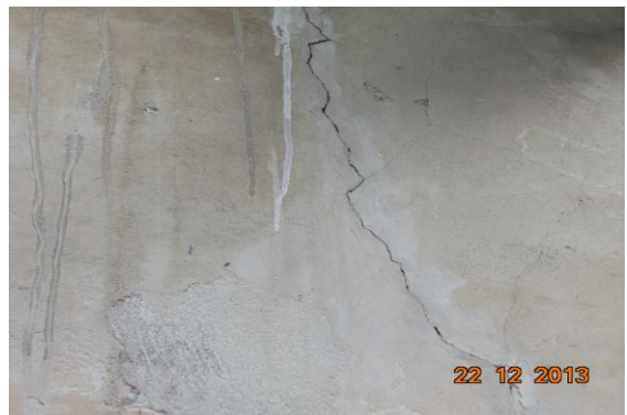
Photo 10 Inclined Crack on Outer Wall of External Façade H. No.476, First Floor Approx. Width = 0.8mm, Approx. Length = 1m. Distance from Leftside Wall = 0.1m, Height from Floor = 3m.
