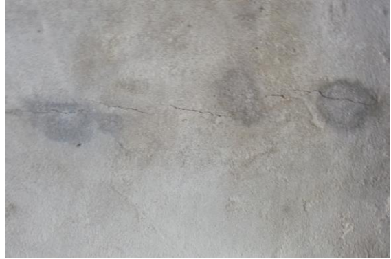
Photo 19 Horizontal Crack on Roof of Varanda of Shop No. 378, Ground Floor Approx. Width = 0.3mm, Approx. Length = 3m. Distance from Backside Left Side Column = 1.5m, Height from Floor = 3.3m.
