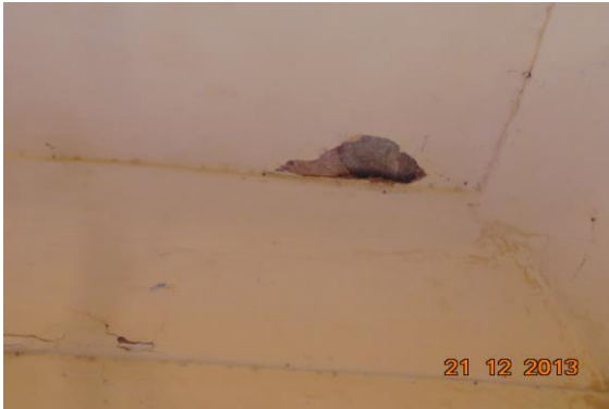
Photo 110 Peeling of Plaster on Roof of Room No. 5 of Temple, Ground Floor
