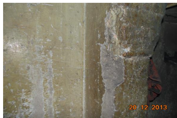
Photo 103 Peeling of Plaster on Roof of Shop No.2 of Ground floor
