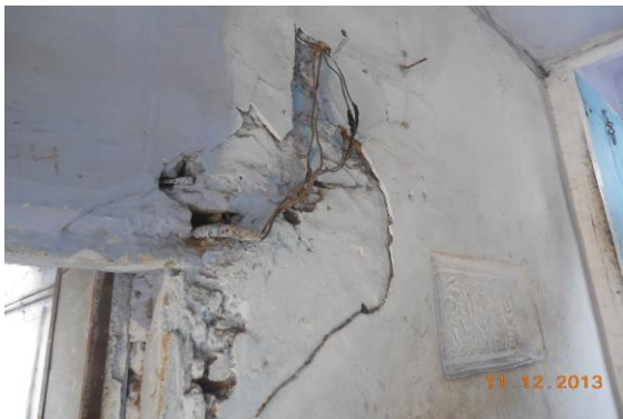
Photo 49 Peeling of Plaster on Wall No. 1 of StairCase of Ground Floor
