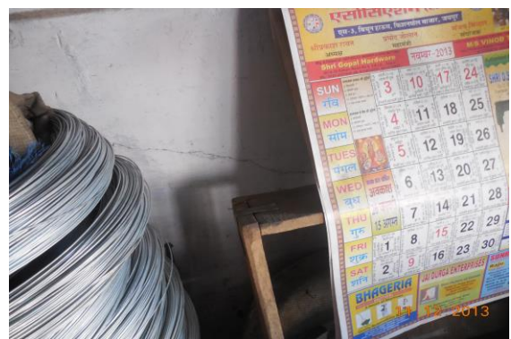
Photo 6 Inclined Crack on Wall No. 2 of Shop No. 310, Ground Floor Approx. Width = 0.5mm, Approx. Length = 1m. Distance from Gate = 1.4m, Height from Floor = 1m.
