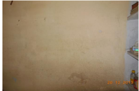
Photo 143 Dampness/Seepage on Wall No. 2 of Room No. 7 of First Floor
