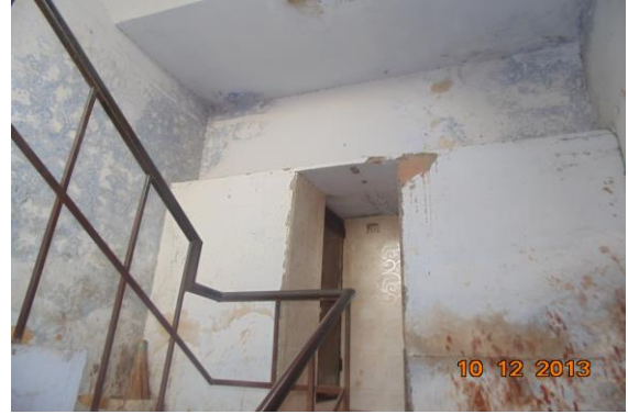
Photo 156 Dampness/Seepage on Wall No. 1, 2 & 4 of Staircase SF to TF of Second Floor
