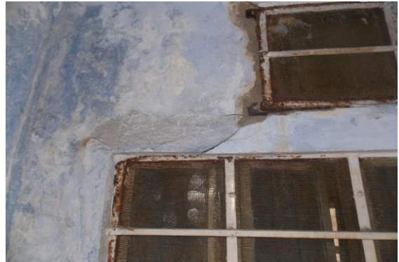
Photo 39 Peeling of Plaster on Wall No. 2 of Open sky area of First floor
