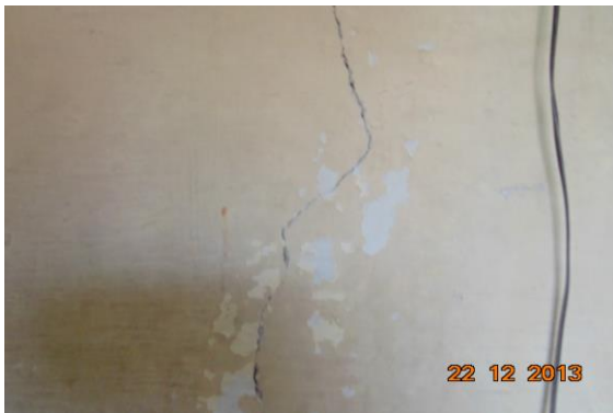
Photo 3 Inclined Crack on Wall No. 1 of Room No. 1, Second Floor Approx. Width = 0.6mm, Approx. Length = 2.5m. Distance from Wall No.1 = 0.7m, Height from Floor = 0m.
