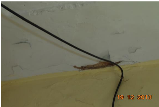
Photo 32 Peeling of Plaster on Roof of Room No. 2 of First Floor
