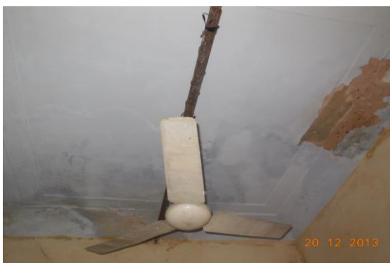
Photo 80 Dampness/Seepage on Roof of Room No. 1 of Part b of Room. Ground Floor
