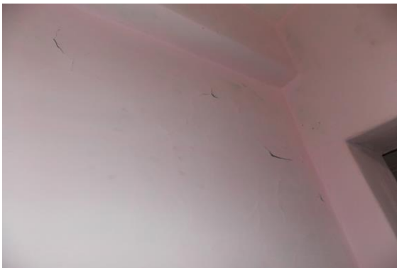
Photo 30 Peeling of Plaster on Wall No. 1 of Room No. 4 of First Floor
