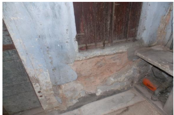
Photo 61 Dampness/Seepage of Sky open of House No. 483, Ground Floor
