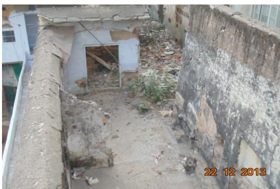
Photo 53 Peeling of Plaster on of Open Area of First Floor Part B
