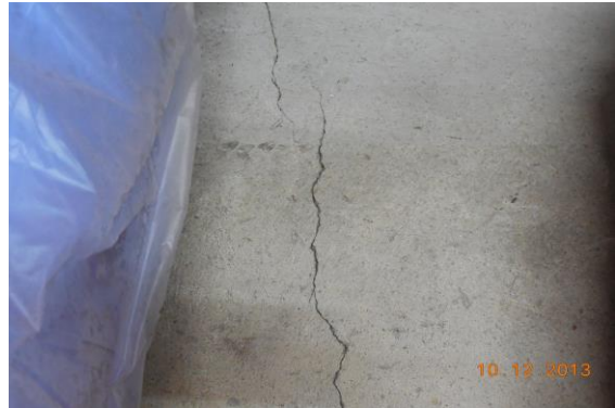
Photo 20 Vertical Crack on Wall No. 4 of Shop No. 298, Ground Floor, Approx. Width = 1mm, Approx. Length = 0.5m. Distance from Wall No. 1 = 1m, Height from Floor = 1.8m.
