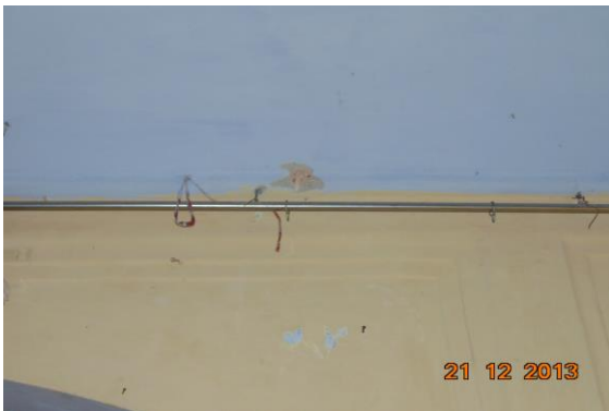
Photo 80 Peeling of Plaster on Wall No. 2 of Varanda No.2 of Ground Floor
