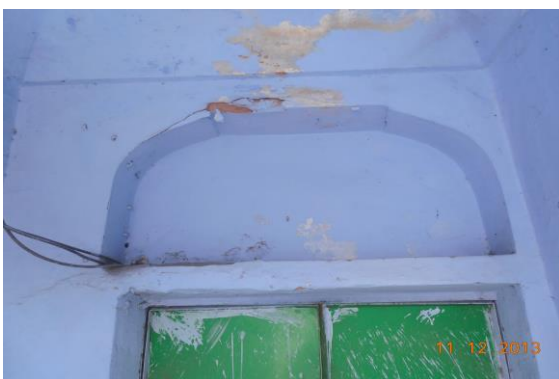
Photo 33 Peeling of Plaster on Wall No. 4 of Passage No.2 of First Floor
