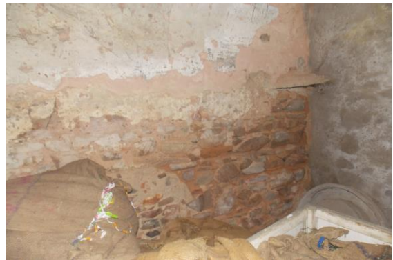
Photo 59 Dampness/Seepage of Room No. 4 of Ground Floor
