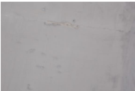
Photo 29 Horizontal Crack on Roof of Varanda of Shop No.206, Ground Floor Approx. Width = 0.15mm, Approx. Length = 2.5m. Distance from leftside External Column = 1.3m, Height from Floor = 3m.
