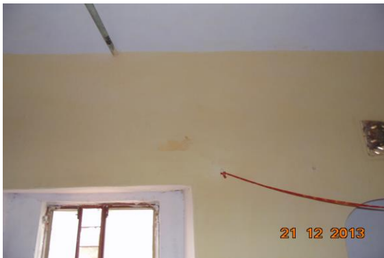
Photo 104 Peeling of Plaster on Wall No. 4 of Room No. 3 of Temple, Ground Floor
