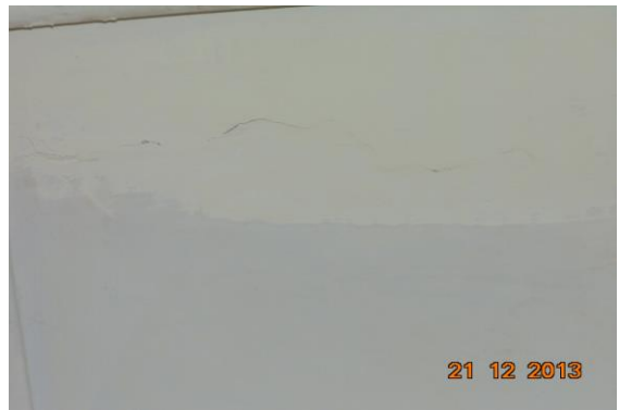
Photo 28 Inclined Crack on Roof of Varanda No.2, Library, Ground floor Approx. Width = 0.5mm, Approx. Length = 1m. Distance from = m, Height from Floor = m.
