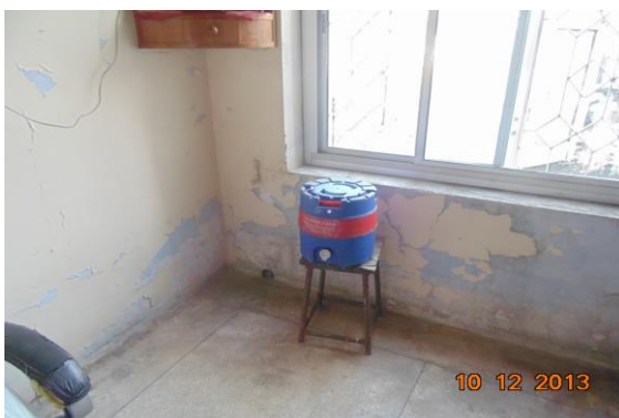
Photo 147 Peeling of Plaster on Wall No. 4 & 1 of Shop No.206 of Second Floor
