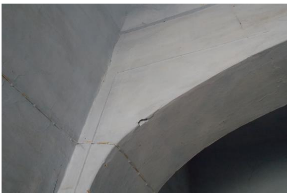
Photo 171 Peeling of Plaster on Roof of Lobby No.1 of Shri Krishna Chandra Ji Temple, First Floor
