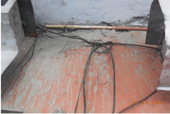
Photo 19 Peeling of Plaster on Wall No. 3 & Out of Side of Shop No. 311 of Ground Floor
