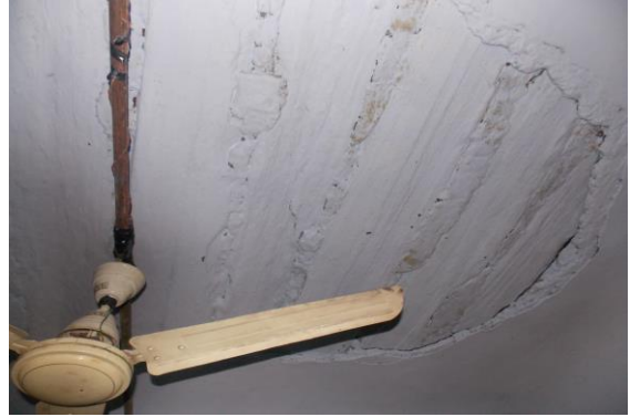
Photo 26 Dampness/Seepage on Roof of Room No. 2 of Temple, First Floor
