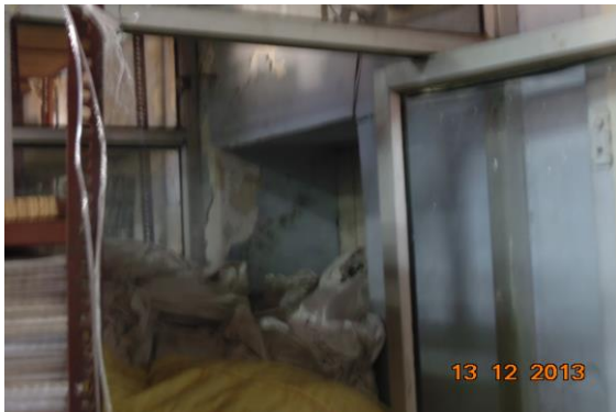
Photo 103 Peeling of Plaster on Roof of Room No. 4 of First Floor
