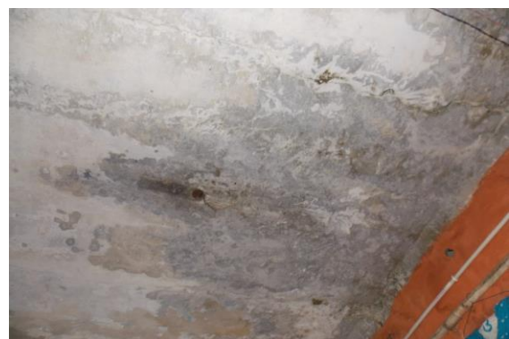
Photo 122 Dampness/Seepage on Roof of Varanda of Shop No.245 of Ground Floor
