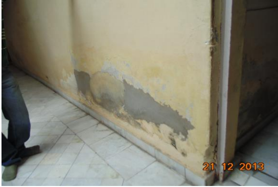
Photo 108 Peeling of Plaster on Wall No. 3 of Open Sky No.2 of Ground Floor
