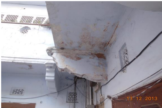
Photo 115 Dampness/Seepage on Roof of Balcony-3 of House No. 635, First Floor
