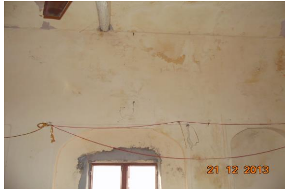
Photo 127 Dampness/Seepage on Wall No. 4 of Room No. 1 of Temple, Ground Floor
