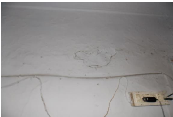
Photo 24 Peeling of Plaster on Roof of Room No. 1 of First Floor
