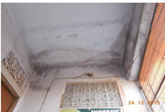
Photo 67 Dampness/Seepage on Roof of Lobby of House No.843,844 of Second Floor
