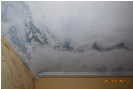
Photo 134 Dampness/Seepage on Roof of Room No. 4 of First Floor
