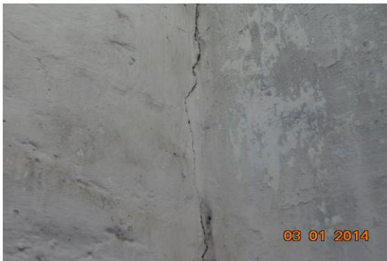
Photo 70 Plaster Crack on Wall No. 2 of Stair TF to Terrace of Third Floor - Part A
