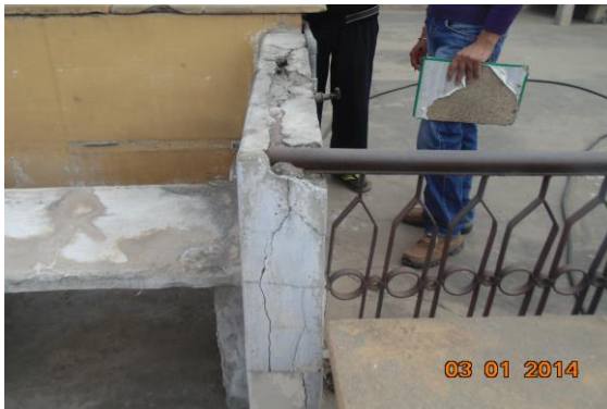
Photo 74 Peeling of Plaster on Tinshed Room of Terrace
