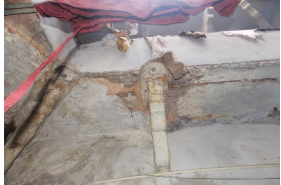
Photo 63 Dampness/Seepage of Sky open Sunshade of House No. 483, Ground Floor
