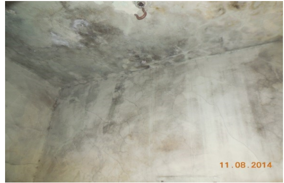
Photo 117 Seepage on All Walls & Roof of Toilet of Hind Hotel, Third Floor
