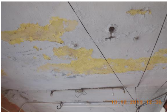
Photo 3 Dampness/Seepage on Roof of Varanda of Shop no.363 of Ground Floor
