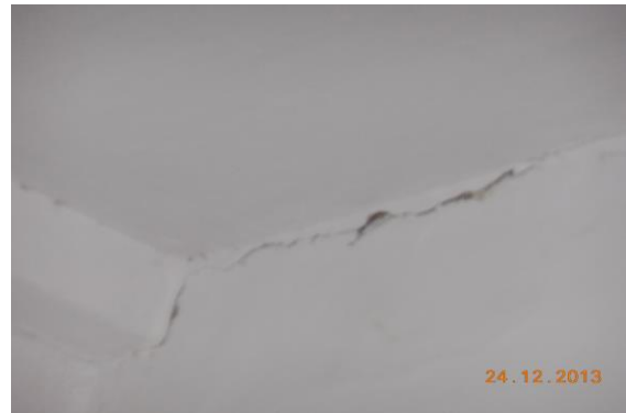
Photo 52 Dampness/Seepage on Roof of Hall No. 1 of First Floor
