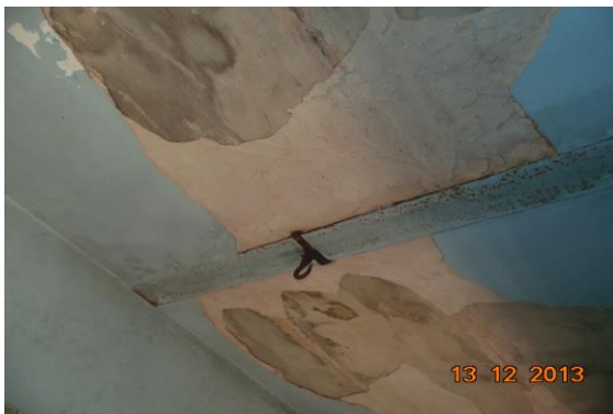
Photo 157 Peeling of Plaster on Roof of Room No. 12 of Second Floor
