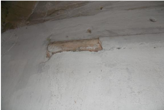
Photo 40 Peeling of Plaster on Wall No. 1 of Passage No.3 of First Floor
