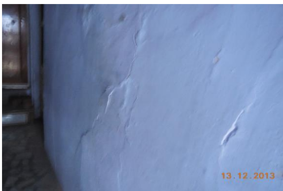
Photo 117 Peeling of Plaster on Roof of Passage-4 of House No. 635, First Floor
