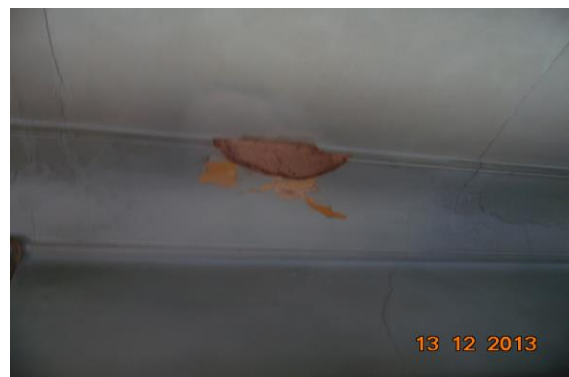
Photo 160 Peeling of Plaster on Roof of House No. 635 of Second Floor
