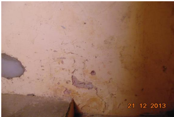
Photo 132 Peeling of Plaster on Wall No. 4 of Staircase of Ground Floor
