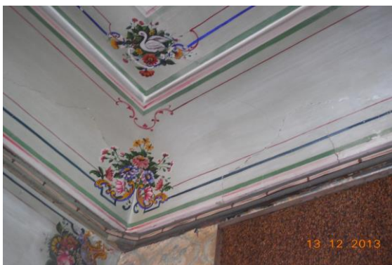
Photo 147 Peeling of Plaster on of House No. 635 of Second Floor
