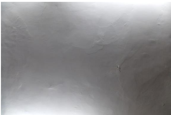
Photo 11 Plaster Crack on Roof of Part A of Shop No.236 of Ground Floor
