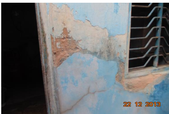
Photo 3 Inclined Crack on Wall No. 1 of Room No. 1, Second Floor Approx. Width = 0.6mm, Approx. Length = 2.5m. Distance from Wall No.1 = 0.7m, Height from Floor = 0m.
