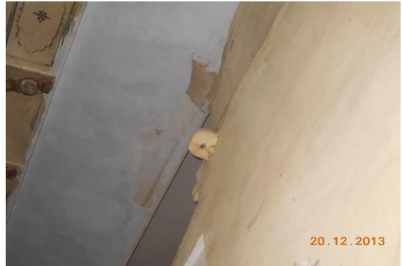
Photo 83 Peeling of Plaster on Roof of Varanda No.2 of Ground Floor
