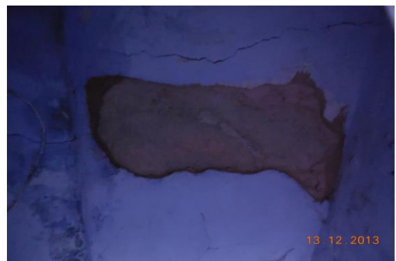
Photo 118 Peeling of Plaster on Roof of Passage-4 of House No. 635, First Floor
