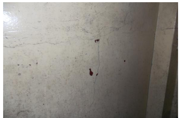
Photo 6 Inclined Crack on Wall No. 1 of Toilet No. 1, First Floor, Approx. Width = 0.3mm, Approx. Length = 0.5m. Distance from Wall No.3 = 2m, Height from Floor = 0.4m.
