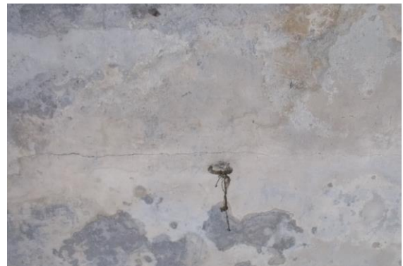
Photo 10 Horizontal Crack on Roof of Varanda of Shop No.275, Ground Floor, Approx. Width = 0.1mm, Approx. Length = 2.5m. Distance from Left External Column = 1.5m, Height from Floor = 3m.
