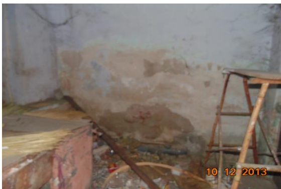
Photo 141 Peeling of Plaster on Wall No. 4 of Lobby of First Floor
