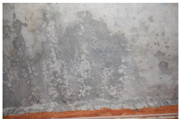
Photo 161 Dampness/Seepage on Roof of Varanda of Shop No.235 of Ground Floor
