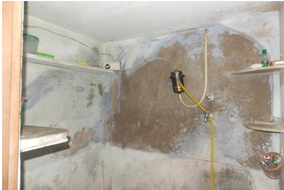
Photo 16 Dampness/Seepage on Bathroom of Ground Floor
