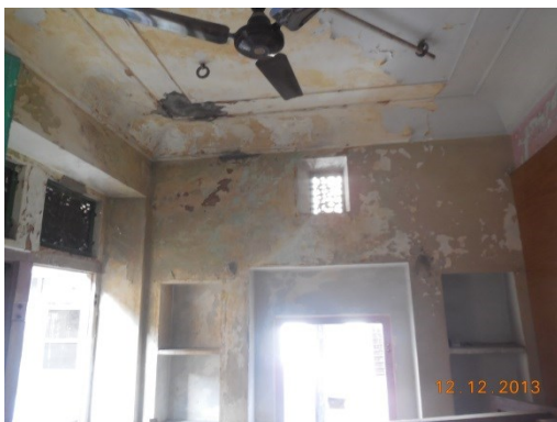
Photo 50 Seepage on Wall No.4,1 & Roof of Room 3 of H.No.481,First Floor
