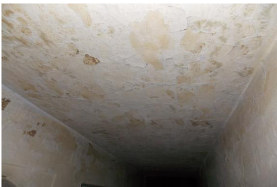
Photo 50 Dampness/Seepage on Roof of Passage No.8 of First Floor
