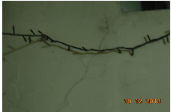
Photo 10 Inclined Crack on Wall No. 1 of Temple, First Floor, Approx. Width = 1mm, Approx. Length = 2m.
