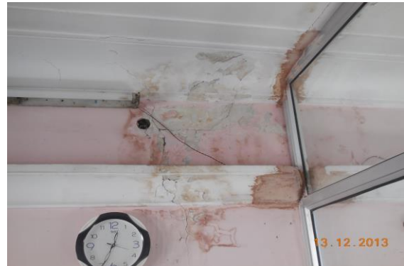
Photo 186 Peeling of Plaster on Wall No.2& Roof of Room No. 5 of Second Floor
