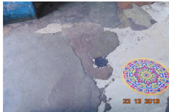
Photo 15 Peeling of Plaster on Floor of Lobby of First Floor
