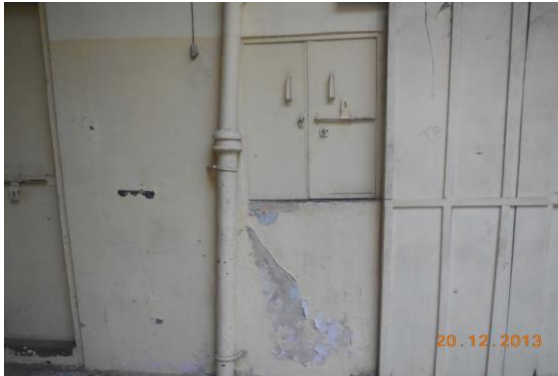
Photo 76 Peeling of Plaster on Wall No. 2 of Open sky of Ground Floor
