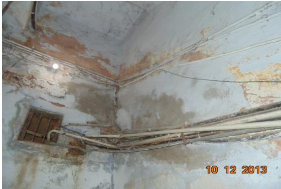
Photo 137 Dampness/Seepage on All Walls of Stair GF to FF of Ground Floor
