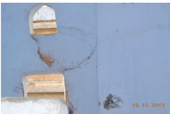
Photo 43 Peeling of Plaster on Wall No. 2 of Toilet & Washroom of Second Floor
