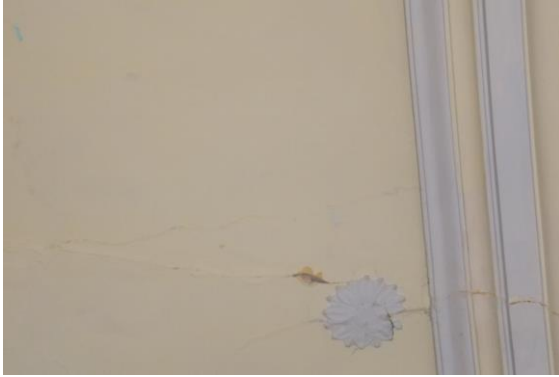
Photo 124 Peeling of Plaster on Roof of Hall No. 5 of Library, First Floor
