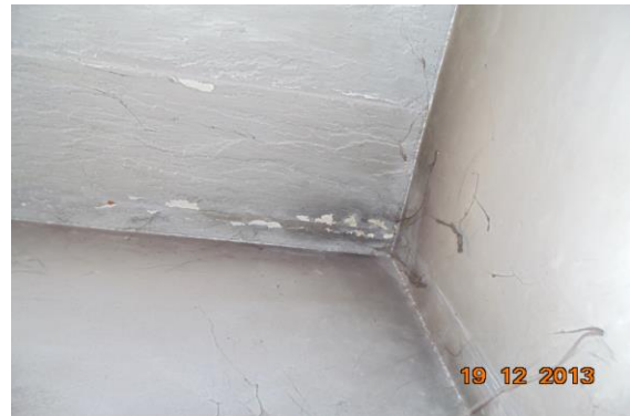
Photo 25 Peeling of Plaster on Roof of Staircase Second Floor To Third Floor of Terrace
