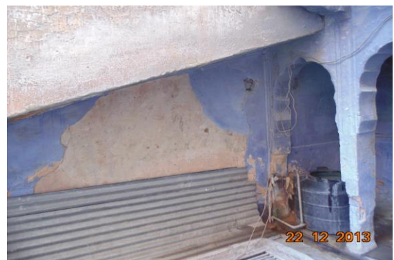
Photo 6 Peeling of Plaster on Wall No. 3 of Open Sky of First Floor
