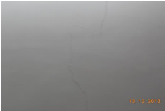
Photo 113 Plaster Crack on Roof of Room No. 2 of First Floor
