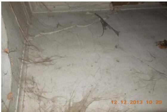
Photo 15 Inclined Crack on Wall No. 6 of Shop No. 3, Ground Floor, Approx. Width = 5mm, Approx. Length = 1.5m. Distance from w3 = 1.3m, Height from Floor = 2.2m.
