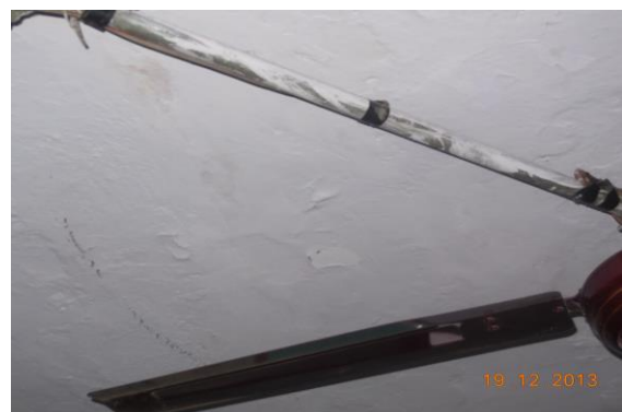
Photo 44 Peeling of Plaster on Roof of Room No. 1 of Second Floor
