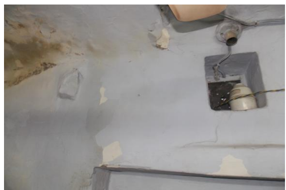
Photo 35 Peeling of Plaster on Wall No. 3 of Room No. 2 of First floor
