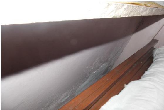
Photo 36 Dampness/Seepage on Room No. 4 of First Floor
