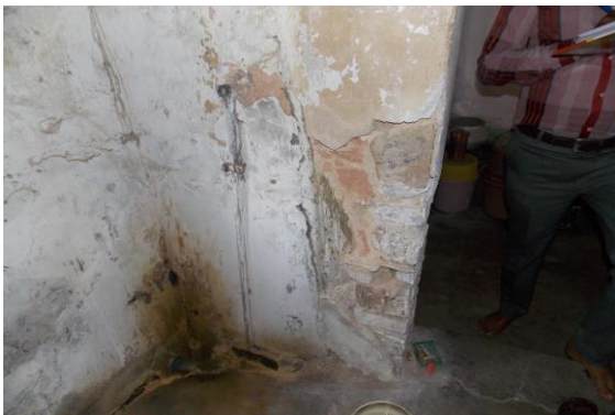
Photo 42 Peeling of Plaster on Wall No. 3 of Passage No.3 of First Floor
