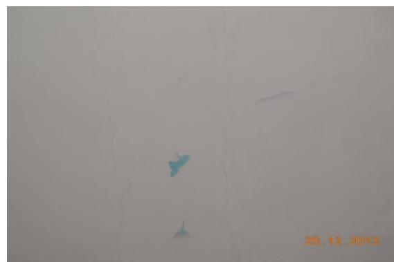
Photo 129 Peeling of Plaster on Roof of Hall No. 3 of Part A of Hall. First Floor
