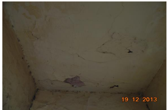
Photo 63 Peeling of Plaster on Roof of Staircase First Floor to Second Floor of First Floor
