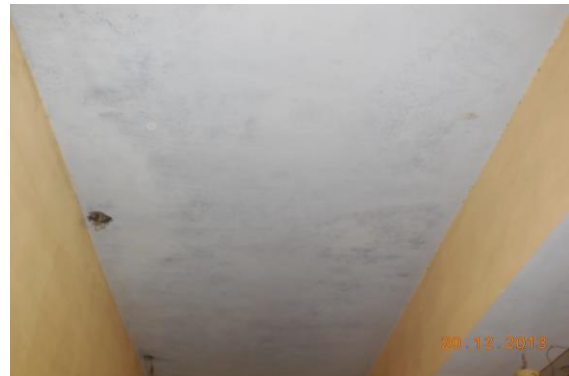
Photo 149 Dampness/Seepage on Roof of Hall No. 2 of Second Floor
