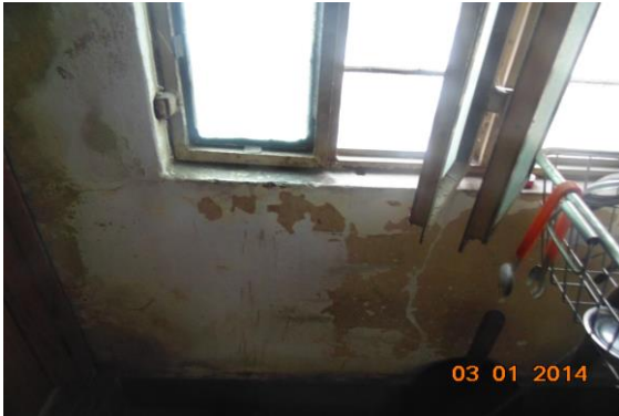
Photo 82 Peeling of Plaster on Roof of Kitchen of Second Floor - Part B
