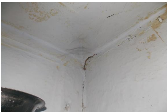
Photo 29 Peeling of Plaster on Wall No.3 & Roof of Kitchen of House No. 483, First Floor
