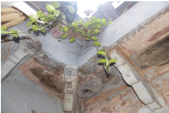
Photo 64 Dampness/Seepage of Sky open Sunshade of House No. 483, Ground Floor
