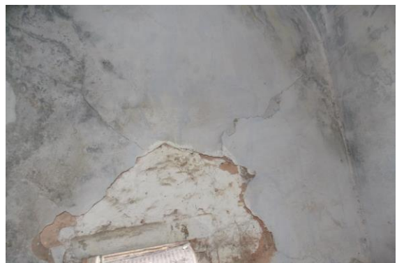
Photo 27 Peeling of Plaster on Wall No. 1 of Passage No.2 of First Floor
