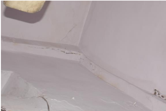
Photo 22 Peeling of Plaster on Roof of Shop No. 4 of Ground Floor
