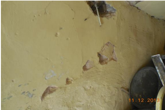
Photo 43 Peeling of Plaster on Wall No. 4 of Passage No.5 of First Floor
