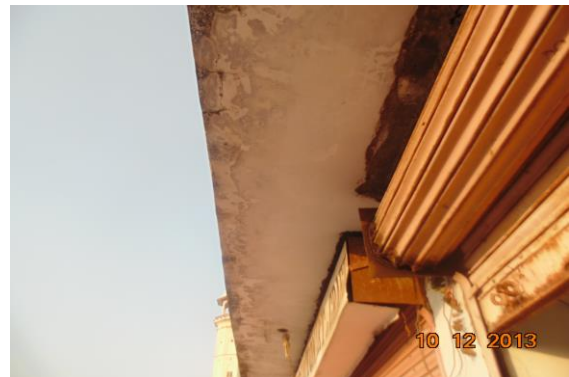
Photo 164 Dampness/Seepage on Shade Roof of Shop No.304 of Third Floor
