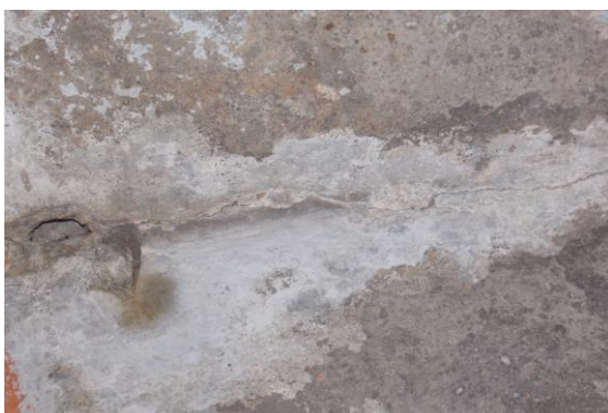
Photo 11 Horizontal Crack on Roof of Varanda of Shop No.195, Ground Floor Approx. Width = 1mm, Approx. Length = 2.5m. Distance from Leftside External Column = Backside, Height from Floor = 3m.
