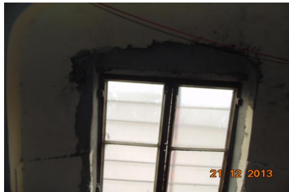
Photo 129 Peeling of Plaster on Wall No. 4 of Room No. 1 of Temple, Ground Floor
