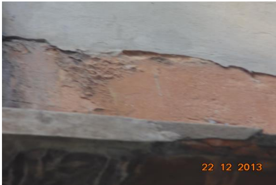
Photo 13 Peeling of Plaster on Outer Wall of External Façade H. No.476 of Second Floor
