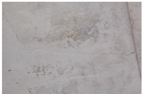
Photo 30 Inclined Crack on Roof of Varanda of Shop No.208, Ground Floor Approx. Width = 0.25mm, Approx. Length = 0.6m. Distance from External Beam = 1m, Height from Floor = 3m.
