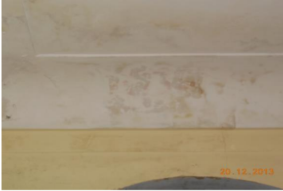
Photo 130 Dampness/Seepage on Roof of Hall No. 3 of Part A of Hall. First Floor
