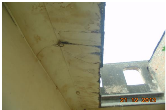
Photo 95 Peeling of Plaster on Wall No. 1 & Shade of Open Sky of Ground Floor
