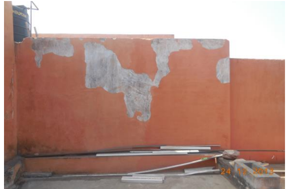
Photo 70 Peeling of Plaster on Wall No. 4 of Open Area of Second Floor
