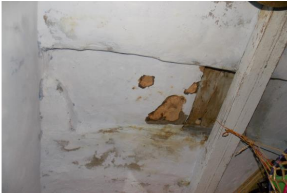
Photo 40 Peeling of Plaster on Roof of Room No. 5 of First Floor
