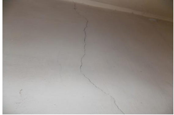
Photo 74 Inclined Crack on Wall No. 1 of Gallery No. 4, Second Floor Approx. Width = 0.6mm, Approx. Length = 2.1m. Distance from Wall no. 3 = 3.2m, Height from Floor = 0.7m.
