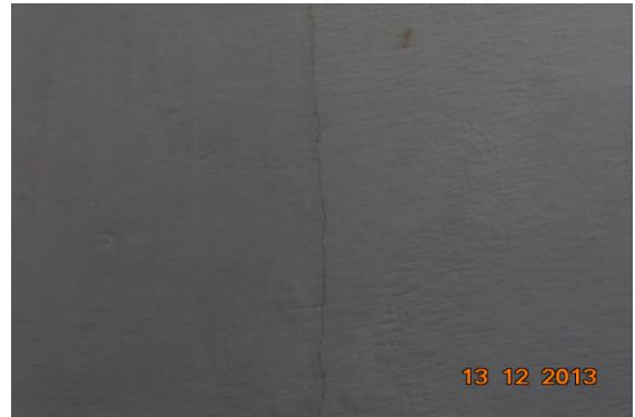
Photo 20 Vertical Crack of Hall No. 2, Ground Floor, Approx. Width = 0.3mm, Approx. Length = 1.5m. Distance from Wall No.3 = 1.5m, Height from Floor = 0m.
