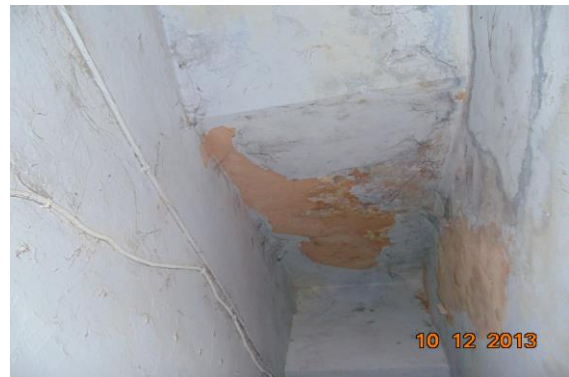
Photo 140 Peeling of Plaster on Roof of Stair GF to FF of Ground Floor
