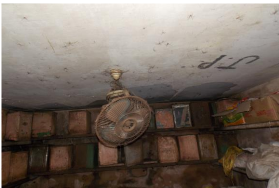
Photo 23 Peeling of Plaster on Roof of Shop No.196 of Basement
