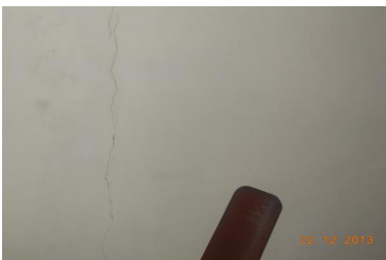
Photo 5 Horizontal Crack on Wall No. 1 & Roof of Room No. 1, House Above Shop No.270 & 271, First Floor Approx. Width = 0.35mm, Approx. Length = 2.9m. Distance from Wall No.1 = 1.6m, Height from Floor = 3m
