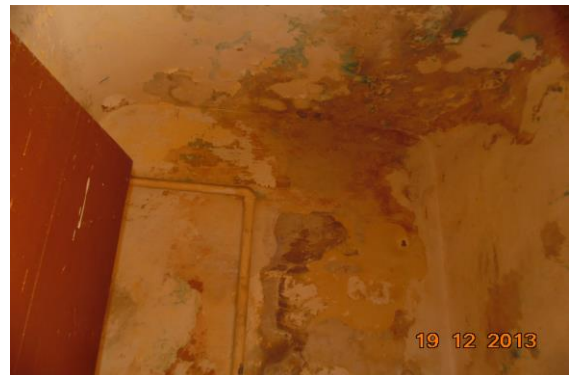
Photo 39 Dampness/Seepage on Wall No. 2, 4 & Roof of Toilet No. 1 of First Floor
