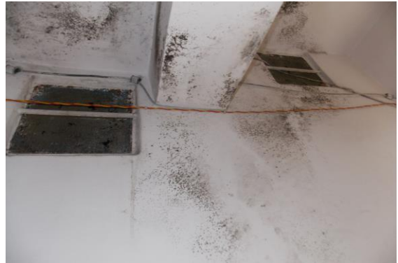
Photo 37 Dampness/Seepage on Wall No.4 & Roof of Staircase FF to SF of First floor
