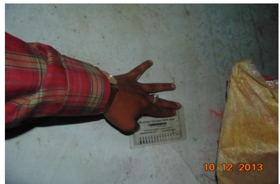
Photo 4A Inclined Crack on Wall No. 1 of Staircase FF to SF, Approx. Width = 0.2mm, Approx. Length = 0.8m. Distance from Wall No.3 = 1m, Height from Floor = 0m.
