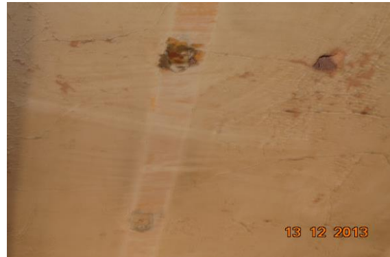
Photo 156 Dampness/Seepage on Roof of Room No. 11 of Second Floor
