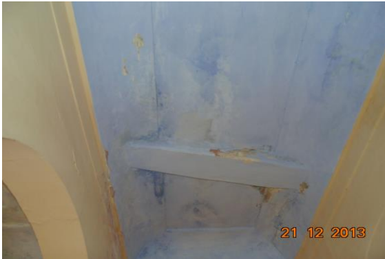
Photo 78 Dampness/Seepage on Roof of Varanda of Ground Floor
