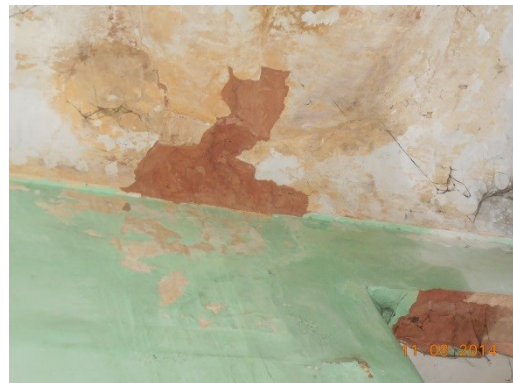
Photo 87 Plaster Crack on Roof of Varanda No. 4 of Hind Hotel,, First Floor
