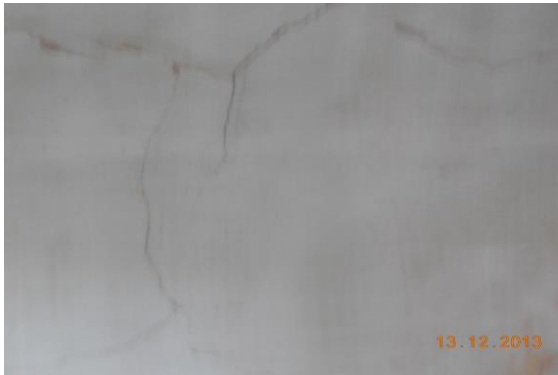
Photo 149 Plaster Crack on Room No. 3 of Second Floor
