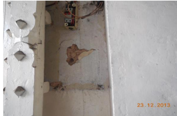
Photo 118 Peeling of Plaster on Wall No. 1 of Entrance of Ground Floor
