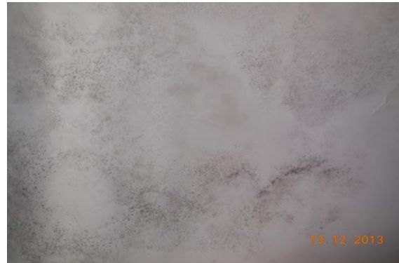
Photo 180 Dampness/Seepage on Roof of Lobby of House No. 635, Third Floor
