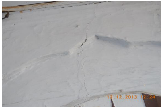
Photo 4 Inclined Crack on Open Sky, House No. 483, First Floor, Approx. Width = 0.4mm, Approx. Length = 0.9m. Distance from Wall No. 1 = 1m, Height from Floor = 2.2m.
