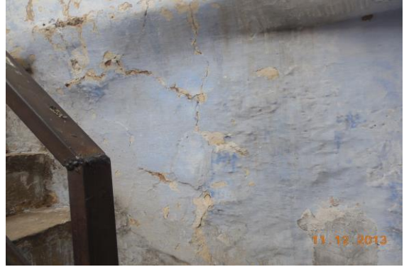
Photo 54 Plaster Crack on Wall No. 4 of Open Sky of First Floor
