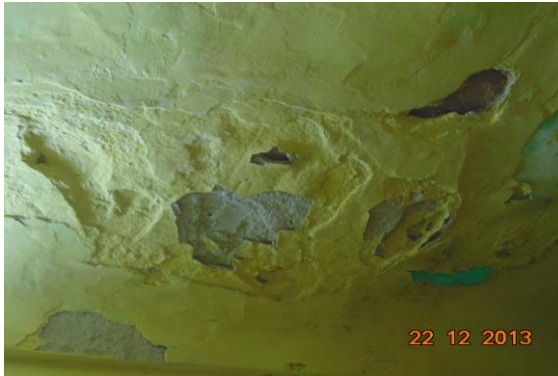
Photo 12 Peeling of Plaster on Roof of Room No. 2 of First Floor
