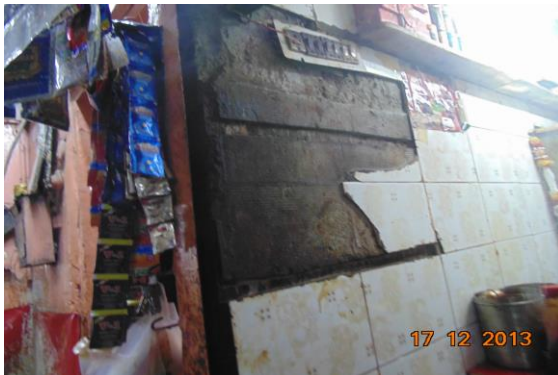
Photo 217 Peeling of Plaster on Wall No. 1 of Murali Pan Bhandar of Ground Floor
