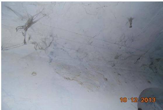
Photo 145 Dampness/Seepage on Wall No. 1 of Lobby of First Floor
