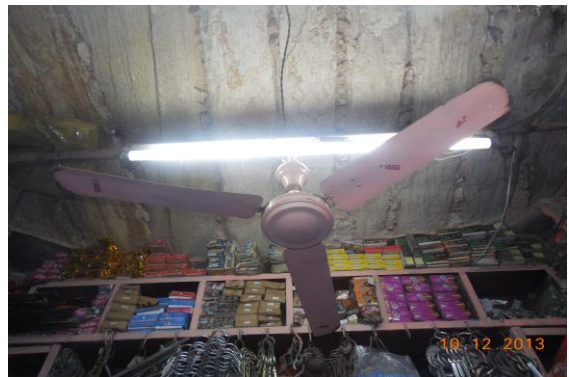
Photo 63 Peeling of Plaster on Roof of Shop No.307 of Ground Floor
