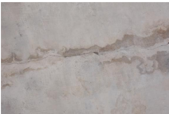
Photo 35 Horizontal Crack on Roof of Varanda of Shop No.264, Ground Floor. Approx. Width = 0.35mm, Approx. Length = 2.5m. Distance from Rightside External Column = 0.5m, Height from Floor = 3.5m.
