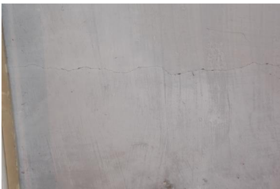
Photo 76 Horizontal Crack on Roof of Varanda of Shop No. 282, Ground Floor Approx. Width = 0.2mm, Approx. Length = 2.2m. Distance from Leftside External Column = 1.2m, Height from Floor = 3m.
