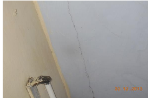
Photo 56 Inclined Crack on Roof of Room No. 8, First Floor Approx. Width = 0.5mm, Approx. Length = 3m.
