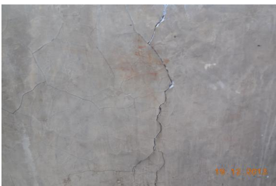
Photo 5 Inclined Crack on Wall No. 4 of Open Varanda No.1, Second Floor Approx. Width = 1.5mm, Approx. Length = 1m. Distance from Wall No.2 = 0.9m, Height from Floor = 0m.
