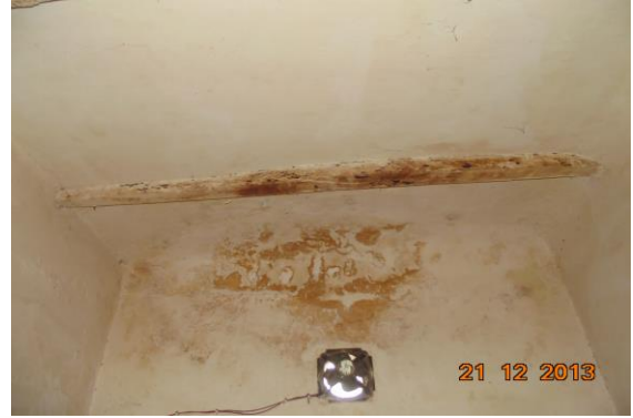
Photo 109 Dampness/Seepage on Wall No. 4 & roof of Room No. 2 of Temple, Ground Floor
