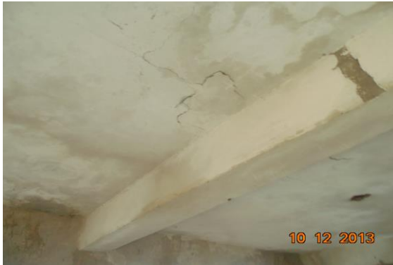
Photo 161 Peeling of Plaster on Roof of Shop No.305 of Third Floor
