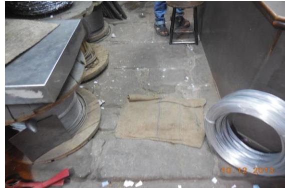
Photo 67 Peeling of Plaster on Floor of Shop No. 308 of Ground Floor
