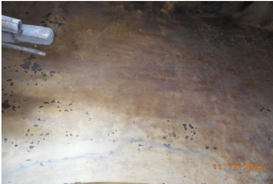
Photo 65 Dampness/Seepage on Wall No. 4 of Store No.1 of First Floor
