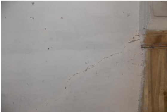
Photo 46 Peeling of Plaster on Wall No. 2 of Lobby No.1 of First Floor
