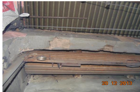
Photo 101 Peeling of Plaster on Roof of Shop of Ground Floor
