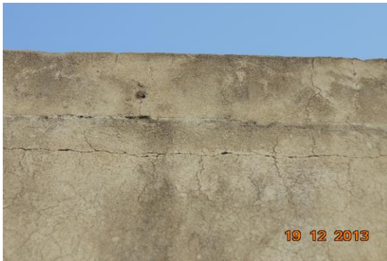
Photo 24 Peeling of Plaster on Shop Radha Gobind Enterprises of Terrace
