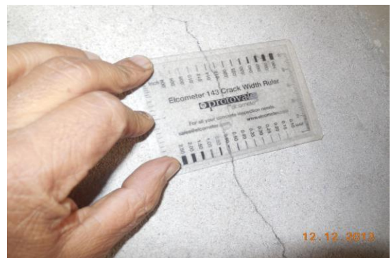
Photo 5A Inclined Crack on of Stair Case FF to SF, House No. 423, First Floor, Approx. Width = 0.6mm, Approx. Length = 1.3m. Distance from Wall No. 1 = 0.9m, Height from Floor = 1m.
