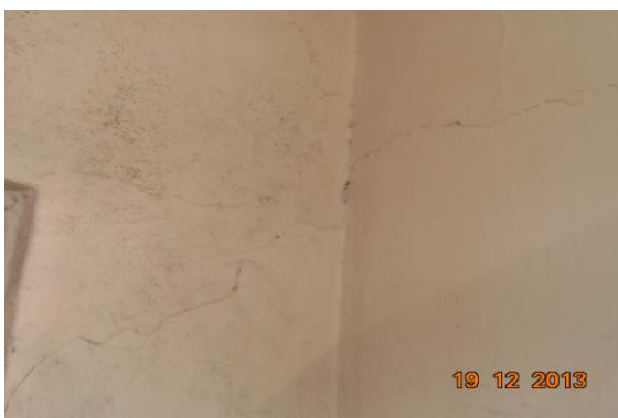
Photo 5 Inclined Crack on Wall No. 2 & 4 of Kitchen of House No.38, First Floor Approx. Width = 0.35mm, Approx. Length = 0.8m. Distance from Wall No.2 = 1.2m, Height from Floor = 1.5m.
