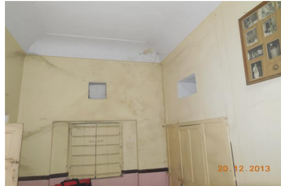
Photo 125 Dampness/Seepage on Wall No. 1 & Roof of Hall No. 3 of Part A of Hall. First Floor
