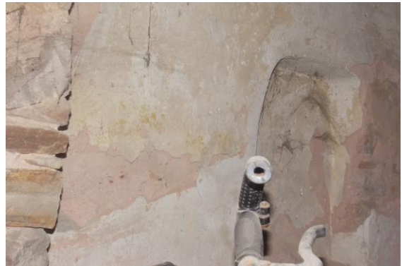
Photo 57 Dampness/Seepage of Room No. 1 & 2 of Ground Floor
