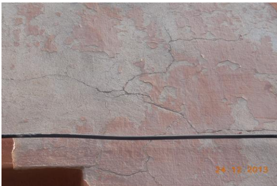
Photo 71 Peeling of Plaster on Wall No. 3 of Open Area of Second Floor
