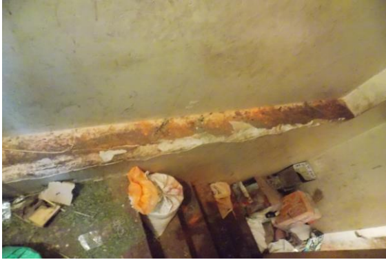
Photo 25 Peeling of Plaster on Wall No. 1 of Staircase of Basement
