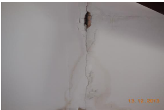
Photo 187 Peeling of Plaster on Roof of Room No. 5 of Second Floor
