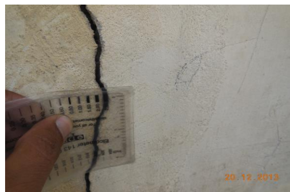
Photo 59A Inclined Crack on Wall No. 3 of Open Sky, Second Floor Approx. Width = 2.5mm, Approx. Length = 2m. Distance from Wall no.2 = 2.5m, Height from Floor = 0m.
