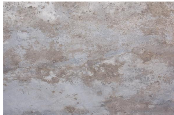
Photo 10 Horizontal Crack on Roof of Varanda of Shop no.195, Ground Floor Approx. Width = 1mm, Approx. Length = 2.5m. Distance from Rightside External Column = 1.05m, Height from Floor = 3m.
