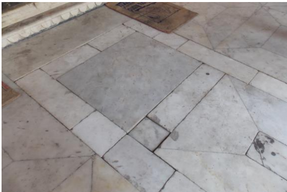
Photo 22 Dampness/Seepage on Floor of Vrand-2 of House No. 483, First Floor
