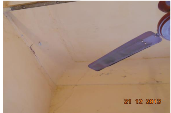
Photo 111 Peeling of Plaster on Roof of Room No. 5 of Temple, Ground Floor
