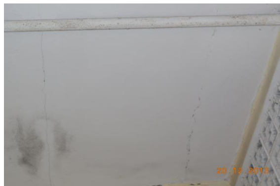
Photo 25 Inclined Crack on Roof of Room No. 1, First Floor Approx. Width = 0.8mm, Approx. Length = 2m.
