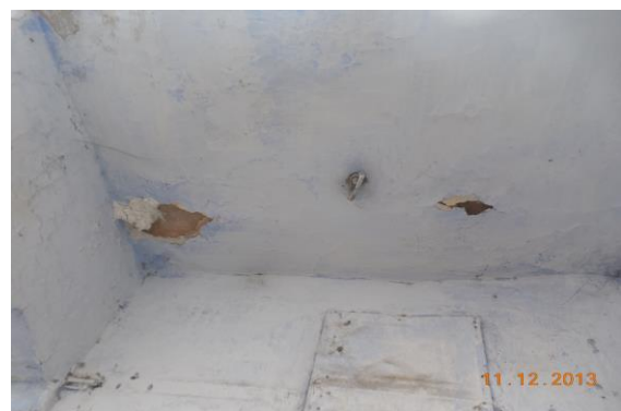
Photo 52 Peeling of Plaster on Wall No. 2 & Roof of Open Sky of First Floor
