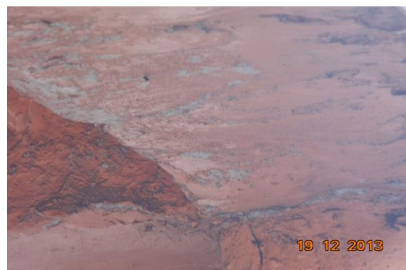
Photo 6 Dampness/Seepage on Beam of Temple of Ground Floor
