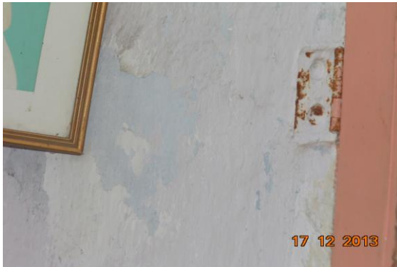
Photo 215 Peeling of Plaster on Wall No. 2 of Shop Ra Rafugar of Ground Floor
