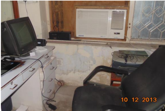
Photo 149 Peeling of Plaster on Wall No. 4 of Shop No.207 of Second Floor
