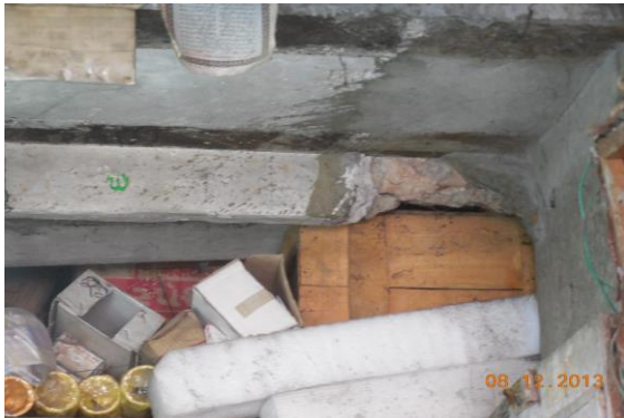
Photo 95 Damaged Portion on Roof of Shop No.370 of Ground Floor
