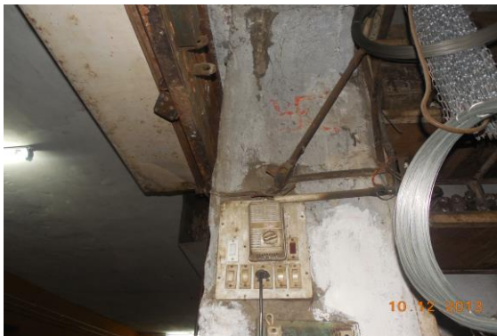
Photo 68 Peeling of Plaster on Roof of Part A of Shop No. 308, Ground Floor
