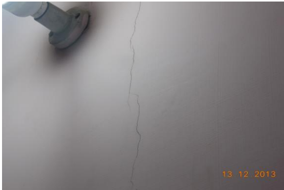
Photo 131 Plaster Crack on Beam of Passage of House No. 635, Second Floor
