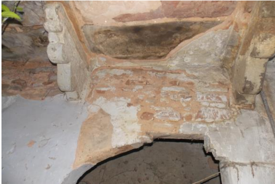
Photo 62 Dampness/Seepage of Sky open of House No. 483, Ground Floor
