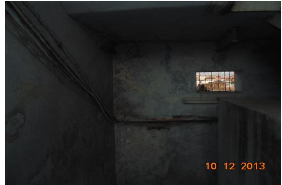
Photo 150 Dampness/Seepage on Wall No. 1, 2 & 4 of Staircase FF to SF of Second Floor
