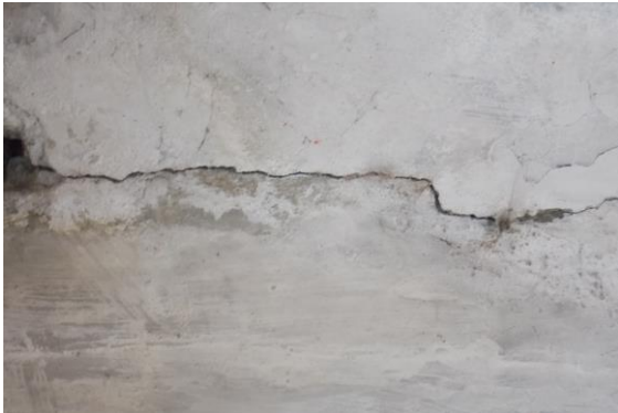
Photo 20 Horizontal Crack on Roof of Varanda of Shop No. 378, Ground Floor Approx. Width = 3mm, Approx. Length = 3m. Height from Floor = 3.3m.
