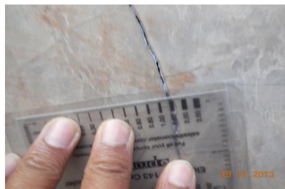
Photo 5A Inclined Crack on Wall No. 4 of Open Varanda No.1, Second Floor Approx. Width = 1.5mm, Approx. Length = 1m. Distance from Wall No.2 = 0.9m, Height from Floor = 0m.
