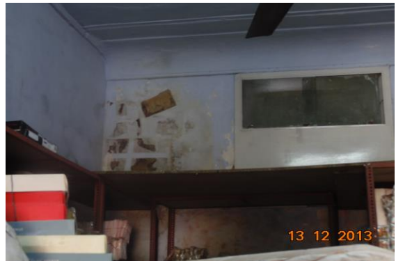
Photo 104 Dampness/Seepage on Roof of Room No. 4 of First Floor
