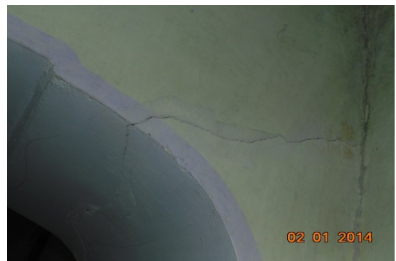
Photo 6 Inclined Crack on Wall No.4 of Varandah No.1 of Temple, First Floor, Approx. Width=1.0mm, Approx.Length= 1.0m. Distance from Wall No.2=0m, Height from Floor= 2.0m.
