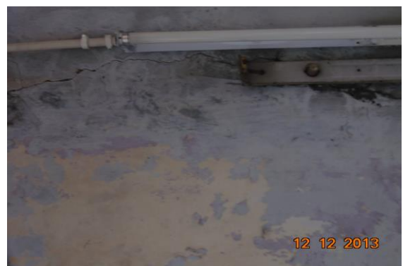
Photo 6 Horizontal Crack on Roof of Varanda , Shop No. 229, Ground Floor, Approx. Width = 2mm, Approx. Length = 2m.
