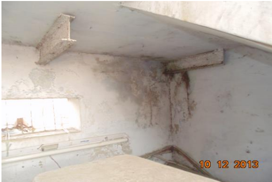
Photo 151 Dampness/Seepage on Wall No. 1, 2 & 4 of Staircase FF to SF of Second Floor
