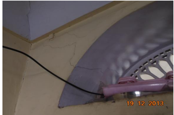
Photo 8 Inclined Crack on Wall No. 3 & Roof of Room No. 1, First Floor, Approx. Width = 1mm, Approx. Length = 3m.
