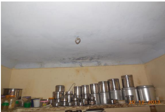
Photo 144 Dampness/Seepage on Roof of Kitchen of First Floor
