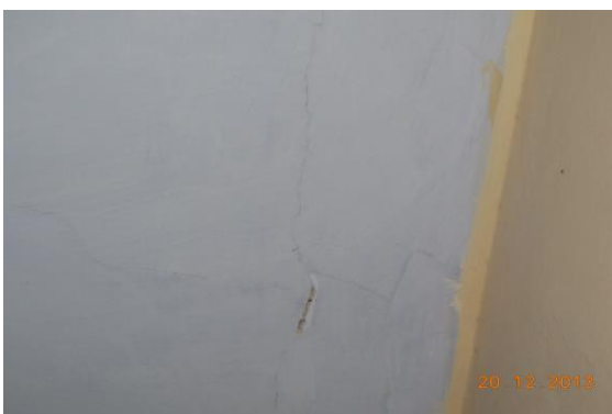
Photo 146 Peeling of Plaster on Roof of Room No. 8 of First Floor
