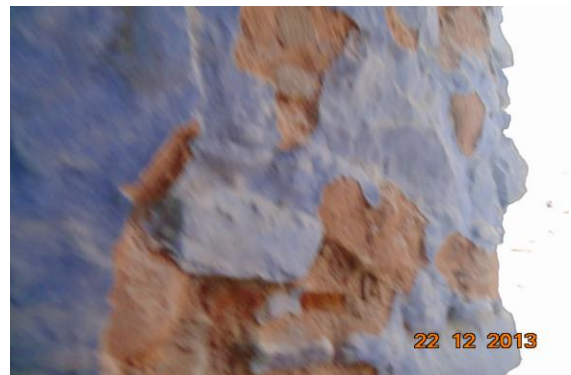
Photo 4 Peeling of Plaster on Wall No. 2 of Staircase GF to FF of Ground Floor
