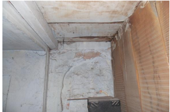
Photo 47 Peeling of Plaster on Wall No. 4 of Passage No.5 of First Floor
