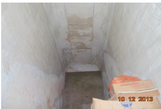
Photo 135 Dampness/Seepage on Wall No. 1 & Roof of Part-II of Shop No.31, Ground Floor
