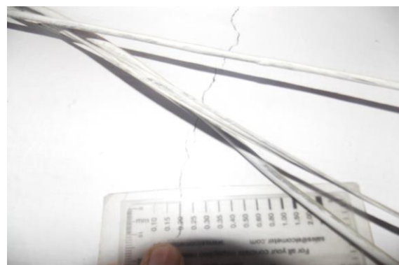
Photo 11A Inclined Crack on Wall No. 3 of Open sky Area, First Floor Approx. Width = 0.2mm, Approx. Length = 0.5m. Distance from Wall no.1 = 1.3m, Height from Floor = 1.7m.
