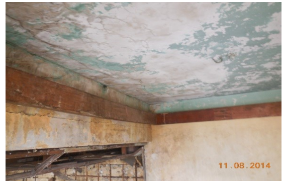
Photo 119 Seepage on Roof of Room No. 1 of Hind Hotel, Terrace
