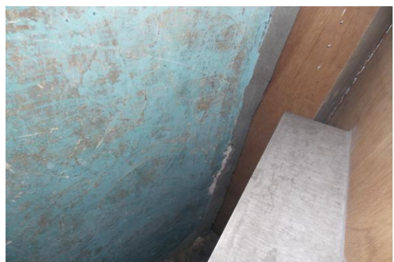
Photo 159 Peeling of Plaster on Wall No. 1 of Part B of Shop No.284 of Ground Floor
