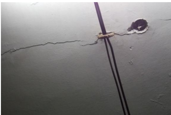
Photo 17 Horizontal Crack on Roof of Varanda of Shop No.328 & 329, Ground Floor, Approx. Width = 1mm, Approx. Length = 3m. Distance from = Backside Rightside external Columnn, Height from Floor = 3m
