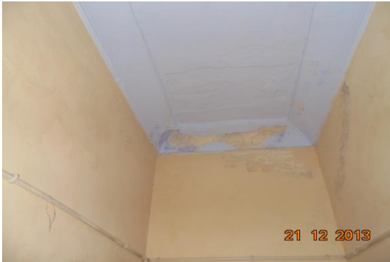
Photo 90 Peeling of Plaster on Roof of Passage No.2 of Ground Floor
