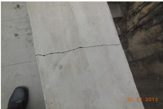
Photo 57 Inclined Crack on Perapet wall of Staircase, Second Floor Approx. Width = 1mm, Approx. Length = 1m.
