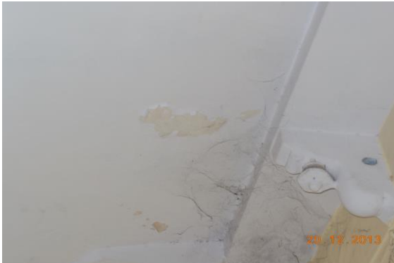
Photo 84 Damaged Portion on Shade of Varanda No.2 of Ground Floor
