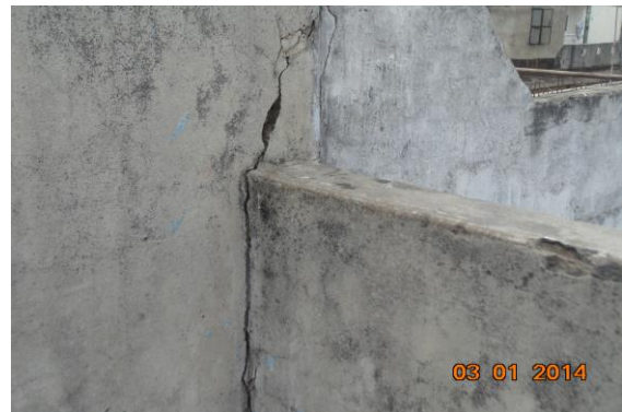
Photo 71 Plaster Crack on Third Floor - Part A
