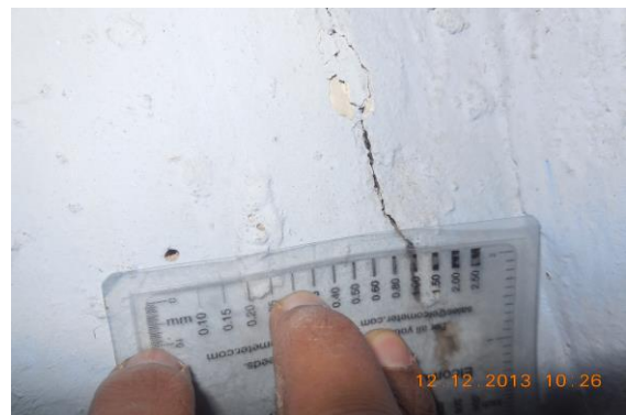
Photo 17A Inclined Crack on Wall No. 4 of Lobby, House No. 651, Ground Floor, Approx. Width = 1mm, Approx. Length = 0.4m. Distance from W2 = 0.03m, Height from Floor = 1.1m.
