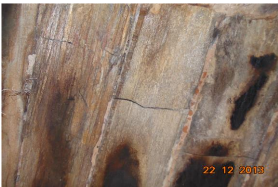
Photo 5 Inclined Crack on Roof of Varanda of H.No.156, Ground Floor Approx. Width = 2.5mm, Approx. Length = 1m. Distance from = m, Height from Floor = m.
