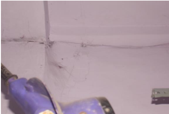
Photo 156 Plaster Crack on Wall No. 2 of Shop No.238 of Ground Floor
