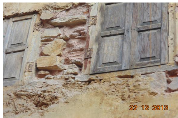
Photo 12 Peeling of Plaster on Outer Wall of Building of Ground Floor
