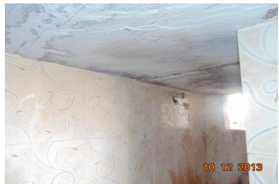
Photo 160 Dampness/Seepage on Roof of Toilet No. 1 of Second Floor
