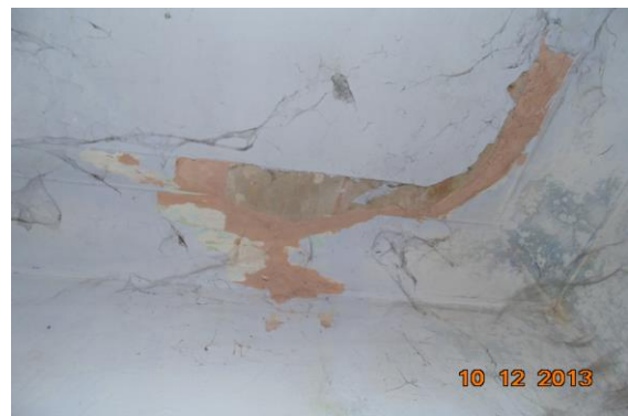
Photo 142 Peeling of Plaster on Roof of Lobby of First Floor
