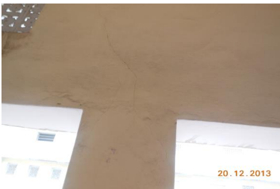
Photo 24 Inclined Crack on Wall No. 4 of Room No. 1, First Floor Approx. Width = 0.5mm, Approx. Length = 1m. Distance from Wall no.2 = 3m, Height from Floor = 1.6m.
