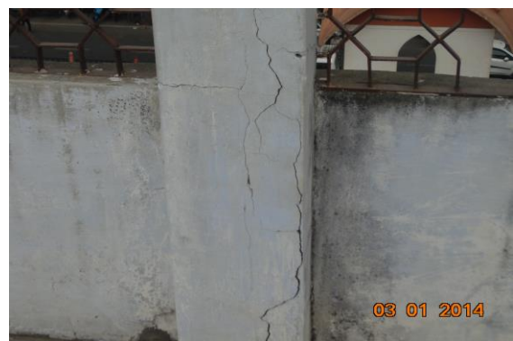
Photo 73 Plaster Crack on Wall No. 3 & 5 of Terrace
