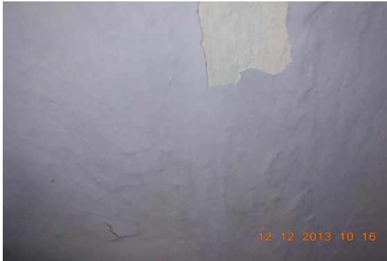
Photo 42 Peeling of Plaster on Roof of Shop No. 2 of Ground Floor
