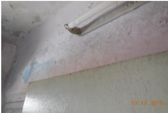
Photo 179 Dampness/Seepage on Roof of Toilet No. 1 of Third Floor
