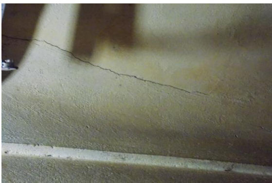
Photo 22 Horizontal Crack on Wall No. 3 of Part B of Shop No.377, Ground Floor Approx. Width = 1.5mm, Approx. Length = 1.5m. Distance from Wall No.1 = 0m, Height from Floor = 3m.
