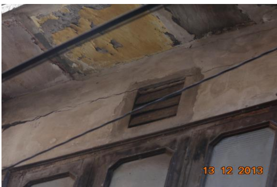
Photo 93 Peeling of Plaster on Front Side Wall of External Façade of House No. 635, First Floor
