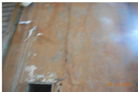
Photo 23 Inclined Crack on Wall No. 3 & Outer wall of Shop of Varanda, Shop No. 304, G. F., Approx. Width = 0.35mm, Approx. Length = 1.5m. Distance from Main Door = 0.4m, Height from Floor = 1.5m.
