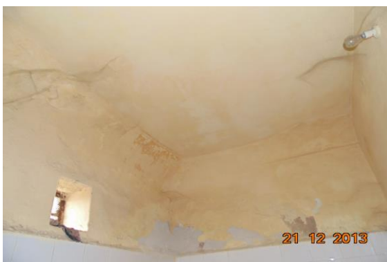
Photo 106 Dampness/Seepage on Wall No. 2, 4 & Roof of Toilet No. 1 of Temple, Ground Floor
