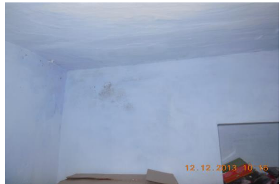
Photo 45 Dampness/Seepage on Wall No. 1 of Shop No. 2 of Ground Floor
