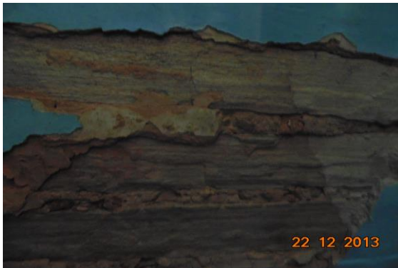
Photo 6 Peeling of Plaster on Roof of Room No. 3 of First Floor
