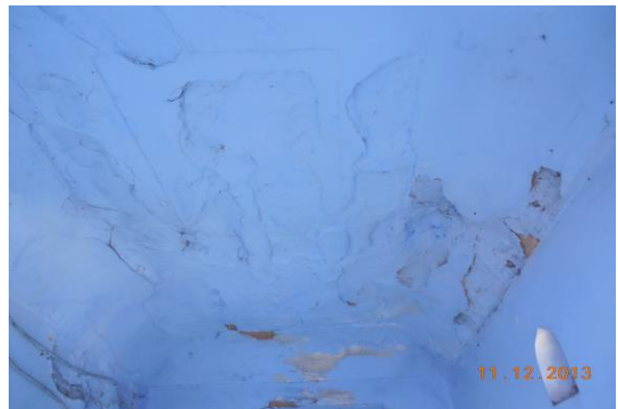
Photo 32 Peeling of Plaster on Roof of Passage No.2 of First Floor
