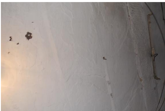
Photo 35 Peeling of Plaster on Roof of Varanda of Shop No.323 of Ground Floor
