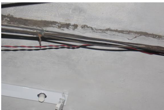
Photo 5 Horizontal Crack on Roof of Varanda of Shop No.235, Ground Floor, Approx. Width = 2mm, Approx. Length = 2.5m. Distance from Left side External Column = Backside, Height from Floor = 3m.
