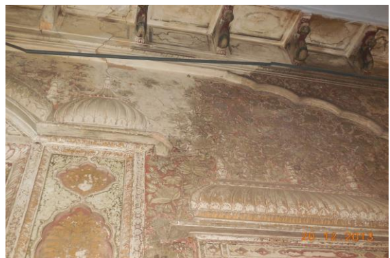
Photo 87 Peeling of Plaster on Frontside Wall of Temple of Ground Floor
