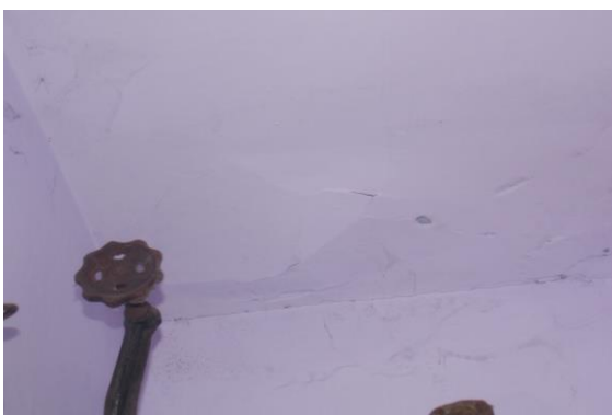
Photo 83 Peeling of Plaster on Roof of Shop No. 2 of Ground Floor
