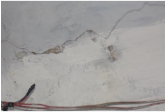
Photo 34 Dampness/Seepage on Wall No. 1 of Temple No.1 of First Floor
