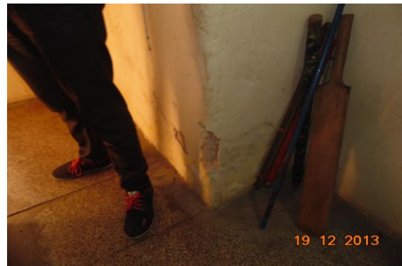
Photo 45 Peeling of Plaster on Wall No. 3 of Lobby of First Floor
