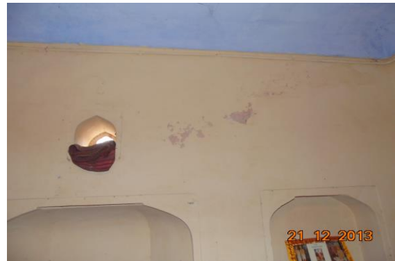
Photo 121 Dampness/Seepage on Wall No. 4 of Room No. 7 of Temple, Ground Floor
