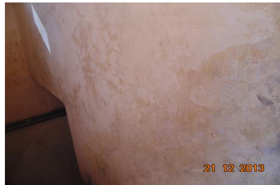
Photo 135 Dampness/Seepage on Wall No. 1 of Staircase of Ground Floor
