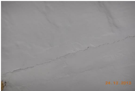
Photo 51 Peeling of Plaster on Wall No. 2 of Room No. 7 of First Floor
