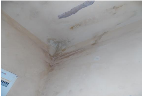
Photo 138 Dampness/Seepage on Wall No. 2, 3 & Roof of Hall No. 8 of Library, First Floor
