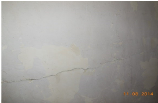
Photo 108 Peeling of Plaster on Wall No. 6 of Room No. 13 of Hind Hotel, Second Floor
