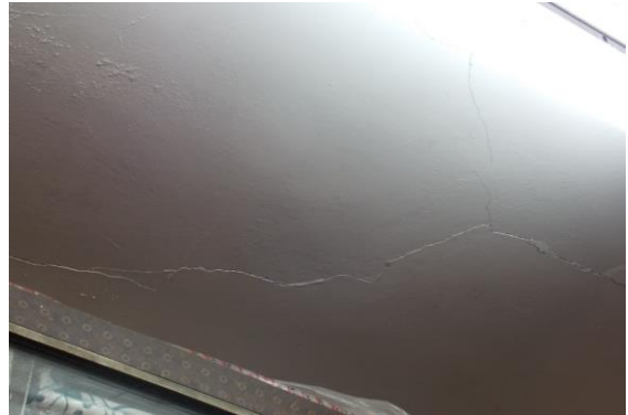
Photo 8 Peeling of Plaster on Roof of Shop No.332 of Ground Floor
