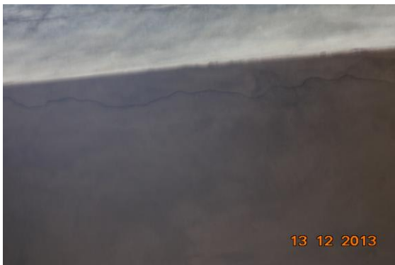
Photo 21 Horizontal Crack on Shade of House No. 635, Third Floor, Approx. Width = 1.5mm, Approx. Length = 3m. Distance from Back Side Wall = 5.3m, Height from Floor = 12m.
