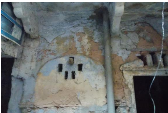
Photo 60 Dampness/Seepage of Sky open of House No. 483, Ground Floor
