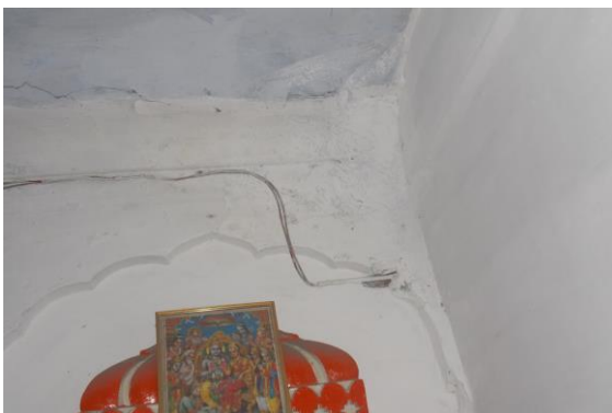
Photo 32 Peeling of Plaster on Wall No. 2 & 3 of Room No. 4 of First Floor
