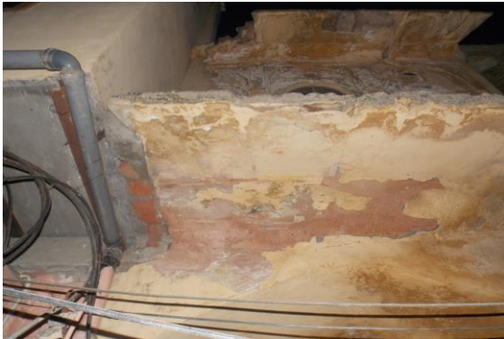
Photo 82 Peeling of Plaster on Front Side Wall of External Façade
