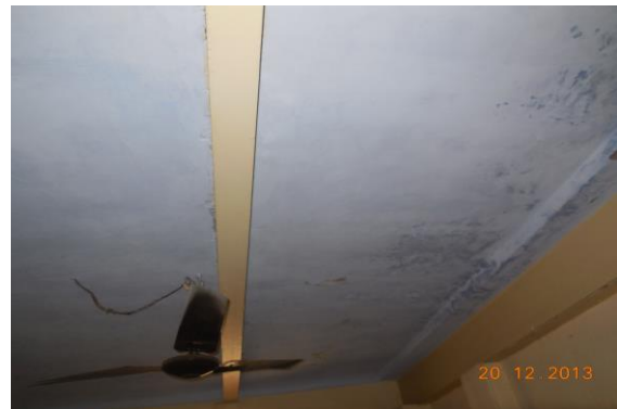
Photo 139 Dampness/Seepage on Roof of Room No. 5 of First Floor
