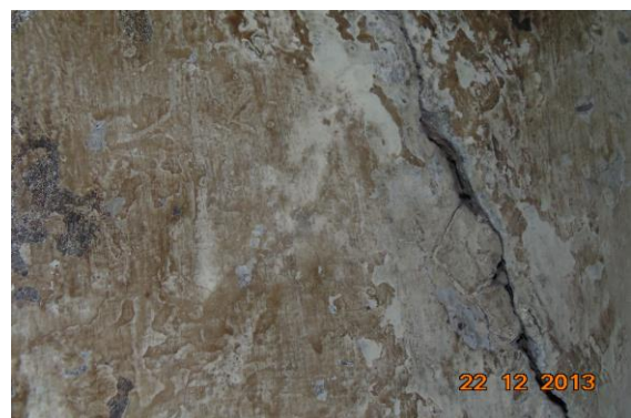
Photo 17 Peeling of Plaster on Wall No. 1 of Staircase FF to SF of First Floor
