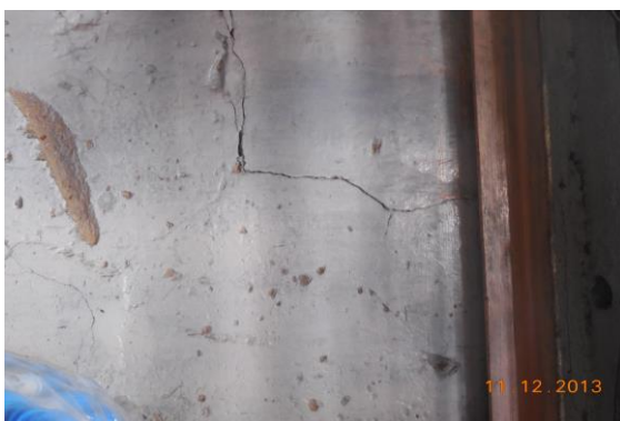
Photo 5 Inclined Crack on Wall No. 2 of Shop No. 310, Ground Floor Approx. Width = 1mm, Approx. Length = 0.5m. Distance from Gate = 0.35m, Height from Floor = 1.7m.
