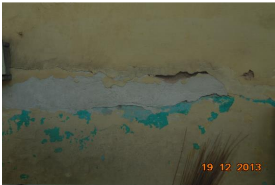
Photo 50 Peeling of Plaster on Wall No. 3 of Open Sky Area of First Floor
