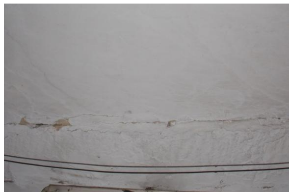
Photo 36 Exposed Reinforcement on Roof of Varanda of Shop No.323 of Ground Floor
