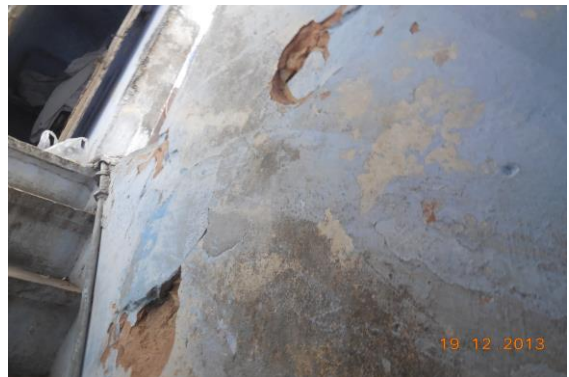
Photo 36 Peeling of Plaster on Wall No. 2 of Staircase First Floor To Second Floor of First Floor
