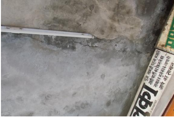
Photo 18 Horizontal Crack on Column & Between Shop No.379 & 378 of Varanda of Shop No.379, Ground Floor Approx. Width = 1.5mm, Approx. Length = 3m. Distance from Backside Right Column = 0m, Height from Floor = 3.3m.
