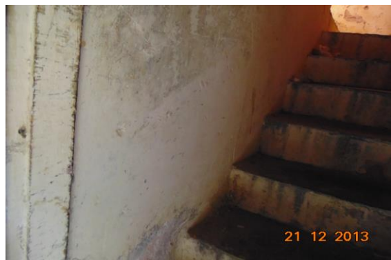
Photo 131 Dampness/Seepage on Wall No. 1 of Staircase of Ground Floor
