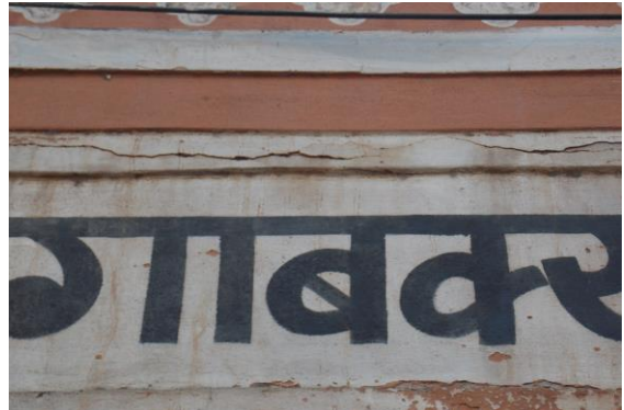
Photo 21 Horizontal Crack on Leftside Column outside of Shop No.377, Ground Floor Approx. Width = 5mm, Approx. Length = 4.5m. Between left & Right Side Column, Height from Floor = 3.3m.
