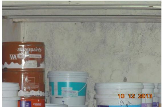
Photo 132 Dampness/Seepage on Wall No. 4 of Shop No.25 of Ground Floor
