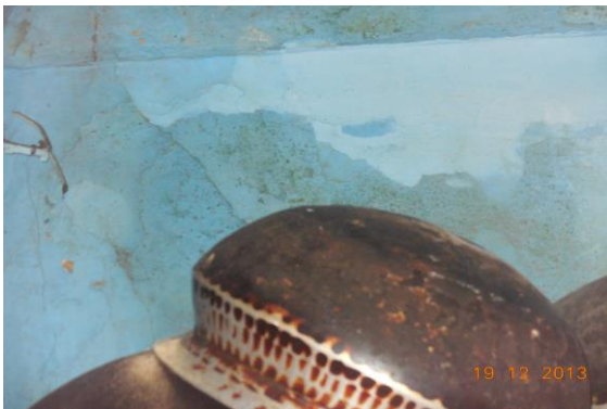
Photo 41 Dampness/Seepage on Wall No. 1 of Bilding Uday Singh Ji Ki Haveli of Second Floor
