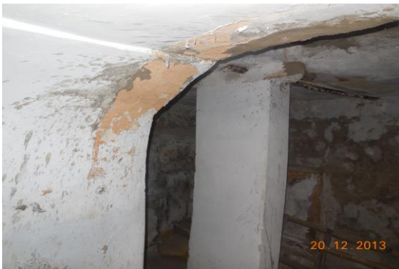
Photo 104 Dampness/Seepage on Outside Wall no.3 of Hall No. 6 of Basement
