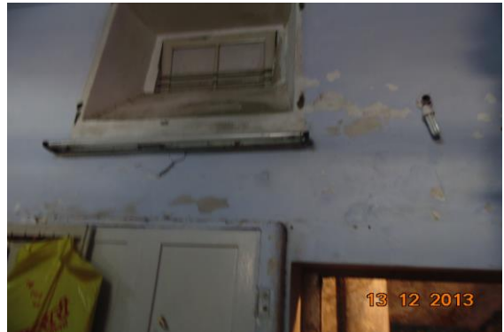
Photo 102 Peeling of Plaster on Roof of Room No. 4 of First Floor
