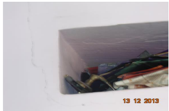
Photo 22 Inclined Crack on Roof of Room No. 3, Second Floor, Approx. Width = 0.15mm, Approx. Length = 1.8m. Distance from Wall No.4 = 2.2m, Height from Floor = 2m.
