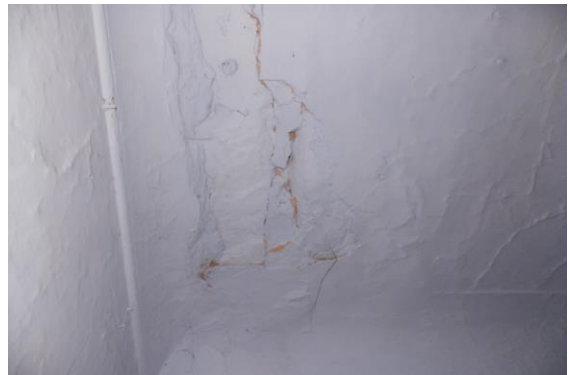
Photo 23 Peeling of Plaster on Roof of Room No. 1 of First Floor
