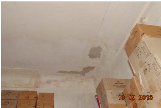
Photo 133 Dampness/Seepage on Wall No. 4 & Roof of Shop No.29 of Ground Floor
