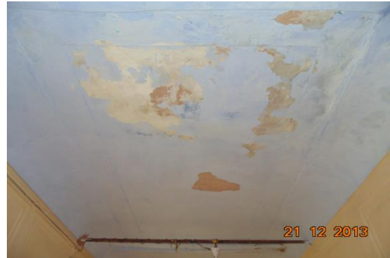
Photo 79 Dampness/Seepage on Roof of Varanda of Ground Floor
