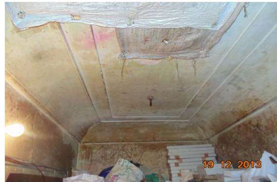
Photo 218 Dampness/Seepage on Wall No. 1, 2 & 4 of Shop Pink city Colour of Upper Ground Floor
