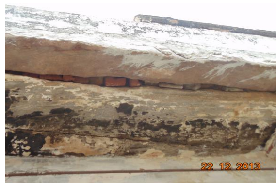
Photo 6 Inclined Crack on Wall No. 4 & Roof of , Ground Floor Approx. Width = 2mm, Approx. Length = 3m. Distance from = m, Height from Floor = m.
