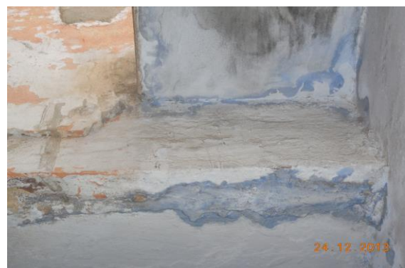
Photo 56 Peeling of Plaster on Wall No. 1 of Passage of First Floor
