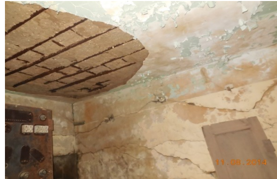
Photo 121 Damage on Shade of Room No. 1 of Hind Hotel, Terrace
