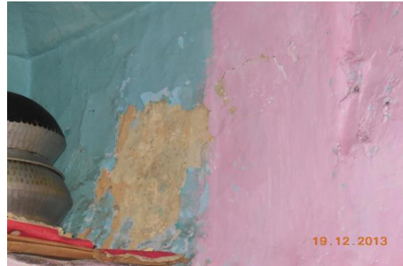
Photo 40 Peeling of Plaster on Wall No. 4 of Bilding Uday Singh Ji Ki Haveli of Second Floor
