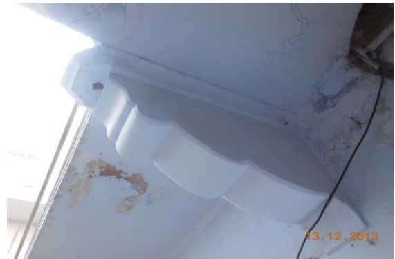
Photo 116 Peeling of Plaster on Roof of Balcony-3 of House No. 635, First Floor
