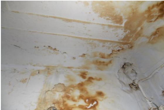
Photo 27 Dampness/Seepage on Wall No. 2 & Roof of Kitchen of House No. 483, First Floor
