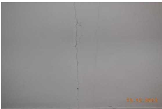
Photo 189 Damaged Portion on Roof of Room No. 5 of Second Floor
