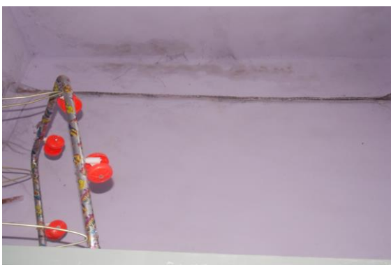
Photo 154 Dampness/Seepage on Wall No. 1 of Shop No.238 of Ground Floor
