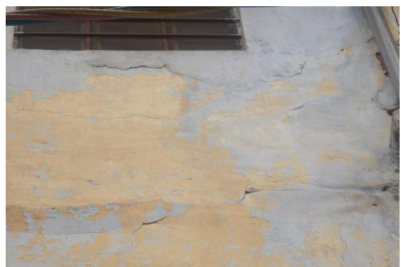
Photo 71 Peeling of Plaster on Front side Wall of House no.410 of Ground Floor
