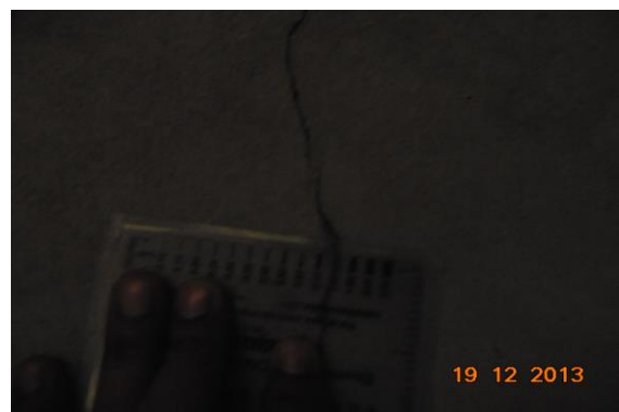
Photo 11A Inclined Crack on Wall No. 2 of Part B of Shop Shyam Store, Ground Floor Approx. Width = 1mm, Approx. Length = 1m. Distance from Wall No.4 = 1.5m, Height from Floor = 0.7m.
