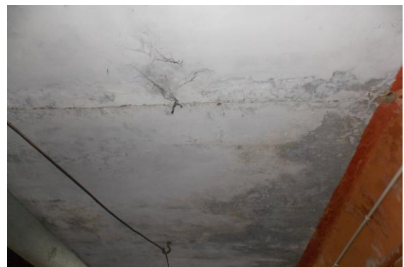
Photo 18 Horizontal Crack on Shop No.330, Ground Floor, Approx. Width = 2mm, Approx. Length = 3m. Distance from = Backside Rightside external Columnn, Height from Floor = 3m
