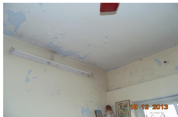
Photo 148 Peeling of Plaster on Wall No. 1, 4 & Roof of Shop No.206 of Second Floor
