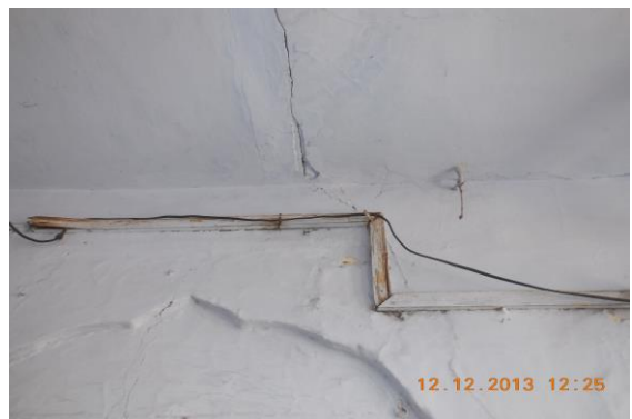
Photo 6 Inclined Crack on Wall No.4 & Sunshade of Open Sky, House No. 483, First Floor Approx. Width = 5mm, Approx. Length = 2.5m. Distance from w1 = 1.6m, Height from Floor = 2.5m.
