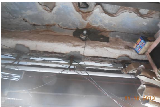
Photo 23 Peeling of Plaster on Wall No. 3 of Shop No. 312 of Ground Floor
