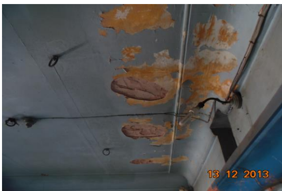
Photo 159 Peeling of Plaster on Roof of Room No. 13 of Second Floor
