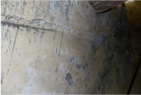
Photo 27 Peeling of Plaster on Wall No. 1 of Staircase
