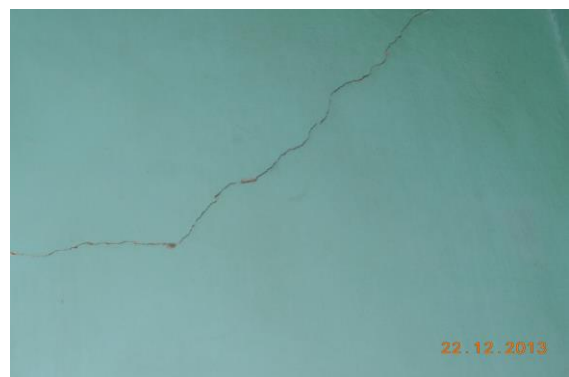
Photo 6 Inclined Crack on Wall No. 4 of Kitchen, House Above Shop No.270 & 271, First Floor Approx. Width = 1.5mm, Approx. Length = 1.2m. Distance from = m, Height from Floor = 2.5m.
