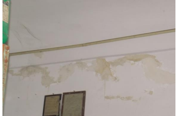
Photo 109 Dampness/Seepage on Wall No. 4 of Shop No.6 of Ground Floor
