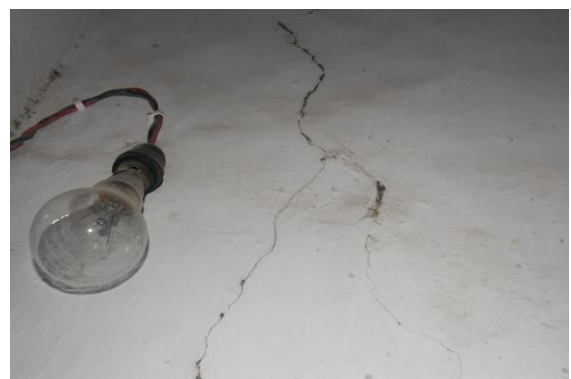
Photo 6 Inclined Crack on Stair Case GF to FF, Ground Floor, Approx. Width = 0.4mm, Approx. Length = 1.7m. Distance from W2 = 0.4m, Height from Floor = 1m.
