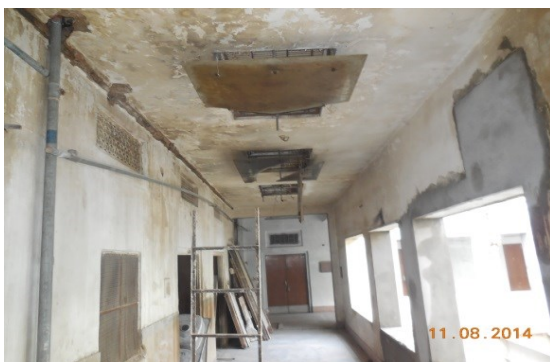
Photo 112 Seepage on All Walls of Varanda No. 2 of Hind Hotel, Second Floor
