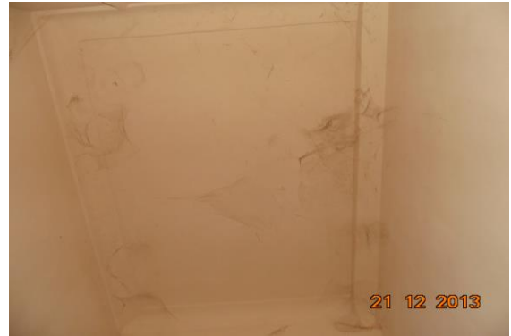
Photo 101 Dampness/Seepage on Roof of Toilet No. 3 of Library, Ground floor
