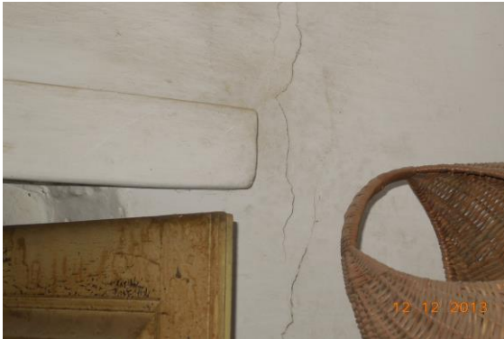
Photo 39 Plaster Crack on Roof of Kitchen of House No. 423, First Floor
