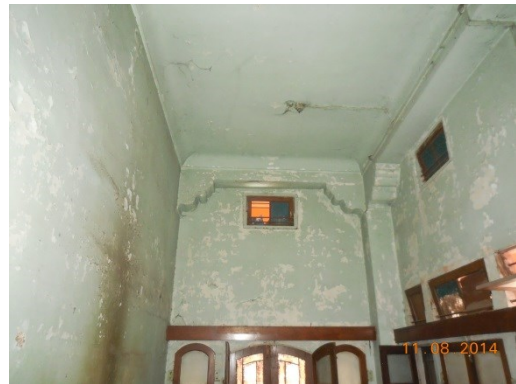
Photo 85 Peeling Plaster on All Walls of Room No. 19 of Hind Hotel, First Floor
