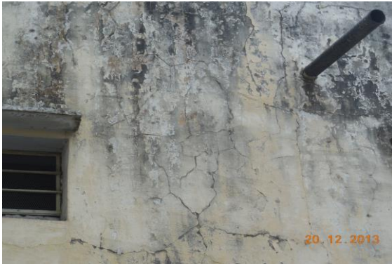
Photo 124 Peeling of Plaster on Wall No. 4 of Open Sky of First Floor
