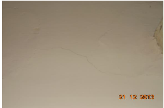
Photo 91 Peeling of Plaster on Wall No. 2 of Passage No.2 of Ground Floor
