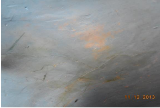
Photo 7 Plaster Crack on Roof of Part B of Shop No.197 of Ground Floor
