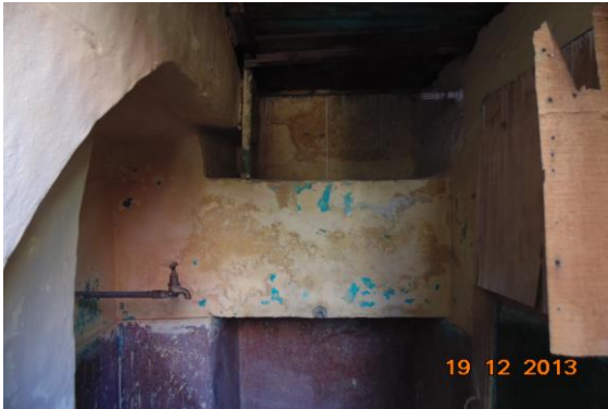
Photo 60 Dampness/Seepage on Wall No. 4 of Water tank Area of First Floor
