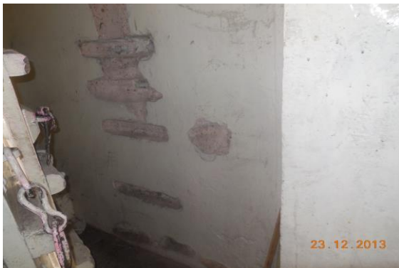
Photo 119 Peeling of Plaster on Wall No. 1 of Entrance of
