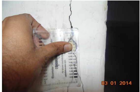
Photo 9A Inclined Crack on Wall No. 3 of Balcony 3, Second Floor - Part A Approx. Width = 3mm, Approx. Length = 1.3m. Distance from w2 = 1.5m, Height from Floor = 1.05m.
