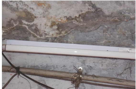
Photo 75 Horizontal Crack on Roof of Varanda of Shop No. 283 A, G/F Approx. Width = 0.6mm, Approx. Length = 2.5m. Distance from Leftside External Column = Backsidem, Height from Floor = 3m.
