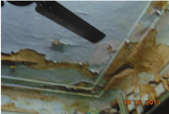
Photo 15 Peeling of Plaster on Wall No. 4 & Roof of Part-III of Shop no.115 of First Floor
