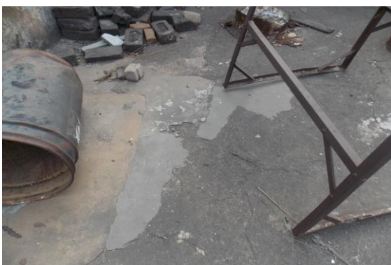
Photo 70 Peeling of Plaster on Floor of House no.410 of Terrace No.2
