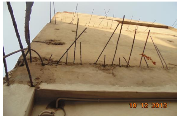
Photo 146 Exposed Reinforcement on Outer Wall of Shop No.10 of First Floor
