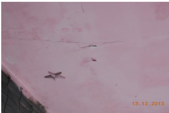
Photo 145 Plaster Crack on Roof of Room No. 4 of Second Floor
