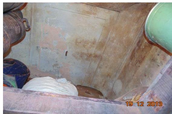
Photo 220 Dampness/Seepage on Wall No.4 & Roof of Part A of Shop Aggarwal Colour of Ground Floor
