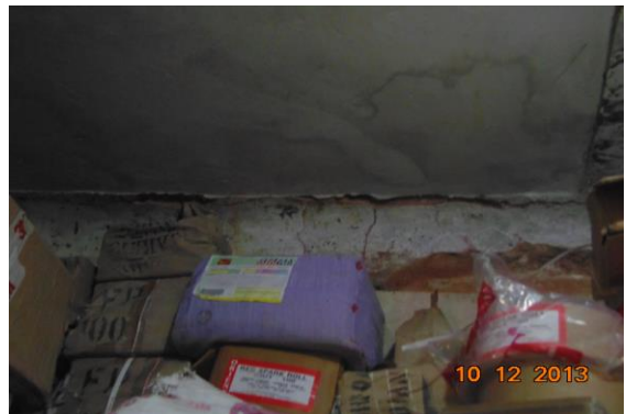
Photo 134 Peeling of Plaster on Wall No. 4 & Roof of Shop No.30 of Ground Floor
