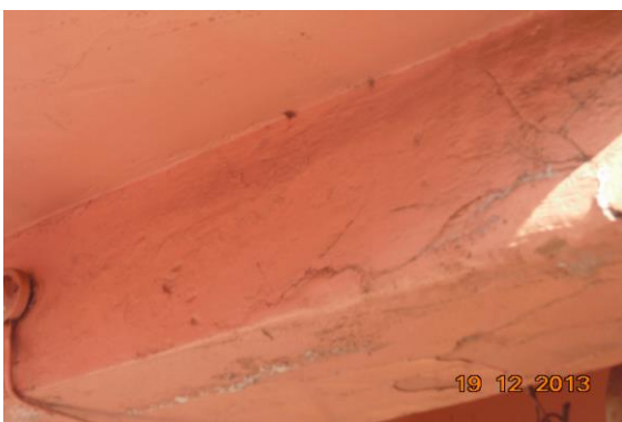
Photo 5 Peeling of Plaster on Beam of Temple of Ground Floor
