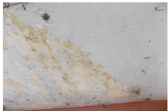
Photo 100 Peeling of Plaster on Roof of Shop No. 364A of Ground Floor
