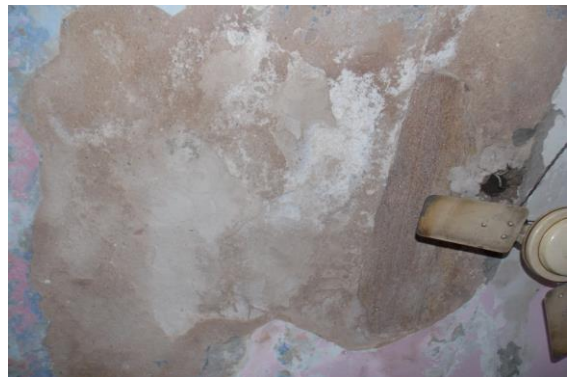
Photo 37 Peeling of Plaster on Roof of Room No. 6 of First Floor
