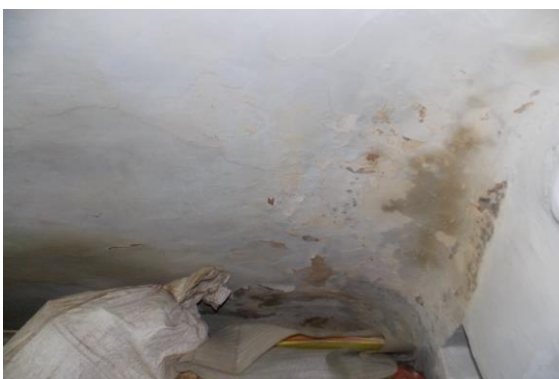
Photo 34 Dampness/Seepage on Roof of Room No. 2 of First floor
