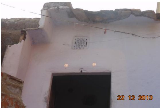
Photo 9 Peeling of Plaster on Roof Shade of of Second Floor
