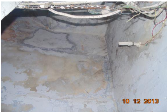
Photo 139 Dampness/Seepage on Wall No. 1 of Stair GF to FF of Ground Floor
