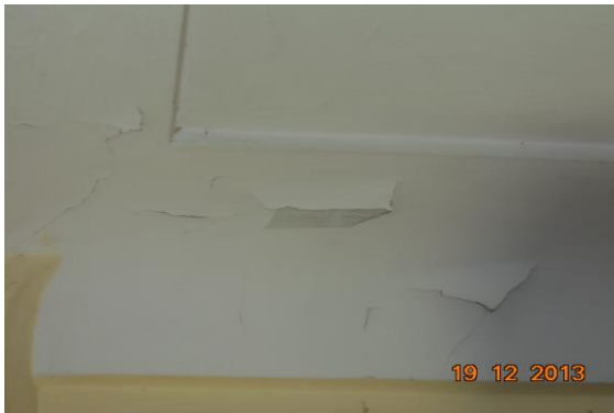
Photo 36 Peeling of Plaster on Roof of Room No. 2 of First Floor
