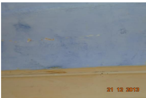
Photo 124 Peeling of Plaster on Roof of Room No. 7 of Temple, Ground Floor
