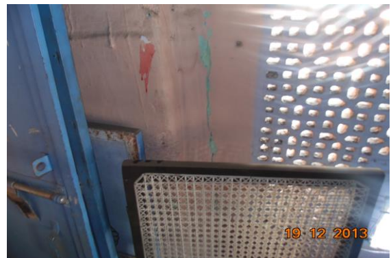
Photo 22 Inclined Crack on Wall No. 1 of Room No. 3, Parshu Ram Public School, First Floor, Approx. Width = 1mm, Approx. Length = 1m. Distance from Wall No.3 = 0.4m, Height from Floor = 0.5m.
