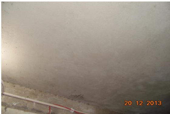
Photo 8 Peeling of Plaster on Roof of Ground Floor
