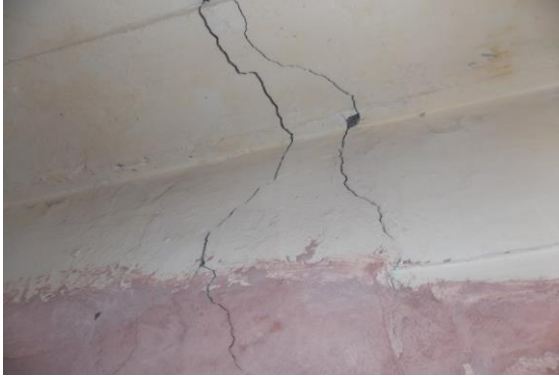
Photo 73A Inclined Crack on Wall No. 1 of Gallery No. 4, Second Floor Approx. Width = 2mm, Approx. Length = 2m. Distance from Wall no. 3 = 3.2m, Height from Floor = 0.7m.
