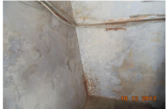
Photo 152 Dampness/Seepage on Wall No. 1, 2 & 4 of Staircase FF to SF of Second Floor
