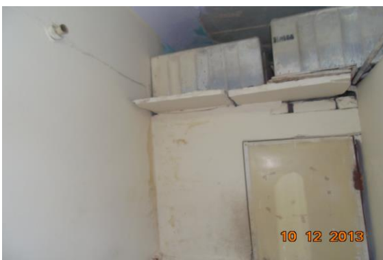
Photo 11 Dampness/Seepage on Wall No. 4 of Toilet No. 2 of Bank of Baroda, First Floor
