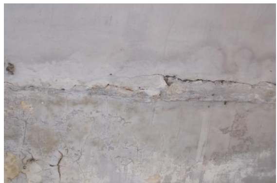
Photo 77 Horizontal Crack on Roof of Varanda of Shop No. 282, Ground Floor Approx. Width = 1mm, Approx. Length = 2.5m. Distance from Leftside External Column = Backsidem, Height from Floor = 3m.
