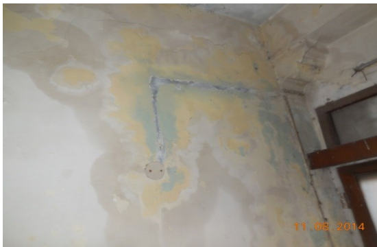
Photo 106 Seepage on Wall No. 3 & 5 of Room No. 13 of Hind Hotel, Second Floor
