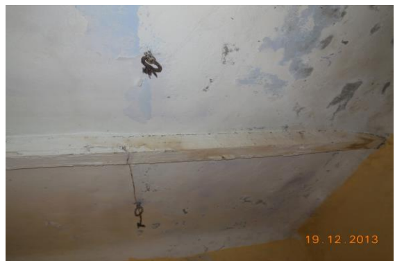
Photo 32 Dampness/Seepage on Roof of Kitchen of First Floor
