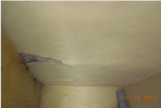
Photo 41 Peeling of Plaster on Roof of Passage No.5 of First Floor
