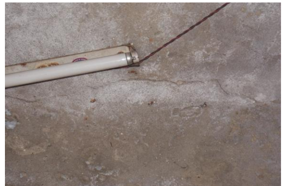
Photo 34 Horizontal Crack on Roof of Varanda of Shop No.265, Ground Floor. Approx. Width = 0.5mm, Approx. Length = 2.5m. Distance from Leftside External Column = 1m, Height from Floor = 3.5m.
