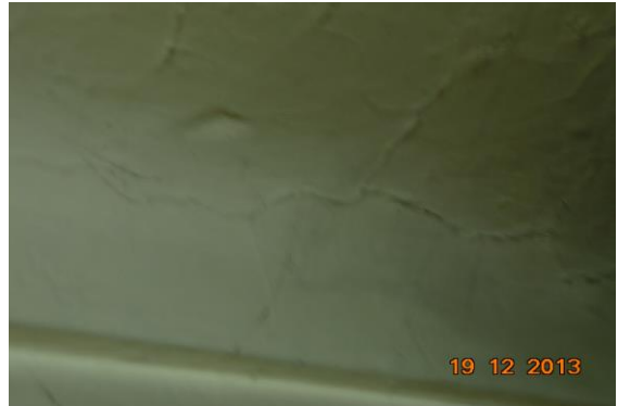
Photo 27 Peeling of Plaster on Roof of Temple of First Floor
