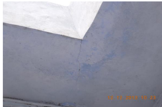
Photo 16 Inclined Crack on Wall No. 3 of Open Area, House No. 651, Ground Floor, Approx. Width = 7mm, Approx. Length = 1m. Distance from = m, Height from Floor = m.
