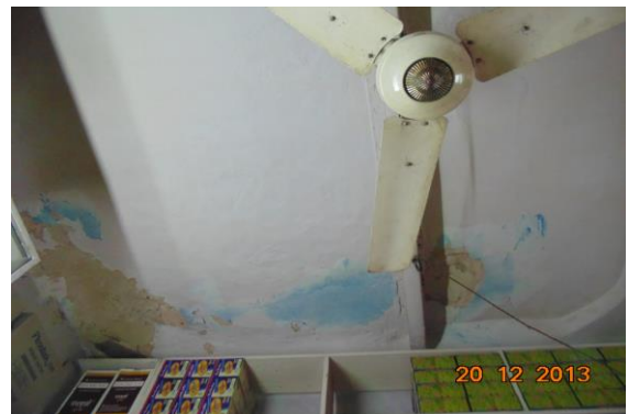
Photo 98 Peeling of Plaster on Roof of Part-B of Shop no. 371, Ground Floor
