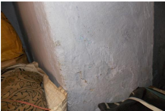
Photo 81 Peeling of Plaster on Wall No.3 & Roof of Shop of Ground Floor
