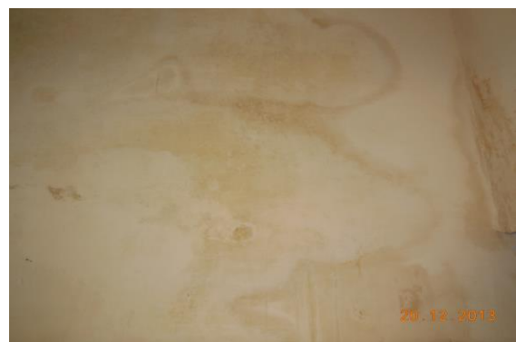
Photo 81 Dampness/Seepage on Wall No. 2 of Room No. 1 of Part b of Room. Ground Floor
