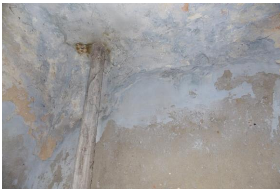
Photo 66 Dampness/Seepage on Roof of Lobby of House No. 483, Ground Floor
