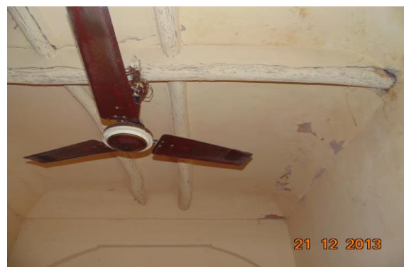
Photo 125 Dampness/Seepage on Roof of Room No. 1 of Temple, Ground Floor
