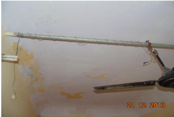
Photo 102 Dampness/Seepage on Roof of Room No. 3 of Temple, Ground Floor
