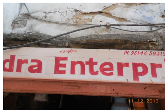
Photo 6 Damaged Portion on Roof Shade of Shop No.196 of Ground Floor
