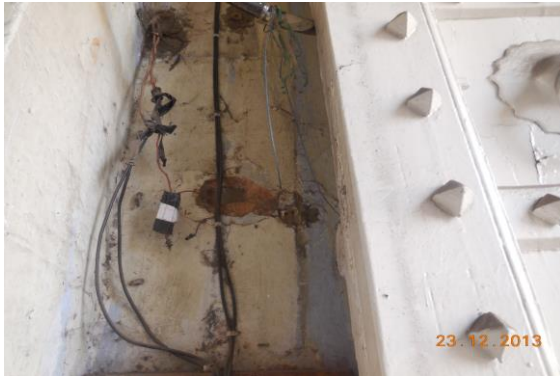
Photo 117 Peeling of Plaster on Wall No. 2 of Entrance of Ground Floor
