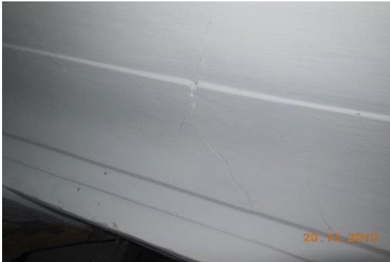
Photo 20 Inclined Crack on Roof of Hall No. 1, Basement Approx. Width = 0.6mm, Approx. Length = 1m.
