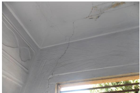
Photo 6 Inclined Crack on Wall No. 4 & Roof of Vranda, House No. 483, First Floor, Approx. Width = 2mm, Approx. Length = 2m. Distance from Wall No. 1 = 2.7m, Height from Floor = 1.9m.
