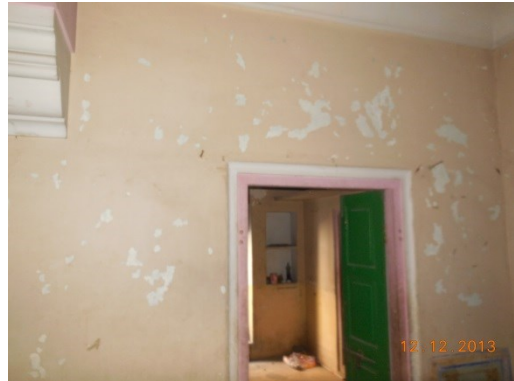
Photo 47 Plaster Removal on Wall No.2 of Room No.2 of H.No.481,First Floor
