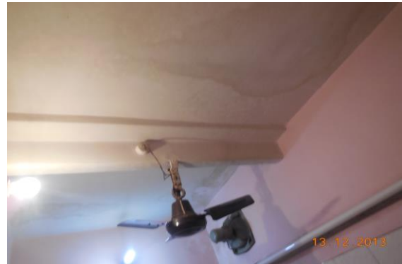
Photo 132 Dampness/Seepage on Roof of Toilet No. 1 of Second Floor
