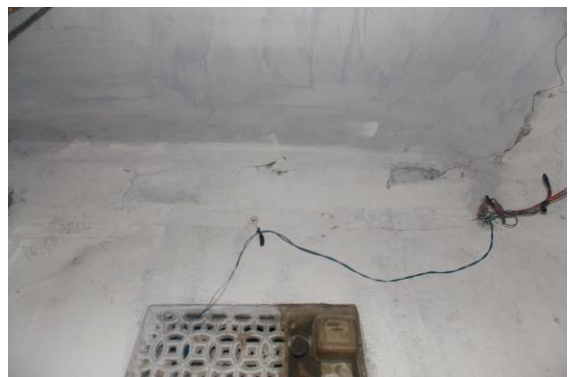
Photo 33 Dampness/Seepage on Wall No. 4 of Temple No.1 of First Floor
