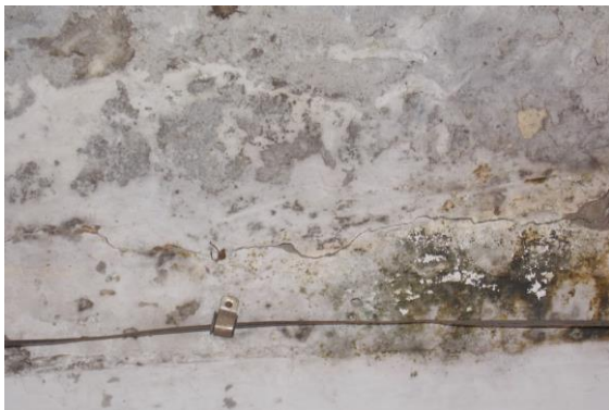
Photo 9 Horizontal Crack on Roof of Varanda of Shop No.275, Ground Floor, Approx. Width = 2mm, Approx. Length = 2.5m. Distance from Back of Right External Column = 0m, Height from Floor = 3m.
