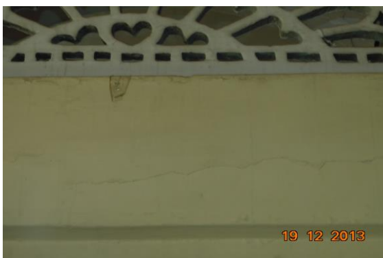
Photo 34 Peeling of Plaster on Wall No. 4 of Room No. 2 of First Floor
