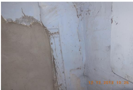
Photo 17 Inclined Crack on Wall No. 4 of Lobby, House No. 651, Ground Floor, Approx. Width = 1mm, Approx. Length = 0.4m. Distance from W2 = 0.03m, Height from Floor = 1.1m.
