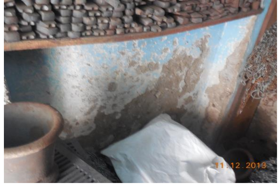
Photo 8 Peeling of Plaster on Wall No. 2 of Part B of Shop No.197 of Ground Floor
