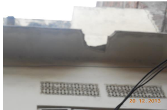
Photo 151 Damaged Portion on Outside Front Wall no.3 of Building of First Floor
