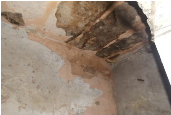
Photo 58 Dampness/Seepage of Room No. 4 of Ground Floor
