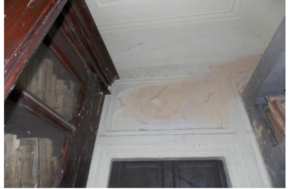
Photo 125 Dampness/Seepage on Roof & 4 of Passage No.3 of Library, First Floor
