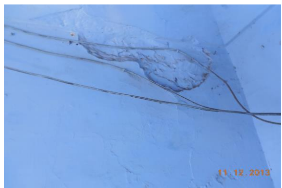
Photo 34 Peeling of Plaster on Wall No. 1 of Passage No.2 of First Floor
