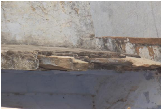
Photo 68 Peeling of Plaster on Wall No. 4 & Roof Shade of House no.410 of Second Floor
