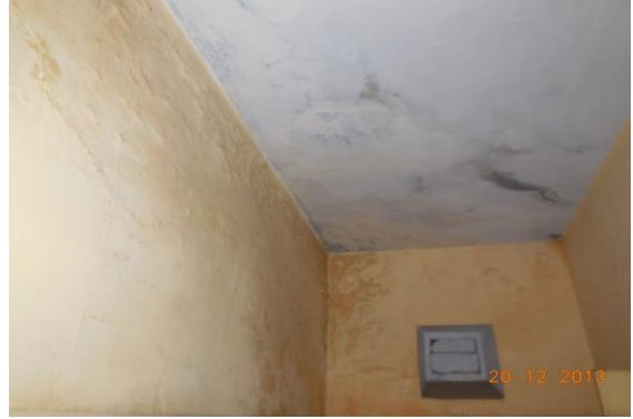
Photo 131 Dampness/Seepage on Wall No. 1, 3 & Roof of Passage No.1 of First Floor
