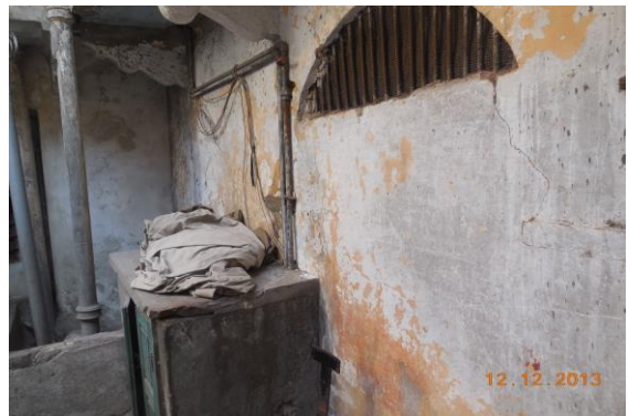
Photo 42 Peeling of Plaster on Roof of Open Area of House No. 424 Part A, Ground Floor
