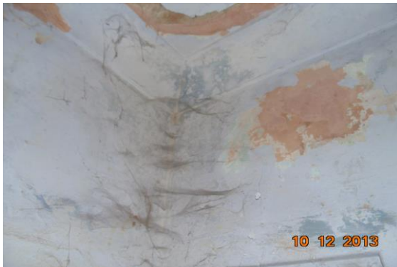
Photo 143 Dampness/Seepage on Wall No. 2 & 3 of Lobby of First Floor
