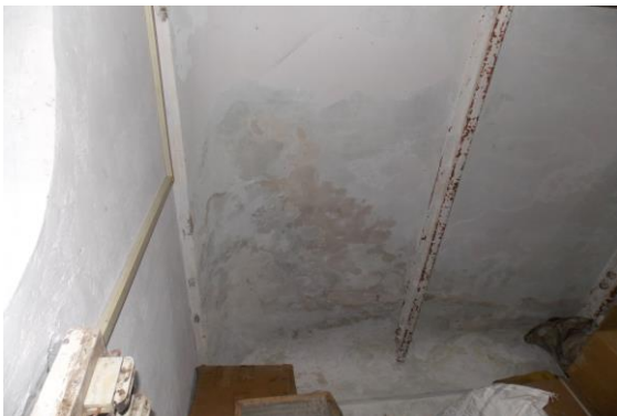
Photo 110 Dampness/Seepage on Roof of Shop No.6 of Ground Floor
