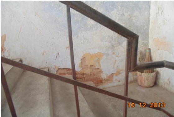
Photo 157 Peeling of Plaster on Wall No. 2 of Staircase SF to TF of Second Floor
