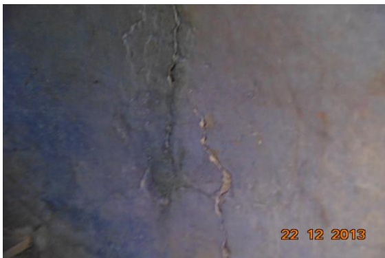
Photo 3 Peeling of Plaster on Open Sky of Ground Floor
