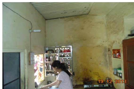
Photo 35 Dampness/Seepage on Wall No. 2 & 4 of Kitchen of First Floor
