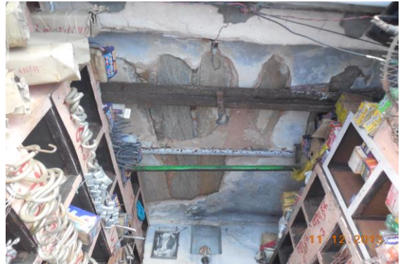
Photo 22 Peeling of Plaster on Roof of Shop No. 312 of Ground Floor
