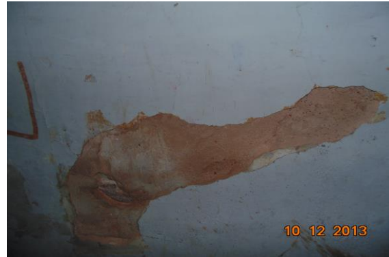
Photo 138 Peeling of Plaster on Wall No. 1 of Stair GF to FF of Ground Floor
