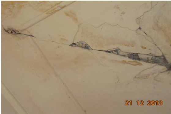
Photo 92 Peeling of Plaster on Wall No. 1 & Shade of Passage No.3 of Ground Floor
