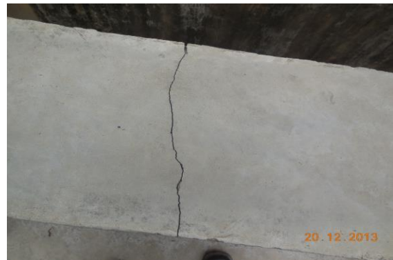
Photo 58 Inclined Crack on Perapet wall No.2 of Staircase, Second Floor Approx. Width = 1mm, Approx. Length = 1m.
