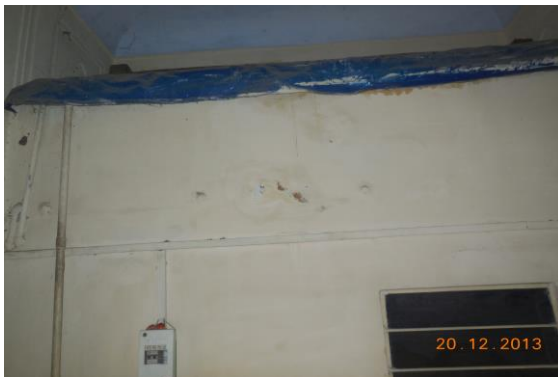
Photo 78 Peeling of Plaster on Wall No. 1 of Hall No. 1 of Ground Floor
