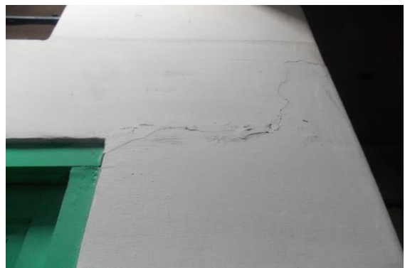
Photo 11 Inclined Crack on Wall No. 2 of Passage No.4, First Floor, Approx. Width = 0.3mm, Approx. Length = 0.8m. Distance from Wall No.3 = 0.4m, Height from Floor = 2.1m.
