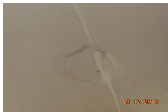
Photo 47 Peeling of Plaster on Roof of Room No. 3 of First Floor
