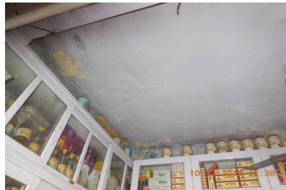
Photo 4 Peeling of Plaster on Roof of Shop No.362 of Ground Floor
