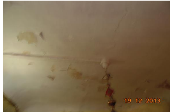
Photo 43 Peeling of Plaster on Roof of Lobby of First Floor
