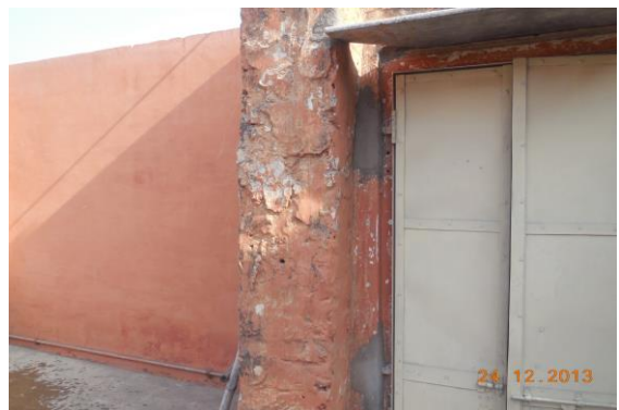
Photo 74 Peeling of Plaster of External Façade of House No.843,844 of Second Floor
