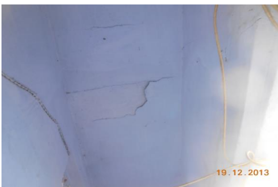
Photo 37 Peeling of Plaster on Roof of Bilding Udey Singh Ji Ki Haveli of First Floor
