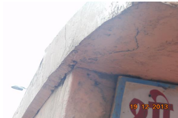
Photo 4 Damaged Portion on Roof Side of Temple of Ground Floor
