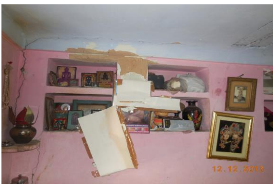
Photo 5 Inclined Crack on Roof of Room No. 1, House No. 424 Part A, Second Floor, Approx. Width = 0.45mm, Approx. Length = 2m. Distance from Wall No. 4 = 0.4m, Height from Floor = 0.5m.
