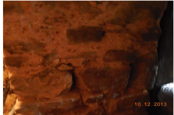
Photo 49 Peeling of Plaster on Right side Wall of Part C of Shop No. 299, Ground Floor
