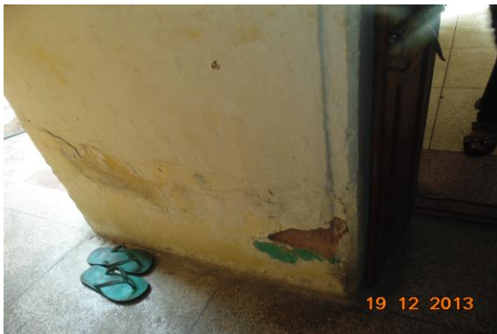
Photo 38 Dampness/Seepage on Wall No. 3 of Passage of First Floor
