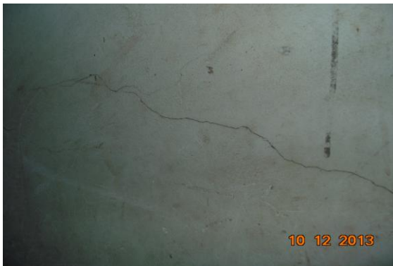
Photo 3 Horizontal Crack on of Staircase FF to SF, Approx. Width = 0.3mm, Approx. Length = 1.1m. Distance from Wall no.4 = 0.25m, Height from Floor = 1.6m.
