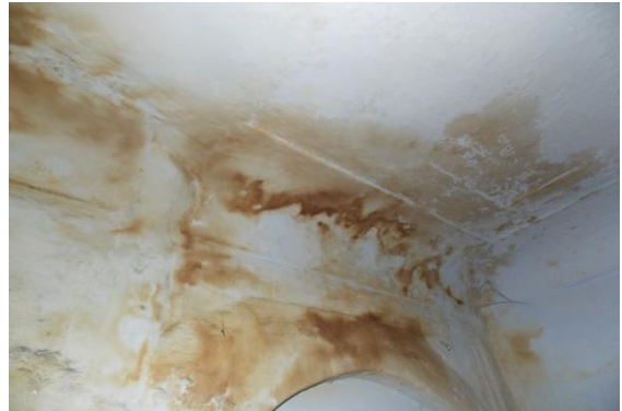
Photo 28 Dampness/Seepage on Wall No.3 & Roof of Kitchen of House No. 483, First Floor
