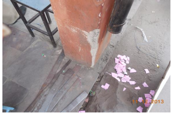
Photo 20 Peeling of Plaster on External Beam Right Side of Shop No. 311 of Ground Floor
