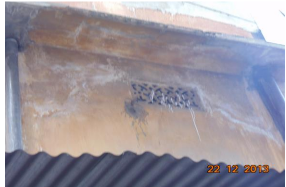
Photo 14 Dampness/Seepage on Outer Wall of External Façade H. No.476 of First Floor
