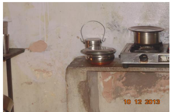
Photo 154 Peeling of Plaster on Wall No. 4 of Kitchen of Second Floor
