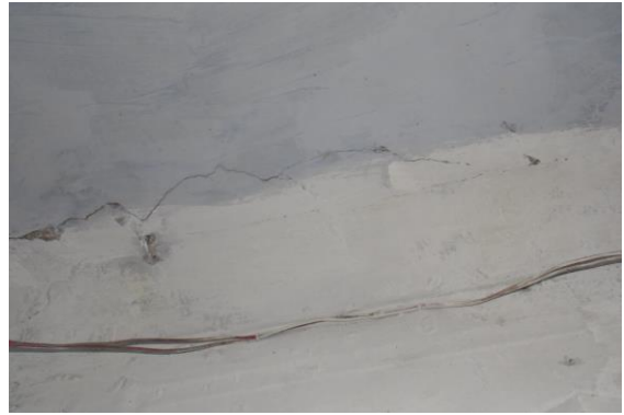
Photo 35 Damaged Portion on Roof of Temple No.1 of First Floor
