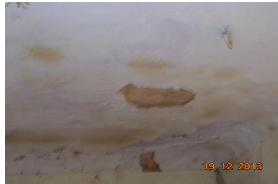
Photo 51 Peeling of Plaster on Roof of Bathroom of First Floor
