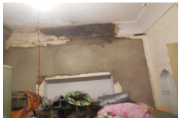
Photo 124 Peeling of Plaster on Roof of Room No. 8 of Second Floor
