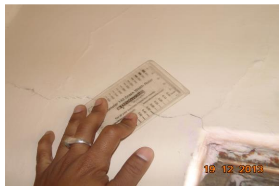
Photo 5A Inclined Crack on Wall No. 2 & 4 of Kitchen of House No.38, First Floor Approx. Width = 0.35mm, Approx. Length = 0.8m. Distance from Wall No.2 = 1.2m, Height from Floor = 1.5m.
