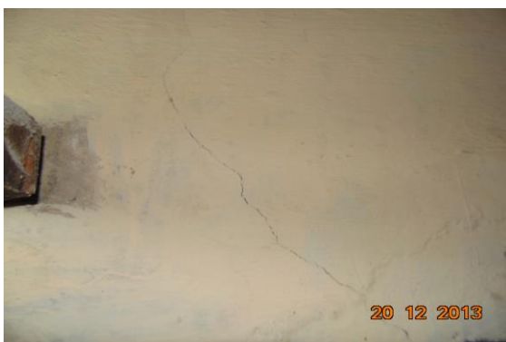
Photo 5 Inclined Crack on Outer Wall of Toilet No. 1, Ground Floor Approx. Width = 0.5mm, Approx. Length = 0.5m. Distance from Wall No.4 = 1m, Height from Floor = 1.8m.
