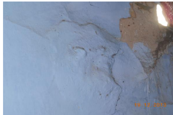
Photo 42 Peeling of Plaster on Wall No. 4 of Toilet & Washroom of Second Floor
