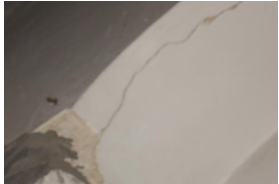
Photo 113 Plaster Crack on Frontside Wall of Shop No.6 of Ground Floor
