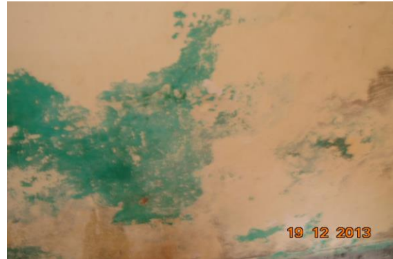
Photo 55 Dampness/Seepage on Wall No. 1 of Bathroom of First Floor
