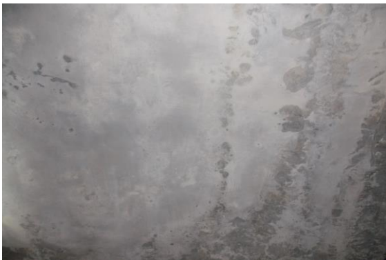
Photo 158 Dampness/Seepage on Roof of Varanda of Shop No.238 of Ground Floor
