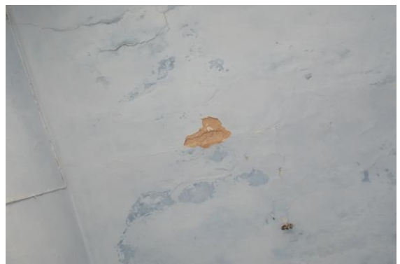
Photo 172 Peeling of Plaster on Roof of Lobby No.1 of Shri Krishna Chandra Ji Temple, First Floor
