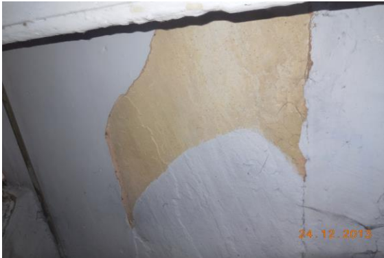
Photo 63 Peeling of Plaster on Roof of Passage of First Floor
