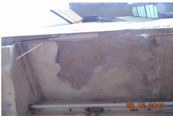
Photo 9 Inclined Crack on Wall No. of External Façade H. No.476, First Floor Approx. Width = 0.6mm, Approx. Length = 1.2m. Distance from Leftside Wall = 1.5m, Height from Floor = 3m.
