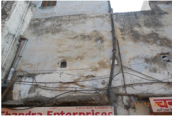
Photo 77 Damaged Portion on Wall No. Outerwall of First Floor
