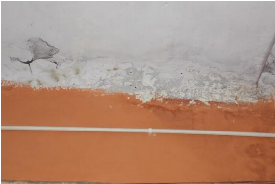
Photo 31 Dampness/Seepage on Roof of Varanda of Shop No.324 of Ground Floor
