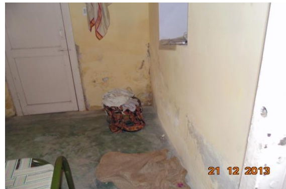
Photo 105 Dampness/Seepage on Wall No. 2 & 3 of Room No. 3 of Temple, Ground Floor
