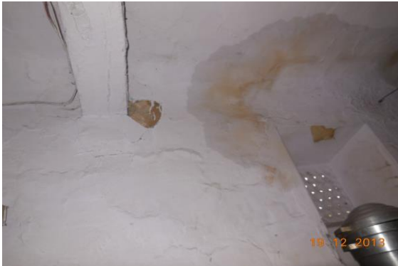
Photo 29 Damaged Portion on Wall No. 3 & Roof of Varanda of First Floor
