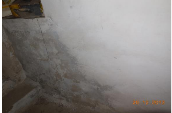
Photo 103 Dampness/Seepage on Wall No. 1 of Passage of Basement
