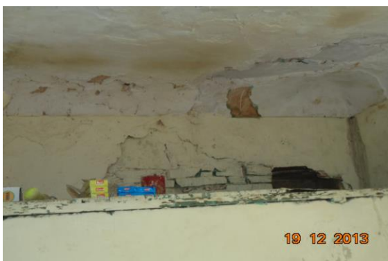
Photo 52 Peeling of Plaster on Wall No. 1 & Roof of Bathroom No. of First Floor
