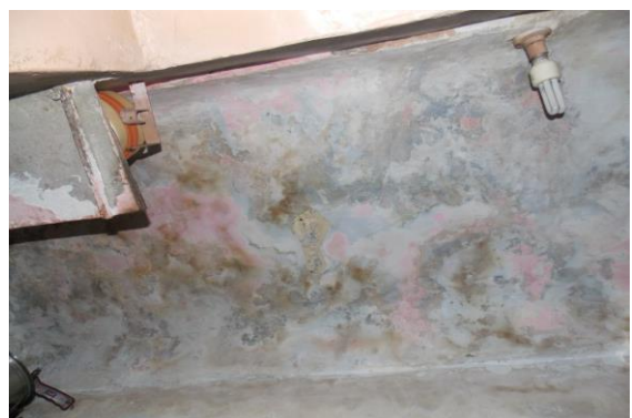
Photo 39 Dampness/Seepage on Roof of Balcony of House No. 478, First Floor
