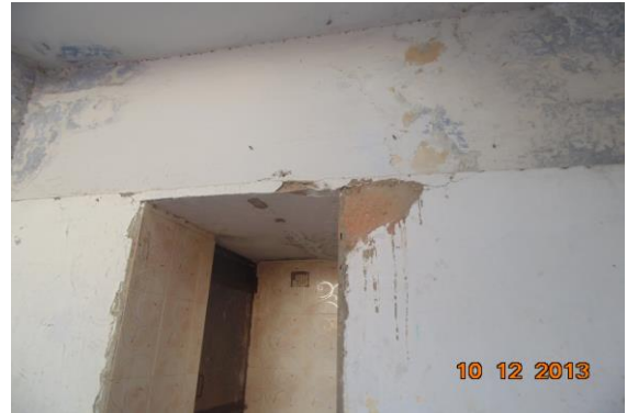
Photo 158 Peeling of Plaster on Wall No. 4 of Staircase SF to TF of Second Floor
