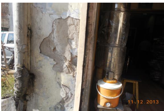
Photo 81 Peeling of Plaster on Wall No. Frontwall of Siyaram Treaders of Ground Floor
