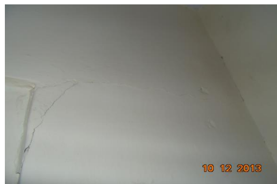
Photo 6 Horizontal Crack on Wall No. 3 of Room No. 1, Bank of Baroda, First Floor Approx. Width = 0.3mm, Approx. Length = 0.35m. Distance from Wall No.1 = 0m, Height from Floor = 2m.
