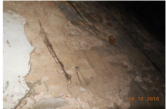
Photo 22 Damaged Portion on Wall No. 1 of Passage of First Floor
