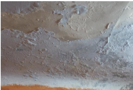
Photo 9 Peeling of Plaster on Roof of Varanda of Shop No.332 of Ground Floor
