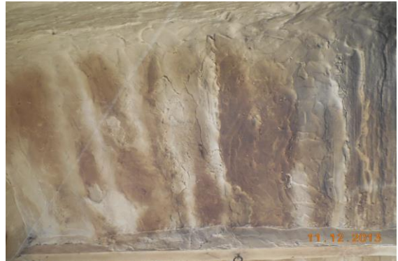
Photo 44 Dampness/Seepage on Roof of Kitchen of First Floor
