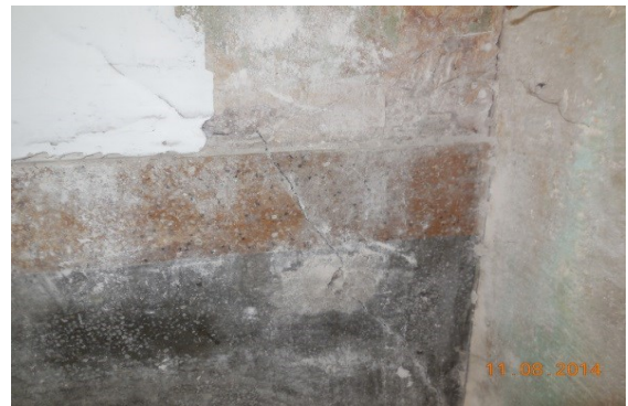
Photo 6A Inclined Crack on Wall No.2 of Passage of Hind Hotel, Ground floor, Approx. Width=1.5mm, Approx.Length=2.5m. Distance from Wall No.4=2.2m, Height from Floor=1.0m.
