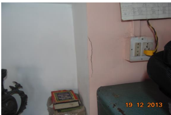
Photo 23 Inclined Crack on Wall No. 1 of Office, First Floor Approx. Width = 1.5mm, Approx. Length = 0.2m. Distance from Wall No.4 = 0.4m, Height from Floor = 1.1m.
