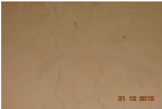
Photo 128 Peeling of Plaster on Wall No. 4 of Room No. 1 of Temple, Ground Floor
