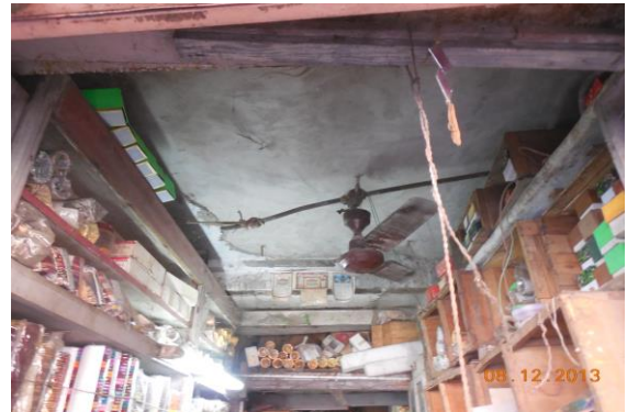
Photo 96 Peeling of Plaster on Roof of Shop No.370 of Ground Floor
