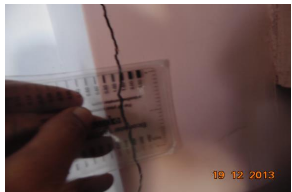
Photo 24 Inclined Crack on Wall No. 1 of Office, First Floor Approx. Width = 1.5mm, Approx. Length = 0.2m. Distance from Wall No.4 = 0.4m, Height from Floor = 1.1m.
