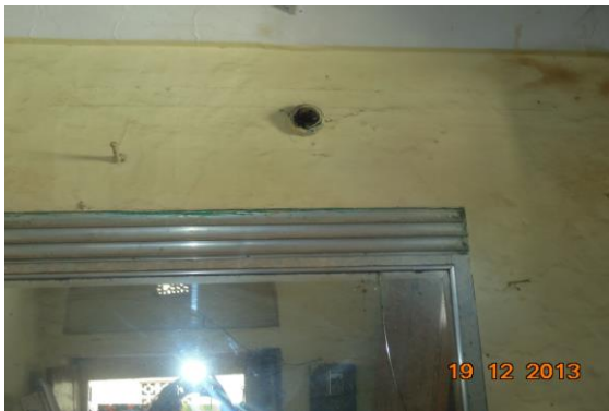
Photo 56 Dampness/Seepage on Wall No. 4 of Store No.3 of First Floor
