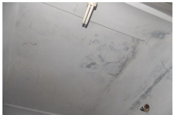
Photo 41 Dampness/Seepage on Roof of Toilet No. 1 of Second Floor
