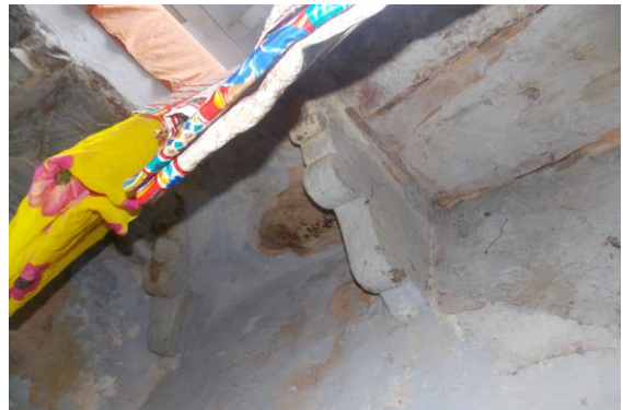
Photo 65 Dampness/Seepage of Sky open Sunshade of House No. 483, Ground Floor
