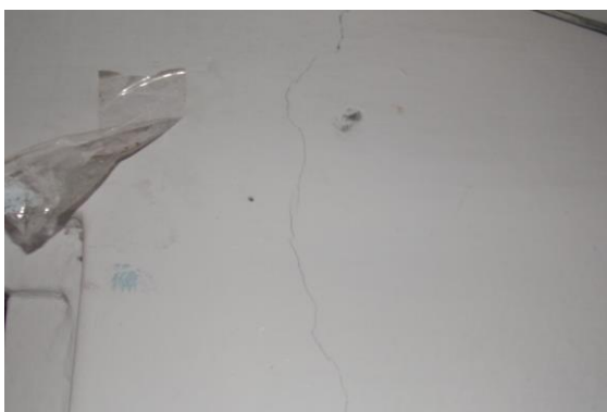
Photo 11 Inclined Crack on Wall No. 3 of Open sky Area, First Floor Approx. Width = 0.2mm, Approx. Length = 0.5m. Distance from Wall no.1 = 1.3m, Height from Floor = 1.7m.
