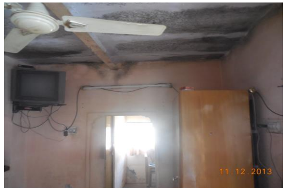
Photo 58 Dampness/Seepage on Wall No. 2 of Room No. 14 of First Floor
