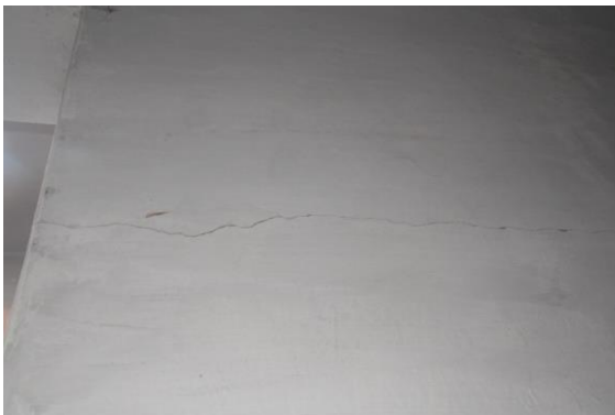
Photo 9 Horizontal Crack on Wall No. 2 of Passage No.2, First Floor, Approx. Width = 1mm, Approx. Length = 2m. Distance from Wall No.2 = 0.6m, Height from Floor = 2.3m.
