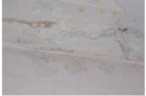
Photo 168 Dampness/Seepage on Wall No. 4 & Roof of Room No. 2 of Temple First Floor
