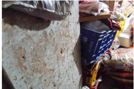
Photo 155 Peeling of Plaster on Wall No. 1 of Part B of Shop No.204 A of Ground Floor
