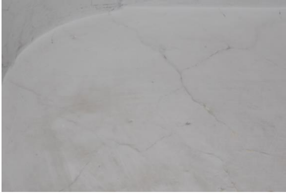
Photo 167 Peeling of Plaster on Wall No. 3 of Room No. 1 of Temple First Floor
