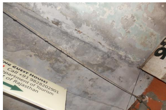
Photo 6 Horizontal Crack on Roof of Varanda of Shop No.236, Ground Floor, Approx. Width = 3mm, Approx. Length = 2.5m. Distance from Left side External Column = Backside, Height from Floor = 3m.
