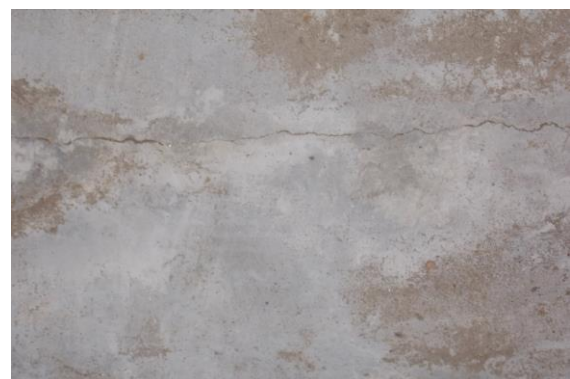
Photo 12 Horizontal Crack on Roof of Varanda of Shop No.195, Ground Floor Approx. Width = 2mm, Approx. Length = 2.5m. Distance from Rightside External Column = Backside, Height from Floor = 3m.
