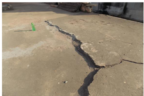
Photo 81 Damaged Portion on Floor of House No.429 of Terrace
