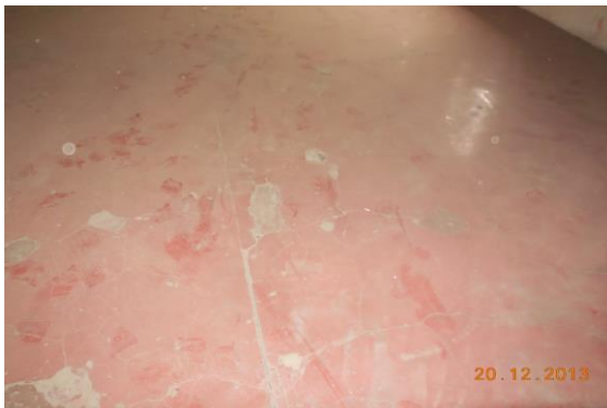
Photo 150 Peeling of Plaster on Floor of Hall No. 3 of Second Floor
