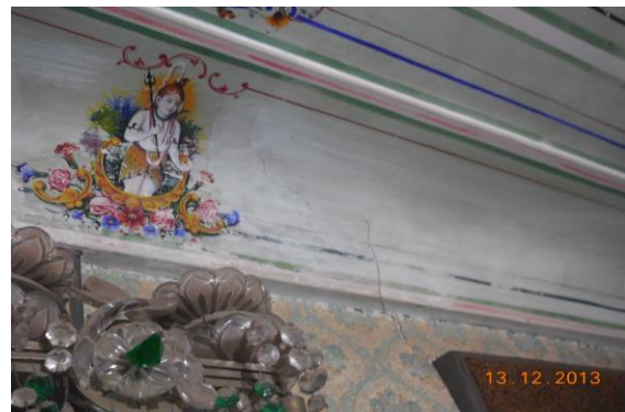
Photo 146 Plaster Crack on Roof of Room No. 3 of Second Floor
