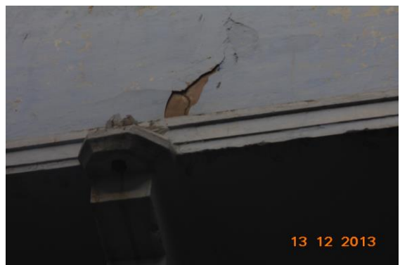
Photo 106 Peeling of Plaster on All Wall of Balcony of House No. 635, Second Floor
