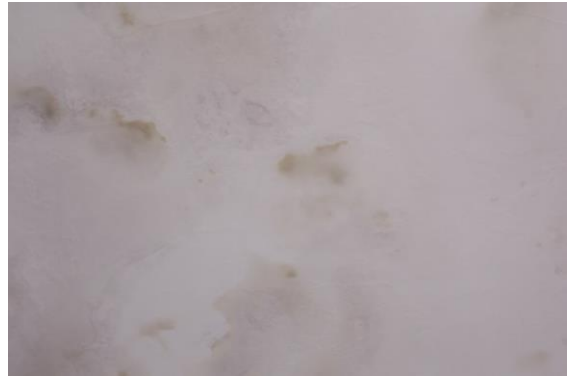
Photo 157 Dampness/Seepage on Roof of Shop No.238 of Ground Floor
