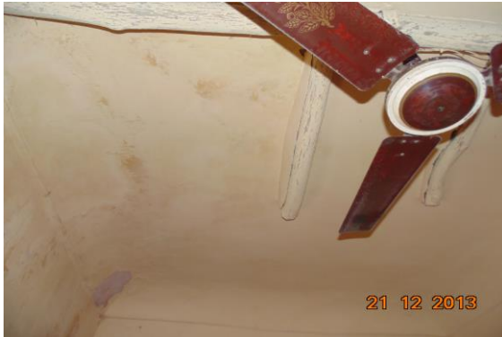
Photo 126 Dampness/Seepage on Roof of Room No. 1 of Temple, Ground Floor
