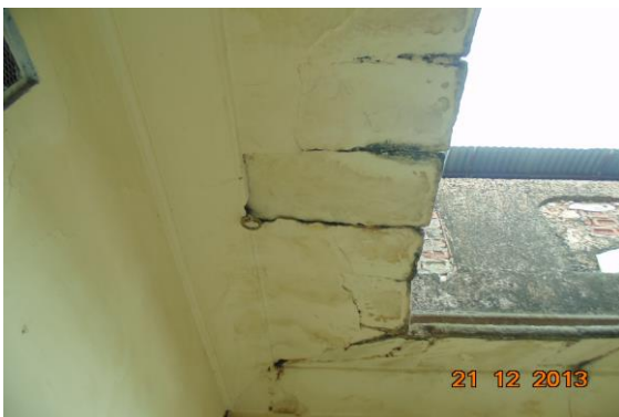
Photo 94 Peeling of Plaster on Wall No. 1 & Shade of Passage No.3 of Ground Floor
