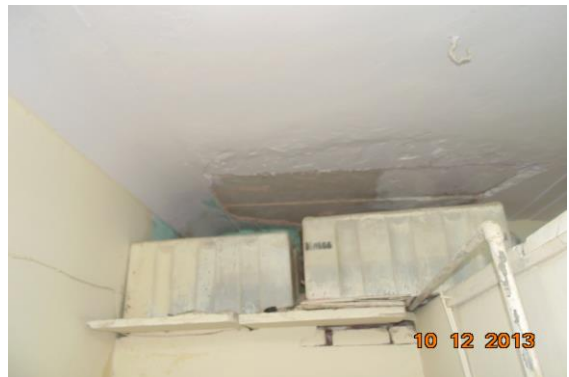
Photo 10 Peeling of Plaster on Roof of Toilet No. 2 of Bank of Baroda, First Floor
