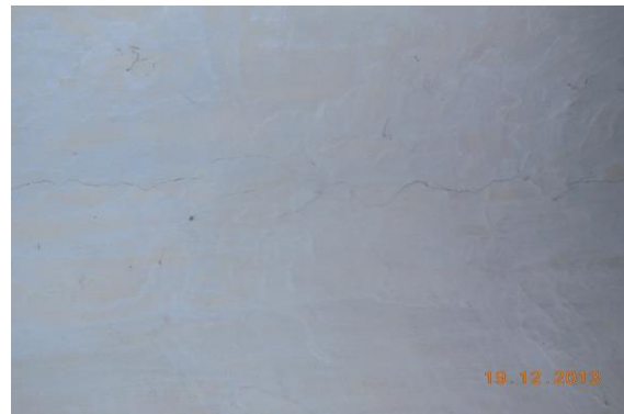
Photo 4 Horizontal Crack on Roof of Room No. 2, First Floor Approx. Width = 0.3mm, Approx. Length = 2.6m. Distance from Wall N0.1 = 0.1m, Height from Floor = 2.3m.
