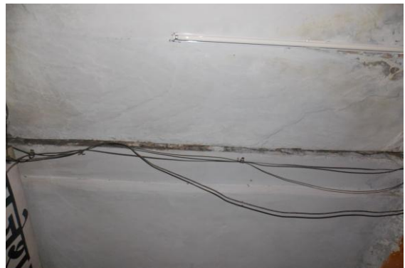
Photo 34 Peeling of Plaster on Roof of Varanda of Shop No.323 of Ground Floor
