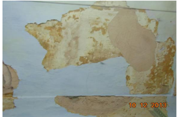
Photo 16 Peeling of Plaster on Roof of Part-IV of Shop No.115 of First Floor
