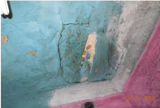
Photo 39 Damaged Portion on Roof of Kitchen of Second Floor
