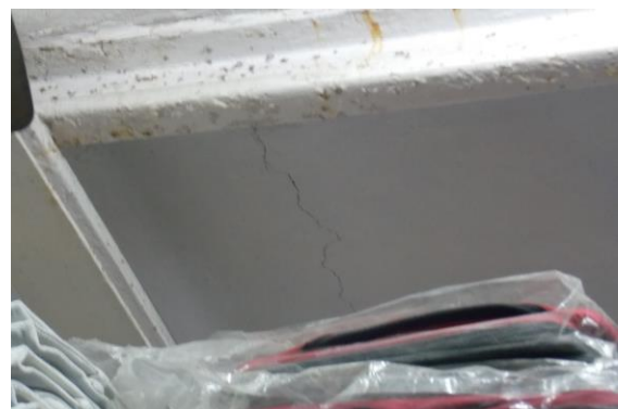
Photo 6 Horizontal Crack on Roof of Part B, Shop Sardari Lal & Sons, Ground Floor, Approx. Width = 0.6mm, Approx. Length = 1m. Distance from Wall No.2 = 2.5m, Height from Floor = 2.8m.
