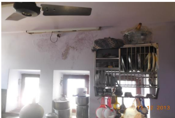
Photo 169 Dampness/Seepage on Outer Wall of Kitchen of House No. 635, Second Floor
