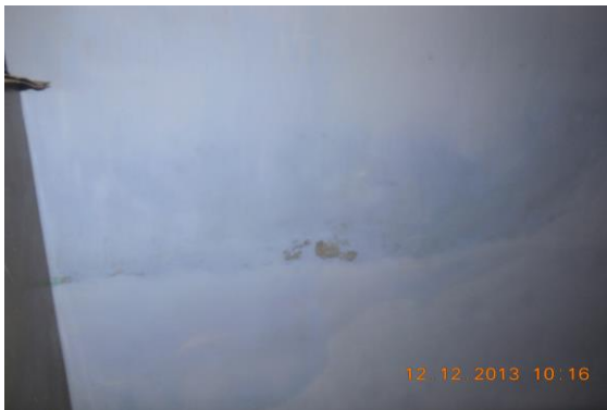
Photo 44 Dampness/Seepage on Wall No. 3 of Shop No. 2 of Ground Floor
