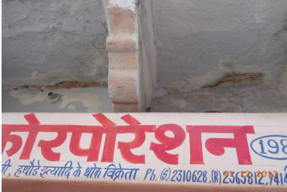
Photo 9 Peeling of Plaster on Roof Shade of Shop No.198 of Ground Floor
