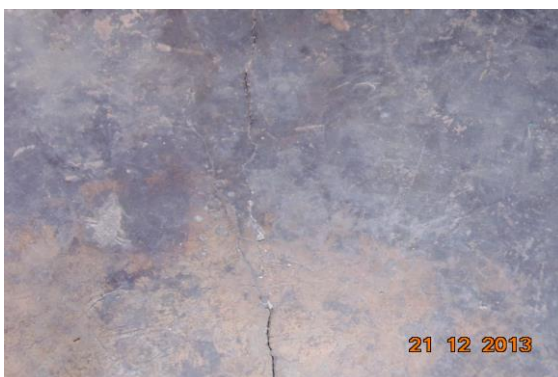
Photo 136 Peeling of Plaster on Floor of Hall No. 1 of Temple, Ground Floor
