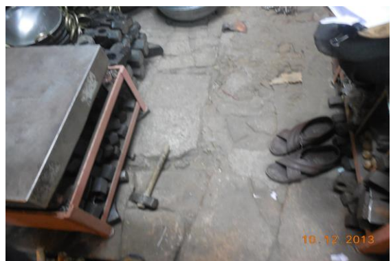
Photo 65 Peeling of Plaster on Floor of Shop No.307 of Ground Floor
