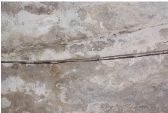
Photo 33 Horizontal Crack on Roof of Varanda of Shop No.266, G/F. Approx. Width = 0.25mm, Approx. Length = 2.3m. Distance from Leftside External Column = Backsidem, Height from Floor = 3.5m.
