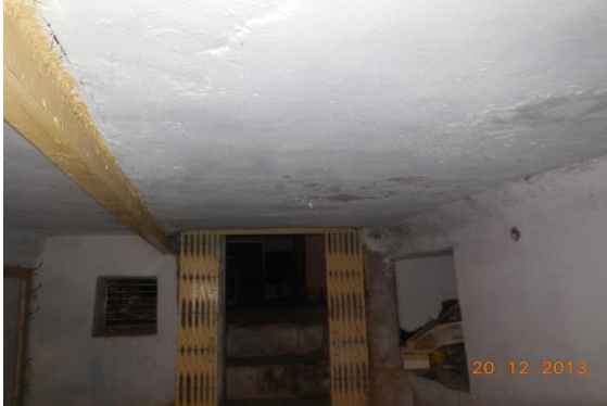
Photo 102 Dampness/Seepage on Roof of Passage of Basement
