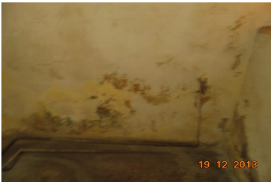
Photo 44 Dampness/Seepage on Wall No. 2 & 3 of Lobby of First Floor
