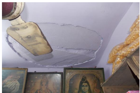
Photo 84 Peeling of Plaster on Roof of Shop No. 2 of Ground Floor
