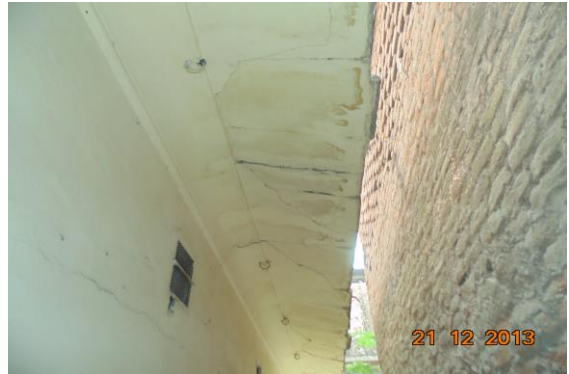
Photo 93 Peeling of Plaster on Wall No. 1 & Shade of Passage No.3 of Ground Floor
