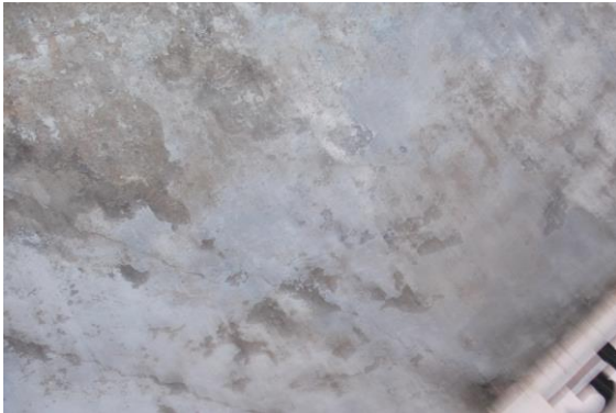
Photo 21 Peeling of Plaster on Roof of Varanda of Shop No.195 of Ground Floor
