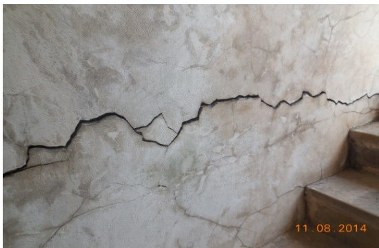
Photo 118 Plaster Removal on Wall No.1 & 4 of Staircase of Hind Hotel, Third Floor
