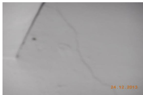
Photo 68 Peeling of Plaster on Wall No. 1 of Hall No. 1 of Second Floor
