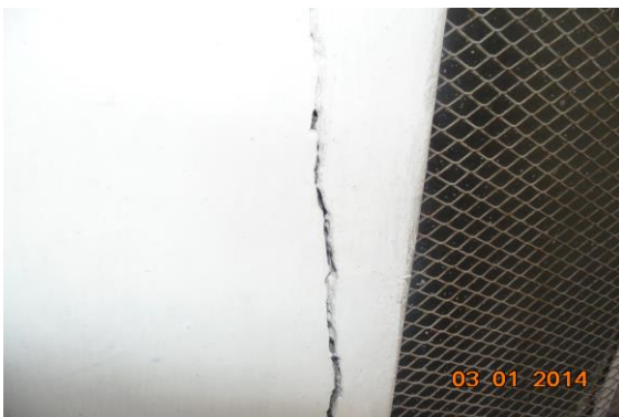
Photo 10 Vertical Crack on Wall No. 3 of Balcony 5, Second Floor - Part A Approx. Width = 2.5mm, Approx. Length = 0.6m. Distance from w1 = 3.5m, Height from Floor = 0.5m.
