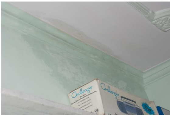
Photo 42 Dampness/Seepage on All Walls & Wall No. 4 of Room No. 7 of First Floor
