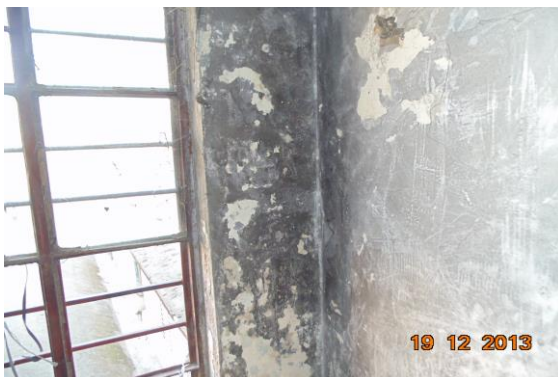
Photo 26 Peeling of Plaster on Wall No. 4 of Staircase Second Floor To Third Floor of Terrace
