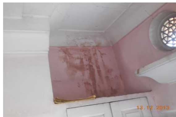
Photo 190 Dampness/Seepage on Wall No.1 & Roof of Room No. 5 of Second Floor
