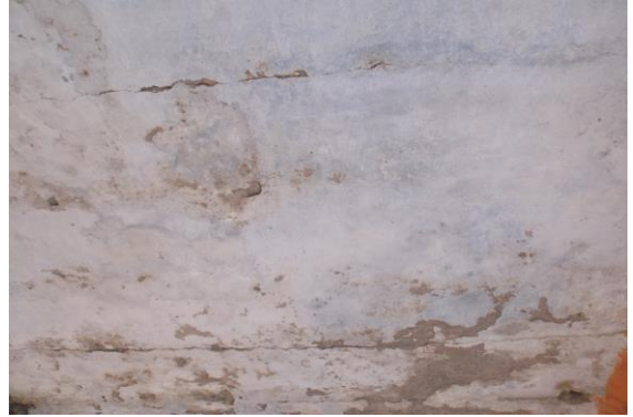
Photo 20 Dampness/Seepage on Roof of Varanda of Shop No.194 of Ground Floor
