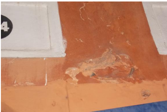
Photo 33 Peeling of Plaster on External Rightside Column of Varanda of Shop No.324 of Ground Floor
