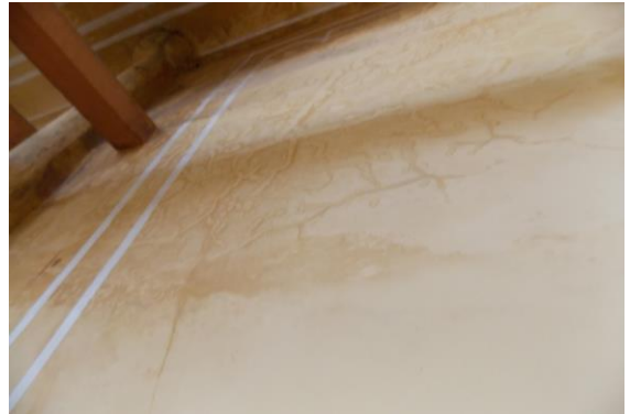
Photo 139 Dampness/Seepage on Wall No. 3 of Balcony of Library, First Floor
