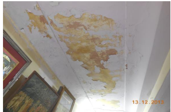
Photo 122 Dampness/Seepage on Roof of Hall No. 1 of Second Floor
