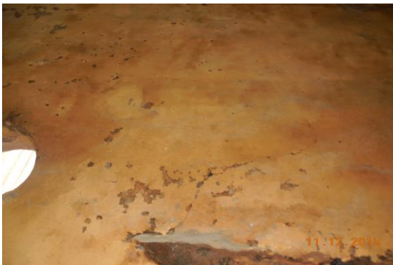
Photo 67 Dampness/Seepage on Wall No. 3 of Store No.1 of First Floor
