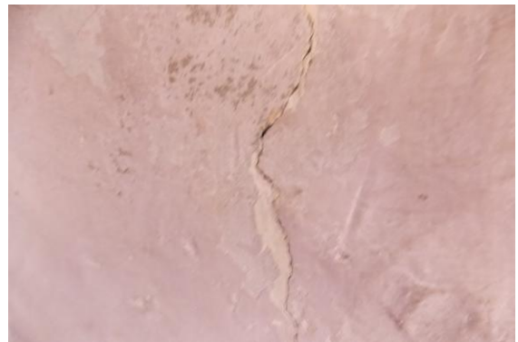
Photo 4 Inclined Crack on Wall No. 2 of Staircase, Ground Floor, Approx. Width = 2.5mm, Approx. Length = 1.8m. Distance from Wall no.3 = 2.3m, Height from Floor = 0m.
