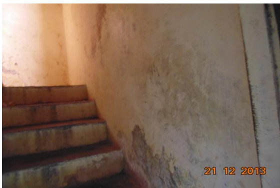
Photo 130 Dampness/Seepage on Wall No. 2 of Staircase of Ground Floor
