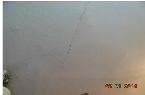
Photo 77 Plaster Crack on Floor of Terrace
