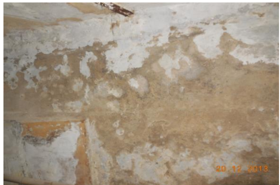
Photo 105 Peeling of Plaster on Wall No. 4 of Hall No. 6 of Basement
