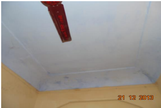
Photo 120 Dampness/Seepage on Roof of Room No. 7 of Temple, Ground Floor
