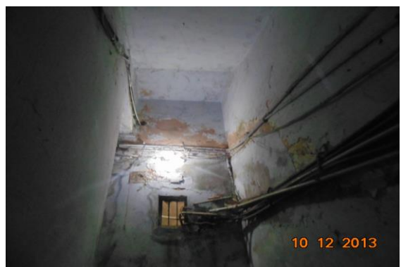
Photo 136 Dampness/Seepage on All Walls of Stair GF to FF of Ground Floor
