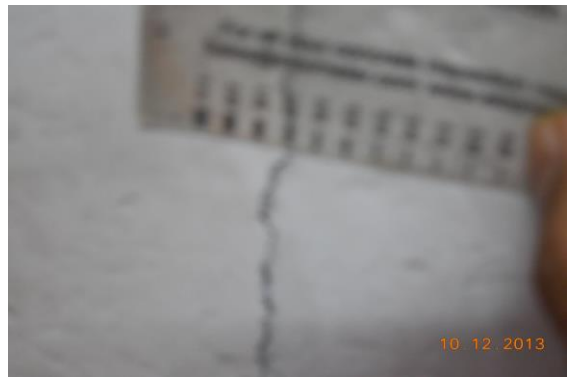
Photo 21A Inclined Crack on Wall No. 1 & Beam Portion of Shop No. 298, Ground Floor, Approx. Width = 1mm, Approx. Length = 1.5m. Distance from Wall No. 3 = 2m, Height from Floor = 0m.
