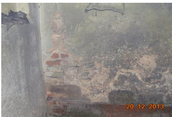
Photo 102 Peeling of Plaster on Shop No.2 of Ground floor
