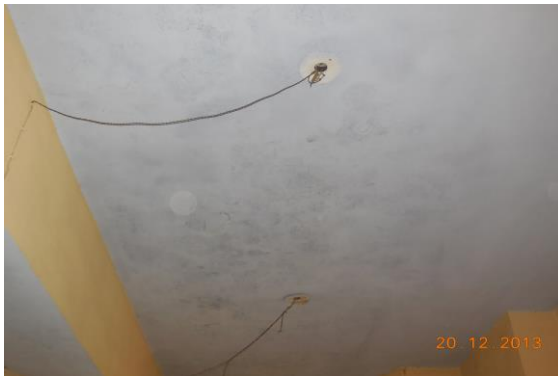
Photo 148 Dampness/Seepage on Roof of Hall No. 2 of Second Floor
