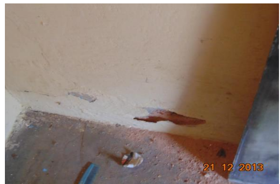
Photo 113 Peeling of Plaster on Wall No. 1 of Room No. 5 of Temple, Ground Floor
