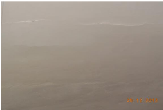
Photo 126 Peeling of Plaster on Roof of Hall No. 3 of Part B of Hall. First Floor
