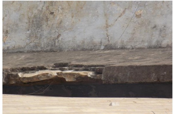
Photo 67 Peeling of Plaster on Wall No.4 & Roof Shade of House no.410 of Second Floor
