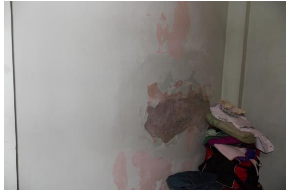
Photo 41 Peeling of Plaster on All Walls & Wall No.4 of Room No. 7 of First Floor
