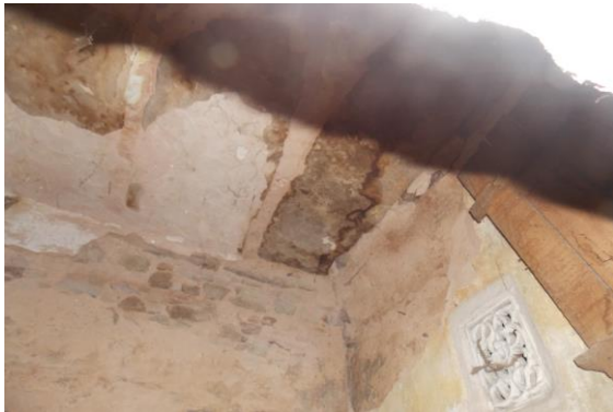
Photo 56 Dampness/Seepage of Room No. 1 & 2 of Ground Floor
