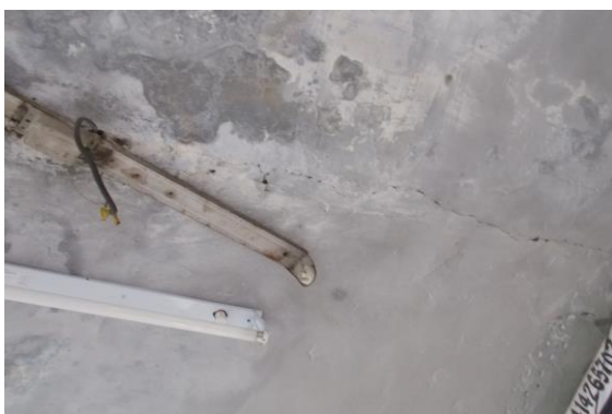
Photo 11 Horizontal Crack on Roof of Varanda of Shop No.275 A, Ground Floor, Approx. Width = 0.5mm, Approx. Length = 2.5m. Distance from Back of Left External Column = 0m, Height from Floor = 3m.
