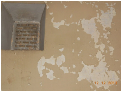
Photo 48 Peeling of Plaster on Wall No.4 of Room No.3 of H.No.481, First Floor
