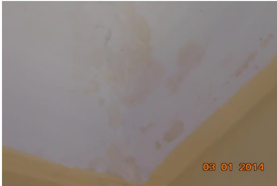
Photo 68 Dampness/Seepage on Roof of Room No. 3 of Third Floor - Part A
