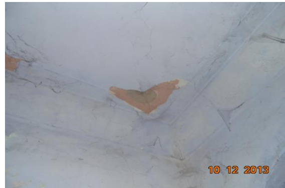
Photo 144 Peeling of Plaster on Roof of Lobby of First Floor
