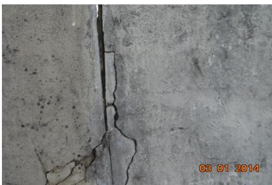
Photo 72 Damaged Portion on Wall No. 2 of Stair TF to Terrace of Third Floor - Part A
