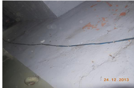
Photo 64 Peeling of Plaster on Wall No. 1 of Staircase No.1 of First Floor
