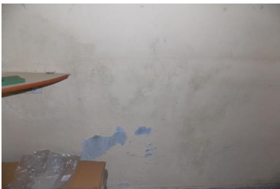
Photo 40 Dampness/Seepage on Wall No. 1 of Room No. 1 of Second Floor
