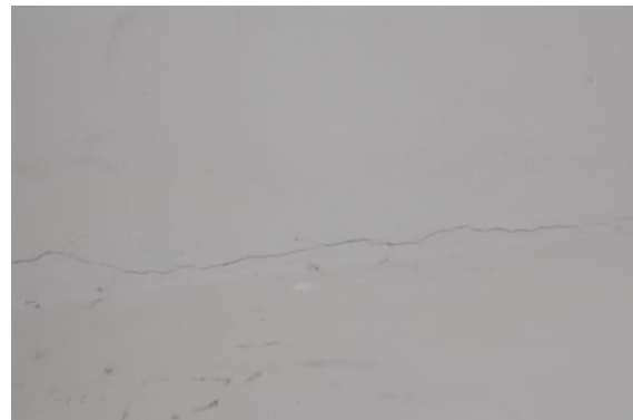
Photo 10 Horizontal Crack on Roof of Room No. 1, Ground Floor Approx. Width = 0.35mm, Approx. Length = 1.6m. Distance from Wall no.1 = 0.05m, Height from Floor = 2.5m.
