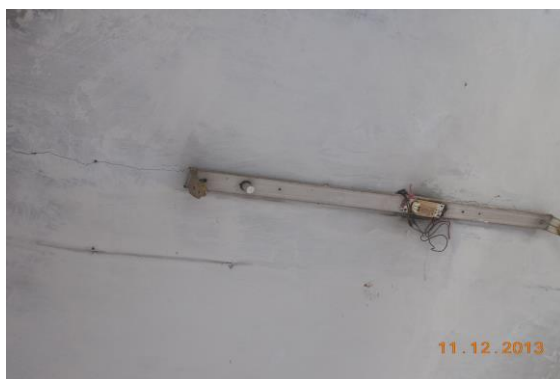
Photo 11 Inclined Crack on Roof of Varanda of Shop No.315, Ground Floor Approx. Width = 0.8mm, Approx. Length = 3m. Distance from Left External Column = 0m, Height from Floor = 3m.
