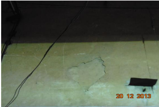
Photo 131 Plaster Crack on Front Wall of Shop No.116 of Ground floor
