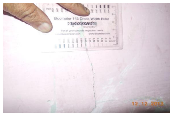
Photo 5A Inclined Crack on Roof of Room No. 1, House No. 424 Part A, Second Floor, Approx. Width = 0.45mm, Approx. Length = 2m. Distance from Wall No. 4 = 0.4m, Height from Floor = 0.5m.
