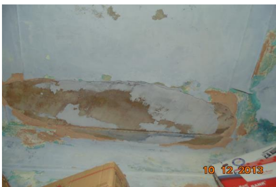
Photo 11 Peeling of Plaster on Roof of Part-I of Shop no.115 of First Floor
