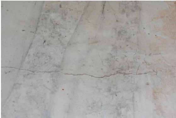
Photo 66 Peeling of Plaster on Wall No. 3 of House no.410 of Second Floor
