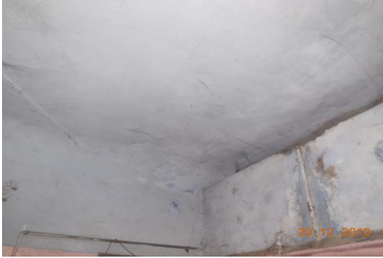
Photo 100 Dampness/Seepage on Roof of Passage of Ground Floor
