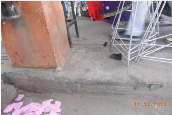
Photo 21 Peeling of Plaster on Floor & Out of Side of Shop No. 312 of Ground Floor
