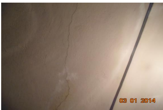
Photo 78 Plaster Crack on Roof of Room No. 1 of Second Floor - Part B
