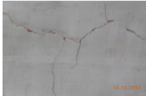
Photo 150 Plaster Crack on House No. 635 of Second Floor
