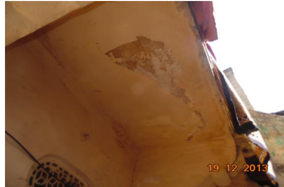
Photo 49 Dampness/Seepage on Wall No. 4 & Sun shade of Open Sky Area of First Floor
