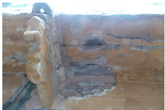
Photo 21 Damaged Portion on Sunshade of Open Area of House No. 478, Ground Floor
