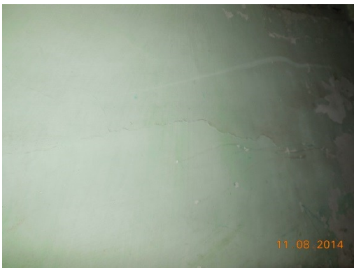
Photo 86 Plaster Crack on Wall No. 1 of Passage No. 3 of Hind Hotel, , First Floor
