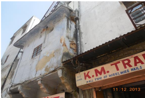
Photo 79 Damaged Portion on Wall No. Outerwall of First Floor
