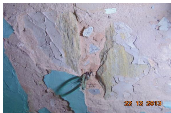
Photo 11 Peeling of Plaster on Roof of Temple of First Floor
