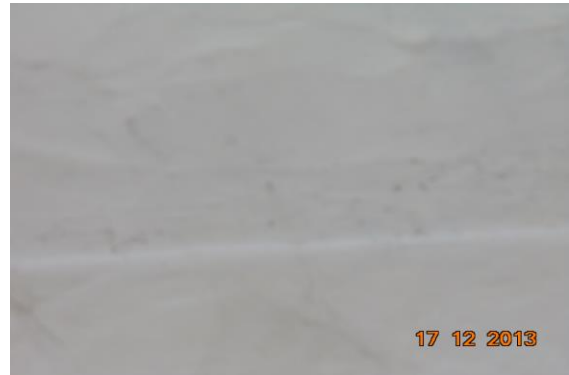
Photo 216 Dampness/Seepage on Roof of Shop Ra Rafugar of Ground Floor
