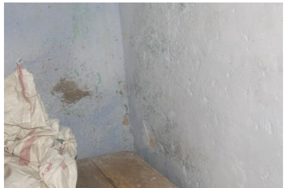
Photo 82 Peeling of Plaster on Wall No. 3 & Roof of Shop of Ground Floor
