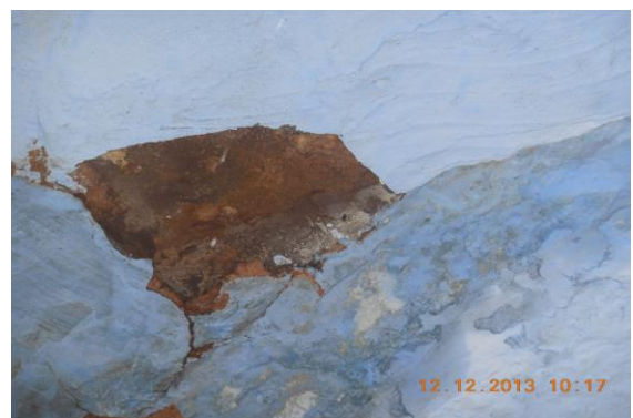
Photo 47 Dampness/Seepage on Roof of Shop No. 2 of Ground Floor
