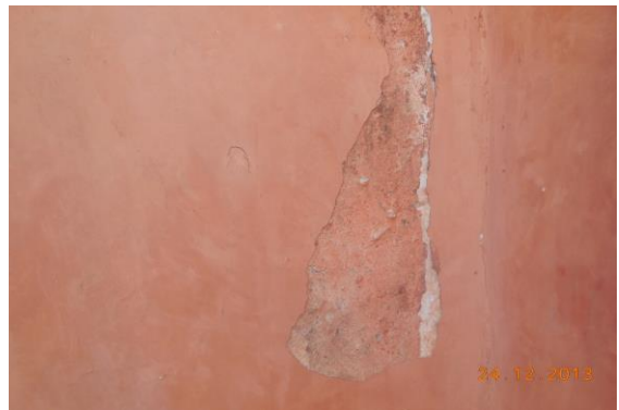
Photo 72 Peeling of Plaster on Outer wall of Toilet No. 2 of Second Floor
