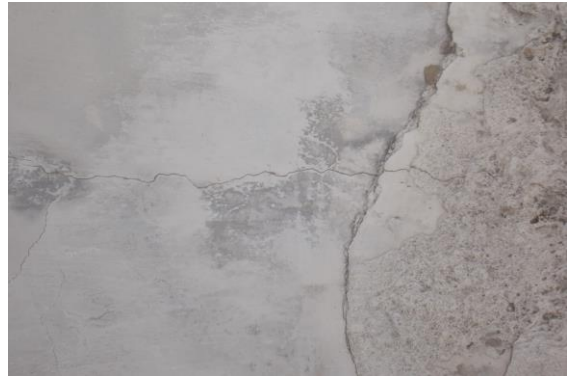
Photo 26 Horizontal Crack on Roof of Varanda of Shop No.204, Ground Floor Approx. Width = 0.3mm, Approx. Length = 1m. Distance from External Beam = 1.1m, Height from Floor = 3m.
