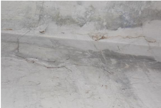
Photo 28 Peeling of Plaster on Roof & 3 of Passage No.2 of First Floor
