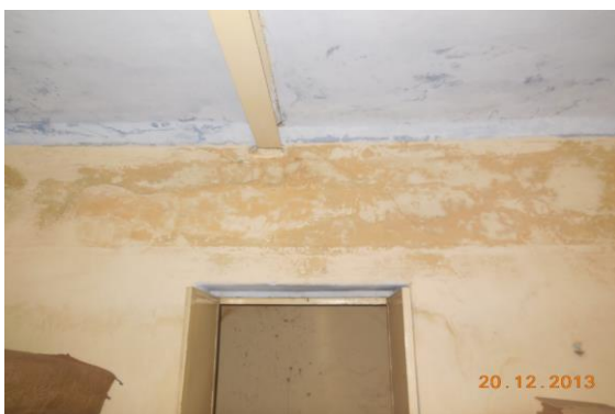
Photo 140 Dampness/Seepage on Wall No. 3 of Room No. 5 of First Floor
