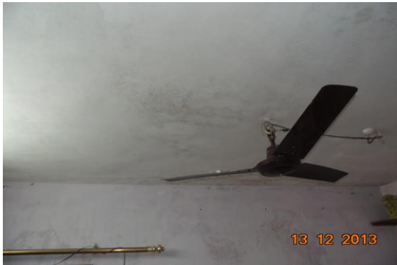
Photo 101 Dampness/Seepage on Roof of Room No. 3 of Second Floor
