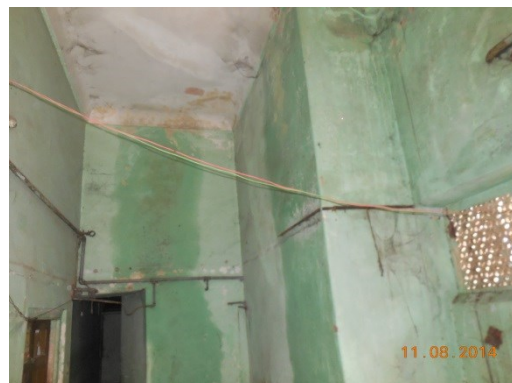
Photo 89 Seepage on Wall No. 2 & 3 of Varanda No. 4 of Hind Hotel, First Floor
