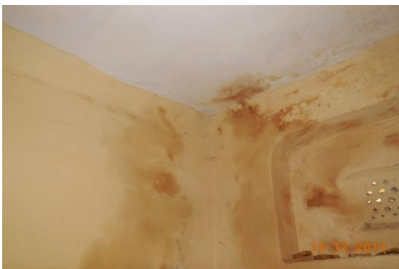
Photo 31 Dampness/Seepage on Wall No. 2, 4 & Roof of Toilet No. Toilet & Washroom of First Floor
