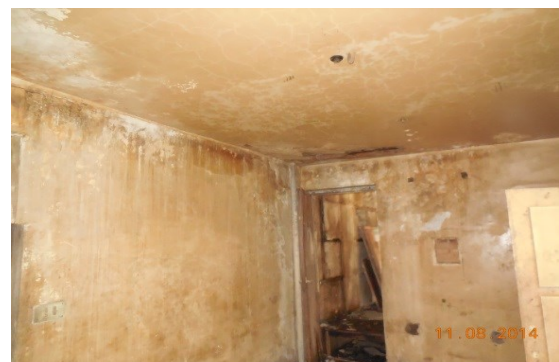
Photo 113 Seepage on All Walls of Room No. 2 of Hind Hotel, Third Floor
