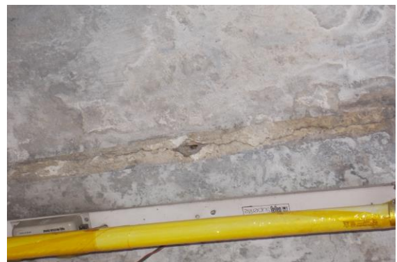
Photo 36 Horizontal Crack on Roof of Varanda of Shop No.264, Ground Floor. Approx. Width = 0.35mm, Approx. Length = 2.5m. Distance from Leftside External Column = 1m, Height from Floor = 3.5m.
