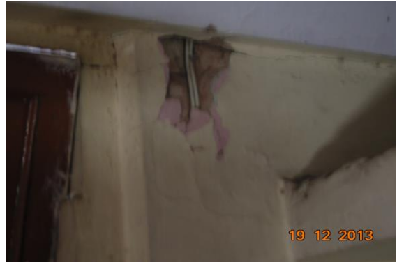
Photo 25 Peeling of Plaster on Wall No. 4 of Passage No.1 of First Floor
