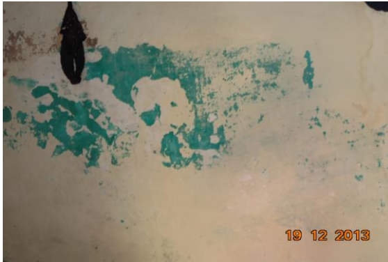
Photo 54 Dampness/Seepage on Wall No. 4 of Bathroom of First Floor
