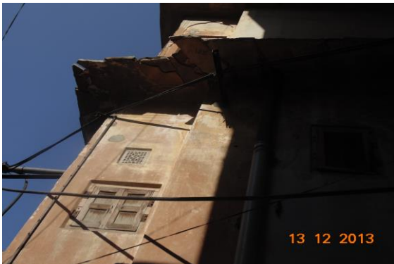
Photo 91 Damaged Portion on Back side Wall of External Façade of House No. 635, First Floor
