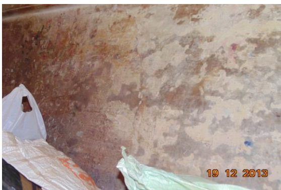
Photo 219 Peeling of Plaster on Wall No. 2 of Shop Pink city Colour of Ground Floor
