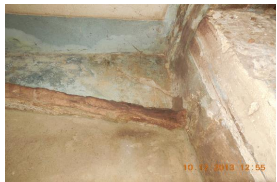
Photo 6 Inclined Crack on Wall No. 2 of Part A of Shop No.357, Ground Floor Approx. Width = 0.6mm, Approx. Length = 0.7m. Distance from Wall no.3 = 0m, Height from Floor = 2.5m.
