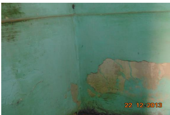
Photo 10 Peeling of Plaster on Wall No. 4 of Temple of First Floor
