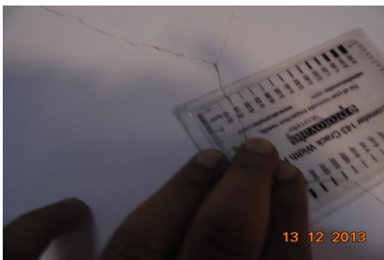
Photo 22A Inclined Crack on Roof of Room No. 3, Second Floor Approx. Width = 0.15mm, Approx. Length = 1.8m. Distance from Wall No.4 = 2.2m, Height from Floor = 2m.
