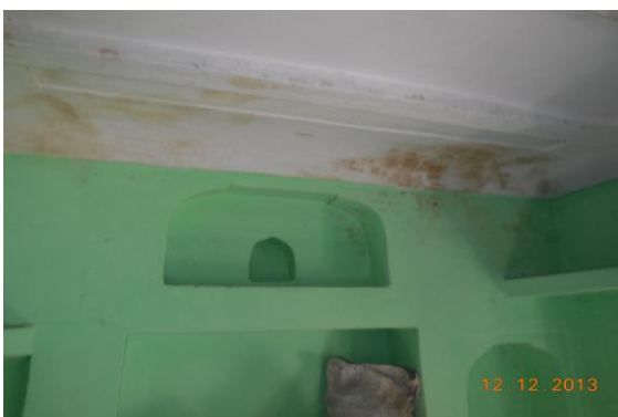
Photo 43 Dampness/Seepage on Wall No. 1 & Roof of Room No. 4 of House No. 423, First Floor
