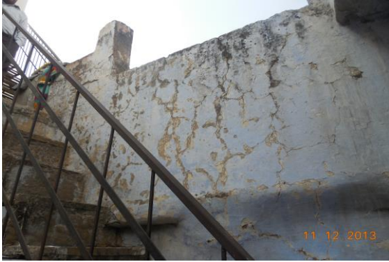
Photo 53 Plaster Crack on Wall No. 4 of Open Sky of First Floor
