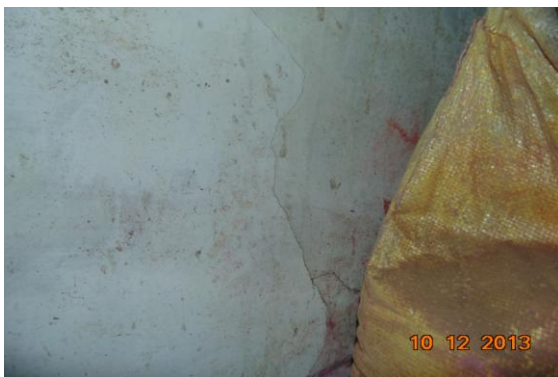
Photo 4 Inclined Crack on Wall No. 1 of Staircase FF to SF, Approx. Width = 0.2mm, Approx. Length = 0.8m. Distance from Wall No.3 = 1m, Height from Floor = 0m.
