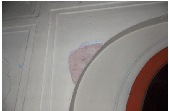
Photo 127 Peeling of Plaster on Wall No. 4 of Hall No. 5 of Library, First Floor
