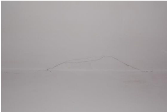
Photo 30 Peeling of Plaster on Roof of Room No. 1 of First Floor
