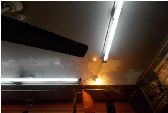
Photo 7 Peeling of Plaster on Roof of Shop No.332 of Ground Floor
