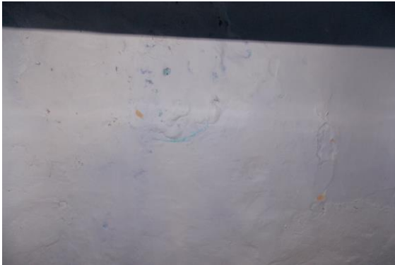
Photo 79 Peeling of Plaster on Roof of Shop of Ground Floor
