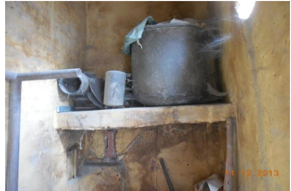
Photo 66 Dampness/Seepage on Wall No. 2 of Store No.1 of First Floor
