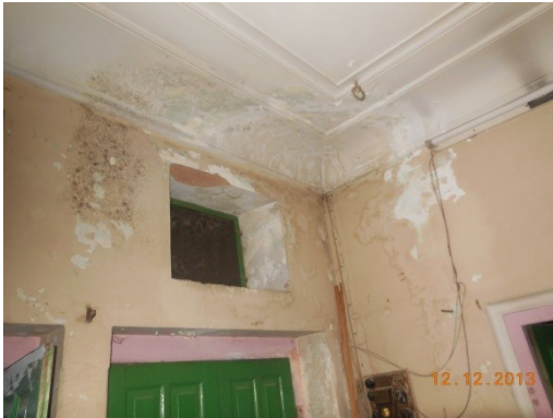
Photo 46 Plaster Removal on Roof of Room 1 of H.No.481,First Floor
