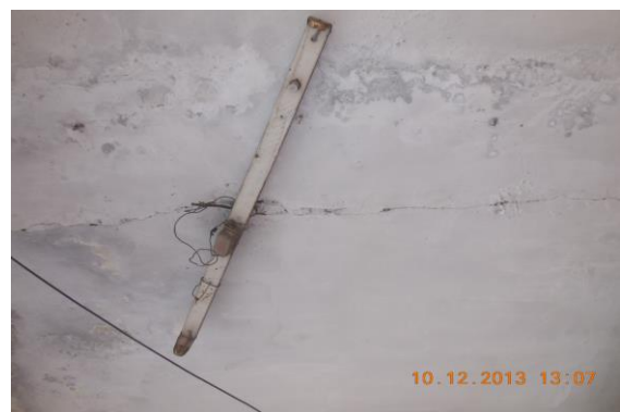
Photo 6 Horizontal Crack on Roof of Varanda of Shop No.359, Ground Floor, Approx. Width = 0.5mm, Approx. Length = 3m. Distance from Right side External Column = Backside, Height from Floor = 3m.
