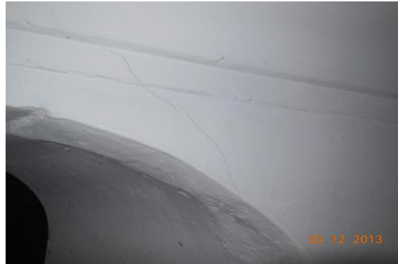
Photo 21 Inclined Crack on Wall No. 3 of Hall No. 1, Basement Approx. Width = 0.6mm, Approx. Length = 1m.
