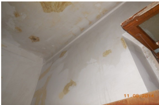
Photo 104 Seepage on Wall No.3 & Roof of Room No. 12 of Hind Hotel, Second Floor
