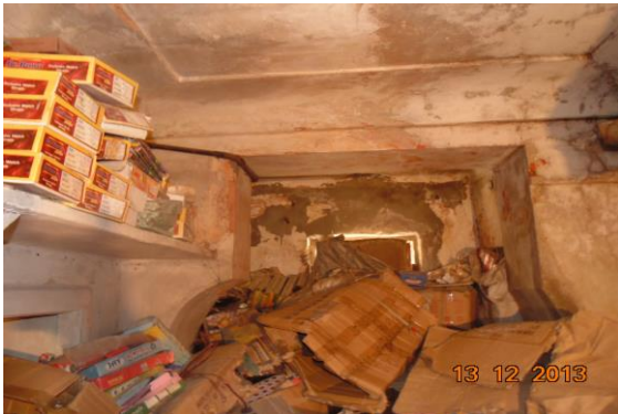
Photo 89 Peeling of Plaster of Room No. 9 of Ground Floor
