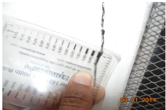
Photo 10A Vertical Crack on Wall No. 3 of Balcony 5, Second Floor - Part A Approx. Width = 2.5mm, Approx. Length = 0.6m. Distance from w1 = 3.5m, Height from Floor = 0.5m.
