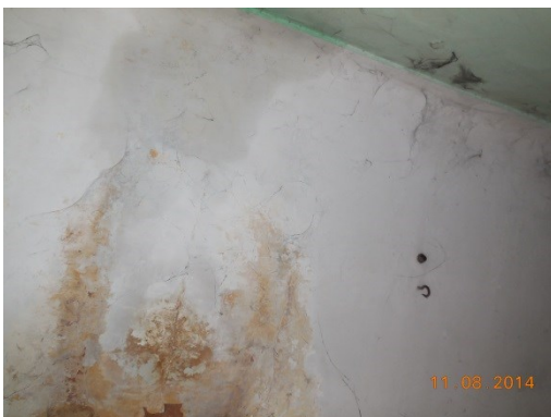
Photo 88 Seepage on Roof of Varanda No. 4 of Hind Hotel, First Floor
