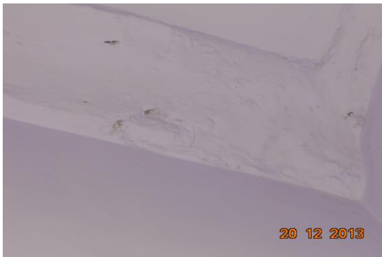
Photo 39 Peeling of Plaster on Roof of Shop No. 2 of Ground Floor
