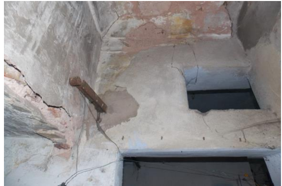
Photo 41 Peeling of Plaster on Wall No. 3 of Passage No.3 of First Floor
