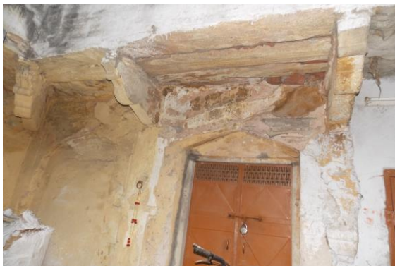
Photo 18 Dampness/Seepage on Open Area of House No. 478, Ground Floor
