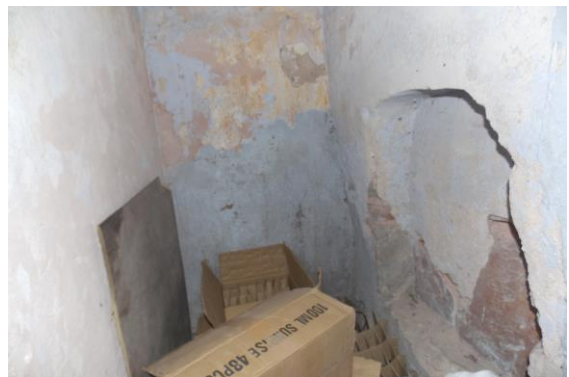
Photo 67 Dampness/Seepage on Roof of Lobby of House No. 483, Ground Floor
