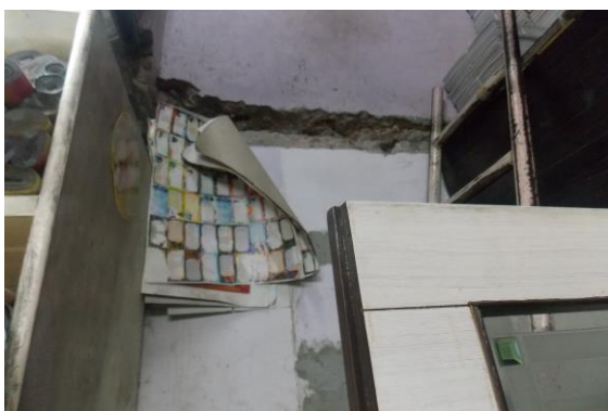
Photo 121 Peeling of Plaster on Wall No. 1 of Shop No.246 of Ground Floor
