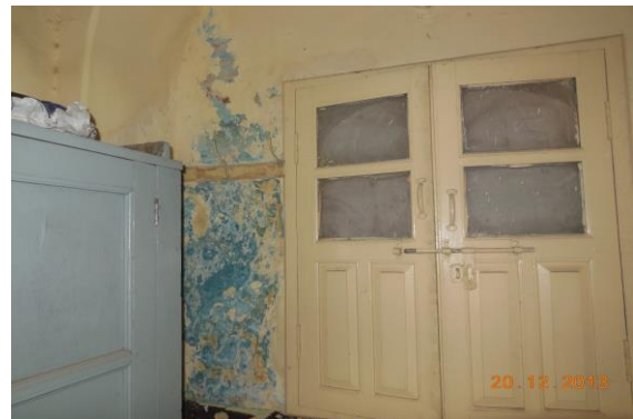
Photo 127 Peeling of Plaster on Wall No. 4 of Hall No. 3 of Part B of Hall. First Floor
