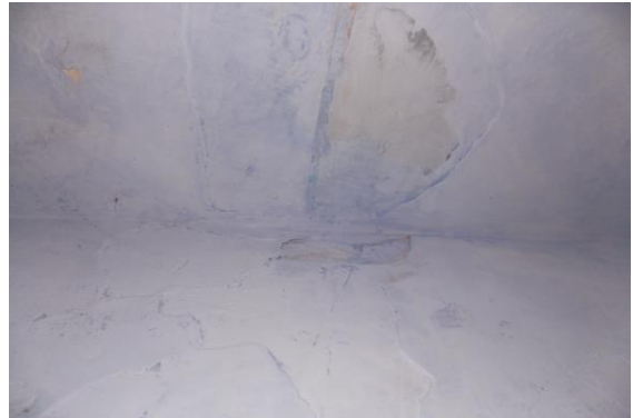
Photo 80 Peeling of Plaster on Wall No. 3 & Roof of Shop of Ground Floor
