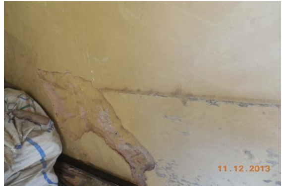
Photo 42 Peeling of Plaster on Wall No. 3 of Passage No.5 of First Floor
