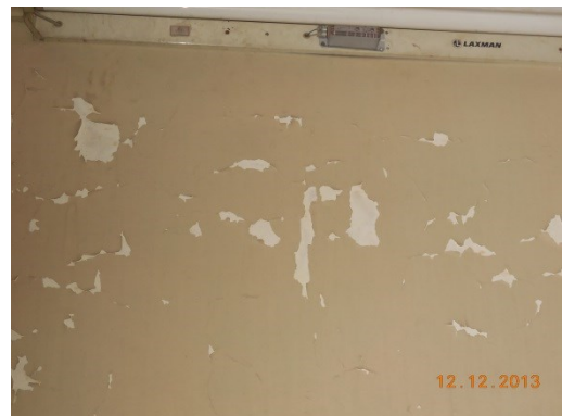
Photo 49 Peeling of Plaster on Wall No.3 of Room No.3 of H.No.481,First Floor
