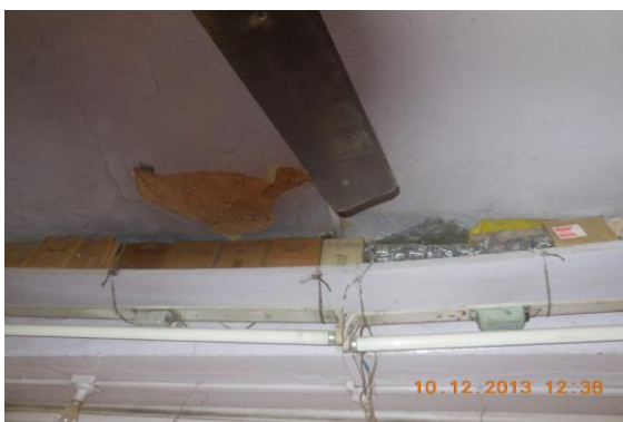
Photo 5 Peeling of Plaster on Roof of Shop No.362 of Ground Floor
