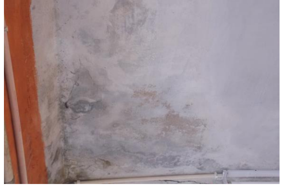
Photo 26 Dampness/Seepage on Roof of Varanda of Shop No.196 of Ground Floor
