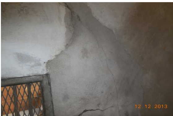
Photo 5 Inclined Crack on of Stair Case FF to SF, House No. 423, First Floor, Approx. Width = 0.6mm, Approx. Length = 1.3m. Distance from Wall No. 1 = 0.9m, Height from Floor = 1m.
