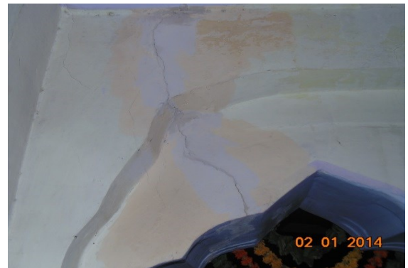
Photo 4 Inclined Crack on Wall No.3 of Varandah No.1 of Temple, First Floor, Approx. Width=0.60mm, Approx.Length= 1.50m. Distance from Wall No.2=1.20m, Height from Floor= 2.0m.
