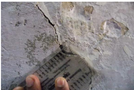
Photo 4A Inclined Crack on Wall No. 2 of Staircase, Ground Floor, Approx. Width = 2.5mm, Approx. Length = 1.8m. Distance from Wall no.3 = 2.3m, Height from Floor = 0m.
