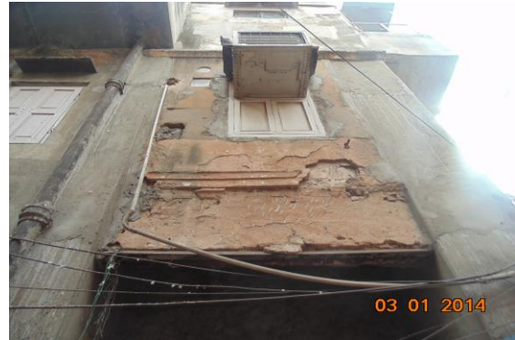
Photo 99 Peeling of Plaster on Entry Gate of Shop 3 of External façade
