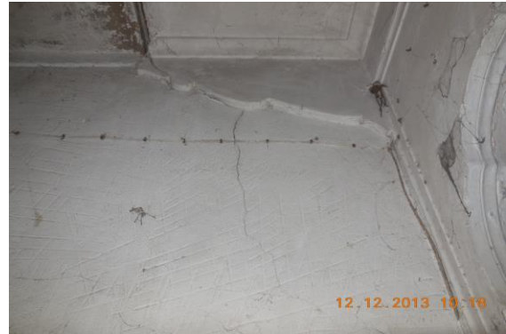
Photo 14 Inclined Crack on Wall No. 1 of Shop No. 3, Ground Floor, Approx. Width = 5mm, Approx. Length = 1.5m. Distance from w3 = 1.3m, Height from Floor = 2.2m.
