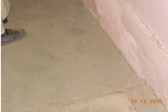
Photo 132 Peeling of Plaster on Floor of Passage No.1 of First Floor
