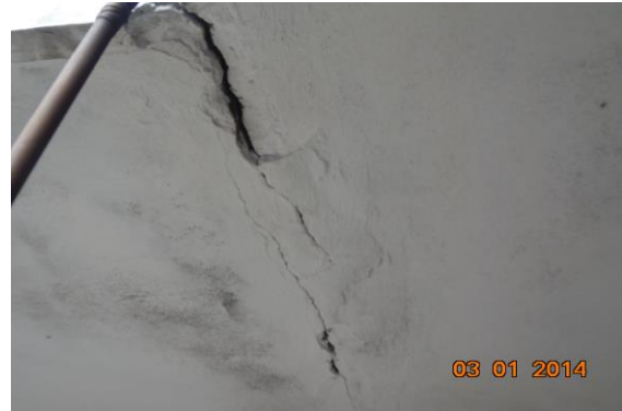
Photo 69 Peeling of Plaster on Balcony 4 Shed of Third Floor - Part A
