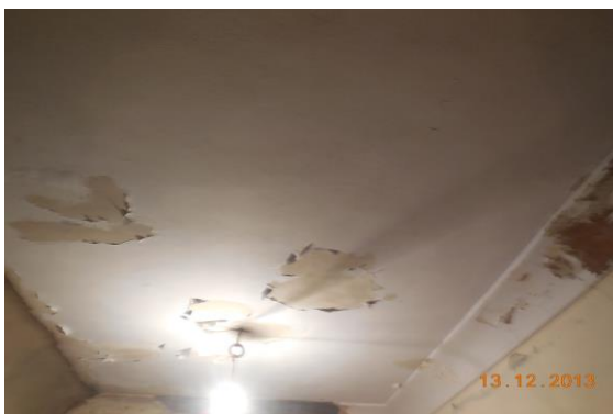
Photo 123 Peeling of Plaster on Roof of Room No. 7 of Second Floor
