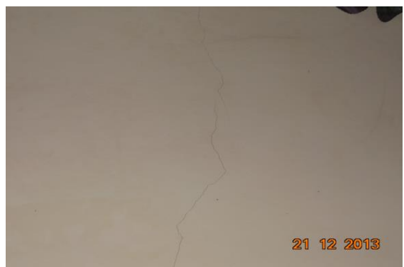
Photo 30 Inclined Crack on Wall No. 1 of, Library, Ground floor Approx. Width = 0.3mm, Approx. Length = 3m. Distance from = m, Height from Floor = m.
