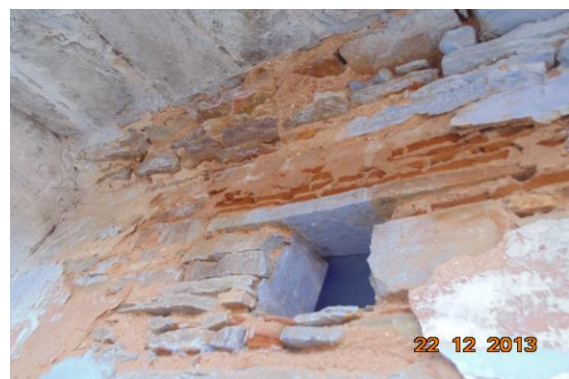
Photo 60 Damaged Portion on Shed of Gallery
