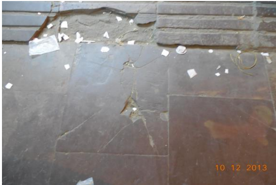
Photo 60 Damaged Portion on Floor of Varanda of Shop No. 304, Ground Floor
