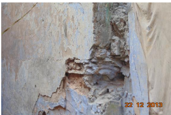
Photo 5 Peeling of Plaster on Wall No. 4 of Open Sky of First Floor
