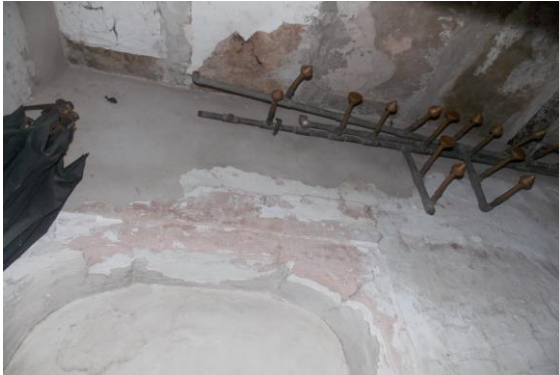
Photo 20 Dampness/Seepage on Wall No. 4 & Roof of Store of House No. 483, First Floor
