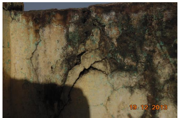
Photo 65 Peeling of Plaster on Wall No. 2 of Open Sky area of Second Floor
