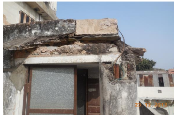
Photo 120 Damaged Portion on of Tower of Terrace
