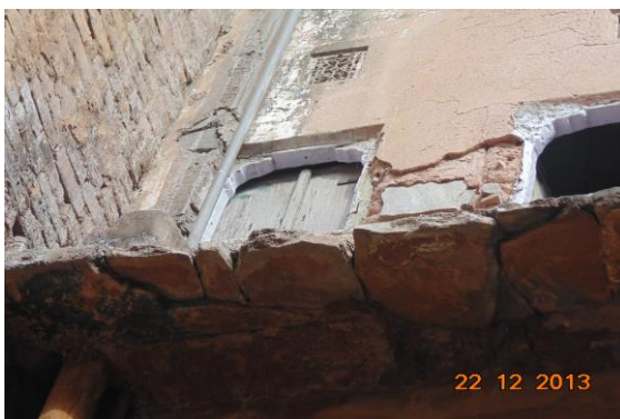
Photo 11 Peeling of Plaster on Outer Wall of Building of Ground Floor
