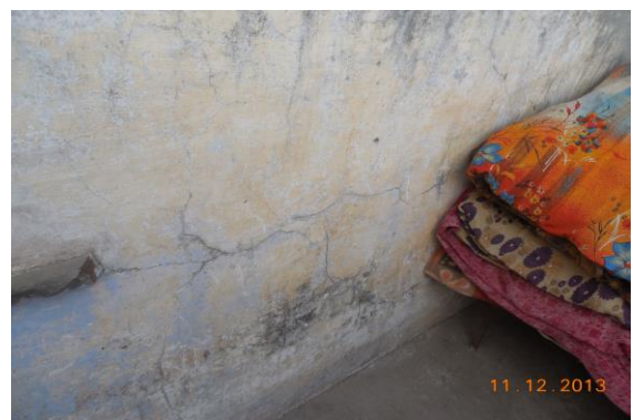
Photo 70 Plaster Crack on Wall No. 1 of Passage of Second Floor
