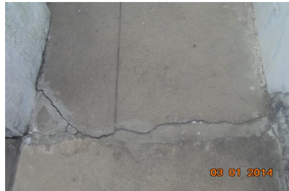
Photo 75 Plaster Crack on Parapet Wall No. 4 of Terrace
