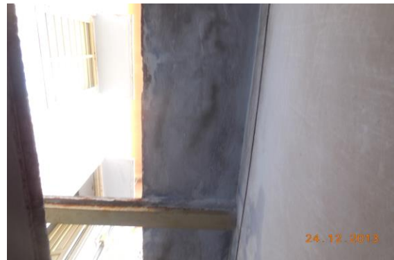
Photo 54 Dampness/Seepage on Wall No. 2 of Passage of First Floor
