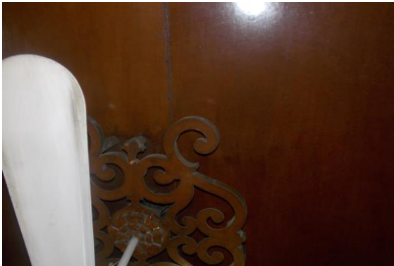
Photo 7 Plaster Crack on Floor of Shop No.235 of Ground Floor
