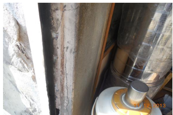
Photo 82 Plaster Crack on Wall No. Frontwall of Siyaram Treaders of Ground Floor
