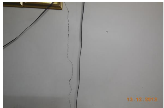
Photo 23 Inclined Crack on Dining Room, House No. 635, First Floor, Approx. Width = 1mm, Approx. Length = 3m. Distance from Wall No.3 = 1.85m, Height from Floor = 0m.
