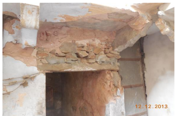
Photo 44 Peeling of Plaster on Sunshade of Open Area of House No. 424 Part A, Ground Floor
