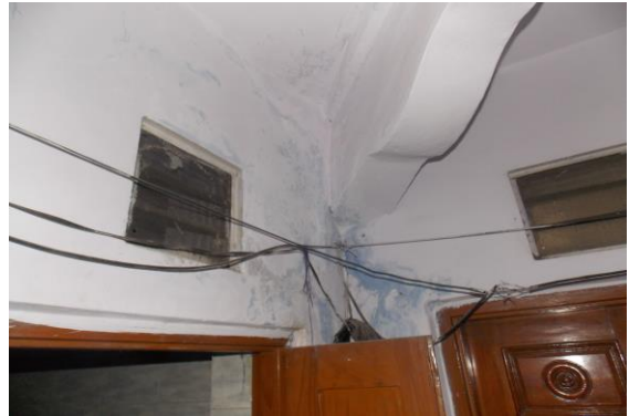
Photo 31 Dampness/Seepage on Wall No. 3 & 1 of Open sky Area of First Floor
