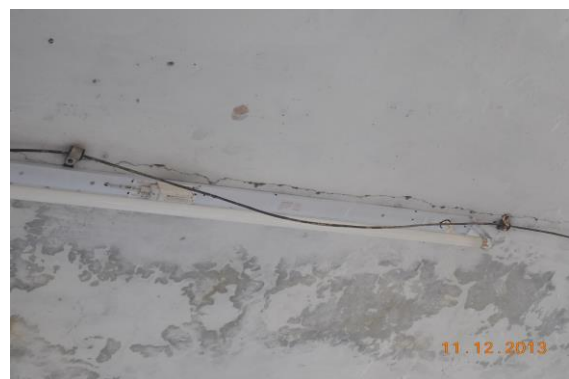
Photo 12 Horizontal Crack on Roof of Varanda of Shop No.316, Ground Floor Approx. Width = 1mm, Approx. Length = 3m. Distance from Left External Column = 0m, Height from Floor = 3m.
