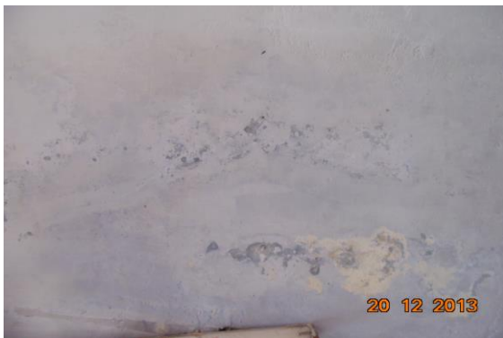
Photo 97 Dampness/Seepage on Roof of Vrandah of Shop no. 371, Ground Floor
