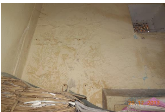
Photo 128 Dampness/Seepage on Wall No. 1 of Hall No. 3 of Part C of Hall. First Floor
