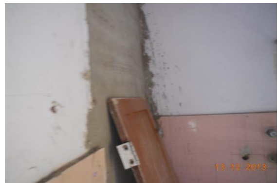
Photo 170 Peeling of Plaster on Outer Wall of Store of House No. 635, Second Floor
