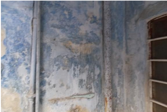
Photo 38 Peeling of Plaster on Wall No. 4 & 2 of Open sky Area of First floor
