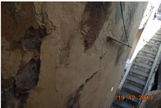
Photo 62 Peeling of Plaster on Wall No. 2 of Staircase First Floor to Second Floor of First Floor
