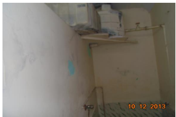
Photo 12 Peeling of Plaster on Wall No. 1 of Toilet No. 1 of Bank of Baroda, First Floor
