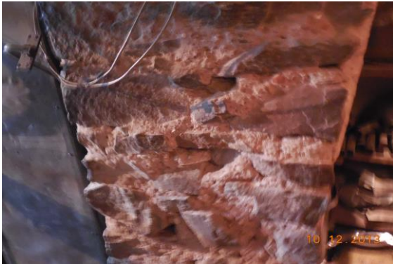
Photo 48 Peeling of Plaster on Part C of Shop No. 299, Ground Floor
