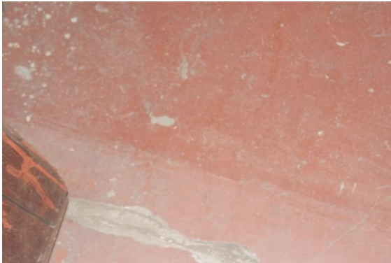
Photo 126 Peeling of Plaster on Floor of Hall No. 5 of Library, First Floor
