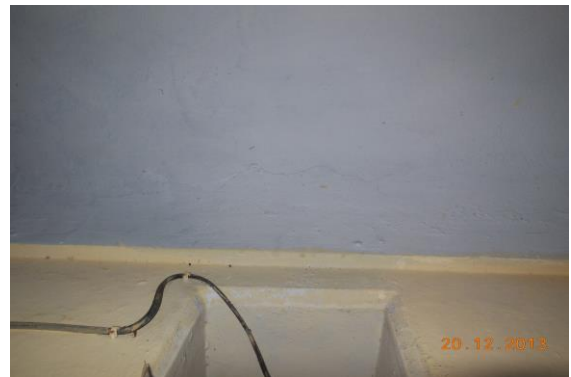
Photo 145 Peeling of Plaster on Roof of Kitchen of First Floor
