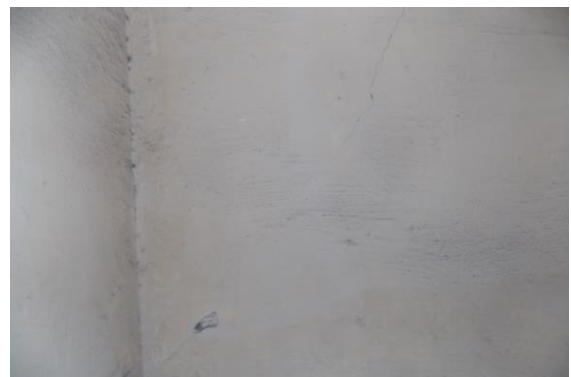
Photo 105 Peeling of Plaster on Wall No. 4 of Gallery of Library, First Floor
