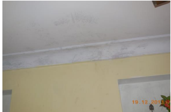
Photo 30 Dampness/Seepage on Wall No. 4 & Roof of Room No. 1 of First Floor
