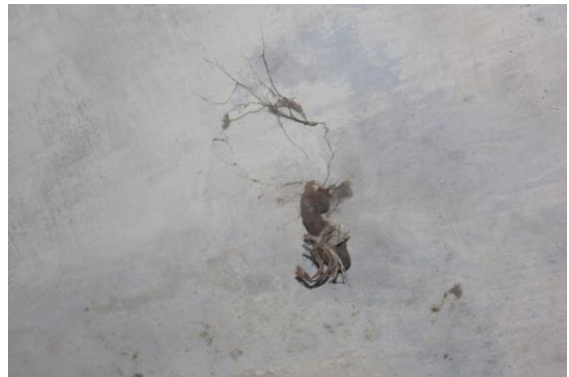
Photo 10 Peeling of Plaster on Roof of Varanda of Shop No.235 of Ground Floor
