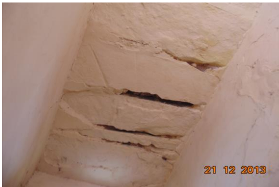
Photo 134 Peeling of Plaster on Roof of Staircase of Ground Floor
