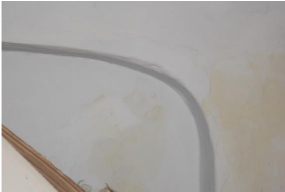
Photo 36 Dampness/Seepage on Wall No. 1 of Room No. 2 of First floor
