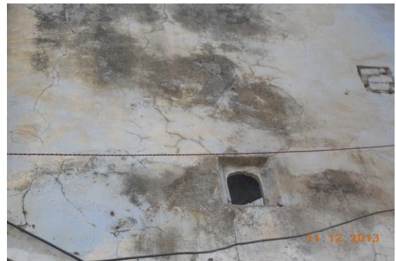
Photo 80 Plaster Crack on Wall No. Outerwall of First Floor
