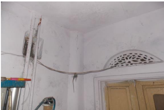
Photo 32 Dampness/Seepage on Wall No. 2 & 4 of Open sky area of First floor
