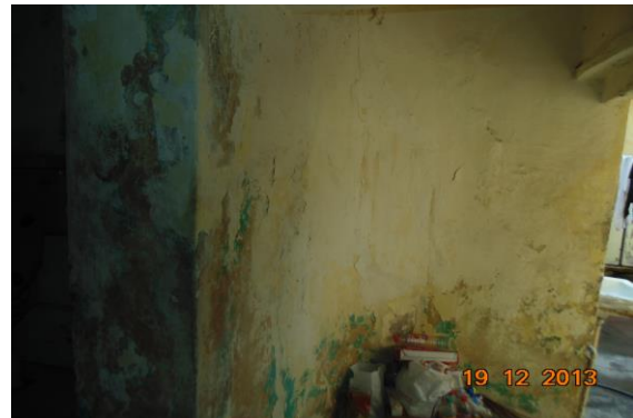
Photo 37 Dampness/Seepage on Wall No. 2 & 4 of Passage of First Floor
