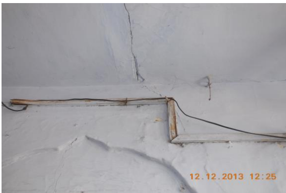
Photo 5 Inclined Crack on Wall No. 4 & Sunshade of Open Sky, House No. 483, First Floor, Approx. Width = 5mm, Approx. Length = 2.5m. Distance from Wall No. 1 = 1.6m, Height from Floor = 2.5m.
