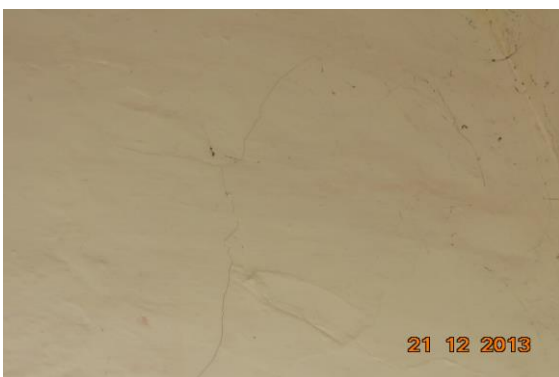
Photo 29 Inclined Crack on Wall No. 4 of Room No. 1, Library, Ground floor Approx. Width = 0.3mm, Approx. Length = 3m. Distance from = m, Height from Floor = m.
