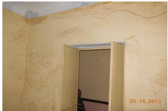
Photo 135 Dampness/Seepage on Wall No. 3 of Room No. 4 of First Floor
