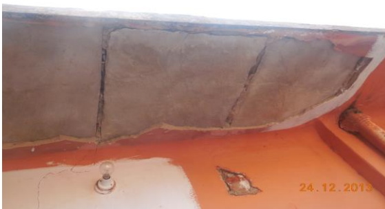
Photo 73 Damaged Portion on Shade of Hall No. 2 of Second Floor
