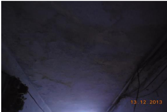
Photo 119 Dampness/Seepage on Roof of Passage-5 of House No. 635, First Floor
