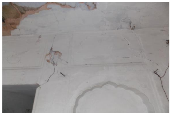
Photo 45 Peeling of Plaster on Wall No. 4 of Lobby No.1 of First Floor
