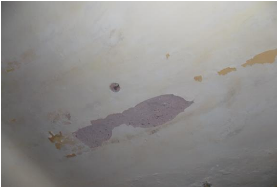
Photo 136 Peeling of Plaster on Roof of Hall No. 7 of Library, First Floor
