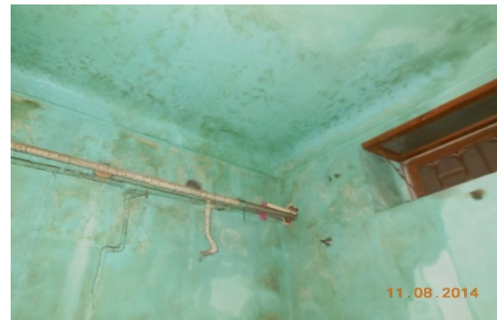
Photo 105 Seepage on All Walls of Toilet & Bath of Room No.12 of Hind Hotel, Second Floor
