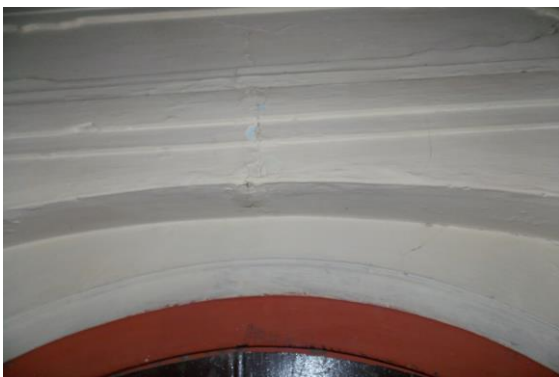
Photo 128 Peeling of Plaster on Wall No. 4 of Hall No. 5 of Library, First Floor
