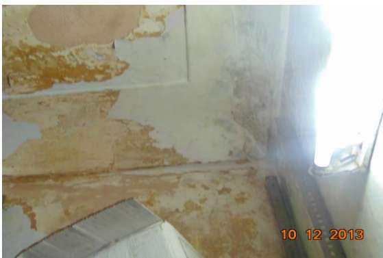
Photo 17 Peeling of Plaster on Wall No. 1 & Roof of Part-IV of Shop No.115 of First Floor
