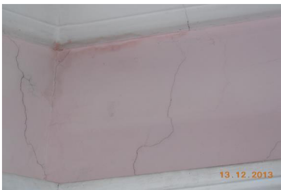
Photo 183 Plaster Crack on Wall No.1,3 & Roof, of Room No. 5 of Second Floor
