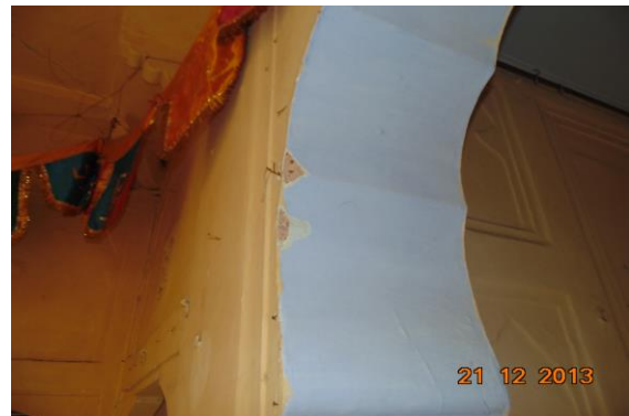
Photo 81 Peeling of Plaster on Wall No. 3 & Outer Wall of Varanda No.2 of Ground Floor
