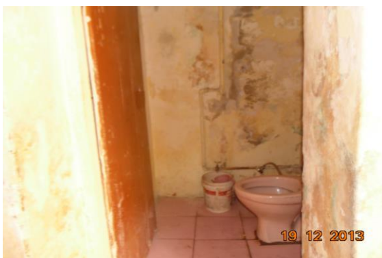
Photo 40 Dampness/Seepage on Left side Gate of Toilet No. 1 of First Floor
