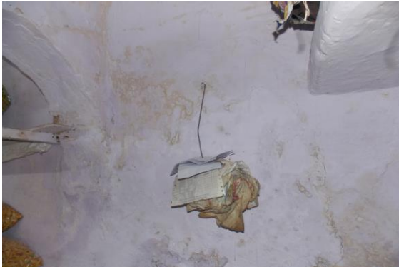
Photo 3 Dampness/Seepage on Shop No. 474 Part B of Ground Floor
