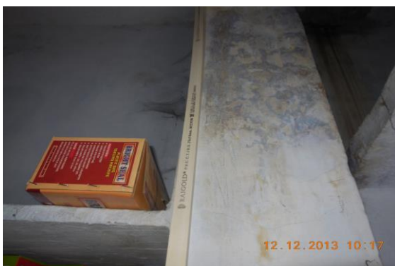
Photo 46 Dampness/Seepage on Wall No. 4 of Shop No. 2 of Ground Floor
