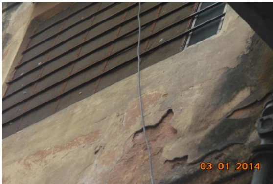
Photo 100 Peeling of Plaster on Shop 3 of External façade
