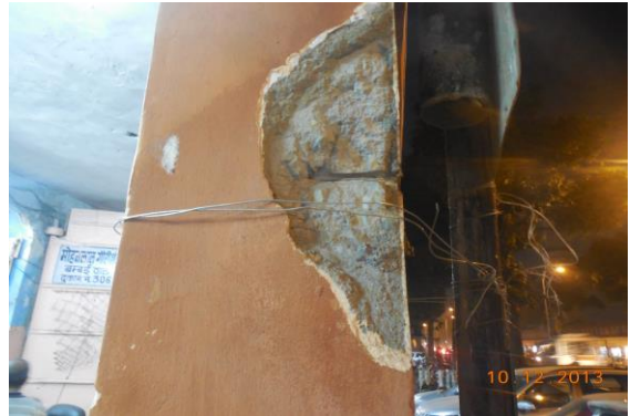
Photo 61 Damaged Portion on Right side External Beam of Shop No. 305 of Ground Floor
