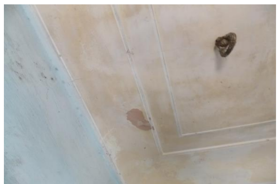
Photo 91 Peeling of Plaster on Roof of Room No. 4 of Third Floor
