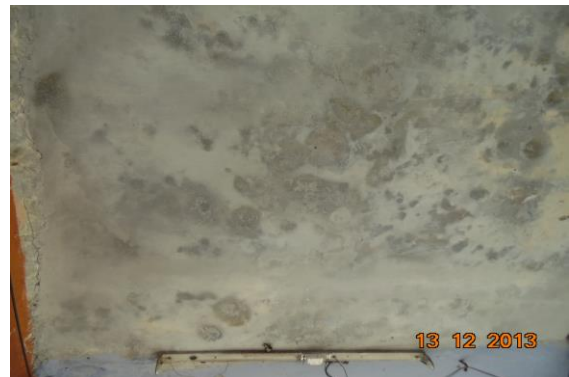
Photo 33 Dampness/Seepage on Roof of Varanda S.No.170A of Ground Floor
