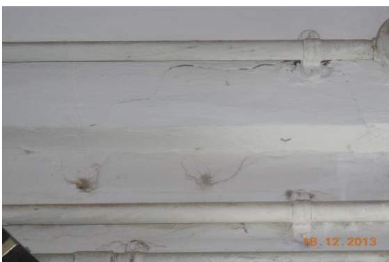
Photo 11 Inclined Crack on Roof of Hall No. 1, First Floor Approx. Width = 1mm, Approx. Length = 2m.
