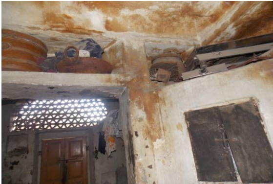
Photo 248 Dampness/Seepage on Wall No. 3 of Room No. 7 of First Floor
