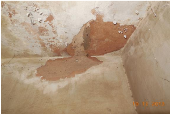
Photo 189 Peeling of Plaster on Roof & 4 of Staircase of First Floor
