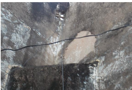
Photo 198 Peeling of Plaster on Wall No. 2 of Open Area of Ground Floor
