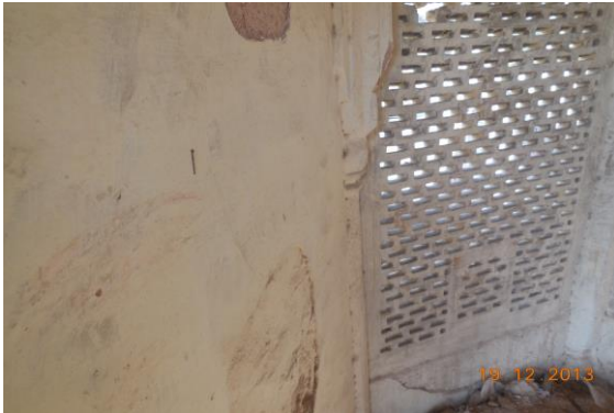
Photo 241 Peeling of Plaster on All walls & Roof of Tomb No.4 of Terrace
