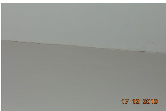
Photo 61 Peeling of Plaster on Roof of Inspect Room of First Floor
