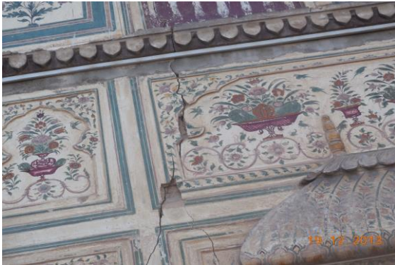
Photo 103 Damaged Portion on Wall No. 1 of Open Sky of Ground Floor
