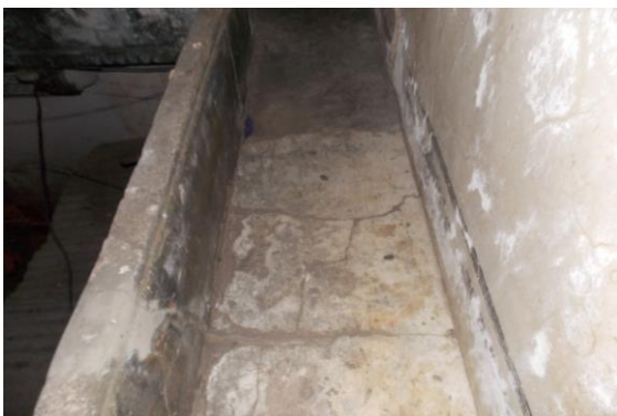
Photo 64 Plaster Crack on Floor of Open Sky of First floor
