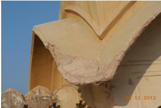
Photo 265 Damaged Portion on Roof Shade of Minarates No.8 of Terrace
