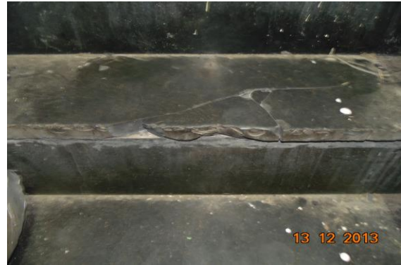
Photo 31 Dampness/Seepage on Stair Step GF to U/GF of Upper Ground Floor
