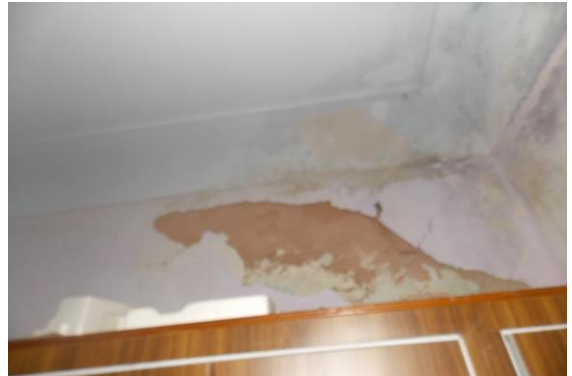
Photo 179 Peeling of Plaster on Wall No. 1 of Room No. 41 of Ground Floor
