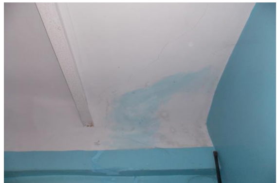
Photo 287 Dampness/Seepage on Roof of Room No. 16 of First Floor
