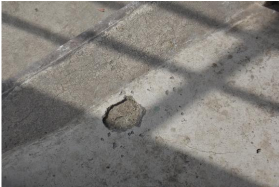
Photo 24 Peeling of Plaster on Floor of Tomb of Isarlat
