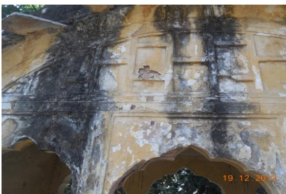
Photo 233 Peeling of Plaster on Outer Wall of Minarates No.3 of First Floor
