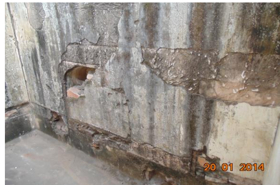
Photo 117 Peeling of Plaster on Wall No. 2 of Room No. 5 of First Floor, Tripoliya Gate
