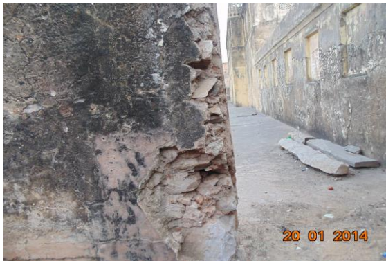
Photo 146 Peeling of Plaster on Wall No. 3 of Outer Wall of Tripoliya Gate, Terrace
