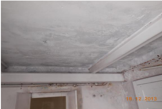
Photo 57 Dampness/Seepage on Roof of Hall No. 2 of First Floor
