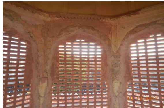
Photo 238 Peeling of Plaster on All walls of Tomb No.2 of Terrace
