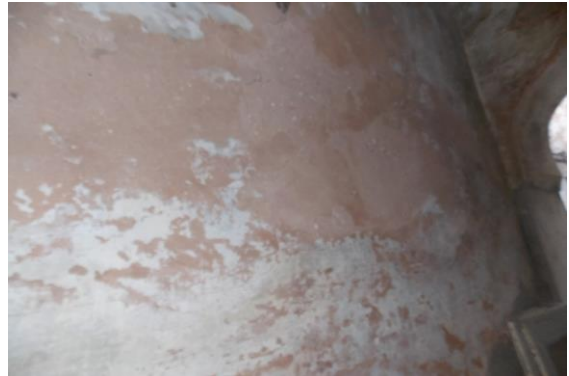
Photo 123 Peeling of Plaster on Wall No. 1 of Passage 1 of Ground Floor
