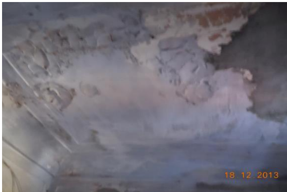
Photo 131 Peeling of Plaster on Roof of Gallery No.3 of Neel mani Ji Ka Temple, First Floor
