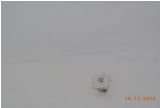
Photo 45 Plaster Crack on Wall No. 4 of Room No. 2 of First Floor
