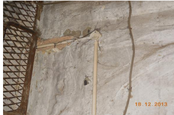
Photo 70 Peeling of Plaster on Wall No. 4 of Varanda No.1 of Ground Floor
