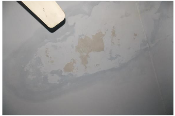
Photo 177 Peeling of Plaster on Roof of Room No. 41 of Ground Floor
