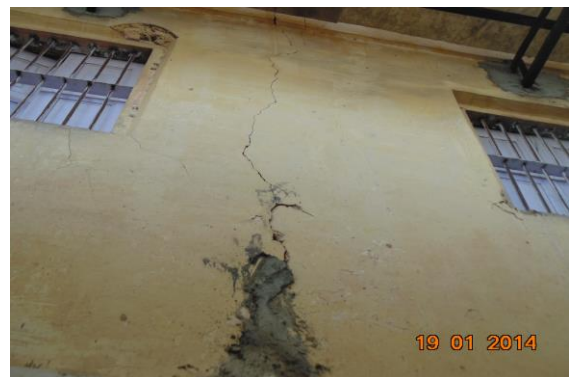
Photo 16 Inclined Crack on Wall No. 1 of , Police H.Q. First Floor, Part B, Approx. Width = 5mm, Approx. Length = 7m. Distance from Wall 4 = 3.2m, Height from Floor = 0m.
