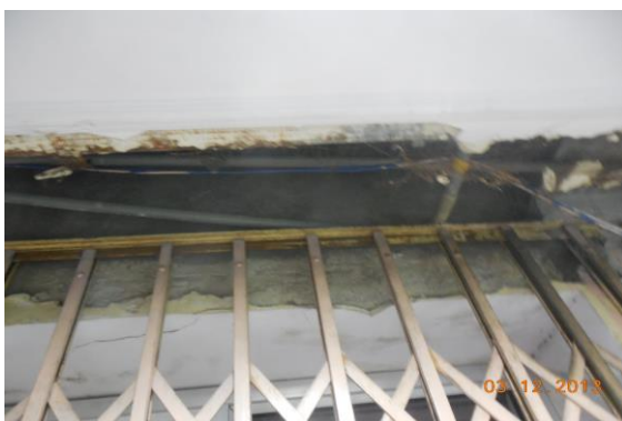
Photo 109 Peeling of Plaster on Wall No. 3 of Shop No. E 144 of Ground Floor
