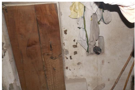
Photo 241 Dampness/Seepage on Wall No. 2 of Room No. 6 of First Floor
