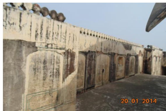
Photo 149 Peeling of Plaster on Wall No. 1 of Minarets of Tripoliya Gate, Terrace
