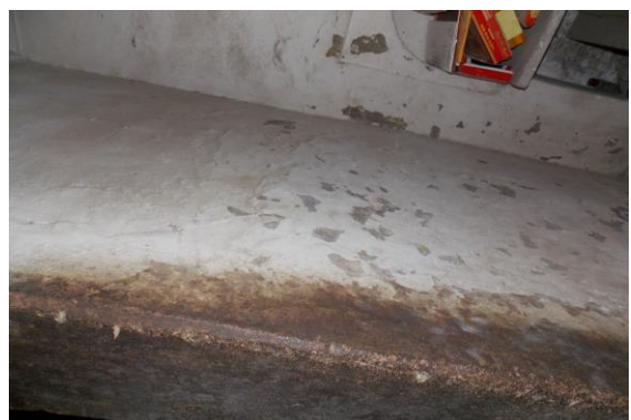
Photo 253 Peeling of Plaster on Wall No. 2 of Store 5 of First Floor
