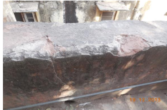
Photo 134 Peeling of Plaster on Wall No. 1 of Open Sky Area No.1 of First Floor
