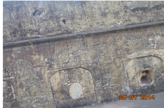
Photo 141 Peeling of Plaster on Wall No. 2 of Tripoliya Gate, Terrace
