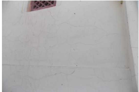
Photo 69 Plaster Crack on Wall No. 4, 5 & 6 of First Floor, Isarlat
