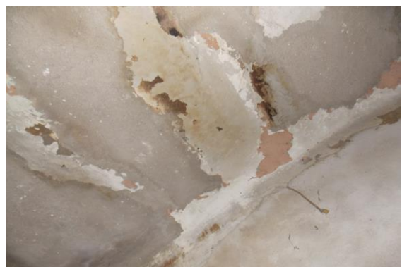
Photo 247 Peeling of Plaster on Roof of Room No. 7 of First Floor
