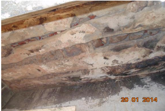
Photo 114 Peeling of Plaster on Roof of Room No. 4 of First Floor, Tripoliya Gate
