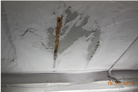
Photo 39 Peeling of Plaster on Roof of Hall No. 1 of First Floor
