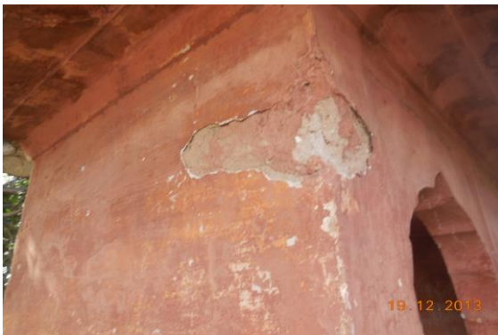
Photo 147 Peeling of Plaster on Outer Wall of Minarates No.1 of First Floor
