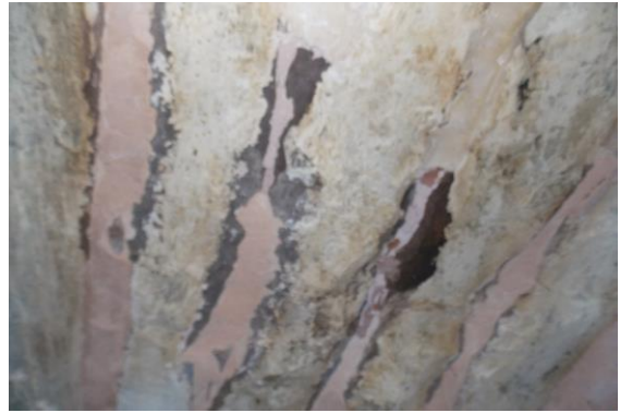
Photo 147 Dampness/Seepage on Roof of Room No. 19 of Ground Floor
