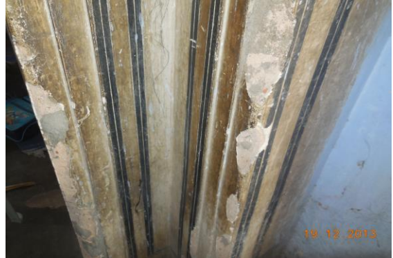
Photo 154 Peeling of Plaster on Wall No. 2 of Room No. 1 of School, First Floor
