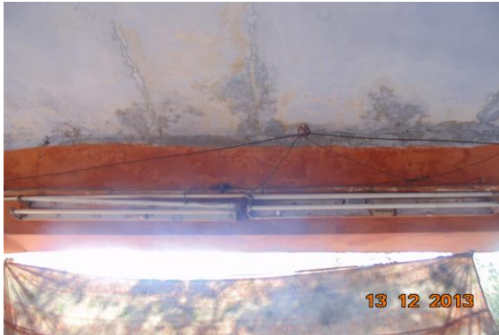
Photo 36 Dampness/Seepage on Roof & Beam of Varanda of Shop No. 171, Ground Floor
