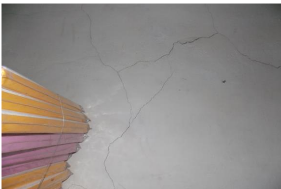
Photo 150 Plaster Crack on Wall No. 1 of Room No. 21 of Ground Floor
