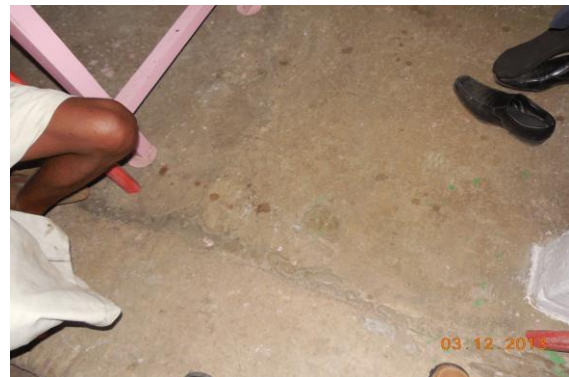
Photo 114 Peeling of Plaster on Floor of Part A of Shop No. D 53, Ground Floor
