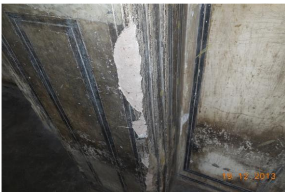
Photo 155 Peeling of Plaster on Wall No. 1 of Room No. 1 of School, First Floor
