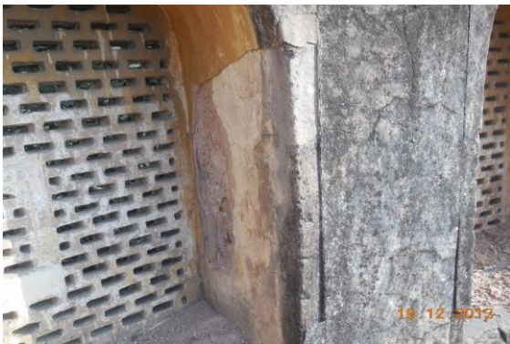
Photo 243 Peeling of Plaster on Wall No. 4 of School of Terrace
