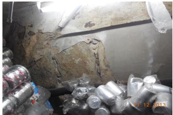
Photo 103 Peeling of Plaster on Roof of Part B of Shop No.167 of Ground Floor
