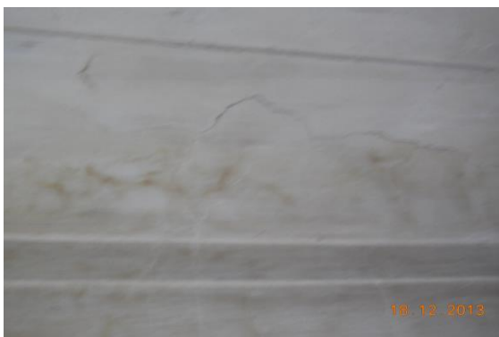
Photo 133 Plaster Crack on Roof of Gallery No.4 of Neel mani Ji Ka Temple, First Floor
