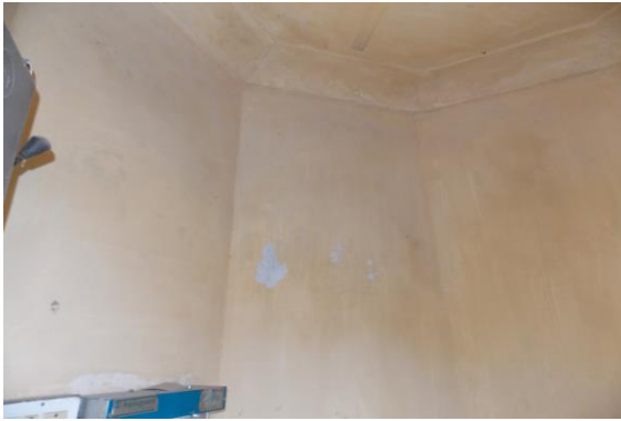
Photo 302 Peeling of Plaster on Wall No. 4 of Tomb 3 of First Floor
