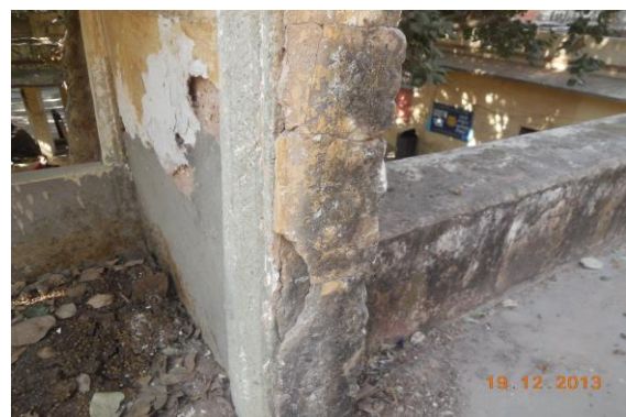
Photo 234 Peeling of Plaster on Outer Wall of Minarates No.3 of First Floor
