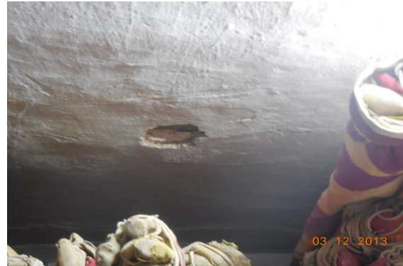
Photo 112 Peeling of Plaster on Roof of Part B of Shop No. D 54, Ground Floor
