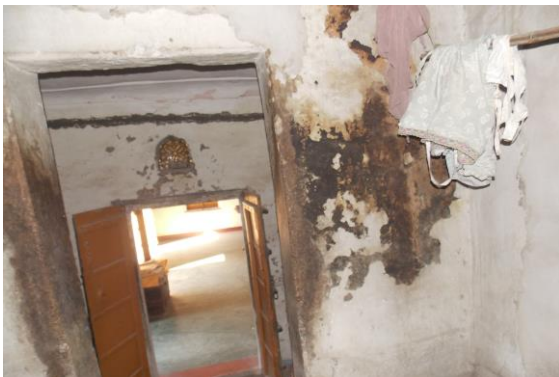
Photo 250 Dampness/Seepage on Wall No. 4 of Room No. 7 of First Floor
