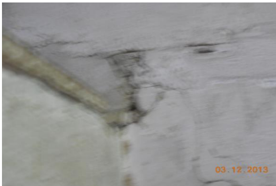
Photo 113 Peeling of Plaster of Stair of Shop No. D 54, Ground Floor
