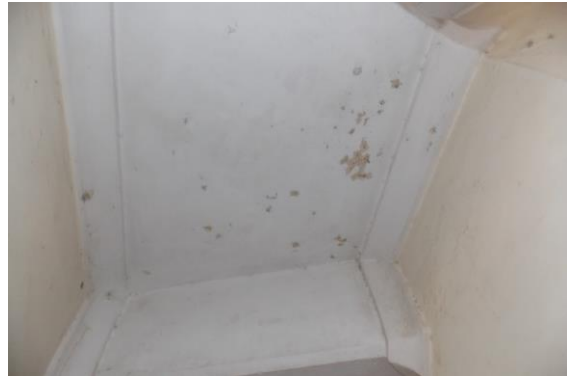
Photo 31 Peeling of Plaster on Roof of Stair of Isarlat
