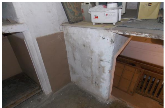
Photo 49 Dampness/Seepage on Wall No. 2 of Room No. 6 of Second Floor
