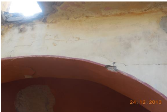
Photo 15 Peeling of Plaster on Backside of Gate No.1 of Ground Floor
