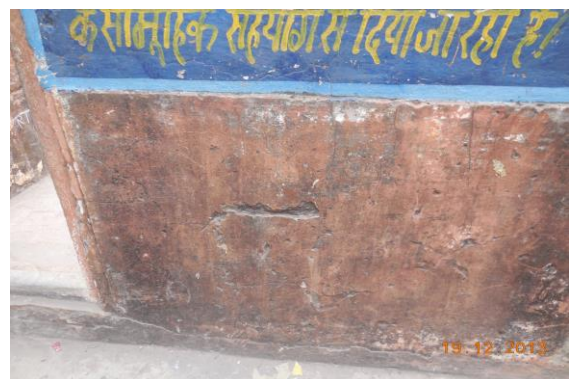
Photo 138 Peeling of Plaster on Wall No. 4 of Open Sky Area No.1 of First Floor
