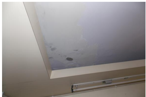
Photo 301 Dampness/Seepage on Roof of Room No. 22 of First Floor
