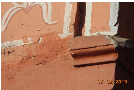
Photo 17 Damaged Portion on Wall No. 4 of Historical Gate No.2 of Ground Floor
