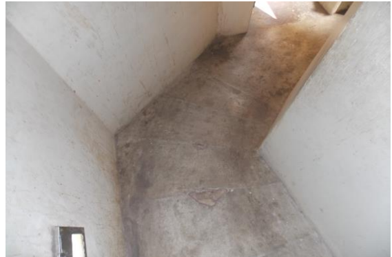
Photo 45 Peeling of Plaster on Stair Steps of Isarlat
