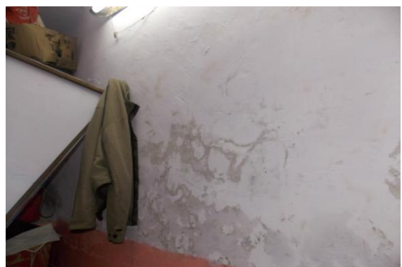
Photo 205 Dampness/Seepage on Wall No. 2 of Shop 1 of Ground Floor
