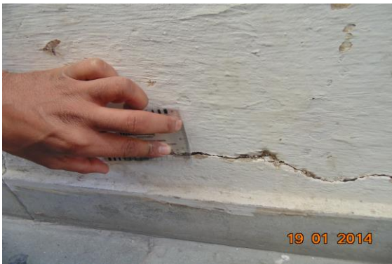
Photo 14A Horizontal Crack on Wall No. 1 of Passage 3, Police H.Q. First Floor, Part B, Approx. Width = 5mm, Approx. Length = 3m. Distance from Wall 4 = 0m, Height from Floor = 0.12m.
