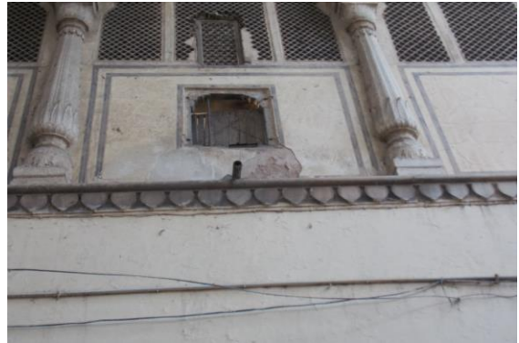
Photo 195 Peeling of Plaster on Wall No. 4 of Open Area of Ground Floor
