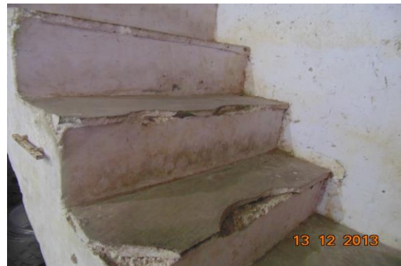
Photo 39 Dampness/Seepage on Stair Step of Shop No. 171, Basement
