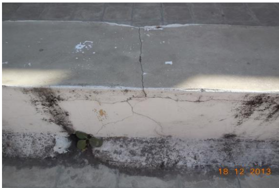
Photo 65 Damaged Portion on Parapet Wall of Post Office of First Floor
