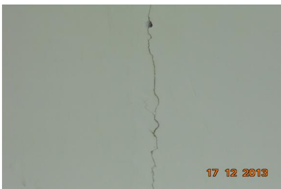
Photo 29 Inclined Crack on Wall No. 4 of Hall No. 2, Poornima Handicrafts, First Floor, Approx. Width = 0.35mm, Approx. Length = 2.5m. Distance from Wall No.1 = 0m, Height from Floor = 1m.
