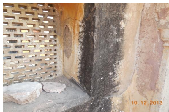
Photo 246 Peeling of Plaster on Wall No. 4 of School of Terrace
