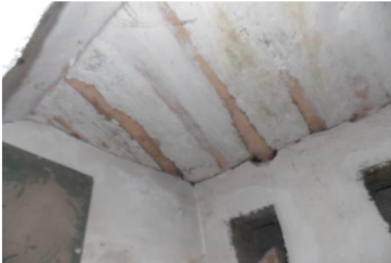
Photo 148 Dampness/Seepage on Roof of Room No. 20 of Ground Floor
