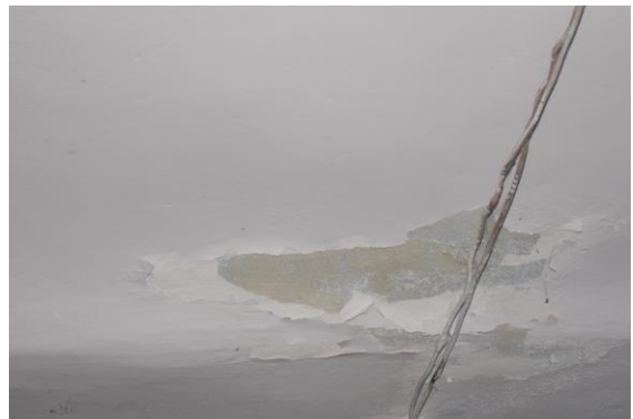
Photo 269 Peeling of Plaster on Roof of Room No. 12 of First Floor
