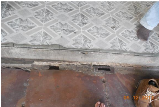
Photo 58 Peeling of Plaster on Floor of Shop No.139 of Ground Floor
