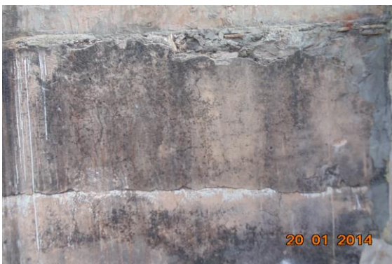
Photo 142 Peeling of Plaster on Wall No. 4 of Tripoliya Gate, Terrace
