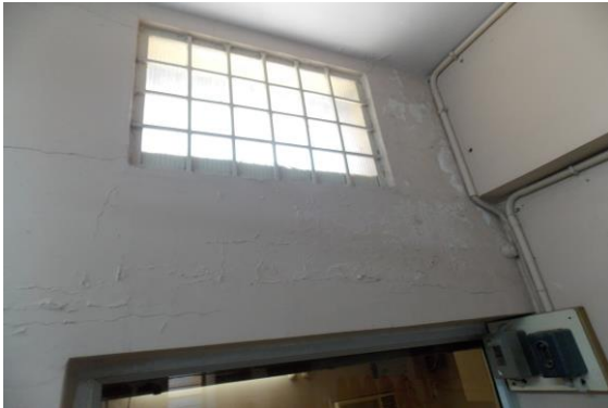
Photo 308 Peeling of Plaster on Wall No. 2 of Room No. 26 of First Floor
