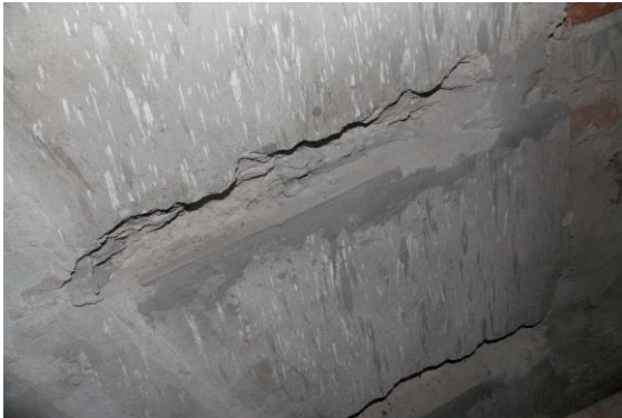
Photo 266 Peeling of Plaster on Wall No. 2 of Passage 1 of First Floor
