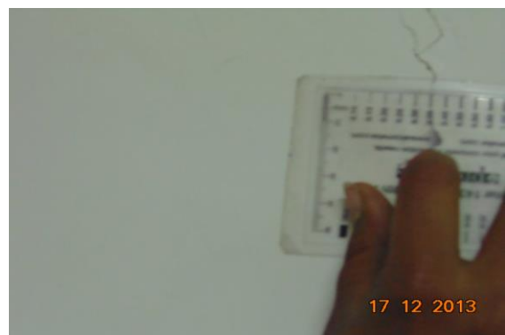
Photo 29A Inclined Crack on Wall No. 4 of Hall No. 2, Poornima Handicrafts, First Floor, Approx. Width = 0.35mm, Approx. Length = 2.5m. Distance from Wall No.1 = 0m, Height from Floor = 1m.
