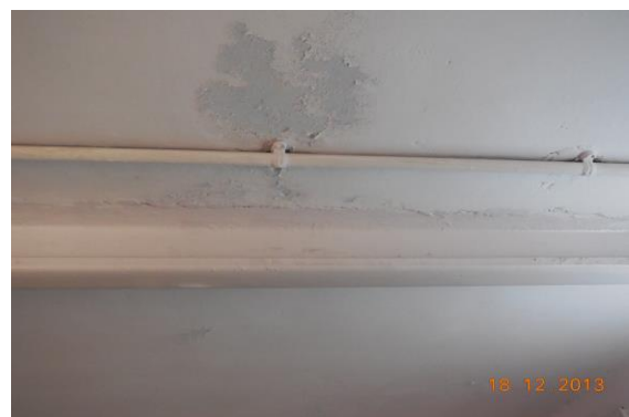
Photo 44 Dampness/Seepage on Roof of Room No. 1 of First Floor
