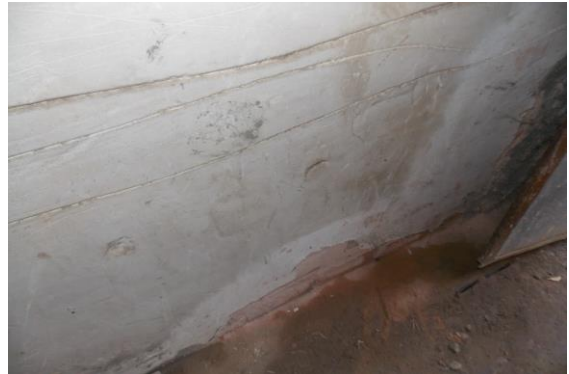
Photo 125 Peeling of Plaster on Wall No. 2 of Passage 1 of Ground Floor
