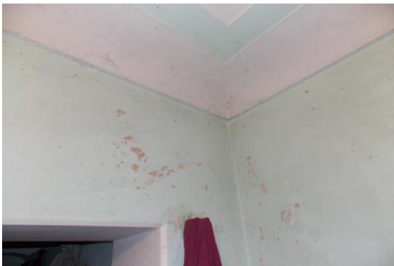
Photo 280 Peeling of Plaster on Wall No. 1 & 4 of Room No. 14 of First Floor
