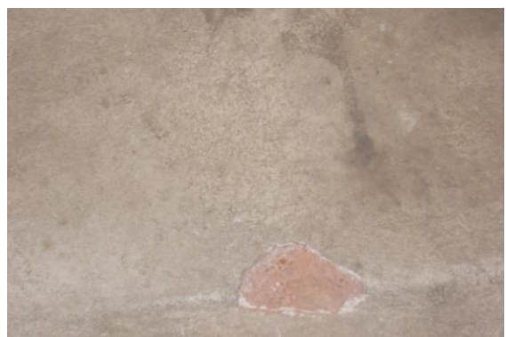
Photo 35 Peeling of Plaster on Stair Steps of Isarlat
