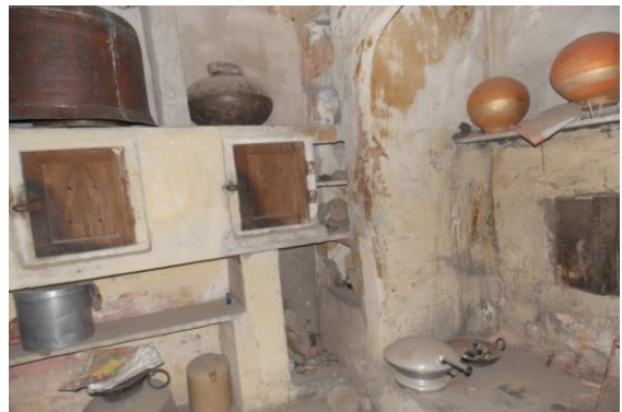
Photo 245 Peeling of Plaster on Wall No. 4 of Kitchen of First Floor
