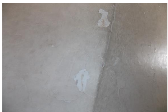
Photo 29 Peeling of Plaster on Wall No. 2 of Stair of Isarlat
