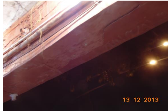
Photo 85 Peeling of Plaster on Roof & Beam of Varanda of Shop No. 187, Ground Floor
