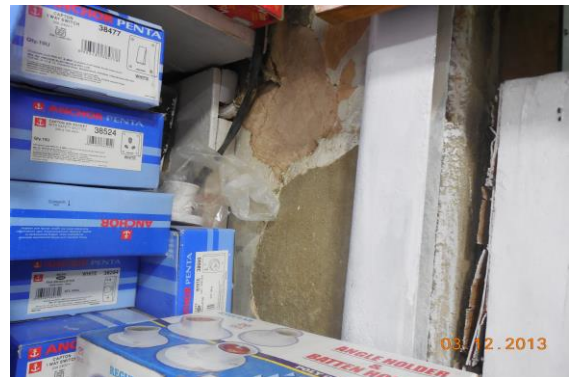
Photo 108 Peeling of Plaster on Wall No. 4 of Part A of Shop No. E 59, Ground Floor
