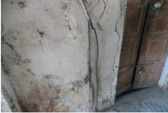
Photo 7 Inclined Crack on Wall No. 1 of Entry passage, Ground Floor Approx. Width = 5mm, Approx. Length = 2m.
