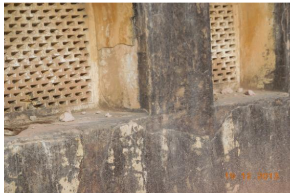
Photo 256 Peeling of Plaster on Wall No. 2 of School of Terrace
