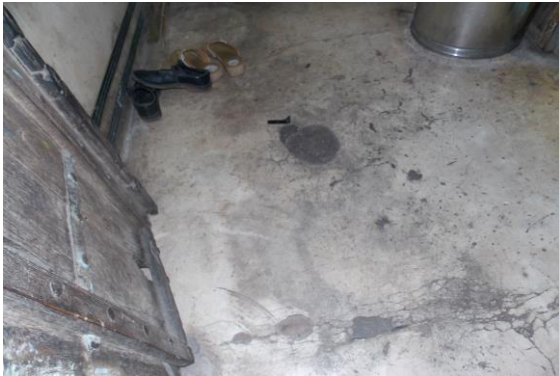
Photo 42 Peeling of Plaster on Floor of Store of First floor
