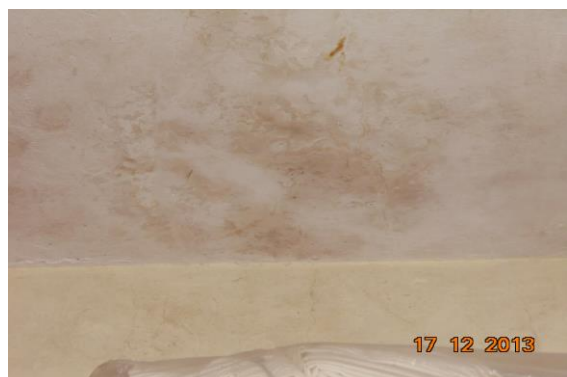
Photo 62 Dampness/Seepage on Roof of Store of First Floor
