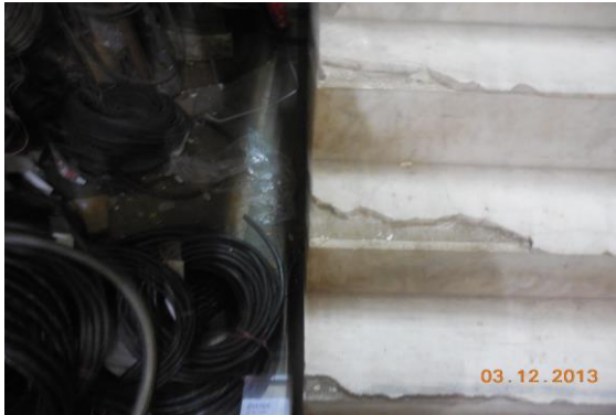
Photo 111 Peeling of Plaster on Tiles of Stair
