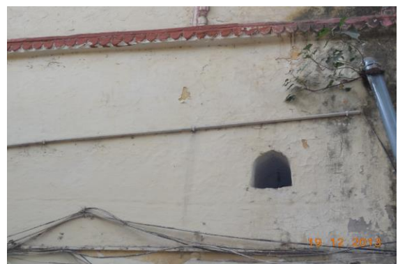
Photo 120 Peeling of Plaster on External Wall of of Lower First Floor
