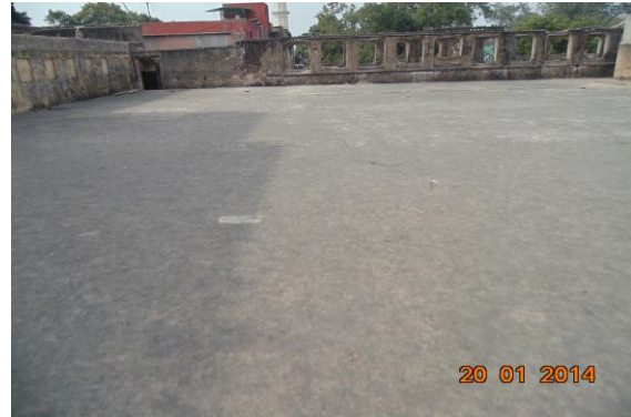
Photo 145 Peeling of Plaster on Floor of Tripoliya Gate, Terrace
