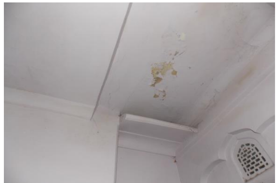
Photo 15 Plaster Crack on Roof of Room No. 3 of Navleshwar Temple, Ground Floor
