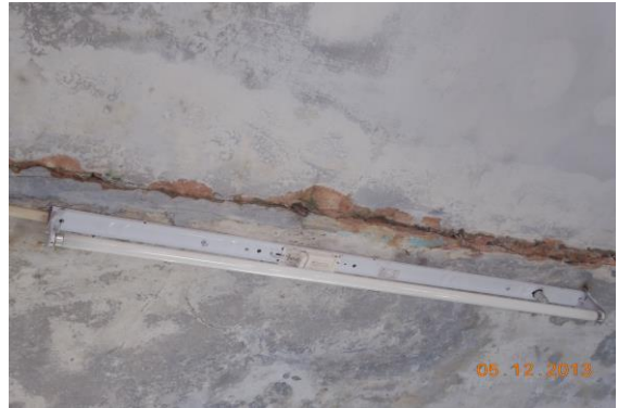
Photo 20 Horizontal Crack on Roof of Varanda of Shop, Ground Floor Approx. Width = 10mm, Approx. Length = 2.9m. Distance from Leftside External Column = 0m, Height from Floor = 3.9m.
