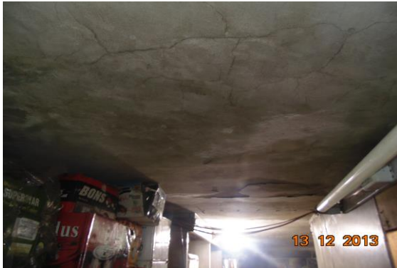
Photo 30 Peeling of Plaster on S.No.170A of Upper Ground Floor
