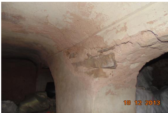
Photo 203 Peeling of Plaster on Roof of Part- N of Neel mani Ji Ka Temple, Basement
