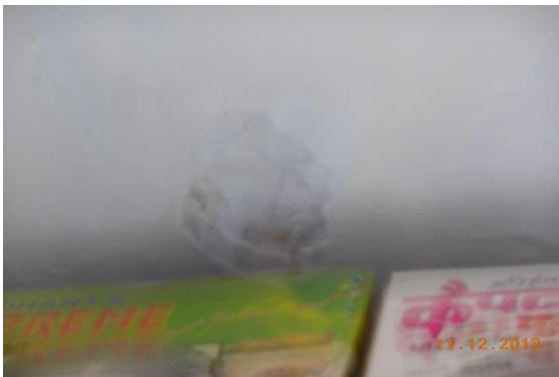
Photo 102 Peeling of Plaster on Roof of Part A of Shop No.167 of Ground Floor
