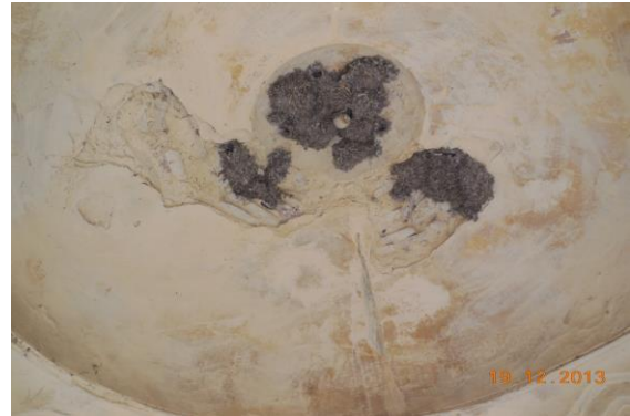
Photo 242 Peeling of Plaster on All walls & Roof of Tomb No.4 of Terrace
