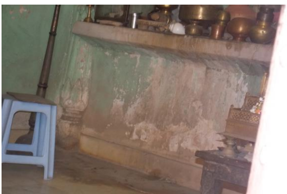
Photo 270 Peeling of Plaster on Wall No. 2 of Temple Area of First Floor
