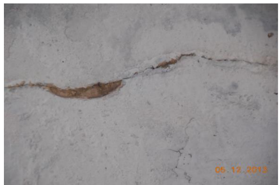
Photo 24 Inclined Crack on Roof of Varanda of Shop, Ground Floor Approx. Width = 0.3mm, Approx. Length = 2.9m. Distance from Leftside External Column = 1.3m, Height from Floor = 3m.
