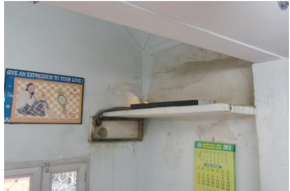
Photo 305 Peeling of Plaster on Wall No. 4 & 5 of Room No. 23 of First Floor
