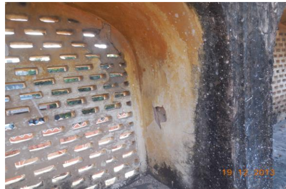
Photo 248 Peeling of Plaster on Wall No. 1 of School of Terrace
