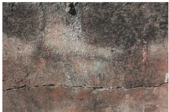
Photo 16 Inclined Crack on Wall No. 3 of Open Area 1, Second Floor Approx. Width = 2.5mm, Approx. Length = 3m. Distance from W2 = 0.25m, Height from Floor = 0.2m.
