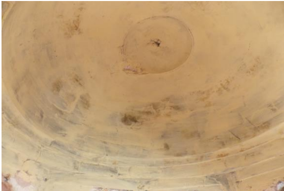
Photo 38 Dampness/Seepage on Roof of Tomb 2 of Second Floor
