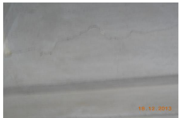
Photo 134 Plaster Crack on Roof of Gallery No.4 of Neel mani Ji Ka Temple, First Floor
