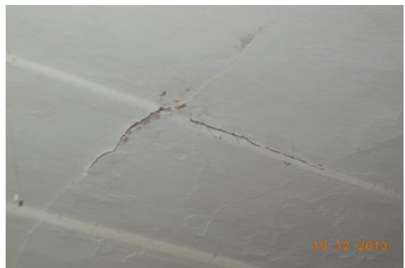
Photo 156 Peeling of Plaster on Roof of Room No. 1 of School, First Floor
