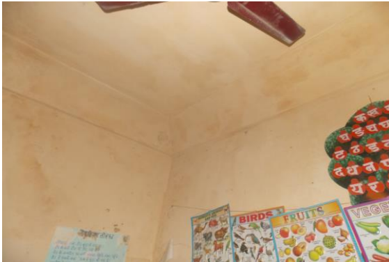
Photo 15 Dampness/Seepage on Wall No. 1, 4 & Roof of Room No. 1 of Ground Floor
