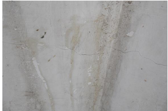
Photo 25 Plaster Crack on Wall No. 2 of Stair of Isarlat
