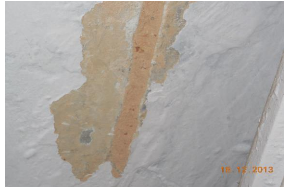
Photo 40 Peeling of Plaster on Roof of Hall No. 1 of First Floor
