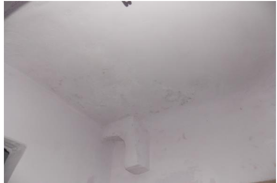
Photo 267 Dampness/Seepage on Roof of Bathroom of First Floor
