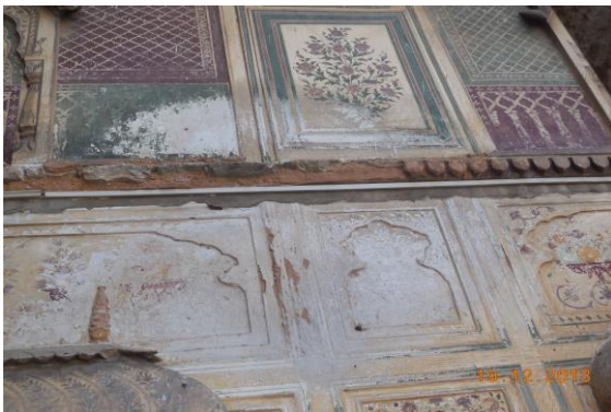
Photo 105 Peeling of Plaster on Wall No. 1 of Open Sky of Ground Floor
