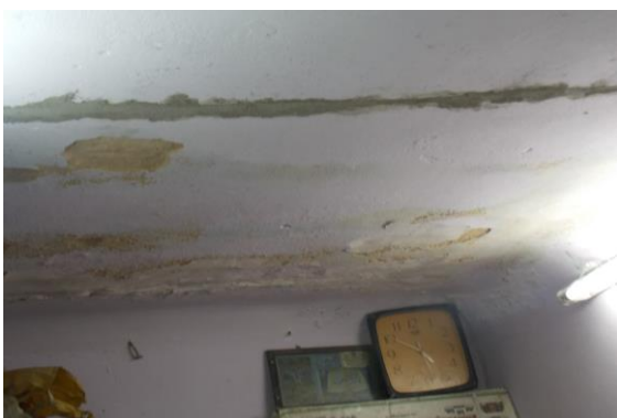
Photo 204 Dampness/Seepage on Roof of Room No. 1 of Ground Floor
