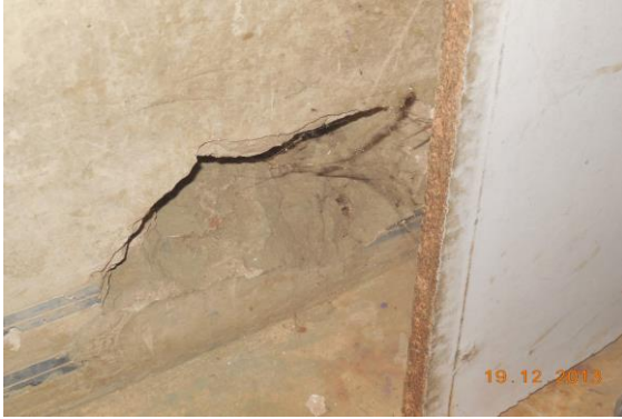
Photo 151 Damaged Portion on Wall No. 1 of Tomb No.2 of First Floor
