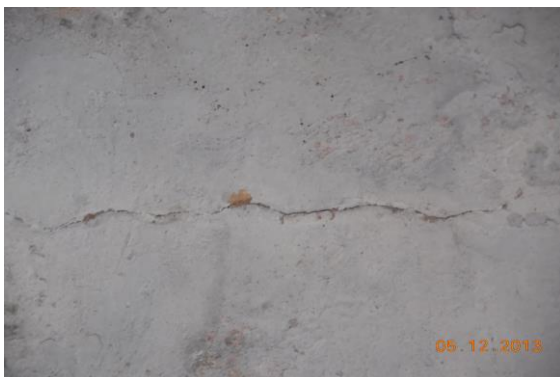
Photo 23 Inclined Crack on Roof of Varanda of Shop, Ground Floor Approx. Width = 0.3mm, Approx. Length = 2.9m. Distance from Leftside External Column = 1.1m, Height from Floor = 3m.
