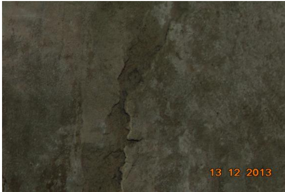
Photo 60 Plaster Crack on Part A of Shop No. 178, Basement
