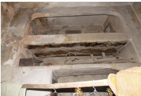
Photo 240 Dampness/Seepage on Wall No. 1 of Room No. 6 of First Floor
