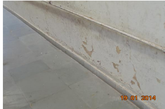
Photo 14 Horizontal Crack on Wall No. 1 of Passage 3, Police H.Q. First Floor, Part B, Approx. Width = 5mm, Approx. Length = 3m. Distance from Wall 4 = 0m, Height from Floor = 0.12m.
