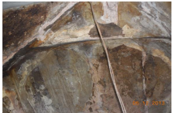
Photo 59 Peeling of Plaster on Roof of Part B of Shop of Ground Floor
