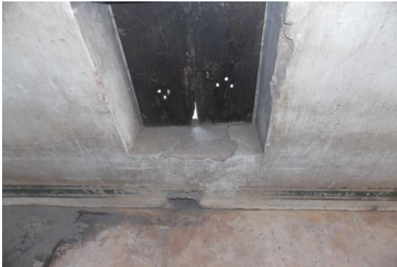
Photo 274 Peeling of Plaster on Wall No. 2 of Veranda of First Floor
