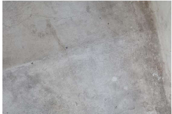
Photo 37 Plaster Crack on Stair Steps of Isarlat
