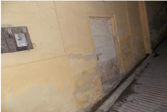
Photo 194 Peeling of Plaster on Wall No. 3 of Open Area of Ground Floor
