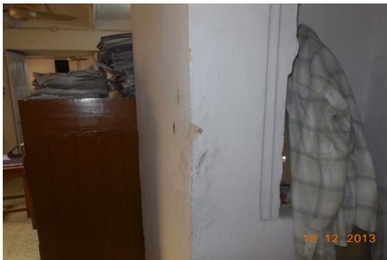
Photo 47 Peeling of Plaster on Wall No. 3 of Room No. 3 of First Floor
