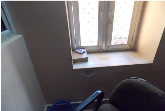
Photo 314 Peeling of Plaster on Wall No. 1 of Room No. 29 of First Floor
