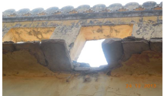
Photo 14 Peeling of Plaster on Roof Shed of Gate No.1 of Ground Floor
