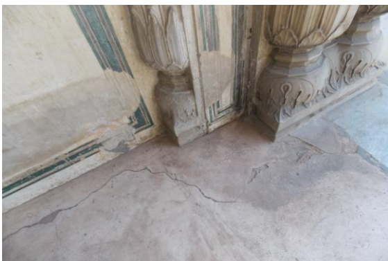
Photo 276 Peeling of Plaster on Floor of Veranda of First Floor
