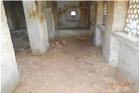
Photo 115 Peeling of Plaster on of Varanda No.1 of Lower First Floor
