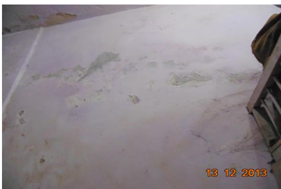
Photo 40 Dampness/Seepage on Basement of Shop No. 171, Basement
