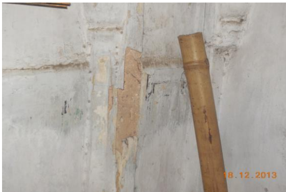
Photo 71 Peeling of Plaster on Wall No. 4 of Varanda No.1 of Ground Floor
