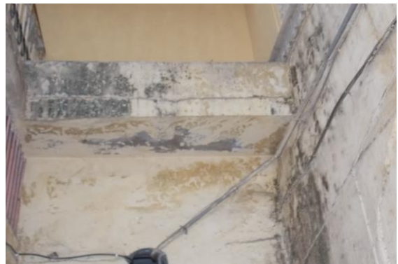
Photo 197 Dampness/Seepage on Wall No. 1 of Open Area of Ground Floor
