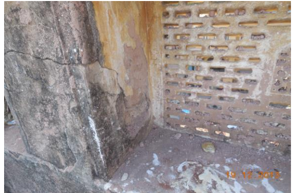
Photo 254 Peeling of Plaster on Wall No. 3 of School of Terrace
