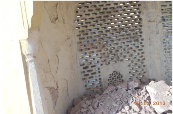
Photo 260 Peeling of Plaster on All walls & Roof of Tomb No.5 of Terrace
