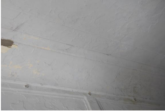
Photo 272 Dampness/Seepage on Roof of Veranda of First Floor
