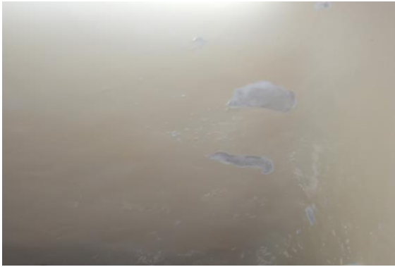
Photo 176 Peeling of Plaster on Roof of Room No. 37 of Ground Floor
