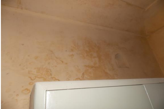
Photo 9 Dampness/Seepage on Wall No. 6 of Room No. 2 of Ground Floor
