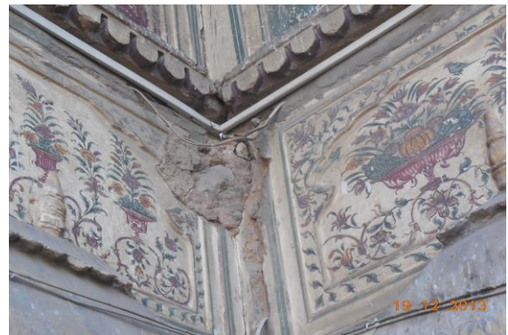
Photo 106 Peeling of Plaster on Wall No. 3 of Open Sky of Ground Floor
