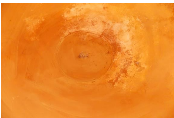
Photo 42 Dampness/Seepage on Roof of Tomb 4 of Second Floor
