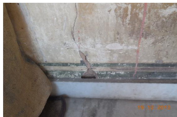
Photo 90 Peeling of Plaster on Wall No. 4 of Varanda No.4 of Ground Floor
