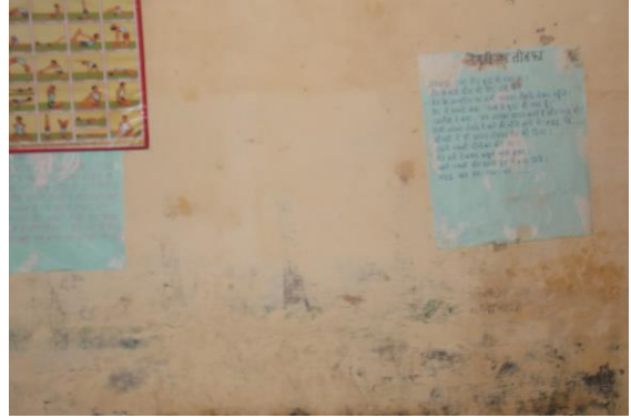
Photo 14 Dampness/Seepage on Wall No. 1 of Room No. 1 of Ground Floor
