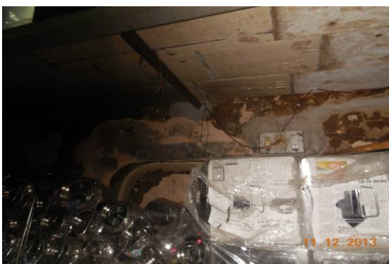
Photo 104 Peeling of Plaster on Wall No. 2 of Part B of Shop No.167 of Ground Floor
