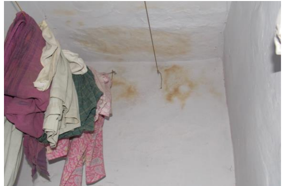
Photo 231 Dampness/Seepage on Wall No. 2 of Store 3 of First Floor
