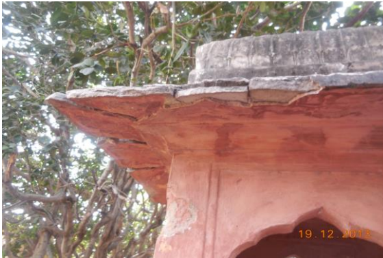
Photo 145 Damaged Portion on Sun Shade of Minarates No.1 of First Floor
