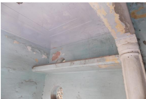
Photo 90 Peeling of Plaster on Wall No. 2 of Tomb of Third Floor
