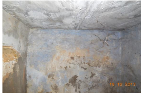
Photo 236 Dampness/Seepage on All walls of Toilet No. 1 of School, First Floor
