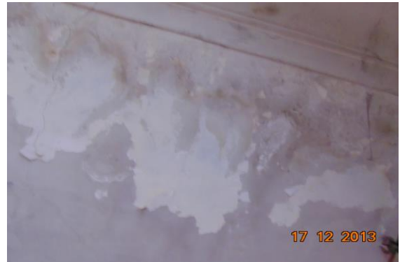
Photo 28 Dampness/Seepage on Roof of Varanda No.2 of Ground Floor
