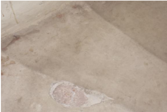
Photo 42 Peeling of Plaster on Stair Steps of Isarlat
