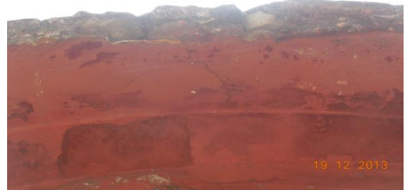
Photo 146 Damaged Portion on Sun Shade of Minarates No.2 of First Floor
