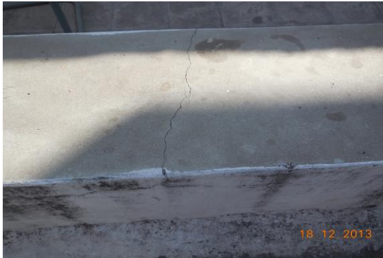
Photo 63 Damaged Portion on Parapet Wall of Post Office of First Floor
