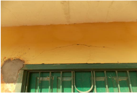
Photo 66 Peeling of Plaster on Wall No. 3 of First Floor, Isarlat
