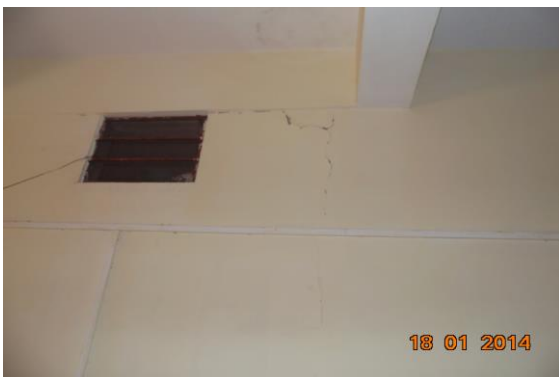
Photo 231 Plaster Crack on Wall No. 4 of Hall No. 4 of Police H.Q. Ground Floor, Part B
