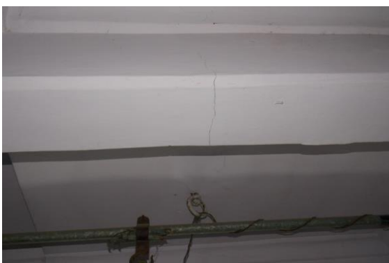
Photo 16 Plaster Crack on Roof & Beam of Room No. 3 of Navleshwar Temple, Ground Floor
