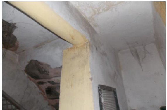
Photo 12 Dampness/Seepage on Wall No. 4 & Roof of Store of Ground Floor
