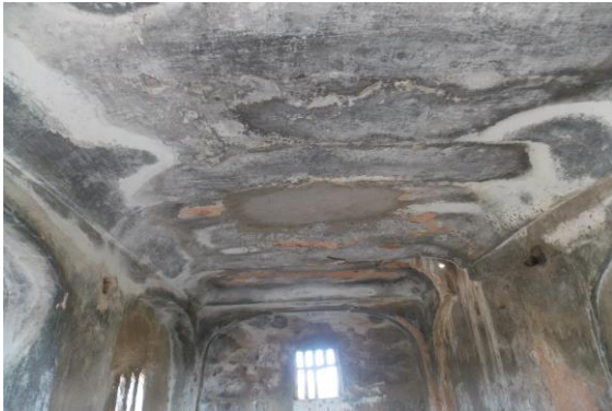
Photo 86 Peeling of Plaster on Roof of Room No. 2 of Third Floor
