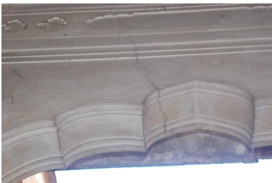
Photo 5 Inclined Crack on Wall No. 4 & Roof of Varanda No.1, Ground Floor Approx. Width = 3.5mm, Approx. Length = 6m. Distance from Wall No.1 = 1m, Height from Floor = 3.2m.
