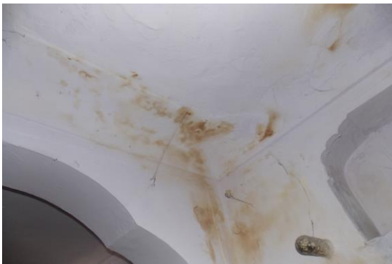
Photo 268 Dampness/Seepage on Roof of Room No. 11 of First Floor
