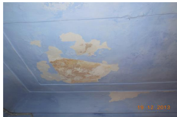
Photo 204 Peeling of Plaster on Roof of Room No. 13 of School, First Floor
