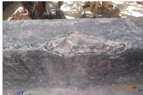
Photo 136 Peeling of Plaster on Wall No. 1 of Open Sky Area No.1 of First Floor
