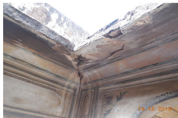
Photo 192 Damaged Portion on Sun Shade of Open Sky of First Floor
