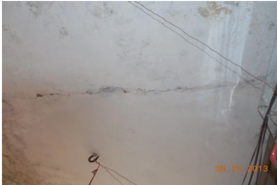
Photo 21 Horizontal Crack on Roof of Varanda of Shop, Ground Floor Approx. Width = 0.8mm, Approx. Length = 2.9m. Distance from Leftside External Column = 1.5m, Height from Floor = 3m.
