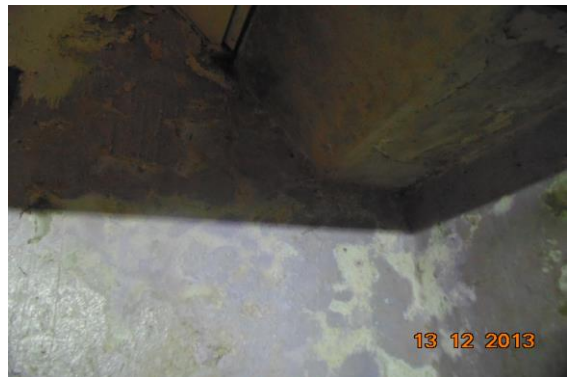
Photo 53 Dampness/Seepage on Roof, 1 & 4 of Stair Case of Shop No.175, Basement
