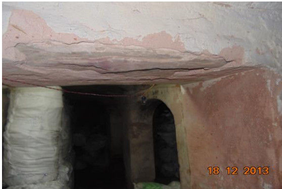
Photo 201 Peeling of Plaster on Roof of Part- M of Neel mani Ji Ka Temple, Basement
