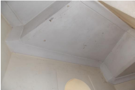
Photo 30 Peeling of Plaster on Roof of Stair of Isarlat
