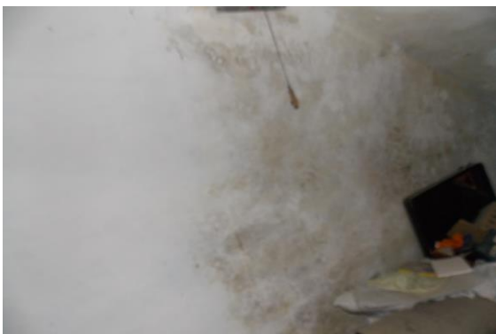
Photo 180 Dampness/Seepage on Wall No. 4 of Store 3 of Ground Floor
