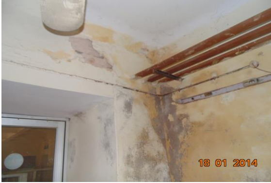
Photo 227 Peeling of Plaster on Wall No. 2 & 4 of Room No. 116 of Police H.Q. Ground Floor, Part B
