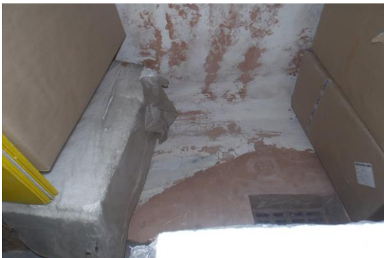
Photo 202 Dampness/Seepage on Wall No. 4 of Room No. 47 of Ground Floor
