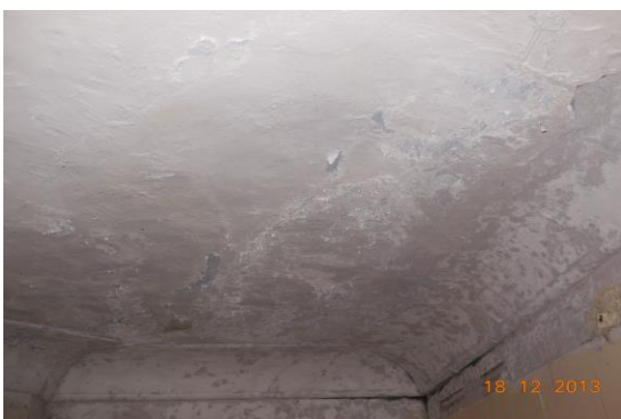
Photo 55 Dampness/Seepage on Roof of Toilet No. 1 of First Floor
