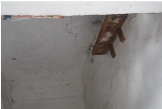
Photo 292 Peeling of Plaster on Roof of Room No. 17 of First Floor
