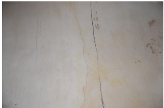
Photo 4 Inclined Crack on Wall No. 4 of Room No. 3, Hall No. 1, Ground Floor Approx. Width = 5mm, Approx. Length = 3m.
