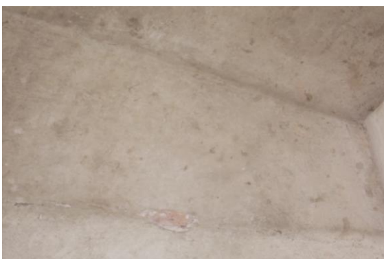
Photo 40 Peeling of Plaster on Stair Steps of Isarlat
