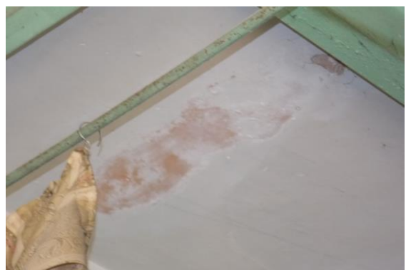
Photo 271 Peeling of Plaster on Roof of Temple Area of First Floor
