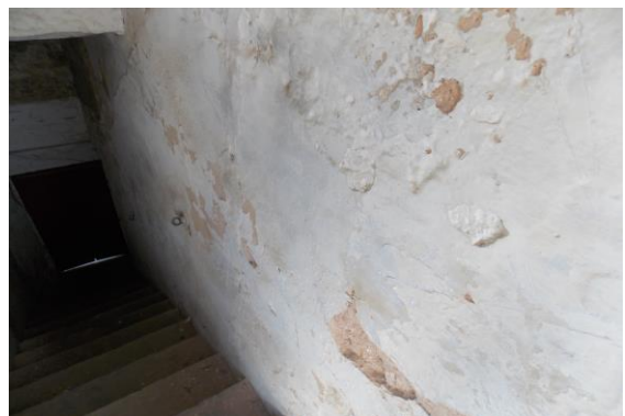
Photo 223 Peeling of Plaster on Wall No. 2 of Stair Case 1 of First Floor
