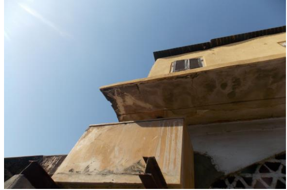
Photo 237 Peeling of Plaster on Sunshade & 3 of Open Area 3 of First Floor
