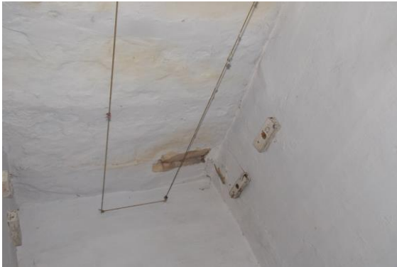
Photo 230 Peeling of Plaster on Roof of Store 3 of First Floor
