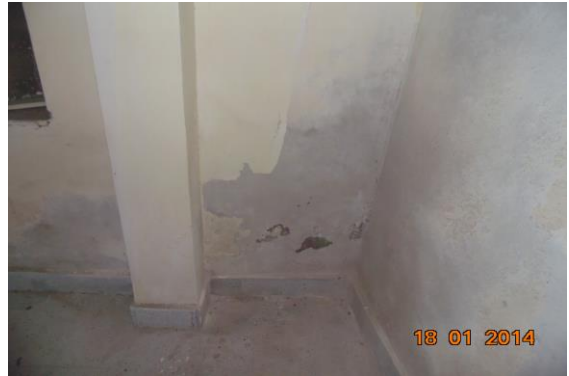
Photo 230 Peeling of Plaster on Wall No. 2 of Hall No. 4 of Police H.Q. Ground Floor, Part B
