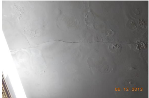
Photo 22 Horizontal Crack on Roof of Shop No.138, Ground Floor Approx. Width = 0.35mm, Approx. Length = 3.3m. Distance from Wall No.3 = 4m, Height from Floor = 3m.
