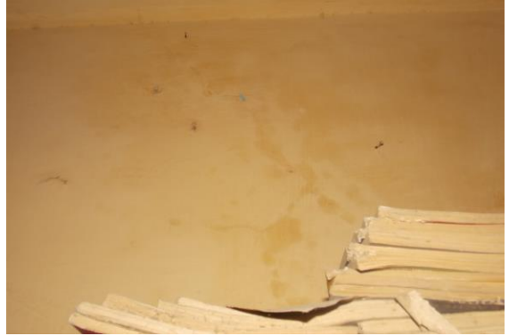
Photo 8 Dampness/Seepage on Wall No. 5 of Room No. 2 of Ground Floor
