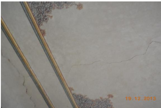
Photo 87 Plaster Crack on Roof of Varanda No.3 of Ground Floor
