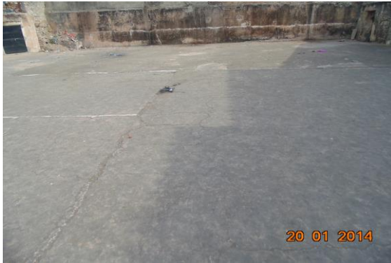
Photo 144 Peeling of Plaster on Floor of Tripoliya Gate, Terrace
