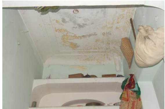
Photo 279 Dampness/Seepage on Roof of Kitchen 2 of First Floor
