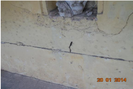
Photo 138 Peeling of Plaster on Wall No. 2 of Tripoliya Gate, Terrace
