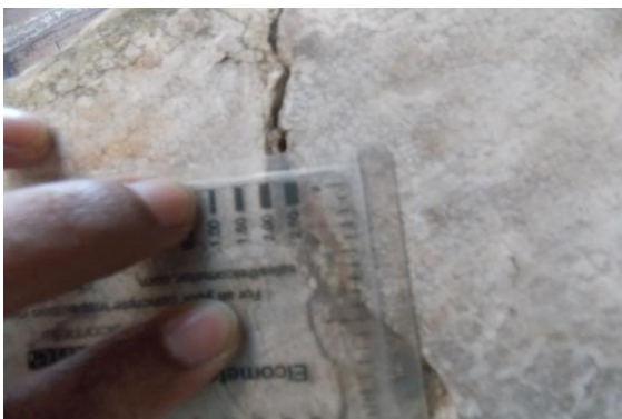
Photo 15A Inclined Crack on Wall No. 2 of Teenset 2, Second Floor Approx. Width = 2.5mm, Approx. Length = 1.5m. Distance from W1 = 4m, Height from Floor = 0.3m.
