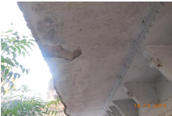
Photo 53 Damaged Portion on Roof Shade of Passage of First Floor
