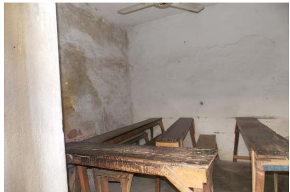
Photo 293 Peeling of Plaster on Wall No. 1 of Room No. 17 of First Floor
