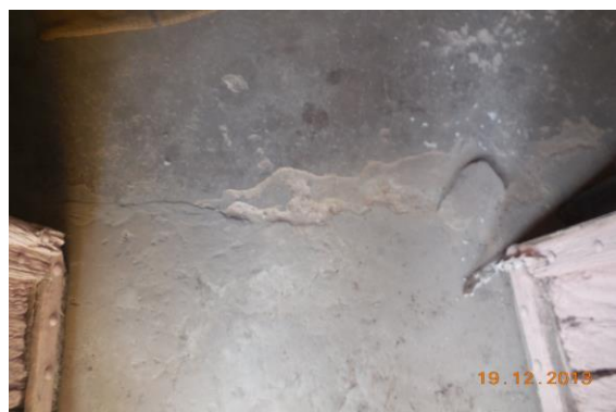
Photo 60 Peeling of Plaster on Floor of Room No. 5 of Ground Floor
