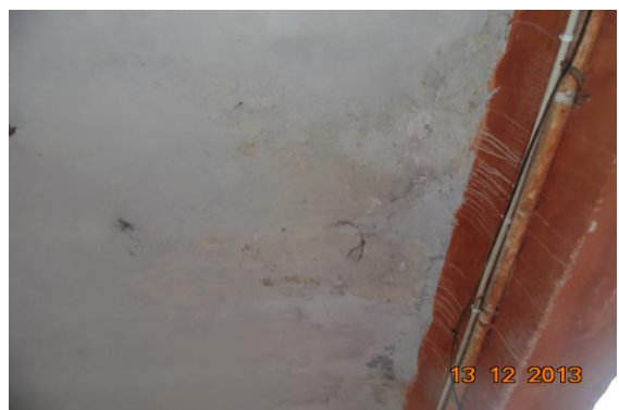
Photo 65 Dampness/Seepage on Roof of Varanda of Shop No. 179, Ground Floor
