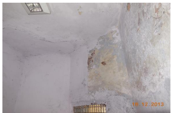
Photo 56 Dampness/Seepage on Wall No. 4, 2 & Roof of Toilet No. 1 of First Floor
