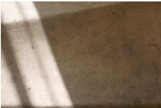
Photo 38 Plaster Crack on Stair Steps of Isarlat
