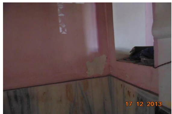
Photo 32 Peeling of Plaster on Wall No. 2 of Room No. 1 of Temple Shri Sankat Haran Mahadev, Ground Floor
