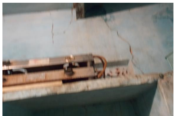
Photo 6 Inclined Crack on Wall No. 1 of Room No. 1, Navleshwar Temple, Ground Floor Approx. Width = 5mm, Approx. Length = 4m. Distance from Wall No.2 = 0.9m, Height from Floor = 2m.
