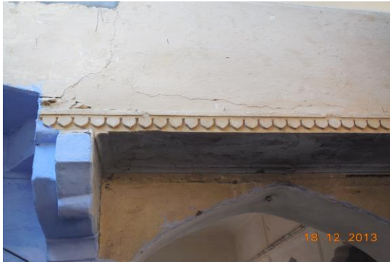
Photo 69 Plaster Crack on Inside Gate of Post Office of Ground Floor
