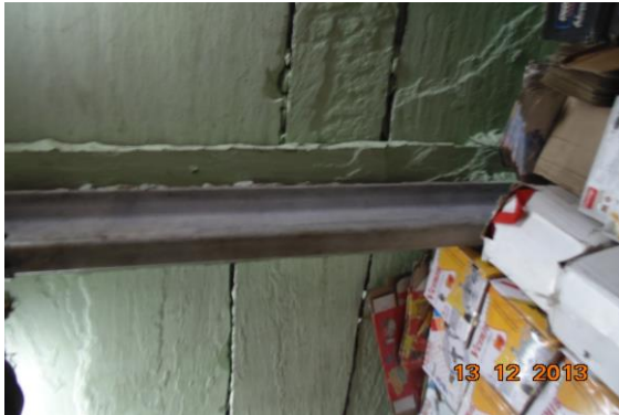
Photo 84 Peeling of Plaster on Roof of Shop No. 186 of Basement
