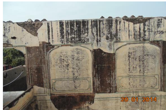
Photo 147 Peeling of Plaster on Wall No. 3 of Minarets of Tripoliya Gate, Terrace
