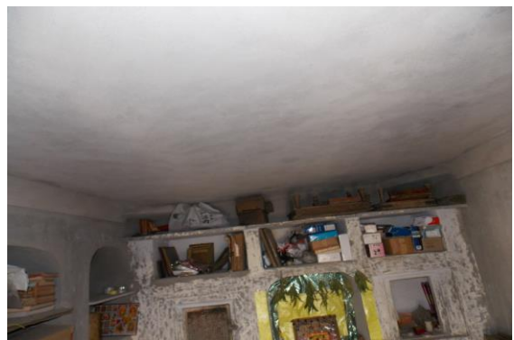
Photo 235 Dampness/Seepage of Room No. 5 of First Floor
