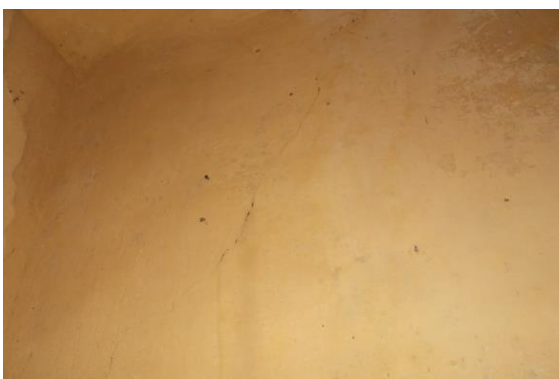
Photo 5 Inclined Crack on Wall No. 2 of Room No. 3, Hall No. 1, Ground Floor Approx. Width = 0.5mm, Approx. Length = 2m.
