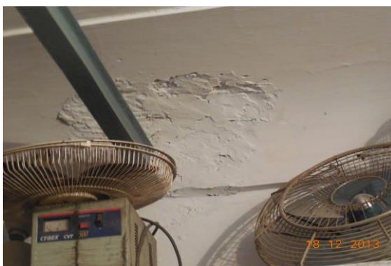
Photo 67 Peeling of Plaster on Roof of Room No. 2 of Ground Floor
