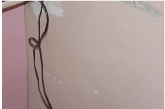
Photo 315 Plaster Crack on Wall No. 2 of Room No. 29 of First Floor
