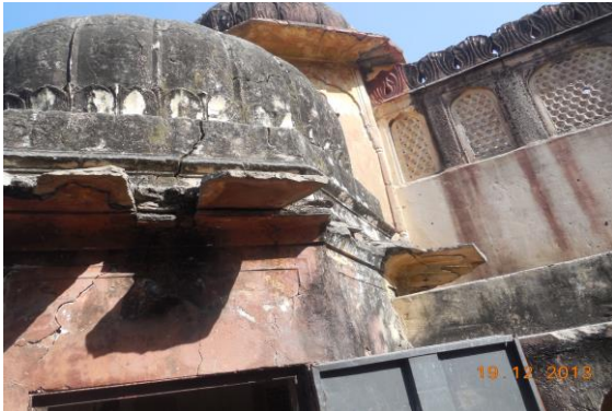
Photo 229 Damaged Portion on Sun Shade of Tomb No.1 of First Floor
