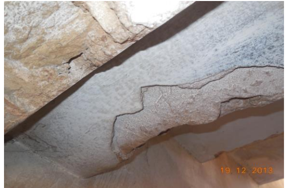
Photo 194 Damaged Portion on Roof of Staircase of First Floor
