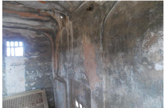
Photo 87 Peeling of Plaster on Wall No. 2 of Room No. 2 of Third Floor
