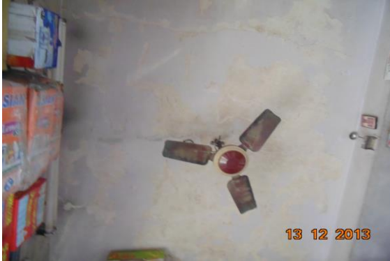
Photo 50 Dampness/Seepage on Roof of Shop No.174 of Ground Floor
