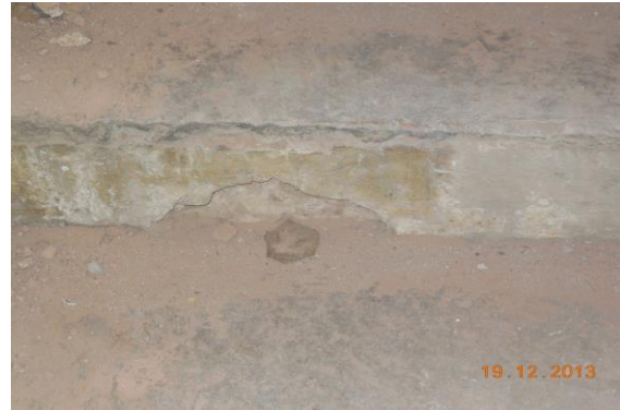
Photo 266 Peeling of Plaster on of staircase First Floor To Terrace of
