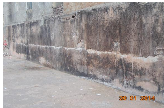
Photo 143 Peeling of Plaster on Wall No. 4 of Tripoliya Gate, Terrace
