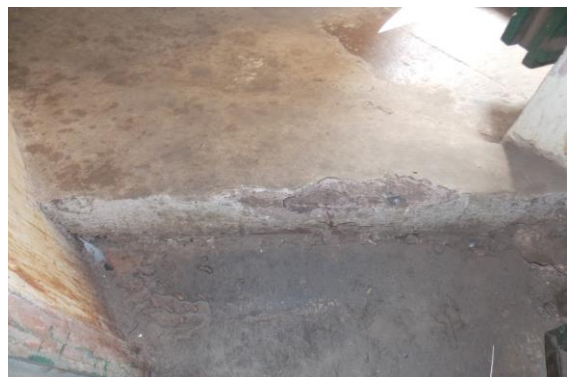
Photo 47 Peeling of Plaster on Stair FF to GF of Isarlat
