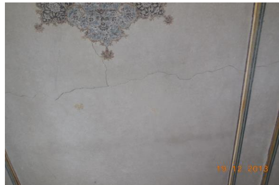
Photo 88 Plaster Crack on Roof of Varanda No.3 of Ground Floor
