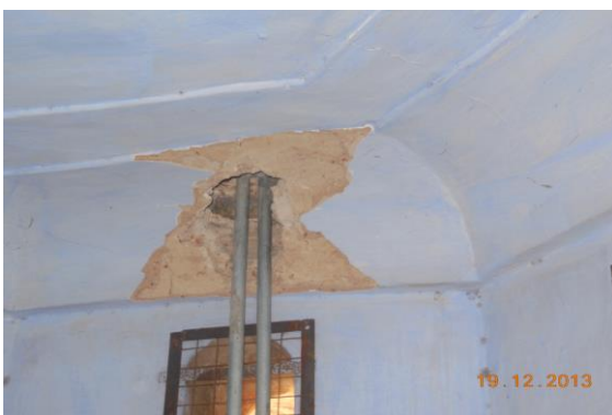
Photo 149 Exposed Reinforcement on Roof & 2 of Tomb No.2 of First Floor
