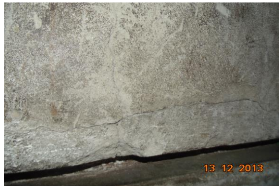
Photo 63 Plaster Crack on Stair Case GF to Basement of Shop No. 178, Basement
