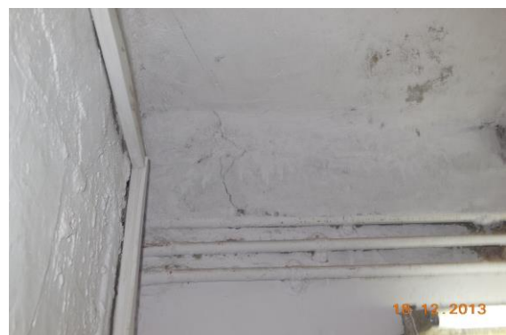
Photo 12 Inclined Crack on Wall No. 1 & Roof of Room No. Registry Room, First Floor Approx. Width = 1mm, Approx. Length = 0.3m. Distance from Wall No.3 = 0.15m, Height from Floor = 2.1m.
