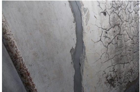
Photo 14 Inclined Crack on Wall No. 2 of Passage 1, Second Floor Approx. Width = 1.5mm, Approx. Length = 2.4m. Distance from W4 = 0m, Height from Floor = 0m.
