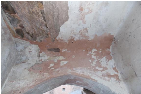
Photo 124 Peeling of Plaster on Wall No. 4 of Passage 1 of Ground Floor
