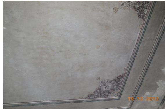
Photo 86 Plaster Crack on Roof of Varanda No.3 of Ground Floor
