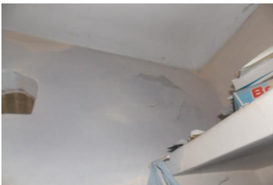
Photo 72 Peeling of Plaster on Wall No. 4 of Store 2 of Second Floor
