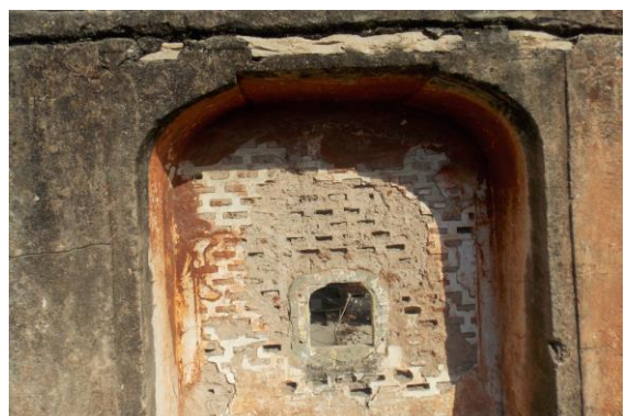
Photo 43 Peeling of Plaster on Wall No. 1 of Open Area 1 of Second Floor
