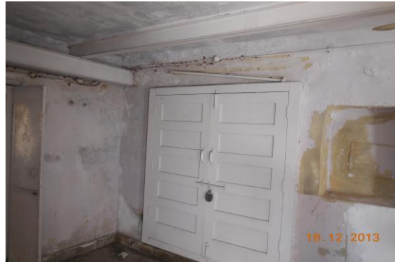
Photo 58 Dampness/Seepage on Wall No. 1 & 3 of Hall No. 2 of First Floor
