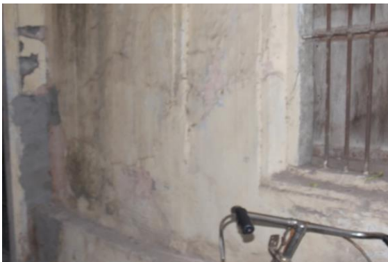
Photo 196 Peeling of Plaster on Wall No. 4 of Open Area of Ground Floor
