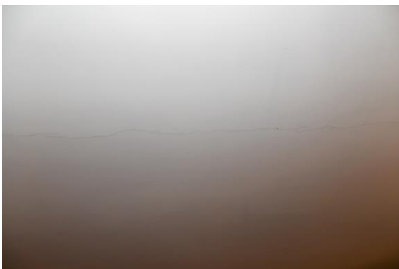
Photo 306 Plaster Crack on Roof of Room No. 25 of First Floor
