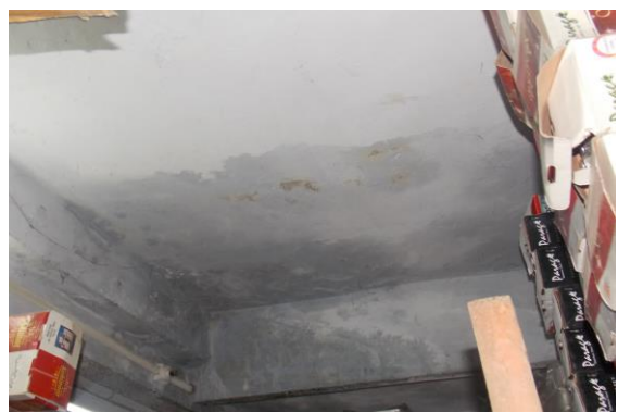
Photo 133 Dampness/Seepage on Roof of Room No. 9 of Ground Floor
