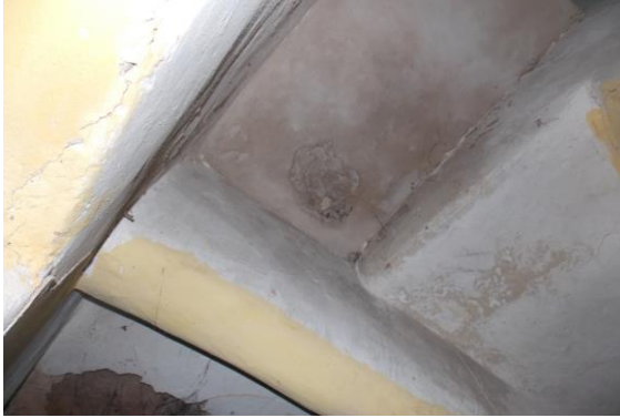
Photo 13 Dampness/Seepage on Roof of Store of Ground Floor
