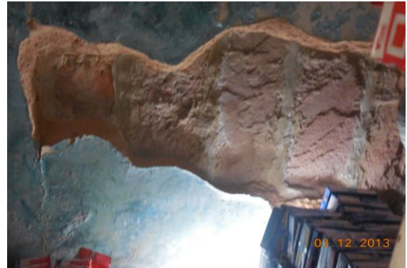
Photo 106 Peeling of Plaster on Roof of Shop No. E 60 of Ground Floor
