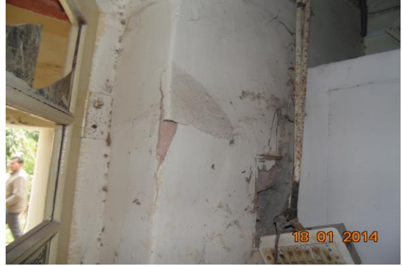
Photo 228 Peeling of Plaster on Wall No. 3 of . Room No. 116 of Police H.Q. Ground Floor, Part B
