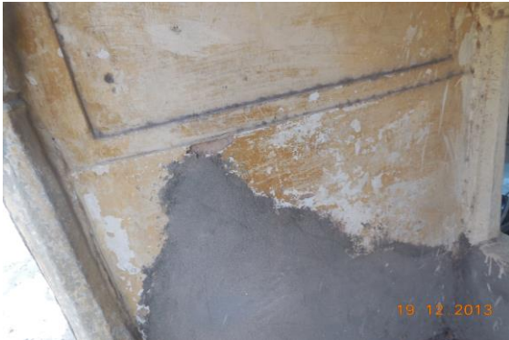
Photo 231 Peeling of Plaster on Wall No. 1 of Minarates No.3 of First Floor
