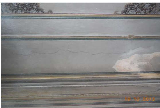
Photo 89 Plaster Crack on Roof of Varanda No.3 of Ground Floor
