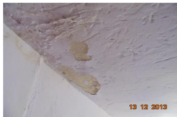
Photo 41 Peeling of Plaster on Roof of Shop No. 171 of Basement
