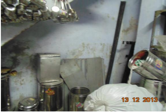
Photo 48 Dampness/Seepage on Floor of Shop No.173 of Basement
