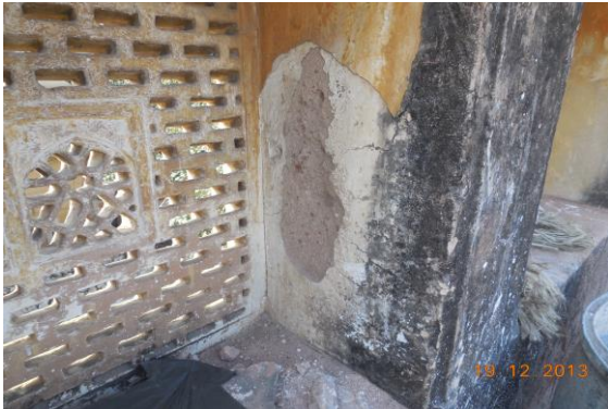
Photo 253 Peeling of Plaster on Wall No. 3 of School of Terrace
