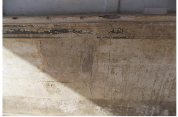
Photo 273 Peeling of Plaster on Wall No. 1 of Veranda of First Floor
