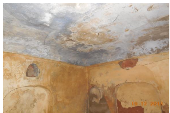
Photo 108 Dampness/Seepage on Wall No. 2, 4 & Roof of Room No. 1 of Lower Ground Floor
