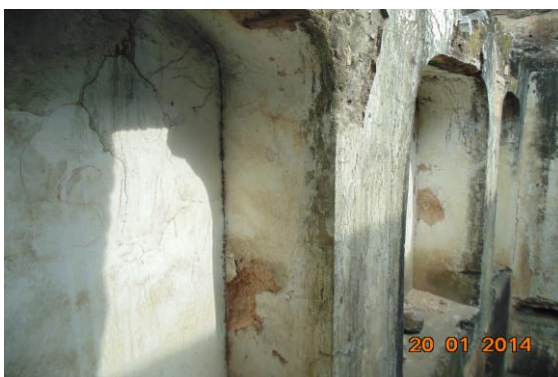
Photo 118 Peeling of Plaster on Wall No. 1 of Room No. 5 of First Floor, Tripoliya Gate
