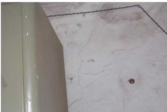
Photo 48 Peeling of Plaster on Wall No. 3 of Room No. 5 of Second Floor
