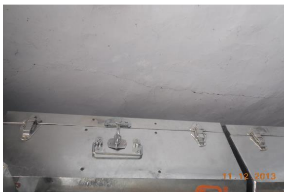
Photo 23 Horizontal Crack on Roof of Shop No.151, Ground Floor Approx. Width = 0.4mm, Approx. Length = 2.15m. Distance from Wall No.1 = 0.35m, Height from Floor = 2.5m.
