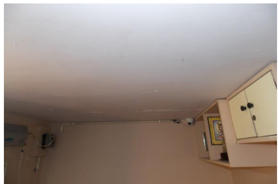
Photo 313 Peeling of Plaster on Roof of Room No. 29 of First Floor
