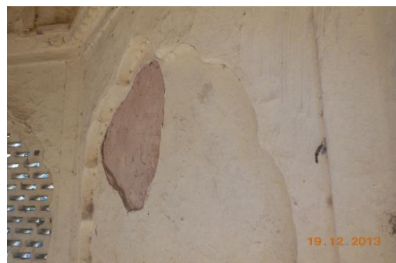
Photo 240 Peeling of Plaster on All walls & Roof of Tomb No.4 of Terrace
