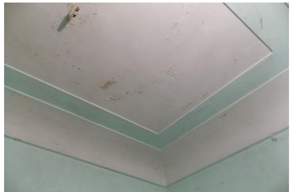
Photo 281 Peeling of Plaster on Roof of Room No. 14 of First Floor
