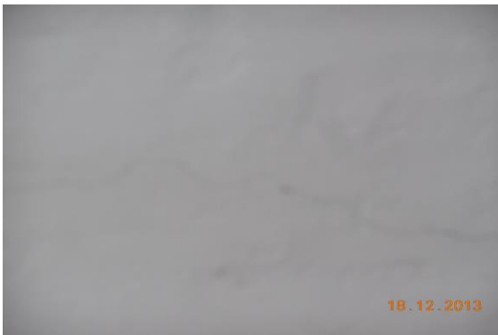
Photo 59 Plaster Crack on Roof of Hall No. 2 of First Floor
