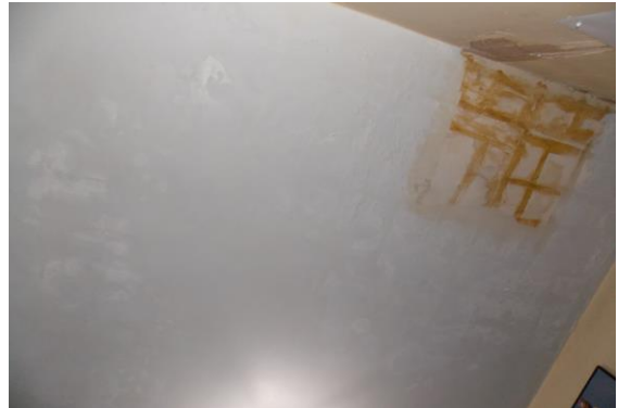
Photo 309 Dampness/Seepage on Roof of Room No. 27 of First Floor
