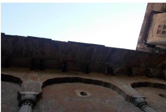
Photo 114 Damaged Portion on Sunshade of Open Area 1 of Second Floor
