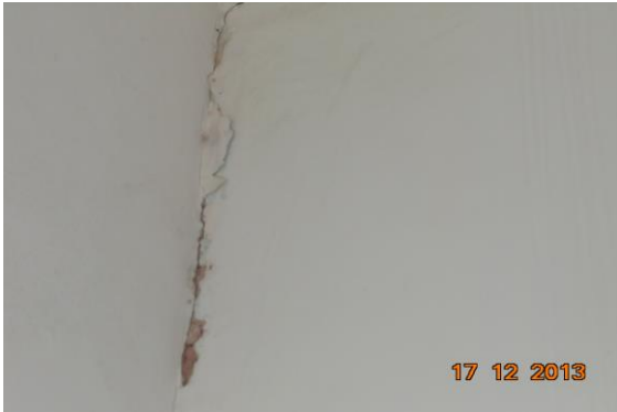
Photo 77 Peeling of Plaster on Wall No. 4 of Toilet No. 1 of Poornima Handicrafts, First Floor
