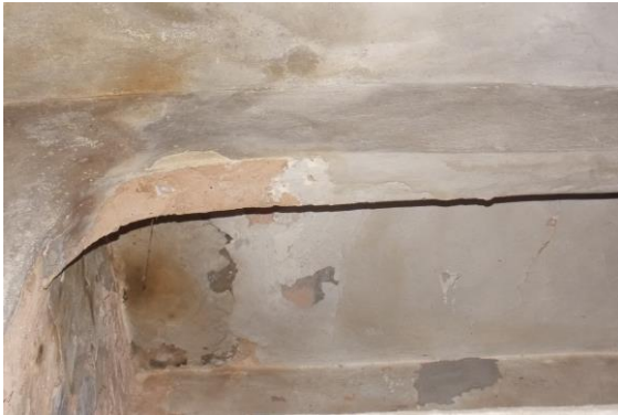
Photo 242 Dampness/Seepage on Roof of Room No. 6 of First Floor
