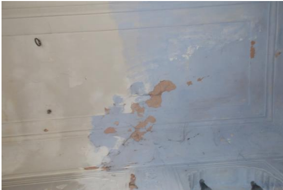
Photo 23 Peeling of Plaster on Roof of Varanda No.3 of Ground Floor
