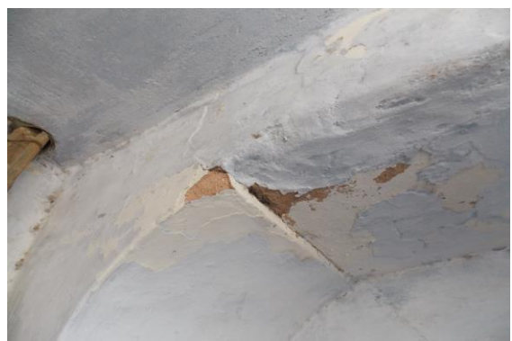
Photo 289 Peeling of Plaster on Roof of Gate of First Floor
