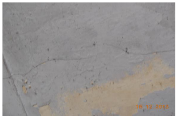
Photo 6 Inclined Crack on Roof of Main Gate, Neel mani Ji Ka Temple, Ground Floor, Approx. Width = 0.5mm, Approx. Length = 2m. Distance from Wall No.1 = 0m, Height from Floor = 3m.
