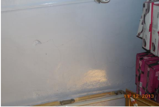
Photo 64 Plaster Crack on Roof of Shop No.157 of Ground Floor
