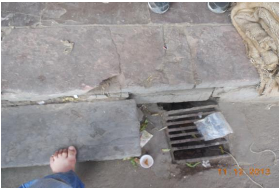
Photo 68 Damaged Portion on Floor of Varanda of Shop No.157 of Ground Floor
