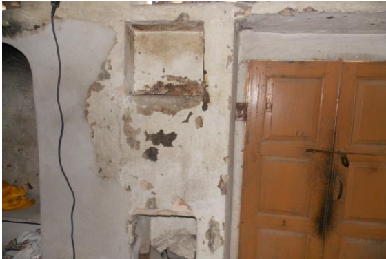
Photo 238 Dampness/Seepage on Wall No. 4 of Room No. 6 of First Floor
