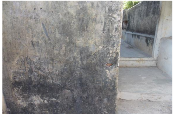
Photo 221 Peeling of Plaster on Wall No. 3 of Open Area 1 of First Floor
