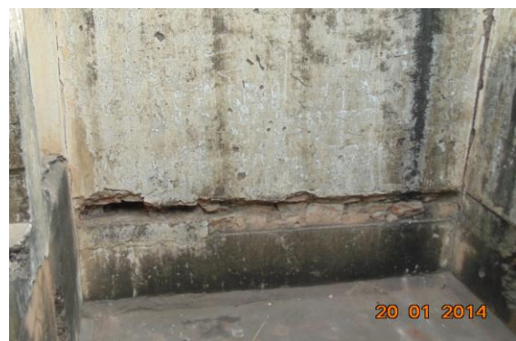
Photo 119 Peeling of Plaster on Wall No. 4 of Room No. 5 of First Floor, Tripoliya Gate
