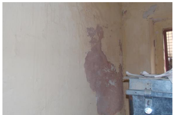
Photo 18 Dampness/Seepage on Wall No. 5 of Room No. 1 of Ground Floor
