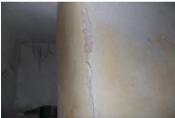
Photo 11 Dampness/Seepage on Wall No. 4 & Roof of Store of Ground Floor
