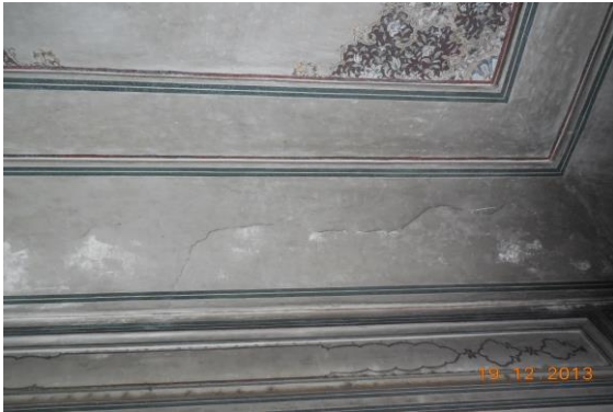
Photo 85 Plaster Crack on Roof of Varanda No.3 of Ground Floor
