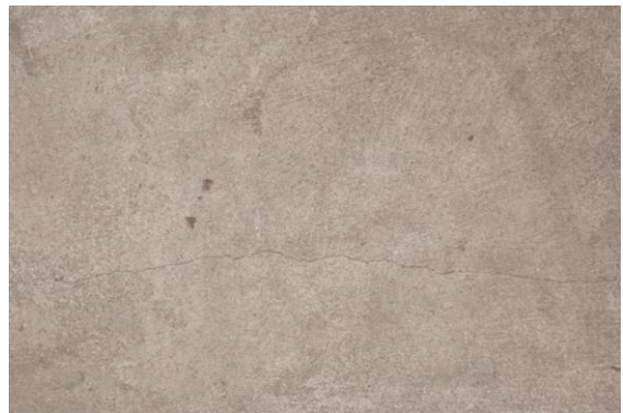
Photo 33 Plaster Crack on Stair Steps of Isarlat
