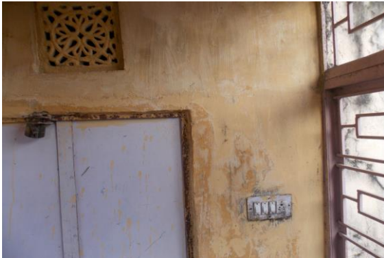
Photo 298 Dampness/Seepage on Room No. 20 of First Floor
