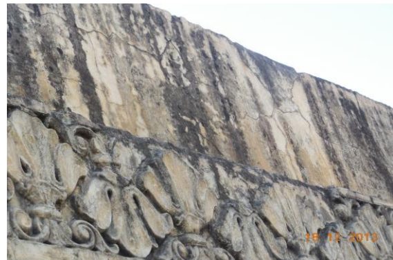
Photo 66 Plaster Crack on Parapet Wall of Post Office of Terrace
