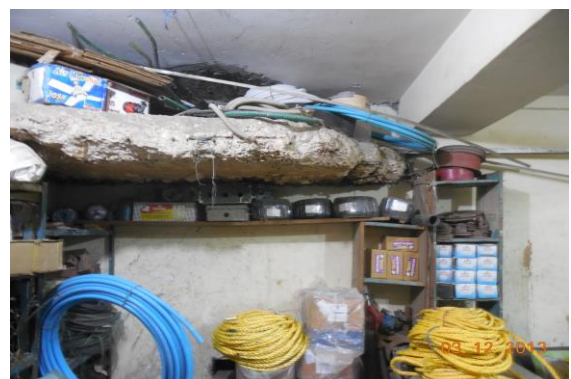
Photo 110 Peeling of Plaster on Wall No. 4 of Shop No. E 144, Basement
