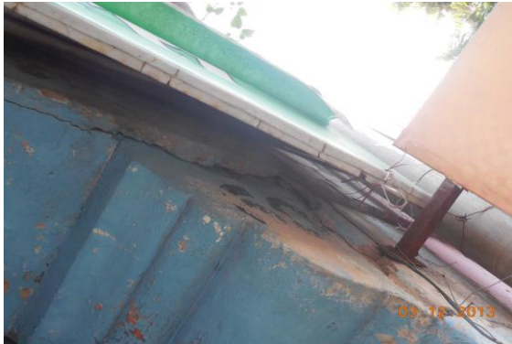
Photo 105 Peeling of Plaster on External Wall No. 3 of Shop No. E 60 of Ground Floor
