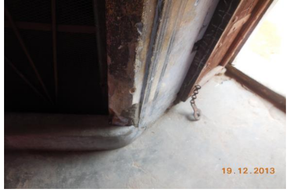
Photo 152 Peeling of Plaster on Outer Wall of Tomb No.2 of First Floor
