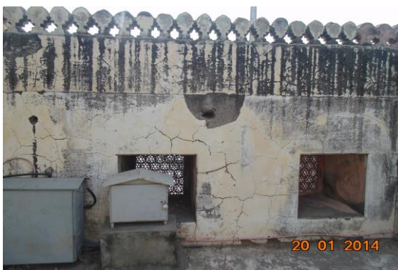
Photo 148 Peeling of Plaster on Wall No. 2 of Minarets of Tripoliya Gate, Terrace
