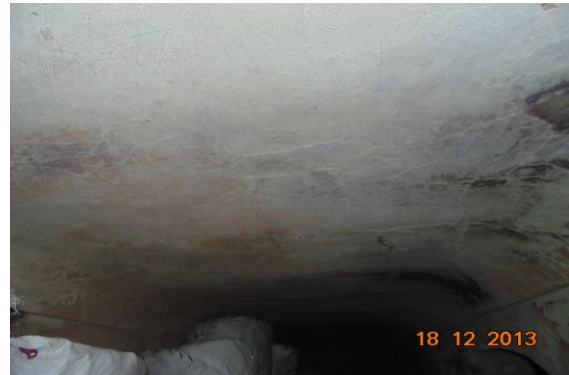
Photo 202 Peeling of Plaster on Roof of Part- N of Neel mani Ji Ka Temple, Basement
