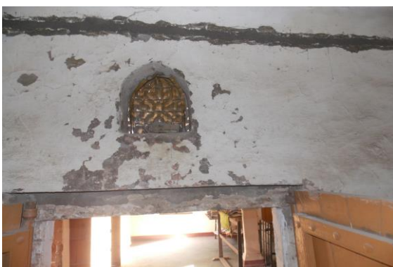
Photo 252 Peeling of Plaster on Wall No. 3 of Store 5 of First Floor
