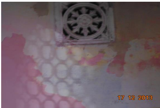
Photo 29 Peeling of Plaster on Wall No. 2 of Varanda No.2 of Ground Floor
