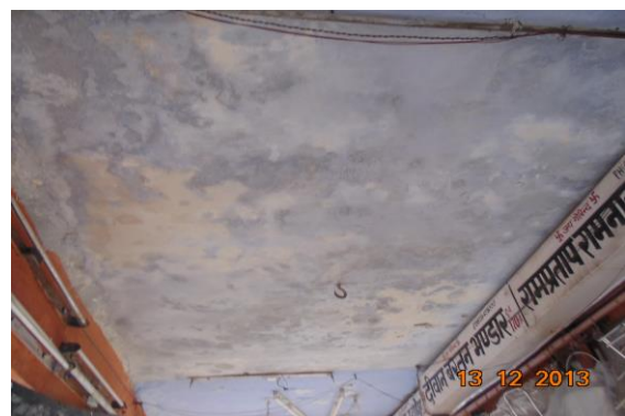
Photo 35 Dampness/Seepage on Roof of Varanda S.No.170B of Ground Floor
