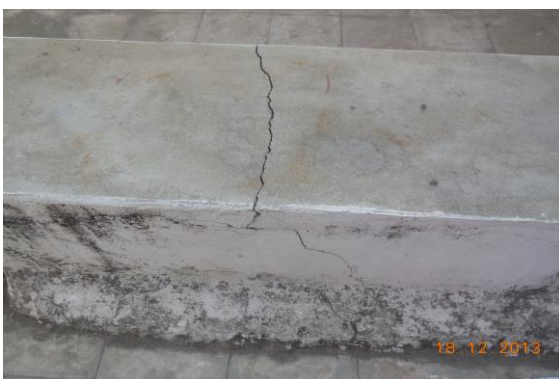
Photo 61 Damaged Portion on Parapet Wall of Post Office of First Floor
