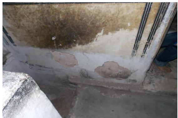
Photo 65 Plaster Crack on Wall No. 3 of Staircase Ground Floor to First Floor
