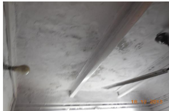
Photo 48 Dampness/Seepage on Roof of Registry Room of First Floor
