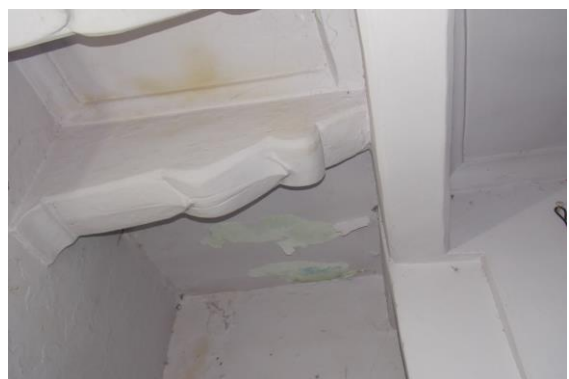
Photo 17 Plaster Crack on Roof of Room No. 3 of Navleshwar Temple, Ground Floor
