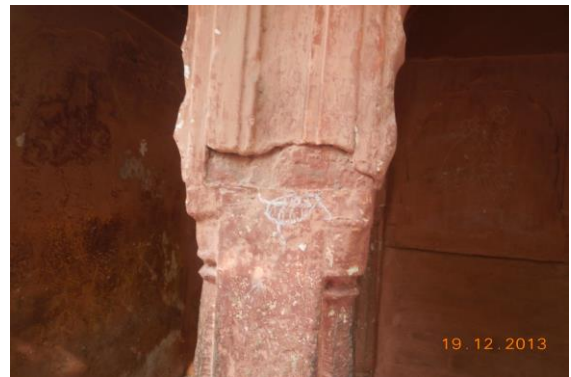
Photo 148 Peeling of Plaster on Outer Wall of Minarates No.2 of First Floor
