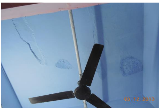
Photo 115 Peeling of Plaster on Roof of Part A of Shop No. D 53, Ground Floor
