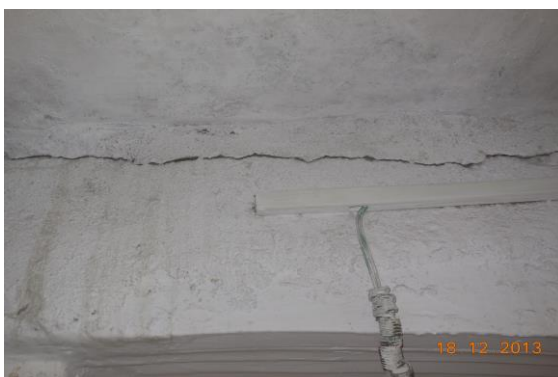
Photo 49 Peeling of Plaster on Wall No. 3 of Registry Room of First Floor
