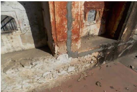
Photo 40 Peeling of Plaster on Wall No. 1 of Teenset 2 of Second Floor
