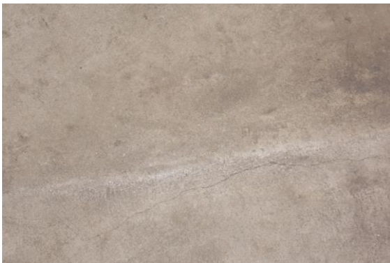
Photo 32 Plaster Crack on Stair Steps of Isarlat
