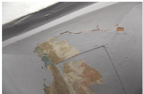
Photo 47 Peeling of Plaster on Roof of Passage of First floor
