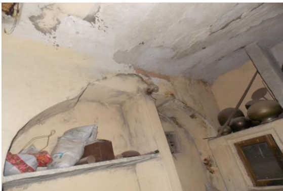
Photo 244 Peeling of Plaster on Wall No. 1 of Kitchen of First Floor
