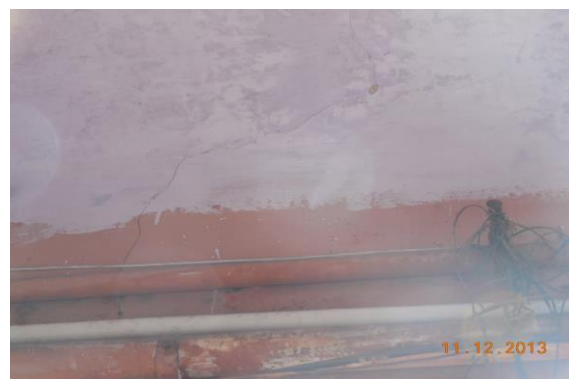
Photo 24 Inclined Crack on Varanda of Shop No.152 A, Ground Floor Approx. Width = 0.25mm, Approx. Length = 1.4m. Distance from Rightside External Column = Backside, Height from Floor = 2.5m.
