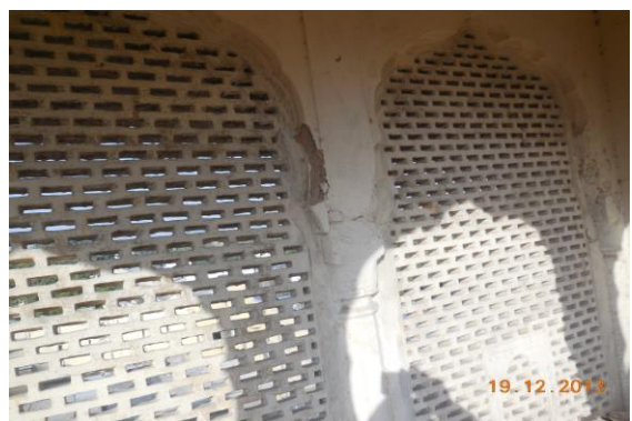
Photo 264 Peeling of Plaster on Wall No. 4 of Minarates No.8 of Terrace
