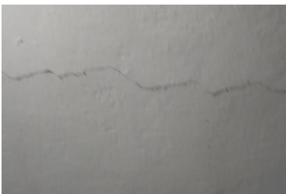
Photo 5 Inclined Crack on Roof of Kitchen, Ground Floor Approx. Width = 0.35mm, Approx. Length = 1.7m. Distance from Wall no.3 = 0m, Height from Floor = 3m.
