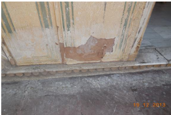
Photo 57 Peeling of Plaster on Wall No. 3 of Open Sky of Ground Floor
