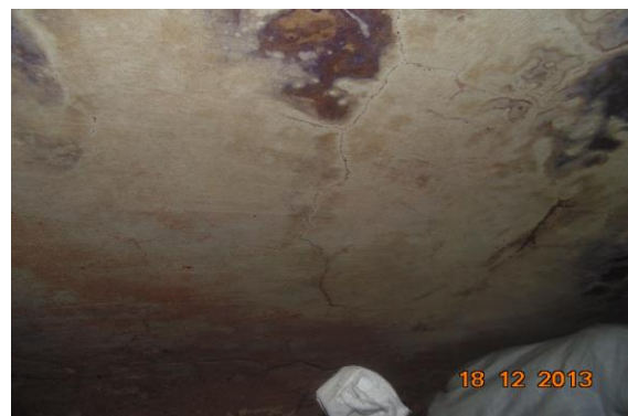
Photo 206 Plaster Crack on Roof of Part- N of Neel mani Ji Ka Temple, Basement
