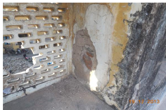
Photo 252 Peeling of Plaster on Wall No. 3 of School of Terrace
