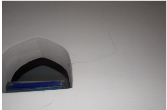
Photo 71 Plaster Crack on Wall No. 1 of Room No. 8 of Second Floor
