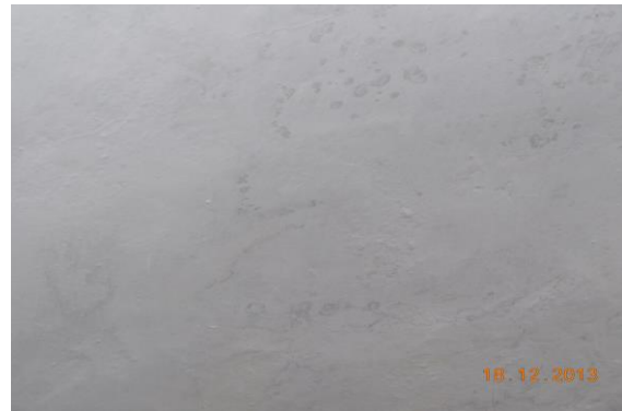
Photo 46 Dampness/Seepage on Roof of Room No. 3 of First Floor
