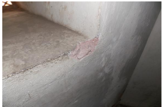
Photo 39 Peeling of Plaster on Wall No. 2 of Stair of Isarlat
