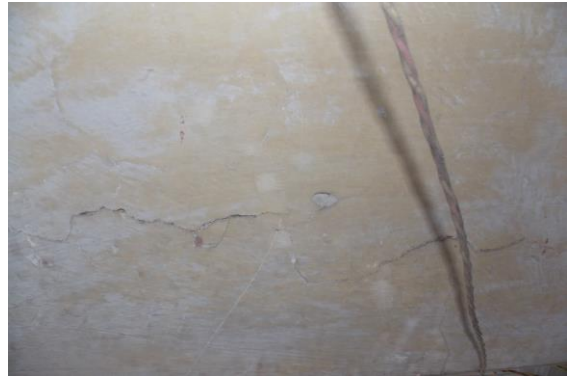
Photo 4 Horizontal Crack on Wall No. Roof & Gate of Temple Naval Bihari Ji, Ground Floor Approx. Width = 1mm, Approx. Length = 1.8m. Distance from Wall No.3 = 0.8m, Height from Floor = 2.2m.
