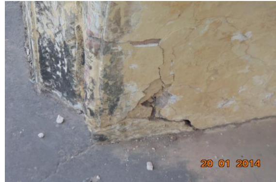
Photo 139 Peeling of Plaster on Wall No. 2 of Tripoliya Gate, Terrace
