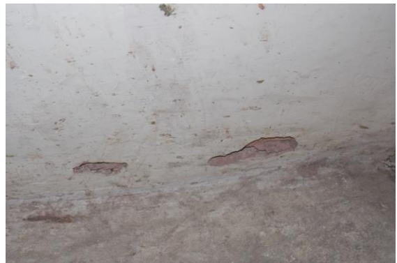
Photo 27 Peeling of Plaster on Wall No. 2 of Stair of Isarlat
