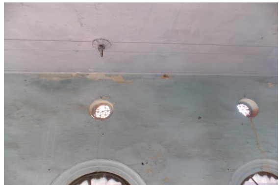
Photo 89 Peeling of Plaster on Wall No. 4 of Tomb of Third Floor
