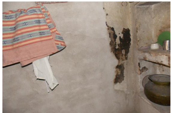
Photo 251 Dampness/Seepage on Wall No. 2 of Room No. 7 of First Floor
