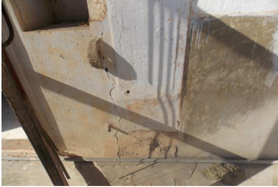
Photo 236 Peeling of Plaster on Wall No. 3 of Open Area 3 of First Floor
