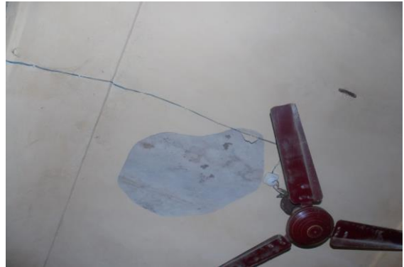
Photo 16 Dampness/Seepage on Roof of Room No. 1 of Ground Floor
