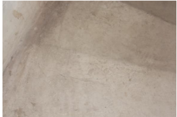
Photo 43 Plaster Crack on Stair Steps of Isarlat
