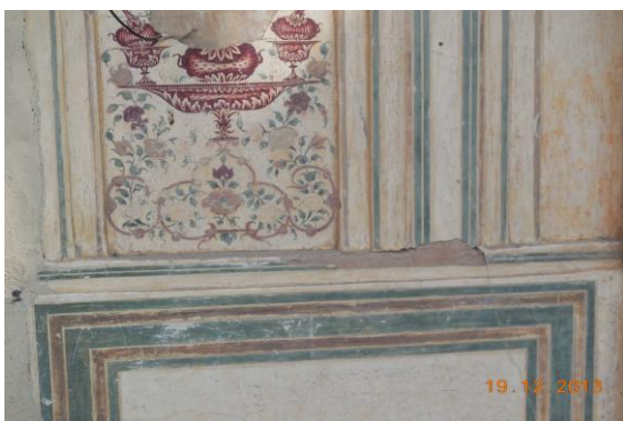
Photo 59 Peeling of Plaster on Wall No. 2 of Open Sky of Ground Floor
