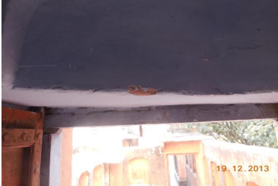
Photo 153 Peeling of Plaster on Wall No. 3 of Room No. 1 of School, First Floor
