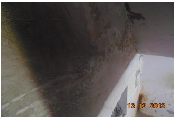
Photo 38 Peeling of Plaster on Stair case of Shop No. 171, Basement
