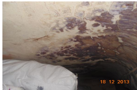
Photo 204 Peeling of Plaster on Wall No. 2 of Part- N of Neel mani Ji Ka Temple, Basement
