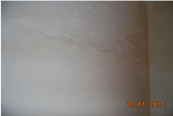
Photo 229 Plaster Crack on Wall No. 3 of Hall No. 4 of Police H.Q. Ground Floor, Part B
