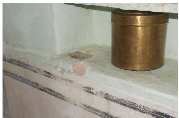
Photo 283 Peeling of Plaster on Wall No. 2 of Store 9 of First Floor
