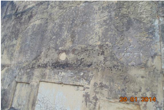
Photo 140 Peeling of Plaster on Wall No. 2 of Tripoliya Gate, Terrace
