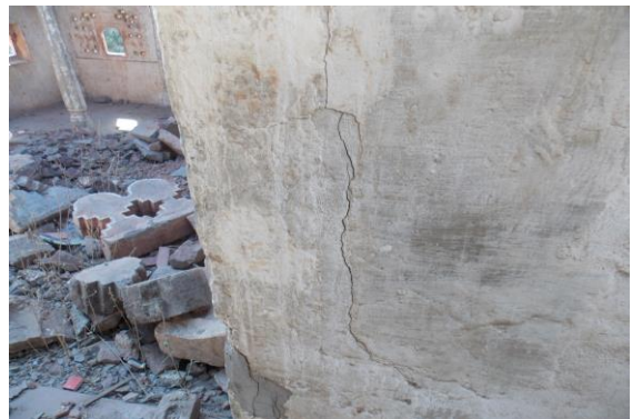
Photo 15 Inclined Crack on Wall No. 2 of Teenset 2, Second Floor Approx. Width = 2.5mm, Approx. Length = 1.5m. Distance from W1 = 4m, Height from Floor = 0.3m.
