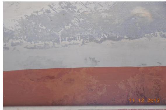
Photo 22 Horizontal Crack on Roof of Varanda of Shop No.151, Approx. Width = 0.15mm, Approx. Length = 2m. Distance from Left External Column = 1.5m, Height from Floor = 3m.
