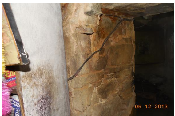
Photo 61 Peeling of Plaster on Entry Gate Left Side of Part C of Shop of Ground Floor
