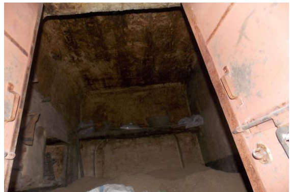
Photo 113 Dampness/Seepage of Room No. 4 of Ground Floor
