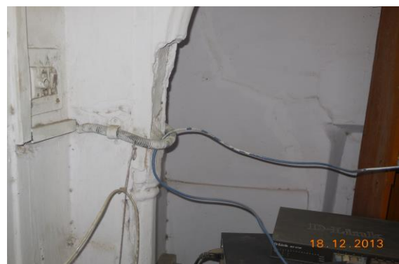
Photo 50 Peeling of Plaster on Wall No. 1 of Registry Room of First Floor
