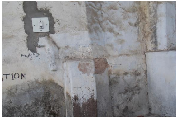
Photo 297 Peeling of Plaster on of Entry Door of R 17 & 18 of First Floor
