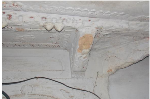
Photo 43 Peeling of Plaster on Roof of Bathroom of Navleshwar Temple, First floor
