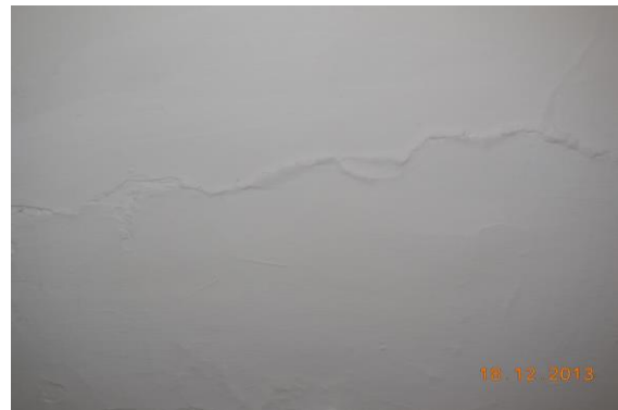
Photo 42 Plaster Crack on Roof of Passage of First Floor
