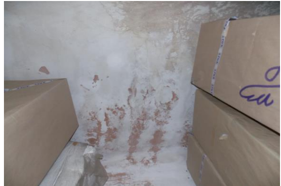
Photo 201 Dampness/Seepage on Roof of Room No. 47 of Ground Floor
