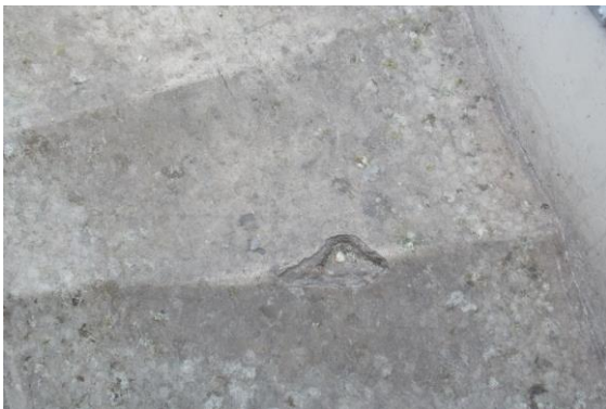
Photo 26 Peeling of Plaster on Stair Steps of Isarlat
