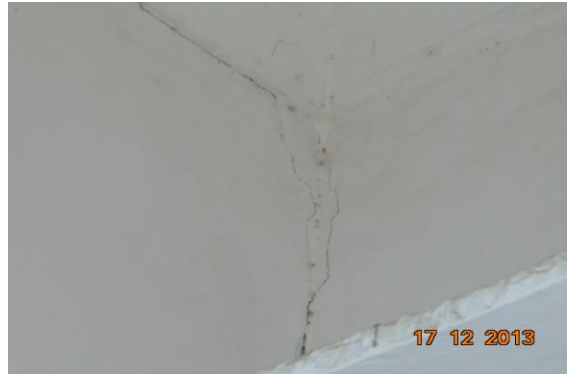
Photo 77 Peeling of Plaster on Wall No. 4 of Toilet No. 1 of Poornima Handicrafts, First Floor
