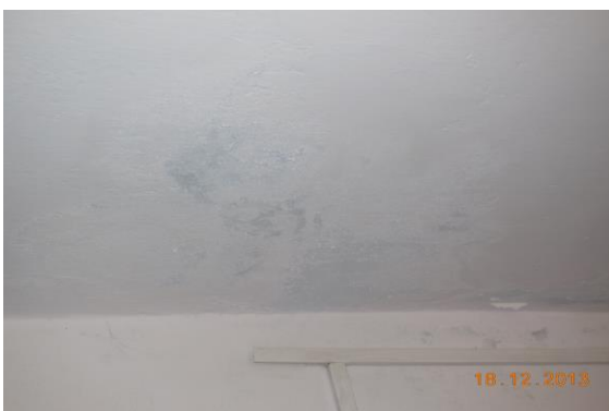
Photo 43 Dampness/Seepage on Roof of Room No. 1 of First Floor
