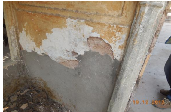
Photo 232 Peeling of Plaster on Wall No. 1 of Minarates No.3 of First Floor
