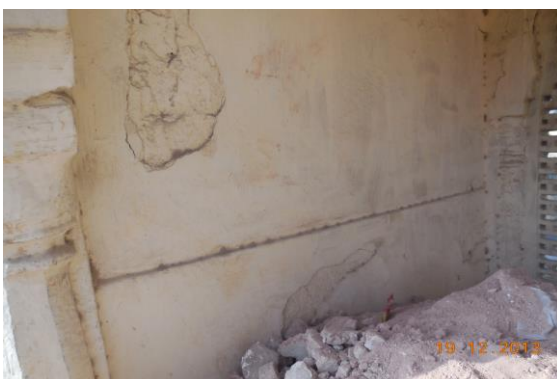
Photo 263 Peeling of Plaster on Wall No. 1 of Minarates No.8 of Terrace
