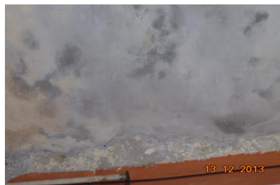
Photo 18 Inclined Crack on Roof of Varanda S.No.170A, Ground Floor Approx. Width = 0.5mm, Approx. Length = 3m. Height from Floor = 3m.
