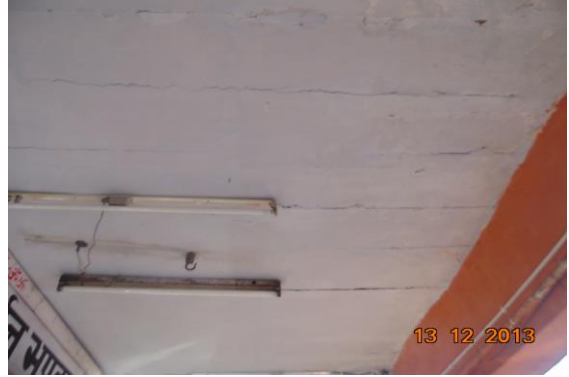
Photo 49 Peeling of Plaster on Roof of Varanda of Shop No.174, Ground Floor
