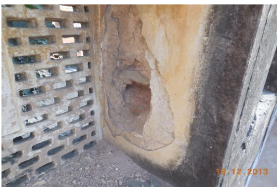
Photo 245 Peeling of Plaster on Wall No. 4 of School of Terrace
