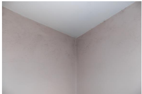
Photo 311 Dampness/Seepage on Wall No. 1 & 4 of Room No. 28 of First Floor
