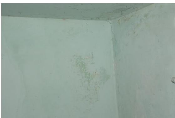
Photo 282 Peeling of Plaster on Wall No. 4 of Store 9 of First Floor
