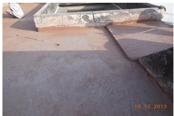
Photo 258 Peeling of Plaster on Floor of School of Terrace
