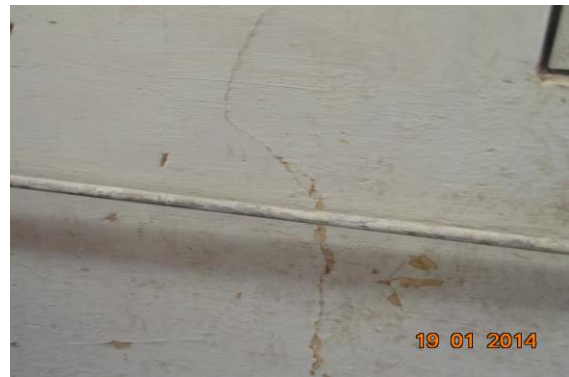
Photo 15 Inclined Crack on Wall No. 1 of , Police H.Q. First Floor, Part B, Approx. Width = 0.35mm, Approx. Length = 1m. Distance from Wall 4 = 3.2m, Height from Floor = 0.12m.
