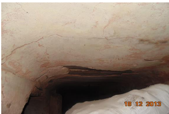
Photo 205 Dampness/Seepage on Roof of Part- N of Neel mani Ji Ka Temple, Basement
