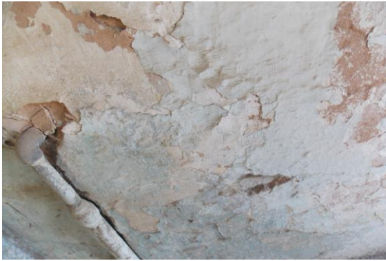
Photo 68 Peeling of Plaster on Wall No. 2 of Gallery 1 of Second Floor
