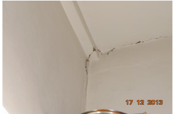
Photo 76 Peeling of Plaster on Wall No. 1 & 3 of Kitchen of First Floor
