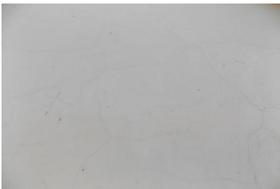
Photo 70 Plaster Crack on Wall No. 4, 5 & 6 of First Floor, Isarlat
