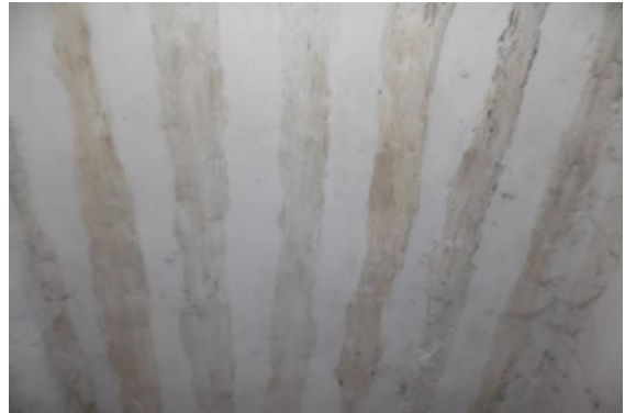
Photo 149 Dampness/Seepage on Roof of Room No. 21 of Ground Floor
