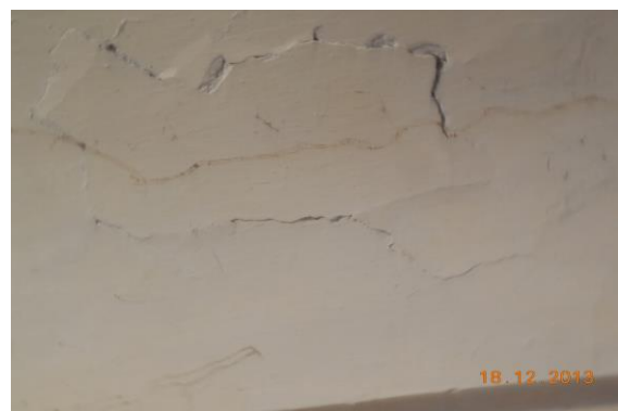
Photo 68 Peeling of Plaster on Roof of Room No. 2 of Ground Floor
