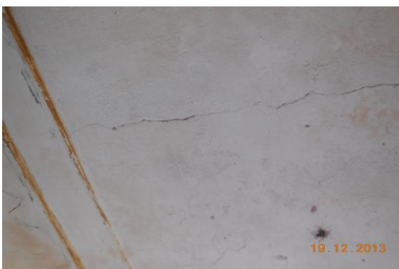
Photo 191 Plaster Crack on Roof of Gallery No.3 of First Floor
