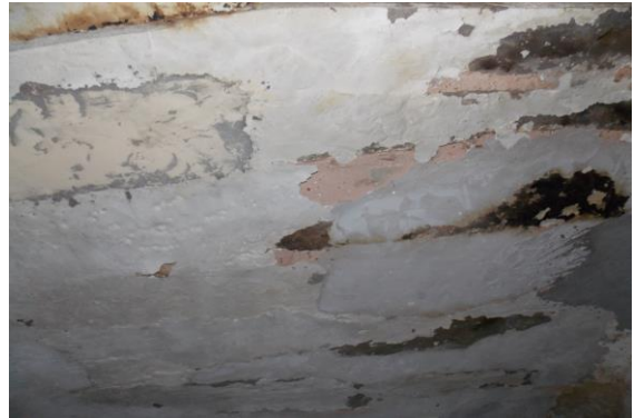
Photo 243 Peeling of Plaster on Roof of Kitchen of First Floor
