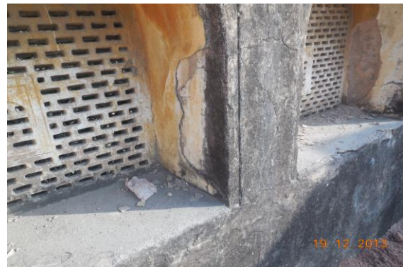
Photo 244 Peeling of Plaster on Wall No. 4 of School of Terrace
