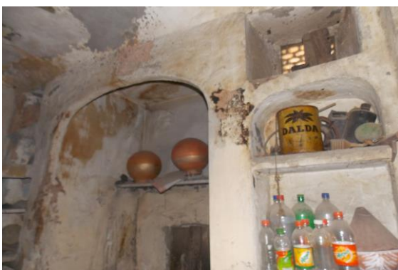
Photo 246 Dampness/Seepage on Wall No. 2 of Kitchen of First Floor
