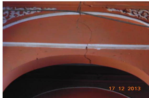
Photo 4 Inclined Crack on Wall No. 1 of Passage, Historical Gate No.2, Ground Floor Approx. Width = 1.5mm, Approx. Length = 0.8m. Distance from Wall No.3 = 5m, Height from Floor = 3.5m.
