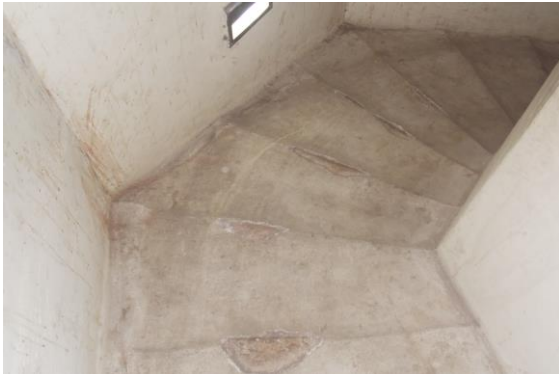
Photo 44 Plaster Crack on Stair Steps of Isarlat
