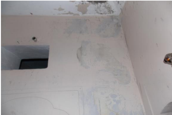
Photo 70 Dampness/Seepage on Wall No. 2 of Room No. 8 of Second Floor
