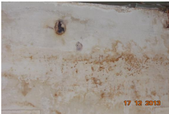
Photo 59 Dampness/Seepage on Wall No. 4 of Hall No. 4 of Poornima Handicrafts, First Floor
