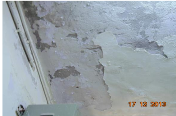
Photo 58 Dampness/Seepage on Roof of Lobby of First Floor
