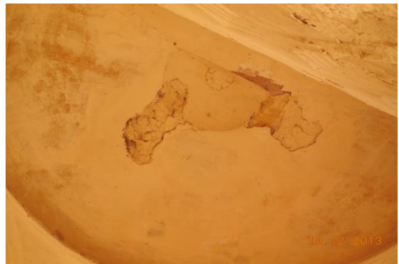
Photo 262 Peeling of Plaster on All walls & Roof of Tomb No.5 of Terrace
