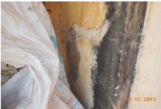
Photo 255 Peeling of Plaster on Wall No. 3 of School of Terrace
