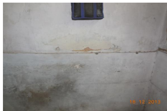
Photo 74 Peeling of Plaster on Wall No. 4 of Room No. 1 of Ground Floor
