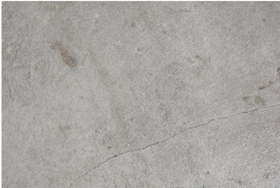
Photo 36 Plaster Crack on Stair Steps of Isarlat
