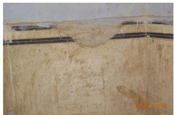
Photo 150 Peeling of Plaster on Wall No. 4 of Tomb No.2 of First Floor
