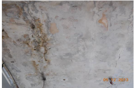
Photo 57 Dampness/Seepage on Roof of Varanda of Shop of Ground Floor
