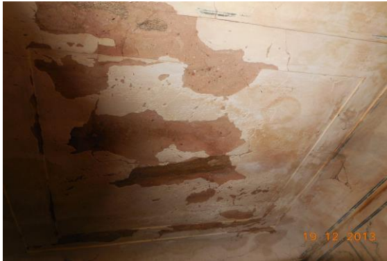
Photo 199 Damaged Portion on Roof of Gallery No.2 of First Floor
