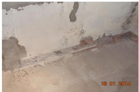
Photo 232 Peeling of Plaster on Wall No. 3 of Hall No. 4 of Police H.Q. Ground Floor, Part B
