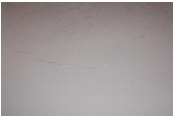
Photo 312 Plaster Crack on Wall No. 1 of Room No. 28 of First Floor
