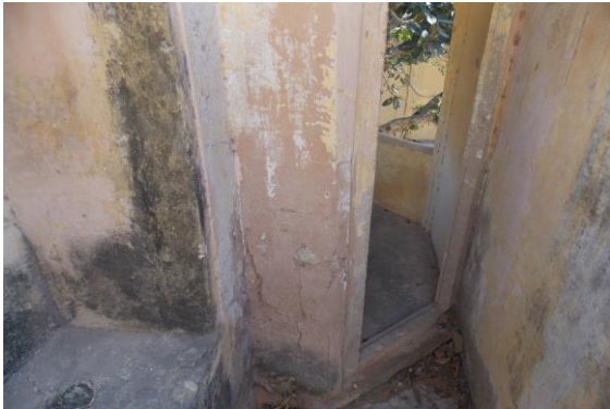
Photo 220 Peeling of Plaster on Wall No. 4 of Open Area 1 of First Floor
