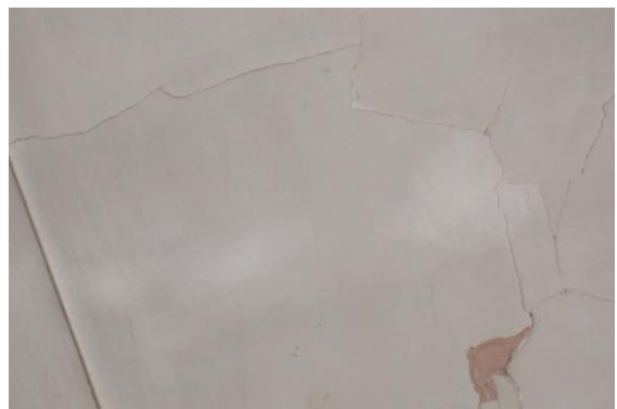
Photo 5A Inclined Crack on Wall No. 4 & Roof of Varanda No.1, Ground Floor Approx. Width = 3.5mm, Approx. Length = 6m. Distance from Wall No.1 = 1m, Height from Floor = 3.2m.
