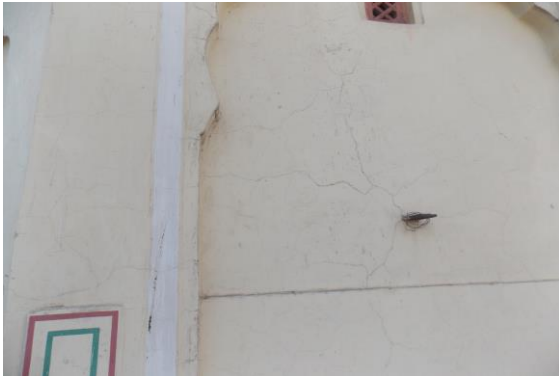
Photo 68 Plaster Crack on Wall No. 4, 5 & 6 of First Floor, Isarlat
