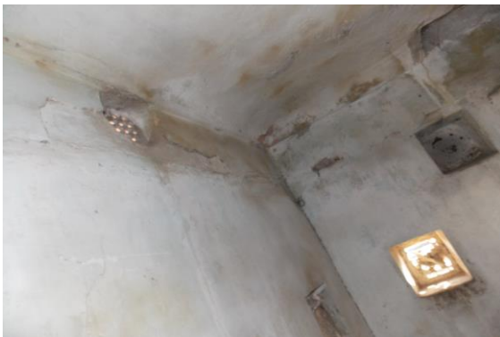
Photo 88 Dampness/Seepage on Wall No. 1, 4 & Roof of Room No. 3 of Third Floor
