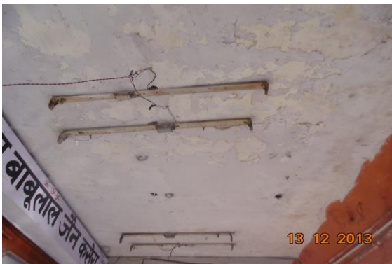
Photo 52 Dampness/Seepage on Roof of Varanda of Shop No.175, Ground Floor
