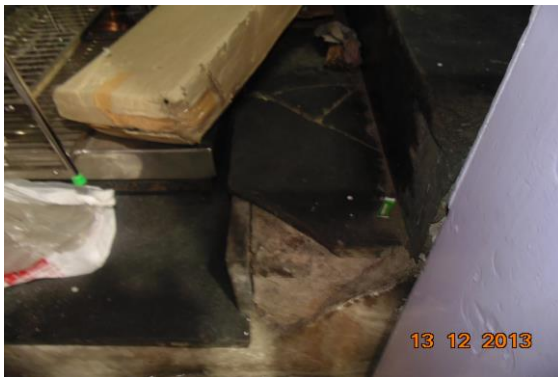
Photo 32 Dampness/Seepage on Stair Step GF to U/GF of Upper Ground Floor
