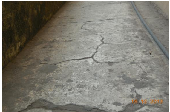
Photo 52 Plaster Crack on Floor of Passage of First Floor
