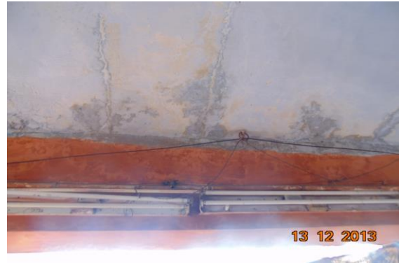
Photo 37 Plaster Crack on Roof & Beam of Varanda of Shop No. 171, Ground Floor
