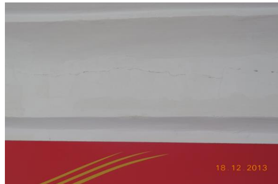
Photo 10 Horizontal Crack on Roof of Lobby of Post Office, Ground Floor Approx. Width = 0.5mm, Approx. Length = 2m.
