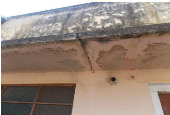
Photo 222 Dampness/Seepage on Sunshade & 2 of Open Area 1 of First Floor
