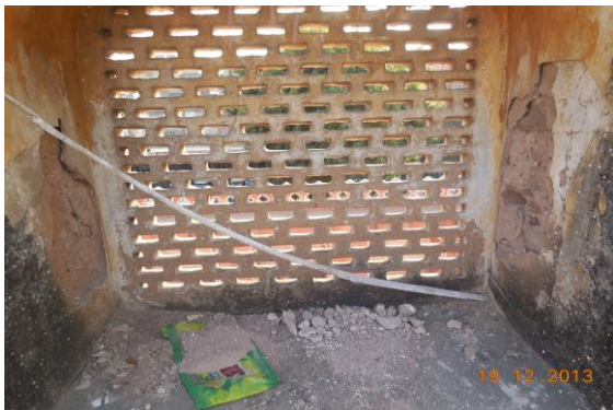
Photo 249 Peeling of Plaster on Wall No. 1 of School of Terrace
