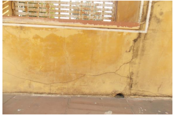
Photo 67 Peeling of Plaster on Wall No. 4 of First Floor, Isarlat
