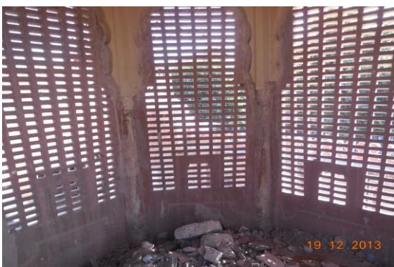
Photo 239 Peeling of Plaster on All walls of Tomb No.3 of Terrace
