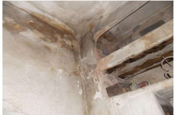
Photo 239 Dampness/Seepage on Wall No. 3 of Room No. 6 of First Floor
