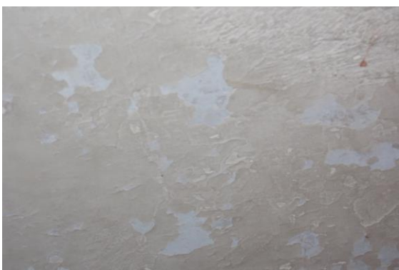
Photo 34 Peeling of Plaster on Wall No. 2 of Stair of Isarlat
