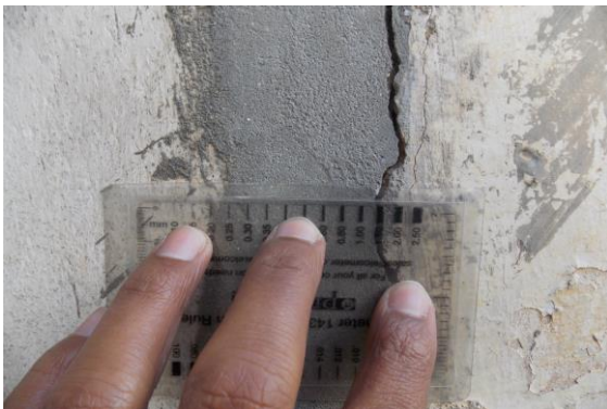
Photo 14A Inclined Crack on Wall No. 2 of Passage 1, Second Floor Approx. Width = 1.5mm, Approx. Length = 2.4m. Distance from W4 = 0m, Height from Floor = 0m.
