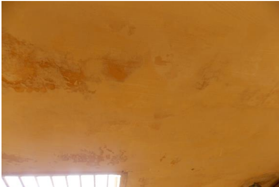
Photo 304 Dampness/Seepage on Roof of Passage 2 of First Floor
