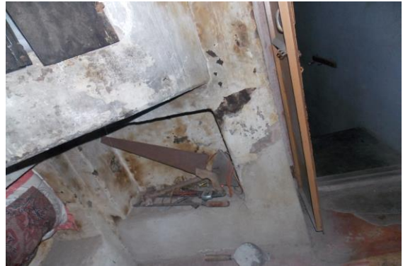
Photo 249 Dampness/Seepage on Wall No. 1 of Room No. 7 of First Floor
