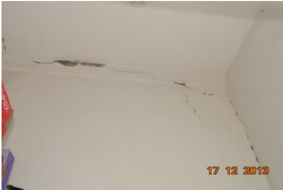
Photo 75 Peeling of Plaster on Wall No. 4 of Kitchen of First Floor
