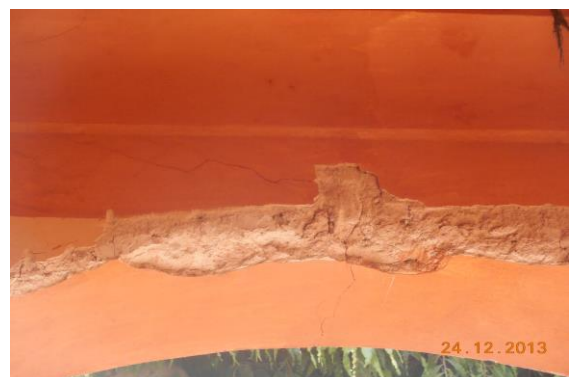
Photo 4 Inclined Crack on Wall No. 1 of Passage, Historical Gate No.2, Ground Floor Approx. Width = 1.5mm, Approx. Length = 0.8m. Distance from Wall No.3 = 5m, Height from Floor = 3.5m.
