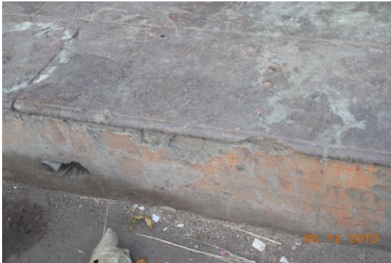
Photo 56 Peeling of Plaster on Floor of Varanda of Shop of Ground Floor
