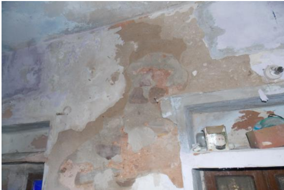
Photo 178 Peeling of Plaster on Wall No. 4 of Room No. 41 of Ground Floor
