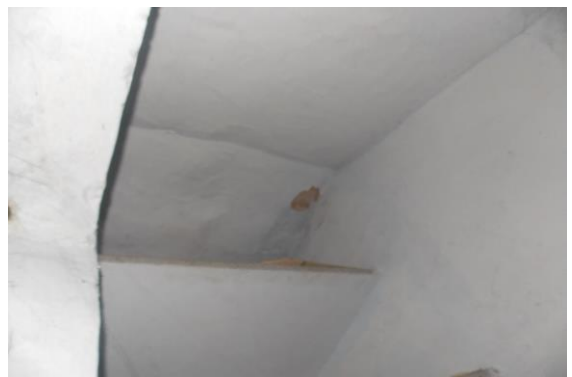
Photo 181 Peeling of Plaster on Roof of Store 3 of Ground Floor
