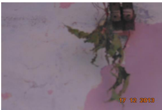
Photo 31 Peeling of Plaster on Wall No. 3 of Varanda No.2 of Ground Floor
