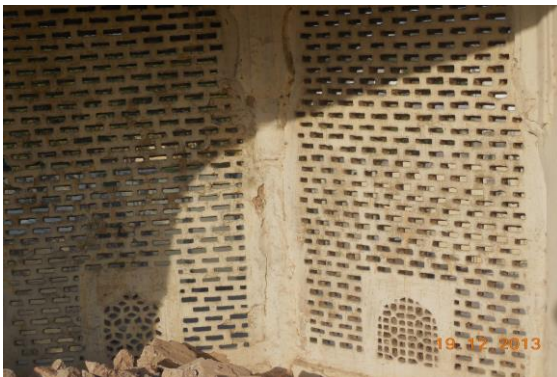
Photo 261 Peeling of Plaster on All walls & Roof of Tomb No.5 of Terrace
