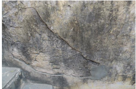
Photo 233 Peeling of Plaster on Wall No. 1 of Open Area 2 of First Floor
