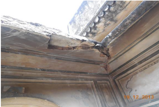
Photo 193 Damaged Portion on Sun Shade of Open Sky of First Floor
