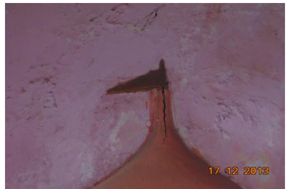
Photo 30 Dampness/Seepage on Wall No. 1 of Varanda No.2 of Ground Floor
