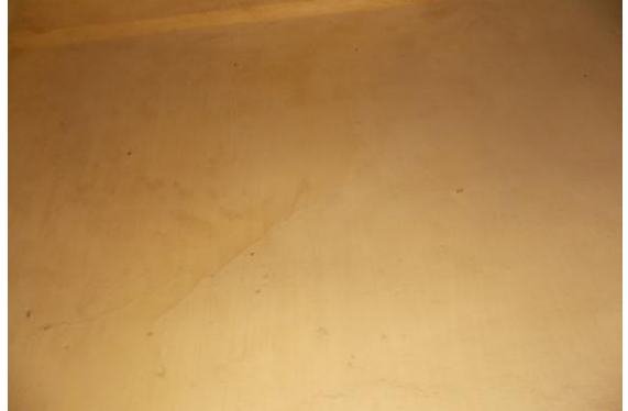
Photo 10 Dampness/Seepage on Wall No. 2 of Room No. 2 of Ground Floor
