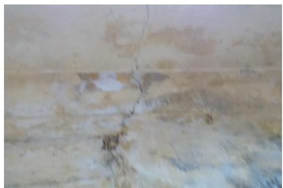
Photo 6 Inclined Crack on Wall No. 2 of Open Area, Ground Floor Approx. Width = 1mm, Approx. Length = 1m. Distance from Wall no.3 = 5m, Height from Floor = 2.5m.
