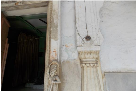
Photo 278 Peeling of Plaster on Wall No. 5 of Veranda of First Floor
