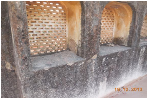
Photo 247 Peeling of Plaster on Wall No. 1 of School of Terrace
