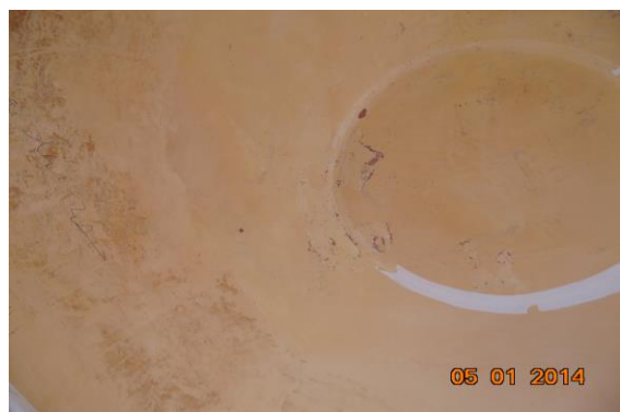
Photo 415 Peeling of Plaster on Roof of Tome 2 of Part B1 Third Floor
