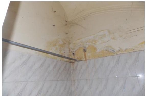
Photo 134 Dampness/Seepage on Wall No. 2, 4 & Roof of Bathroom of Second Floor
