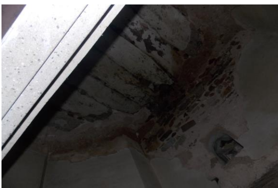
Photo 271 Damaged Portion on Roof of Store of Ground Floor
