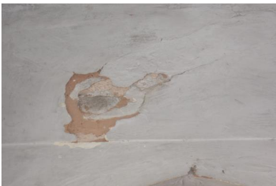
Photo 277 Peeling of Plaster on Wall No. 1 of Varanda No.2 of Ground Floor
