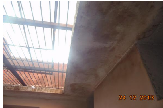
Photo 46 Dampness/Seepage on Wall No. 3 of Open Sky of First Floor
