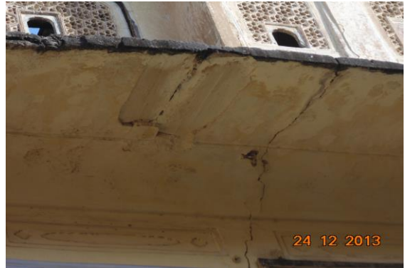
Photo 235 Damaged Portion on Wall No. 4 & Shade of Balcony of First Floor
