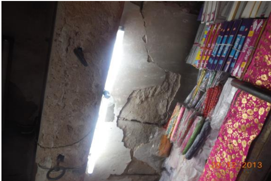
Photo 39 Inclined Crack on Roof of Shop No.2, Ground Floor Approx. Width = 4mm, Approx. Length = 0.5m.
