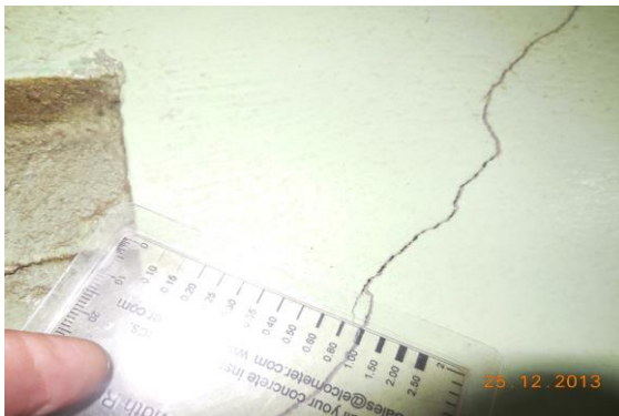
Photo 21 Inclined Crack on Wall No. 3 of Room No. 4, Part 3 Gyarah Rudra Mandir, Second Floor, Approx. Width = 1mm, Approx. Length = 0.6m. Distance from Wall No. 2 = 2m, Height from Floor = 1.7m.
