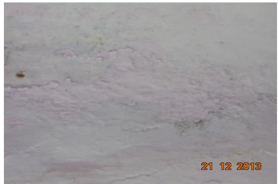
Photo 42 Dampness/Seepage on Roof of Part A of shop no.13 of Ground Floor
