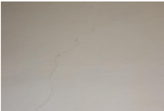
Photo 250 Plaster Crack on Wall No. 1 of Gallery 8 of Part B2 Upper Ground Floor
