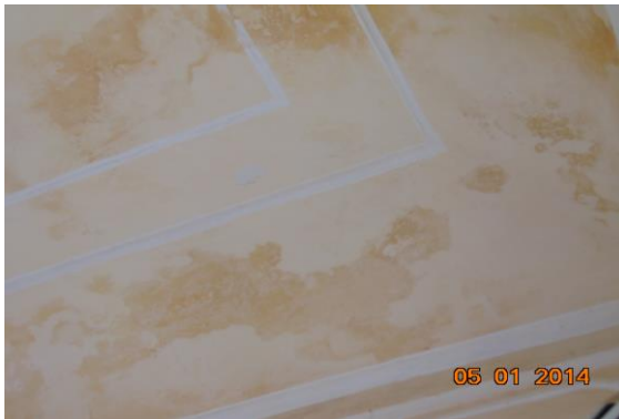
Photo 392 Dampness/Seepage on Roof of Room No. 2 of Part B1 First Floor
