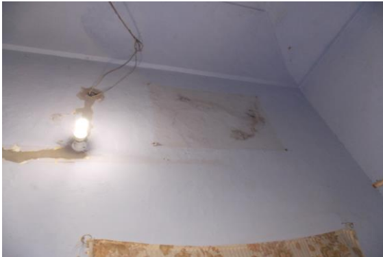
Photo 153 Peeling of Plaster on Wall No. 3 of Room No. 6 of Second Floor
