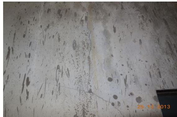
Photo 4 Inclined Crack on Wall No. 2 of Room No. 1, Second Floor, Approx. Width = 0.6mm, Approx. Length = 0.6m. Distance from Wall no.4 = 2.8m, Height from Floor = 1.8m.
