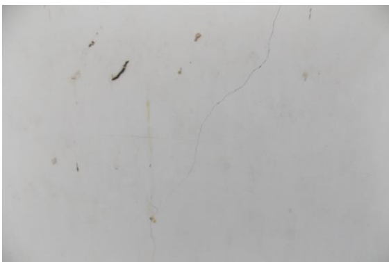
Photo 168 Plaster Crack on Wall No. 4 of Open Area of Part A2 Upper Ground Floor
