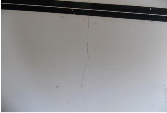
Photo 158 Plaster Crack on Wall No. 4 of Vrandha 3 of Part A2 Upper Ground Floor
