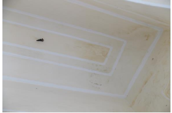
Photo 165 Dampness/Seepage on Roof of Vrandha 4 of Part A2 Upper Ground Floor
