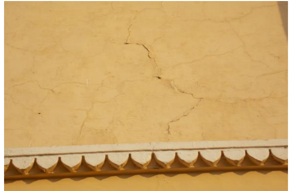
Photo 299 Plaster Crack on Wall No. 3 of Outer wall of Upper Ground Floor
