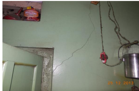
Photo 20 Inclined Crack on Wall No. 3 of Room No. 4, Part 3 Gyarah Rudra Mandir, Second Floor, Approx. Width = 1mm, Approx. Length = 0.6m. Distance from Wall No. 2 = 2m, Height from Floor = 1.7m.
