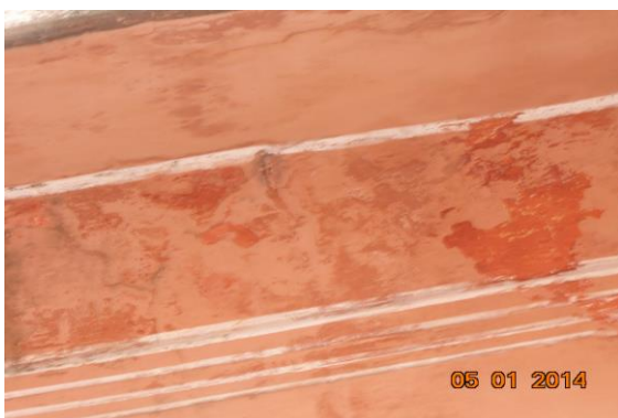
Photo 408 Dampness/Seepage on Wall No. 2 of Open Area 1 Shade of Part B1 Second Floor
