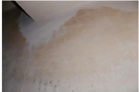
Photo 105 Dampness/Seepage on Wall No. 2 of Stair Case of Part A1 Upper Ground Floor
