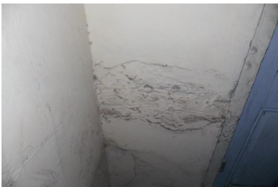
Photo 145 Peeling of Plaster on Wall No. 4 of Room No. 1 of Second Floor
