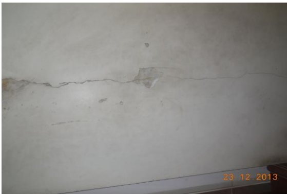
Photo 8 Horizontal Crack on Wall No. 1 of Staircase Third Floor to Fourth Floor Approx. Width = 0.6mm, Approx. Length = 2m. Distance from Wall No.4 = 0.6m, Height from Floor = 1.5m.
