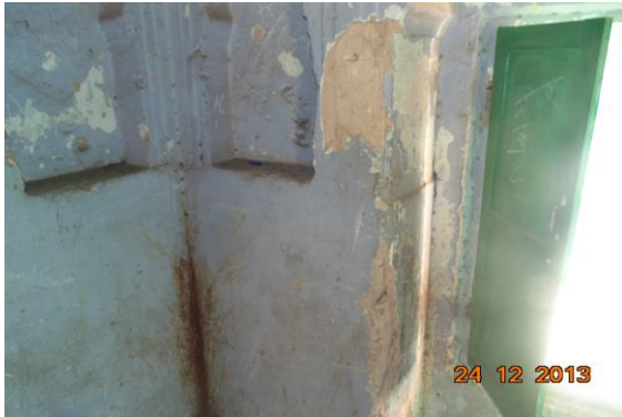
Photo 120 Peeling of Plaster on Roof of Hall No. 8 (Part A) of Shahid Amit Bhardwaj School, First Floor
