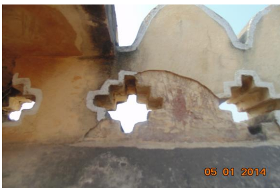
Photo 414 Peeling of Plaster on Wall No. 2 of Passage 1 of Part B1 Third Floor
