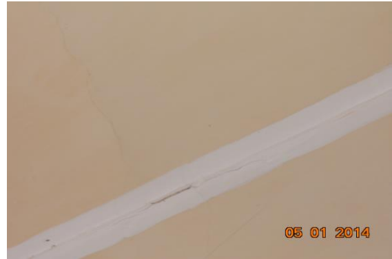
Photo 405 Plaster Crack on Roof of Room No. 1 of Part B1 Second Floor
