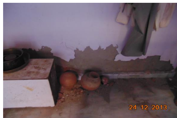
Photo 48 Peeling of Plaster on Wall No. 4 of Kitchen of First Floor
