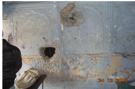
Photo 123 Peeling of Plaster on Roof of Hall No. 8 (Part B) of Shahid Amit Bhardwaj School, First Floor
