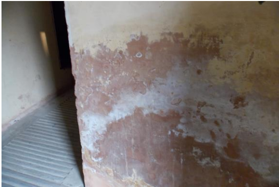
Photo 104 Dampness/Seepage on Wall No. 3 & 4 of Room No. 15 of Part A1 Upper Ground Floor
