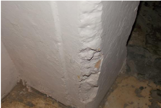
Photo 161 Peeling of Plaster on Wall No. 1 of Varanda No.3 of Second Floor
