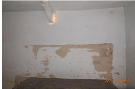
Photo 106 Dampness/Seepage on Wall No. 1, 3 & Roof of Hall No. 1 of Second Floor
