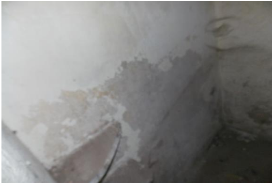
Photo 141 Peeling of Plaster on Wall No. 3 of Lobby of Second Floor
