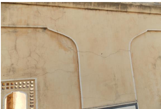
Photo 288 Plaster Crack on Wall No. 4 of Open Area 6 of Terrace of (A2+B2) Open Area
