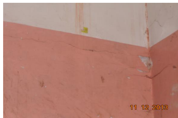
Photo 84 Horizontal Crack on Wall No. 1 of Staircase Area, First Floor Approx. Width = 0.3mm, Approx. Length = 1.2m. Distance from Wall No.4 = 0m, Height from Floor = 1.8m.
