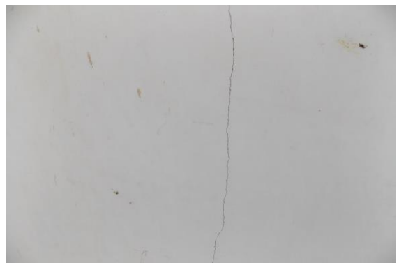
Photo 169 Plaster Crack on Wall No. 4 of Open Area of Part A2 Upper Ground Floor
