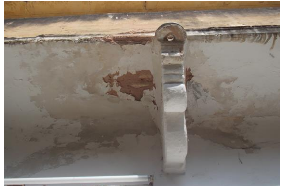
Photo 292 Peeling of Plaster on Sun Shade of Open sky of Ground Floor
