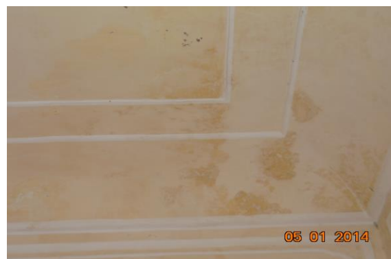
Photo 385 Dampness/Seepage on Roof of Room No. 4 of Part B1 First Floor
