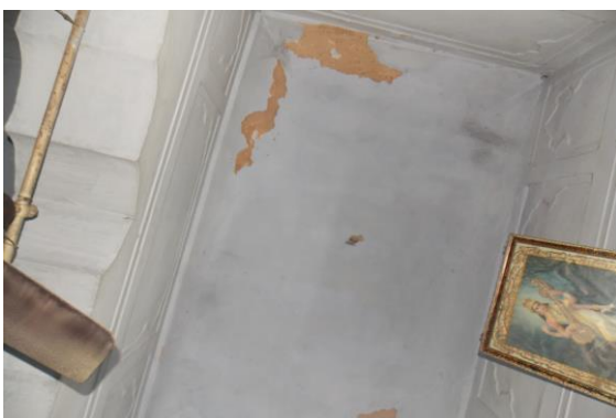
Photo 253 Peeling of Plaster on Roof of Hall No. 1 of Part B - Temple Shri Anand Bihari Ji, First Floor
