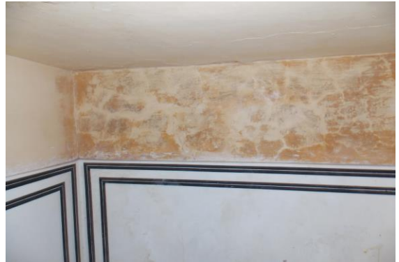
Photo 95 Dampness/Seepage on Wall No. 4 of Room No. 10 of Part A1 Upper Ground Floor
