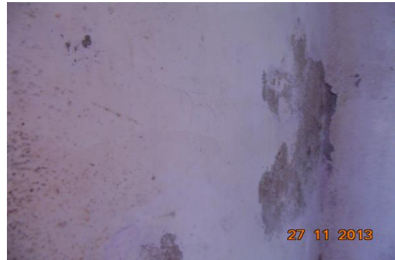
Photo 42 Dampness/Seepage on Outer Wall of First Floor
