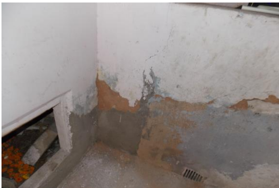
Photo 269 Peeling of Plaster on Wall No. 1 & 4 of Hanuman temple of Ground Floor
