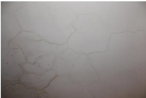
Photo 280 Dampness/Seepage on Roof of Open Gallery 1 of Terrace of (A2+B2) Open Area
