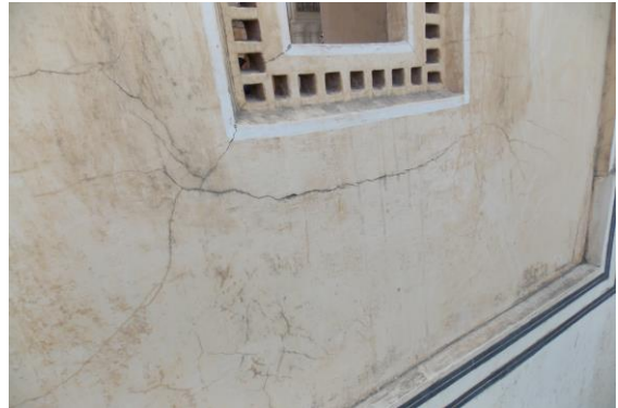
Photo 286 Peeling of Plaster on Parapet wall of Open Area 6 of Terrace of (A2+B2) Open Area
