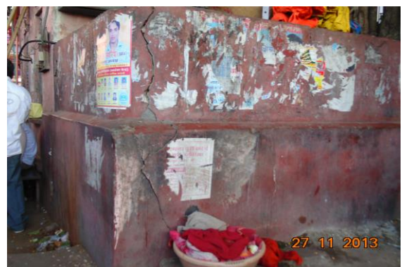
Photo 6 Peeling of Plaster on external Wall No. 2 of Ground Floor
