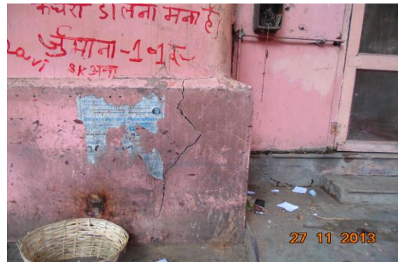
Photo 10 Peeling of Plaster on external Wall No. 3 of Ground Floor
