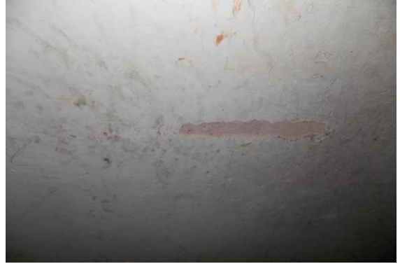
Photo 172 Peeling of Plaster on Wall No. 2 of Staircase First Floor To Second Floor of Second Floor
