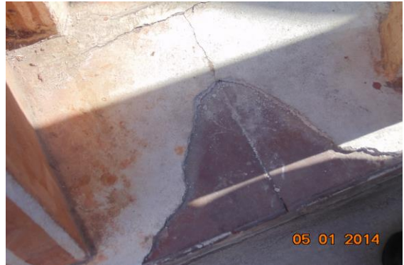
Photo 425 Peeling of Plaster on Floor of Balcony 3 of Part B1 Third Floor
