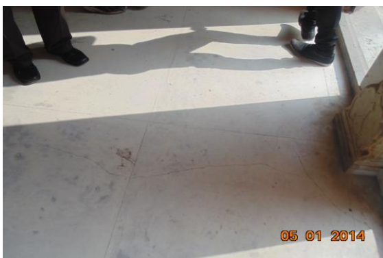
Photo 384 Plaster Crack on Floor of Room No. 4 of Part B1 First Floor
