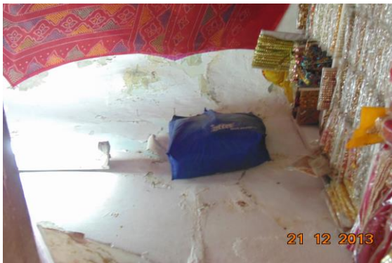
Photo 47 Dampness/Seepage on Wall No. 2 & Roof of Shop no.14 of Upper ground Floor
