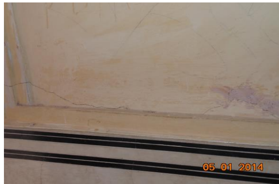
Photo 413 Plaster Crack on Wall No. 2 of Vranda 1 of Part B1 Second Floor
