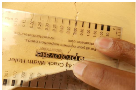
Photo 22A Horizontal Crack on of Minarate 1 L/S of Hawa Mahal , Part A1 Upper Ground Floor Approx. Width = 0.6mm, Approx. Length = 0.6m. Distance from Wall No.1 of Gate = 0m, Height Floor = 1.2m.
