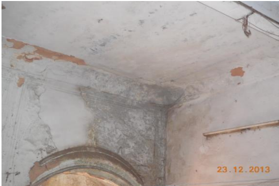
Photo 107 Dampness/Seepage on Wall No. 1, 4 & Roof of Police Station of Second Floor
