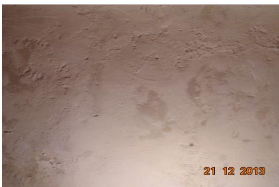
Photo 15 Horizontal Crack on Roof of Varanda of shop, Ground floor Approx. Width = 3mm, Approx. Length = 2.5m. Distance from Rightside External Column = 0m, Height from Floor = 3m.
