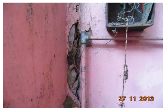
Photo 12 Peeling of Plaster on external Wall No. 1 of Ground Floor
