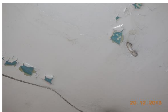
Photo 77 Peeling of Plaster on Roof of Varanda of Shop no. 9, Ground Floor
