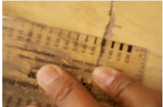
Photo 21A Horizontal Crack on of Minarate 1 L/S of Hawa Mahal , Part A1 Upper Ground Floor Approx. Width = 1mm, Approx. Length = 0.5m Distance from Wall No.1 of Gate = 0.7m, Height from Floor = 1m.
