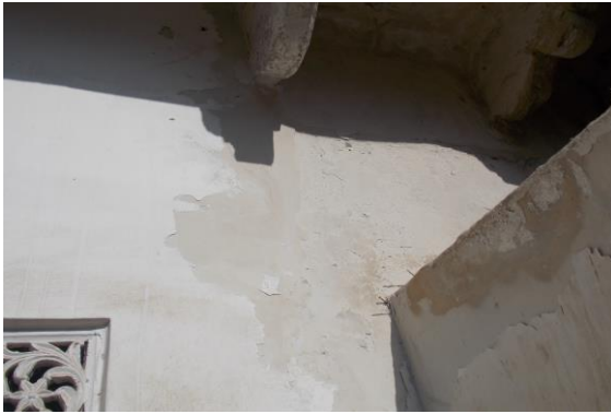
Photo 291 Peeling of Plaster on Wall No. 2 of Open sky of Ground Floor
