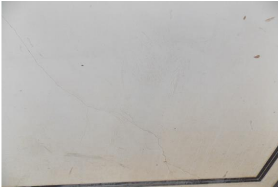
Photo 202 Plaster Crack on Wall No. 4 of Open Area 2 of Part A2 Upper Ground Floor
