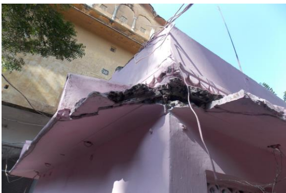
Photo 295 Damaged Portion on Sun Shade of Part B of Temple Shri Anand Bihari Ji of Ground Floor
