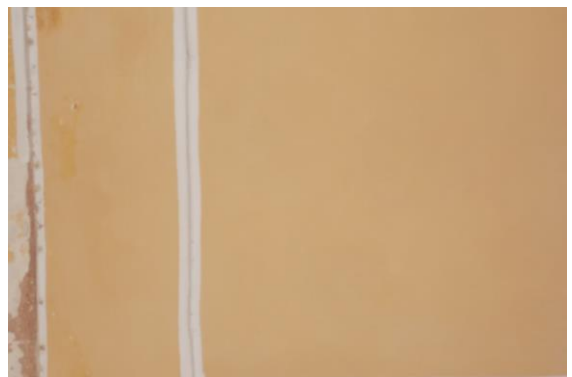
Photo 97 Peeling of Plaster on Roof of Room No. 10 of Part A1 Upper Ground Floor
