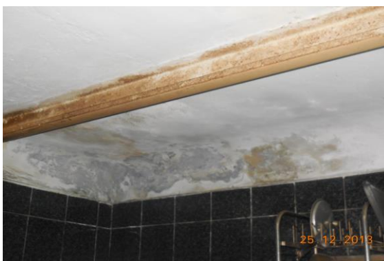
Photo 15 Dampness/Seepage on Roof & Wall No.4 of Kitchen of First Floor
