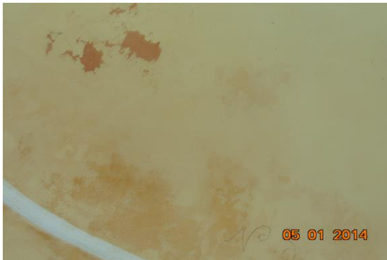
Photo 410 Dampness/Seepage on Roof of Tomb 2 of Part B1 Second Floor
