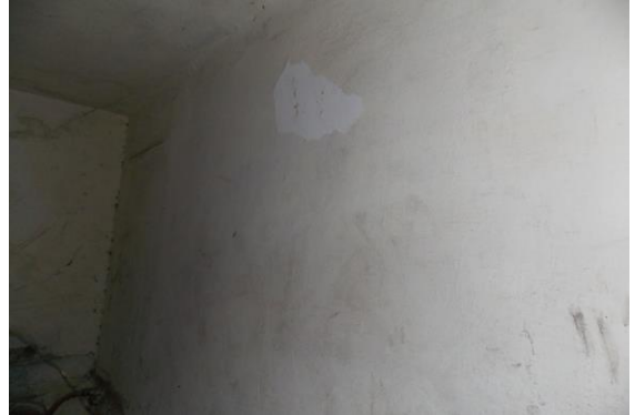
Photo 132 Peeling of Plaster on Wall No. 3 of Toilet & Washroom of Second Floor
