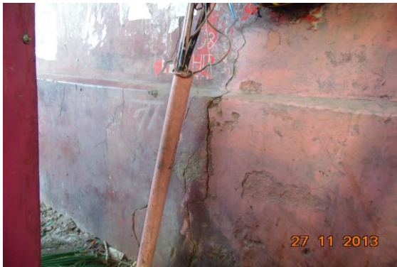
Photo 7 Peeling of Plaster on external Wall No. 2 of Ground Floor
