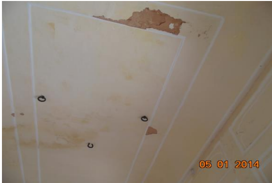
Photo 386 Dampness/Seepage on Roof of Vrandra 3 of Part B1 First Floor
