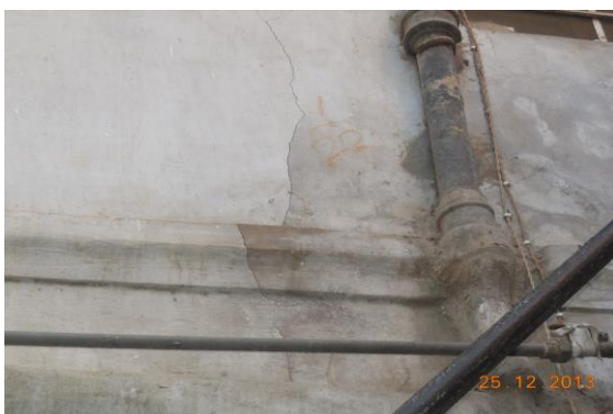
Photo 23 Inclined Crack on External Wall of Back Side, Approx. Width = 1.6mm, Approx. Length = 2.6m. Distance from Shop No. 1 = 1.8m, Height from Floor = 1.6m.
