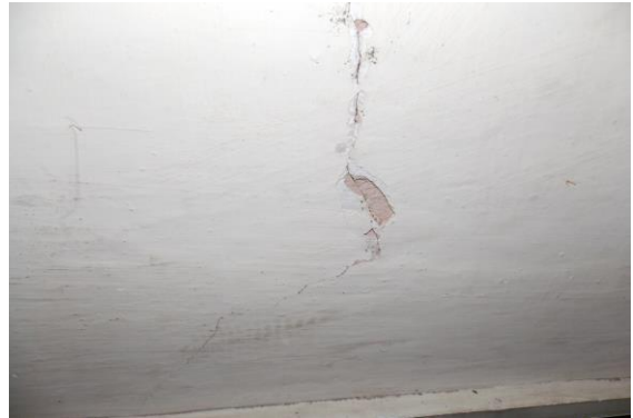
Photo 249 Plaster Crack on Wall No. 2 of Gallery 8 of Part B2 Upper Ground Floor
