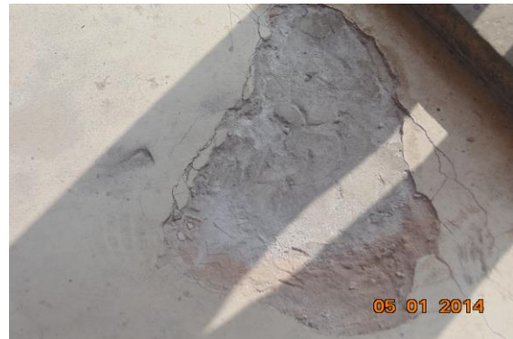
Photo 381 Peeling of Plaster on Floor of Room No. 4 of Part B1 First Floor
