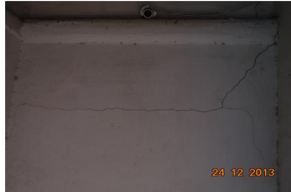
Photo 14 Inclined Crack on Wall No. 2 of Bathroom No. 1, Temple Shri Chandra Vihari Ji, First Floor, Approx. Width = 0.6mm, Approx. Length = 1m. Distance from Wall No. 4 = 0m, Height from Floor = 1.7m.
