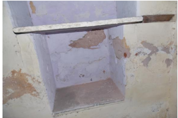
Photo 142 Peeling of Plaster on Wall No. 4 of Room No. 2 of Second Floor
