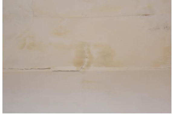
Photo 244 Peeling of Plaster on Wall No. 3 & Roof of Passage No.5 of First Floor
