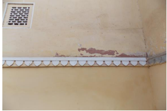
Photo 297 Peeling of Plaster on Wall No. 3 of Outer wall of Ground Floor
