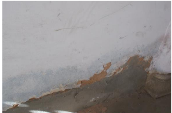
Photo 268 Peeling of Plaster on Wall No. 1 of Hanuman temple of Ground Floor
