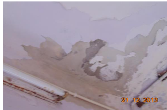
Photo 48 Dampness/Seepage on Roof of Varanda of shop of Ground Floor
