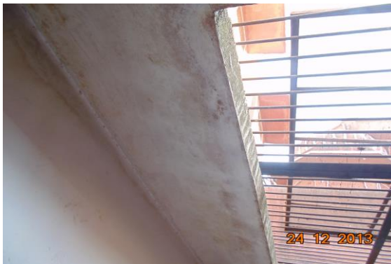
Photo 45 Dampness/Seepage on Wall No. 1 of Open Sky of First Floor
