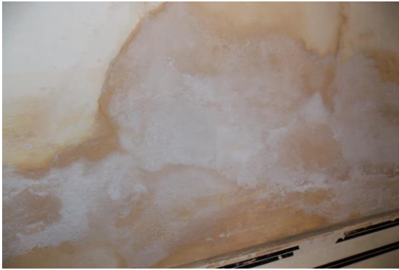
Photo 218 Dampness/Seepage on Wall No. 1 of Gallery 8 of Part A2 Upper Ground Floor
