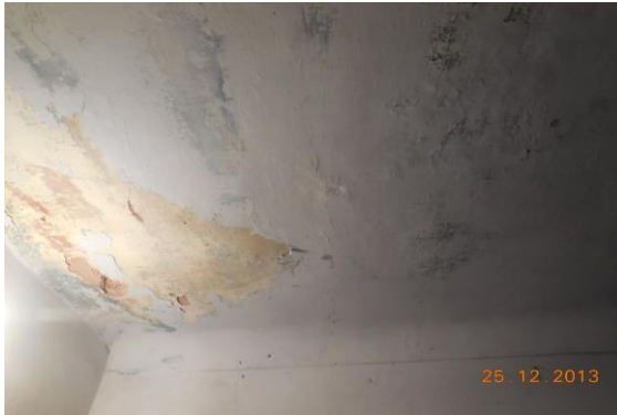
Photo 11 Dampness/Seepage on Roof of Lobby of Second Floor
