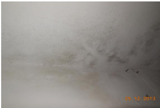
Photo 13 Dampness/Seepage on Roof of Passage No.2 of Second Floor
