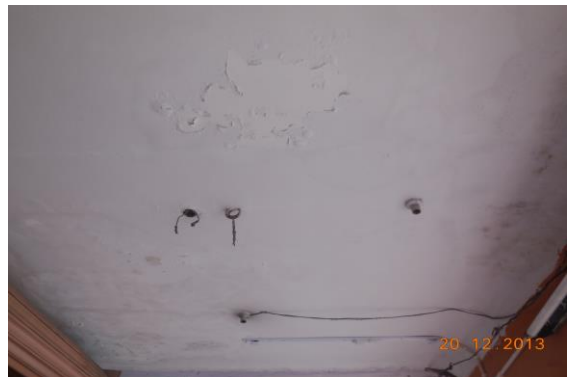
Photo 75 Dampness/Seepage on Roof of Varanda of Shop no.8, Ground Floor
