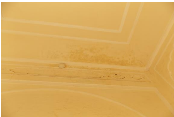
Photo 222 Dampness/Seepage on Wall No. Roof & 1 of Vrandra 10 of Part A2 Upper Ground Floor
