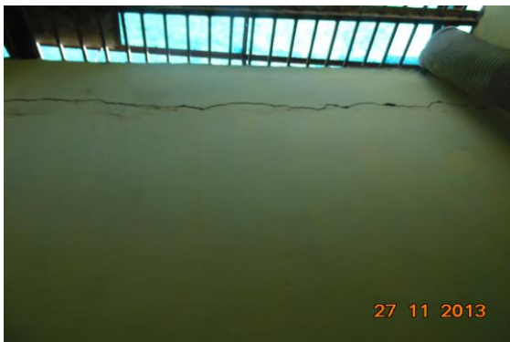
Photo 15 Horizontal Crack on Wall No. 1, 3 & 4 of Passage, First Floor Approx. Width = 4mm, Approx. Length = 4.5m. Distance from Wall No. 3 = 0m, Height from Floor = 3.2m.
