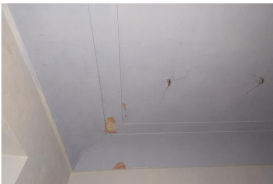
Photo 157 Peeling of Plaster on Roof of Room No. 7 of Second Floor
