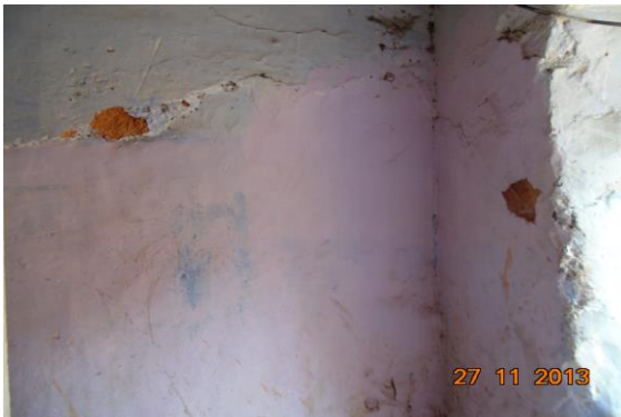
Photo 43 Peeling of Plaster on Wall No. 2 & 3 of Passage Area of First Floor
