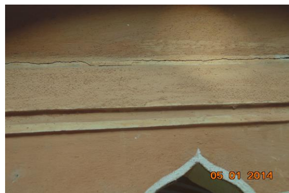
Photo 409 Plaster Crack on Wall No. 3 of Tomb 2 Outer Wall of Part B1 Second Floor
