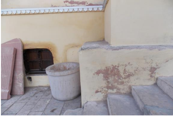
Photo 296 Peeling of Plaster on Outer wall of Ground Floor
