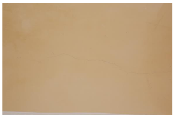
Photo 109 Plaster Crack on Roof of Vrandha 4 of Part A1 Upper Ground Floor
