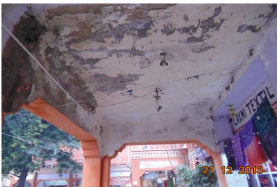
Photo 55 Dampness/Seepage on Roof of Varanda of shop of Ground Floor
