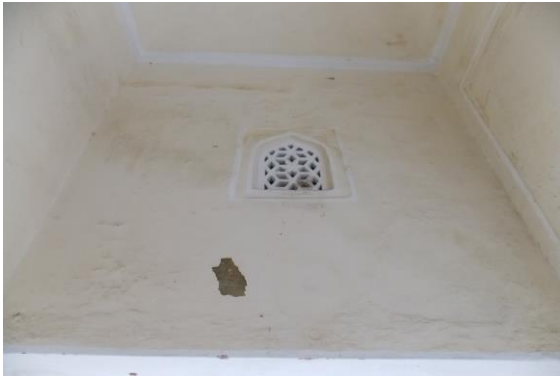
Photo 166 Dampness/Seepage on Wall No. 3 of Vrandha 4 of Part A2 Upper Ground Floor
