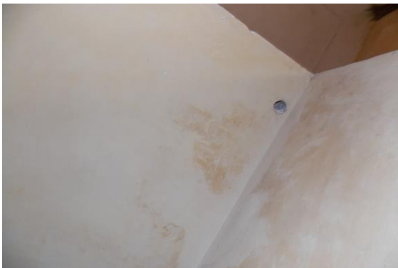
Photo 106 Dampness/Seepage on Roof of Stair Case of Part A1 Upper Ground Floor
