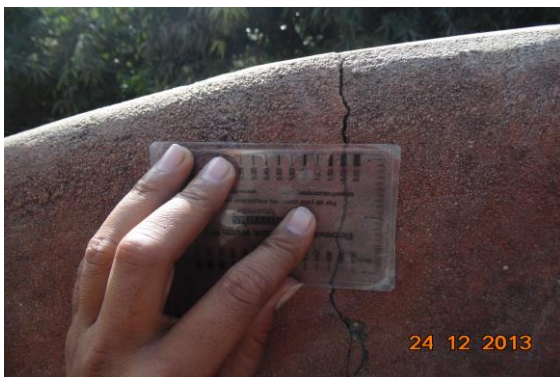
Photo 15A Inclined Crack on Wall No. 2 of Second Floor, Approx. Width = 2mm, Approx. Length = 1.5m. Distance from Wall No. 3 = 0.1m, Height from Floor = 0m.
