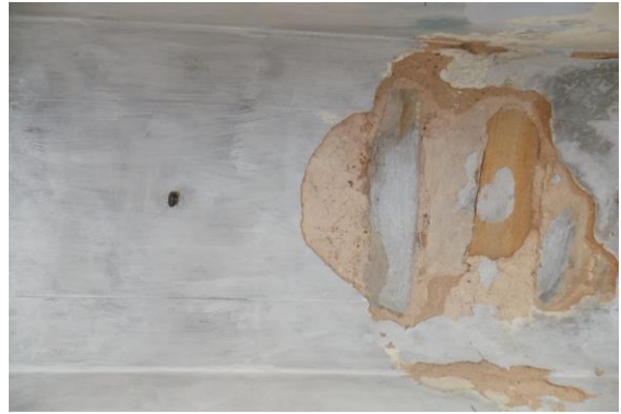
Photo 274 Peeling of Plaster on Roof of Varanda No.2 of Ground Floor
