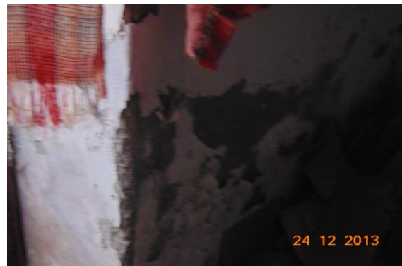
Photo 52 Peeling of Plaster on Wall No. 3 of Kitchen of First Floor
