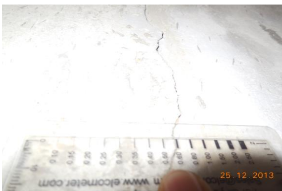
Photo 4A Inclined Crack on Wall No. 2 of Room No. 1, Second Floor, Approx. Width = 0.6mm, Approx. Length = 0.6m. Distance from Wall no.4 = 2.8m, Height from Floor = 1.8m.
