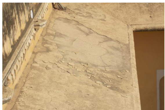
Photo 253 Peeling of Plaster on Sunshade of Open Area 2 of Terrace of (A2+B2) Open Area
