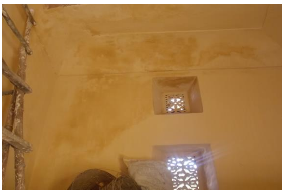
Photo 241 Dampness/Seepage on Roof & Wall No. 4 of Hall No. 5 of Temple Shri Anand Bihari Ji, First Floor
