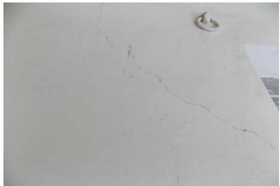
Photo 205 Plaster Crack on Wall No. 1 of Gallery 7 of Part A2 Upper Ground Floor
