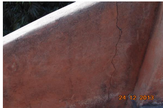
Photo 15 Inclined Crack on Wall No. 2 of Second Floor, Approx. Width = 2mm, Approx. Length = 1.5m. Distance from Wall No. 3 = 0.1m, Height from Floor = 0m.
