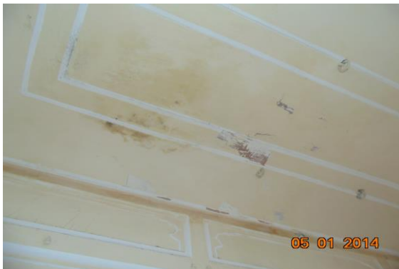
Photo 406 Dampness/Seepage on Roof of Vrandra 2 of Part B1 Second Floor
