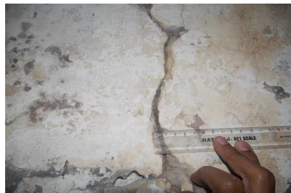
Photo 28A Inclined Crack on Wall No. 4 of Open Varanda No.2, Second Floor Approx. Width = 5mm, Approx. Length = 1.2m. Distance from Wall No.1 = 2.2m, Height from Floor = 1.3m.
