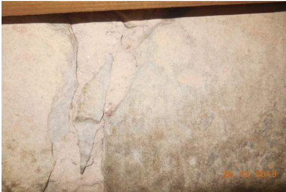
Photo 24 Peeling of Plaster on Wall No. 1 of Shop No. 3 of Ground Floor
