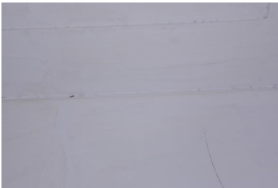
Photo 155 Peeling of Plaster on Roof of Room No. 6 of Second Floor
