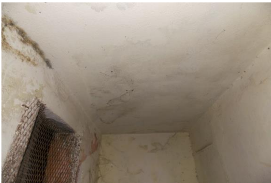
Photo 133 Dampness/Seepage on Roof of Toilet & Washroom of Second Floor
