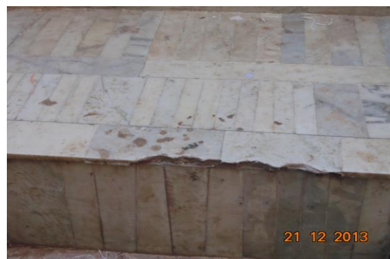
Photo 50 Peeling of Plaster on Floor of Varanda of shop of Ground Floor
