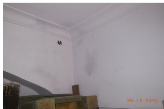
Photo 22 Horizontal Crack on Wall No. 4 of Room No. 4, Part 3 Gyarah Rudra Mandir, Second Floor Approx. Width = 0.8mm, Approx. Length = 0.9m. Distance from Wall No. 1 = 0m Height from Floor = 2.4m
