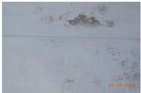
Photo 80 Peeling of Plaster on of Police Station of Ground Floor
