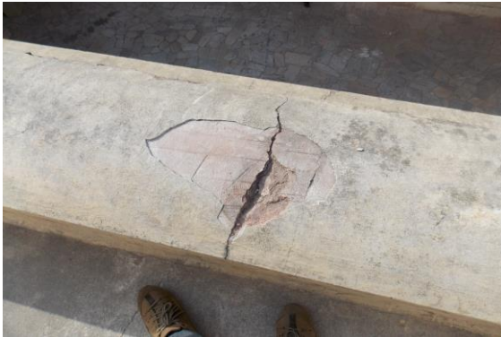
Photo 286 Peeling of Plaster on Parapet wall of Open Area 6 of Terrace of (A2+B2) Open Area
