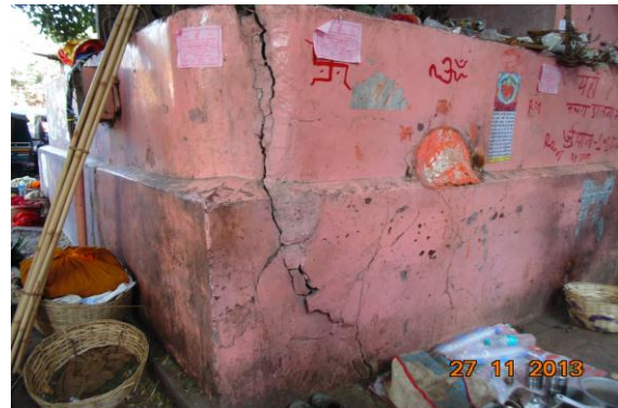
Photo 8 Peeling of Plaster on external Wall No. 3 of Ground Floor
