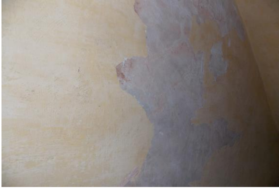
Photo 92 Peeling of Plaster on Wall No. 4 of Room No. 3 of Part A1 Upper Ground Floor
