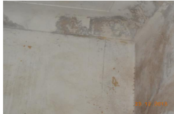
Photo 108 Peeling of Plaster on Roof of Hall No. 2 of Second Floor
