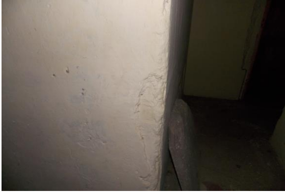
Photo 171 Peeling of Plaster on Wall No. 3 of Open Varanda of Second Floor
