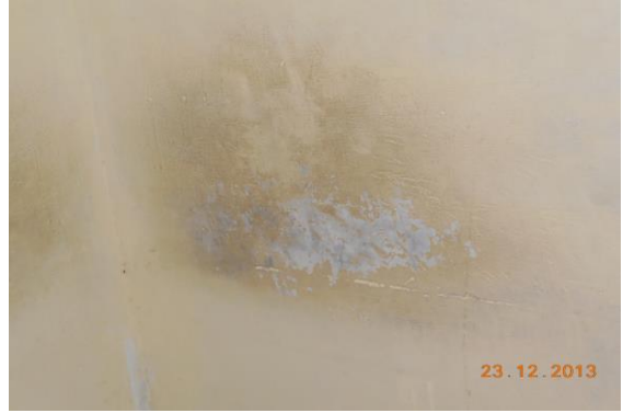
Photo 76 Peeling of Plaster on Wall No. 4 of Room No. 4 of Ground Floor
