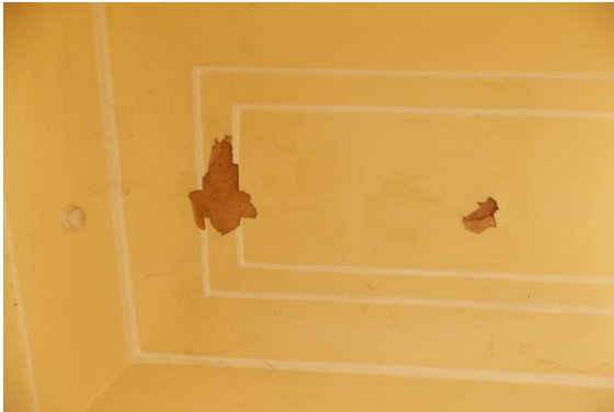
Photo 160 Peeling of Plaster on Roof of Vrandha 2 of Part A2 Upper Ground Floor
