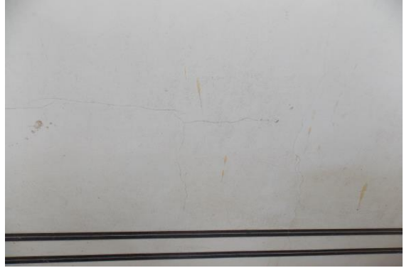
Photo 201 Plaster Crack on Wall No. 3 of Open Area 2 of Part A2 Upper Ground Floor
