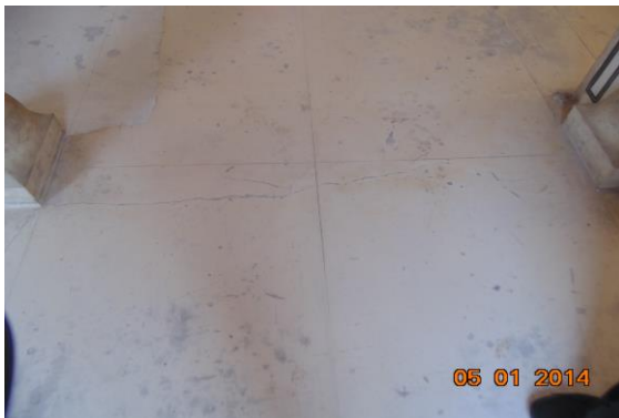
Photo 388 Plaster Crack on Floor of Vrandra 2 of Part B1 First Floor
