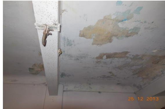
Photo 12 Dampness/Seepage on Roof of Lobby of Second Floor
