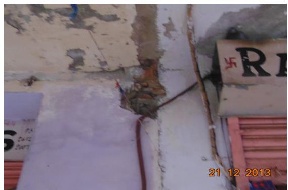
Photo 56 Peeling of Plaster on Frontside Wall No.3 of Shop No.17 of Ground Floor
