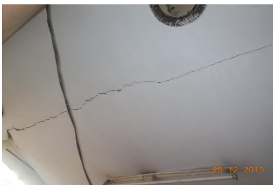
Photo 5 Inclined Crack on Corridor, Part 4 Gyarah Rudra Mandir of First floor, Approx. Width = 5mm, Approx. Length = 6m. Distance from Main Door = 1m, Height from Floor = 3m.
