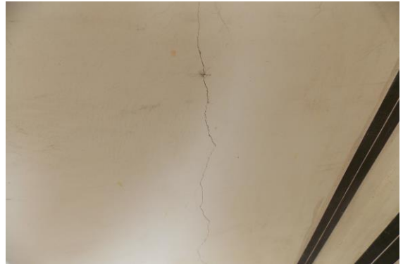
Photo 161 Plaster Crack on Wall No. 2 of Vrandha 2 of Part A2 Upper Ground Floor
