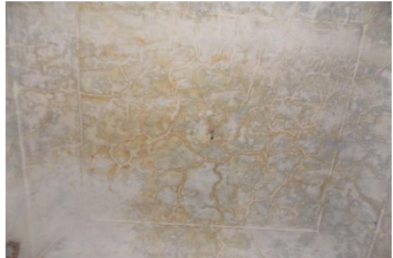
Photo 126 Dampness/Seepage on Roof of Varanda of Second Floor
