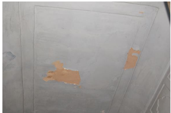
Photo 252 Peeling of Plaster on Roof of Hall No. 1 of Part B - Temple Shri Anand Bihari Ji, First Floor
