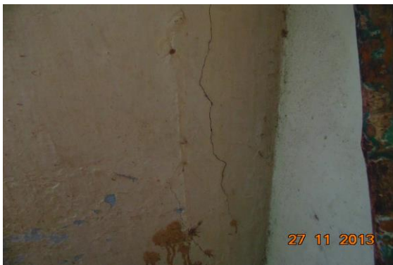
Photo 21 Inclined Crack on Wall No. 3 of Bsnl Office, First Floor Approx. Width = 0.5mm, Approx. Length = 1m. Distance from Wall No. 1 = 0m, Height from Floor = 0.4m.
