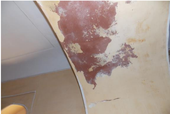
Photo 278 Peeling of Plaster on Roof of Open Gallery 1 of Terrace of (A2+B2) Open Area
