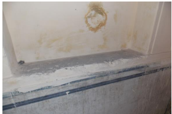
Photo 240 Peeling of Plaster on Wall No. 4 of Varanda No.3 of First Floor
