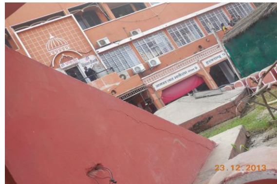
Photo 4 Horizontal Crack on Outside Wall No.2 of Staircase, Ground Floor Approx. Width = 0.4mm, Approx. Length = 1.5m. Distance from Main Gate = 2m, Height from Floor = 0m.
