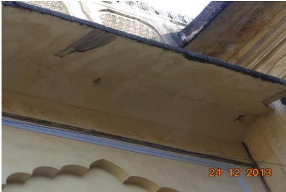
Photo 234 Damaged Portion on Wall No. 1 & Shade of Balcony of First Floor
