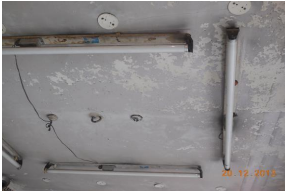
Photo 72 Dampness/Seepage on Roof of Varanda of Shop no.6, Ground Floor
