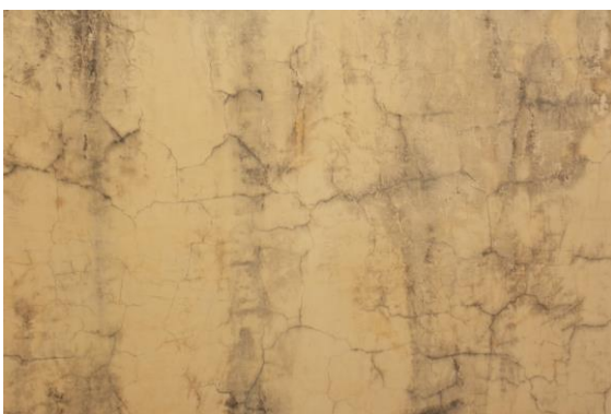
Photo 252 Dampness/Seepage on Wall No. 1 of Open Area 2 of Terrace of (A2+B2) Open Area
