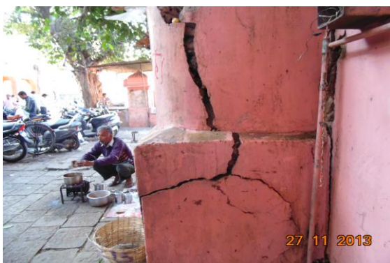
Photo 11 Peeling of Plaster on external Wall No. 1 of Ground Floor
