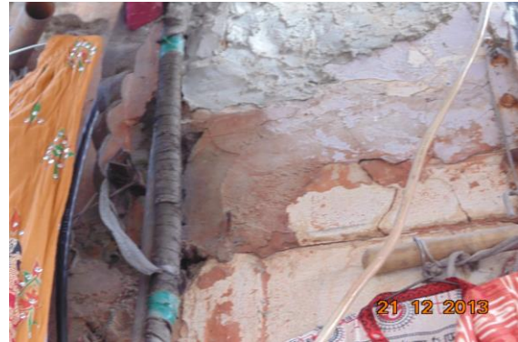
Photo 25 Peeling of Plaster on Wall No. 5 of Keshi international of Ground Floor
