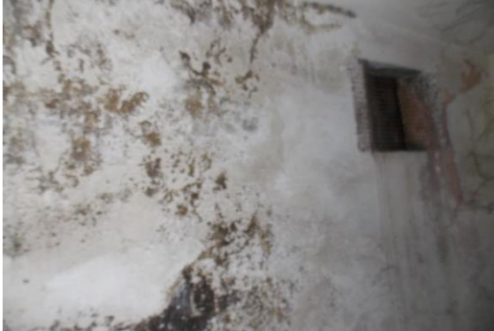
Photo 131 Peeling of Plaster on Wall No. 4 of Toilet & Washroom of Second Floor
