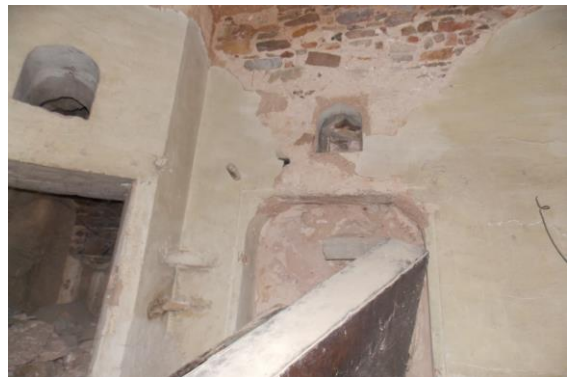
Photo 270 Damaged Portion on Wall No. 4 of Store of Ground Floor
