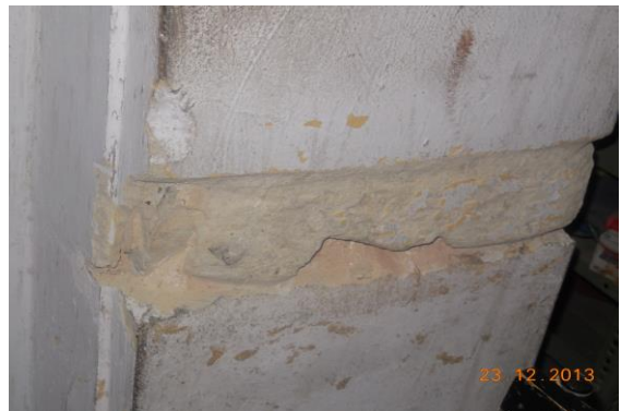
Photo 86 Peeling of Plaster on Wall No. 4 of Room No. 8 of Ground Floor
