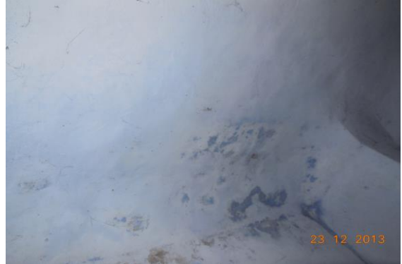
Photo 84 Dampness/Seepage on Roof of Room No. 7 of Ground Floor
