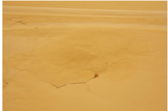
Photo 221 Peeling of Plaster on Wall No. 2 of Vrandra 10 of Part A2 Upper Ground Floor
