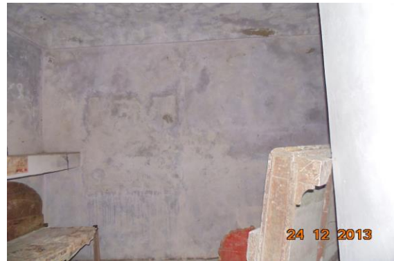
Photo 50 Dampness/Seepage on Wall No. 4 of Gallery No.3 of First Floor
