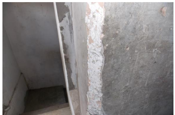
Photo 248 Peeling of Plaster on Wall No. 4 of Passage No.7 of First Floor
