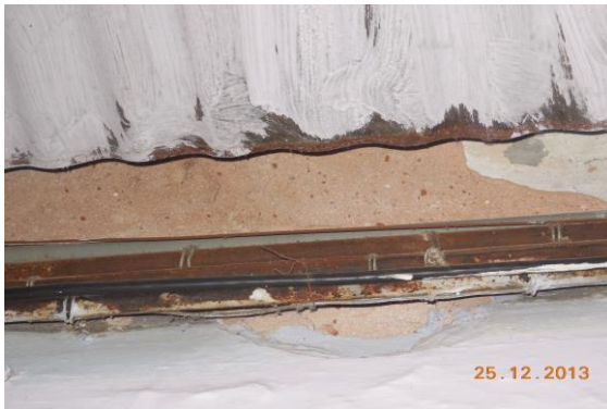
Photo 37 Peeling of Plaster on Wall No. 4 of Shop No. 1 of Ground Floor
