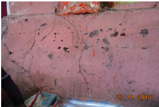
Photo 9 Peeling of Plaster on external Wall No. 3 of Ground Floor
