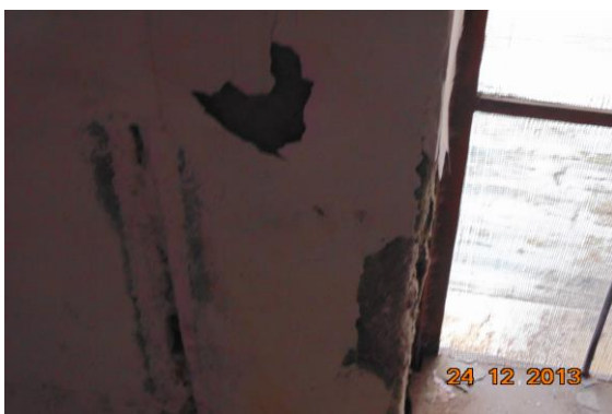
Photo 53 Peeling of Plaster on Wall No. 3 of Kitchen of First Floor
