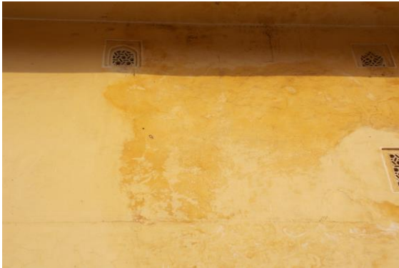
Photo 298 Dampness/Seepage on Wall No. 3 of Outer wall of Upper Ground Floor
