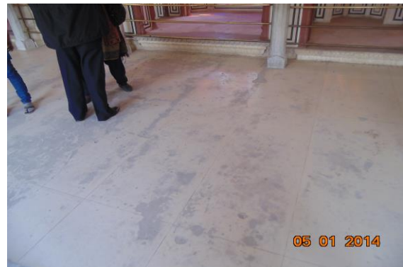
Photo 389 Dampness/Seepage on Floor of Room No. 3 of Part B1 First Floor
