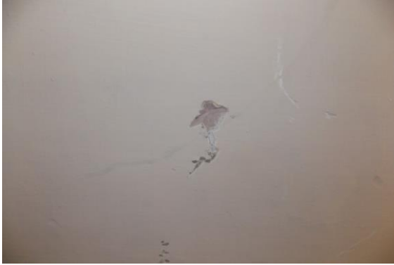
Photo 243 Peeling of Plaster on Wall No. 3 of Passage No.5 of First Floor
