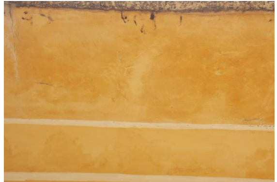
Photo 167 Dampness/Seepage on Wall No. 3 of Sunshade of Part A2 Upper Ground Floor
