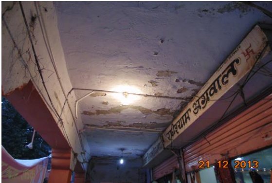
Photo 57 Dampness/Seepage on the roof of the Varanda of a shop on the ground floor
