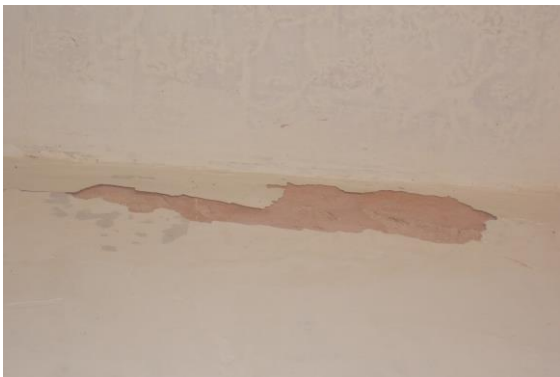
Photo 204 Peeling of Plaster on Wall No. 1 of Gallery 5 of Part A2 Upper Ground Floor
