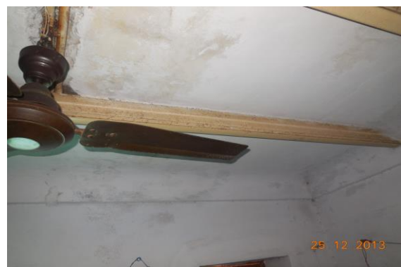
Photo 16 Dampness/Seepage on Roof & Wall No.4 of Kitchen of First Floor
