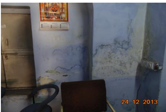
Photo 28 Peeling of Plaster on Outer Wall No.3 of Varanda of Ground Floor
