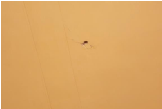
Photo 237 Peeling of Plaster on Roof of Passage No.3 of First Floor
