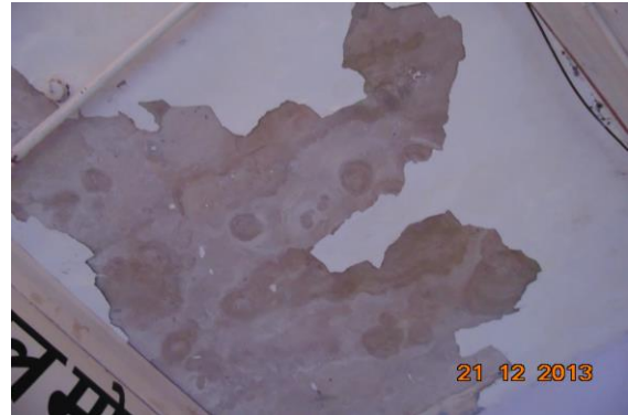
Photo 58 Peeling of Plaster on Roof of Varanda of Shop of Ground floor
