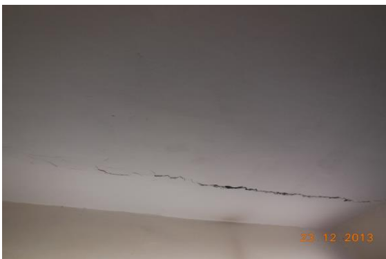
Photo 9 Horizontal Crack on Roof of Toilet No. 1, K.K.Saree Godown Above Shop No.15 & 16, Fourth Floor, Approx. Width = 5mm, Approx. Length = 1.2m. Distance from Wall No 3 = 0m Height from Floor = 2.5m
