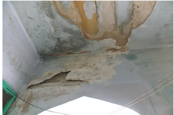
Photo 276 Peeling of Plaster on Wall No. 3 & Roof of Varanda No.2 of Ground Floor
