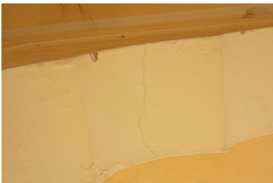
Photo 162 Plaster Crack on Roof of Gate of Part A2 Upper Ground Floor
