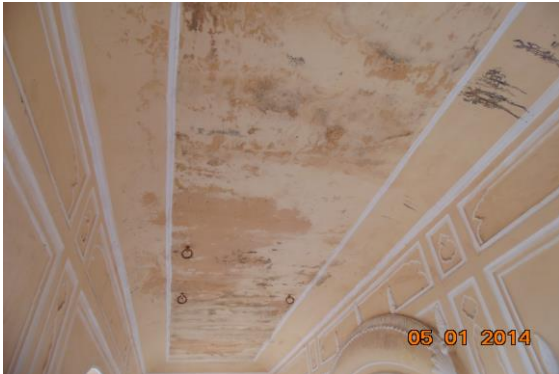
Photo 424 Dampness/Seepage on Roof of Vranda 1 of Part B1 Third Floor
