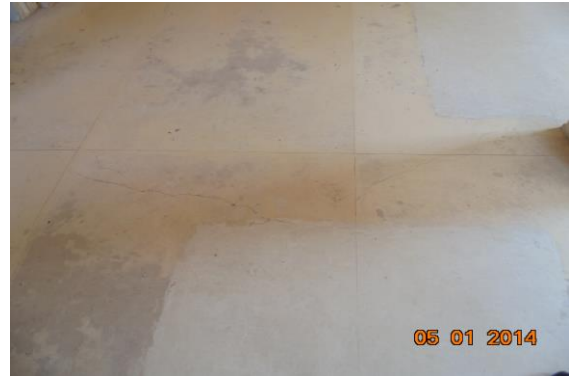
Photo 387 Plaster Crack on Floor of Vrandra 3 of Part B1 First Floor
