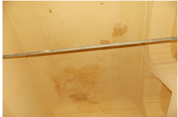
Photo 238 Dampness/Seepage on Roof of Varanda No.3 of First Floor
