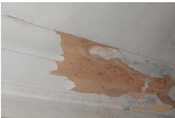
Photo 109 Dampness/Seepage on Wall No. 1 & Roof of Room No. 1 (Part A) of Second Floor
