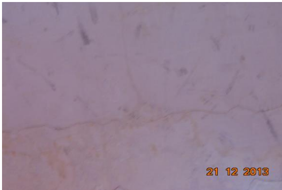
Photo 45 Peeling of Plaster on Beam of Part c of shop no.12 of Ground Floor
