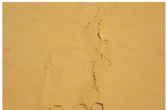
Photo 301 Plaster Crack on Wall No. 3 of Upper Ground Floor
