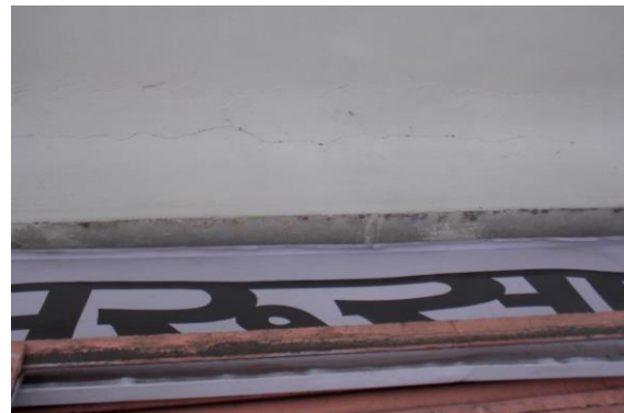
Photo 16 Horizontal Crack on Varandah Roof, Shop No. 195, Ground Floor Approx. Width = 0.35mm, Approx. Length = 2.5m. Distance from Right External Col = 0m, Height from Floor = 3m.
