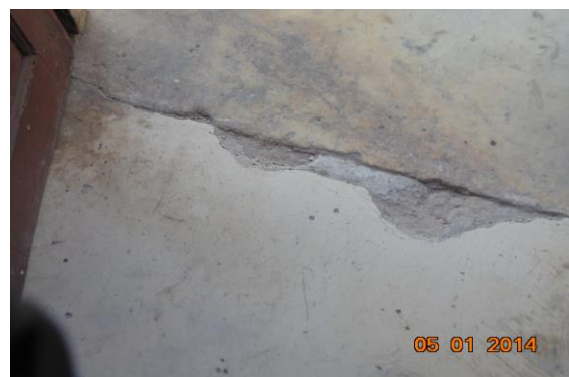
Photo 391 Peeling of Plaster on Floor of Vrandra 1 of Part B1 First Floor
