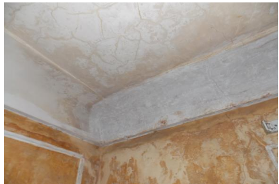
Photo 281 Dampness/Seepage on Wall No. 1, 4 & Roof of Open Gallery 1 of Terrace of (A2+B2) Open Area
