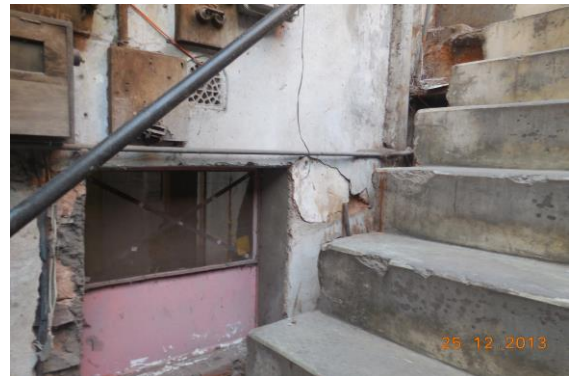
Photo 38 Peeling of Plaster on External Wall of Back Side of Gyarah Rudrah Mandir
