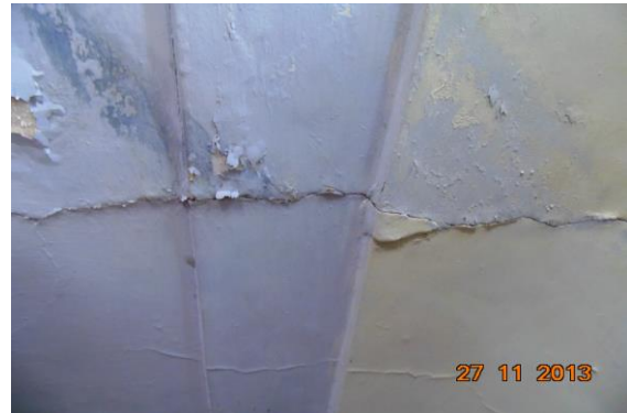
Photo 20 Inclined Crack on Roof of Bsnl Office , First Floor Approx. Width = 1mm, Approx. Length = 2.5m. Distance from Wall No. 1 = 2.6m, Height from Floor = 2.1m.
