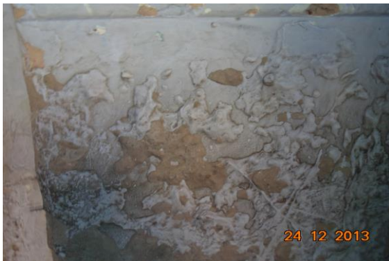
Photo 122 Peeling of Plaster on Wall No. 4 of Hall No. 8 (Part A) of Shahid Amit Bhardwaj School, First Floor
