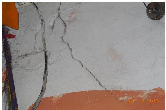
Photo 42 Horizontal Crack on Internal Column Right Side of Varanda, Shop no.2, Ground Floor Approx. Width = 2mm, Approx. Length = 0.2m. Distance Internal Column Right side = 0m, Height Floor = 3m.
