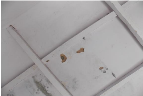
Photo 267 Peeling of Plaster on Floor of Hanuman temple of Ground Floor
