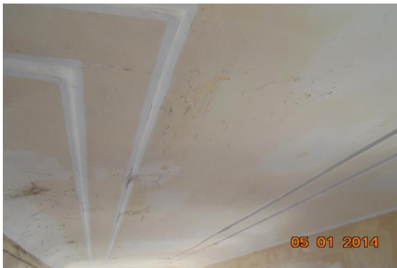
Photo 442 Dampness/Seepage on Roof of Passage 4 of Part B1 4th Floor
