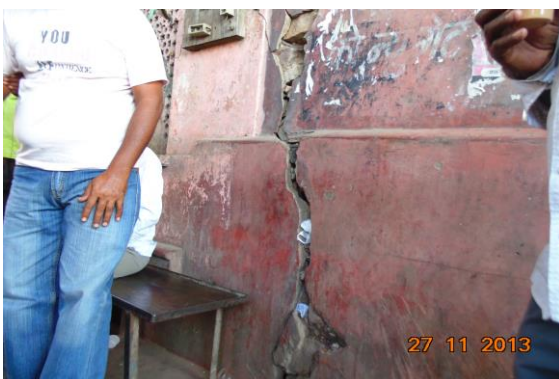
Photo 5 Peeling of Plaster on External Wall No. 4 of Ground Floor
