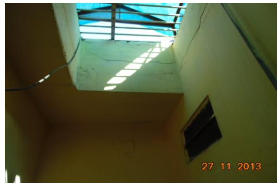
Photo 16 Horizontal Crack on Wall No. 1, 3 & 4 of Passage, First Floor Approx. Width = 4mm, Approx. Length = 4.5m. Distance from Wall No. 3 = 0m, Height from Floor = 3.2m.
