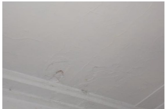
Photo 156 Peeling of Plaster on Roof of Room No. 7 of Second Floor
