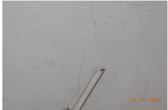
Photo 40 Horizontal Crack on Roof of Varanda, Shop no.2, Ground Floor Approx. Width = 0.4mm, Approx. Length = 2m. Distance External Column Left side = 1.5m, Height Floor = 3.5m.
