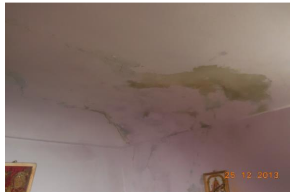
Photo 14 Dampness/Seepage on Roof of Varanda of First Floor
