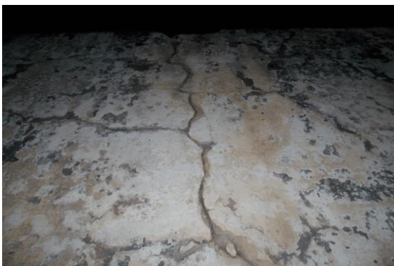
Photo 28 Inclined Crack on Wall No. 4 of Open Varanda No.2, Second Floor Approx. Width = 5mm, Approx. Length = 1.2m. Distance from Wall No.1 = 2.2m, Height from Floor = 1.3m.
