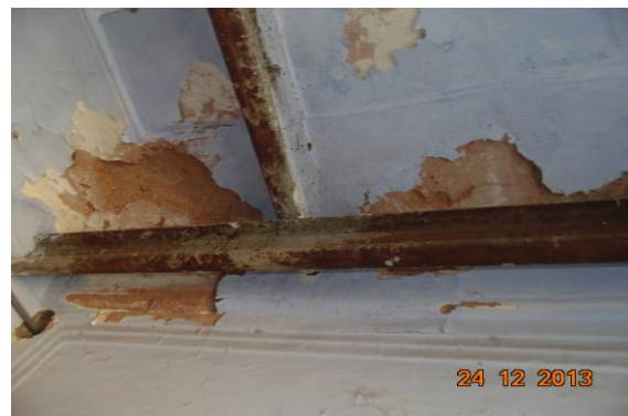
Photo 125 Peeling of Plaster on Wall No. 4 of Hall No. 8 (Part B) of Shahid Amit Bhardwaj School, First Floor
