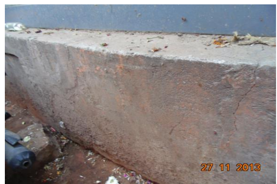
Photo 6 Plaster Crack on Platform of Transformer of Ground Floor
