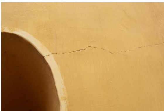
Photo 22 Horizontal Crack on of Minarate 1 L/S of Hawa Mahal , Part A1 Upper Ground Floor Approx. Width = 0.6mm, Approx. Length = 0.6m. Distance from Wall No.1 of Gate = 0m, Height Floor = 1.2m.
