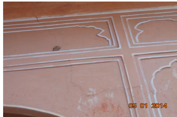
Photo 407 Plaster Crack on Wall No. 3 of Open Area 1 of Part B1 Second Floor
