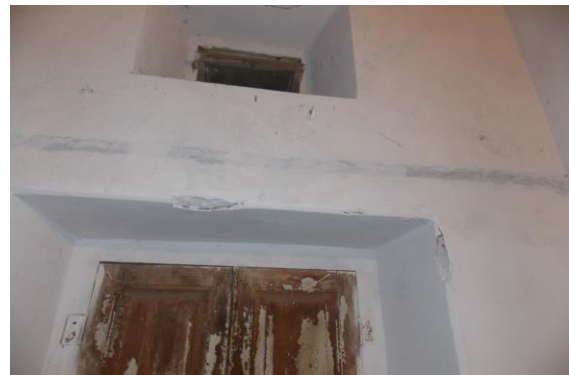
Photo 27 Horizontal Crack on Roof of Varanda No.3, Second Floor Approx. Width = 3mm, Approx. Length = 1.3m. Distance from Wall No.3 = 0.02m, Height from Floor = 3.3m.
