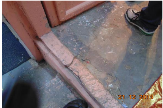
Photo 40 Peeling of Plaster on Floor of Part A of shop no.13 of Ground Floor
