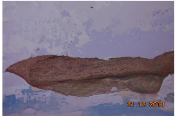
Photo 52 Peeling of Plaster on Roof of Varanda of shop of Ground Floor
