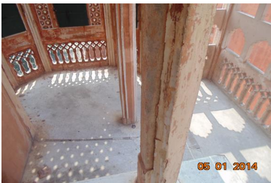
Photo 426 Dampness/Seepage on Pillor of Balcony 3 of Part B1 Third Floor
