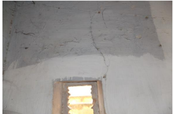
Photo 250 Peeling of Plaster on Wall No. 1 of Passage No.7 of First Floor
