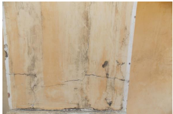
Photo 251 Plaster Crack on Wall No. 4 of Open Area 2 of Terrace of (A2+B2) Open Area
