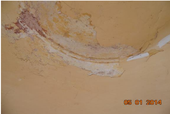
Photo 422 Peeling of Plaster on Roof of Tomb 6 of Part B1 Third Floor
