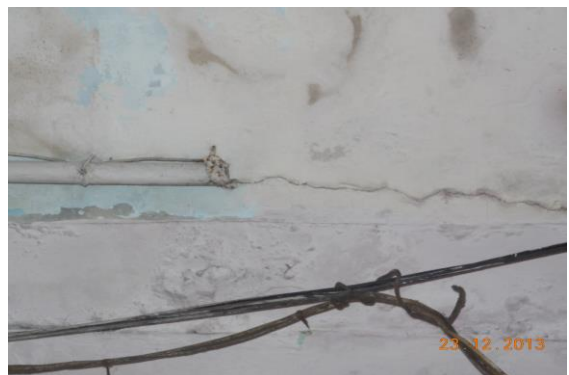
Photo 10 Horizontal Crack on Roof of Varanda of Shop No.16, Ground Floor, Approx. Width = 1mm, Approx. Length = 2.5m. Distance from Rightside External Column = 0m, Height from Floor = 3m.
