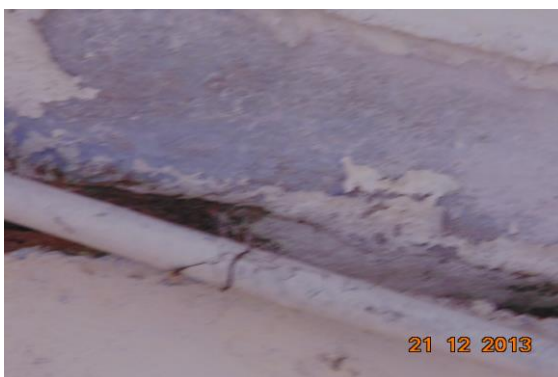
Photo 49 Peeling of Plaster on Roof of Varanda of shop of Ground Floor
