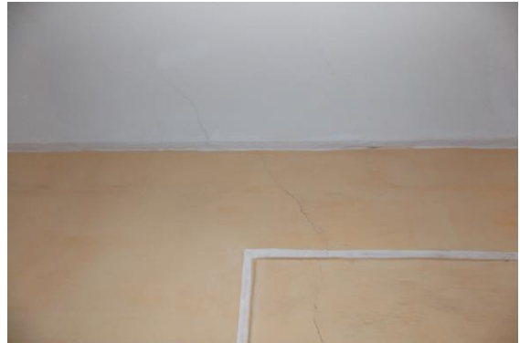
Photo 279 Plaster Crack on Wall No. 4 & Roof of Open Gallery 1 of Terrace of (A2+B2) Open Area
