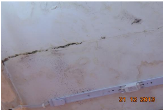
Photo 59 Peeling of Plaster on Roof of Varanda of Shop of Ground floor
