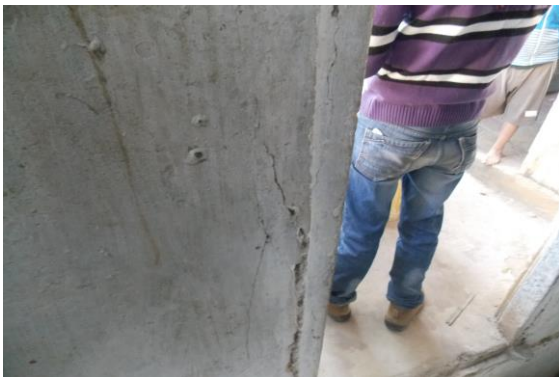
Photo 251 Peeling of Plaster on Wall No. 1 of Passage No.7 of First Floor
