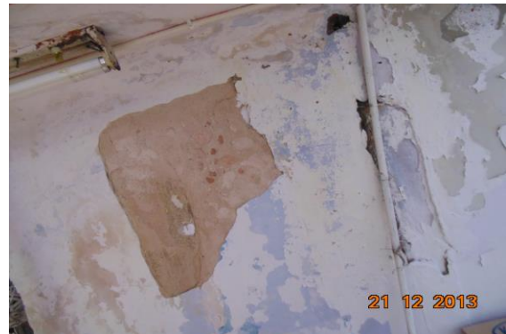
Photo 46 Dampness/Seepage on of varanda of shop of Ground Floor
