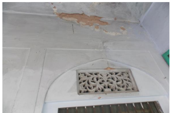
Photo 278 Peeling of Plaster on Wall No. 4 of Varanda No.2 of Ground Floor
