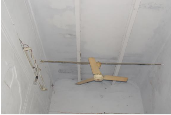
Photo 129 Dampness/Seepage on Roof of Room No. 3 of Second Floor
