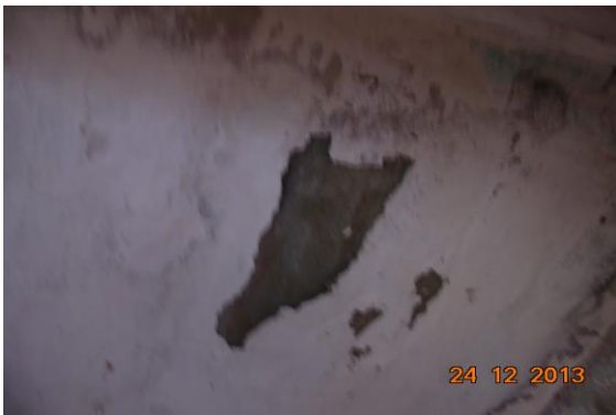
Photo 57 Dampness/Seepage on Roof of Toilet & Washroom of Third Floor
