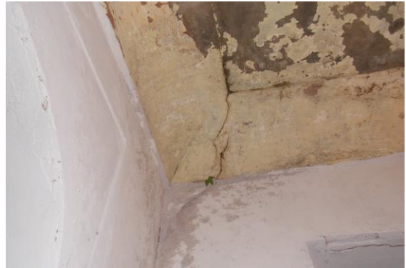
Photo 160 Peeling of Plaster on Roof of Varanda No.3 of Second Floor
