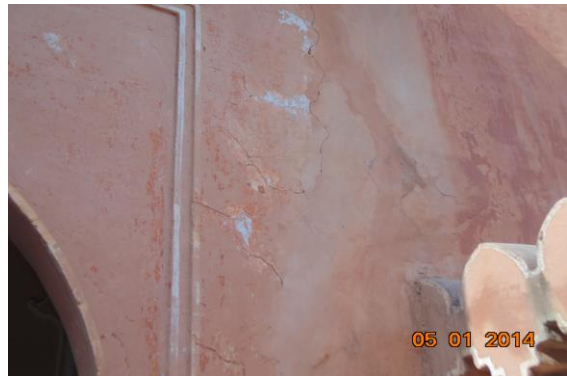
Photo 411 Plaster Crack on Wall No. 3 of Open Area 1 of Part B1 Second Floor
