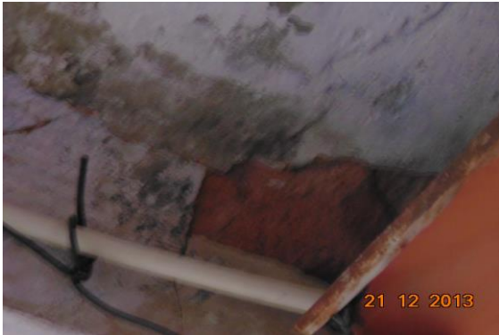
Photo 39 Peeling of Plaster on Roof of Varanda of shop of Ground Floor
