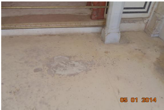
Photo 382 Peeling of Plaster on Floor of Room No. 4 of Part B1 First Floor
