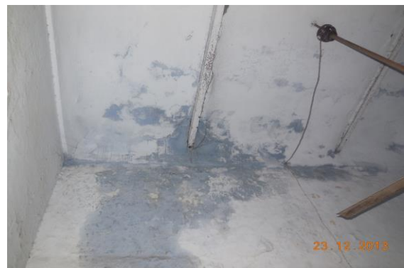
Photo 110 Dampness/Seepage on Wall No. 2, 4 & Roof of Room No. 1 (Part B) of Second Floor
