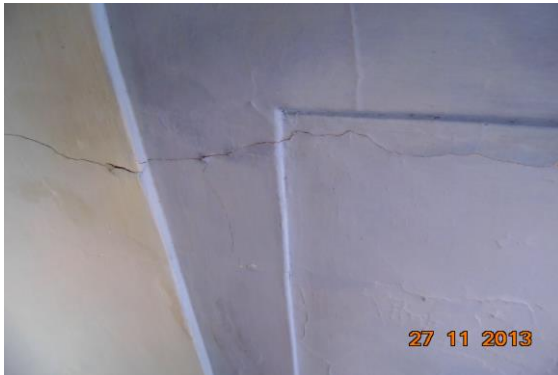
Photo 19 Inclined Crack on Roof of Bsnl Office , First Floor Approx. Width = 1mm, Approx. Length = 2.2m. Distance from Wall No. 1 = 0.45m, Height from Floor = 2.1m.
