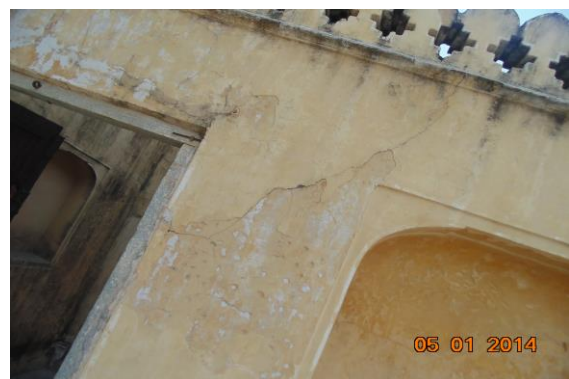
Photo 397 Plaster Crack on Wall No. 2 of Open Area 3 of Part B1 First Floor
