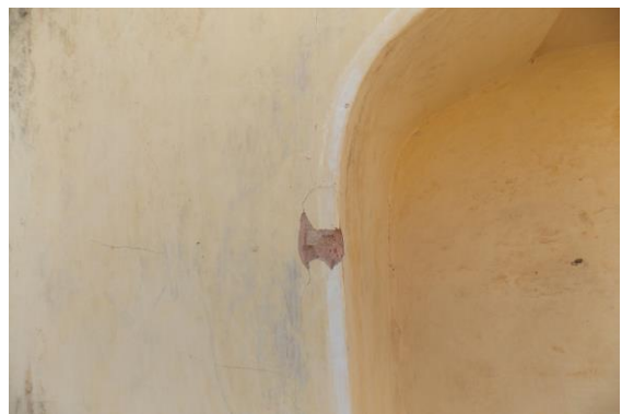
Photo 289 Peeling of Plaster on Wall No. 2 of Open Area 6 of Terrace of (A2+B2) Open Area
