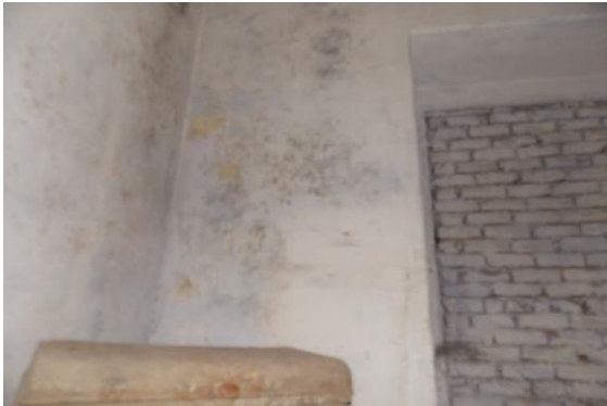
Photo 125 Dampness/Seepage on Wall No. 4 of Varanda of Second Floor
