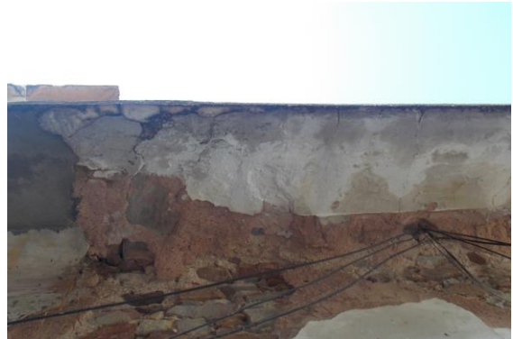
Photo 294 Peeling of Plaster on Wall No. 4 of Sun Shade, Open sky of Ground Floor
