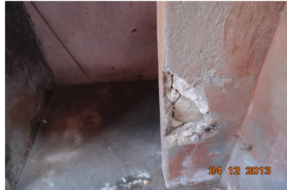
Photo 56 Damaged Portion on Outer Wall No.3 of Toilet & Washroom of Third Floor
