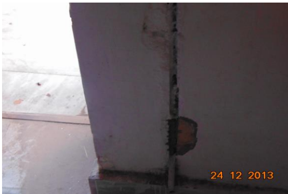
Photo 51 Peeling of Plaster on Wall No. 3 of Kitchen of First Floor
