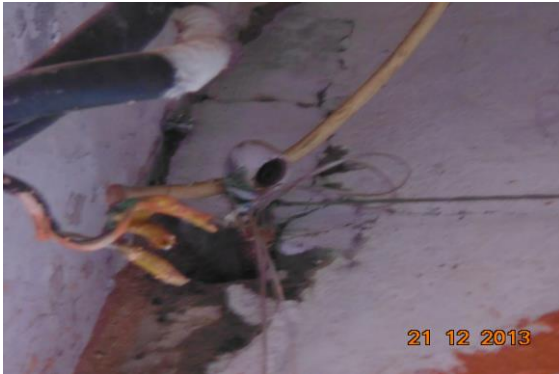
Photo 53 Peeling of Plaster on Right side External column of Varanda of shop of Ground Floor
