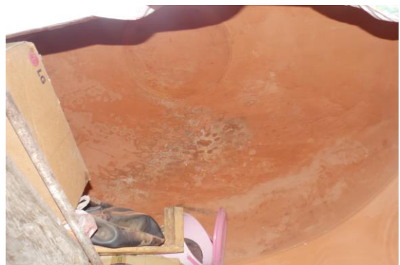
Photo 158 Dampness/Seepage on Roof of Tomb No.3 of Second Floor
