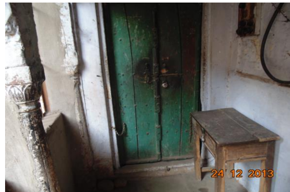
Photo 27 Peeling of Plaster on Wall No. 1 & Main Gate of Shahid Amit Bhardwaj School of Ground Floor
