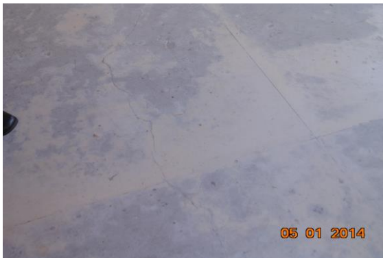
Photo 394 Plaster Crack on Floor of Room No. 2 of Part B1 First Floor
