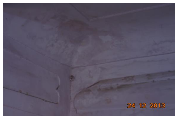
Photo 54 Dampness/Seepage on Wall No. 1, 4 & Roof of Room No. 1 of Temple Shri Chandra Vihari Ji, First Floor
