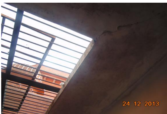
Photo 47 Dampness/Seepage on Wall No. 2 of Open Sky of First Floor
