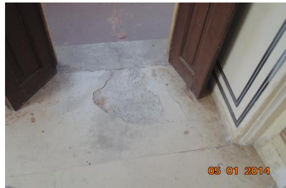
Photo 383 Peeling of Plaster on Floor of Room No. 4 of Part B1 First Floor
