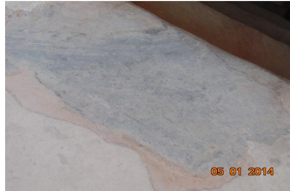
Photo 441 Peeling of Plaster on Floor of Passage 1 of Part B1 4th Floor
