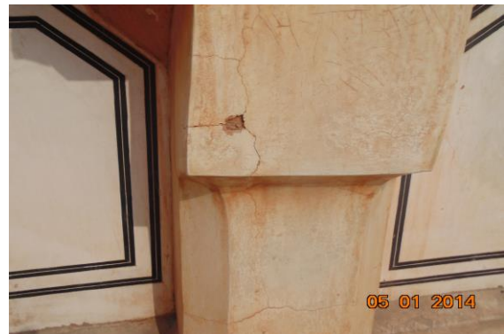
Photo 395 Plaster Crack on Wall No. 4 of Open Area 5 of Part B1 First Floor
