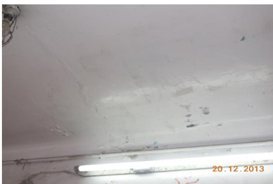
Photo 76 Peeling of Plaster on Roof of Varanda of Shop no. 9, Ground Floor
