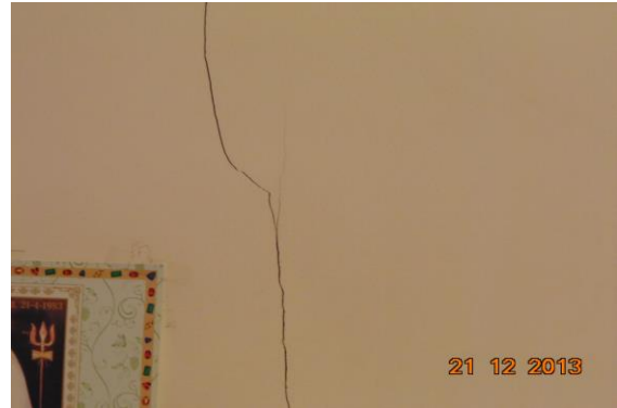
Photo 26 Horizontal Crack on Wall No. 2 of Shop no.20, Ground floor Approx. Width = 2mm, Approx. Length = 3m. Distance from Wall no.3 = 2m, Height from Floor = 0m.
