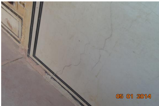
Photo 412 Plaster Crack on Wall No. 2 of Vranda 1 of Part B1 Second Floor
