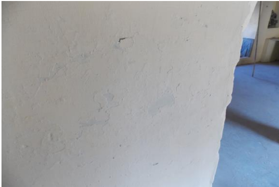
Photo 245 Peeling of Plaster on Wall No. 1 of Passage No.5 of First Floor
