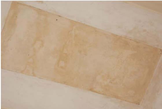
Photo 220 Dampness/Seepage on Roof of Gallery 8 of Part A2 Upper Ground Floor
