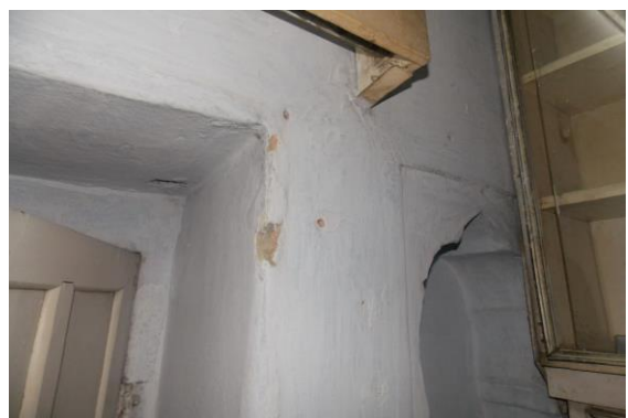
Photo 254 Peeling of Plaster on Wall No. 3 of Hall No. 1 of Part B - Temple Shri Anand Bihari Ji, First Floor
