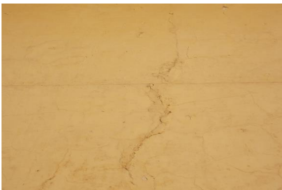
Photo 300 Plaster Crack on Wall No. 3 of Outer wall of Upper Ground Floor
