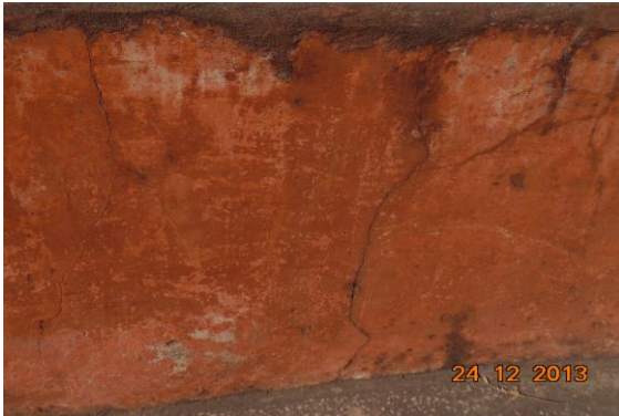
Photo 55 Peeling of Plaster on Parapet Wall of Second Floor
