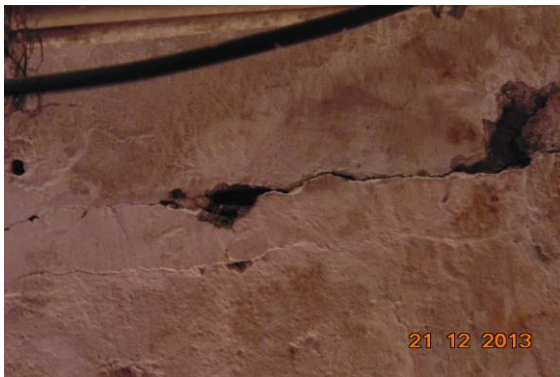
Photo 15 Horizontal Crack on Roof of Varanda of shop, Ground floor Approx. Width = 3mm, Approx. Length = 2.5m. Distance from Rightside External Column = 0m, Height from Floor = 3m.
