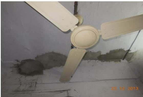
Photo 85 Peeling of Plaster on Roof of Room No. 8 of Ground Floor
