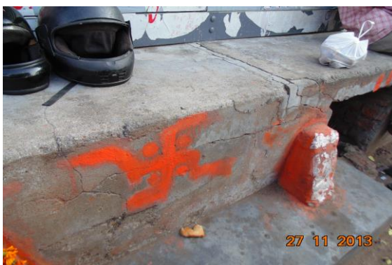
Photo 5 Peeling of Plaster on Platform of Transformer of Ground Floor
