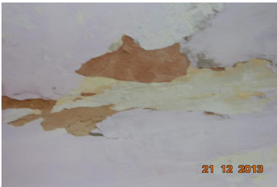
Photo 41 Peeling of Plaster on Roof of Part A of shop no.13 of Ground Floor
