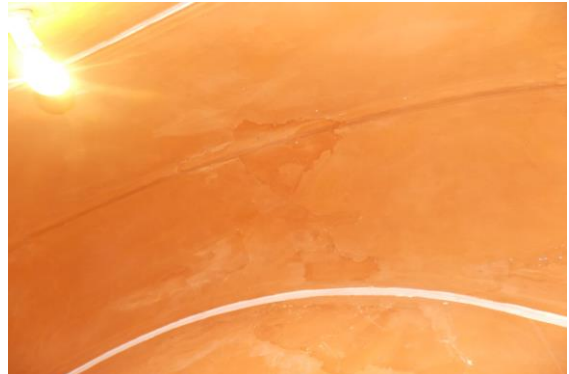
Photo 162 Peeling of Plaster on Roof of Toilet & Washroom of Second Floor
