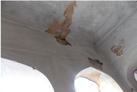
Photo 275 Peeling of Plaster on Wall No. 3 & Roof of Varanda No.2 of Ground Floor
