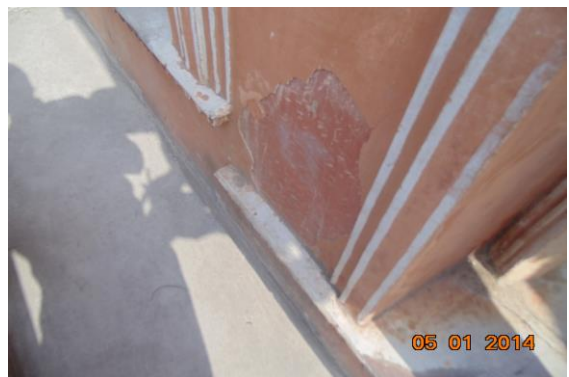
Photo 427 Peeling of Plaster on Wall No. 1 of Passage 2 of Part B1 Third Floor
