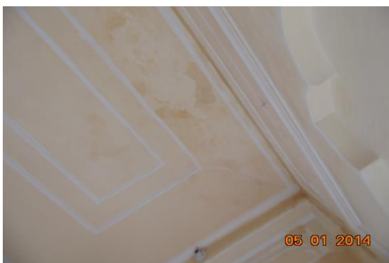
Photo 390 Dampness/Seepage on Roof of Vrandra 1 of Part B1 First Floor
