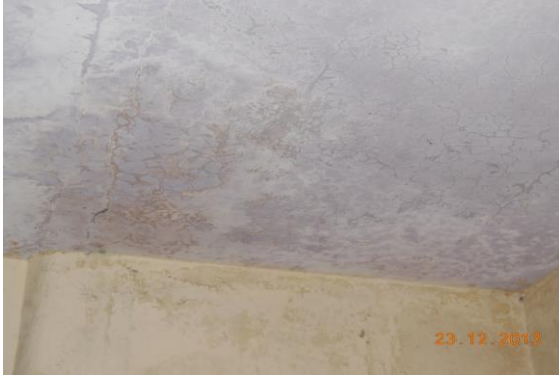
Photo 75 Dampness/Seepage on Roof of Lock Up Room of Ground Floor
