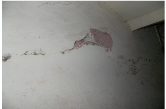
Photo 174 Peeling of Plaster on Wall No. 2 of Staircase First Floor To Second Floor of Second Floor
