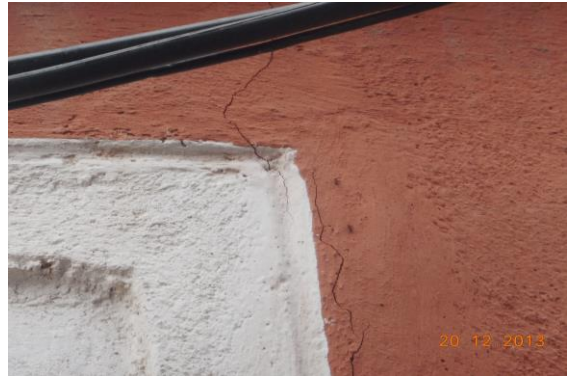
Photo 38 Inclined Crack on External Column Rightside of Varanda, Shop no.2, Ground Floor Approx. Width = 0.2mm, Approx. Length = 0.2m. Distance from External Column Left side = 2.5m, Height from Floor = 3.5m.
