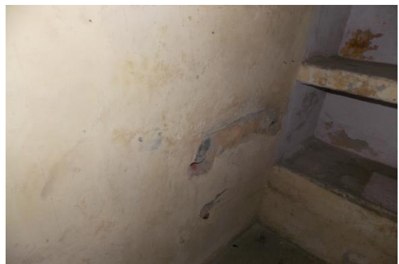
Photo 146 Peeling of Plaster on Wall No. 1 of Room No. 1 of Second Floor
