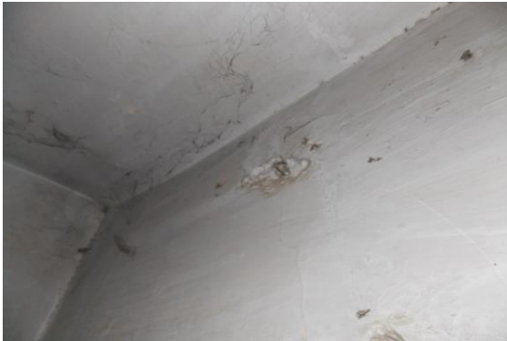
Photo 249 Peeling of Plaster on Wall No. 3 of Passage No.7 of First Floor
