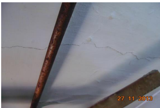
Photo 22 Inclined Crack on Roof of Bsnl Office 2 , First Floor Approx. Width = 0.8mm, Approx. Length = 3m. Distance from Wall No.4 = 0m, Height from Floor = 2.25m.
