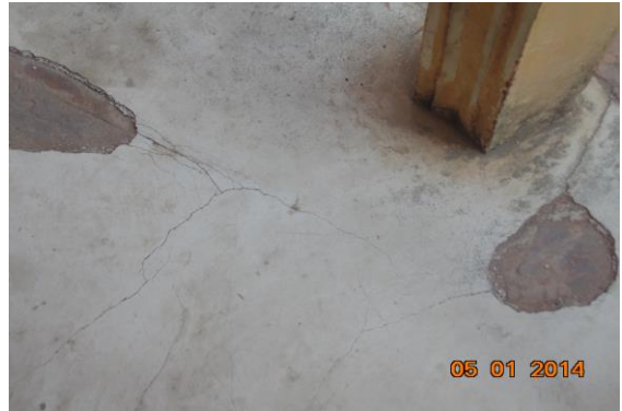
Photo 423 Peeling of Plaster on Floor of Tomb 5 of Part B1 Third Floor
