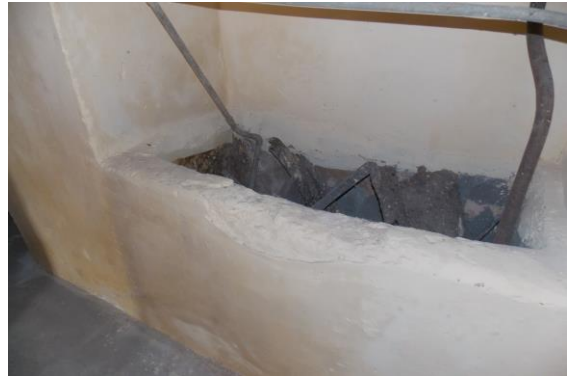
Photo 246 Peeling of Plaster on Wall No. 1 of Hall No. 5 of Temple Shri Anand Bihari Ji, First Floor
