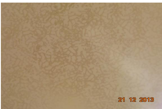
Photo 61 Dampness/Seepage on Roof of Shop no.20 of Ground floor
