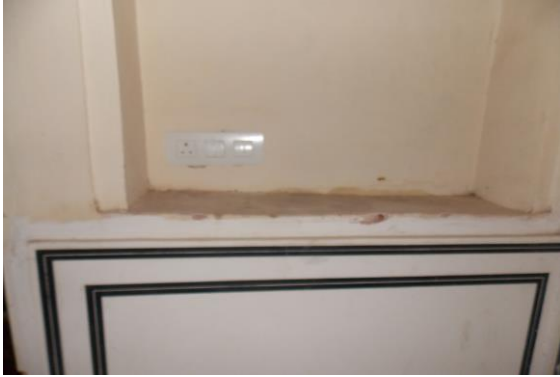
Photo 200 Peeling of Plaster on Wall No. 3 of Open Area 2 of Part A2 Upper Ground Floor
