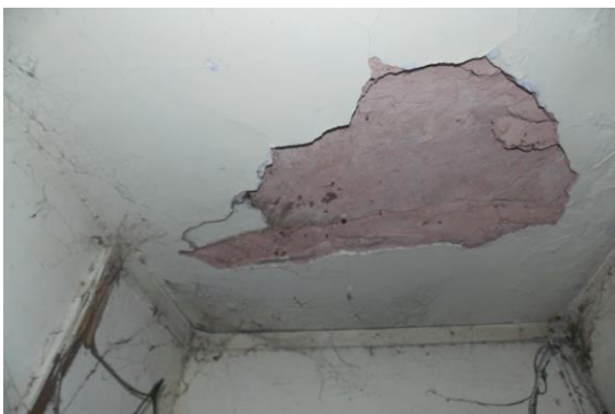
Photo 175 Peeling of Plaster on Roof of Staircase First Floor To Second Floor of Second Floor
