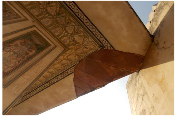
Photo 285 Dampness/Seepage on Sunshade of Tomb 1 of Terrace of (A2+B2) Open Area
