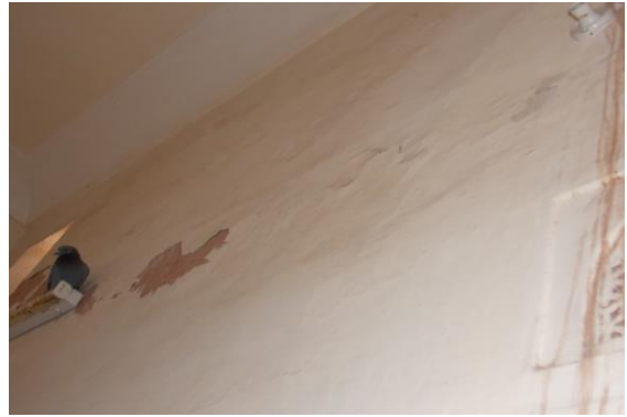
Photo 219 Peeling of Plaster on Wall No. 2 of Gallery 8 of Part A2 Upper Ground Floor
