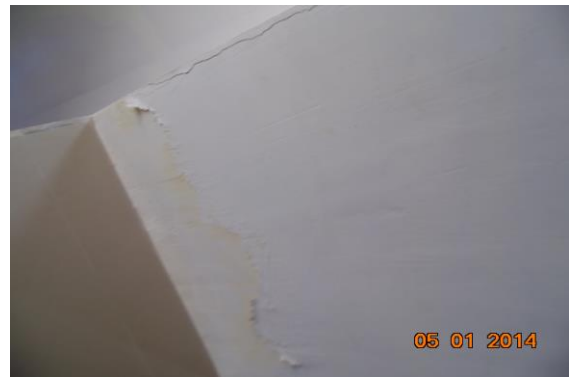
Photo 443 Dampness/Seepage on Wall No. Roof & 3 of Toilet Vranda of Lower Ground Floor
