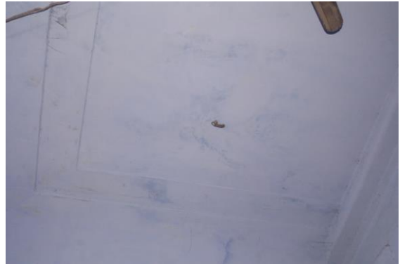
Photo 154 Dampness/Seepage on Roof of Room No. 6 of Second Floor
