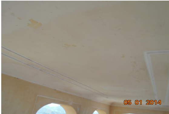
Photo 440 Dampness/Seepage on Roof of Passage 3 of Part B1 4th Floor
