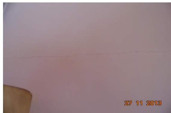
Photo 18 Horizontal Crack on Roof of Office , First Floor Approx. Width = 0.35mm, Approx. Length = 2.5m. Distance from Wall No. 2 = 1.8m, Height from Floor = 2.8m.
