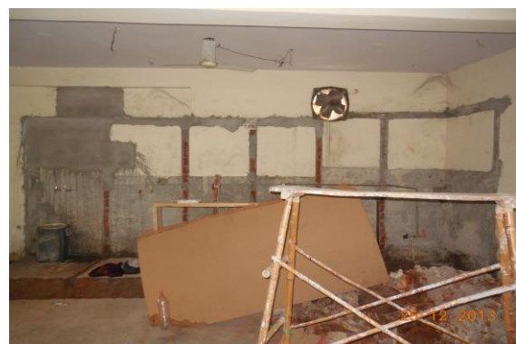
Photo 6 Peeling of Plaster on Wall No. 4 of Hall No. 1 of First floor
