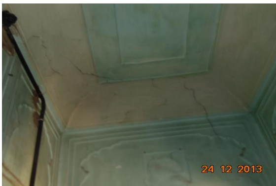
Photo 124 Peeling of Plaster on Wall No. 4 of Hall No. 8 (Part B) of Shahid Amit Bhardwaj School, First Floor
