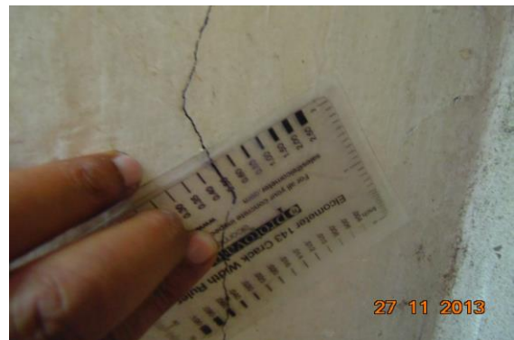
Photo 21A Inclined Crack on Wall No. 3 of Bsnl Office, First Floor Approx. Width = 0.5mm, Approx. Length = 1m. Distance from Wall No. 1 = 0m, Height from Floor = 0.4m.
