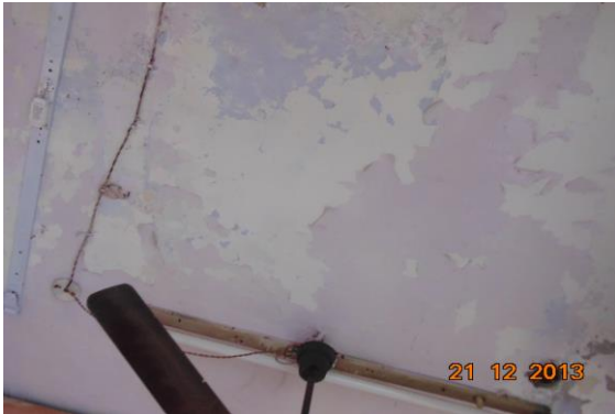
Photo 51 Dampness/Seepage on Roof of Varanda of shop of Ground Floor
