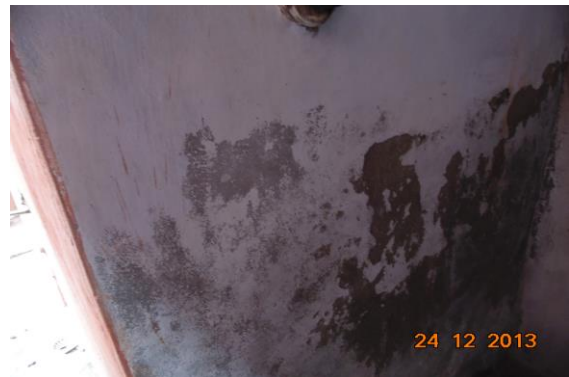
Photo 58 Dampness/Seepage on Wall No. 1 of Toilet & Washroom of Third Floor
