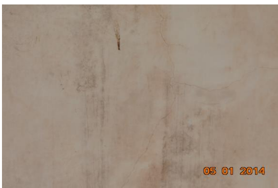
Photo 396 Plaster Crack on Wall No. 1 of Open Area 5 of Part B1 First Floor
