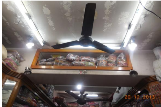
Photo 73 Peeling of Plaster on Roof of Shop No.6 of Ground Floor
