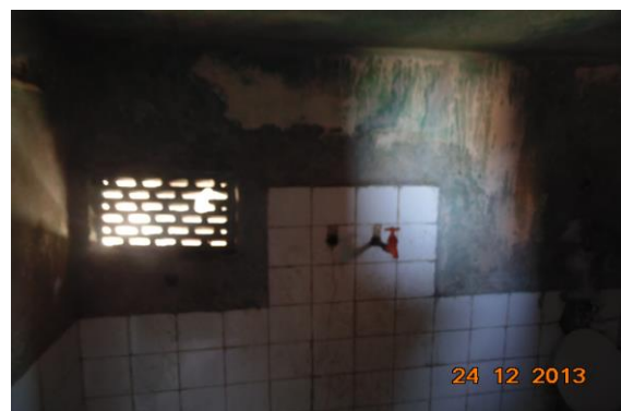
Photo 60 Dampness/Seepage on Wall No. 4 of Toilet & Washroom of Third Floor
