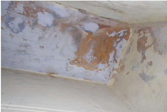
Photo 123 Dampness/Seepage on Roof of Varanda of Second Floor
