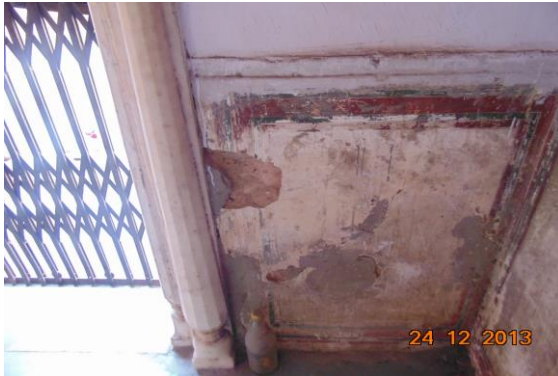
Photo 43 Peeling of Plaster on Wall No. 3 of Varanda of First Floor
