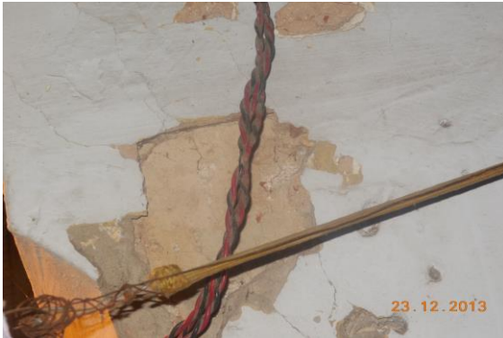
Photo 105 Peeling of Plaster on Wall No. 3 of Hall No. 1 of Second Floor
