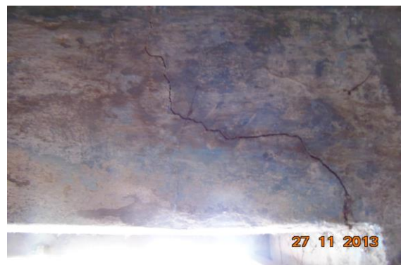
Photo 23 Inclined Crack on Wall No. 4 of Bathroom , First Floor Approx. Width = 2.5mm, Approx. Length = 0.5m. Distance from Wall No. 2 = 1.1m, Height from Floor = 1.6m.
