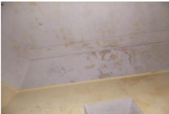
Photo 143 Dampness/Seepage on Roof of Room No. 2 of Second Floor
