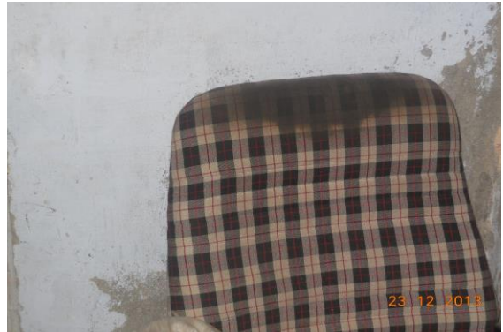
Photo 78 Peeling of Plaster on All Walls & Roof of Hall No. 1 of Ground Floor
