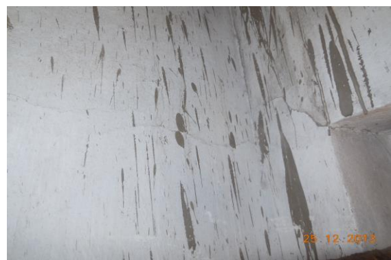
Photo 5 Horizontal Crack on Wall No. 1 of Room No. 1, Second Floor, Approx. Width = 0.4mm, Approx. Length = 0.4m. Distance from = Wall No.1 & 4 Cornern, Height from Floor = 1.8m.
