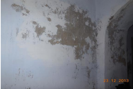
Photo 83 Dampness/Seepage on Wall No. 1 of Room No. 7 of Ground Floor
