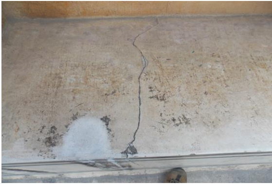
Photo 284 Plaster Crack on Wall No. 1 of Terrace of (A2+B2) Open Area
