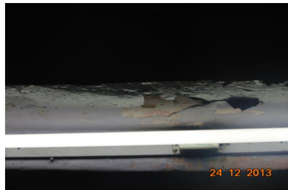
Photo 4 Peeling of Plaster on Roof of Shop Jagdish Narain Badri Prasad of Ground Floor
