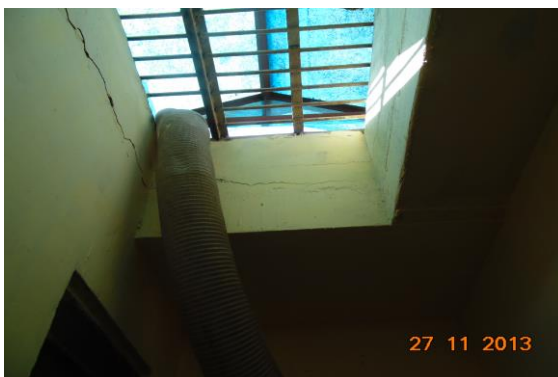
Photo 17 Horizontal Crack on Wall No. 1, 3 & 4 of Passage, First Floor Approx. Width = 4mm, Approx. Length = 4.5m. Distance from Wall No. 3 = 0m, Height from Floor = 3.2m.
