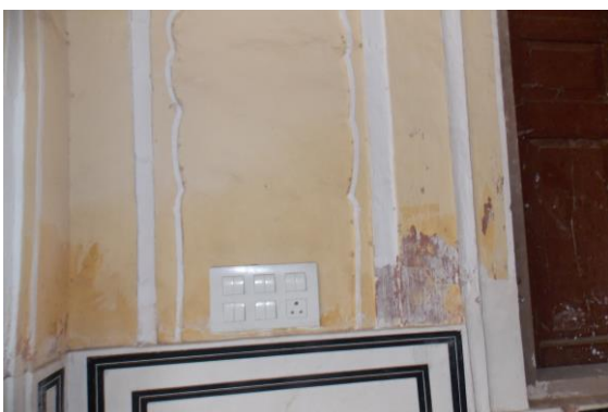
Photo 108 Peeling of Plaster on Wall No. 1 of Vrandha 4 of Part A1 Upper Ground Floor
