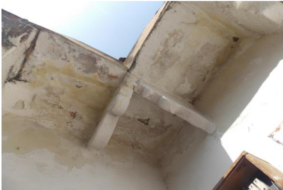
Photo 293 Peeling of Plaster on Sun Shade of Open sky of Ground Floor
