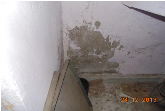
Photo 49 Peeling of Plaster on Wall No. 1 of Gallery No.2 of First Floor
