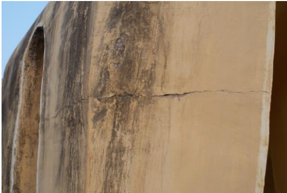
Photo 21 Horizontal Crack on of Minarate 1 L/S of Hawa Mahal , Part A1 Upper Ground Floor Approx. Width = 1mm, Approx. Length = 0.5m. Distance Wall No.1 of Gate = 0.7m, Height from Floor = 1m.
