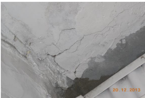
Photo 41 Inclined Crack on Roof of Varanda, Shop no.2, Ground Floor Approx. Width = 4mm, Approx. Length = 0.5m.
