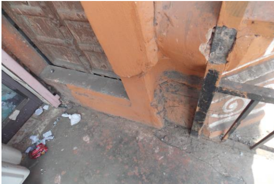
Photo 452 Peeling of Plaster
