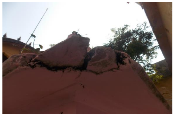
Photo 296 Damaged Portion on Sun Shade of Part B of Temple Shri Anand Bihari Ji of Ground Floor
