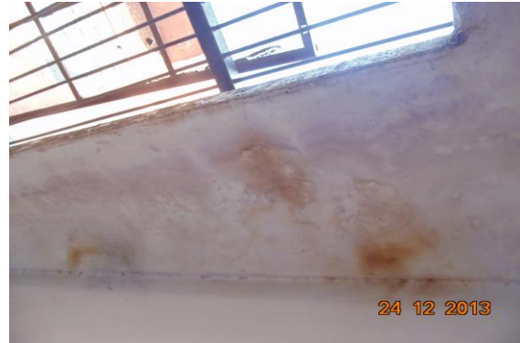
Photo 44 Dampness/Seepage on Wall No. 4 & Shade of Open Sky of First Floor
