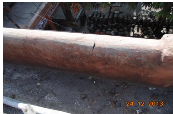
Photo 16 Inclined Crack on Wall No. 2 of Second Floor, Approx. Width = 0.6mm, Approx. Length = 1m. Distance from Wall No. 3 = 3.1m, Height from Floor = 0m.
