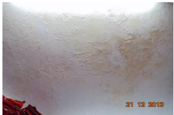
Photo 44 Dampness/Seepage on Roof of Part c of shop no.12 of Ground Floor
