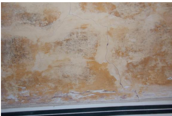
Photo 96 Peeling of Plaster on Wall No. 4 of Room No. 10 of Part A1 Upper Ground Floor
