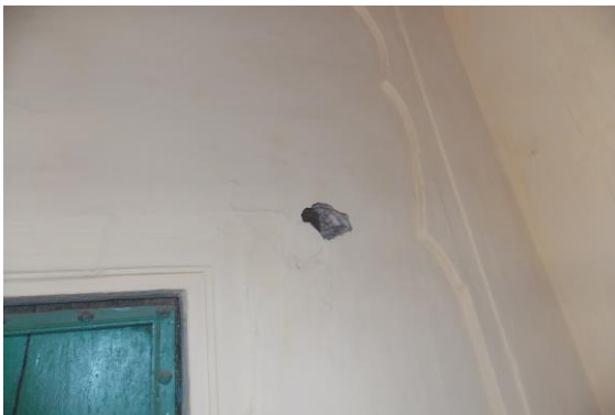
Photo 239 Peeling of Plaster on Wall No. 1 of Varanda No.3 of First Floor
