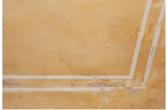
Photo 93 Dampness/Seepage on Roof of Room No. 4 of Part A1 Upper Ground Floor
