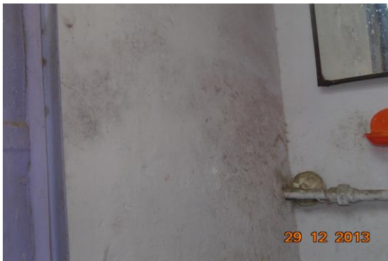
Photo 20 Dampness/Seepage on Wall No. 1 of Toilet No. 1 of House No. 339, Third Floor
