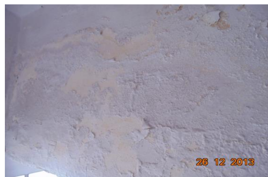
Photo 39 Dampness/Seepage on Wall No. 1 of Staircase SF to TF of Second Floor
