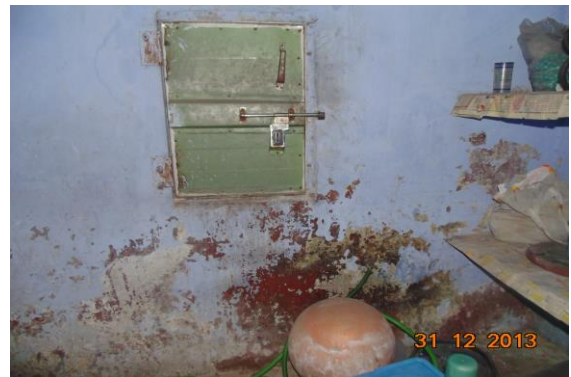
Photo 21 Peeling of Plaster on Wall No. 4 of Bathroom of First Floor
