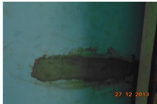
Photo 35 Damaged Portion on Wall No. 1 of Room No. 2 of Second Floor
