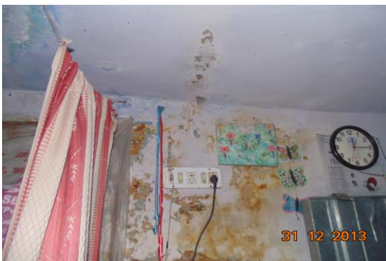
Photo 33 Dampness/Seepage on Wall No. 4 & Roof of Room No. 2 of Second Floor
