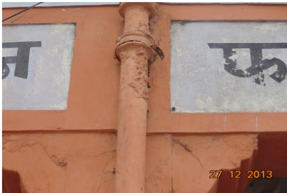
Photo 100 Peeling of Plaster on Roof & Wall No.1 of Third Floor
