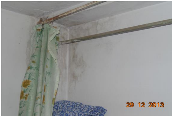
Photo 18 Dampness/Seepage on Wall No. 2 & 4 of Third Floor
