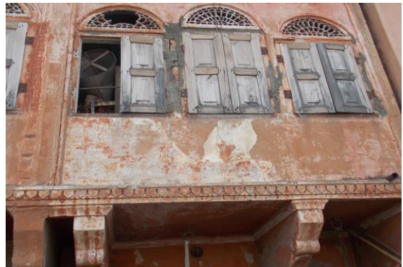
Photo 56 Peeling of Plaster
