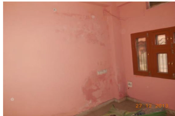
Photo 98 Dampness/Seepage on Wall No. 4 & 2 of Room No. 2 of Second Floor
