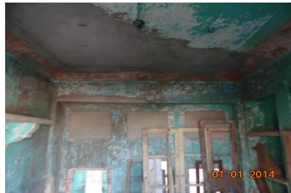
Photo 127 Dampness/Seepage on Wall No. 3 of Third Floor
