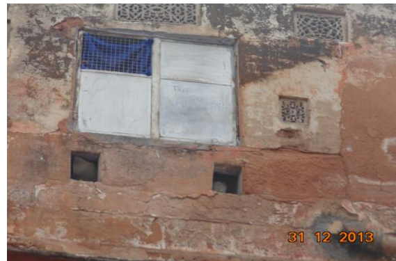
Photo 56 Dampness/Seepage on Outer Wall of Third Floor
