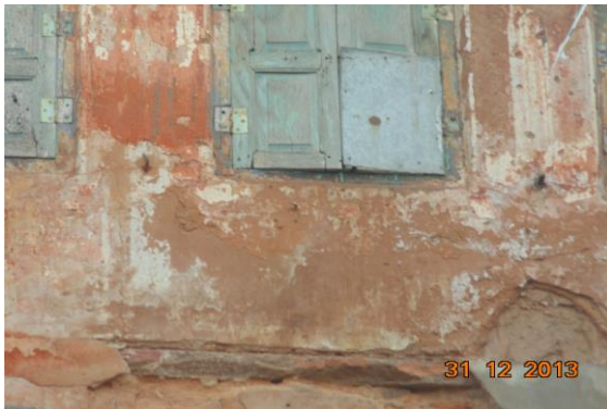
Photo 53 Peeling of Plaster on Outer Wall of Second Floor
