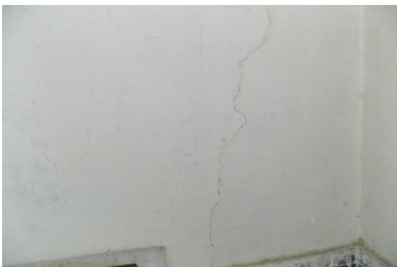
Photo 183 Plaster Crack on Wall No. 2 of Varanda 10 of Navjeevan Chikitsalaya of First Floor
