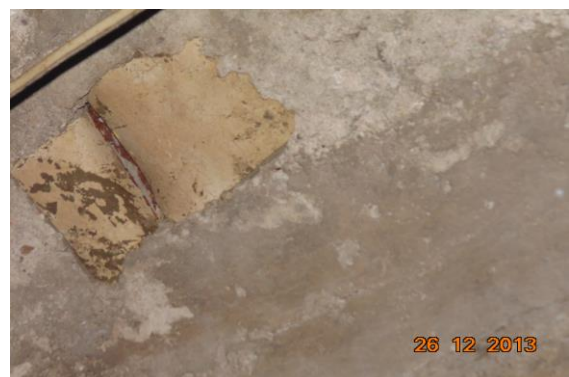
Photo 39 Dampness/Seepage on Roof of Room No. 2 of Fourth Floor
