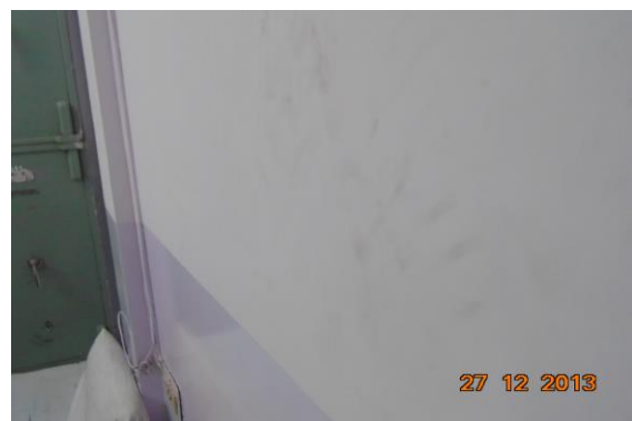
Photo 6 Dampness/Seepage on Wall No. 1 of Shop of Ground Floor
