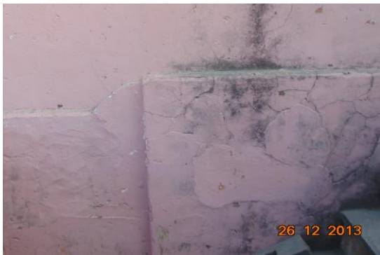
Photo 17 Damaged Portion on Wall No. 3 of Open Sky of External Façade
