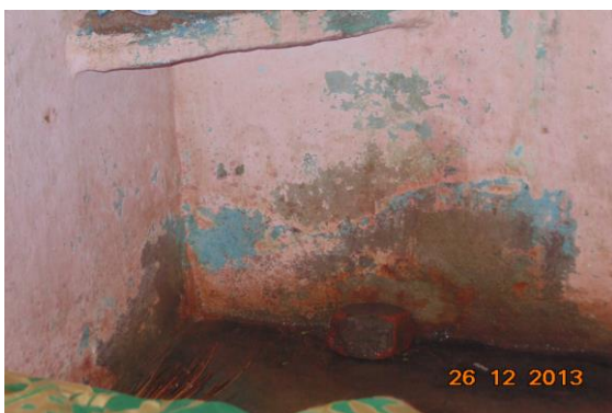
Photo 38 Dampness/Seepage on Wall No. 1 & 4 of Room No. 1 of Fourth Floor
