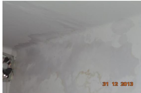
Photo 8 Dampness/Seepage on Hall No. 1 of Third Floor
