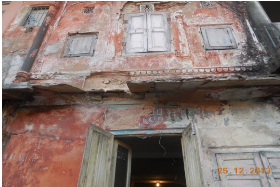
Photo 26 Peeling of Plaster on Shade of Part-II of First Floor
