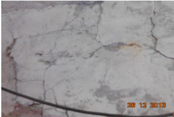
Photo 10 Inclined Crack on front side of Staircase GF to FF, Ground Floor, Approx. Width = 2mm, Approx. Length = 1m. , Height from Floor = m.
