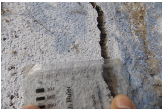
Photo 9A Inclined Crack on Wall No. 3 of Hall No. 1, Second Floor Approx. Width = 8mm, Approx. Length = 1.6m. Distance from Wall no.2 = 0.7m, Height from Floor = 1m.
