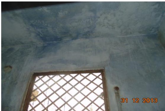
Photo 26 Dampness/Seepage on Wall No. 4 & Roof of Toilet No. 1 of Fifth Floor
