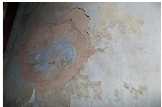
Photo 37 Peeling of Plaster on Wall No. 2 of Staircase FF to SF
