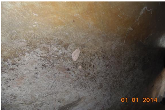
Photo 90 Peeling of Plaster on Wall No. 4 of Third Floor
