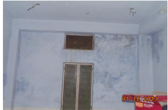
Photo 25 Dampness/Seepage on Wall No. 1, 4 & 2 of Room No. 2 of Third Floor
