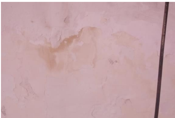
Photo 22 Peeling of Plaster on Roof of Varanda of Ground Floor
