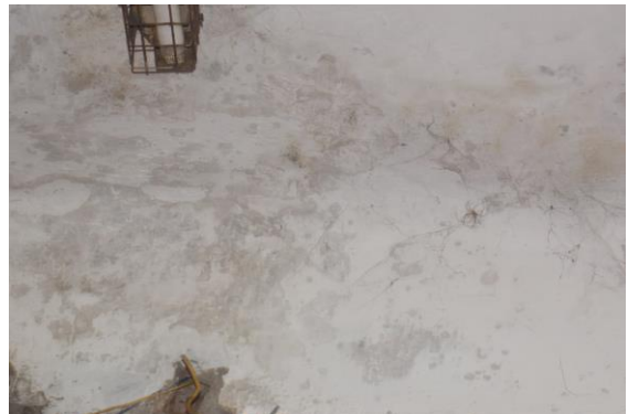
Photo 62 Dampness/Seepage on Beam of Varanda of Shop No.75 of Ground Floor
