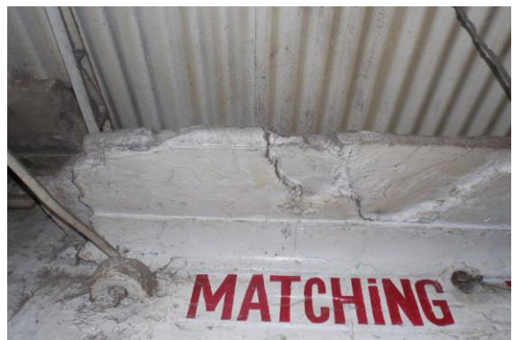
Photo 12 Damaged Portion on Wall No. 3 & Sunshade of Shop No.1 of Ground Floor
