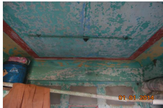
Photo 121 Dampness/Seepage of Third Floor
