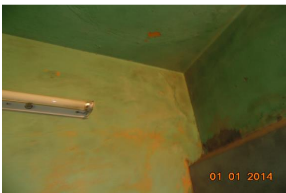
Photo 116 Dampness/Seepage on Wall No. 4 of Third Floor
