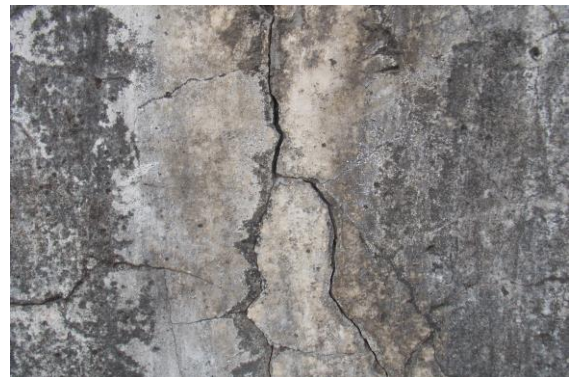
Photo 4 Inclined Crack on Wall No. 4 of Open Area, Third Floor, Approx. Width = 4mm, Approx. Length = 2m. Distance from Wall No. 2 = 0.2m, Height from Floor = 0m.
