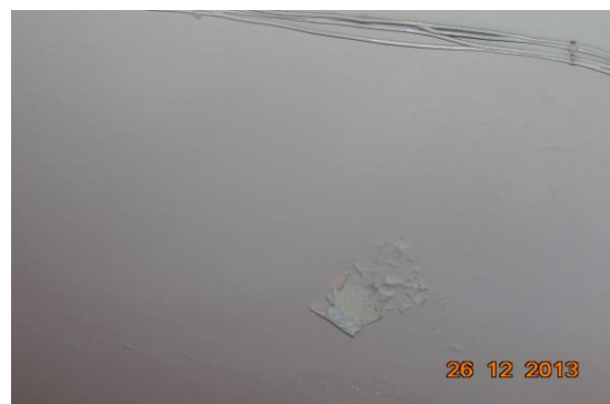
Photo 22 Peeling of Plaster on Roof of Room No. 1 of External Façade
