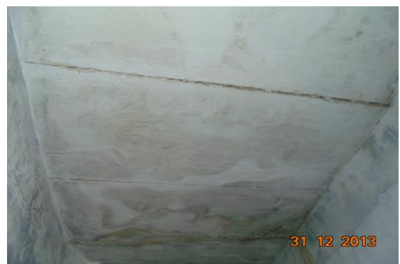
Photo 29 Dampness/Seepage on Roof of Stair 5Th Floor To Terrace
