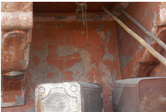
Photo 57 Peeling of Plaster on Outside Wall of External Façade
