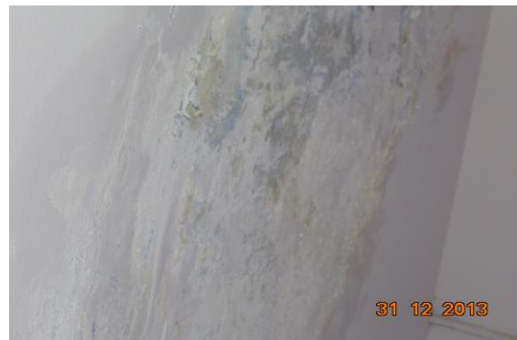
Photo 10 Dampness/Seepage on Wall No. 1 of Hall No. 1 of Fourth Floor
