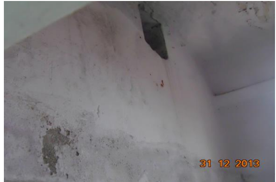
Photo 14 Dampness/Seepage on Wall No. 1 of Toilet No. 1 of Third Floor
