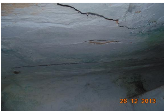
Photo 5 Inclined Crack on Roof of Toilet No. 1, First Floor, Approx. Width = 3mm, Approx. Length = 1m, Height from Floor = m.
