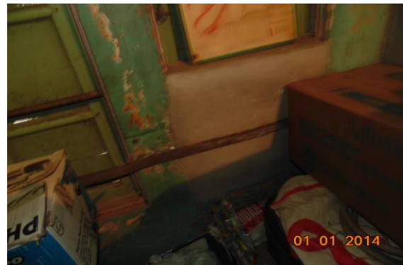
Photo 115 Peeling of Plaster on Wall No. 4 of Third Floor
