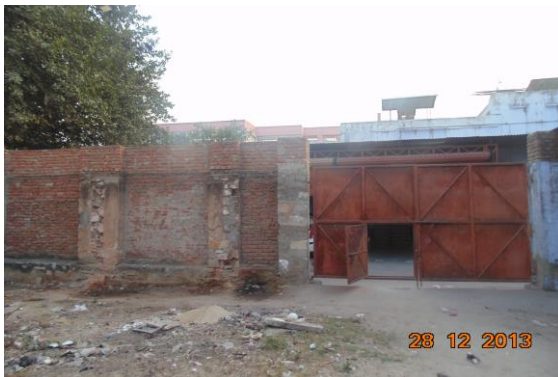
Photo 3 Peeling of Plaster on Wall No. 3 of Open Sky of House No. 61 of Ground Floor
