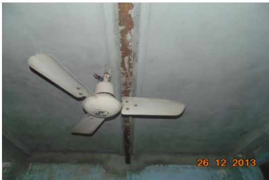
Photo 34 Peeling of Plaster on Roof of Room No. 2 of Third Floor
