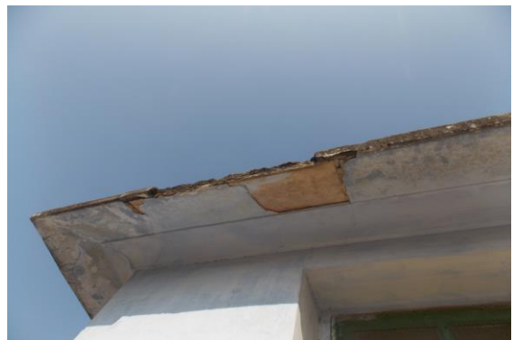
Photo 80 Peeling of Plaster on Wall No. 8 & Sun Shade of Open Sky of Second Floor
