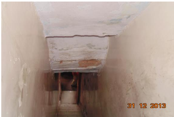
Photo 33 Dampness/Seepage on Wall No. 1, 2 & Roof of Stair GF to FF of Third Floor
