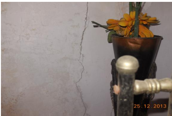
Photo 3A Inclined Crack on Wall No. 4 of Room No. 2, First Floor Approx. Width = 1mm, Approx. Length = 2m. Distance from Wall No.2 = 0.3m, Height from Floor = 0m.
