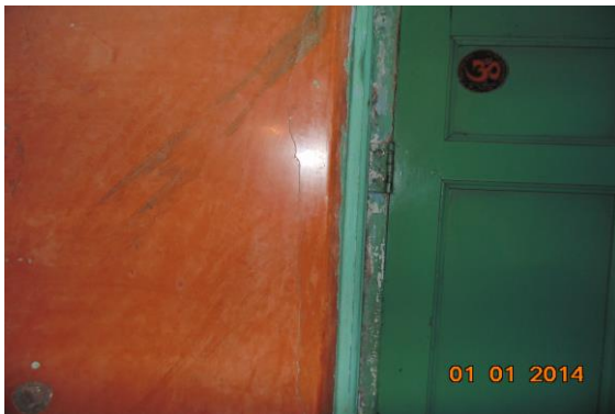
Photo 78 Plaster Crack on Wall No. 4 of Second Floor
