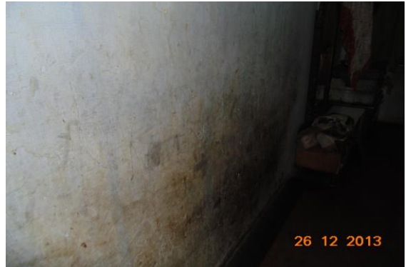
Photo 16 Dampness/Seepage on Wall No. 4 of Room No. 1 of Third Floor
