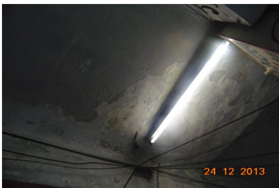
Photo 5 Dampness/Seepage on Roof of Varanda of Shop No.21 of Ground Floor
