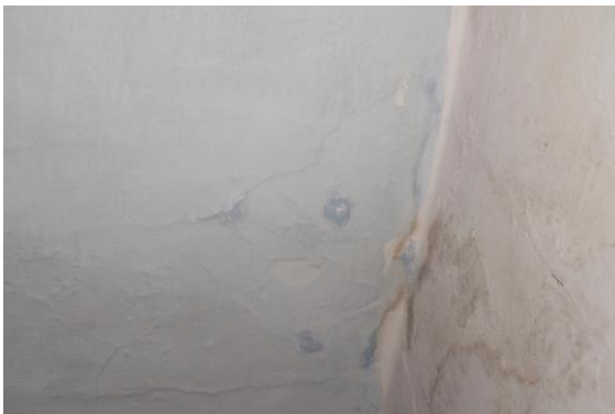
Photo 16 Dampness/Seepage on Roof of Staircase SF to TF of Second Floor
