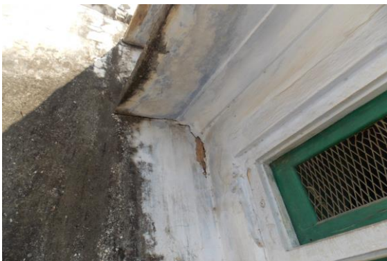
Photo 73 Peeling of Plaster on Wall No. 3 of Open Sky of Second Floor
