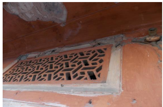
Photo 45 Peeling of Plaster on Wall No. 3 of Balcony of Second Floor
