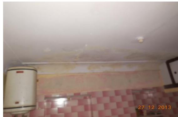
Photo 74 Dampness/Seepage on Wall No. 4 & Roof of Bathroom No. of Second Floor
