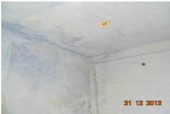
Photo 32 Dampness/Seepage on Wall No. 1, 4 & Roof of Room No. 1 of Terrace
