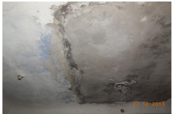
Photo 56 Damaged Portion on Roof of Varanda of Ground Floor
