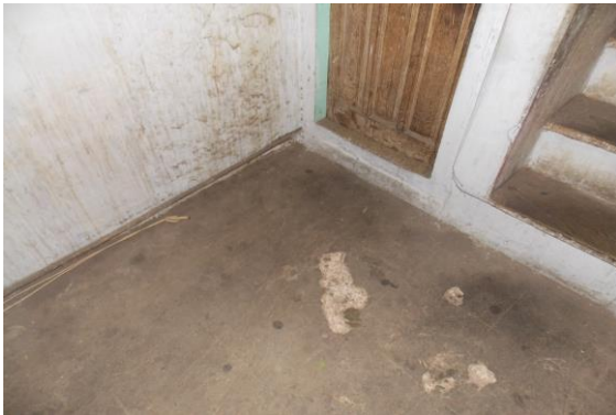
Photo 29 Peeling of Plaster on Floor of Lobby of First Floor
