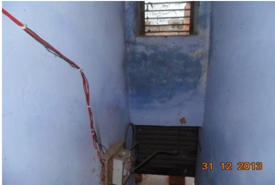
Photo 24 Dampness/Seepage on Wall No. 3 of Stair GF to FF
