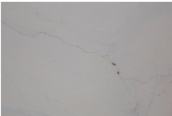
Photo 17 Inclined Crack on Wall No. 4 & Roof of Room No. 2, First Floor Approx. Width = 0.6mm, Approx. Length = 3m. Distance from Wall No.1 = 0.4m, Height from Floor = 2.5m.
