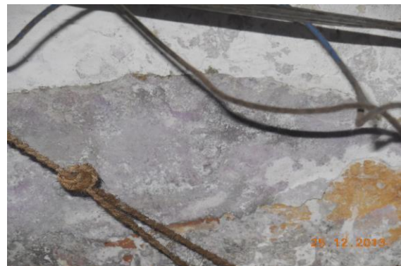
Photo 4 Horizontal Crack on Backside & Leftside External Column of Shop No.31, Ground Floor Approx. Width = 0.5mm, Approx. Length = 2m. Distance from Leftside External Column = Backside Height from Floor
