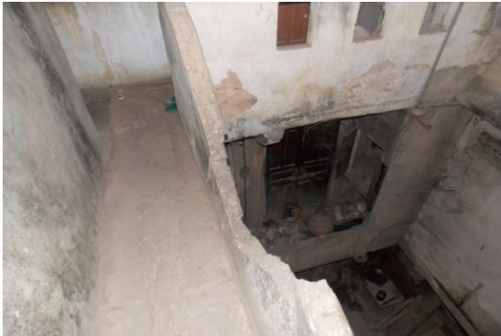
Photo 61 Peeling of Plaster on Wall No. 3 of Balcony of Second Floor
