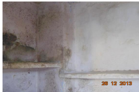
Photo 11 Horizontal Crack on Roof of Varanda of Shop No. 35, Ground Floor Approx. Width = 3mm, Approx. Length = 2.5m. Distance from Right side External Column = 0m, Height from Floor = 3m.
