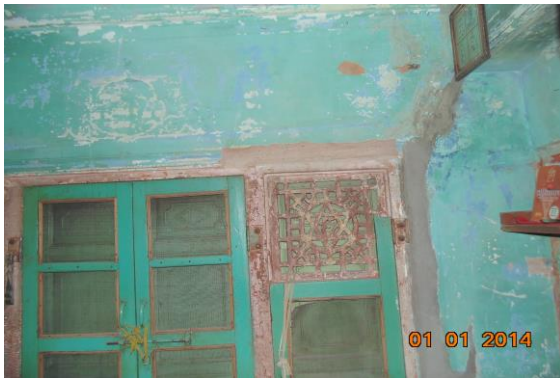
Photo 76 Peeling of Plaster on Wall No. 1 of Second Floor
