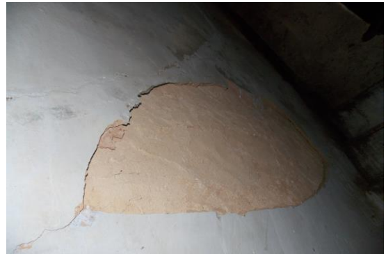
Photo 35 Peeling of Plaster on Wall No. 1 of Staircase FF to SF
