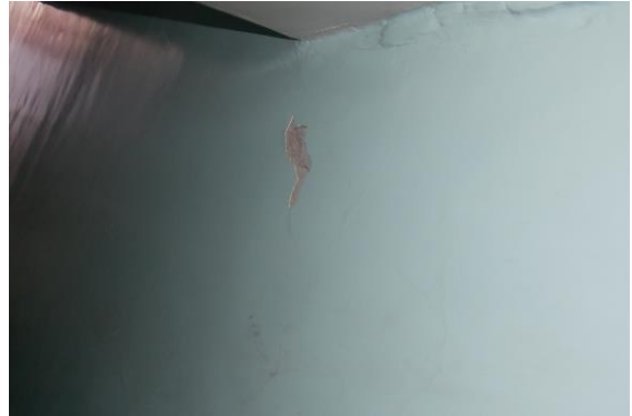
Photo 8 Peeling of Plaster on Wall No. 1 of Staircase GF to FF
