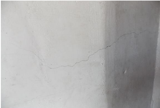
Photo 14 Peeling of Plaster on Wall No. 2 of Lobby of Second Floor
