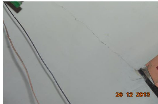
Photo 21 Horizontal Crack on Roof of Varanda, Shop No.57, Ground Floor Approx. Width = 1mm, Approx. Length = 2.5m. Distance from Left side External Column = 0m, Height from Floor = 3m.
