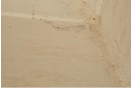
Photo 179 Peeling of Plaster on Wall No. 1 of Varanda 11 of Navjeevan Chikitsalaya of First Floor
