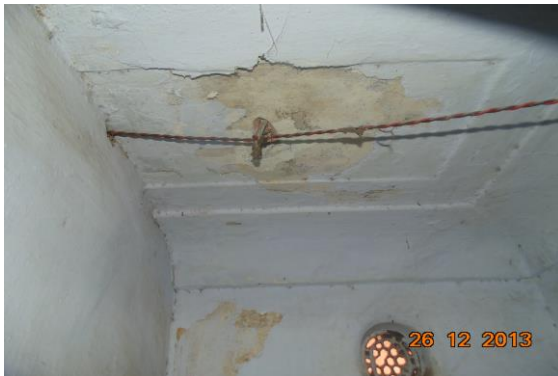
Photo 19 Peeling of Plaster on Roof of Passage of First Floor
