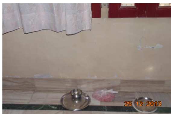
Photo 111 Peeling of Plaster on Wall No. 4 of Hall No. 1 of House No. 347 Part A, Second Floor
