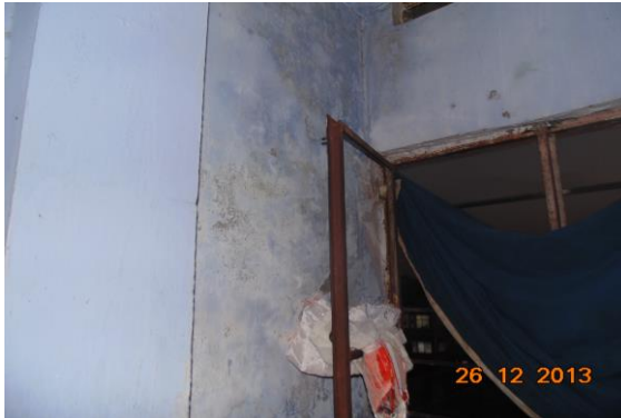
Photo 25 Dampness/Seepage on Wall No. 1 of Kitchen of Fourth Floor
