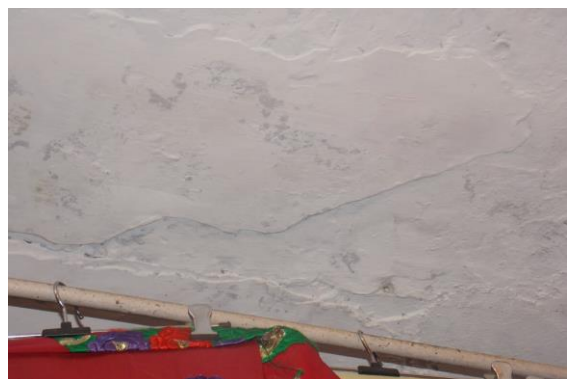
Photo 28 Peeling of Plaster on Roof of Varanda of Shop No.77 of Ground Floor
