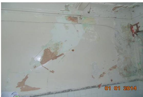
Photo 38 Dampness/Seepage on Wall No. 1 of Room No. 1 of First Floor
