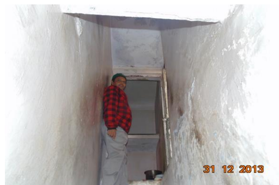
Photo 18 Peeling of Plaster on Wall No. 1, 2 & Roof of Stair SF to TF of Second Floor
