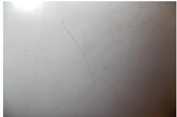
Photo 4 Inclined Crack on Wall No. 1 of Staircase FF to SF
