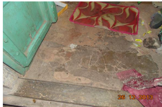
Photo 22 Peeling of Plaster on Wall No. Floor of Kitchen of First Floor
