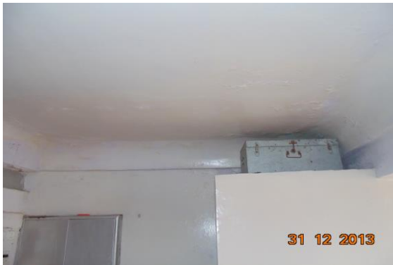
Photo 41 Dampness/Seepage on Wall No. 5 & Roof of Lobby of First Floor
