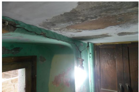
Photo 28 Peeling of Plaster on Wall No. 1, 4 & Roof of Kitchen of First Floor
