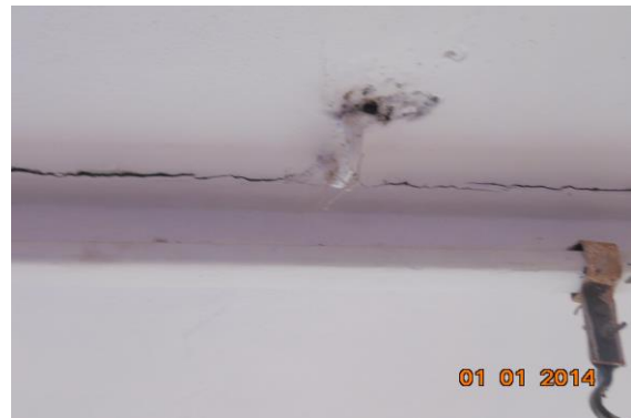
Photo 49 Plaster Crack on Roof of First Floor
