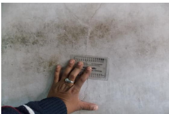
Photo 4A Inclined Crack on Wall No. 2 of Shop No. 84, Ground Floor Approx. Width = 0.3mm, Approx. Length = 2m. Distance from Wall No. 3 = 1.2m, Height from Floor = 0m.
