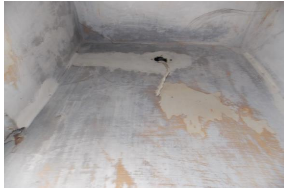
Photo 12 Peeling of Plaster on Roof & 4 of Stair SF to TF of Third Floor
