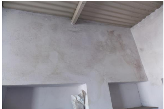
Photo 19 Dampness/Seepage on Wall No. 4 of Room No. 1 of Second Floor
