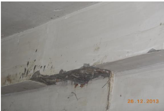
Photo 154 Peeling of Plaster on Wall No. 2 of Shop No. F 1 of First Floor
