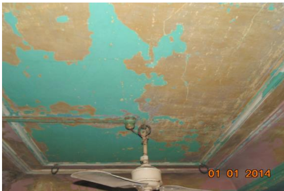
Photo 66 Dampness/Seepage on Roof of Second Floor
