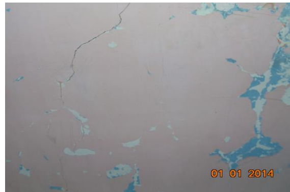
Photo 73 Peeling of Plaster on Roof of Hall No. 1 of Second Floor
