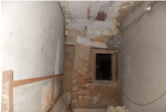
Photo 85 Peeling of Plaster on Wall No. 4 of Shop of Ground Floor
