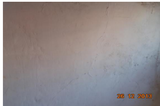
Photo 19 Inclined Crack on Wall No. 2 of Staircase GF to FF, Ground Floor Approx. Width = 0.3mm, Approx. Length = 2m.
