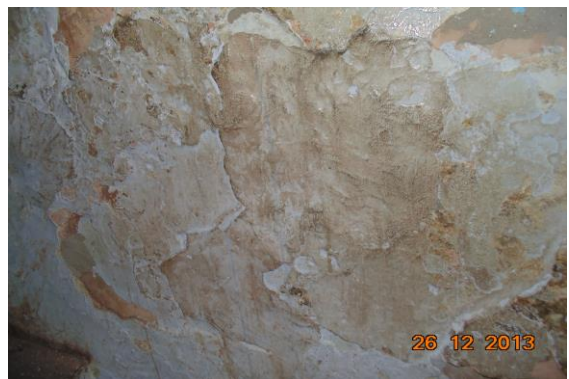
Photo 45 Peeling of Plaster on Wall No. 2 of Staircase GF to FF of Ground Floor
