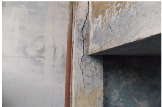
Photo 9 Inclined Crack on Wall No. 3 of Hall No. 1, Second Floor Approx. Width = 8mm, Approx. Length = 1.6m. Distance from Wall no.2 = 0.7m, Height from Floor = 1m.
