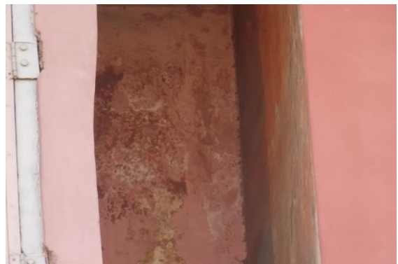
Photo 23 Dampness/Seepage on Frontwall of Building of First Floor
