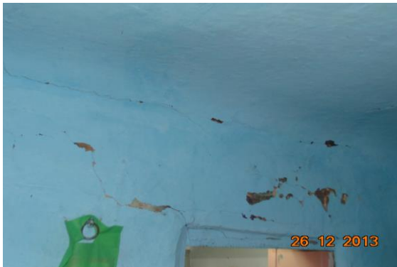
Photo 34 Peeling of Plaster on Wall No. 1 of Lobby of Third Floor
