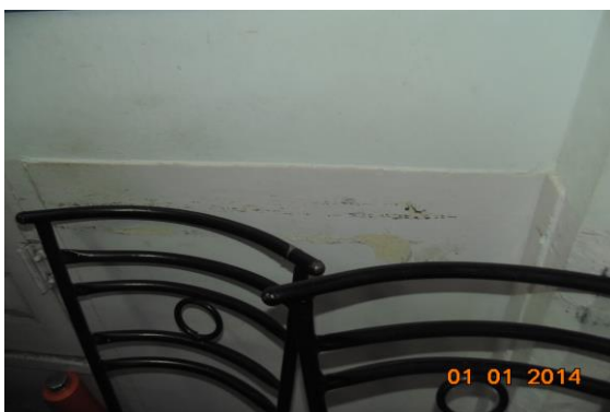
Photo 86 Peeling of Plaster on Wall No. 3 of Hall No. 1 of Second Floor
