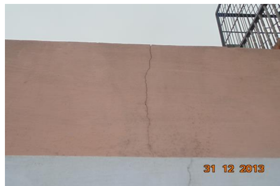
Photo 6 Inclined Crack on Wall No. 3 of Terrace Approx. Width = 1mm, Approx. Length = 0.4m. Distance from Wall No. 1 = 1m, Height from Floor = 2.2m.
