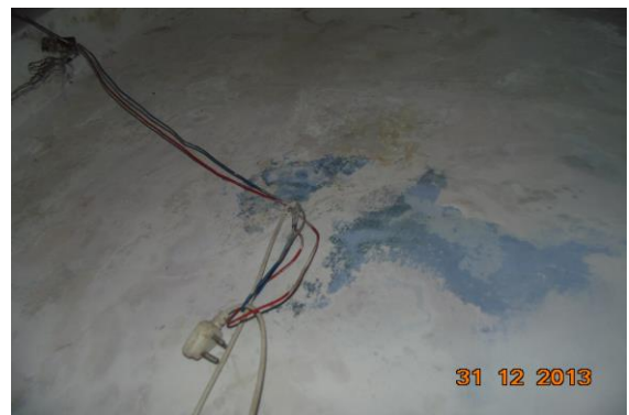
Photo 41 Dampness/Seepage on Wall No. 1 of Stair GF to FF
