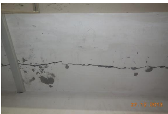
Photo 107 Horizontal Crack on Roof of Part -II of Shop No.27 & 36, Second Floor, Approx. Width = 3mm, Approx. Length = 2.5m. Distance from Wall no.1 = 0m, Height from Floor = 2.3m.
