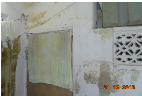
Photo 27 Dampness/Seepage on Wall No. 4 of Lobby of Second Floor
