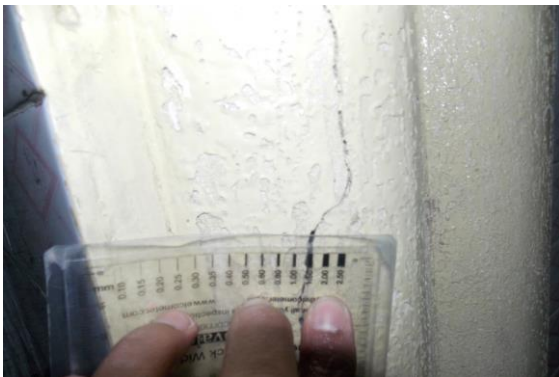
Photo 8A Inclined Crack on Wall No. 3 of Open Sky, Ground Floor Approx. Width = 1.5mm, Approx. Length = 0.9m. Distance from Wall no.8 = 0.05m, Height from Floor = 0m.
