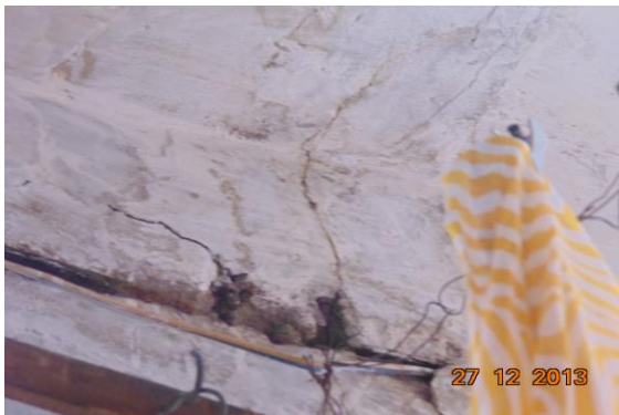
Photo 102 Plaster Crack on Roof of Kitchen of Third Floor
