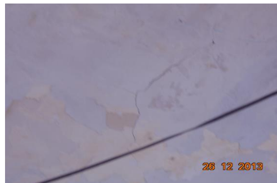
Photo 21 Inclined Crack on Roof of Varanda, Shop No. 37, Ground Floor Approx. Width = 1mm, Approx. Length = 1m.
