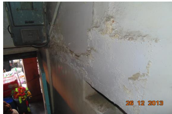
Photo 24 Damaged Portion on Wall No. 1 of Staircase GF to FF
