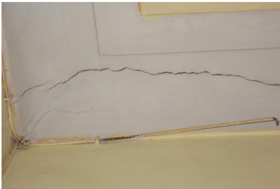
Photo 15 Horizontal Crack on Wall No. 1 of Varanda No.2, First Floor Approx. Width = 3mm, Approx. Length = 1.5m. Distance from Wall No.1 = 0.15m, Height from Floor = 3.5m.
