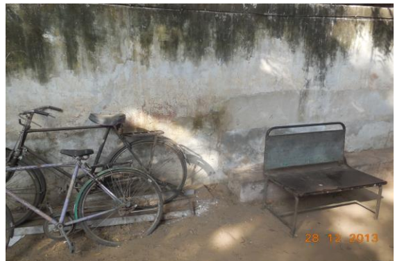
Photo 98 Peeling of Plaster on Wall No. 4 of Open Area 1 of Navjeevan Chikitsalaya of Ground Floor
