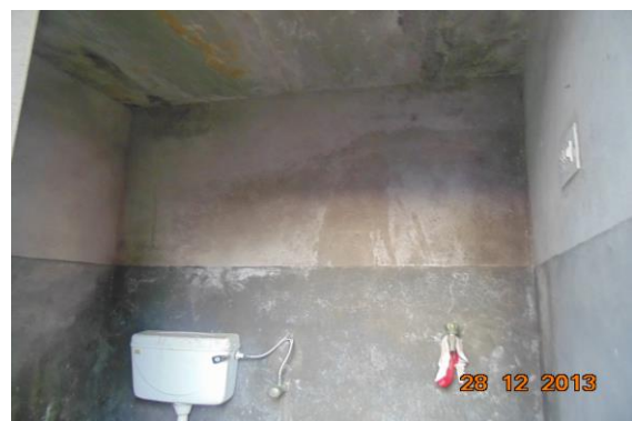
Photo 6 Dampness/Seepage on All Wall & roof of Toilet No. 1 of House No. 61, Ground Floor
