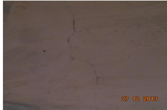
Photo 2 Horizontal Crack on Roof of Room No. 2, First Floor Approx. Width = 0.8mm, Approx. Length = 2m. Distance from Wall No.4 = 0m, Height from Floor = 2.1m.
