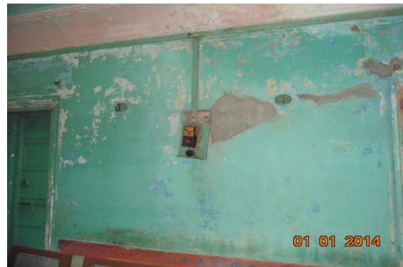
Photo 79 Dampness/Seepage on Wall No. 2 of Second Floor
