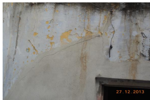
Photo 36 Inclined Crack on Wall No. 2 of Open Varanda, Second Floor Approx. Width = 0.5mm, Approx. Length = 1.5m. Distance from Wall no.4 = 0m, Height from Floor = 1.5m.
