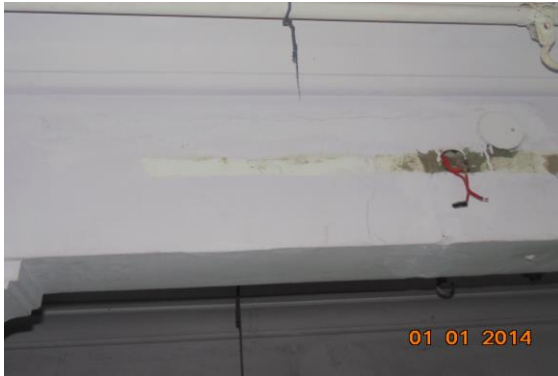
Photo 34 Plaster Crack on Roof of Lobby 2 of First Floor
