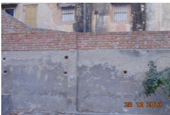
Photo 5 Peeling of Plaster on Wall No. 4 of Open Sky of House No. 61 of Ground Floor
