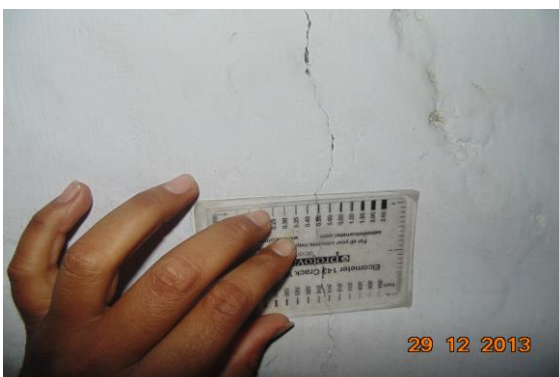
Photo 4A Inclined Crack on Wall No. 2 of Staircase Ground Floor to First Floor of House No.339, Ground Floor Approx. Width = 0.5mm, Approx. Length = 2m. Distance from = m, Height from Floor = m.
