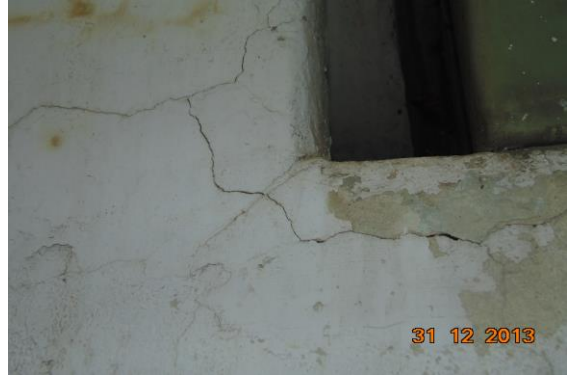
Photo 30 Peeling of Plaster on Wall No. 4 of Second Floor
