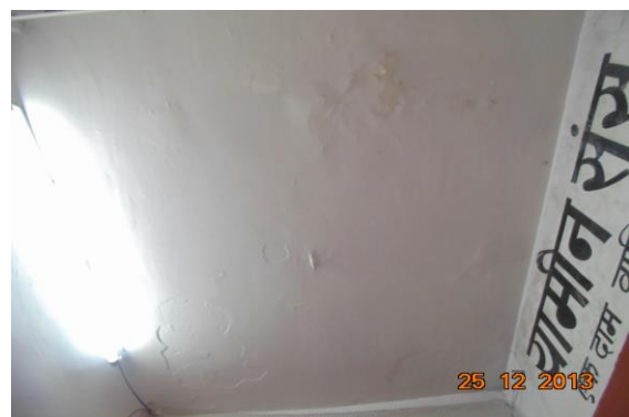
Photo 28 Peeling of Plaster on Roof of Varanda of Shop No. 46, Ground Floor
