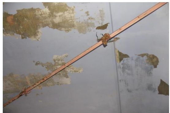
Photo 21 Peeling of Plaster on Roof of Room No. 1 of First Floor
