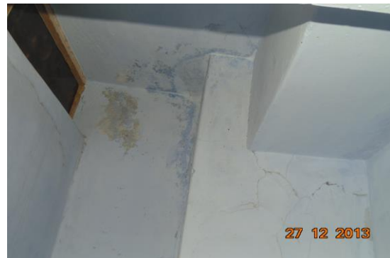
Photo 27 Dampness/Seepage on Wall No. 4 & Roof of Toilet No. 1 of First Floor
