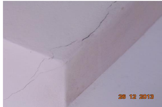
Photo 8 Inclined Crack on Wall No. 1 & Roof of Staircase, Second Floor Approx. Width = 0.6mm, Approx. Length = 1m. Distance from Wall no.2 = 1m, Height from Floor = 2.5m.
