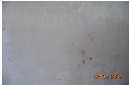
Photo 51 Dampness/Seepage on Wall No. 1 of Room No. 1 of Fifth Floor
