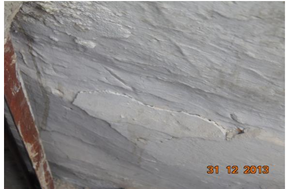
Photo 24 Peeling of Plaster on Wall No. 1 of Terrace
