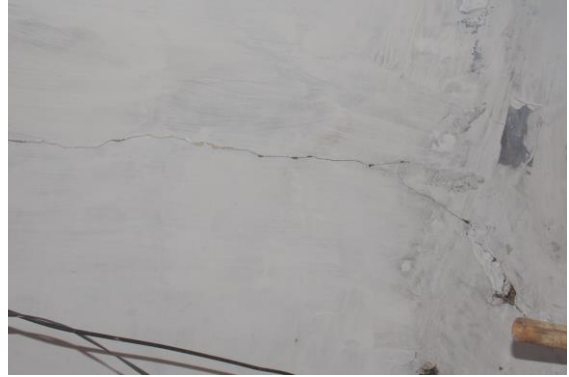
Photo 14 Inclined Crack on Roof & R/S External column of Varanda, Shop No. 90 & 91, G/F Approx. Width = 1.5mm, Approx. Length = 3m. Distance from R/s External column = 0m, Height from Floor = 2.8m.
