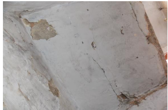
Photo 4 Inclined Crack on Roof of Staircase GF to FF Approx. Width = 20mm, Approx. Length = 1m.
