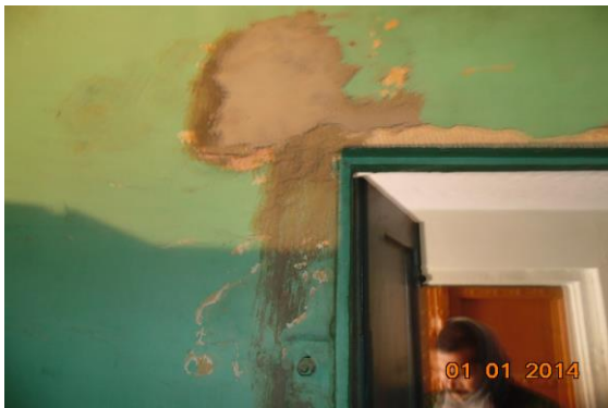
Photo 114 Peeling of Plaster on Wall No. 3 of Third Floor
