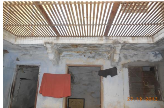
Photo 68 Dampness/Seepage on Wall No. 4 & Roof of Open To sky area of First Floor
