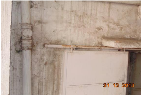
Photo 25 Dampness/Seepage on Wall No. 3 of Room No. 1 of Third Floor
