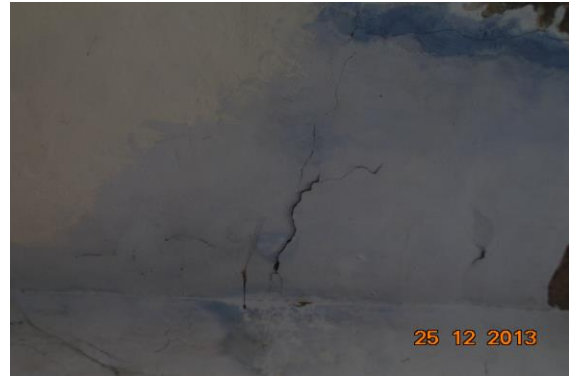
Photo 71 Damaged Portion on Shade of Balcony No.4 of Second Floor
