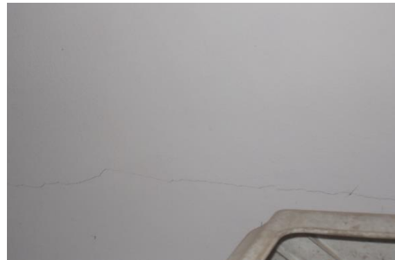
Photo 4 Horizontal Crack on Roof of Room No. 1, First Floor Approx. Width = 0.35mm, Approx. Length = 2.7m. Distance from Wall no.4 = 0.15m, Height from Floor = 2.5m.
