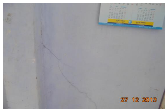
Photo 6 Inclined Crack on Wall No. 3 of Hall No. 1, First Floor Approx. Width = 0.5mm, Approx. Length = 2m. Distance from Wall no.1 = 3m, Height from Floor = 0.15m.
