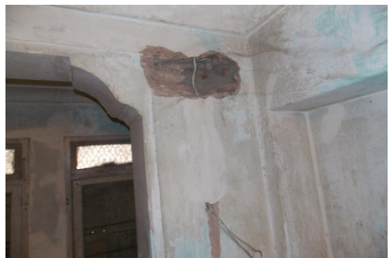
Photo 16 Peeling of Plaster on Wall No. 1 of Lobby of Second Floor
