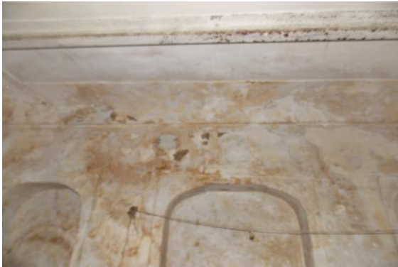
Photo 169 Dampness/Seepage on Wall No. 4 & Roof of Room No. 16 of Navjeevan Chikitsalaya, First Floor
