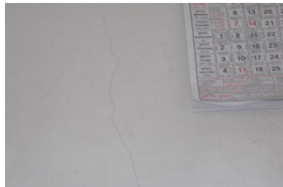
Photo 6 Inclined Crack on Wall No. 4 of Room No. 2, First Floor Approx. Width = 0.1mm, Approx. Length = 3m.
