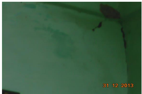
Photo 16 Dampness/Seepage on Wall No. 1 of Room No. 1 of Third Floor
