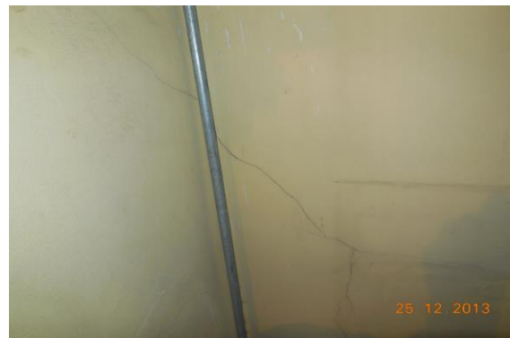
Photo 3 Inclined Crack on Wall No. 1 & 4 of Hall No. 1, First Floor Approx. Width = 0.6mm, Approx. Length = 2m. Distance from Corner Wall No.1 = 4m, Height from Floor = 0m.
