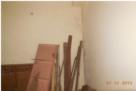
Photo 71 Dampness/Seepage on Wall No. 2 & 4 of Shop of First Floor
