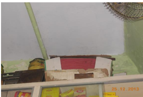
Photo 57 Peeling of Plaster on Wall No. 2 of Shop No.34 of Ground Floor
