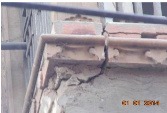
Photo 54 Peeling of Plaster on Left Side Shed of First Floor
