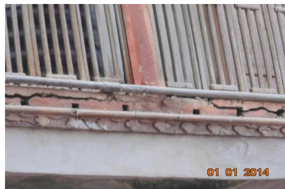
Photo 55 Peeling of Plaster on Left Side Shed of Ground Floor
