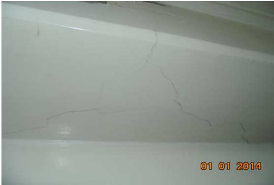
Photo 40 Plaster Crack on Roof of First Floor
