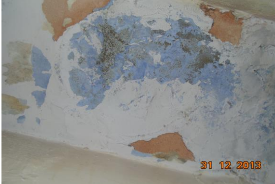
Photo 19 Dampness/Seepage on Roof of Second Floor
