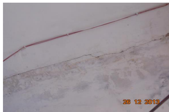
Photo 6 Horizontal Crack on Roof of Varanda, Shop No. 40, Ground Floor, Approx. Width = 1mm, Approx. Length = 2.5m. Distance from = m, Height from Floor = m.
