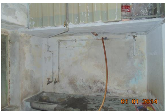
Photo 32 Dampness/Seepage on Wall No. 2 of First Floor
