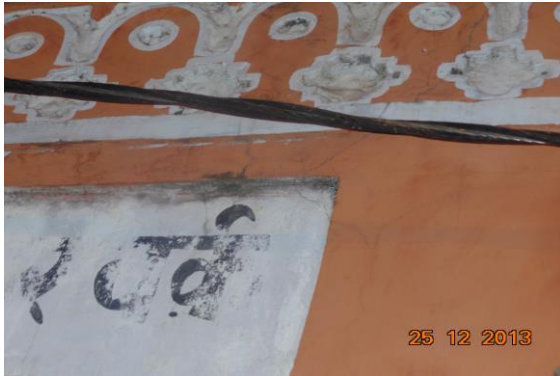
Photo 42 Peeling of Plaster on Beam of Varanda of Shop No. 49, Ground Floor
