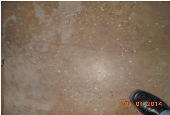
Photo 64 Plaster Crack on Floor of Second Floor
