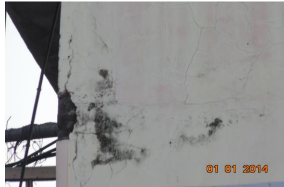
Photo 51 Peeling of Plaster on External Wall of FF External Hazard
