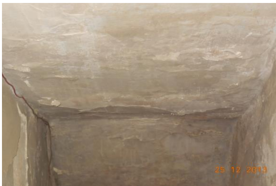
Photo 34 Peeling of Plaster on Wall No. 1 of Room No. 1 of Second Floor
