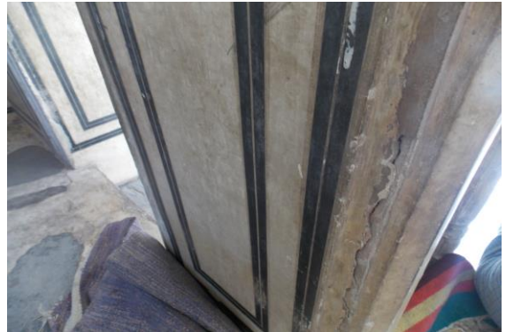
Photo 182 Peeling of Plaster on Wall No. 3 of Varanda 10 of Navjeevan Chikitsalaya of First Floor
