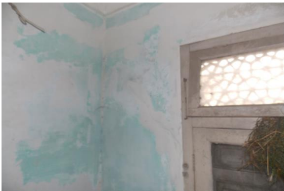
Photo 13 Peeling of Plaster on Wall No. 1 & 4 of Varanda of Second Floor
