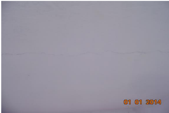
Photo 44 Plaster Crack on Roof of Stair TF to 4Th Floor
