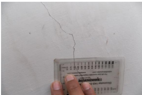
Photo 11 Inclined Crack on Wall No. 4 of Room No. 1, Fourth Floor, Approx. Width = 0.2mm, Approx. Length = 2.5m. Distance from Wall No. 5 = 0.3m, Height from Floor = 0m.
