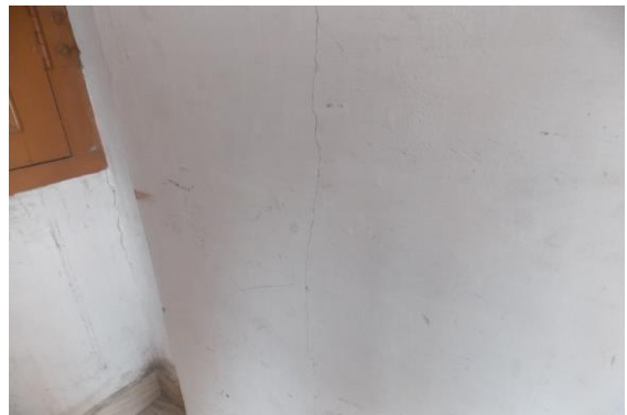
Photo 10 Inclined Crack on Wall No. 4 of Room No. 1, Fourth Floor, Approx. Width = 0.2mm, Approx. Length = 2.5m. Distance from Wall No. 5 = 0.3m, Height from Floor = 0m.
