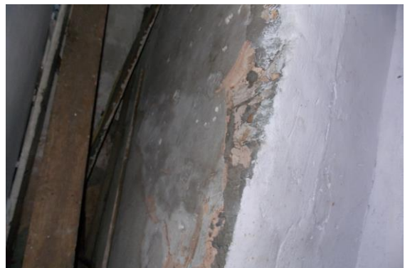
Photo 64 Peeling of Plaster on Wall No. 4 of Part A of Shop No.76 of Ground Floor
