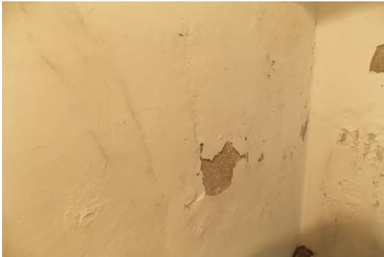
Photo 42 Peeling of Plaster on Wall No. 6 of Lobby of Ground Floor
