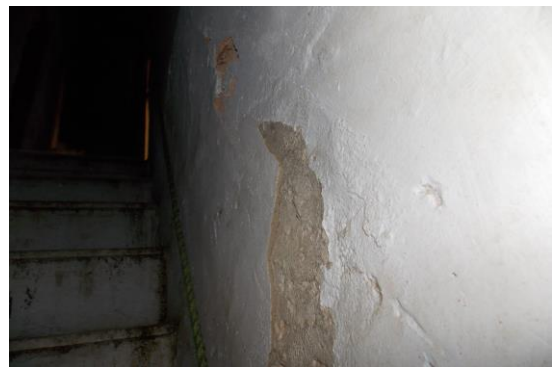
Photo 19 Peeling of Plaster on Wall No. 2 of Staircase GF to FF
