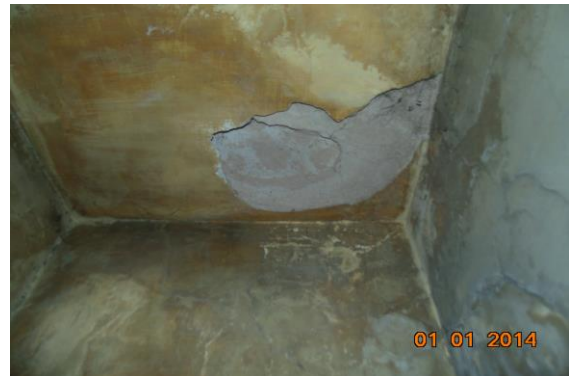
Photo 89 Peeling of Plaster on Roof of Third Floor
