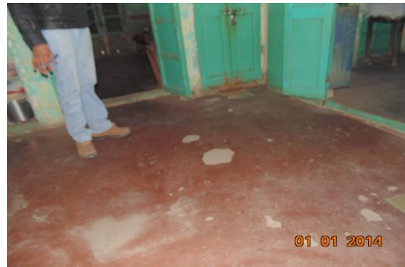
Photo 65 Peeling of Plaster on Floor of Room No. 1 of Second Floor
