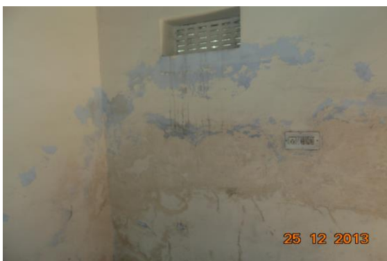
Photo 74 Dampness/Seepage on Wall No. 2 & 4 of Lobby of Second Floor
