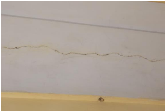
Photo 13 Horizontal Crack on Roof of Varanda, First Floor Approx. Width = 2.5mm, Approx. Length = 2m. Distance from Wall No.3 = 0.15m, Height from Floor = 6m.
