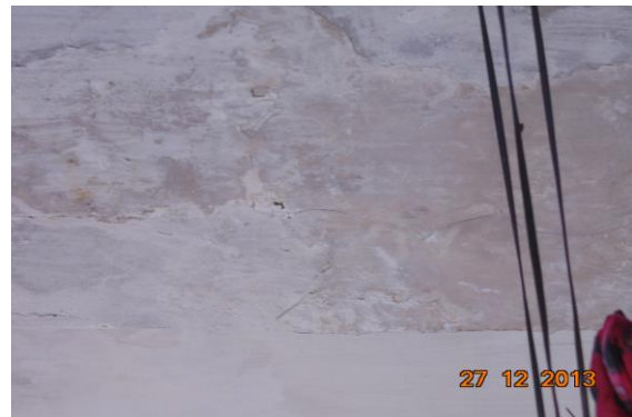
Photo 103 Peeling of Plaster on Wall No. 4 of Kitchen of Third Floor
