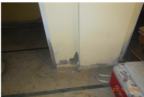
Photo 69 Peeling of Plaster on Wall No. 2 of Room No. 1 of First Floor
