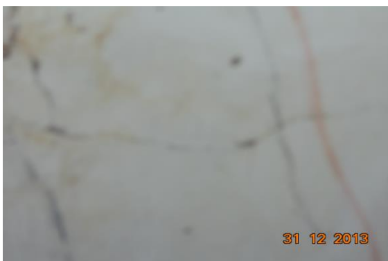
Photo 16 Peeling of Plaster on Wall No. 4 of Room No. 1 of Fourth Floor
