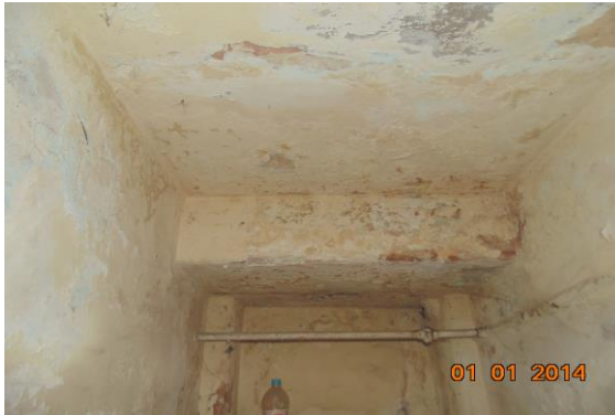
Photo 52 Dampness/Seepage on Roof of Toilet No. 1 of First Floor
