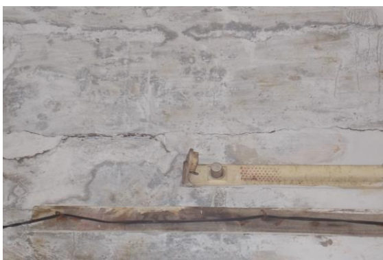
Photo 28 Peeling of Plaster on External Beam of Varanda of Ground Floor
