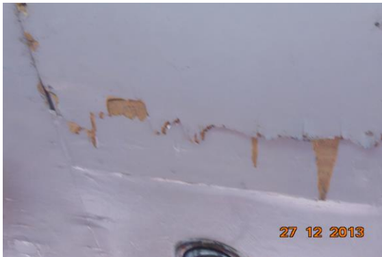
Photo 106 Peeling of Plaster on Wall No. 4 of Third Floor
