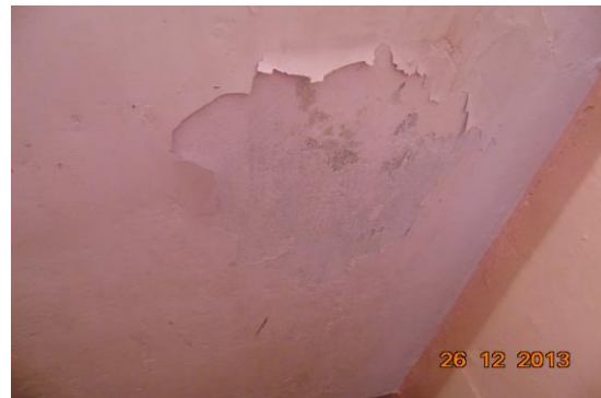
Photo 14 Peeling of Plaster on Roof of H.NO.302 of Third Floor
