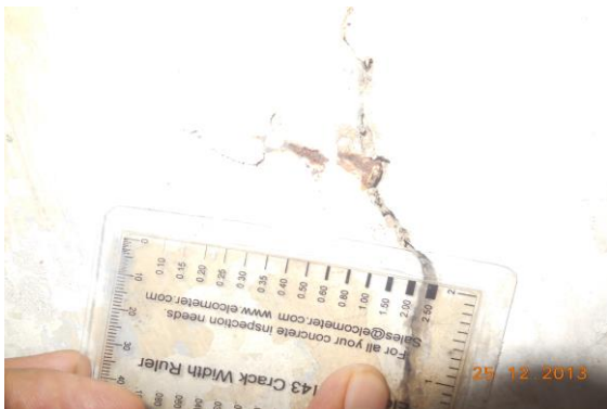
Photo 2A Vertical Crack on Wall No. 2 of Staircase Ground Floor to First Floor Approx. Width = 3mm, Approx. Length = 1.8m. Distance from Wall No.3 = 2m, Height from Floor = 0m.
