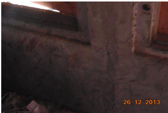
Photo 25 Peeling of Plaster on Wall No. 1 of Lobby of Second Floor
