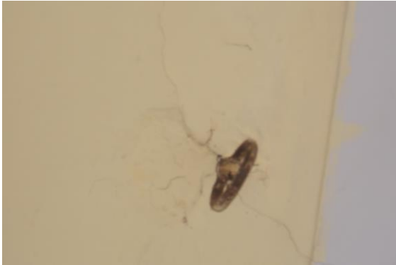
Photo 45 Peeling of Plaster on Roof of Varanda No.2 of First Floor
