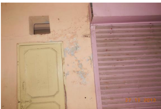
Photo 57 Dampness/Seepage on Outer Wall of Toilet No. 2 of Ground Floor
