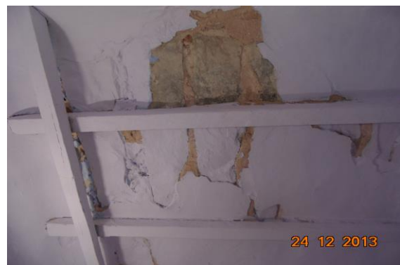
Photo 6 Peeling of Plaster on Roof of Part B of Shop No.20 of Ground Floor
