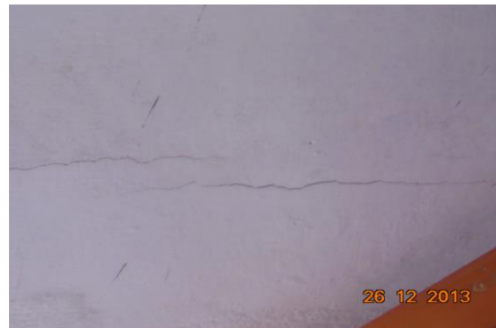
Photo 17 Inclined Crack on Wall No. 1 of Staircase SF to TF, Second Floor Approx. Width = 1mm, Approx. Length = 1m.
