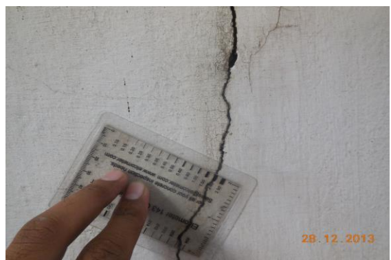
Photo 17A Inclined Crack on Wall No. 4 of Open Area 1 of Navjeevan Chikitsalaya, Ground Floor Approx. Width = 2mm, Approx. Length = 1.3m. Distance from Wall No.2 = 5m, Height from Floor = 1m.
