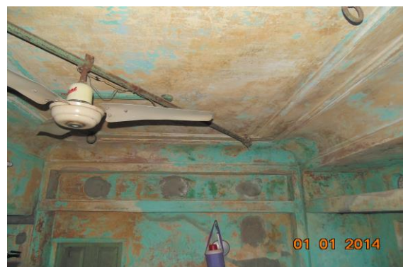
Photo 69 Dampness/Seepage on Roof & Wall No.4 of Room No. 2 of Second Floor
