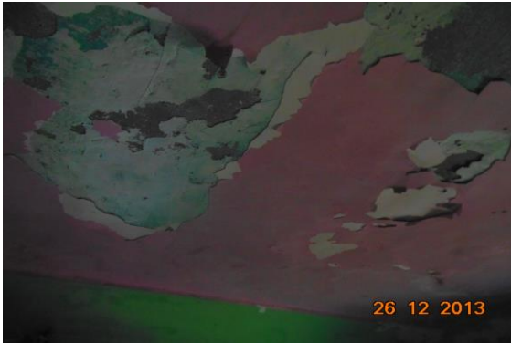
Photo 25 Peeling of Plaster on Roof of Lobby of Second Floor
