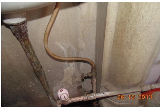
Photo 13 Peeling of Plaster on Wall No. 4 of Lobby of First Floor
