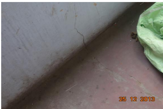
Photo 22 Inclined Crack on Parapet wall no.1 & Floor of Balcony No.4, First Floor Approx. Width = 0.6mm, Approx. Length = 0.8m. Distance from Wall No.3 = 1.5m, Height from Floor = 0m.
