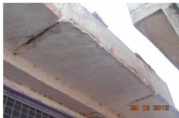
Photo 23 Damaged Portion on Wall No. 3 & Sunshade of Toilet No. 1 of House No. 339, Third Floor
