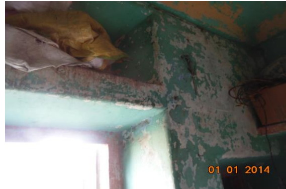
Photo 125 Dampness/Seepage on Wall No. 2 of Third Floor
