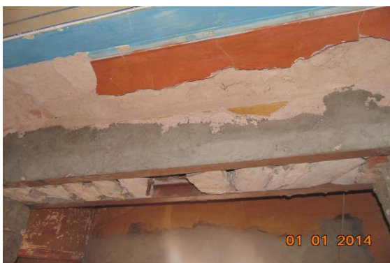
Photo 56 Damaged Portion on Roof of Lobby of Second Floor
