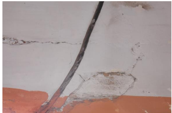
Photo 26 Damaged Portion on Beam of Varanda of Ground Floor
