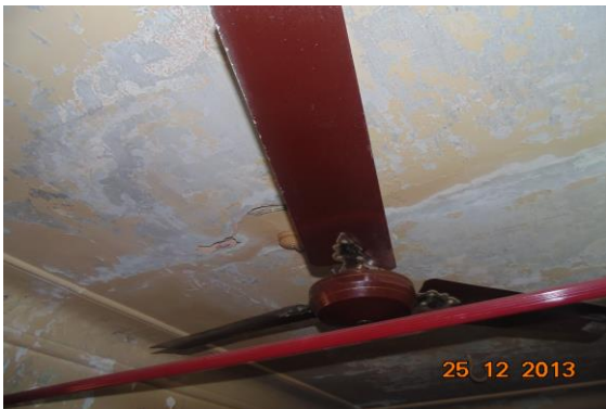
Photo 108 Plaster Crack on Roof of Lobby of House No. 347 Part A, Second Floor
