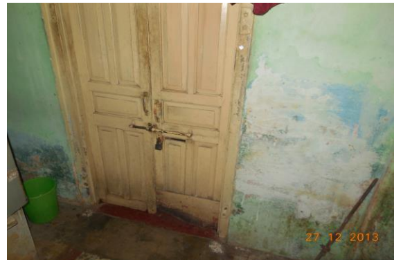
Photo 66 Dampness/Seepage on Wall No. 1 of Varanda No.1 of First Floor
