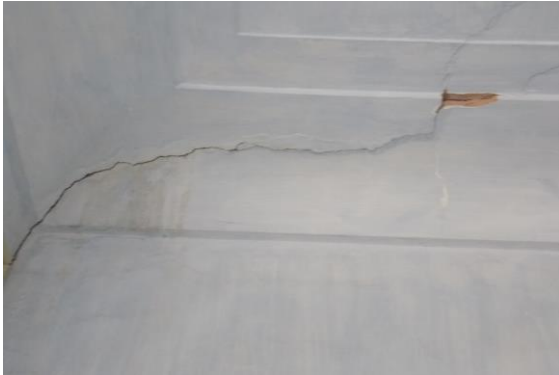
Photo 69 Damaged Portion on Roof of Hall No. 2 of Second Floor
