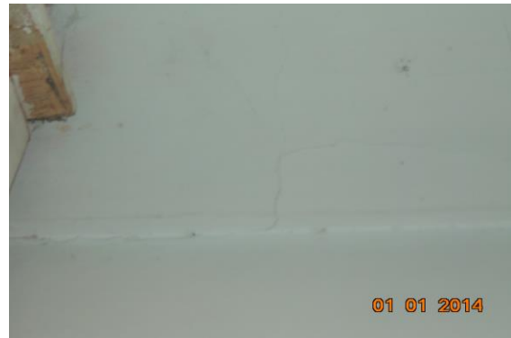
Photo 29 Plaster Crack on Roof & Wall No. 3 of First Floor
