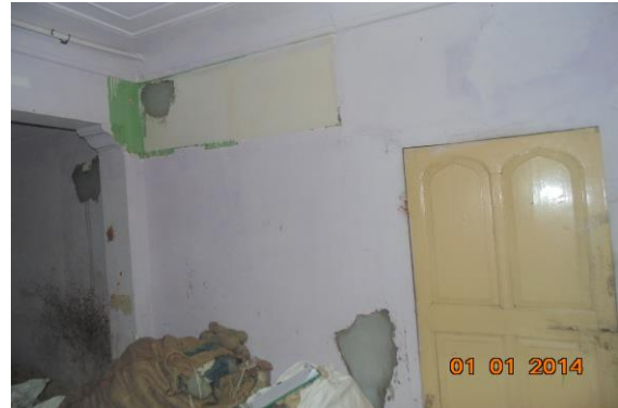
Photo 35 Peeling of Plaster on Wall No. 3 of First Floor
