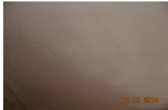
Photo 109 Plaster Crack on Roof of Third Floor
