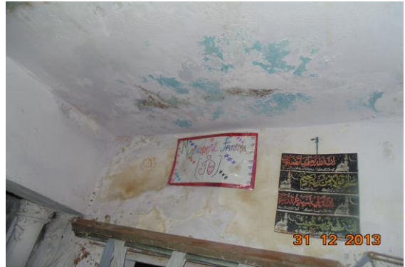
Photo 32 Dampness/Seepage on Wall No. 2 of Lobby Shed of Second Floor
