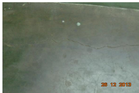
Photo 6 Inclined Crack on Floor of Room No. 2, First Floor, Approx. Width = 0.3mm, Approx. Length = 2m. , Height from Floor = m.
