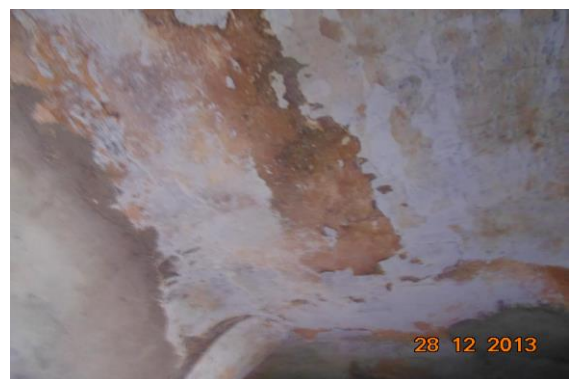
Photo 6 Dampness/Seepage on Roof of Passage of House No 290 & 291 of Ground Floor
