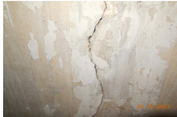
Photo 2 Vertical Crack on Wall No. 2 of Staircase Ground Floor to First Floor Approx. Width = 3mm, Approx. Length = 1.8m. Distance from Wall No.3 = 2m, Height from Floor = 0m.
