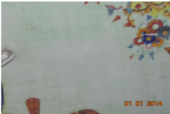
Photo 84 Plaster Crack on Roof of Hall No. 1 of Second Floor
