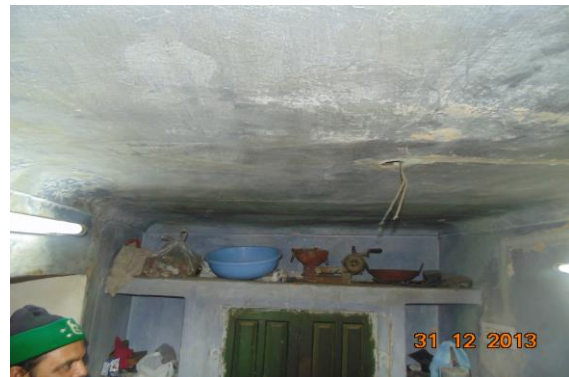
Photo 28 Dampness/Seepage on Wall No. 1, 4 & Roof of Room No. 2 of Third Floor
