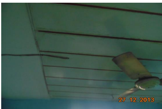
Photo 36 Peeling of Plaster on Roof of Room No. 2 of Second Floor
