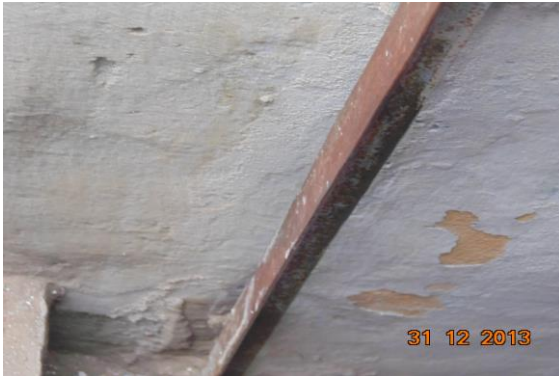
Photo 23 Peeling of Plaster on Wall No. 2 of Stair SF to TF of Terrace
