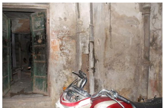
Photo 90 Peeling of Plaster on Outer wall of Building of Ground Floor
