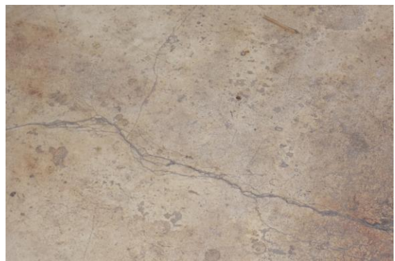
Photo 28 Plaster Crack on Floor of Varanda of First Floor
