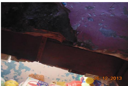
Photo 27 Damaged Portion on Roof of Part B of Shop No.42 of Ground Floor
