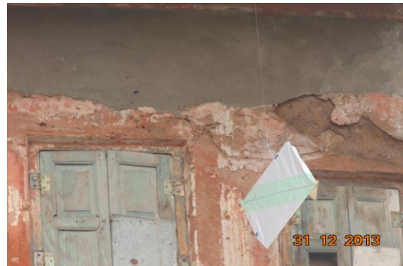
Photo 54 Peeling of Plaster on Outer Wall of Second Floor
