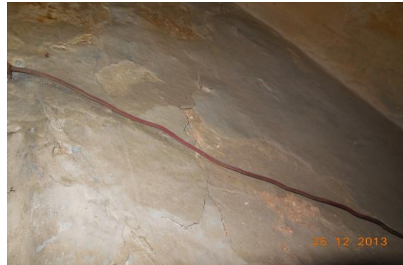
Photo 33 Peeling of Plaster on Wall No. 2 of Staircase First Floor to Second Floor
