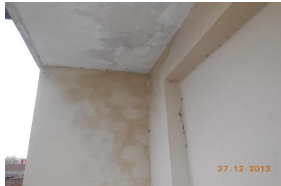
Photo 96 Dampness/Seepage on Wall No. RHS outer Wall of Open Area of Terrace
