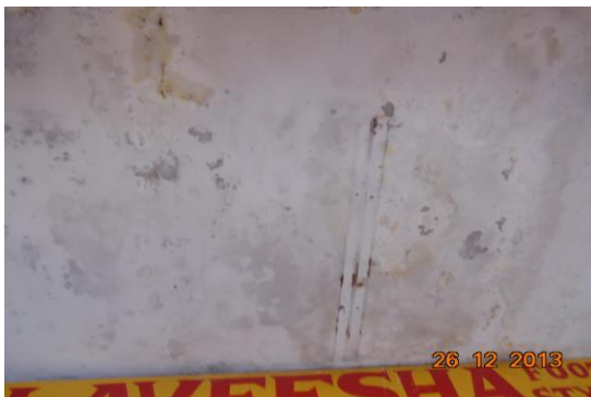
Photo 15 Peeling of Plaster on Roof of Varanda of Shop No.42, Ground Floor
