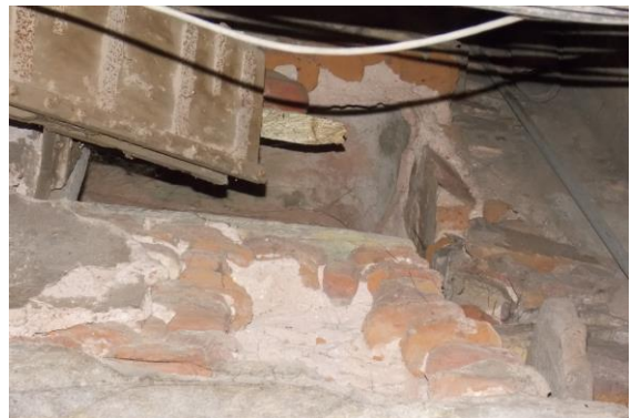
Photo 88 Peeling of Plaster on Outer wall of H.No.286 of Ground Floor
