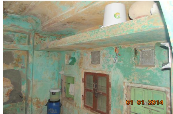
Photo 71 Dampness/Seepage on Wall No. 2 of Second Floor
