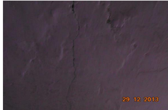
Photo 4 Inclined Crack on Wall No. 2 of Staircase Ground Floor to First Floor of House No.339, Ground Floor Approx. Width = 0.5mm, Approx. Length = 2m. Distance from = m, Height from Floor = m.
