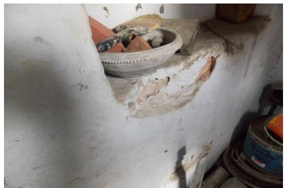
Photo 19 Peeling of Plaster on Wall No. 3 of Room No. 1 of Above Shop No. 74, Third Floor
