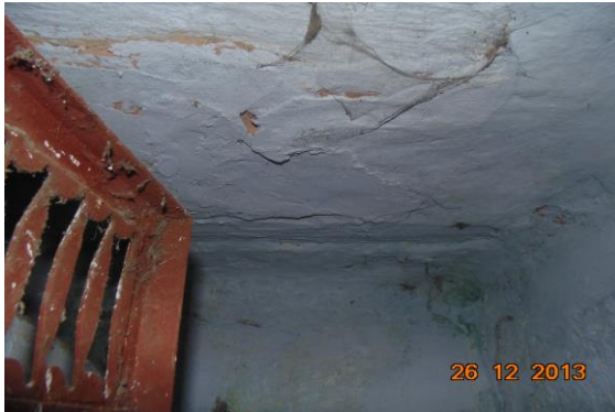
Photo 10 Inclined Crack on front side of Staircase GF to FF, Ground Floor, Approx. Width = 2mm, Approx. Length = 1m. , Height from Floor = m.
