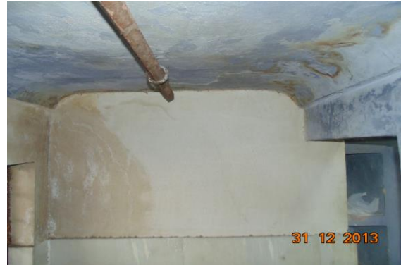
Photo 26 Dampness/Seepage on Wall No. 1, 3, 4 & Roof of Room No. 2 of Third Floor
