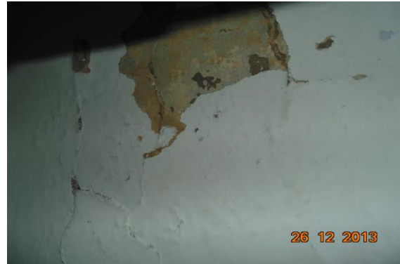
Photo 29 Peeling of Plaster on Roof of Staircase SF to TF of Second Floor
