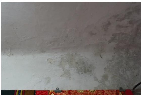
Photo 26 Dampness/Seepage on Roof of Varanda of Shop No.69 of Ground Floor
