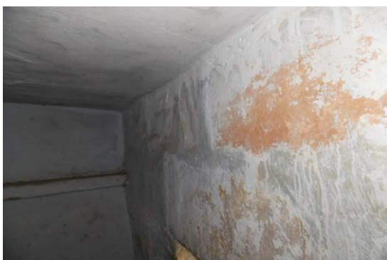
Photo 32 Peeling of Plaster on Wall No. 2 of Toilet No. 1 of First Floor
