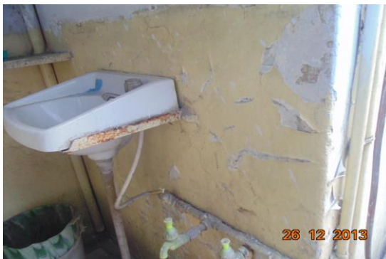
Photo 12 Peeling of Plaster on Wall No. 2 of Lobby of Third Floor
