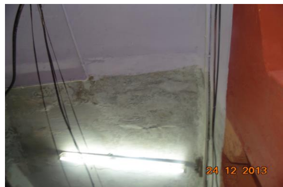
Photo 6 Dampness/Seepage on Roof of Varanda of Shop No.25 of Ground Floor
