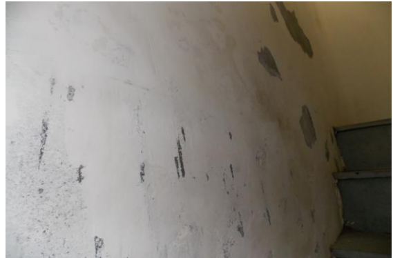
Photo 43 Peeling of Plaster on Wall No. 1 of Staircase Ground Floor To First Floor of Ground Floor
