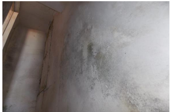
Photo 15 Dampness/Seepage on Wall No. 2 of Staircase FF to SF
