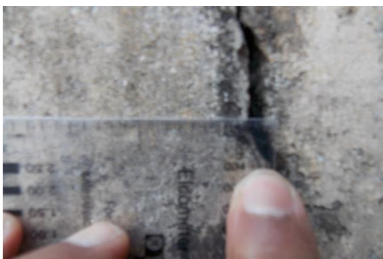
Photo 4A Inclined Crack on Wall No. 4 of Open Area, Third Floor, Approx. Width = 4mm, Approx. Length = 2m. Distance from Wall No. 2 = 0.2m, Height from Floor = 0m.
