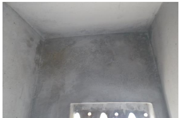
Photo 22 Dampness/Seepage on Wall No. 2 of Staircase SF to TF
