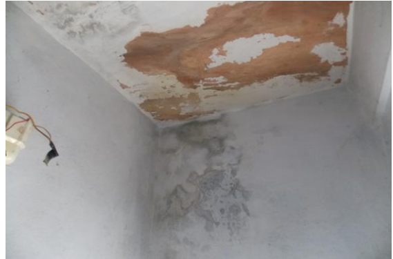
Photo 18 Dampness/Seepage on Wall No. 2 & 4 of Toilet No. 1 of Second Floor
