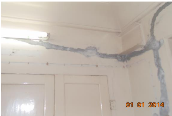
Photo 42 Plaster Crack on Wall No. 2 & 3 of Room No. 3 of First Floor
