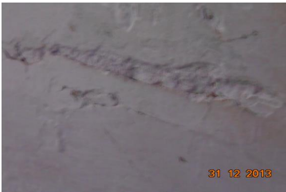
Photo 25 Peeling of Plaster on Wall No. 2 of Terrace
