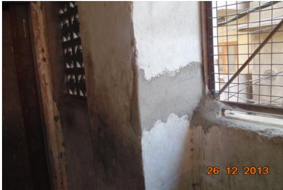
Photo 17 Damaged Portion on Wall No. 4 of Passage of First Floor
