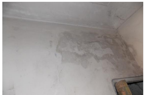
Photo 39 Dampness/Seepage on Wall No. 3 of Room No. 1 of Second Floor
