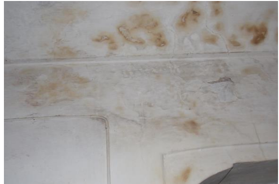
Photo 170 Dampness/Seepage on Wall No. 3 & Roof of Room No. 16 of Navjeevan Chikitsalaya, First Floor
