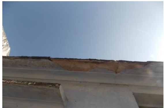
Photo 72 Peeling of Plaster on Sun Shade of Digamber Jain of Second Floor
