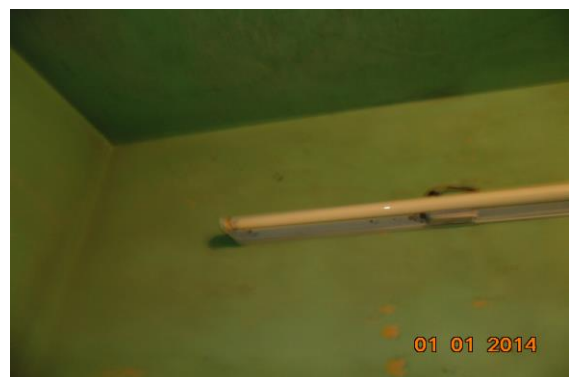
Photo 117 Dampness/Seepage on Wall No. 4 of Third Floor
