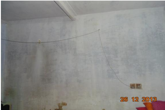
Photo 15 Dampness/Seepage on Wall No. 3 of Room No. 1 of Third Floor
