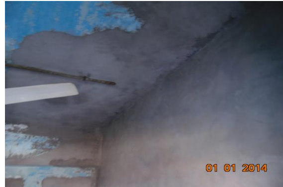
Photo 119 Peeling of Plaster on Roof & Wall No.2 of Room No. 3 of Third Floor
