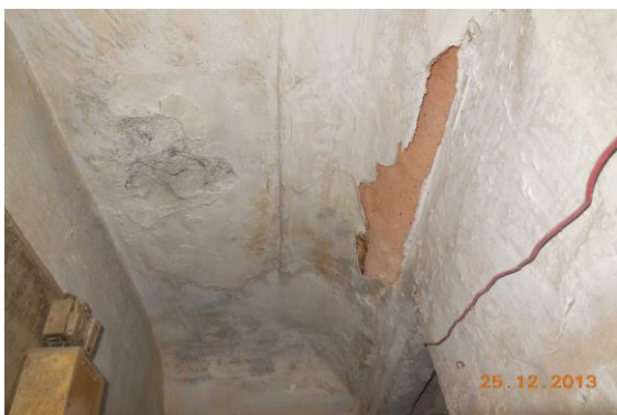
Photo 30 Peeling of Plaster on Roof of Passage of First Floor
