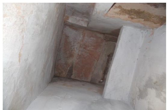
Photo 33 Peeling of Plaster on Roof of Toilet No. 1 of First Floor
