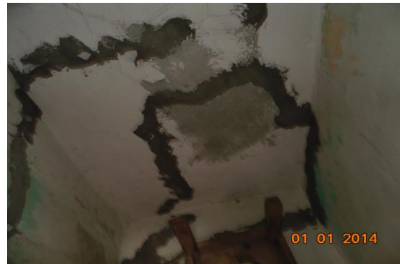
Photo 95 Peeling of Plaster on Roof of Toilet No. 1 of Third Floor
