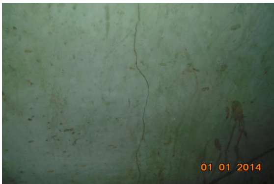
Photo 9 Inclined Crack on Wall No. 1 of House No. 458, First Floor Approx. Width = 1mm, Approx. Length = 1.2m. Distance from Wall No. 3 = 1.1m, Height from Floor = 1m.
