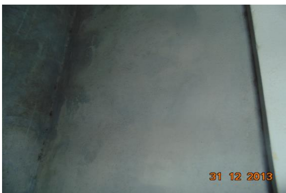
Photo 28 Dampness/Seepage on Wall No. 2 of Fifth Floor
