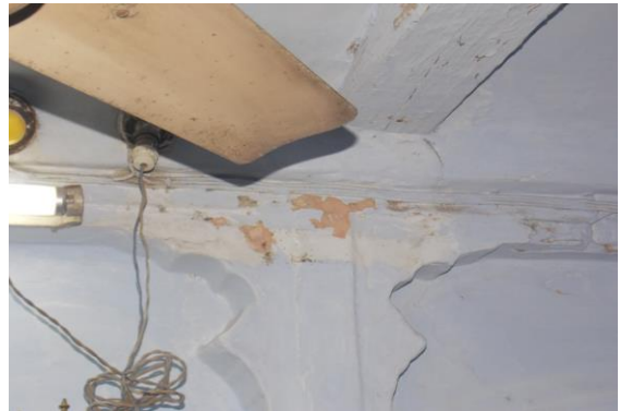
Photo 30 Peeling of Plaster on Wall No. 4 of Room No. 2 of Second Floor
