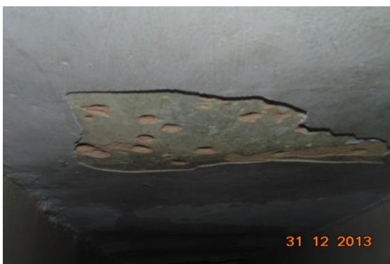
Photo 35 Peeling of Plaster on Roof of Third Floor
