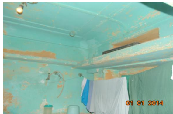
Photo 61 Dampness/Seepage on Wall No. 2 & 4 of Second Floor
