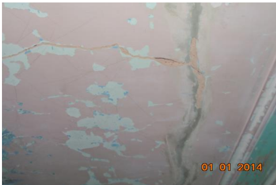
Photo 72 Peeling of Plaster on Roof of Hall No. 1 of Second Floor
