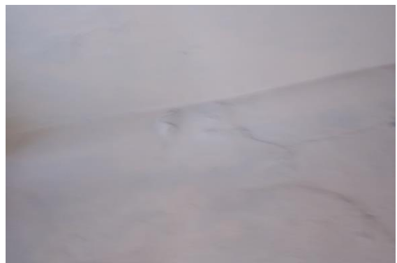
Photo 10 Inclined Crack on Wall No. 4 of Room No. 1, Fourth Floor, Approx. Width = 0.2mm, Approx. Length = 2.5m. Distance from Wall No. 5 = 0.3m, Height from Floor = 0m.
