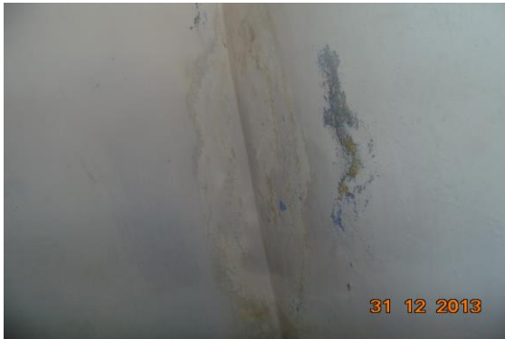
Photo 7 Dampness/Seepage on Wall No. 1 of Stair SF to TF
