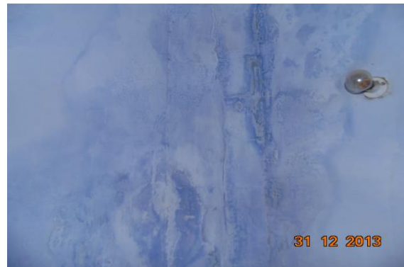
Photo 15 Dampness/Seepage on Wall No. 4 & 1 of Stair TF to 4Th Floor
