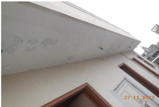
Photo 97 Dampness/Seepage on Wall No. Mumty Shade of Open Area of Terrace
