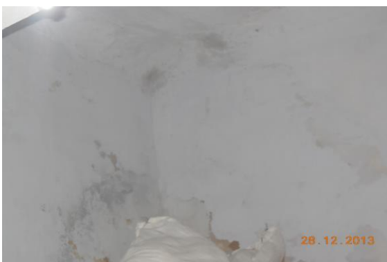
Photo 99 Dampness/Seepage on Wall No. 1, 4 & Roof of Room No. 9 of Part D of Navjeevan Chikitsalaya, Ground Floor
