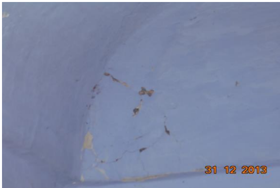
Photo 6 Peeling of Plaster on Wall No. 2 of Room No. 1 of Second Floor
