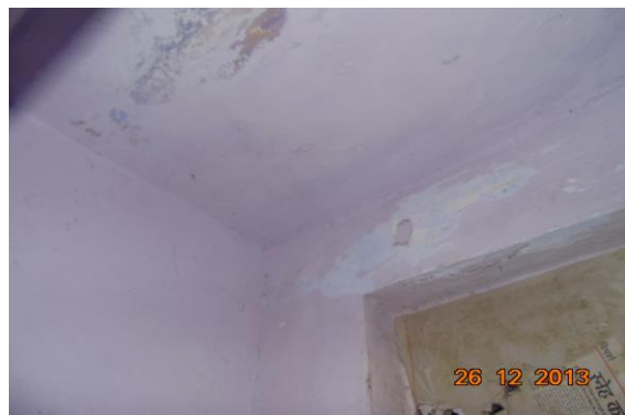
Photo 12 Dampness/Seepage on Wall No. 4 & Roof of Passage of Second Floor
