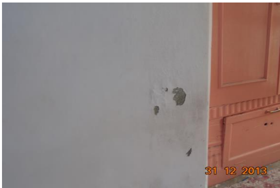
Photo 43 Dampness/Seepage on Wall No. 4 of First Floor
