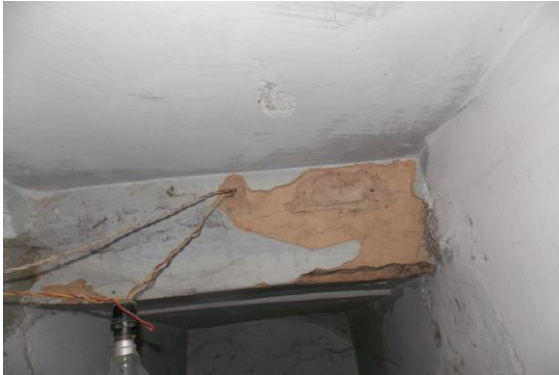
Photo 23 Peeling of Plaster on Wall No. 3 of Staircase GF to FF
