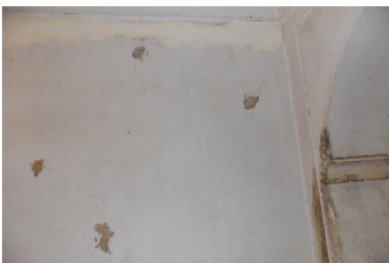
Photo 33 Peeling of Plaster on Wall No. 3 of Lobby of First Floor
