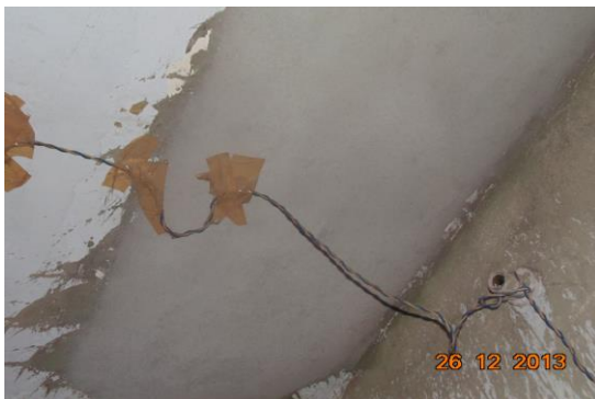
Photo 36 Peeling of Plaster on Roof of Room No. 1 of Third Floor
