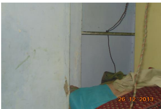
Photo 5 Peeling of Plaster on Room No. 1 of First Floor
