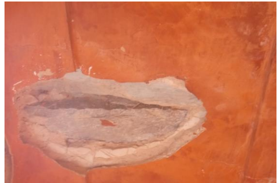
Photo 41 Peeling of Plaster on Roof of Balcony of Second Floor
