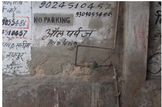
Photo 25 Damaged Portion on Backside Wall of Building of Ground Floor
