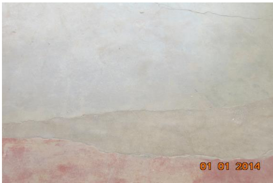
Photo 30 Plaster Crack on Floor of First Floor
