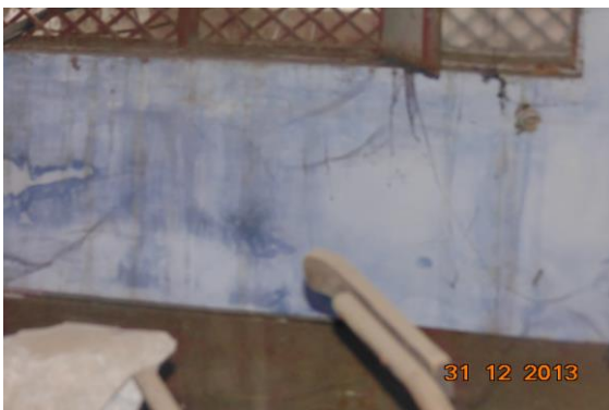
Photo 40 Dampness/Seepage on Wall No. 2 of First Floor
