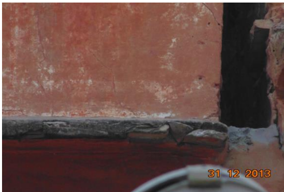
Photo 26 Damaged Portion on Front Wall of Shed of First Floor
