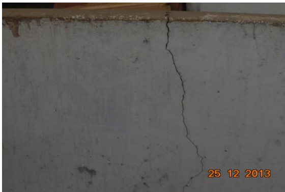
Photo 21 Vertical Crack on Wall No. 1 of Open Sky, First Floor, Approx. Width = 2mm, Approx. Length = 1m. Distance from Wall No.4 = 2.5m, Height from Floor = 0m.
