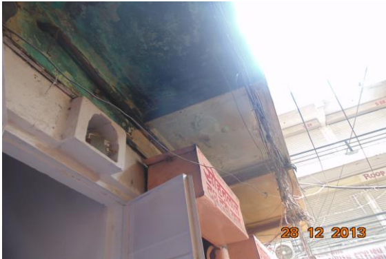
Photo 13 Dampness/Seepage on Wall No. 3 of House No.289 of Ground Floor
