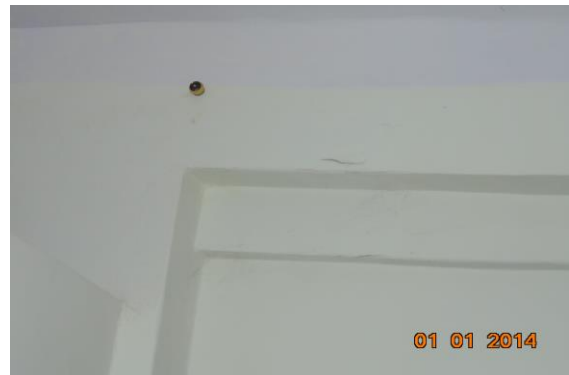
Photo 85 Peeling of Plaster on Wall No. 4 of Room No. 3 of Second Floor
