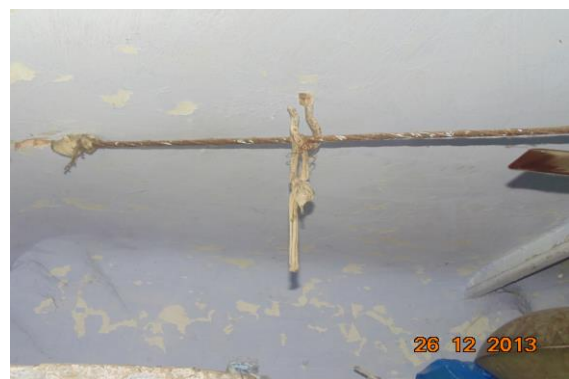
Photo 6 Peeling of Plaster on Wall No. 4 & Roof of Room No. 2 of First Floor
