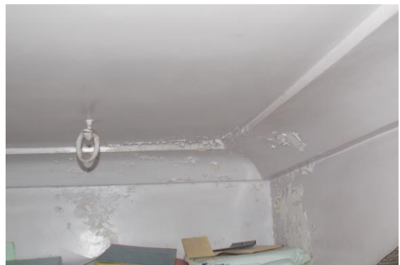
Photo 12 Dampness/Seepage on Wall No. 2, 3 & Roof of Room No. 1 of Second Floor
