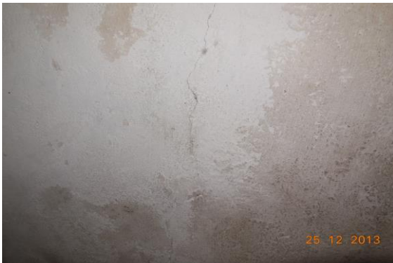
Photo 2A Vertical Crack on Wall No. 1 of Staircase Ground To First Floor Approx. Width = 1mm, Approx. Length = 1.5m. Distance from Wall No.4 = 0.9m, Height from Floor = 0m.
