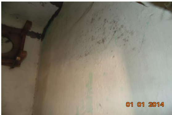
Photo 96 Dampness/Seepage on Wall No. 2 of Third Floor
