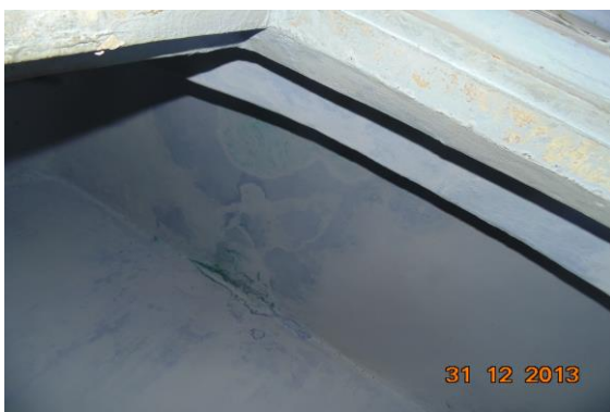
Photo 22 Dampness/Seepage on Roof of First Floor
