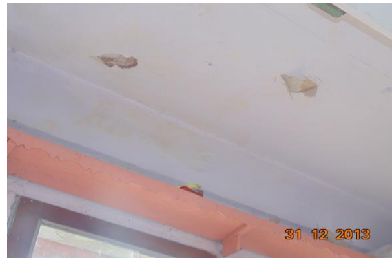
Photo 44 Dampness/Seepage on Wall No. 4 of Varanda of First Floor
