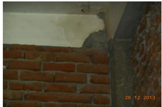
Photo 155 Peeling of Plaster on Entry Gate & 4 of Shopping Complex of Basement
