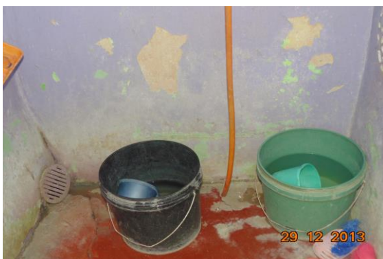
Photo 22 Peeling of Plaster on Wall No. 1, 2 & 4 of Bathroom of House No. 339, Third Floor
