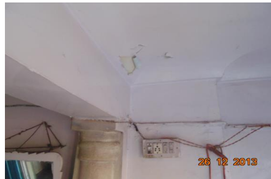
Photo 12 Peeling of Plaster on Roof of Varanda of First Floor
