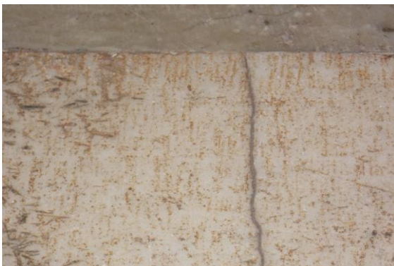
Photo 49 Peeling of Plaster on Floor of Varanda No.2 of First Floor
