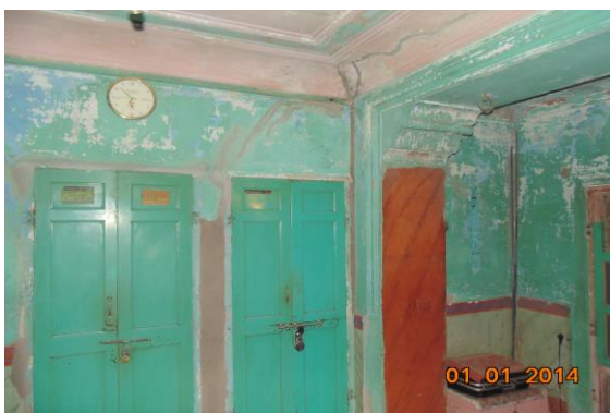
Photo 80 Dampness/Seepage on Wall No. 3 of Second Floor
