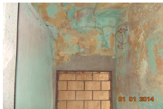
Photo 63 Dampness/Seepage on Wall No. 1, 2 & 4 of Second Floor
