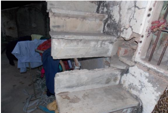
Photo 81 Damaged Portion on Steps of Staircase TF to Terrace of
