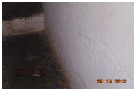
Photo 11 Peeling of Plaster on Wall No. 2 of Passage 2 of House No.339 of Second Floor
