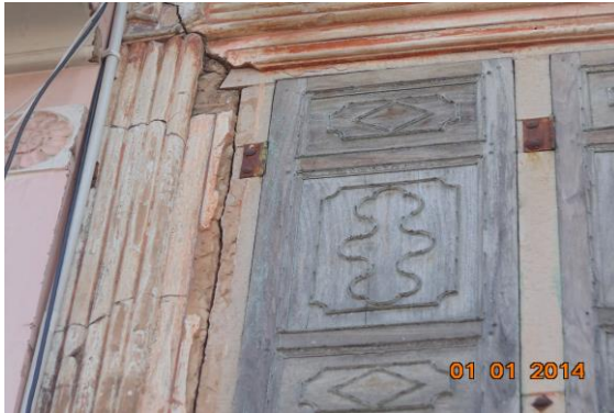
Photo 136 Peeling of Plaster on Outer Wall of SF External Façade
