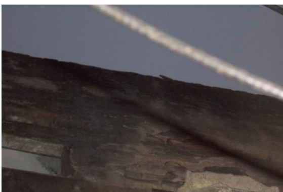
Photo 89 Peeling of Plaster on Outer wall of H.No.286 of Ground Floor
