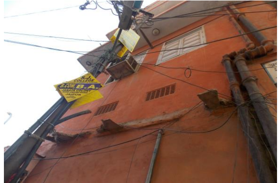
Photo 23 Peeling of Plaster on Sun Shade of Building of Ground Floor
