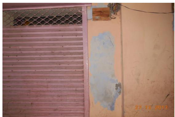
Photo 58 Peeling of Plaster on Outer Wall of Shop No.1 of Ground Floor
