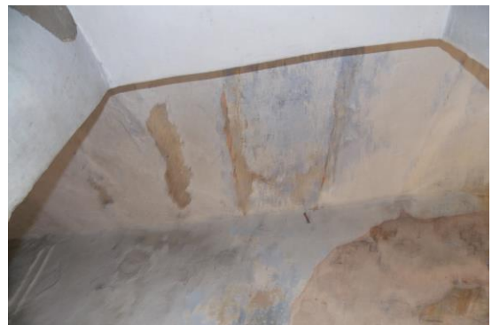
Photo 31 Peeling of Plaster on Roof of Store of First Floor
