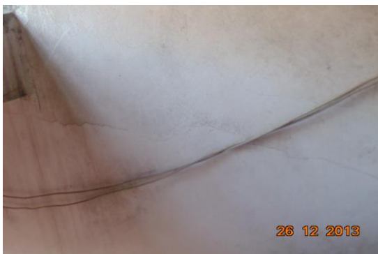
Photo 20 Inclined Crack on Wall No. 1 of Staircase GF to FF, Ground Floor Approx. Width = 0.5mm, Approx. Length = 2m.
