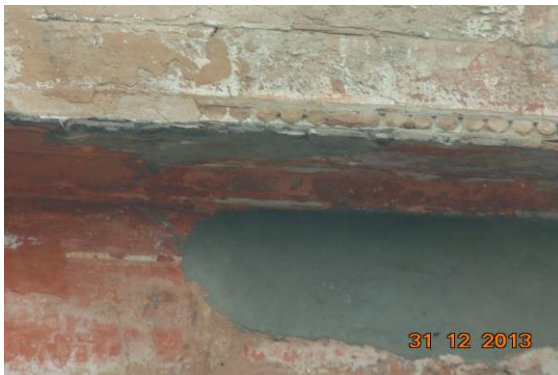
Photo 55 Peeling of Plaster on Shed of Second Floor
