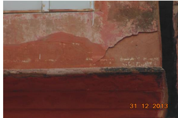
Photo 25 Peeling of Plaster on Front Wall of Third Floor
