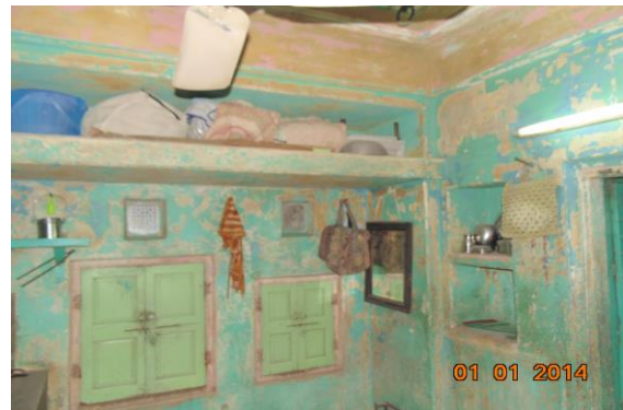
Photo 67 Dampness/Seepage on Wall No. 2 & 4 of Second Floor
