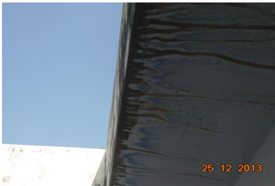
Photo 72 Dampness/Seepage on Shade of Balcony No.3 of Second Floor
