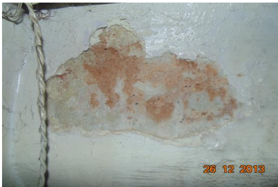
Photo 23 Peeling of Plaster on Roof of Staircase GF to FF
