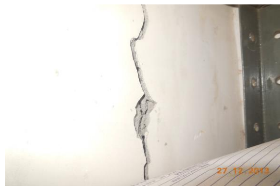
Photo 108 Vertical Crack on Wall No. 2 of Part -II of Shop No.27 & 36, Second Floor Approx. Width = 5mm, Approx. Length = 2.3m. Distance from Wall no.3 = 0.1m Height from Floor = 0m
