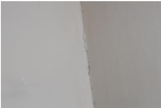
Photo 3 Inclined Crack on Wall No. 2, 4 & joint Crack of Store , Second Floor Approx. Width = 1mm, Approx. Length = 2m.
