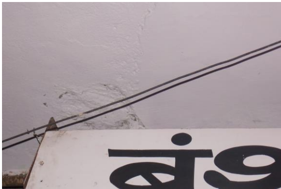
Photo 3 Peeling of Plaster on Roof of Varanda of Shop No.29 of Ground Floor
