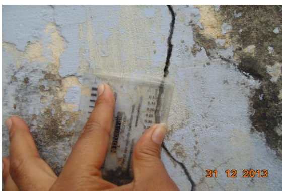
Photo 4A Inclined Crack on Wall No. 5 of Open Area 1, Terrace, Approx. Width = 4mm, Approx. Length = 3m. Distance from Wall No. 2 = 1.1m, Height from Floor = 0m.
