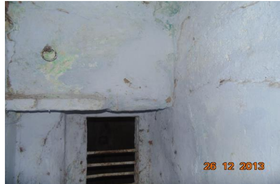
Photo 11 Horizontal Crack on Roof of Varanda, Shop No. 50, Ground Floor, Approx. Width = 0.6mm, Approx. Length = 2.5m. Distance from Right External Column = 0m, Height from Floor = 3m.
