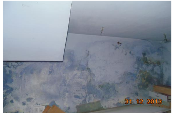
Photo 39 Dampness/Seepage on Wall No. 1 of Hall No. 1 of First Floor
