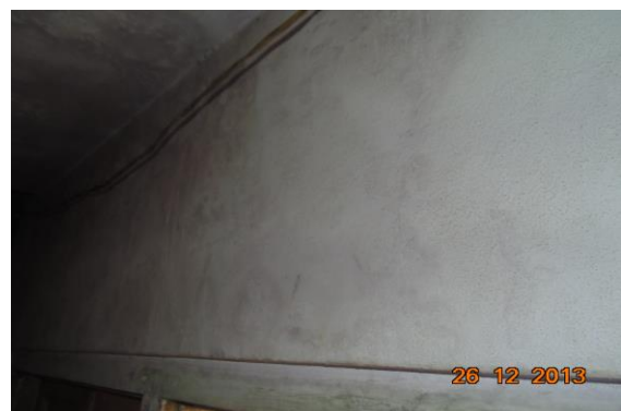
Photo 22 Dampness/Seepage on Wall No. 1 of Passage of Second Floor
