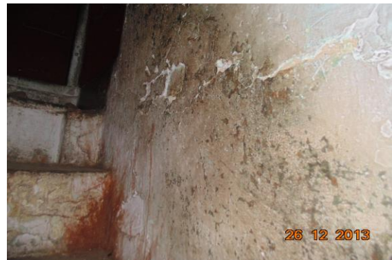
Photo 25 Dampness/Seepage on Wall No. 2 of Staircase FF to SF of First Floor
