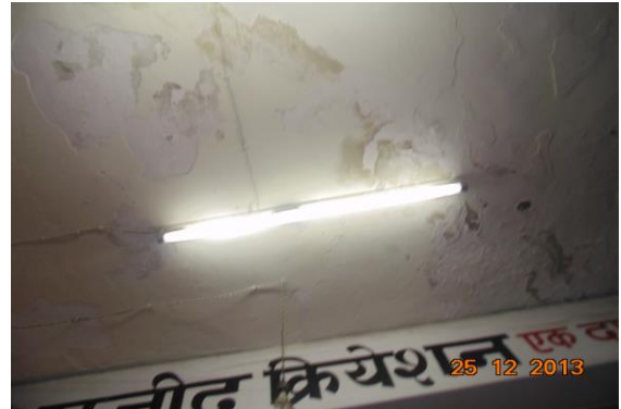
Photo 26 Dampness/Seepage on Roof of Varanda of Shop No. 55, Ground Floor
