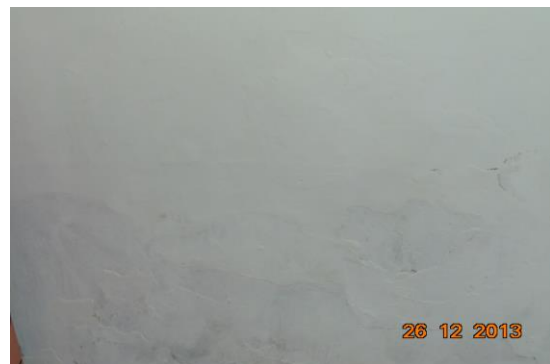
Photo 55 Peeling of Plaster on Roof of Varanda of Shop No.57, Ground Floor
