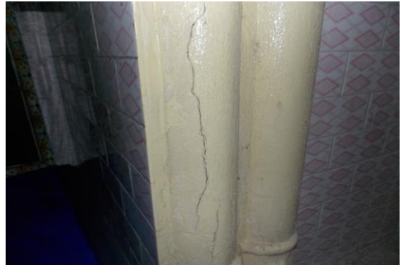
Photo 8 Inclined Crack on Wall No. 3 of Open Sky, Ground Floor Approx. Width = 1.5mm, Approx. Length = 0.9m. Distance from Wall no.8 = 0.05m, Height from Floor = 0m.
