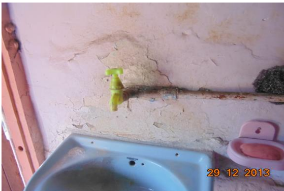
Photo 8 Peeling of Plaster on Wall No. 2 of Varanda of House No. 339 of First Floor
