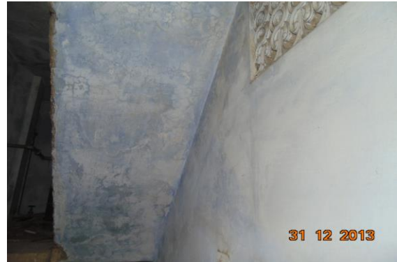
Photo 31 Dampness/Seepage on Wall No. 2 & Roof of Fifth Floor
