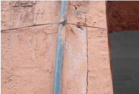
Photo 15 Vertical Crack on External Column of Varanda , Shop No. 93, Ground Floor, Approx. Width = 0.8mm, Approx. Length = 3.5m. Distance from External Column = 0m, Height from Floor = 0m.
