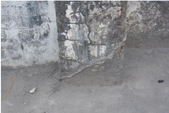
Photo 11 Plaster Crack on Wall No. 4 of Open Area of Third Floor
