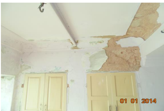
Photo 44 Peeling of Plaster on Roof & Wall No.4 of First Floor
