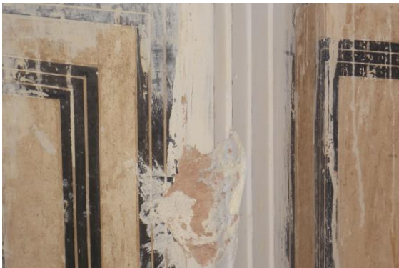
Photo 47 Peeling of Plaster on Wall No. 1 of Room No. 2 of First Floor
