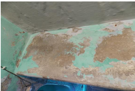
Photo 27 Peeling of Plaster on Wall No. 2 of Passage of First Floor
