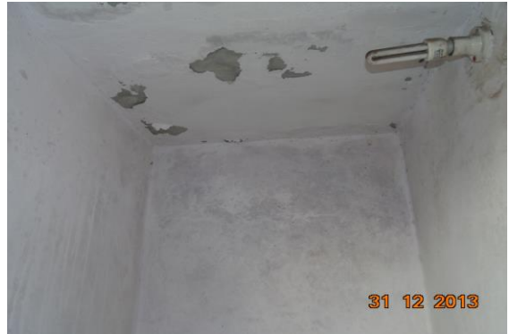
Photo 22 Dampness/Seepage on Wall No. 1, 4, 2 & Roof of Toilet No. 1 of Third Floor
