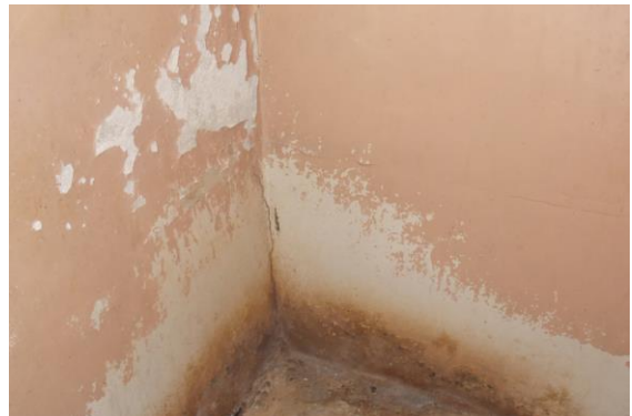
Photo 10 Dampness/Seepage on Wall No. 1 & 4 of Toilet No. 1 of First Floor
