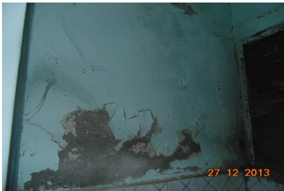
Photo 3 Dampness/Seepage on Wall No. 1 of Toilet No. 1 of House No.472, Second floor
