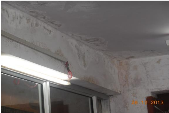
Photo 152 Dampness/Seepage on Wall No. 1 & 4 of Shop No. F 13 of First Floor
