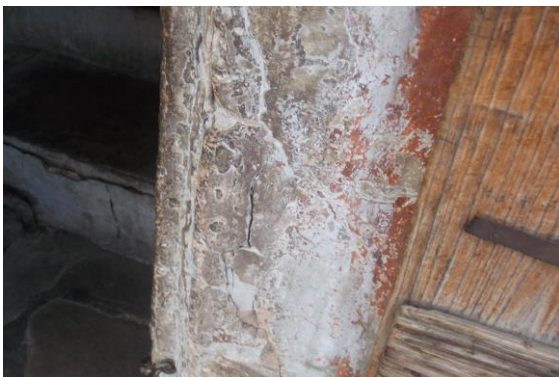
Photo 5 Vertical Crack on Wall No. 4 of Staircase GF to FF Approx. Width = 2.5mm, Approx. Length = 0.5m.
