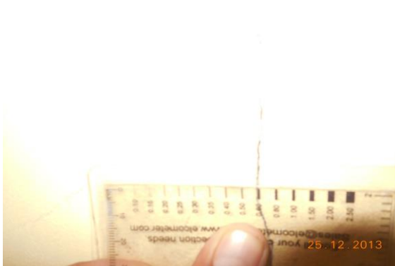
Photo 3A Inclined Crack on Wall No. 1 & 4 of Hall No. 1, First Floor Approx. Width = 0.6mm, Approx. Length = 2m. Distance from Corner Wall No.1 = 4m, Height from Floor = 0m.
