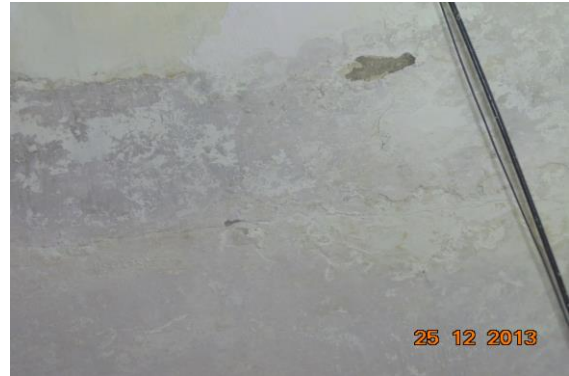
Photo 11 Horizontal Crack on Roof of Varanda, Shop No. 50, Ground Floor, Approx. Width = 0.6mm, Approx. Length = 2.5m. Distance from Right External Column = 0m, Height from Floor = 3m.
