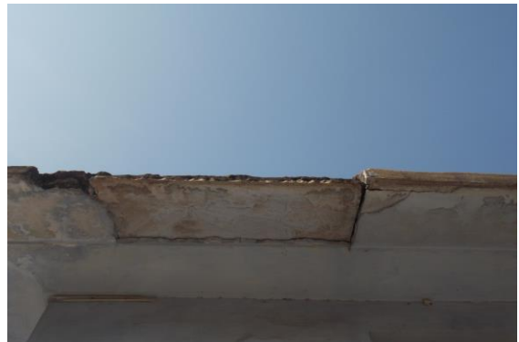
Photo 78 Peeling of Plaster on Wall No. 7 & Sun Shade of Open Sky of Second Floor
