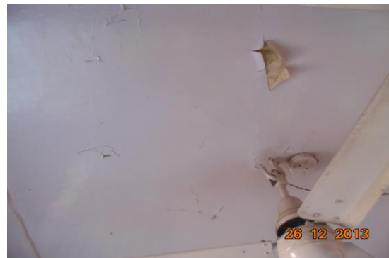
Photo 14 Peeling of Plaster on Roof of Lobby of Second Floor
