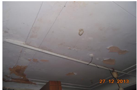
Photo 4 Peeling of Plaster on Roof of Lobby of House No.472 of Second floor
