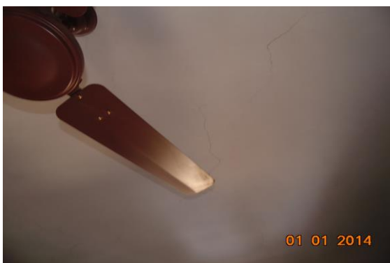
Photo 110 Plaster Crack on Roof of Third Floor
