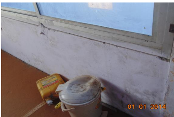
Photo 48 Dampness/Seepage on Wall No. 3 of Fourth Floor
