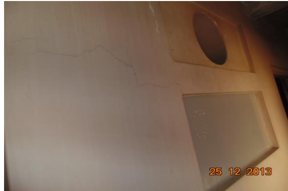
Photo 107 Plaster Crack on Wall No. 3 of Passage of House No. 347 Part A, Second Floor
