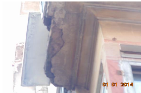
Photo 53 Peeling of Plaster on Back Side Shed of Second Floor
