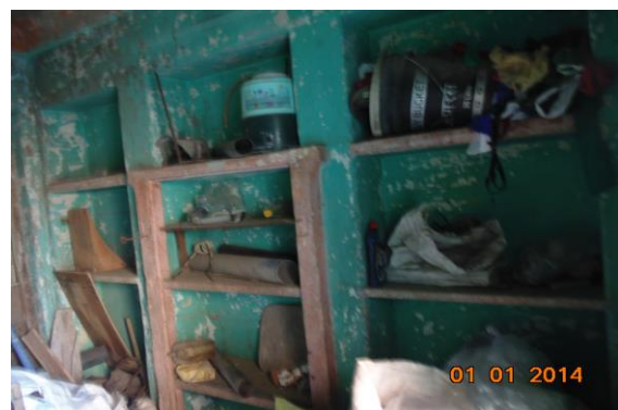
Photo 129 Dampness/Seepage on Wall No. 1 of Third Floor
