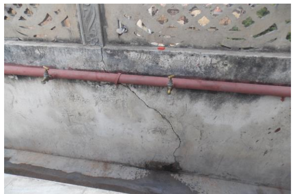
Photo 10 Inclined Crack on Wall No. 2 of Open Area, Third Floor Approx. Width = 2.5mm, Approx. Length = 1.2m. Distance from Wall No.4 = 3.5m, Height from Floor = 0m.
