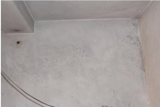
Photo 17 Dampness/Seepage on Wall No. 4 of Staircase FF to SF
