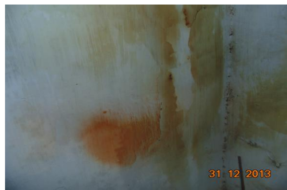
Photo 11 Dampness/Seepage on Wall No. 2 & 4 of Room No. 1 of Third Floor
