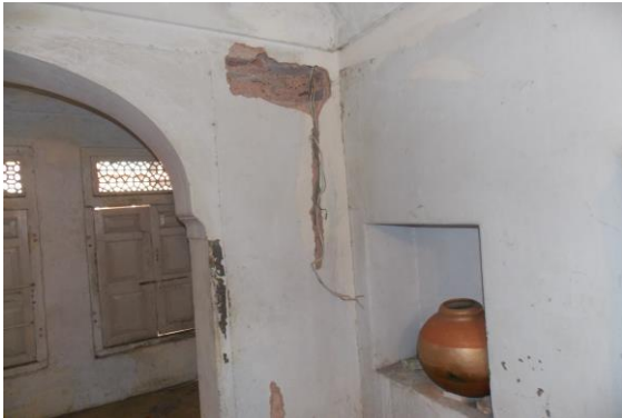
Photo 29 Peeling of Plaster on Wall No. 1 of Lobby of First Floor
