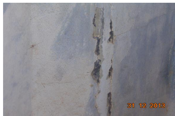
Photo 35 Peeling of Plaster on Wall No. 1 of Stair 5Th Floor To Terrace of Terrace
