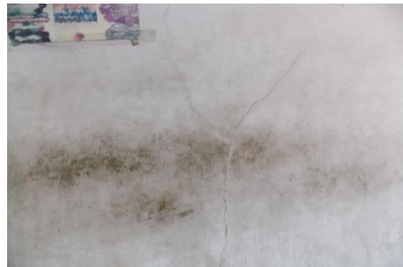
Photo 4 Inclined Crack on Wall No. 2 of Shop No. 84, Ground Floor Approx. Width = 0.3mm, Approx. Length = 2m. Distance from Wall No. 3 = 1.2m, Height from Floor = 0m.
