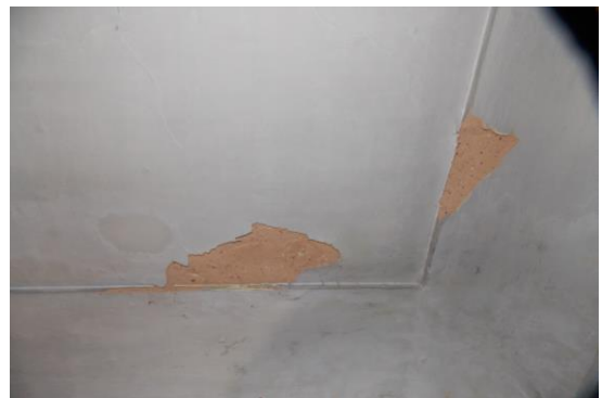
Photo 25 Peeling of Plaster on Roof of Room No. 2 of First Floor
