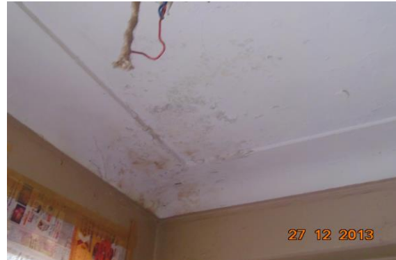
Photo 21 Dampness/Seepage on Roof of Balcony of Second Floor
