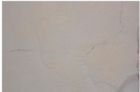
Photo 48 Peeling of Plaster on Wall No. 4 of Room No. 2 of First Floor
