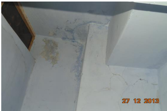
Photo 20 Inclined Crack on Wall No. 4 & Roof of Toilet No. 1, First Floor Approx. Width = 1mm, Approx. Length = 2m.
