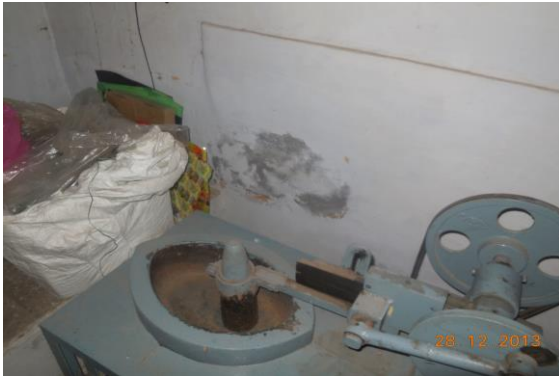
Photo 95 Dampness/Seepage on Wall No. 2 of Room No. 3 of Part A of Navjeevan Chikitsalaya, Ground Floor
