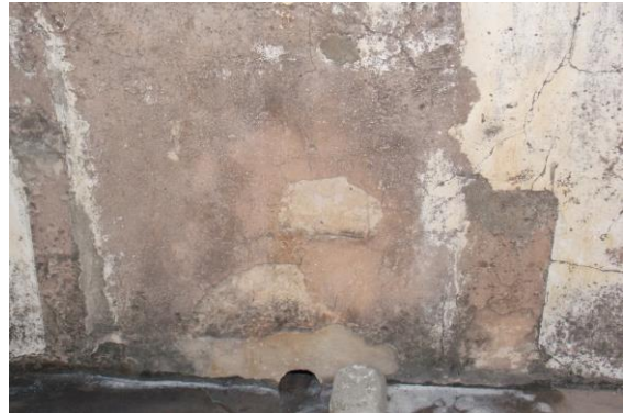
Photo 82 Damaged Portion on All Walls of H.No.287 of Terrace
