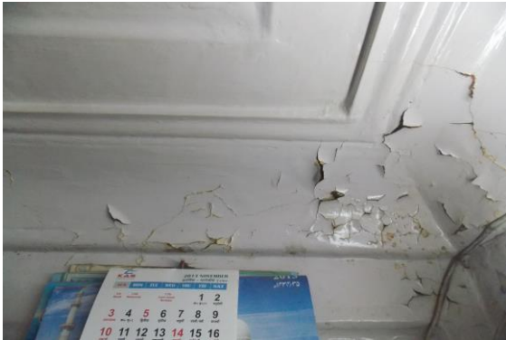
Photo 9 Peeling of Plaster on Wall No. 3 of Shop No.1 of Ground Floor
