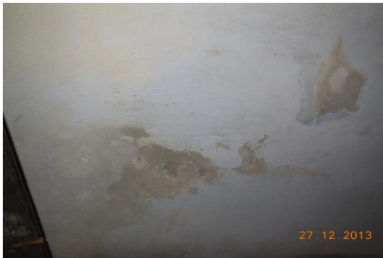
Photo 65 Peeling of Plaster on Wall No. 1 of Store of First Floor
