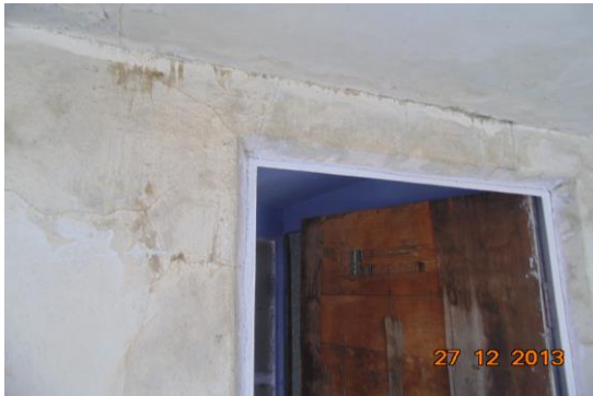
Photo 50 Dampness/Seepage on Wall No. 3 of Room No. 1 of Fifth Floor
