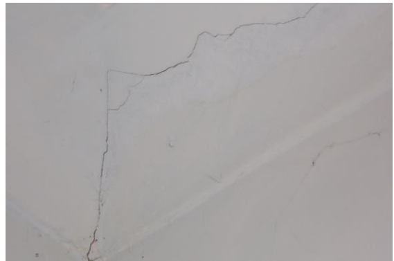
Photo 16 Inclined Crack on Wall No. 2, 4 & Roof of Room No. 2, First Floor Approx. Width = 0.8mm, Approx. Length = 1.2m. Distance from = Corner Wall no.2 & 4m, Height from Floor = 3m.
