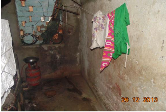
Photo 40 Dampness/Seepage on Wall No. 2 & 4 of Room No. 2 of Fourth Floor
