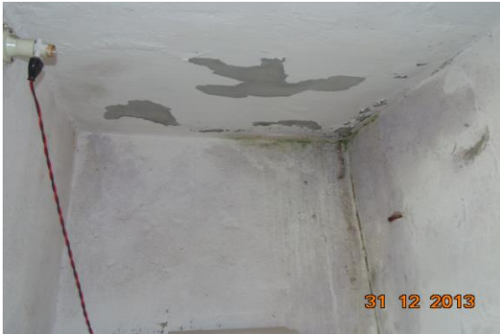
Photo 21 Dampness/Seepage on Wall No. 1, 2 & Roof of Bathroom No. 1 Third Floor
