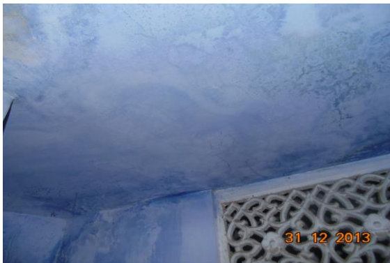
Photo 14 Dampness/Seepage on Roof of Stair TF to 4Th Floor
