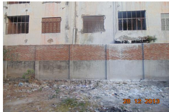
Photo 4 Peeling of Plaster on Wall No. 2 of Open Sky of House No. 61 of Ground Floor
