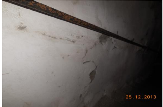
Photo 2 Vertical Crack on Wall No. 1 of Staircase Ground To First Floor Approx. Width = 1mm, Approx. Length = 1.5m. Distance from Wall No.4 = 0.9m, Height from Floor = 0m.
