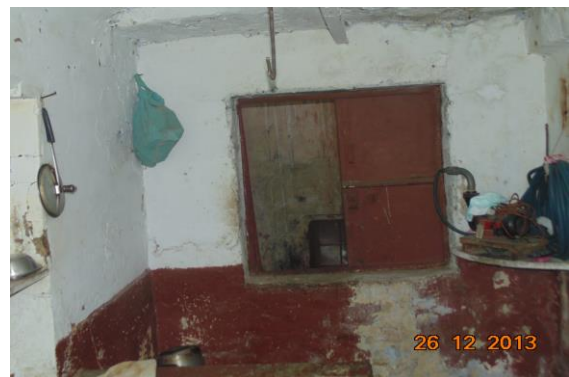
Photo 33 Dampness/Seepage on Wall No. 1, 2, 4 & Roof of Room No. 2 of Third Floor
