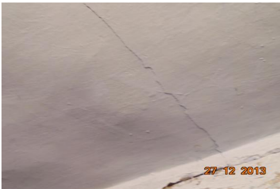
Photo 2A Horizontal Crack on Roof of Room No. 2, First Floor Approx. Width = 0.8mm, Approx. Length = 2m. Distance from Wall No.4 = 0m, Height from Floor = 2.1m.
