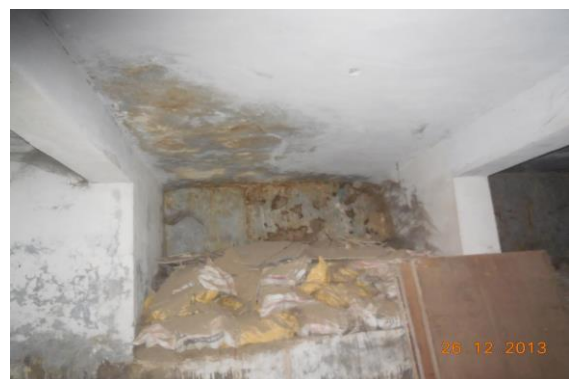
Photo 157 Dampness/Seepage on Wall No. 4 & Roof of Shopping Complex of Basement
