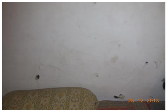
Photo 4 Horizontal Crack on Wall No. 3 of Room No. 2, First Floor Approx. Width = 0.3mm, Approx. Length = 0.7m. Distance from Wall No.1 = 0.85m, Height from Floor = 1.6m.
