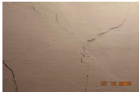
Photo 5 Inclined Crack on Wall No. 3 of Room No. 2, First Floor Approx. Width = 2mm, Approx. Length = 1m.
