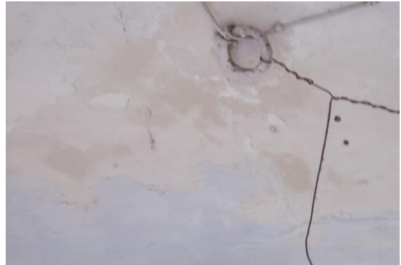
Photo 2 Peeling of Plaster on Roof of Varanda of Ground Floor
