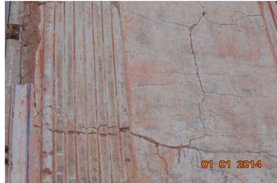
Photo 137 Peeling of Plaster on Outer Wall of SF External Façade
