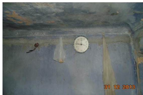
Photo 30 Peeling of Plaster on Wall No. 2 of Room No. 2 of Third Floor
