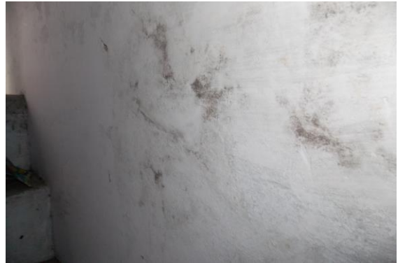
Photo 15 Dampness/Seepage on Wall No. 2 of Staircase SF to TF of Second Floor
