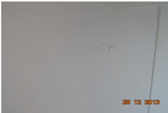
Photo 9 Peeling of Plaster on Room No. 2 of House No.289, First Floor
