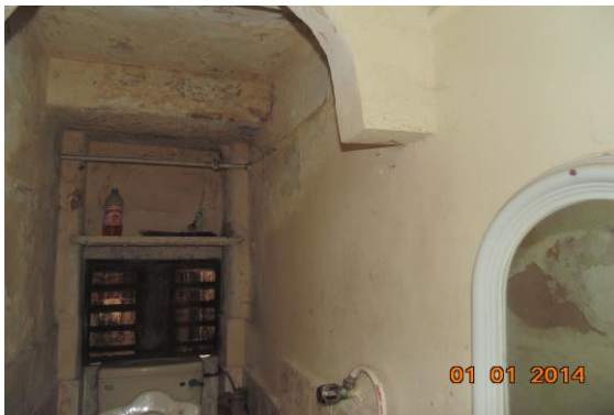
Photo 54 Dampness/Seepage on Wall No. 2 of First Floor
