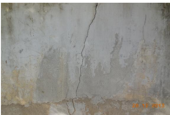
Photo 17 Inclined Crack on Wall No. 4 of Open Area 1 of Navjeevan Chikitsalaya, Ground Floor Approx. Width = 2mm, Approx. Length = 1.3m. Distance from Wall No.2 = 5m, Height from Floor = 1m.
