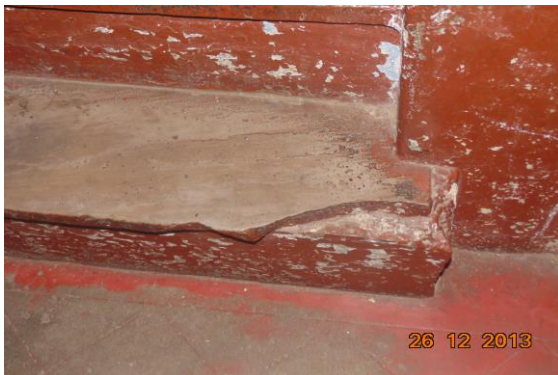
Photo 36 Damaged Portion on Steps of Staircase Area of Third Floor
