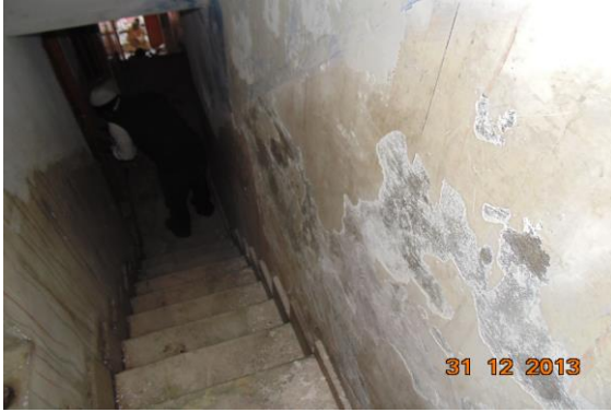
Photo 36 Dampness/Seepage on Wall No. 1 of Stair FF to SF
