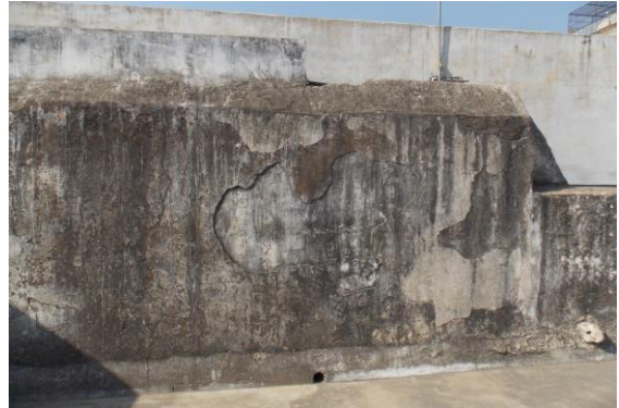
Photo 76 Peeling of Plaster on Wall No. 2 of Open Sky of Second Floor
