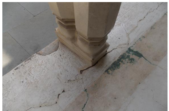
Photo 184 Plaster Crack on Floor of Varanda 12 of Navjeevan Chikitsalaya of First Floor
