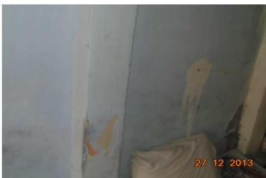
Photo 22 Inclined Crack on Wall No. 1 of Shop No.57, Ground Floor Approx. Width = 0.5mm, Approx. Length = 1m. Distance from = m, Height from Floor = m.
