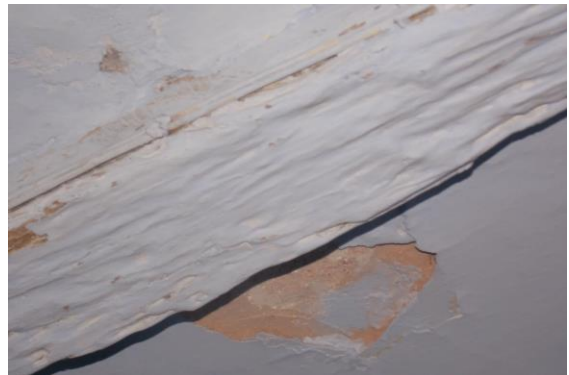
Photo 32 Peeling of Plaster on Roof of Room No. 2 of Second Floor
