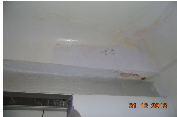
Photo 42 Dampness/Seepage on Wall No. 1 & Roof of First Floor
