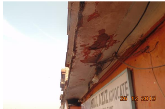
Photo 20 Peeling of Plaster on Shade of Gallery of First Floor
