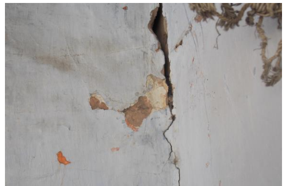
Photo 6 Vertical Crack on Wall No. 2 & 3 of Open area, Third Floor Approx. Width = 20mm, Approx. Length = 2.5m. Height from Floor = 0m.
