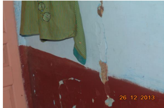
Photo 31 Peeling of Plaster on Wall No. 2 of Room No. 1 of Third Floor
