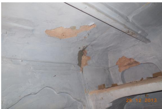
Photo 36 Peeling of Plaster on Wall No. 3 & Roof of Room No. 1 of Second Floor
