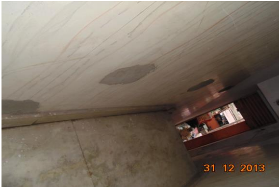
Photo 38 Peeling of Plaster on Wall No. 2 of Stair GF to FF
