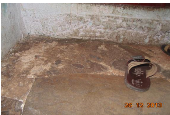
Photo 26 Peeling of Plaster on Steps of Staircase FF to SF of First Floor
