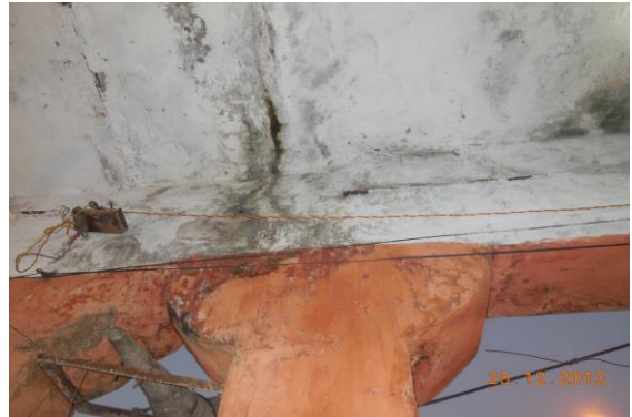
Photo 60 Dampness/Seepage on Roof of Shop No.34 of Ground Floor
