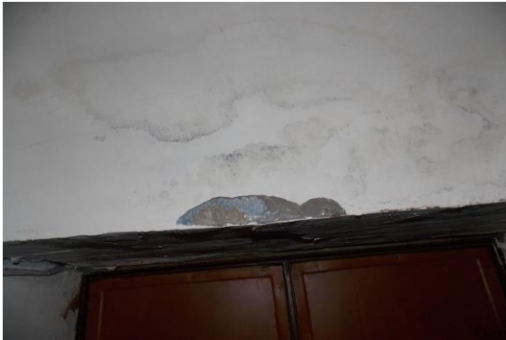
Photo 40 Peeling of Plaster on Wall No. 3 of Lobby of Ground Floor
