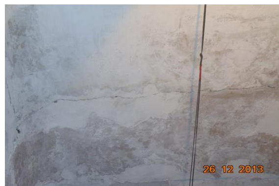
Photo 6 Horizontal Crack on Roof of Varanda, Shop No. 60, Ground Floor, Approx. Width = 2mm, Approx. Length = 2.5m. Distance from Left side External Column = 0m, Height from Floor = 3m.
