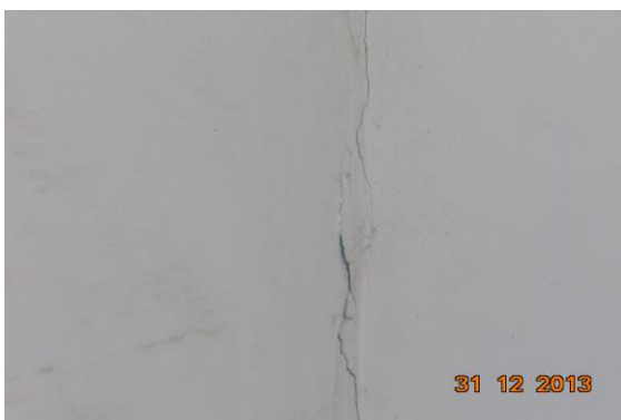
Photo 17 Peeling of Plaster on Wall No. 2 & 4 of Room No. 2 of Second Floor
