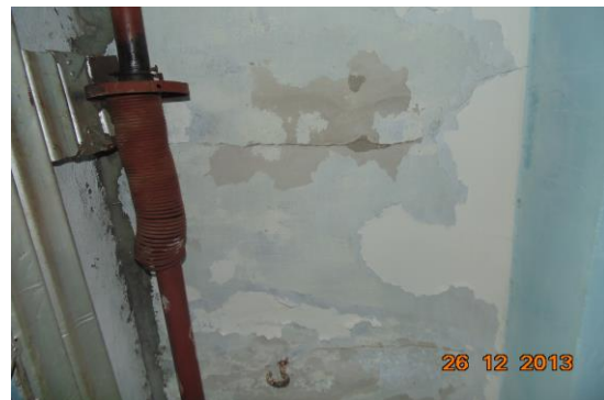
Photo 37 Dampness/Seepage on Roof of Bathroom of Third Floor
