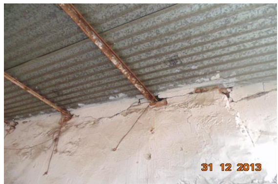
Photo 24 Peeling of Plaster on Room No. 1 of Third Floor
