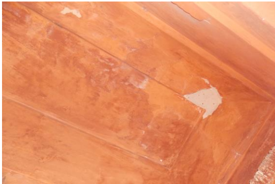
Photo 40 Peeling of Plaster on Roof of Balcony of Second Floor
