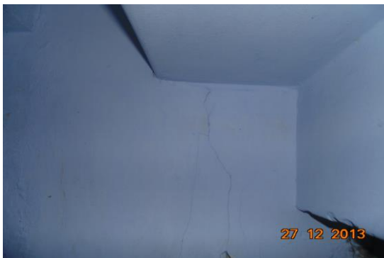
Photo 28 Peeling of Plaster on Wall No. 4 of Bathroom of First Floor
