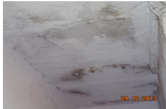
Photo 19 Dampness/Seepage on Roof of Toilet No. 1 of House No. 339, Third Floor
