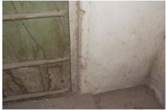
Photo 168 Peeling of Plaster on Wall No. 4 of Room No. 15 of Navjeevan Chikitsalaya, First Floor
