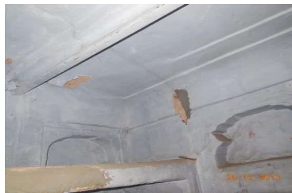
Photo 37 Peeling of Plaster on Wall No. 4 & Roof of Room No. 1 of Second Floor
