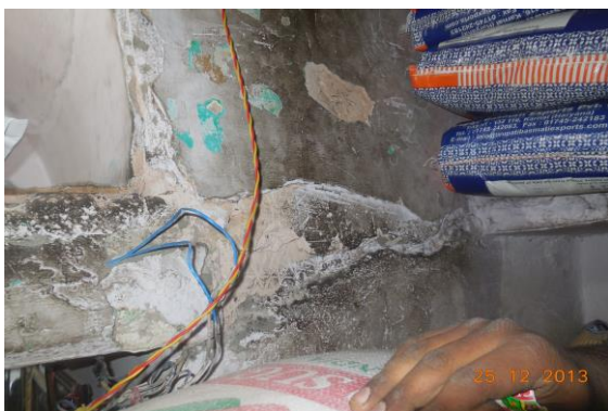
Photo 5 Peeling of Plaster on Wall No. 3 of Part-II of Shop No.32 of Ground Floor
