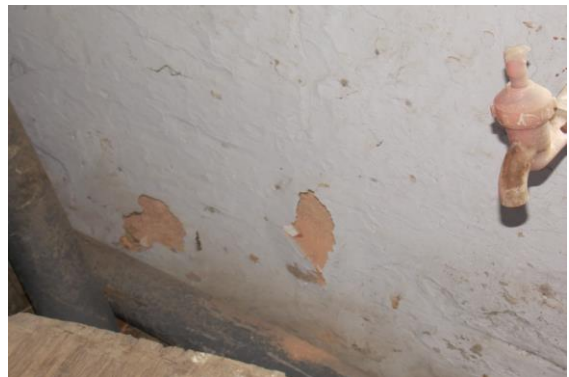
Photo 17 Peeling of Plaster on Wall No. 4 of Room No. 1 of Above Shop No. 74, Third Floor
