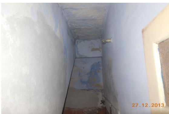
Photo 75 Dampness/Seepage on All walls of Toilet No. 2 of Second Floor
