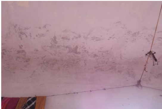
Photo 16 Dampness/Seepage on Roof of Varanda of Shop of Ground Floor
