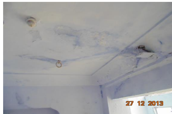
Photo 29 Dampness/Seepage on Roof of Room No. 1 of Second Floor
