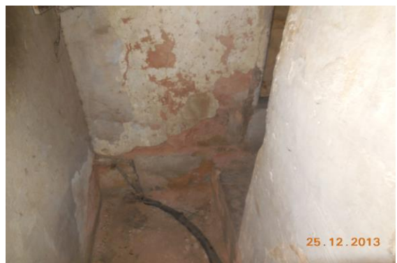
Photo 31 Dampness/Seepage on Staircase First Floor to Second Floor
