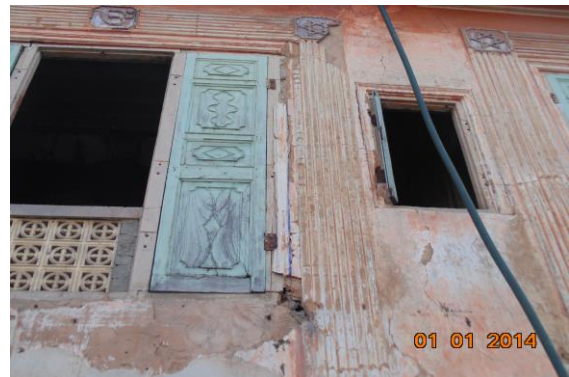
Photo 139 Peeling of Plaster on Outer Wall of SF External Façade
