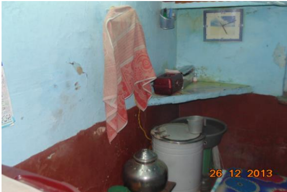
Photo 30 Peeling of Plaster on Wall No. 1 & 4 of Room No. 1 of Third Floor
