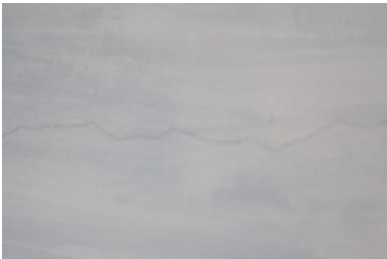
Photo 71 Peeling of Plaster on Roof of Hall No. 2 of Second Floor
