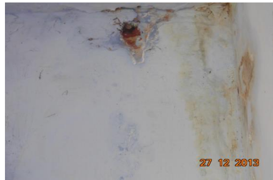
Photo 33 Dampness/Seepage on Wall No. 2 of Room No. 1 of Second Floor
