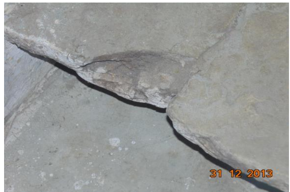
Photo 26 Damaged Portion on Stair Step of Second Floor
