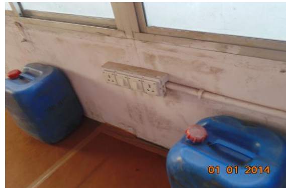
Photo 47 Dampness/Seepage on Wall No. 3 of Fourth Floor
