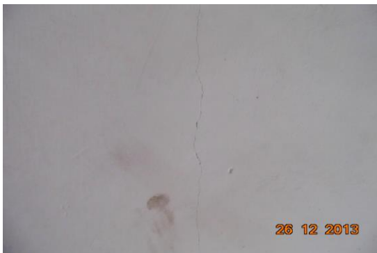
Photo 18 Vertical Crack on Wall No. 2 of Staircase FF to SF, First Floor Approx. Width = 0.5mm, Approx. Length = 2m.
