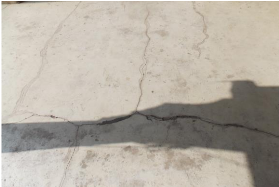
Photo 181 Plaster Crack on Floor of Varanda 10 of Navjeevan Chikitsalaya of First Floor
