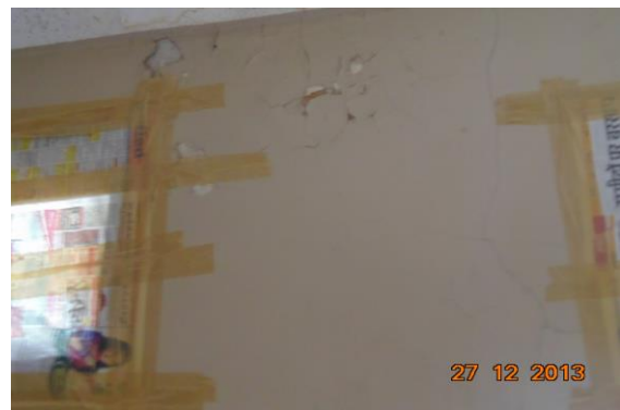
Photo 23 Dampness/Seepage on Wall No. 4 of Balcony of Second Floor
