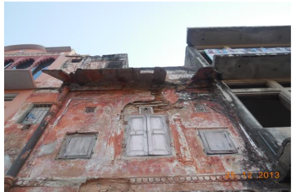
Photo 27 Peeling of Plaster on Shade of Part-II of First Floor
