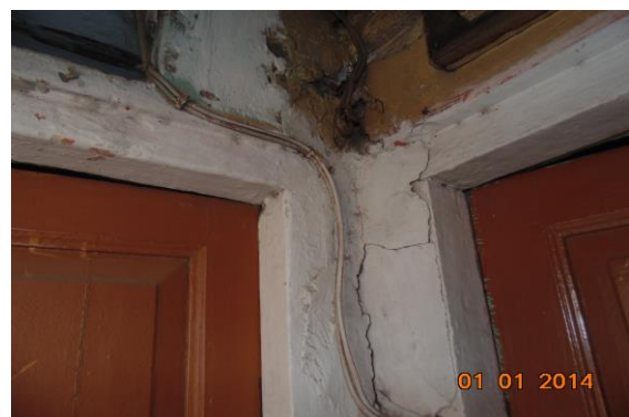
Photo 93 Peeling of Plaster on Wall No. 4 of Third Floor
