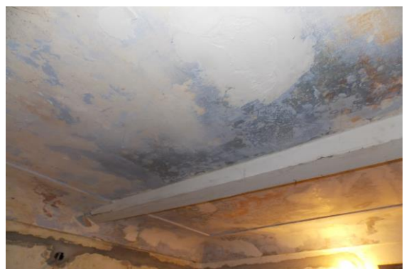
Photo 34 Dampness/Seepage on Roof of Room No. 1 of First Floor
