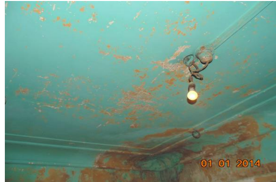
Photo 59 Dampness/Seepage on Roof of Toilet No. 1 of Second Floor
