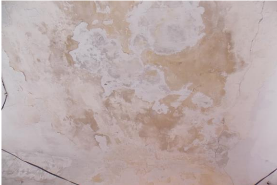
Photo 22 Dampness/Seepage on Roof of Varanda of Ground Floor
