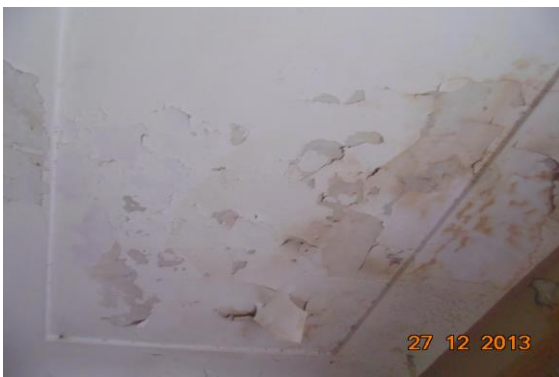
Photo 22 Dampness/Seepage on Roof of Balcony of Second Floor
