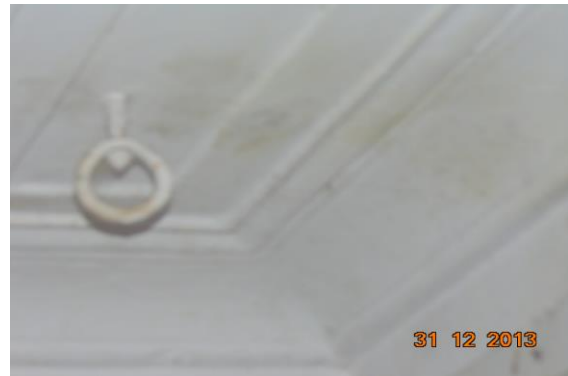
Photo 14 Dampness/Seepage on Roof of Varanda of Second Floor
