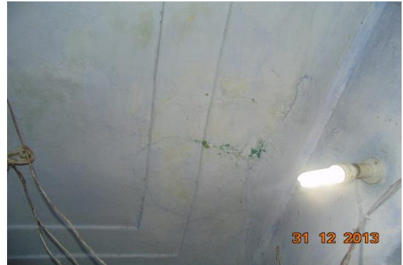
Photo 19 Peeling of Plaster on Roof of Room No. 1 of First Floor
