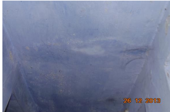
Photo 8 Dampness/Seepage on Roof of Passage of First Floor
