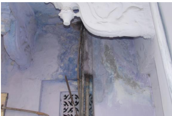
Photo 44 Dampness/Seepage on Wall No. 2 of Balcony of First Floor
