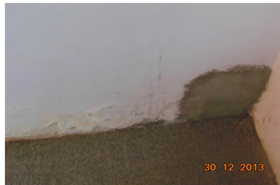
Photo 4 Peeling of Plaster on Wall No. 2 of Room No. 2 of House No. 329 First Floor
