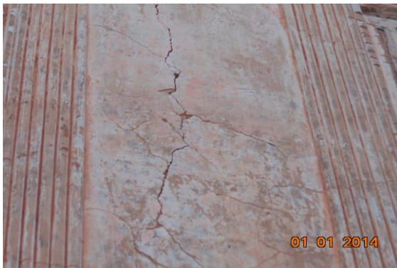
Photo 138 Peeling of Plaster on Outer Wall of SF External Façade
