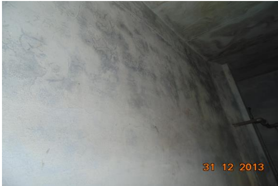
Photo 30 Dampness/Seepage on Wall No. 1 of Fifth Floor
