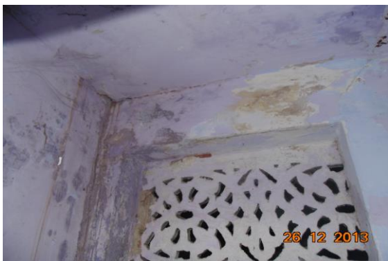
Photo 11 Dampness/Seepage on Wall No. 4 & Roof of Passage of Second Floor
