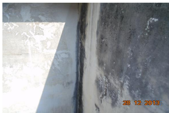
Photo 12 Dampness/Seepage on Wall No. 1 & 3 of Staircase FF-Terrace of House No.289 of First Floor
