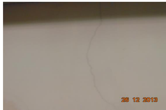
Photo 10 Inclined Crack on Wall No. 2 of Hall No. 1, Second Floor Approx. Width = 0.3mm, Approx. Length = 1m.
