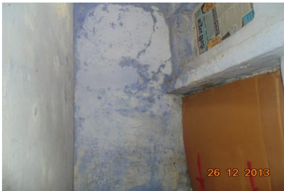
Photo 9 Dampness/Seepage on Wall No. 1 of Passage of First Floor
