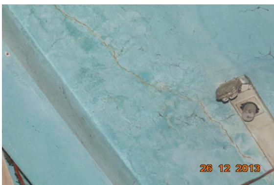
Photo 5 Inclined Crack on Roof of Shop No.59, Ground Floor Approx. Width = 0.3mm, Approx. Length = 2m.
