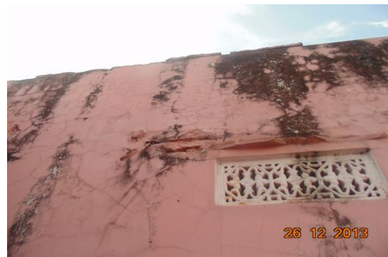
Photo 20 Peeling of Plaster on Wall No. 4 & Shade of Open Sky of External Façade
