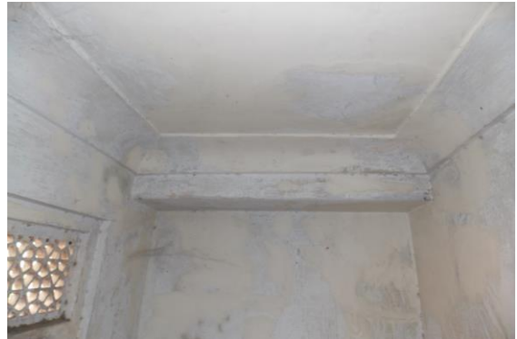
Photo 26 Dampness/Seepage on Wall No. 2, 3 & 4 of Varanda of First Floor
