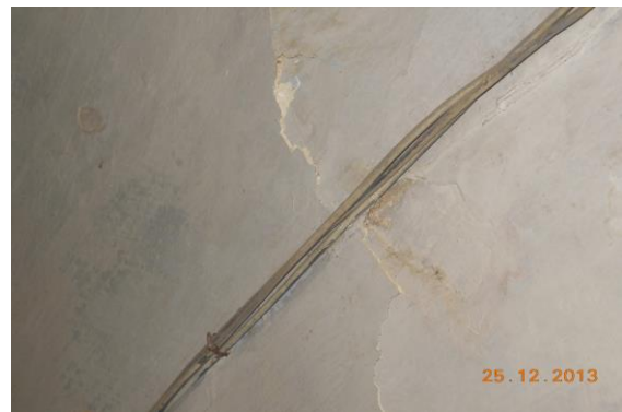
Photo 35 Peeling of Plaster on Wall No. 1 of Room No. 1 of Second Floor
