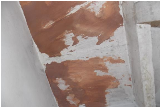
Photo 19 Peeling of Plaster on Roof of Staircase Area of Second Floor
