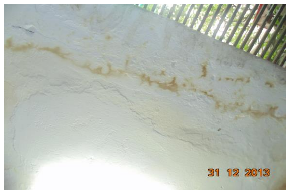
Photo 28 Dampness/Seepage on Wall No. 1 of Lobby of Second Floor
