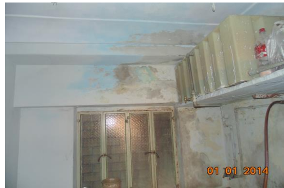
Photo 31 Dampness/Seepage on Roof & Wall No. 4 of Hall No. 1 of First Floor
