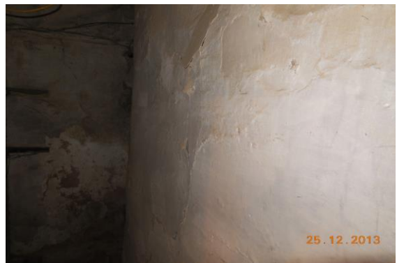
Photo 29 Peeling of Plaster on Wall No. 3 of Passage of First Floor
