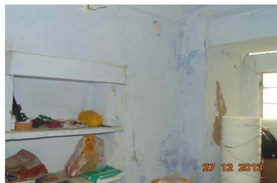
Photo 25 Dampness/Seepage on Wall No. 4 of Hall No. 1 of First Floor
