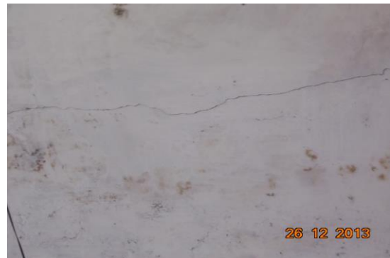
Photo 11 Horizontal Crack on Roof of Varanda of Shop No. 35, Ground Floor Approx. Width = 3mm, Approx. Length = 2.5m. Distance from Right side External Column = 0m, Height from Floor = 3m.
