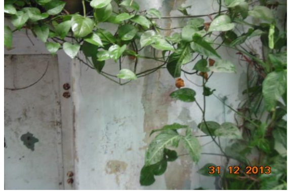
Photo 12 Peeling of Plaster on Wall No. 4 of Third Floor
