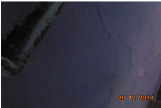
Photo 10 Inclined Crack on Wall No. 2 of Staircase GF to FF, Approx. Width = 1mm, Approx. Length = 1m.
