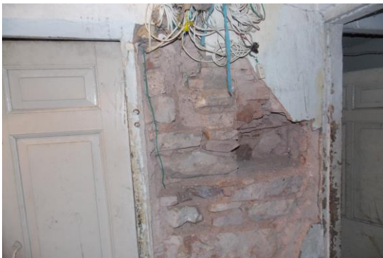
Photo 31 Peeling of Plaster on Wall No. 2 of Lobby of First Floor
