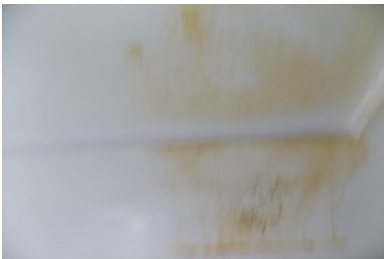
Photo 11 Dampness/Seepage on Wall No. 3 & Roof of Room No. 1 of Second Floor
