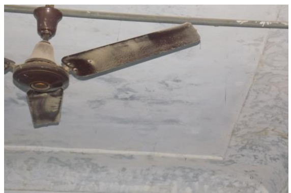
Photo 12 Dampness/Seepage on Roof of Shop No.4, Part C of Ground Floor
