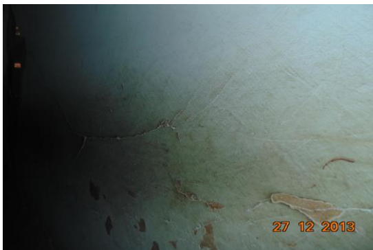
Photo 52 Peeling of Plaster on Staircase FF to SF
