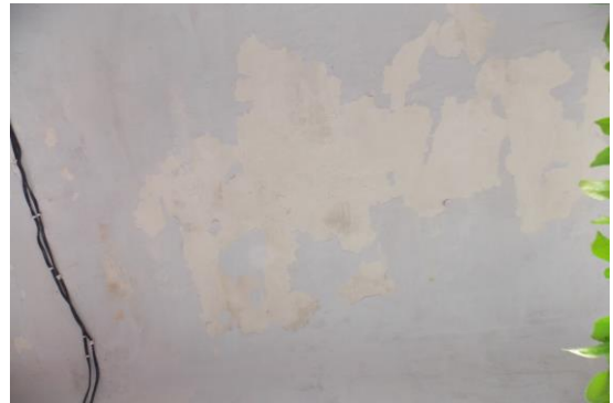
Photo 17 Peeling of Plaster on Roof of Varanda of Shop of Ground Floor
