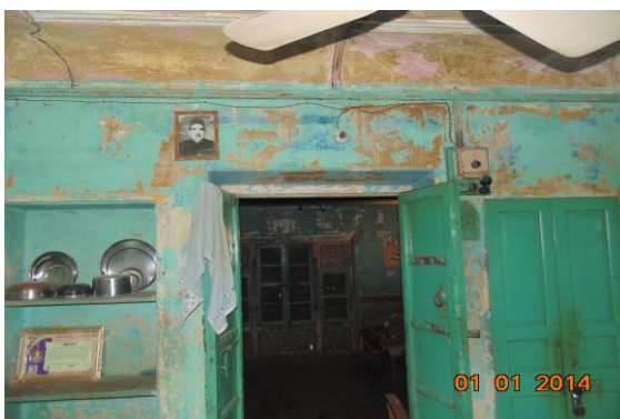
Photo 68 Dampness/Seepage on Wall No. 3 of Second Floor
