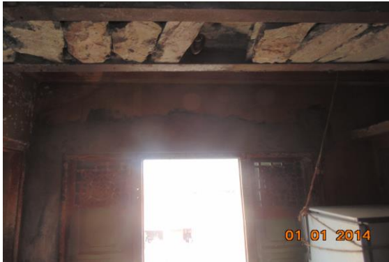
Photo 58 Peeling of Plaster on Wall No. 1 of Second Floor
