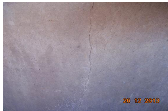
Photo 4 Inclined Crack on Wall No. 4 of Lobby, First Floor Approx. Width = 0.25mm, Approx. Length = 0.7m. Distance from Wall No.1 = 1.5m, Height from Floor = 0.05m.
