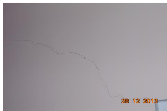
Photo 6 Inclined Crack on Wall No. 4 of Room No. 5, H.No.284,First floor Approx. Width = 0.5mm, Approx. Length = 1.2m. Distance from Wall No.1 = 1.6m, Height from Floor = 17m.
