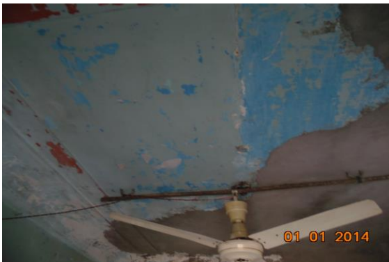
Photo 120 Dampness/Seepage on Roof of Third Floor
