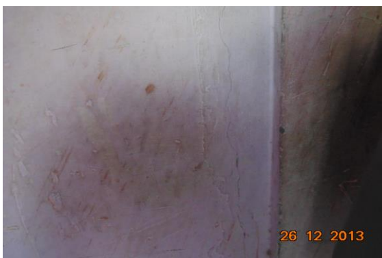
Photo 27 Peeling of Plaster on Wall No. 4 of Staircase Area of First Floor
