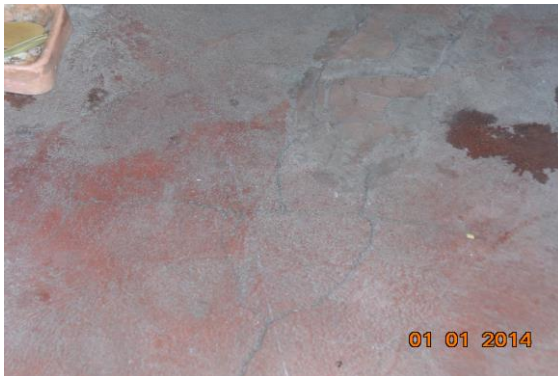
Photo 94 Plaster Crack on Floor of Bathroom No. 1 of Third Floor
