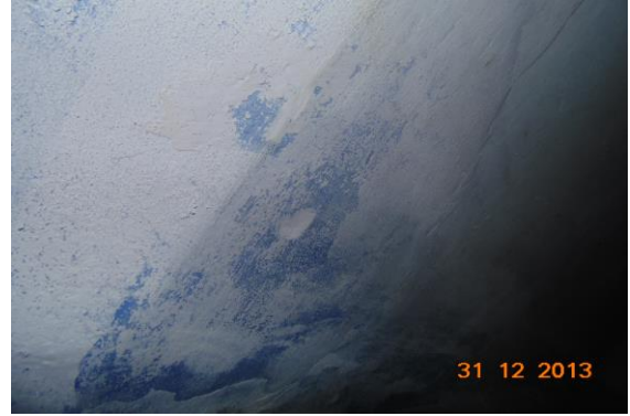
Photo 37 Dampness/Seepage on Roof of Terrace
