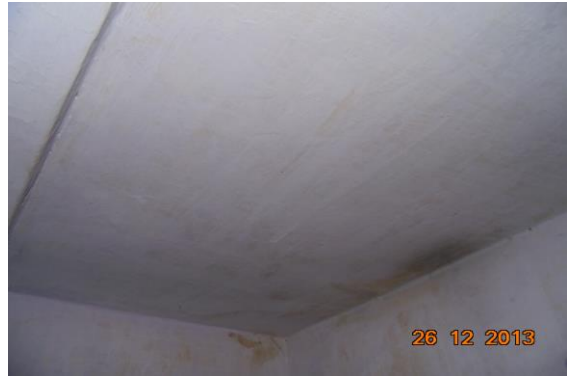
Photo 14 Dampness/Seepage on Wall No. 2 of Room No. 1 of Third Floor
