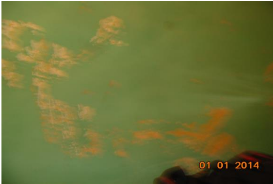
Photo 118 Peeling of Plaster on Wall No. 1 of Third Floor
