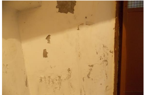
Photo 41 Peeling of Plaster on Wall No. 5 of Lobby of Ground Floor
