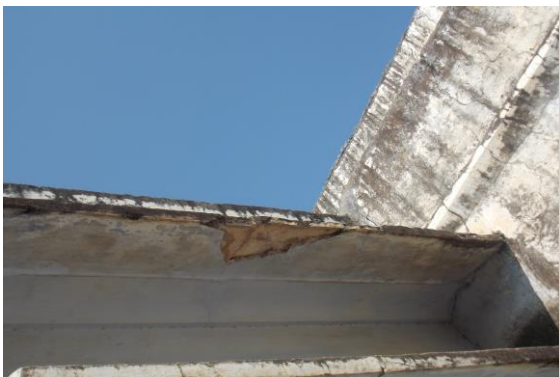
Photo 79 Peeling of Plaster on Wall No. 7 & Sun Shade of Open Sky of Second Floor
