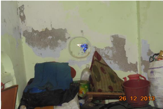
Photo 27 Dampness/Seepage on Wall No. 2 of Varanda of Second Floor
