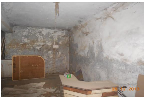
Photo 156 Dampness/Seepage on Wall No. 4 of Shopping Complex of Basement
