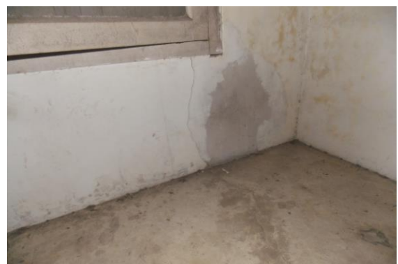
Photo 5 Inclined Crack on Floor & Wall No. 4 of Varandah, Second Floor, Approx. Width = 1mm, Approx. Length = 1.3m. Distance from Wall No. 2 = 0.8m, Height from Floor = 0m.
