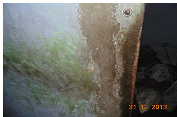
Photo 17 Dampness/Seepage on Wall No. 4, 2 & Roof of Toilet No. 1 of First Floor
