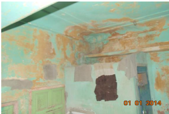
Photo 60 Dampness/Seepage on Wall No. 1 & 4 of Second Floor
