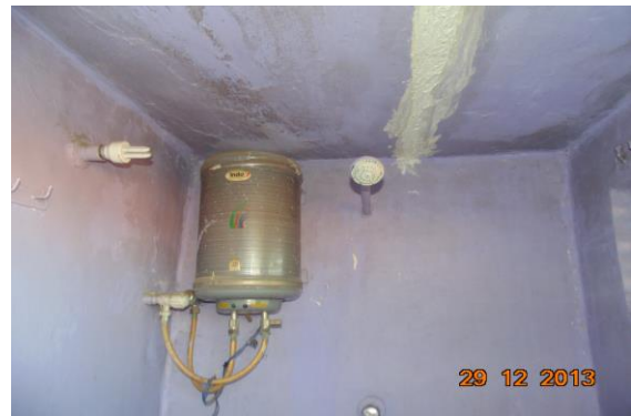
Photo 21 Dampness/Seepage on Wall No. 1 & Roof of Bathroom of House No. 339, Third Floor
