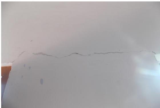
Photo 9 Horizontal Crack on Wall No. 1 of Room No. 1, Fourth Floor, Approx. Width = 0.35mm, Approx. Length = 0.6m. Distance from Wall No. 1 = 1m, Height from Floor = 2.7m.
