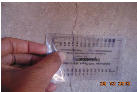
Photo 4A Inclined Crack on Wall No. 4 of Lobby, First Floor Approx. Width = 0.25mm, Approx. Length = 0.7m. Distance from Wall No.1 = 1.5m, Height from Floor = 0.05m.
