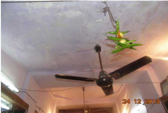
Photo 6 Dampness/Seepage on Roof of Shop No.23 of Ground Floor
