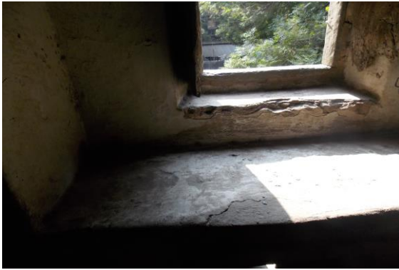
Photo 167 Peeling of Plaster on Wall No. 1 of Room No. 15 of Navjeevan Chikitsalaya, First Floor
