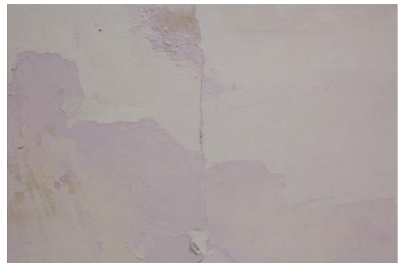
Photo 6 Horizontal Crack on Roof of Varanda of Shop No.73, Ground Floor Approx. Width = 0.25mm, Approx. Length = 2.5m. Height from Floor = 3m.
