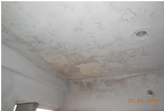
Photo 95 Dampness/Seepage on Wall No. 1 & Roof of Store No.2 of Terrace
