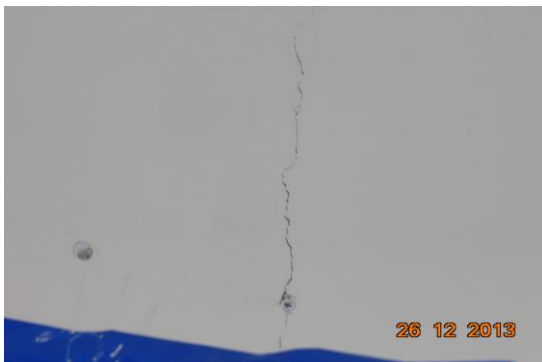
Photo 22 Inclined Crack on Wall No. 1 of Shop No.57, Ground Floor Approx. Width = 0.5mm, Approx. Length = 1m. Distance from = m, Height from Floor = m.
