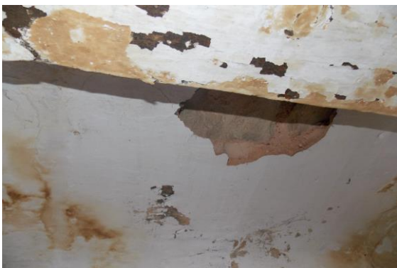
Photo 18 Dampness/Seepage on Roof of Room No. 1 of Above Shop No. 74, Third Floor
