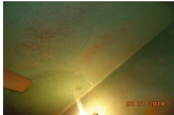
Photo 113 Plaster Crack on Roof of Room No. 2 of Third Floor
