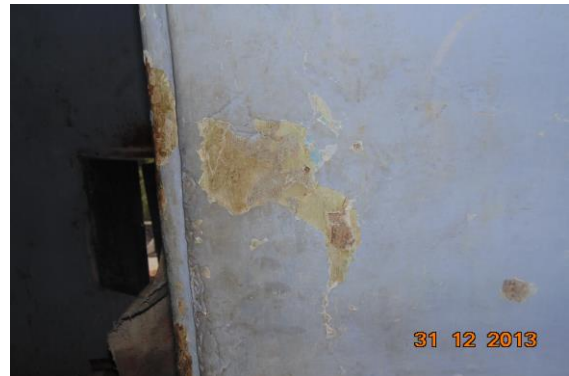
Photo 7 Peeling of Plaster on Wall No. 4 of Toilet No. 1 of Second Floor
