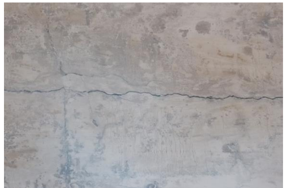
Photo 16 Vertical Crack on External Column of Varanda, Shop No. 93, Ground Floor, Approx. Width = 0.8mm, Approx. Length = 3.5m. Distance from External Column = 0m, Height from Floor = 0m.
