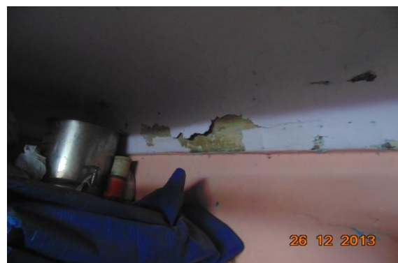
Photo 27 Peeling of Plaster on Roof of Lobby of Second Floor
