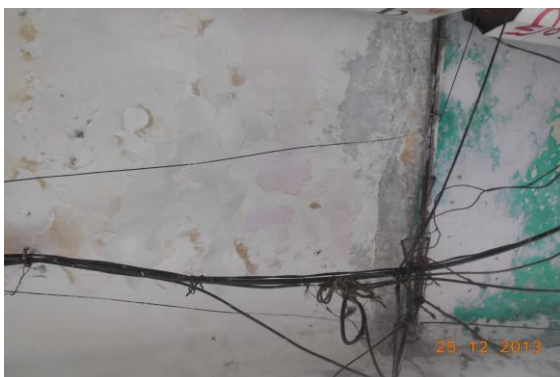
Photo 3 Inclined Crack on Backside & Leftside External Column of Shop No.31, Ground Floor Approx. Width = 0.8mm, Approx. Length = 0.8m. Distance from Leftside External Column = Backside Height from Floor
