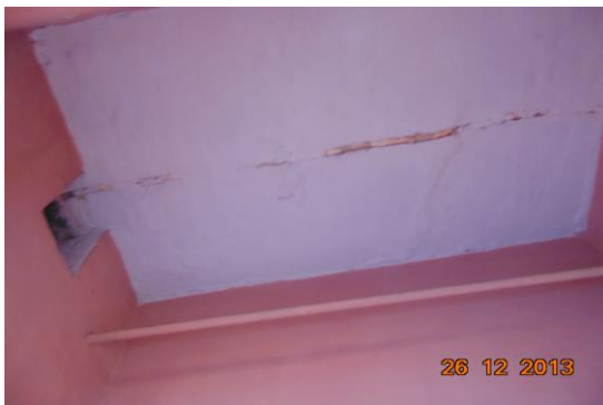
Photo 19 Peeling of Plaster on Roof of Toilet No. 1 of External Façade
