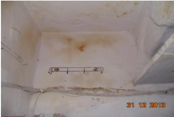
Photo 31 Dampness/Seepage on Wall No. 4 & Roof of Bathroom of Second Floor
