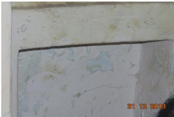
Photo 15 Dampness/Seepage on Wall No. 1 of Second Floor
