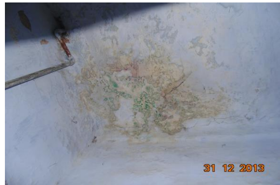
Photo 9 Peeling of Plaster on Wall No. 4 of Third Floor
