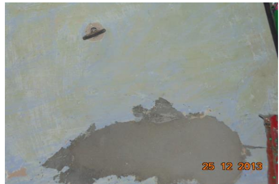
Photo 28 Peeling of Plaster on Roof of Shop No. 55 of Ground Floor
