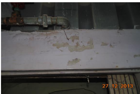
Photo 5 Peeling of Plaster on Wall No. 3 of Lobby of House No.472 of Second floor
