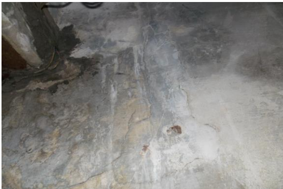
Photo 25 Damaged Portion on Wall No. 1 of Staircase GF to FF
