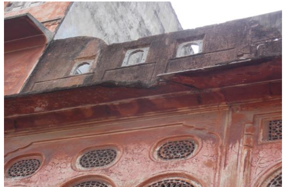
Photo 54 Damaged Portion on Outerwall Sun Shade of Second Floor
