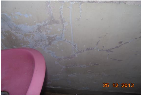
Photo 106 Plaster Crack on Wall No. 4 of Passage of House No. 347 Part A, Second Floor
