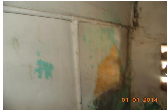
Photo 97 Dampness/Seepage on Wall No. 1 & 4 of Third Floor
