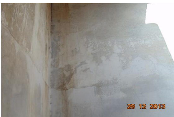
Photo 11 Dampness/Seepage on Wall No. 1 & 4 of Staircase FF-Terrace of House No.289 of First Floor
