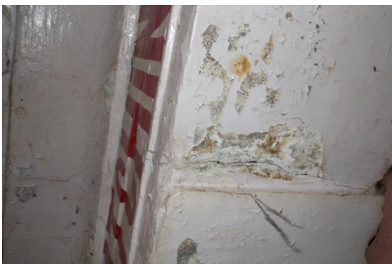
Photo 11 Plaster Crack on Roof of Shop No.1 of Ground Floor
