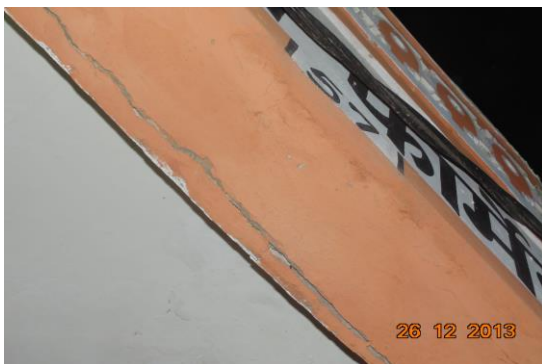
Photo 54 Peeling of Plaster on Beam of Varanda of Shop No.57, Ground Floor
