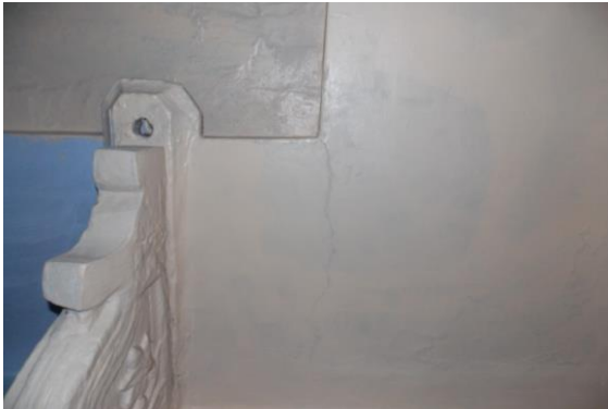
Photo 13 Peeling of Plaster on Roof of Open Sky of First Floor
