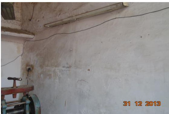
Photo 23 Dampness/Seepage on Wall No. 4 of Room No. 1 of Third Floor
