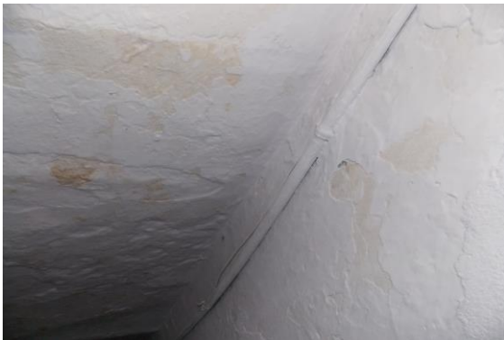
Photo 20 Peeling of Plaster on Wall No. 1 & Roof of Staircase GF to FF
