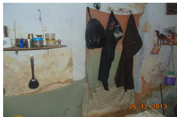
Photo 10 Inclined Crack on Wall No. 1 of Kitchen, First Floor Approx. Width = 2mm, Approx. Length = 2m. Distance from = m, Height from Floor = m.
