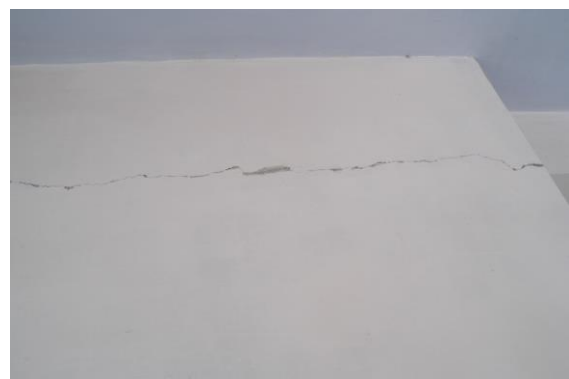
Photo 24 Horizontal Crack on Wall No. 1 of Room No. 1, Part B of House No. 347, Fourth Floor, Approx. Width = 0.4mm, Approx. Length = 1.3m. Distance from Wall No. 4 = 0.6m, Height from Floor = 2.1m.
