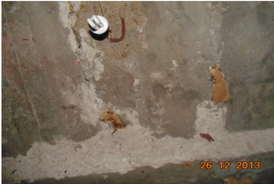
Photo 42 Peeling of Plaster on Roof of Room No. 2 of Fourth Floor
