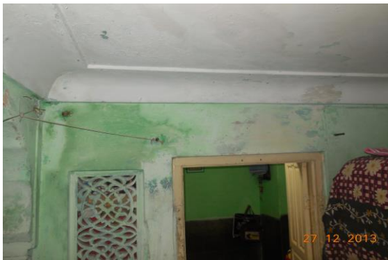
Photo 67 Dampness/Seepage on Wall No. 1 of Varanda No.1 of First Floor
