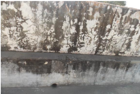
Photo 77 Peeling of Plaster on Wall No. 4 of Open Sky of Second Floor
