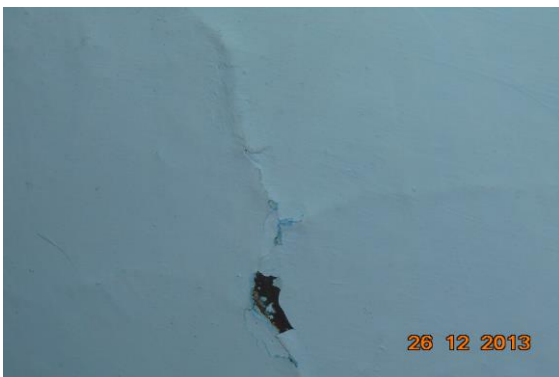
Photo 32 Peeling of Plaster on Roof of Room No. 1 of Third Floor
