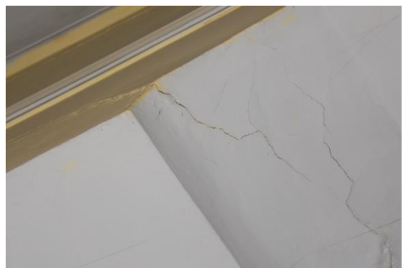
Photo 12 Inclined Crack on Roof of Varanda, First Floor Approx. Width = 2mm, Approx. Length = 1m. Distance from Wall No.3 = 0.8m, Height from Floor = 3m.
