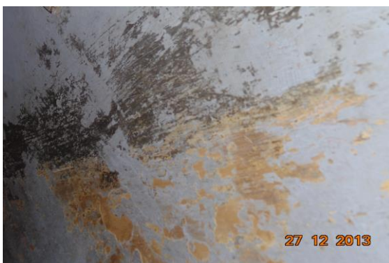
Photo 5 Dampness/Seepage on Wall No. 1 of Staircase GF to FF of Ground Floor
