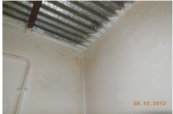
Photo 96 Dampness/Seepage on Wall No. 1 & 3 of Room No. 4 of Part A of Navjeevan Chikitsalaya, Ground Floor
