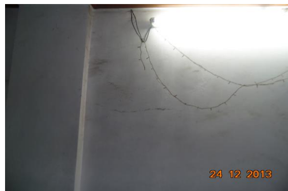
Photo 6 Dampness/Seepage on Wall No. 3 of Room No. 1 of Second Floor
