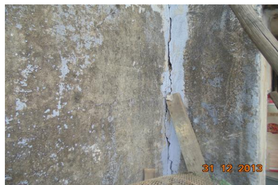
Photo 5 Vertical Crack on Wall No. 5 of Open Area, Terrace, Approx. Width = 5mm, Approx. Length = 2m. Distance from = m, Height from Floor = m.
