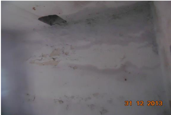
Photo 13 Dampness/Seepage on Roof of Toilet No. 1 of Third Floor
