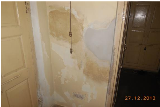
Photo 73 Dampness/Seepage on Wall No. 1 of Room No. 1 of Second Floor
