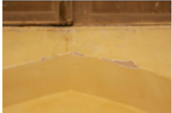
Photo 46 Peeling of Plaster on Wall No. 4 of Room No. 3 of First Floor
