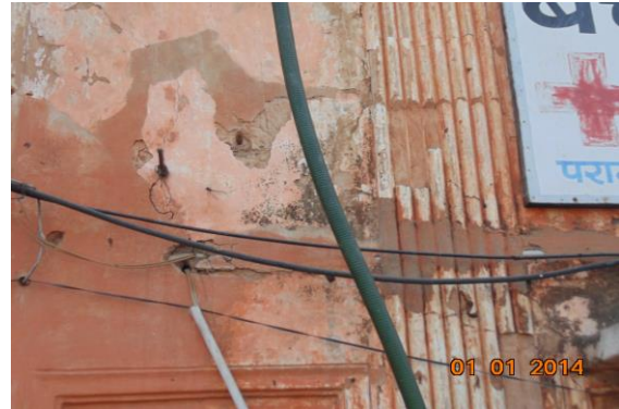
Photo 143 Peeling of Plaster on Outer Wall of FF External Façade
