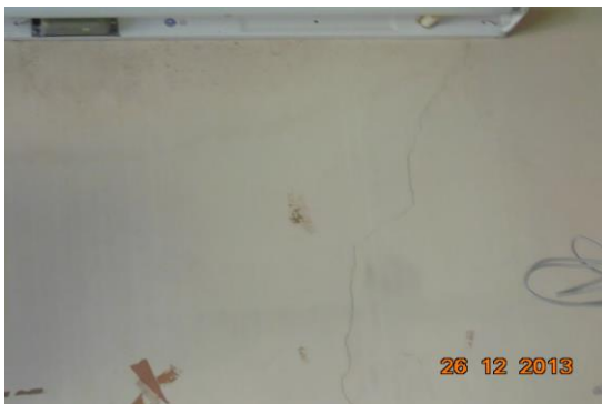
Photo 9 Inclined Crack on Wall No. 4 of Hall No. 1, Second Floor Approx. Width = 0.3mm, Approx. Length = 1m.
