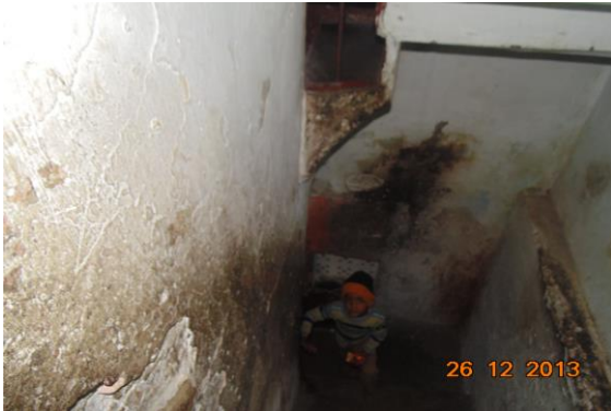
Photo 28 Dampness/Seepage on Wall No. 2, 3 & 4 of Staircase SF to TF of Second Floor
