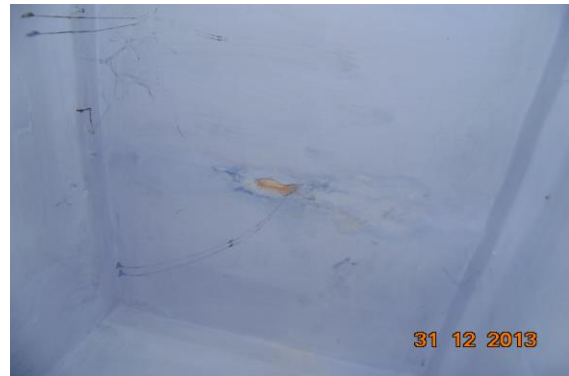
Photo 13 Peeling of Plaster on Stair Step SF to TF of
