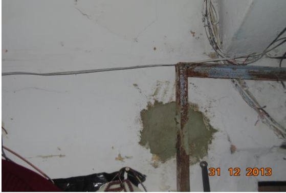
Photo 29 Peeling of Plaster on Wall No. 3 of Second Floor
