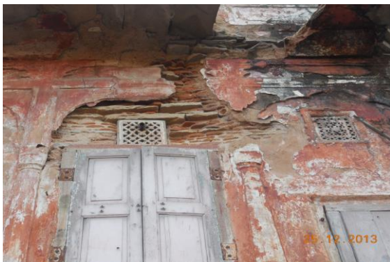
Photo 28 Peeling of Plaster on Outer Wall of Part-II of First Floor
