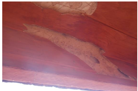
Photo 43 Peeling of Plaster on Wall No. 4 of Balcony of Second Floor
