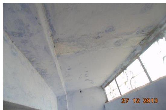
Photo 31 Peeling of Plaster on Roof of Room No. 1 of Second Floor
