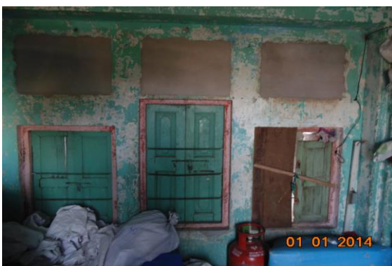
Photo 122 Dampness/Seepage on Roof & Wall No. 4 of Room No. 4 of Third Floor
