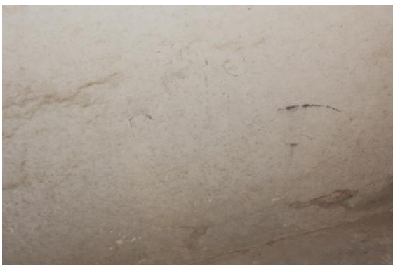
Photo 171 Peeling of Plaster on Wall No. 2 of Room No. 16 of Navjeevan Chikitsalaya, First Floor
