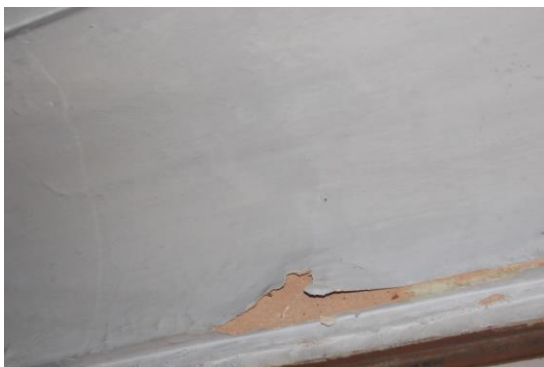
Photo 26 Peeling of Plaster on Wall No. 2 of Room No. 2 of First Floor
