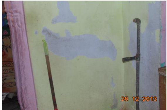
Photo 26 Peeling of Plaster on Wall No. 1 & 4 of Lobby of Second Floor
