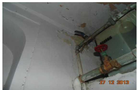
Photo 6 Dampness/Seepage on Wall No. 2 of Lobby of House No.472 of Second floor
