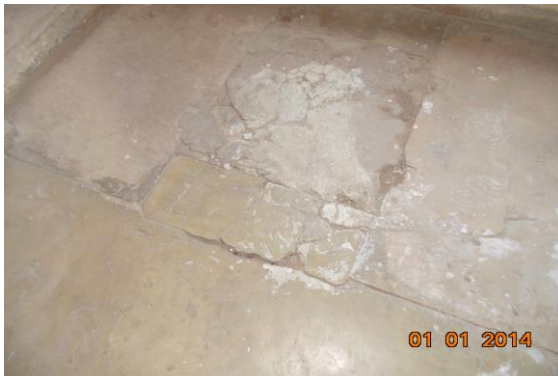
Photo 82 Peeling of Plaster on Floor of Lobby Wall No.1 of Second Floor
