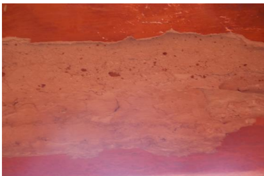
Photo 44 Peeling of Plaster on Wall No. 4 of Balcony of Second Floor
