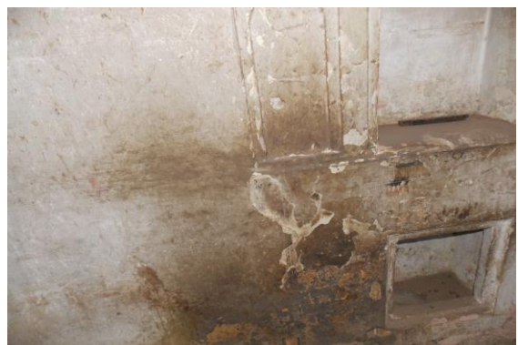
Photo 34 Peeling of Plaster on Wall No. 1 of Room No. 4 of Second Floor
