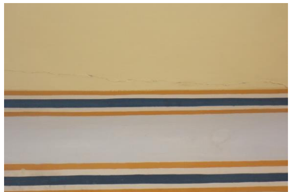
Photo 18 Horizontal Crack on Roof of Varanda No.3, First Floor Approx. Width = 1mm, Approx. Length = 1.5m. Distance from Wall No.3 = 0.3m, Height from Floor = 4m.
