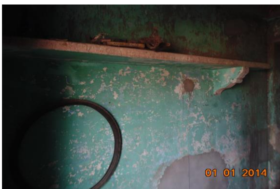
Photo 128 Dampness/Seepage on Roof & Wall No. 4 of Room No. 5 of Third Floor
