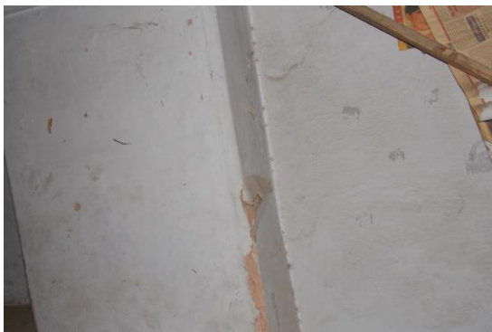
Photo 24 Peeling of Plaster on Wall No. 4 of Room No. 2 of First Floor
