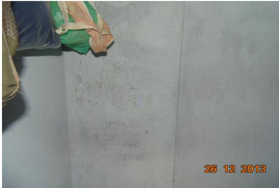
Photo 22 Dampness/Seepage on Wall No. 4 of Room No. 1 of First Floor
