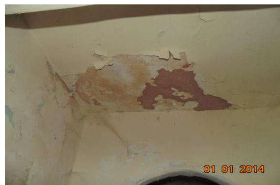
Photo 51 Dampness/Seepage on Roof of Toilet No. 1 of First Floor
