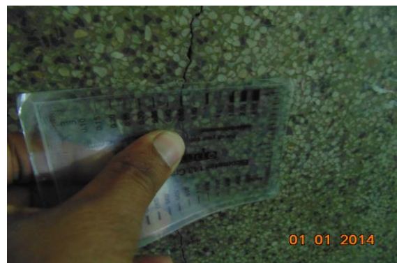
Photo 10A Inclined Crack on Wall No. 4 of House No. 458, First Floor Approx. Width = 0.4mm, Approx. Length = 1.5m. Distance from Wall No. 1 = 0.6m, Height from Floor = 0m.
