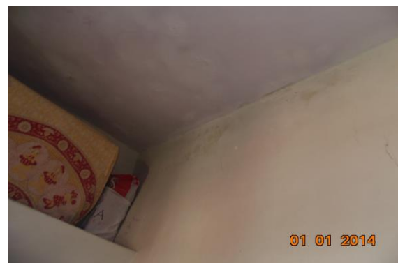
Photo 111 Dampness/Seepage on Wall No. 1 of Third Floor
