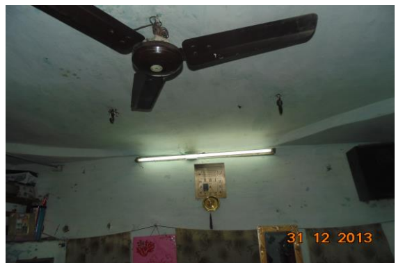
Photo 34 Dampness/Seepage on Wall No. 4 & Roof of Room No. 1 of Second Floor
