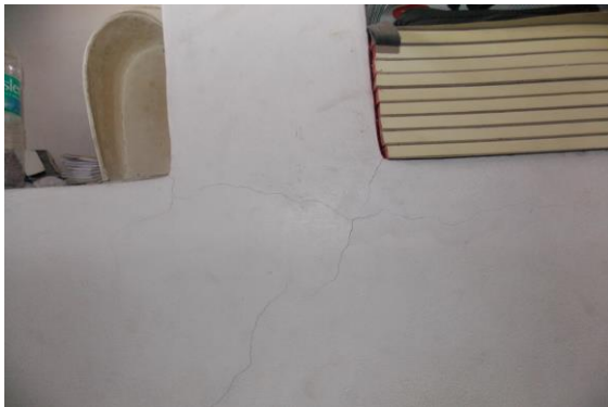
Photo 3 Inclined Crack on Wall No. 4 of Room No. 1, First Floor Approx. Width = 0.1mm, Approx. Length = 2m.
