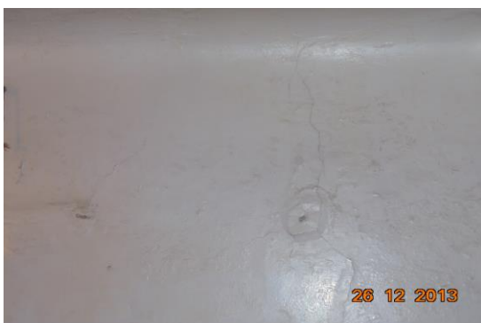
Photo 21 Peeling of Plaster on Wall No. 2 of Room No. 1 of External Façade
