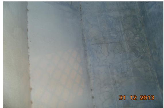
Photo 27 Dampness/Seepage on Wall No. 1 of Fifth Floor
