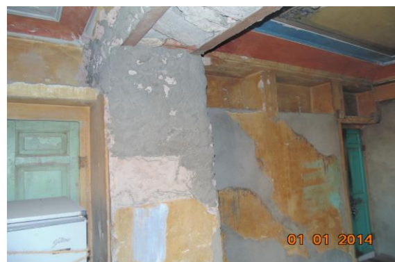
Photo 57 Peeling of Plaster on Wall No. 4 of Second Floor
