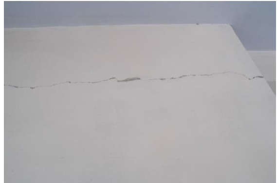
Photo 8 Horizontal Crack on Wall No. 1 of Room No. 1, Fourth Floor, Approx. Width = 0.4mm, Approx. Length = 1.3m. Distance from Wall No. 4 = 0.6m, Height from Floor = 2.1m.
