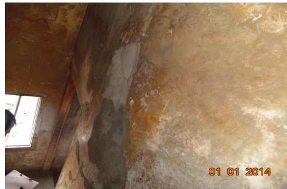
Photo 91 Damaged Portion on Wall No. 3 of Third Floor
