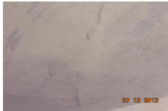
Photo 3 Inclined Crack on Roof of Room No. 2, First Floor Approx. Width = 0.5mm, Approx. Length = 2m.
