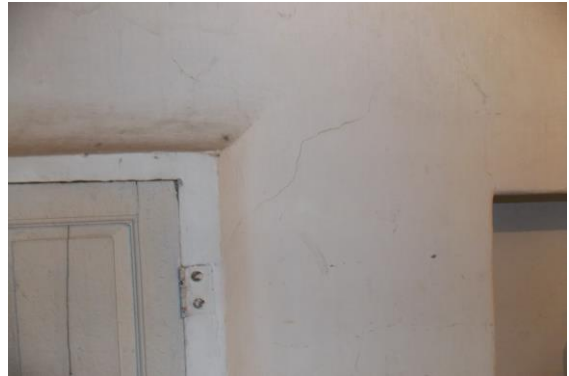
Photo 30 Plaster Crack on Wall No. 4 of Lobby of First Floor
