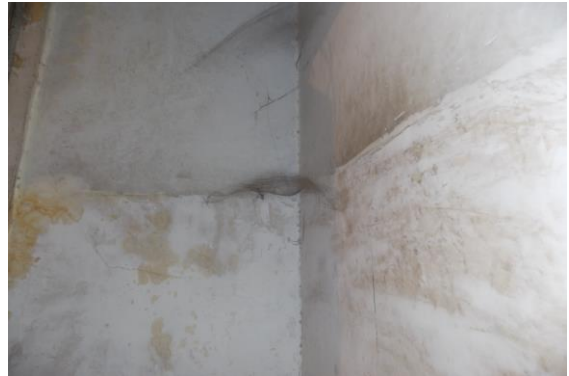
Photo 24 Dampness/Seepage on Wall No. 1 & 4 of Stair FF to SF of Second Floor
