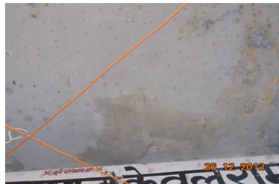
Photo 26 Peeling of Plaster on Roof of Varanda of Shop No.41, Ground Floor
