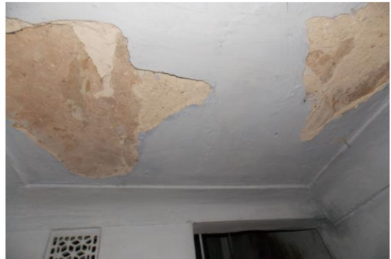
Photo 24 Peeling of Plaster on Roof of Lobby of First Floor
