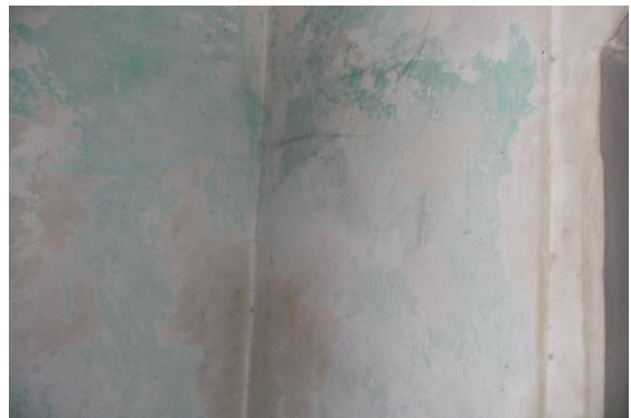
Photo 14 Peeling of Plaster on Wall No. 2 & 3 of Varanda of Second Floor
