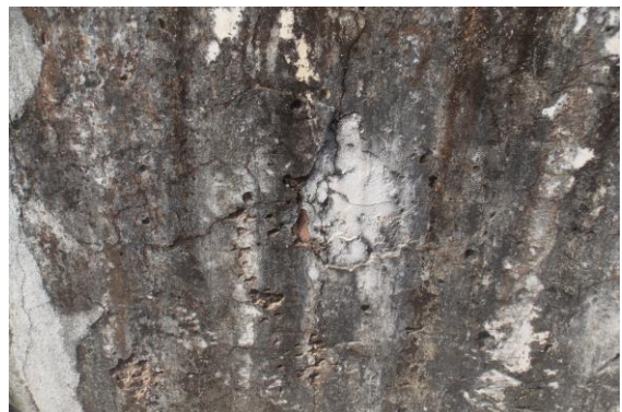
Photo 74 Peeling of Plaster on Wall No. 2 of Open Sky of Second Floor
