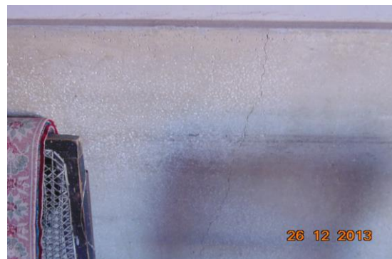
Photo 5 Inclined Crack on Wall No. 4 of Lobby, Second Floor Approx. Width = 0.35mm, Approx. Length = 1m. Distance from Wall No.1 = 1.5m, Height from Floor = 0m.
