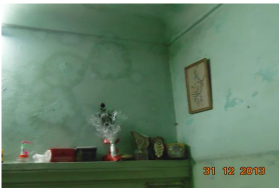
Photo 15 Dampness/Seepage on Wall No. 2 of Room No. 1 of Third Floor
