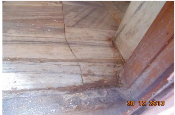
Photo 14 Damaged Portion on Floor of Temple of Ground Floor
