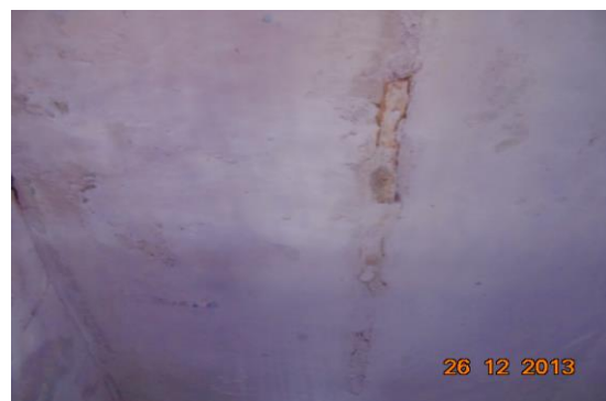
Photo 15 Dampness/Seepage on Roof of Kitchen of Third Floor
