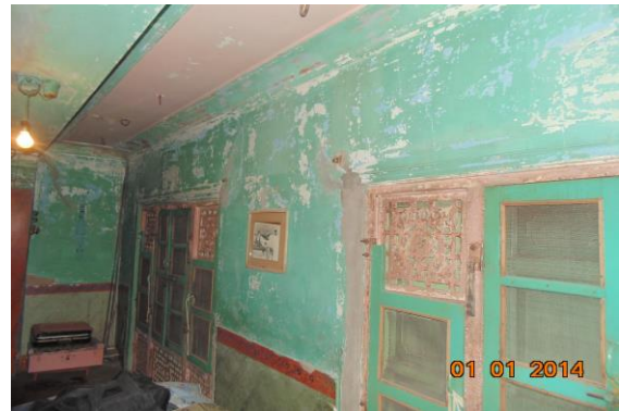
Photo 77 Peeling of Plaster on Wall No. 1 of Second Floor
