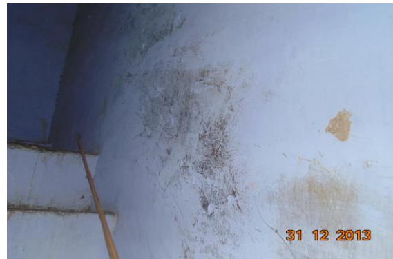
Photo 15 Dampness/Seepage on Wall No. 1, 2 & 3 of Stair FF to SF
