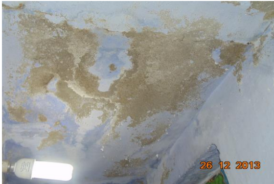
Photo 7 Dampness/Seepage on Roof of Passage of First Floor
