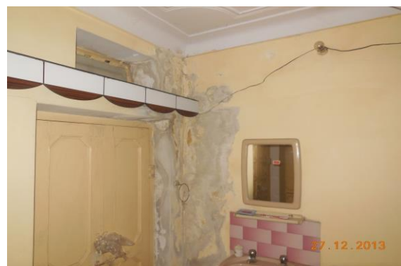
Photo 76 Dampness/Seepage on Wall No. 1 & 3 of Room No. 4 of Second Floor
