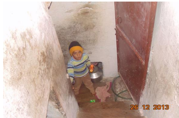
Photo 37 Dampness/Seepage on Wall No. 1, 3 & 4 of Staircase Area TF to Fourth of Third Floor
