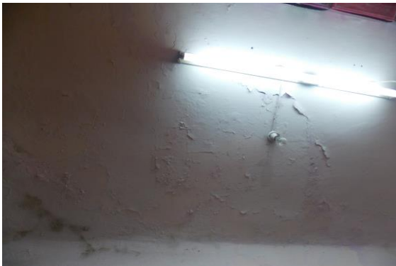
Photo 26 Peeling of Plaster on Roof of Varanda of Shop No.72 of Ground Floor
