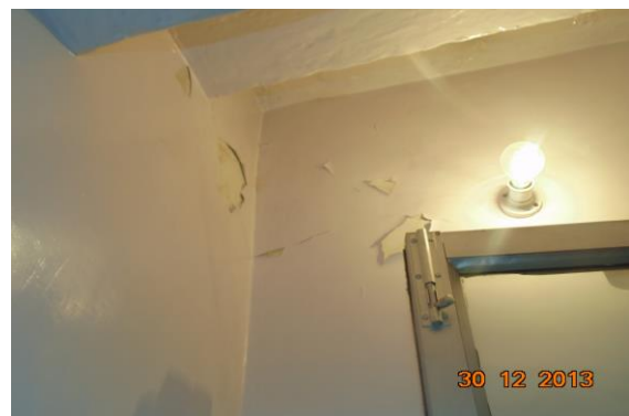
Photo 6 Peeling of Plaster on Wall No. 1 & 4 of Stair SF to TF of House No. 329
