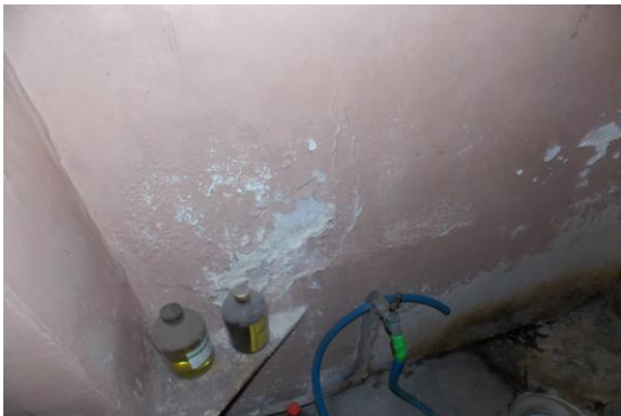
Photo 9 Dampness/Seepage on Wall No. 1 of Toilet No. 1 of First Floor
