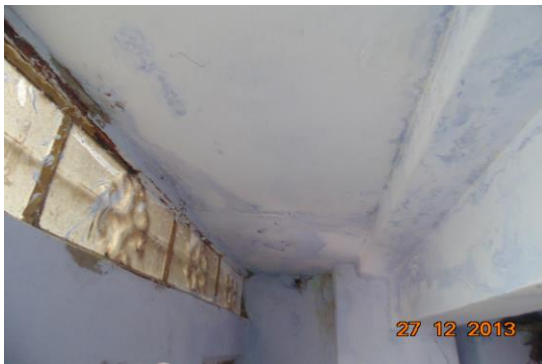
Photo 32 Peeling of Plaster on Roof of Room No. 1 of Second Floor
