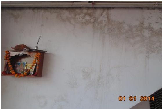
Photo 46 Dampness/Seepage on Wall No. 1 of Hall No. 1 of Fourth Floor
