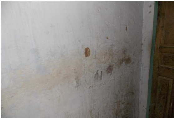
Photo 23 Peeling of Plaster on Wall No. 1 of Lobby of First Floor
