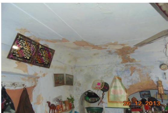
Photo 23 Peeling of Plaster on Roof of Kitchen of First Floor
