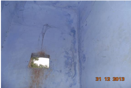
Photo 18 Dampness/Seepage on Roof of Room No. 1 of First Floor
