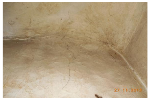
Photo 24 Inclined Crack on Wall No. 1 & Roof of Part C, Ground Floor Approx. Width = 1.5mm, Approx. Length = 1m. Distance from Wall No. 3 = 0.6m, Height from Floor = 1.5m.
