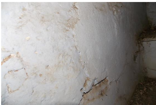
Photo 20 Damaged Portion on Wall No. 1 of Staircase GF to FF
