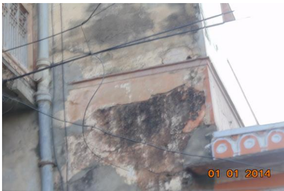
Photo 52 Peeling of Plaster on External Wall
