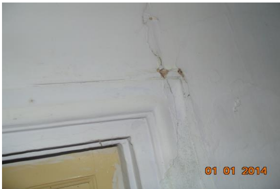
Photo 36 Plaster Crack on Wall No. 1 of First Floor
