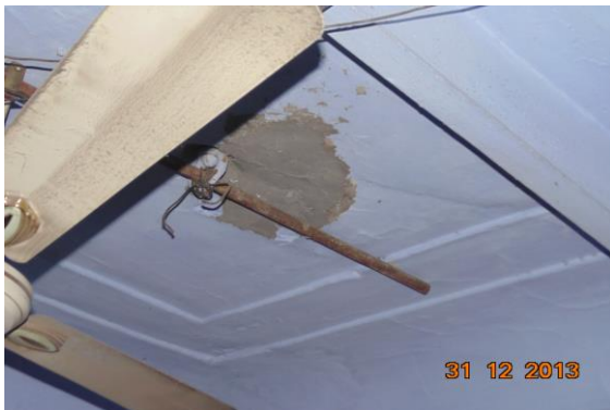
Photo 20 Peeling of Plaster on Roof of Room No. 1 of First Floor
