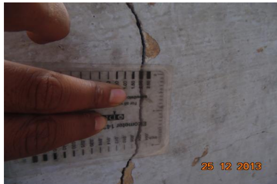
Photo 21A Vertical Crack on Wall No. 1 of Open Sky, First Floor, Approx. Width = 2mm, Approx. Length = 1m. Distance from Wall No.4 = 2.5m, Height from Floor = 0m.
