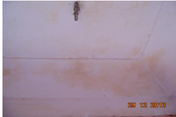
Photo 7 Dampness/Seepage on Roof of Varanda of House No. 339 of First Floor
