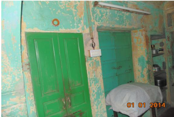
Photo 70 Dampness/Seepage on Wall No. 1 of Second Floor
