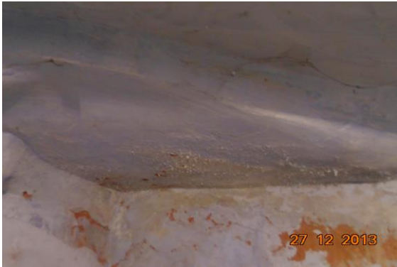
Photo 18 Dampness/Seepage on Roof of Room No. 2 of First Floor
