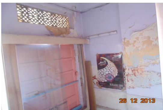
Photo 15 Peeling of Plaster on Wall No. 2 & 3 of Lobby of Second Floor
