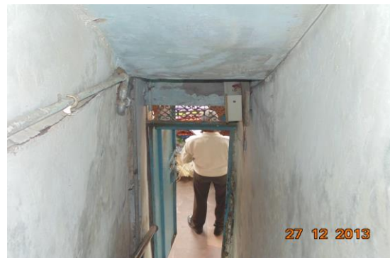
Photo 53 Dampness/Seepage on Wall No. 1, 2 & Roof of Staircase FF to GF
