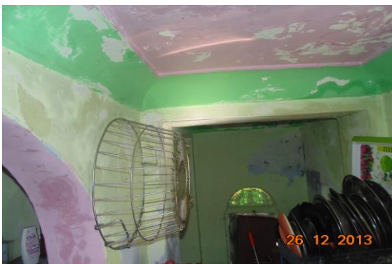
Photo 29 Dampness/Seepage on Wall No. 1, 3 & Roof of Kitchen of Second Floor
