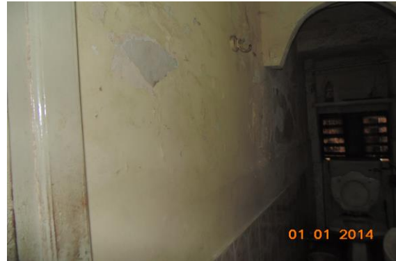
Photo 53 Dampness/Seepage on Wall No. 1 of First Floor
