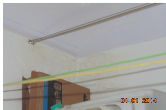
Photo 87 Dampness/Seepage on Wall No. 2 & 4 of Room No. 4 of Second Floor
