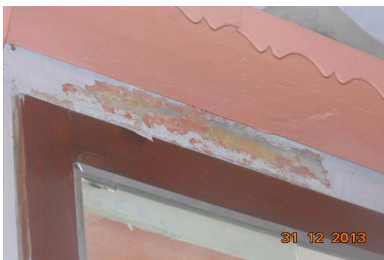
Photo 45 Peeling of Plaster on Wall No. 4 of First Floor
