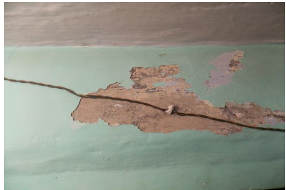
Photo 26 Peeling of Plaster on Wall No. 4 of Passage of First Floor
