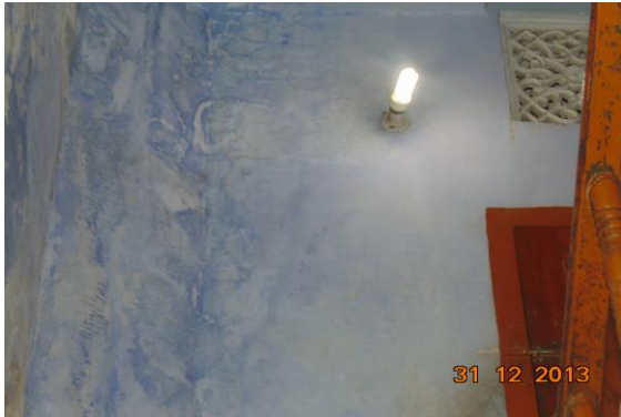
Photo 12 Dampness/Seepage on Wall No. 4 of Stair SF to TF
