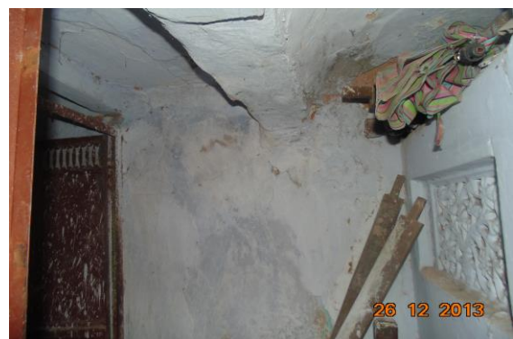
Photo 15 Dampness/Seepage on Wall No. 2 & Roof of Passage of First Floor
