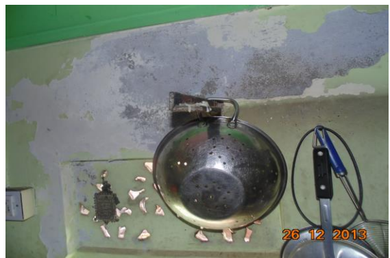
Photo 30 Dampness/Seepage on Wall No. 4 of Kitchen of Second Floor
