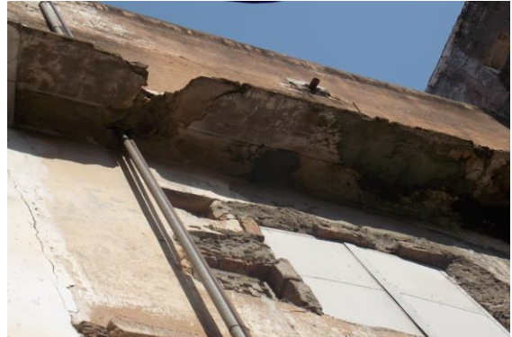
Photo 60 Damaged Portion on Chajja of External Façade
