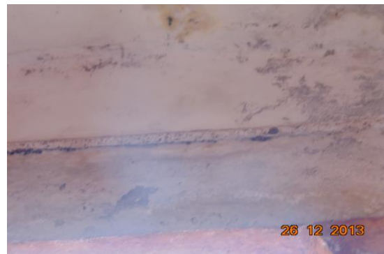
Photo 16 Dampness/Seepage on Beam of Varanda of Shop No.42, Ground Floor
