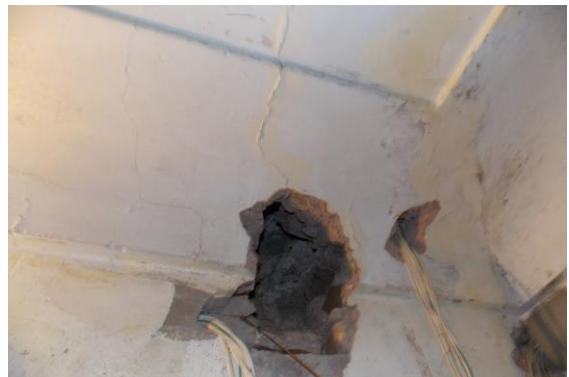
Photo 32 Peeling of Plaster on Roof of Lobby of First Floor
