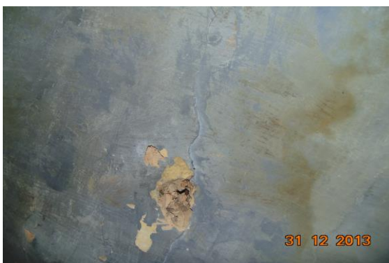
Photo 29 Peeling of Plaster on Roof of Room No. 2 of Third Floor
