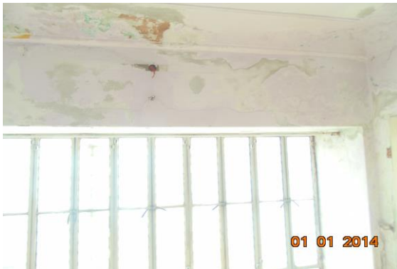
Photo 46 Dampness/Seepage on Roof, Wall No.1 & 4 of First Floor
