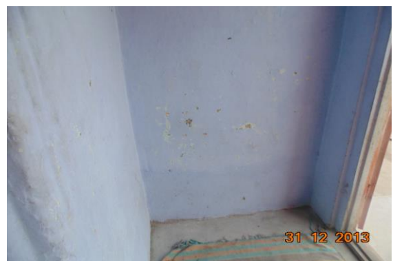
Photo 23 Peeling of Plaster on Wall No. 1 of Varandah of First Floor
