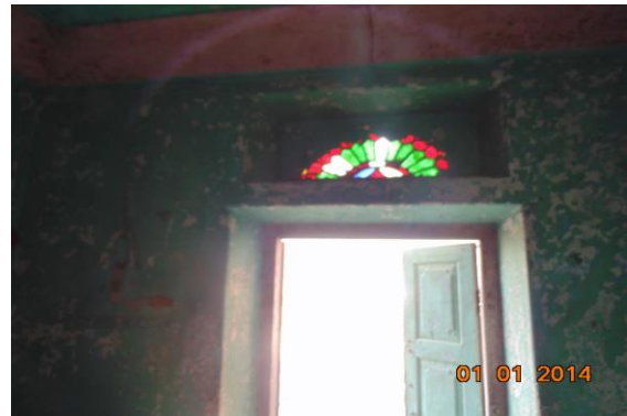
Photo 131 Dampness/Seepage on Wall No. 3 of Third Floor
