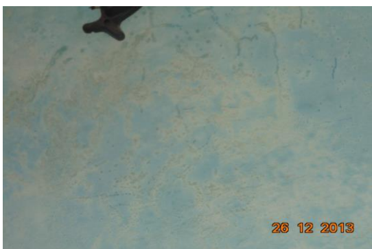
Photo 38 Dampness/Seepage on Wall No. 2 of Bathroom of Third Floor
