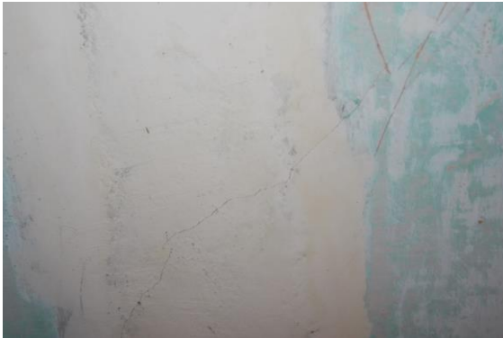
Photo 23 Plaster Crack on Wall No. 3 of Lobby of Second Floor
