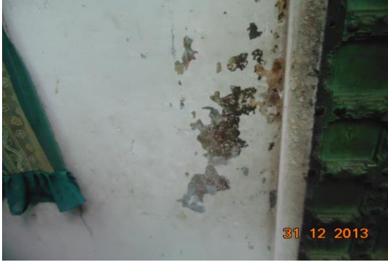
Photo 11 Peeling of Plaster on Wall No. 1 of Third Floor
