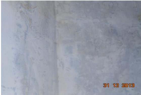
Photo 24 Dampness/Seepage on Wall No. 1 of Fourth Floor
