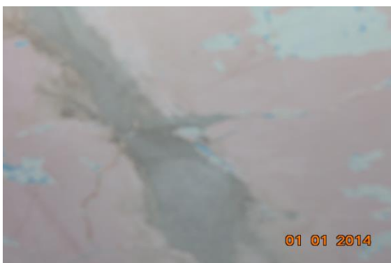
Photo 74 Peeling of Plaster on Roof of Hall No. 1 of Second Floor
