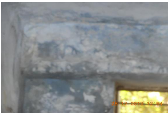
Photo 59 Horizontal Crack on Wall No. 4 of Toilet No. 2, Sarraf Katla, Ground Floor Approx. Width = 0.8mm, Approx. Length = 0.5m. Distance from Wall No. 1 = 0m, Height from Floor = 2.8m.
