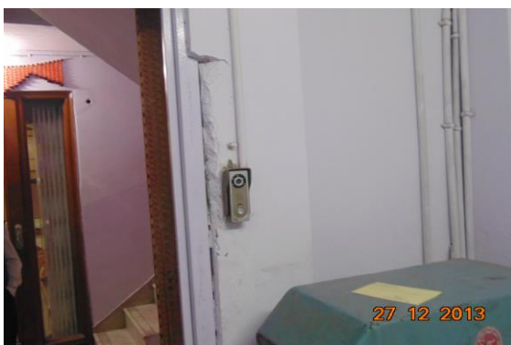
Photo 5 Peeling of Plaster on Wall No. 4 of Passage of Ground Floor
