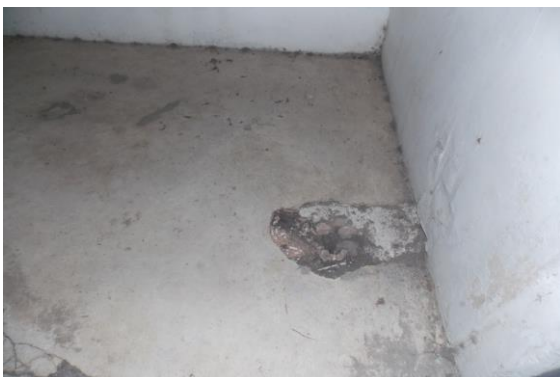
Photo 15 Peeling of Plaster on Floor of Varanda of Second Floor
