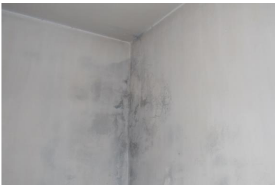
Photo 21 Dampness/Seepage on Wall No. 4 & 1 of Room No. 1 of Third Floor
