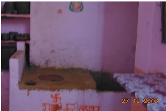
Photo 3 Dampness/Seepage on Wall No. 4 of Shop of Ground Floor
