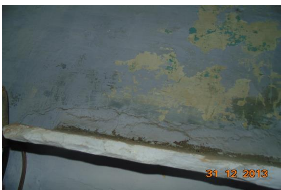
Photo 10 Peeling of Plaster on Wall No. 3 of Third Floor
