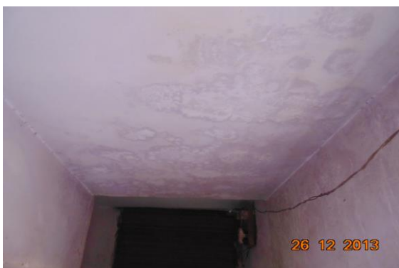
Photo 21 Dampness/Seepage on Roof of Passage of Second Floor
