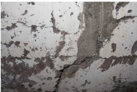
Photo 83 Damaged Portion on All Walls of H.No.287 of Terrace
