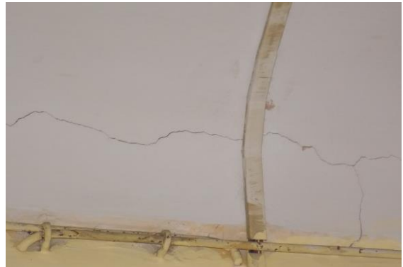
Photo 14 Horizontal Crack on Roof of Varanda No.2, First Floor Approx. Width = 0.6mm, Approx. Length = 1m. Distance from Wall No.3 = 4.8m, Height from Floor = 3.5m.
