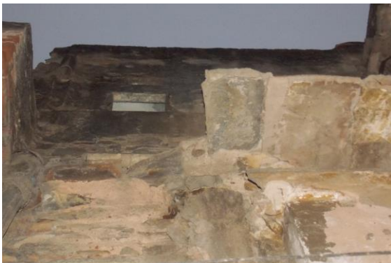
Photo 87 Peeling of Plaster on Outer wall of H.No.286 of Ground Floor
