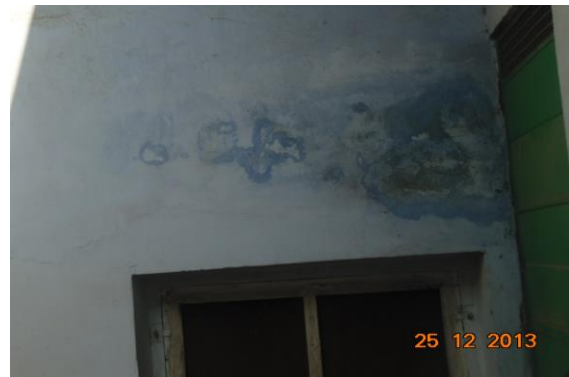
Photo 73 Dampness/Seepage on Wall No. 2 of Balcony No.2 of Second Floor
