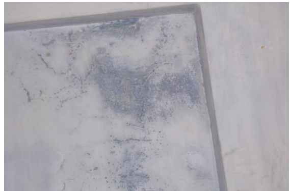
Photo 20 Dampness/Seepage on Wall No. 4 of Room No. 1 of Second Floor
