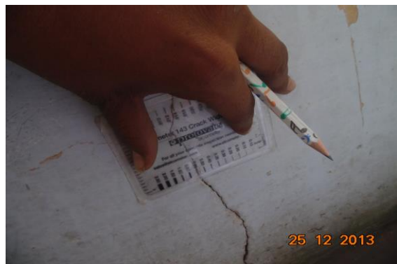
Photo 22A Inclined Crack on Parapet wall no.1 & Floor of Balcony No.4, First Floor Approx. Width = 0.6mm, Approx. Length = 0.8m. Distance from Wall No.3 = 1.5m, Height from Floor = 0m.
