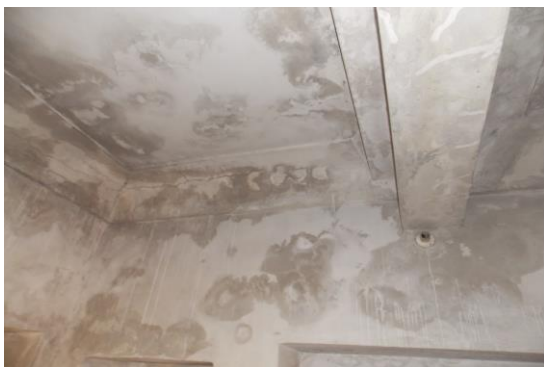
Photo 38 Dampness/Seepage on Wall No. 4 & Roof of Room No. 1 of Second Floor
