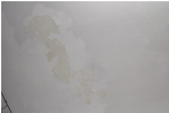
Photo 3 Peeling of Plaster on Roof of Varanda of Shop No.71 of Ground Floor
