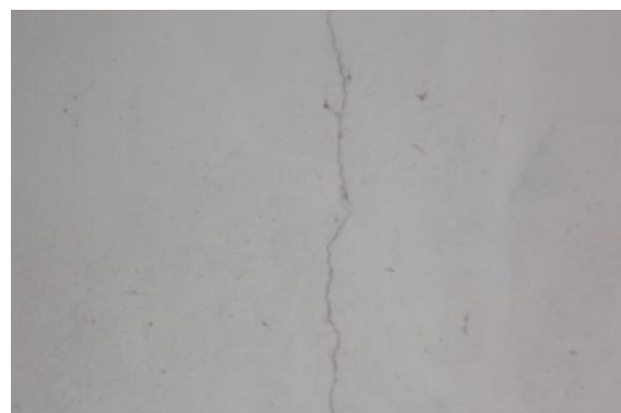
Photo 5 Vertical Crack on Wall No. 4 of Room No. 1, House No. 672, First Floor Approx. Width = 0.3mm, Approx. Length = 1m. Distance from Wall No. 1 = 0.3m, Height from Floor = 2m.
