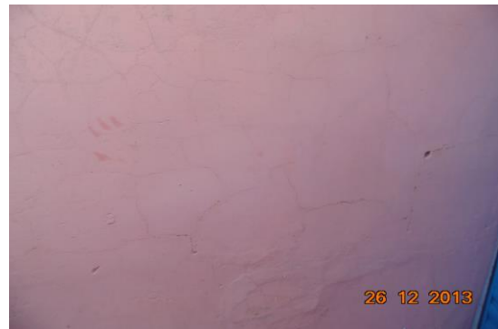
Photo 18 Peeling of Plaster on Wall No. 3 of Open Sky of External Façade
