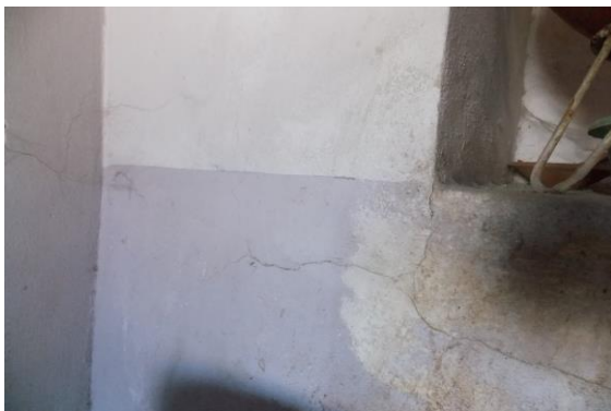
Photo 5 Inclined Crack on Wall No. 2 of Room No. 1, First Floor Approx. Width = 0.3mm, Approx. Length = 2m.
