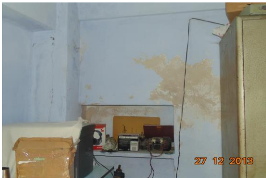
Photo 26 Dampness/Seepage on Wall No. 7 of Hall No. 1 of First Floor
