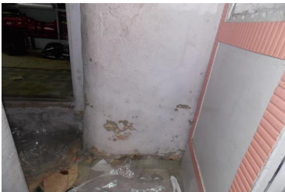
Photo 63 Peeling of Plaster on Wall No. 4 of Part A of Shop No.76 of Ground Floor
