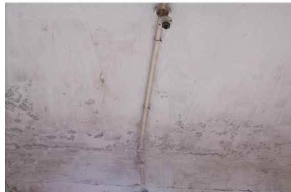
Photo 27 Dampness/Seepage on Roof of Varanda of Ground Floor
