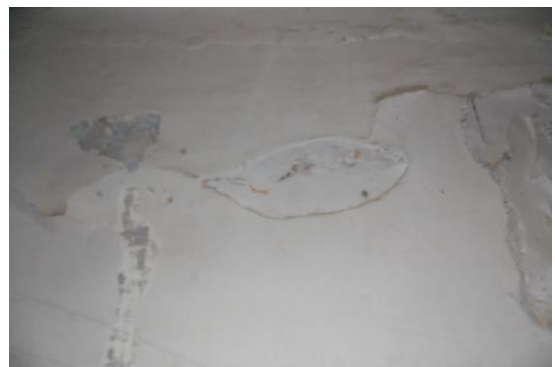
Photo 27 Peeling of Plaster on Wall No. 3 of Room No. 2 of First Floor
