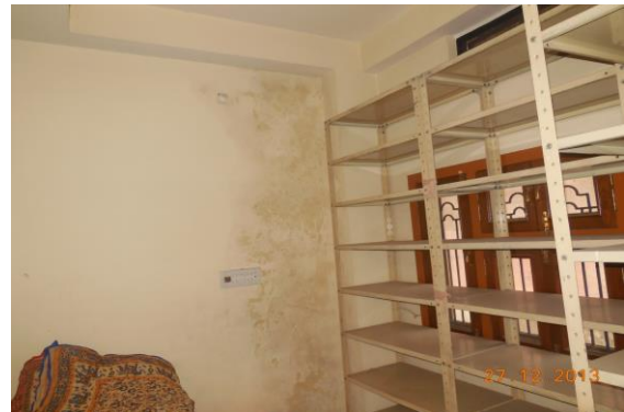
Photo 72 Dampness/Seepage on Wall No. 1 of Hall No. 1 of First Floor
