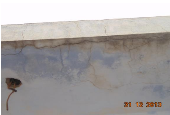
Photo 34 Dampness/Seepage on Wall No. 3 of Room No. 1 of Terrace
