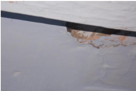
Photo 31 Damaged Portion on Roof of Room No. 2 of Second Floor
