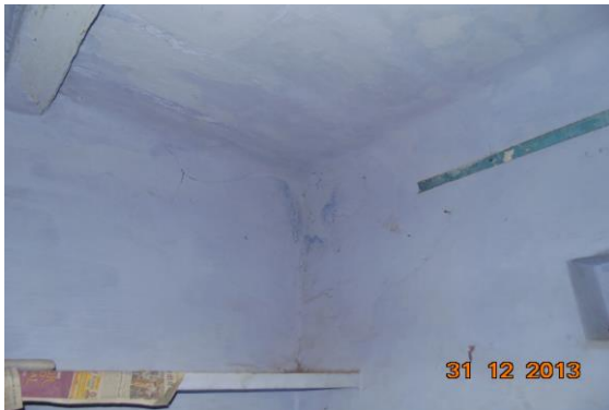
Photo 12 Dampness/Seepage on Roof of Varandah of Third Floor
