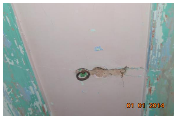
Photo 81 Peeling of Plaster on Roof of Second Floor
