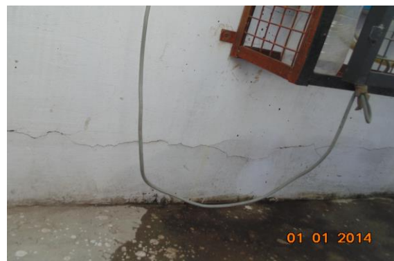
Photo 49 Plaster Crack on Wall No. 4 of Balcony 2 of Fourth Floor
