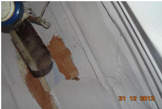
Photo 13 Dampness/Seepage on Roof of Varanda of Second Floor
