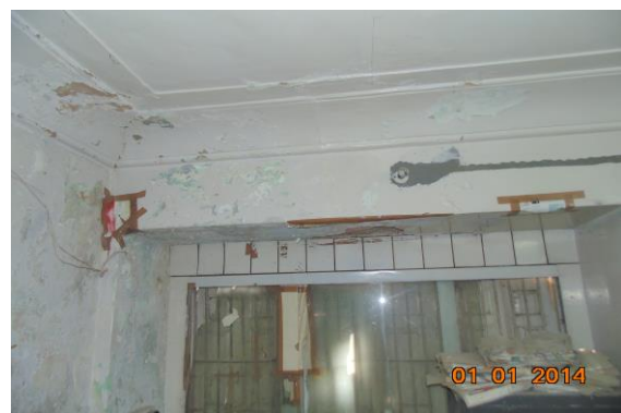
Photo 39 Dampness/Seepage on Roof & Wall No.4 of First Floor
