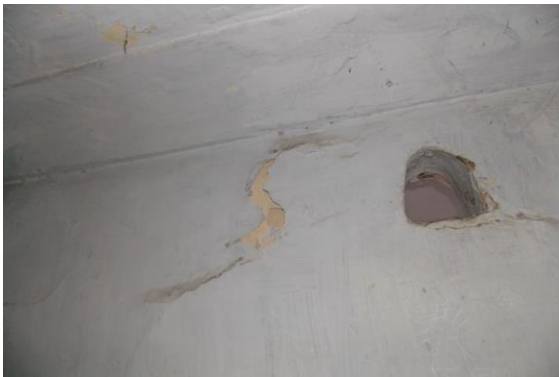
Photo 25 Peeling of Plaster on Wall No. 4 of Lobby of First Floor
