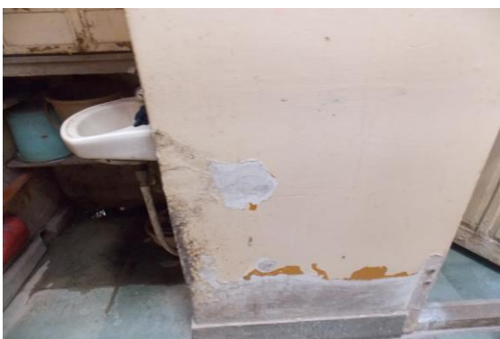
Photo 17 Peeling of Plaster on Wall No. 4 of Open Sky of Second Floor
