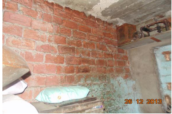
Photo 41 Peeling of Plaster on Wall No. 1 of Room No. 2 of Fourth Floor
