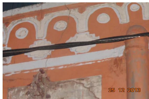
Photo 6 Inclined Crack on Beam of Varanda, Shop No. 56, Ground Floor, Approx. Width = 1mm, Approx. Length = 1m. Distance from Left External Col = 0m, Height from Floor = 3m.
