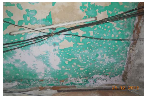
Photo 6 Dampness/Seepage on Roof of Shop No.32 of Ground Floor
