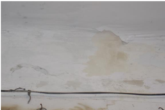
Photo 61 Peeling of Plaster on Roof of Varanda of Shop No.75 of Ground Floor
