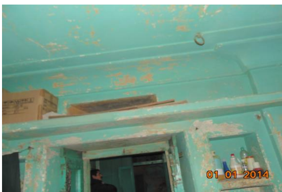
Photo 62 Dampness/Seepage on Wall No. 3 of Second Floor
