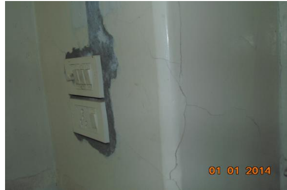
Photo 41 Plaster Crack on Wall No. 3 of First Floor
