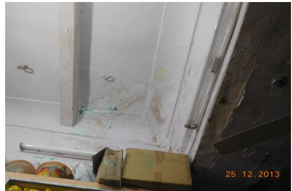
Photo 4 Dampness/Seepage on Roof of Shop No.32 of Ground Floor
