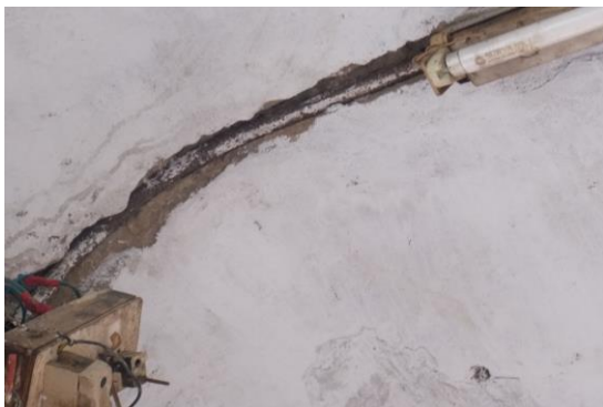
Photo 18 Damaged Portion on Roof of Varanda of Shop of Ground Floor
