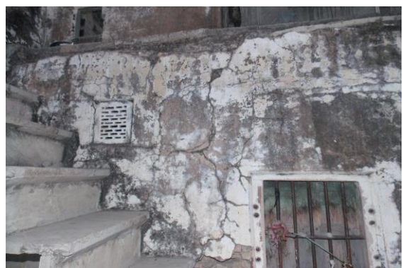
Photo 78 Damaged Portion on Outside Wall of Room No. 2 of Third Floor
