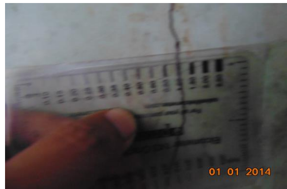
Photo 9A Inclined Crack on Wall No. 1 of House No. 458, First Floor Approx. Width = 1mm, Approx. Length = 1.2m. Distance from Wall No. 3 = 1.1m, Height from Floor = 1m.
