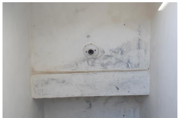
Photo 45 Dampness/Seepage on Wall No. 3 of Staircase First Floor to Second Floor of First Floor
