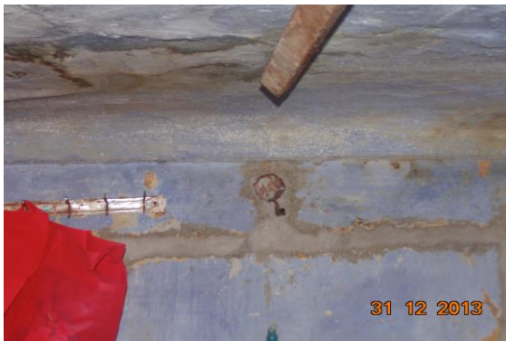
Photo 27 Dampness/Seepage on Wall No. 2 & Roof of Room No. 2 of Third Floor
