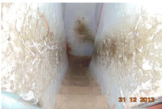
Photo 16 Peeling of Plaster on Wall No. 2 of Passage of Second Floor
