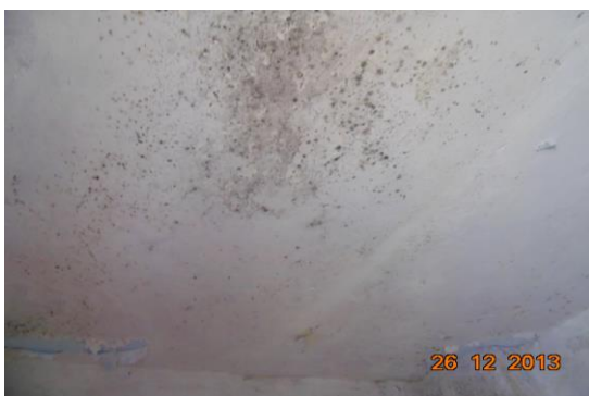
Photo 14 Dampness/Seepage on Roof of Kitchen of Third Floor
