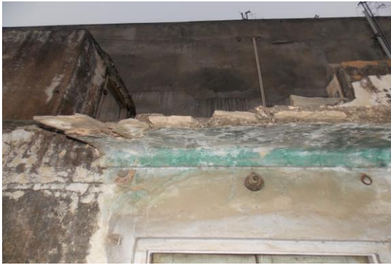
Photo 79 Damaged Portion on SunShade of Room No. 2 of Third Floor
