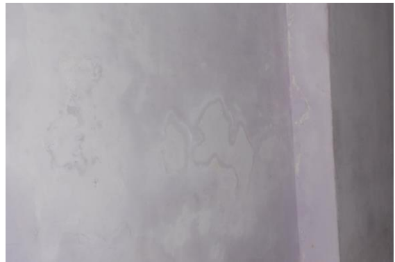
Photo 4 Dampness/Seepage on Wall No. 1 of Shop No.29 of Ground Floor
