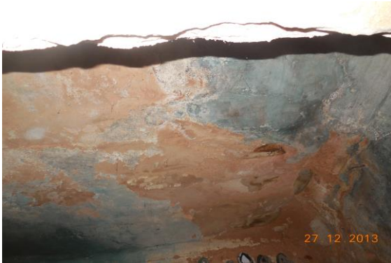
Photo 53 Damaged Portion on Roof of Kohtari of Ground Floor
