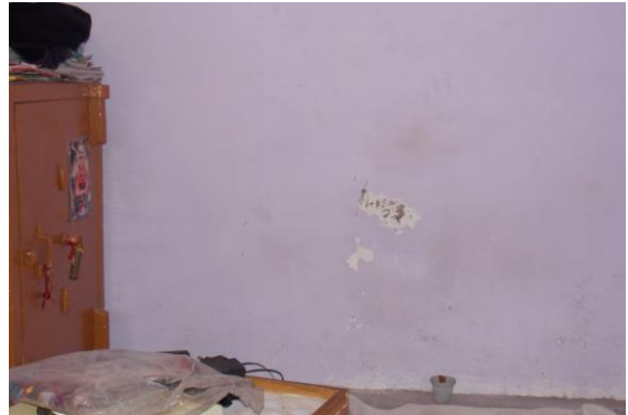
Photo 86 Peeling of Plaster on Wall No. 4 of Shop No.2 of Ground Floor
