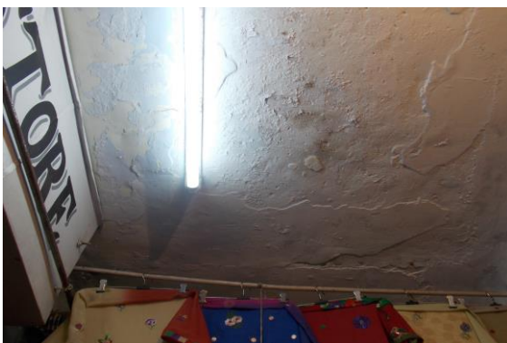
Photo 27 Peeling of Plaster on Roof of Varanda of Shop No.77 of Ground Floor
