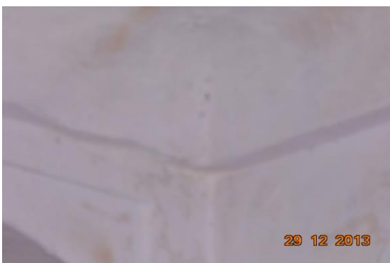
Photo 10 Dampness/Seepage on Roof of Room No. 1 of House No. 339, First Floor
