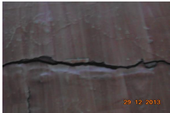
Photo 9 Damaged Portion on Wall No. Floor of Room No. 1 of House No. 339, First Floor
