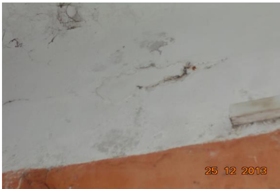
Photo 27 Peeling of Plaster on Beam of Varanda of Shop No. 55, Ground Floor
