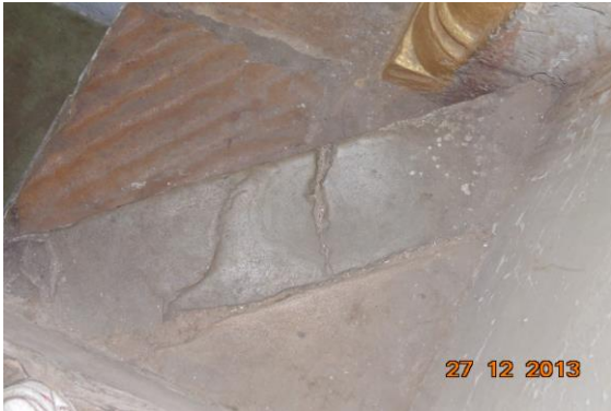
Photo 32 Damaged Portion on Steps of Staircase FF to SF of First Floor
