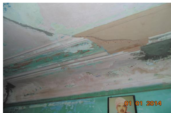
Photo 75 Peeling of Plaster on Roof of Hall No. 1 of Second Floor
