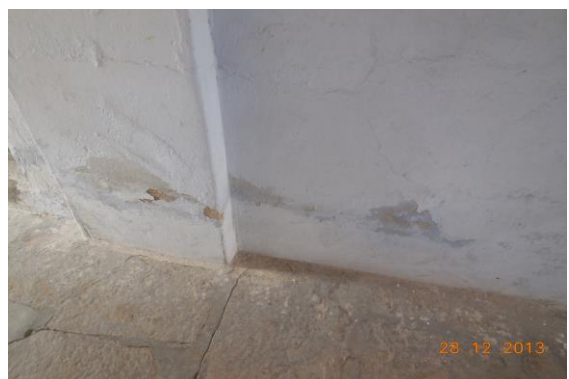
Photo 100 Dampness/Seepage on Wall No. 2 of Passage 2 of Navjeevan Chikitsalaya of Ground Floor
