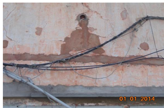
Photo 141 Peeling of Plaster on Outer Wall of FF External Façade
