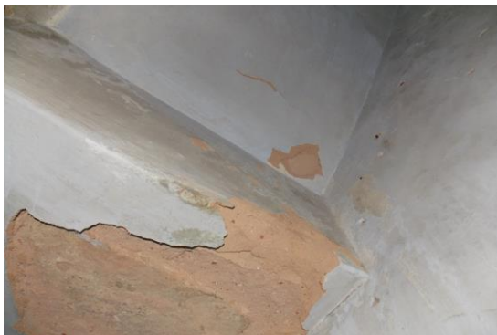
Photo 36 Peeling of Plaster on Roof of Staircase FF to SF
