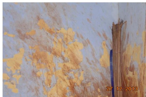
Photo 6 Dampness/Seepage on Wall No. 2 & 4 of Staircase GF to FF of Ground Floor
