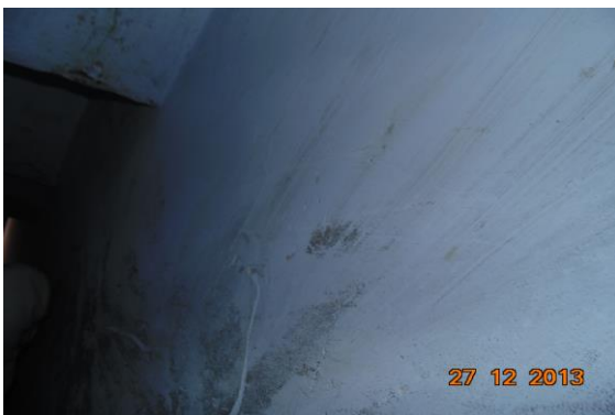
Photo 34 Peeling of Plaster on Wall No. 1 of Staircase GF to FF of First Floor
