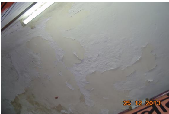
Photo 44 Dampness/Seepage on Roof of Varanda of Shop No. 49, Ground Floor
