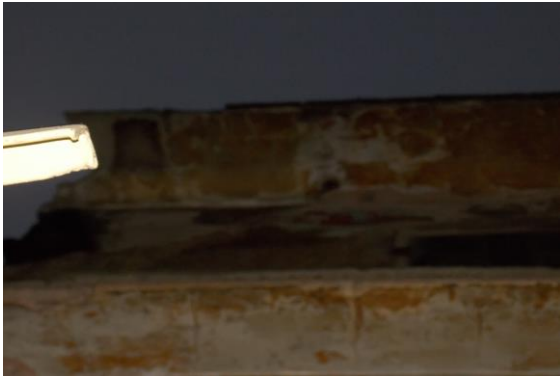
Photo 91 Peeling of Plaster on SunShade of Building of Second Floor
