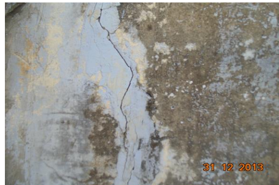
Photo 4 Inclined Crack on Wall No. 5 of Open Area 1, Terrace, Approx. Width = 4mm, Approx. Length = 3m. Distance from Wall No. 2 = 1.1m, Height from Floor = 0m.
