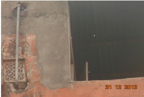
Photo 37 Peeling of Plaster on Outer Wall of Third Floor
