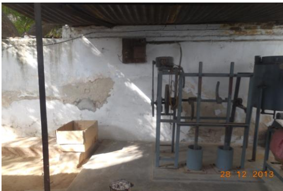
Photo 97 Peeling of Plaster on Wall No. 4 of Open Area 1 of Navjeevan Chikitsalaya of Ground Floor
