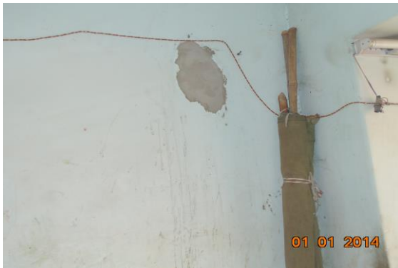
Photo 28 Peeling of Plaster on Wall No. 3 of First Floor
