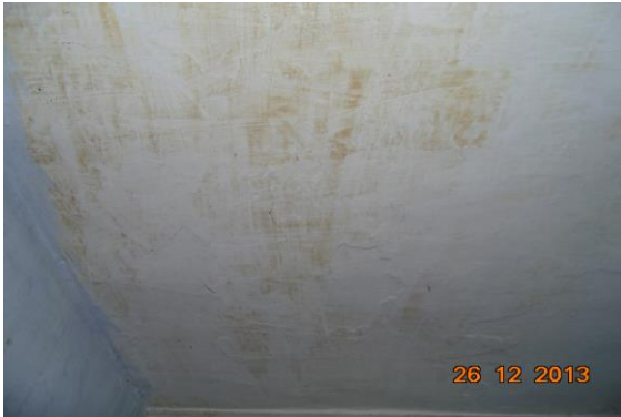
Photo 13 Dampness/Seepage on Roof of Room No. 1 of Third Floor
