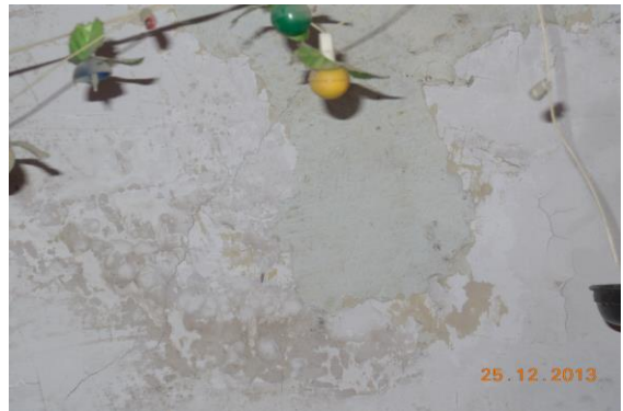
Photo 3 Inclined Crack on Wall No. 4 of Room No. 2, First Floor Approx. Width = 1mm, Approx. Length = 2m. Distance from Wall No.2 = 0.3m, Height from Floor = 0m.
