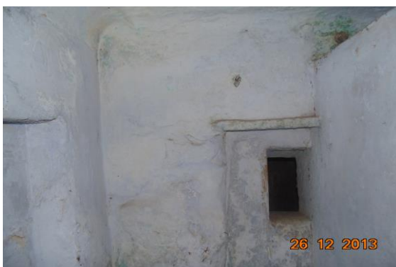
Photo 14 Dampness/Seepage on Wall No. 1, 2 & 4 of Toilet No. 1 of First Floor
