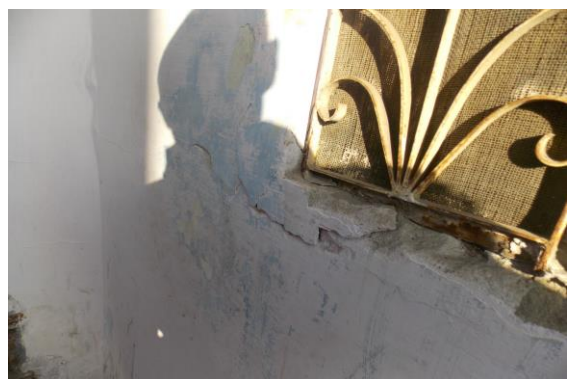
Photo 18 Peeling of Plaster on Wall No. 3 of Balcony of Second Floor
