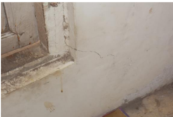
Photo 27 Plaster Crack on Wall No. 4 of Varanda of First Floor
