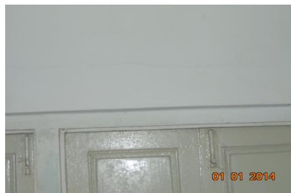
Photo 33 Plaster Crack on Wall No. 1 of Hall No. 2 of First Floor
