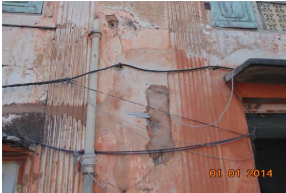
Photo 142 Peeling of Plaster on Outer Wall of FF External Façade
