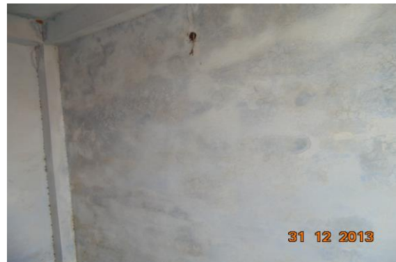
Photo 33 Dampness/Seepage on Wall No. 2 of Room No. 1 of Terrace
