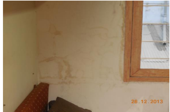
Photo 153 Dampness/Seepage on Wall No. 4 of Shop No. F 13 of First Floor
