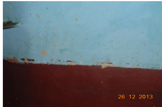
Photo 35 Peeling of Plaster on Wall No. 4 of Lobby of Third Floor
