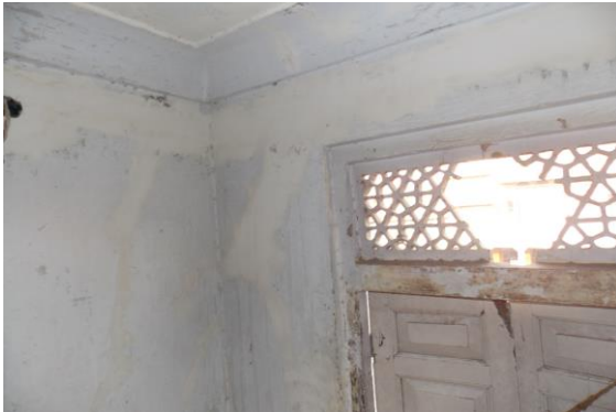
Photo 25 Dampness/Seepage on Wall No. 1 & 4 of Varanda of First Floor
