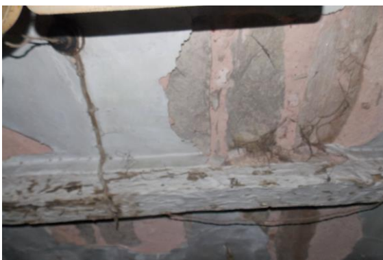
Photo 33 Peeling of Plaster on Roof of Room No. 4 of Second Floor
