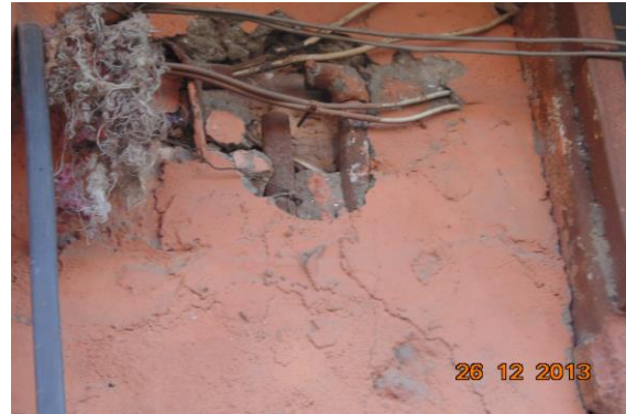
Photo 18 Damaged Portion on Wall No. 3 of Gallery of First Floor
