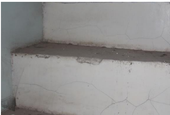
Photo 5 Inclined Crack on Steps of Staircase TF to Terrace Approx. Width = 0.2mm, Approx. Length = 3m.
