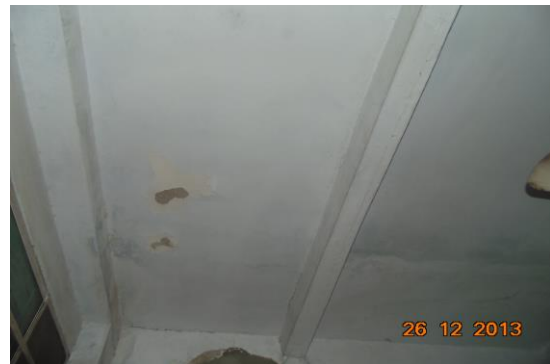
Photo 35 Peeling of Plaster on Roof of Room No. 1 of Third Floor
