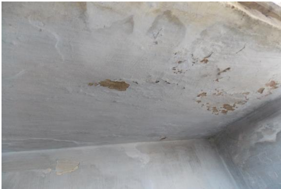
Photo 53 Peeling of Plaster on Staircase TF to Terrace
