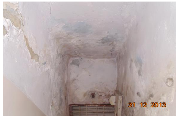
Photo 34 Dampness/Seepage on Wall No. 1, 2 & Roof of Stair GF to FF of Third Floor
