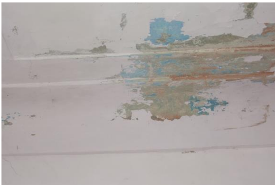
Photo 139 Peeling of Plaster on Roof of First Floor
