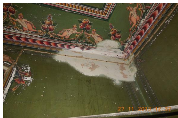
Photo 152 Dampness/Seepage on Wall No. 2 of Room No. 2 of Ground Floor
