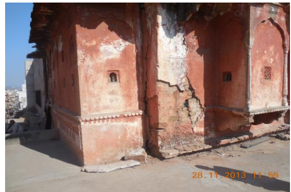
Photo 187 Peeling of Plaster on Side B of External Façade
