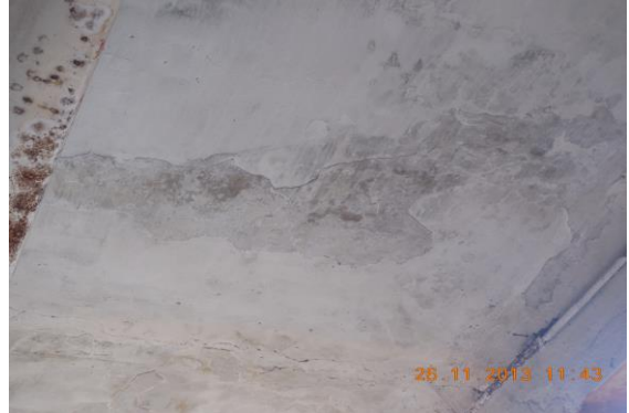
Photo 48 Dampness/Seepage on Roof of Varanda of Shop No.350 of Ground Floor
