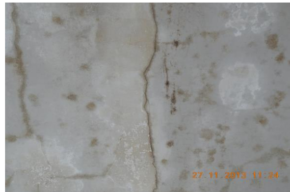
Photo 96 Plaster Crack on Wall No. 1, 4 & Roof of Varanda of First Floor
