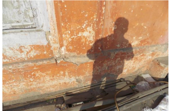
Photo 49 Peeling of Plaster on Frontside Wall of First Floor
