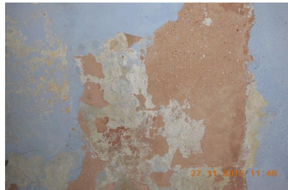
Photo 120 Peeling of Plaster on Roof of Room No. 3 of First Floor
