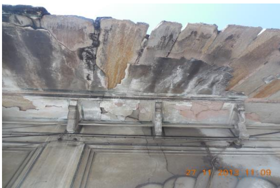
Photo 79 Damaged Portion on Roof of Varandah Temple Gate 4 of First Floor
