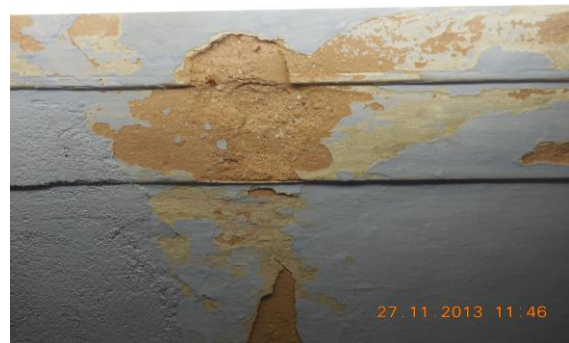
Photo 116 Peeling of Plaster on Roof of Room No. 2 of First Floor
