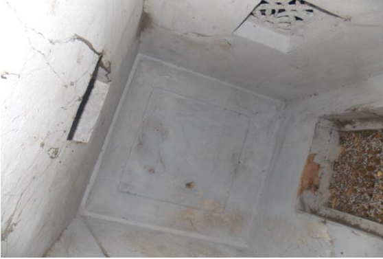
Photo 41 Dampness/Seepage on Roof of Bathroom of Ground Floor
