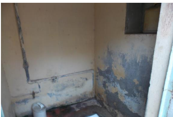
Photo 111 Dampness/Seepage on Wall No. 2 & 4 of Toilet No. 1 of Ground Floor
