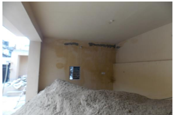
Photo 110 Dampness/Seepage on Wall No. 1 of Lobby of Ground Floor
