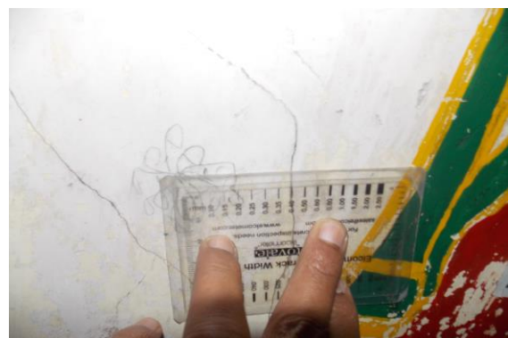
Photo 5A Inclined Crack on Wall No. 5 of Varanda 2, Part A, House No. 2414, First Floor Approx. Width = 0.4mm, Approx. Length = 1.2m. Distance from Wall No.1 = 1.3m, Height from Floor = 0m.
