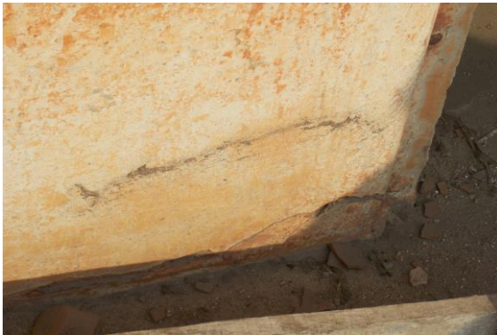
Photo 24 Peeling of Plaster on Wall No. 3 of First Floor
