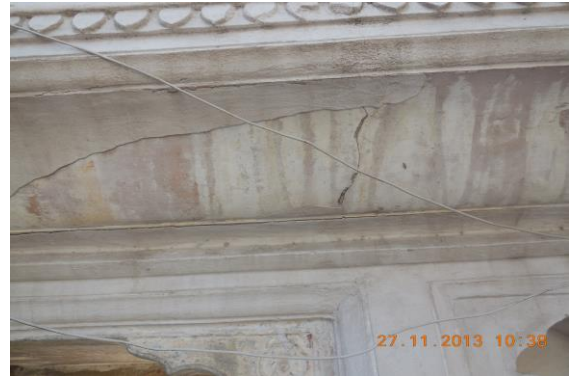
Photo 64 Peeling of Plaster on Wall No. 3 of Entrance Open Area of First Floor
