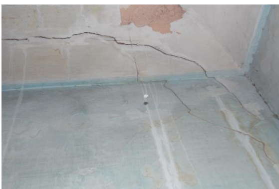
Photo 5 Inclined Crack on Wall No. Roof & 1 of Toilet No. 3, House No. 2198, First Floor Approx. Width = 2.5mm, Approx. Length = 3m. Distance from Wall No. 4 = 0.05m, Height from Floor = 2.4m.
