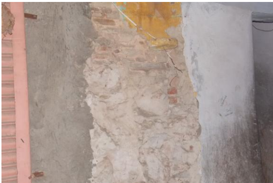
Photo 18 Peeling of Plaster on Left Side Wall of of Ground Floor
