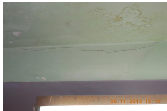
Photo 4 Horizontal Crack on Wall No. 3 of Part B of Shop no.349, Ground Floor Approx. Width = 0.6mm, Approx. Length = 2.3m. Distance from Wall no.2 = 0m, Height from Floor = 3m.
