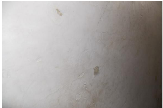
Photo 25 Peeling of Plaster on Wall No. 1 of Stair FF to SF
