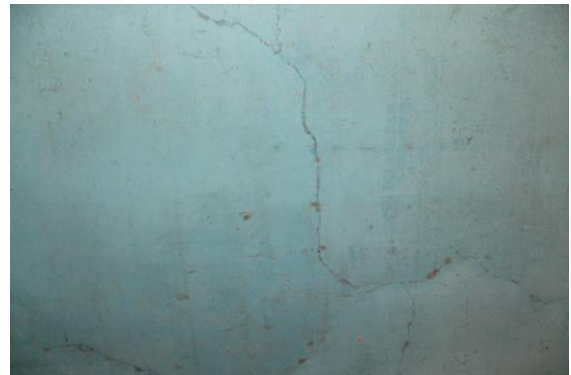
Photo 4 Inclined Crack on Wall No. 4 of Part B of Shop No.297, Ground Floor Approx. Width = 0.5mm, Approx. Length = 1.8m. Distance from Wall No.2 = 1.1m, Height from Floor = 0m.
