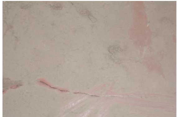
Photo 37 Plaster Crack on Floor of Third Floor
