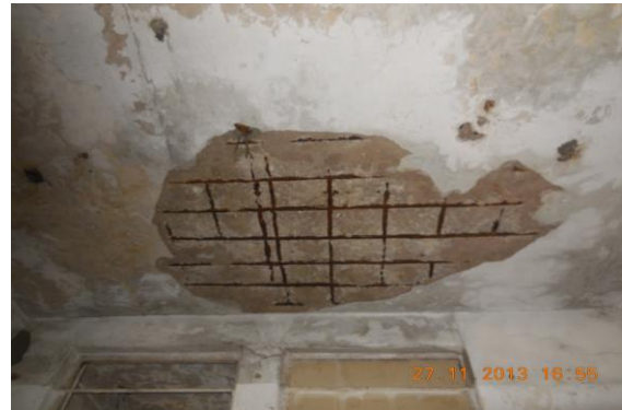
Photo 85 Exposed Reinforcement on Roof of Passage 1 of Munshi Shopping Complex, Second Floor
