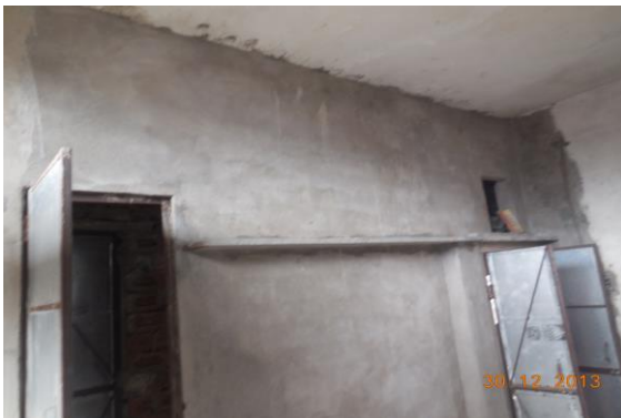
Photo 35 Peeling of Plaster on of Room No. 1 of House No. 2465, Third Floor
