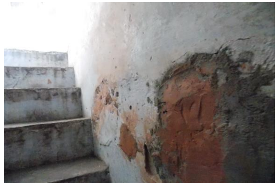
Photo 27 Peeling of Plaster on Wall No. 2 of Staircase Second Floor To Third Floor
