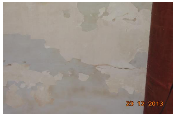
Photo 4 Horizontal Crack on Roof of Varanda of Shop No.299, Ground Floor Approx. Width = 0.8mm, Approx. Length = 2m. Distance from Leftside External Column = 0.6m, Height from Floor = 3m
