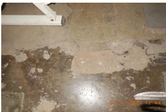
Photo 175 Damaged Portion on Floor of Hall No. 1 of Ground Floor
