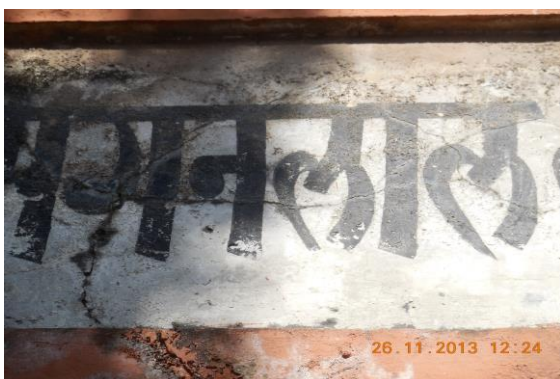
Photo 5 Inclined Crack on Outer Wall & Leftside External Wall of Varanda of Shop no.349, Ground Floor Approx. Width = 0.35mm, Approx. Length = 1.3m. Distance from Leftside External Column = 0m, Height from Floor = 2.8m
