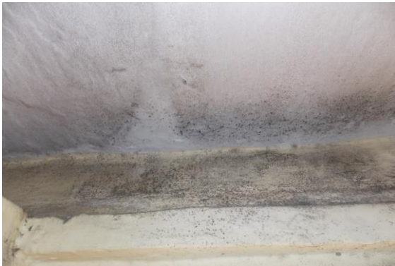
Photo 36 Dampness/Seepage on Wall No. 3 of Third Floor
