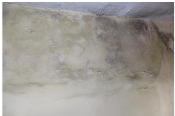
Photo 35 Dampness/Seepage on Wall No. 4 of Room No. 1 of Third Floor
