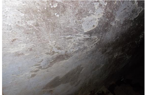
Photo 17 Peeling of Plaster on Wall No. 1 of Stair GF to FF
