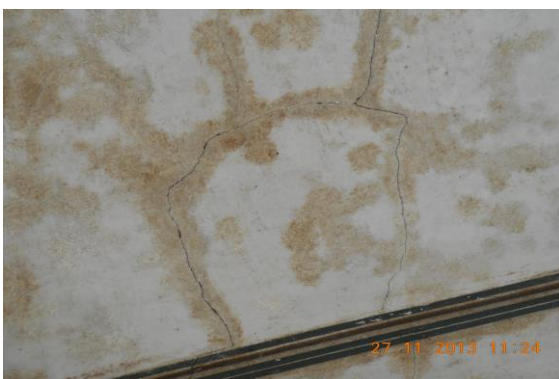
Photo 97 Plaster Crack on Wall No. 1, 4 & Roof of Varanda of First Floor
