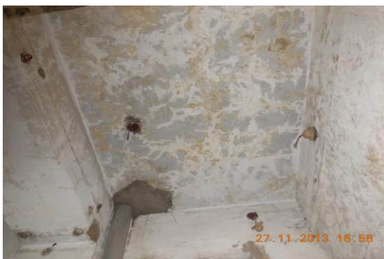
Photo 88 Dampness/Seepage on Roof of Bathroom of Munshi Shopping Complex, Second Floor
