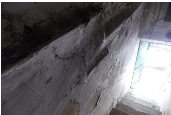
Photo 16 Peeling of Plaster on Wall No. 2 of Stair GF to FF
