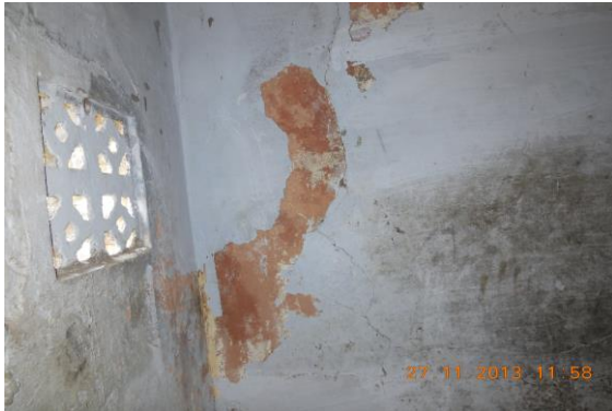
Photo 135 Peeling of Plaster on Wall No. 4 of Stair 3 of Second Floor
