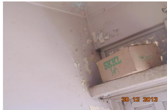
Photo 3 Dampness/Seepage on Wall No. 2 & Roof of Room No. 1 of House No. 2469, First Floor
