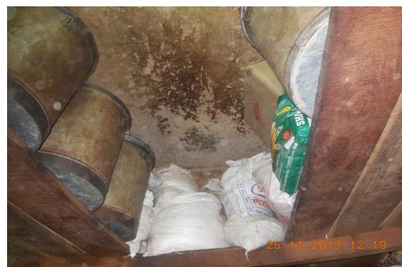
Photo 90 Peeling of Plaster on Roof of Room No. 1 of Ground Floor
