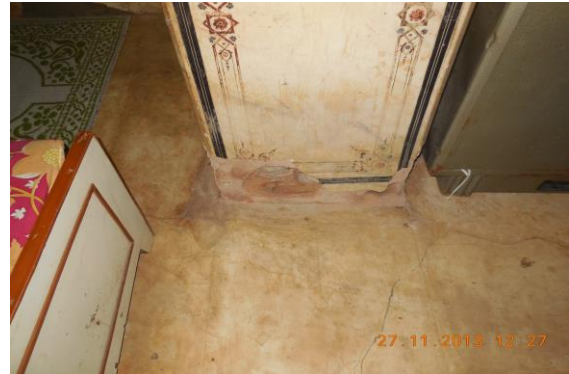
Photo 150 Peeling of Plaster on Wall No. 1 of Room No. 2 of Ground Floor
