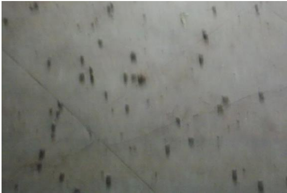
Photo 97 Plaster Crack on Floor of Toilet No. 9 of House No. 2198, First Floor
