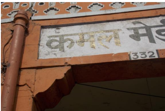
Photo 117 Peeling of Plaster on Outer Wall of Shop No. 332 of Ground Floor
