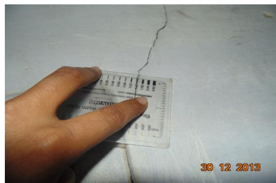
Photo 5A Inclined Crack on Wall No. 2 of Room No. 1, House No. 44 E/20, Second Floor Approx. Width = 1mm, Approx. Length = 1m. Distance from Wall 4 = 1m, Height from Floor = 1.65m.
