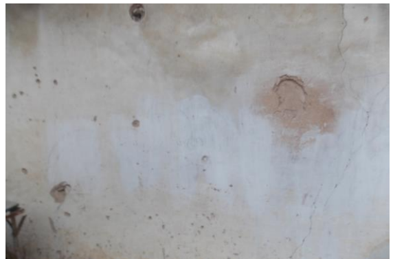
Photo 99 Peeling of Plaster on Wall No. 2 & 3 of Toilet No. 10 of House No. 2198, First Floor
