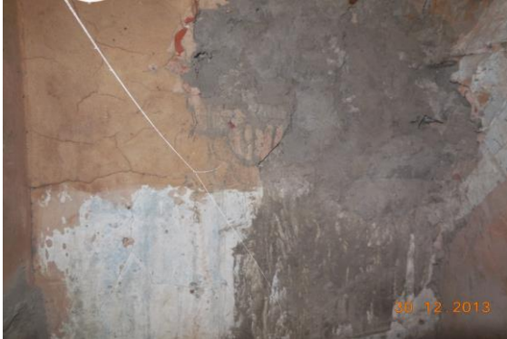
Photo 33 Peeling of Plaster on Wall No. 3 of Staircase Second Floor to Third Floor of House No. 2465, Second Floor
