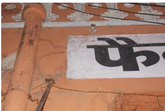
Photo 17 Inclined Crack on L/s External Column of Varanda of shop No.313, G/F Approx. Width = 0.5mm, Approx. Length = 1.5m. Distance from = Front of L/s External column, Height from Floor = 3m.
