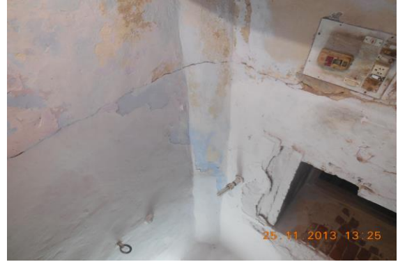
Photo 8 Horizontal Crack on Roof of Room No. 1, Shop Kailash Chand Sharma, Ground Floor Approx. Width = 10mm, Approx. Length = 2.3m. Distance from Wall No.2 = 0m, Height from Floor = 1.5m.
