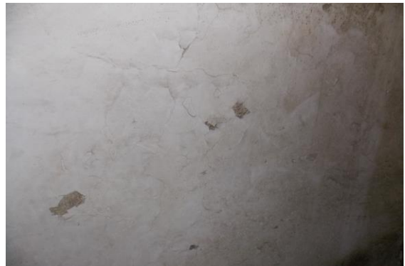
Photo 33 Peeling of Plaster on Wall No. 1 of Stair SF to TF
