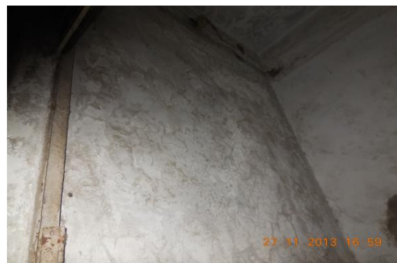
Photo 89 Dampness/Seepage on Wall No. 1 of Toilet No. 1 of Munshi Shopping Complex, Second Floor
