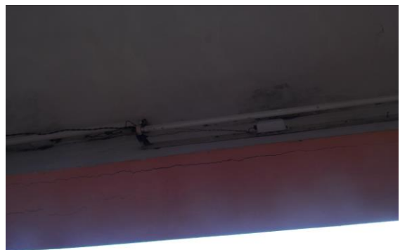
Photo 40 Horizontal Crack on Beam of Varanda of shop no.324, Ground Floor Approx. Width = 0.5mm, Approx. Length = 1.3m. Distance Backside of Leftside external column = 0m, Height Floor = 3.3m.
