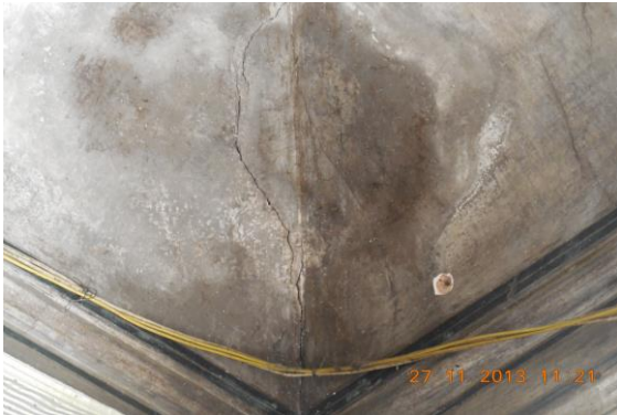
Photo 93 Plaster Crack on Wall No. 1, 4 & Roof of Varanda of First Floor
