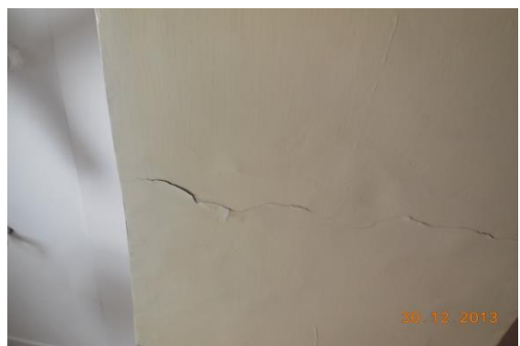
Photo 6 Peeling of Plaster on Wall No. 3 of Varanda No. 2 of House No. 2463, First Floor
