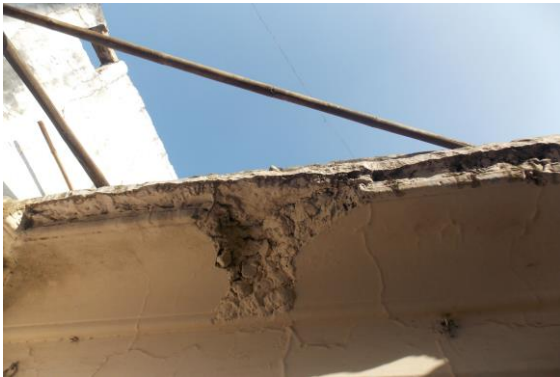
Photo 24 Peeling of Plaster on Wall No. 4 of Open Sky of Second Floor
