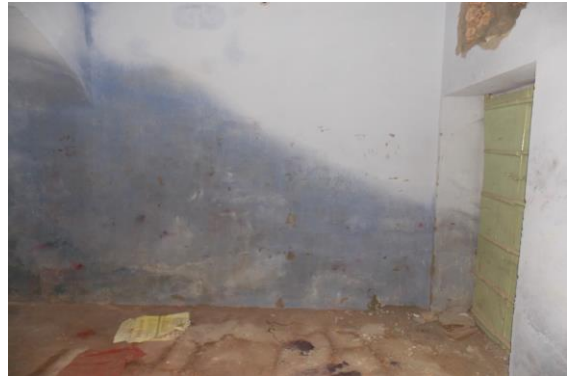
Photo 56 Dampness/Seepage on Wall No. 2 of Room No. 1 of Ground Floor
