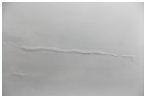
Photo 24 Peeling of Plaster on Roof of Shop No. 10, Upper Ground Floor
