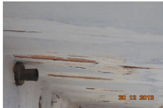
Photo 15 Peeling of Plaster on Wall No. 3 & Sunshade of Open Sky of House No. 2469, Terrace
