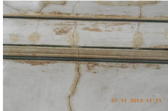
Photo 94 Plaster Crack on Wall No. 1, 4 & Roof of Varanda of First Floor
