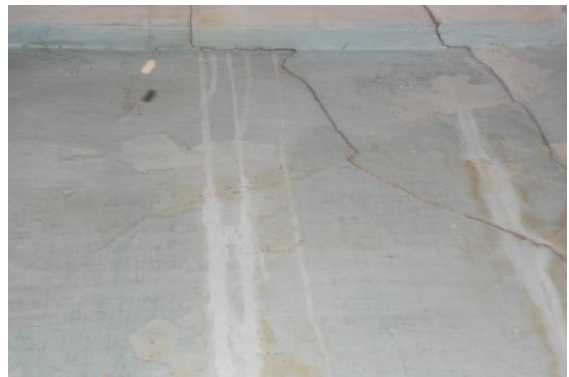
Photo 4 Inclined Crack on Wall No. 1 of Toilet No. 3, House No. 2198, First Floor Approx. Width = 1.5mm, Approx. Length = 0.8m. Distance from Wall No. 4 = 0.03m, Height from Floor = 2.3m.
