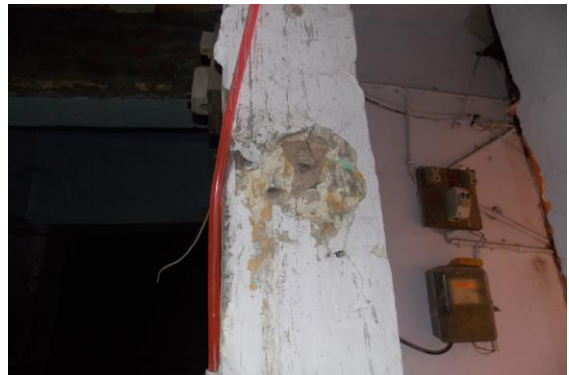
Photo 19 Peeling of Plaster on Fornt Wall of of Ground Floor
