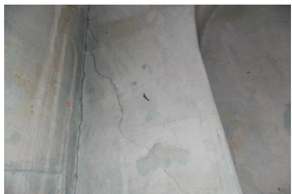
Photo 6 Inclined Crack on Wall No. 4 of Toilet No. 3, House No. 2198, First Floor Approx. Width = 1mm, Approx. Length = 1.2m. Distance from Wall No. 1 = 0.25m, Height from Floor = 1.6m.
