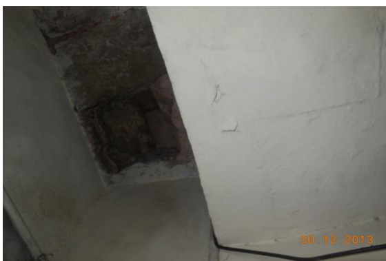
Photo 5 Peeling of Plaster on Roof of Toilet No. 1 of House No. 2463, First Floor
