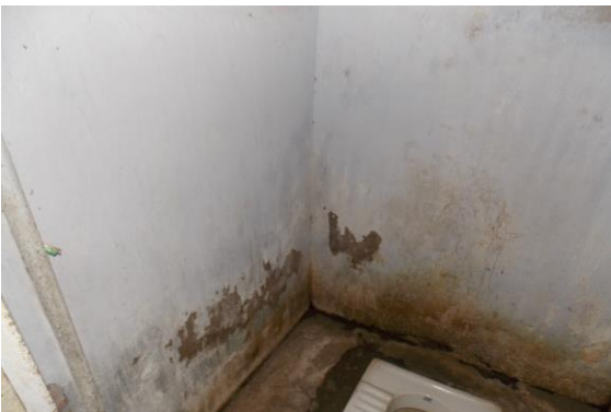
Photo 45 Dampness/Seepage on Wall No. 1 & 4 of Toilet No. 1 of Ground Floor
