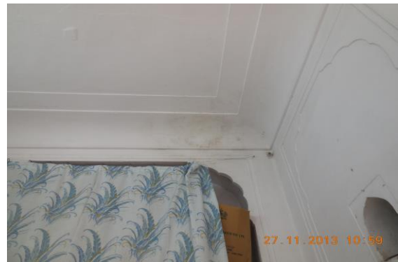
Photo 72 Dampness/Seepage on Roof Office 1 of First Floor
