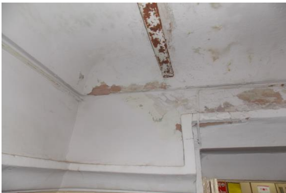
Photo 127 Peeling of Plaster on Wall No. 4 of Lobby 2 of First Floor
