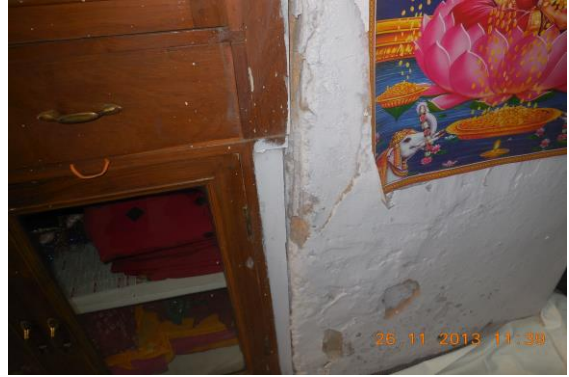
Photo 46 Peeling of Plaster on Entry Gate of Part C of Leftside Wall Part C of Shop No.350 of Ground Floor
