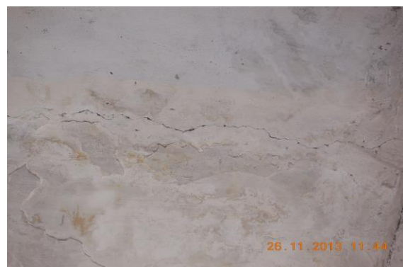
Photo 12 Inclined Crack on Roof of Varanda of Shop No.350, Ground Floor Approx. Width = 0.8mm, Approx. Length = 2m.Distance from Rightside External Column = 0m, Height from Floor = 3.5m.
