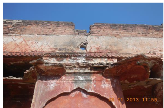
Photo 189 Peeling of Plaster on Side B of External Façade
