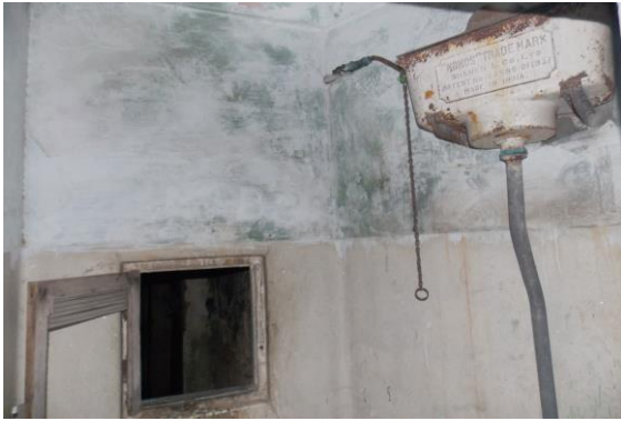
Photo 113 Dampness/Seepage on All Walls of Toilet No. 2 of Fourth Floor
