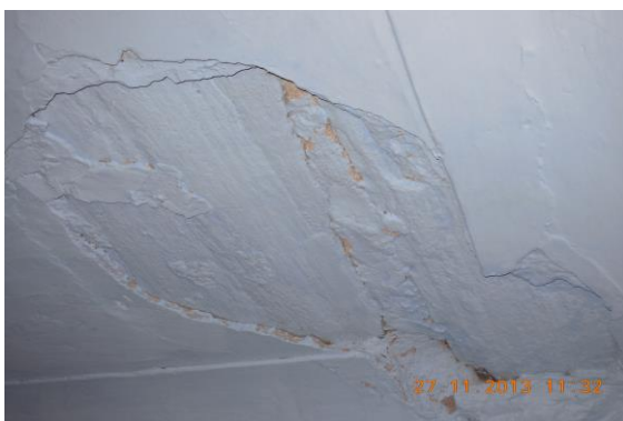
Photo 103 Peeling of Plaster on Roof of Stair 2 of First Floor
