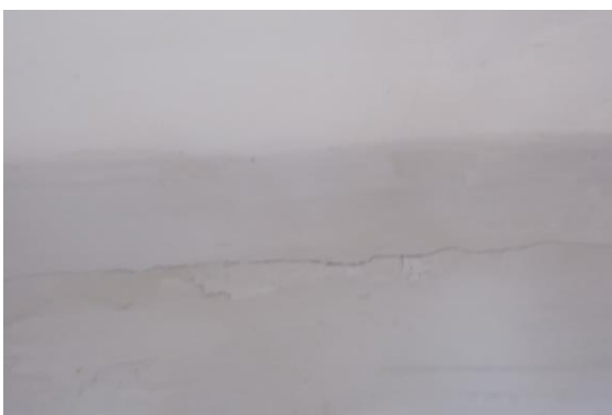
Photo 11 Inclined Crack on External Beam Right side of Varanda of Shop No.329, Ground Floor Approx. Width = 0.35mm, Approx. Length = 2.5m. Distance from L.S. Ext Col = 0.6m, Height from Floor = 3.3m.
