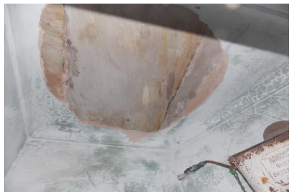
Photo 112 Peeling of Plaster on Roof of Toilet No. 2 of Fourth Floor
