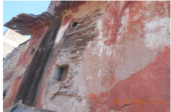
Photo 185 Peeling of Plaster on Front Side of External Façade
