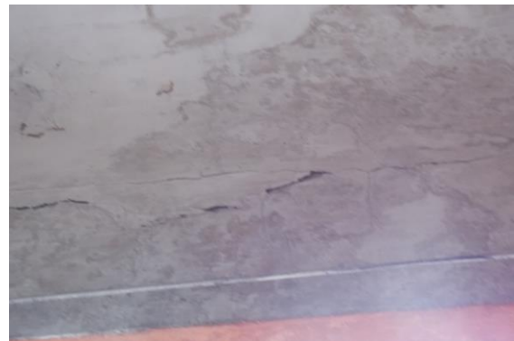
Photo 4 Horizontal Crack on Roof of Varanda of Shop No.331, Ground Floor Approx. Width = 0.25mm, Approx. Length = 2.5m. Distance from = Right side external column, Height from Floor = 3.3m.
