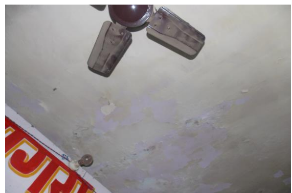
Photo 16 Horizontal Crack on Roof of Varanda of shop No.313, Ground Floor Approx. Width = 0.35mm, Approx. Length = 2m. Distance from Leftside External Column = 0.4m, Height from Floor = 3.5m.
