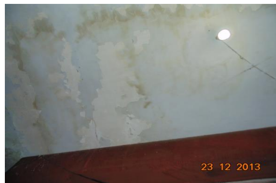
Photo 4 Horizontal Crack on Roof of Varanda of Shop No.299, Ground Floor Approx. Width = 0.8mm, Approx. Length = 2m. Distance from Leftside External Column = 0.6m, Height from Floor = 3m
