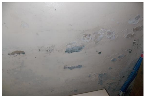
Photo 130 Peeling of Plaster on Wall No. 2 of Room No. 5 of First Floor
