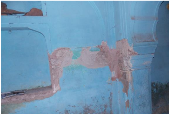
Photo 113 Peeling of Plaster on Wall No. 1 of Hall No. 1 of Ground Floor
