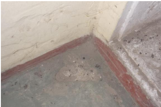
Photo 20 Peeling of Plaster on Floor of Room No. 1 of First Floor
