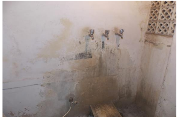
Photo 108 Dampness/Seepage on Wall No. 4 of Toilet No. 2 of Second Floor
