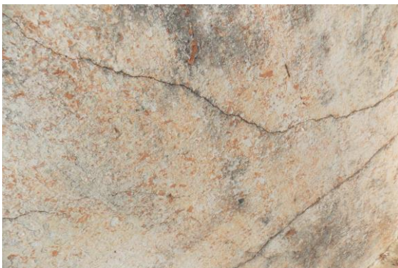
Photo 40 Plaster Crack on Parapet Wall 1 of Terrace
