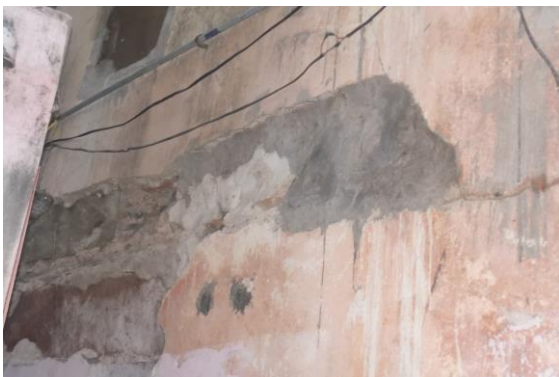
Photo 39 Peeling of Plaster on Back Wall of of Ground Floor
