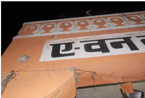
Photo 15 Inclined Crack on External L/s Column & Beam of Varanda of Shop no.314, Ground Floor Approx. Width = 0.8mm, Approx. Length = 1.5m. Dist. from L/s Wall = 0.3m, Height from Floor = 3m.
