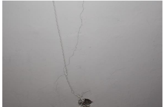
Photo 16 Inclined Crack on Roof of Shop No.213, Ground floor Approx. Width = 0.6mm, Approx. Length = 1.1m. Distance from Wall No.2 = 1m, Height from Floor = 2.8m.
