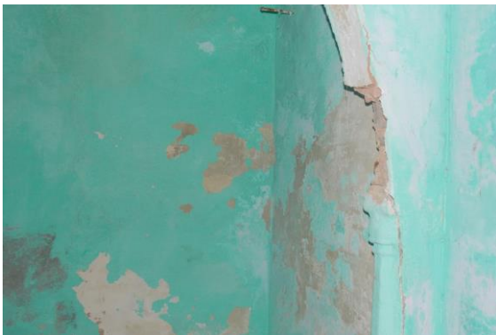
Photo 99 Peeling of Plaster on Wall No. 2 & 3 of Toilet No. 10 of House No. 2198, First Floor
