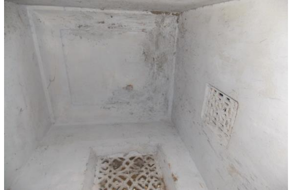
Photo 44 Dampness/Seepage on Roof of Toilet No. 1 of Ground Floor
