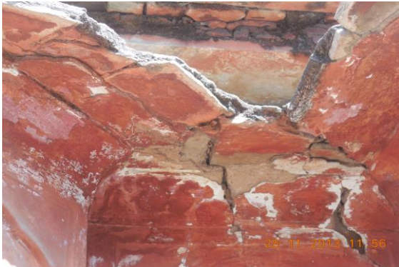
Photo 192 Peeling of Plaster on of Side B of External Façade
