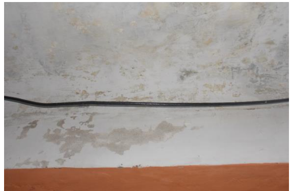
Photo 15 Peeling of Plaster on External Beam of Shop No. 295 of Ground Floor
