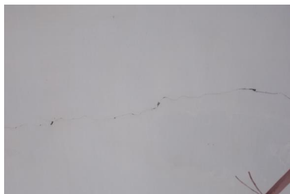
Photo 12 Horizontal Crack on Roof of Varanda of Shop No.329, Ground Floor Approx. Width = 0.3mm, Approx. Length = 1.7m. Distance from Rightside External Column = 0.4m, Height from Floor = 3.5m.
