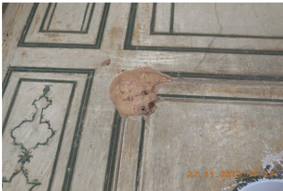
Photo 101 Peeling of Plaster on Wall No. 4 of Varanda 1 of First Floor
