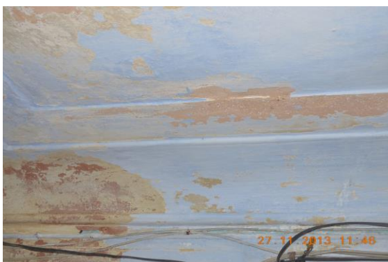
Photo 115 Peeling of Plaster on Wall No. 2 of Room No. 2 of First Floor
