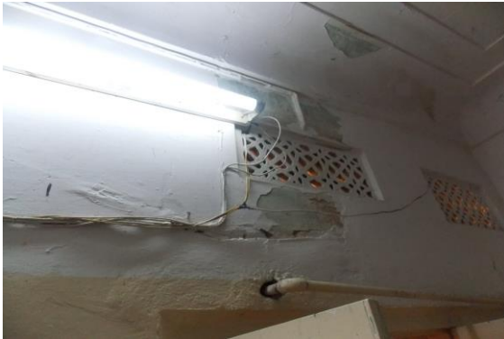
Photo 137 Peeling of Plaster on Wall No. 1 of First Floor
