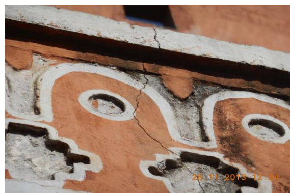
Photo 6 Inclined Crack on Outer Wall & Rightside External Wall of Varanda of Shop no.349, Ground Floor Approx. Width = 0.6mm, Approx. Length = 0.5m. Distance from Rightside External Column = 0m, Height from Floor = 3m
