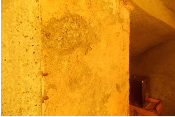
Photo 15 Peeling of Plaster on Wall No. 1 of Shop No.284 of Ground Floor
