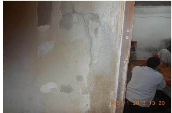
Photo 9 Inclined Crack on Wall No. 3 of Room No. 2, Shop Kailash Chand Sharma, Ground Floor Approx. Width = 0.5mm, Approx. Length = 1.5m. Distance from Wall No.1 = 1m, Height from Floor = 0m.
