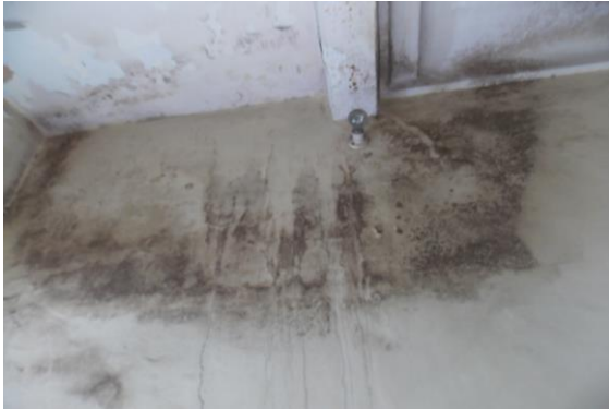
Photo 30 Dampness/Seepage on Wall No. 3 of Second Floor
