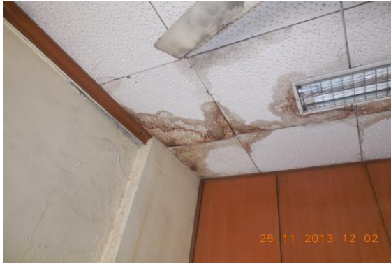
Photo 85 Dampness/Seepage on Roof of Shop No.377 of Ground Floor
