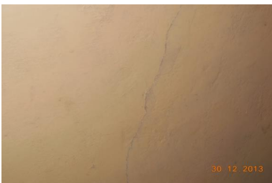
Photo 5 Inclined Crack on Wall No. 4 of Toilet No. 1, House No. 2462 First Floor Approx. Width = 0.4mm, Approx. Length = 2.6m. Distance from Wall No.2 = 0.4m, Height from Floor = 0m.
