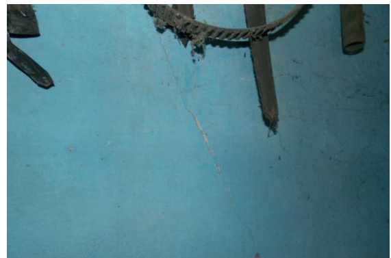
Photo 5 Inclined Crack on Wall No. 4 of Part B of Shop No.297, Ground Floor Approx. Width = 0.6mm, Approx. Length = 1.2m. Distance from Wall No.2 = 0.25m, Height from Floor = 1.2m.
