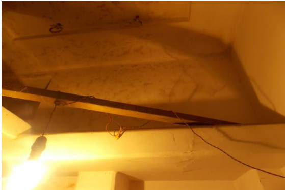
Photo 109 Dampness/Seepage on Roof & 2 of Toilet No. 2 of Second Floor
