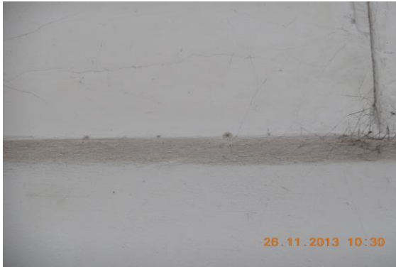
Photo 23 Peeling of Plaster on Roof of Shop No.358A of Ground Floor
