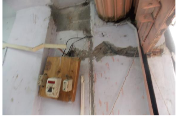
Photo 20 Peeling of Plaster on Wall No. 2 of Shop No. 5 of Ground Floor
