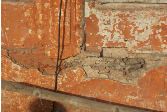
Photo 48 Peeling of Plaster on Frontside Wall of First Floor
