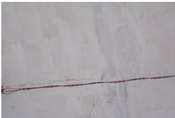
Photo 11 Horizontal Crack on Roof of Varanda of Shop No.286, Ground Floor Approx. Width = 0.35mm, Approx. Length = 2m. Distance from Leftside External Column = Backsidem, Height from Floor = 3.5m.
