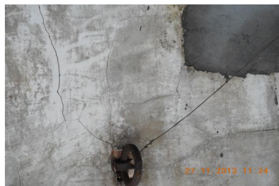
Photo 98 Plaster Crack on Wall No. 1, 4 & Roof of Varanda of First Floor
