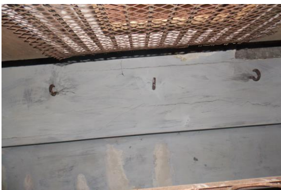
Photo 5 Horizontal Crack on Beam of Shop No. 294, Ground Floor Approx. Width = 2.5mm, Approx. Length = 2.7m. Distance from Wall No. 1 & 2 = 0m, Height from Floor = 3m.
