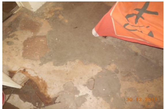
Photo 4 Peeling of Plaster on Floor of Room No. 1 of House No. 2463, First Floor
