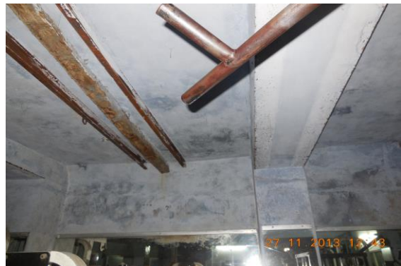
Photo 174 Dampness/Seepage on Wall No. 2 & Roof of Hall No. 1 of Ground Floor
