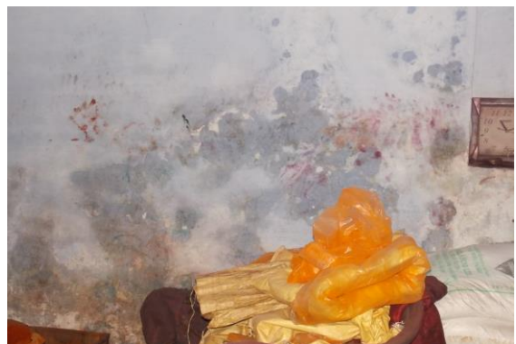
Photo 58 Dampness/Seepage on Wall No. 4 of Hall No. 2 of Ground Floor
