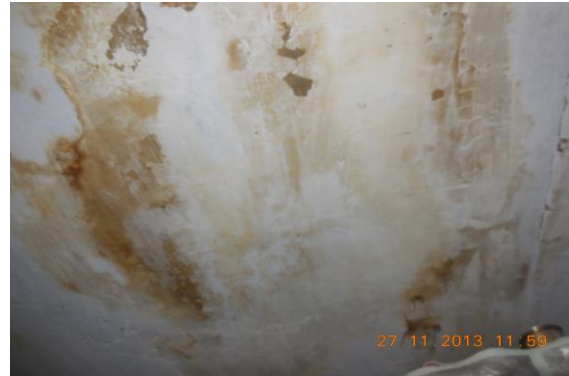
Photo 136 Dampness/Seepage on Roof of Room No. 1 of Second Floor
