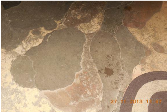
Photo 117 Peeling of Plaster on Floor of Room No. 3 of First Floor
