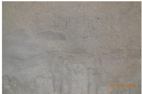
Photo 36 Plaster Crack on Wall No. 1 of Balcony of House No. 2465, Third Floor
