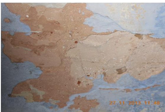
Photo 121 Damaged Portion on Roof of Room No. 3 of First Floor
