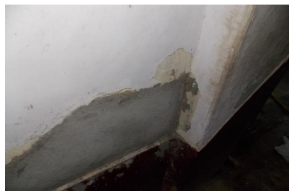
Photo 12 Peeling of Plaster on Wall No. 1 of Passage 1 of House No. 2405 to 2408 of Ground Floor
