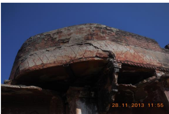
Photo 188 Peeling of Plaster on Side B of External Façade
