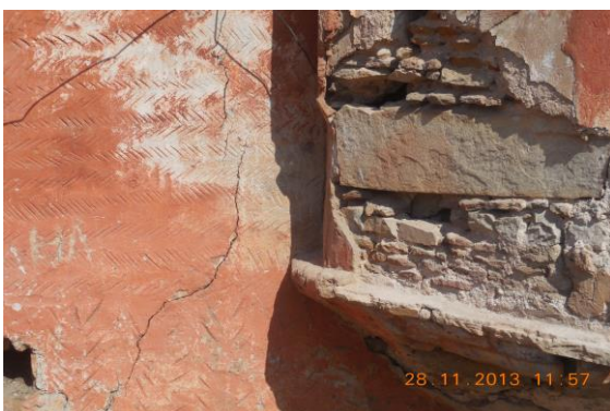
Photo 194 Peeling of Plaster on of Side B of External Façade
