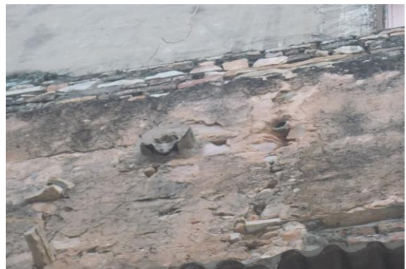
Photo 21 Peeling of Plaster on Back Side Wall of of First Floor
