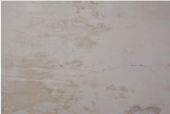
Photo 39 Horizontal Crack on Roof of Varanda of Shop No.325, Ground Floor Approx. Width = 0.25mm, Approx. Length = 1.8m. Distance Backside of Rightside external column = 1m, Height Floor = 3.5m.
