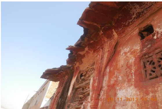
Photo 186 Peeling of Plaster on Front Side of External Façade
