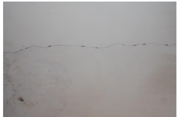
Photo 4 Horizontal Crack on Roof of Varanda of shop No.326, Ground Floor Approx. Width = 1.5mm, Approx. Length = 2m. Distance from Backside of L.S. Ext. column = 0m, Height from Floor = 3.5m.
