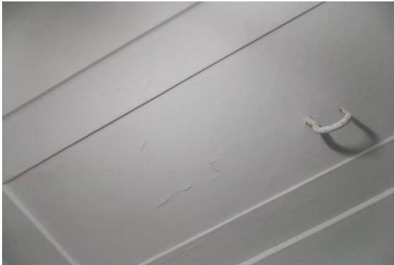
Photo 101 Peeling of Plaster on Roof of Kitchen No.2 of Second Floor
