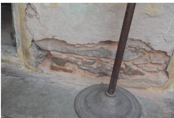
Photo 117 Peeling of Plaster on Wall No. 2 of Open Sky No.2 of Ground Floor
