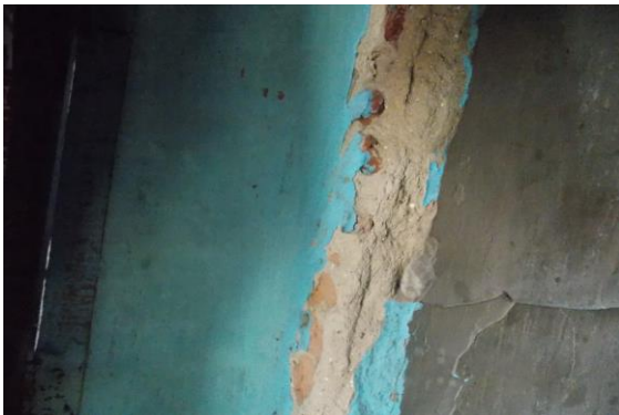
Photo 13 Peeling of Plaster on Wall No. 4 of Part A of Shop No.297 of Ground Floor
