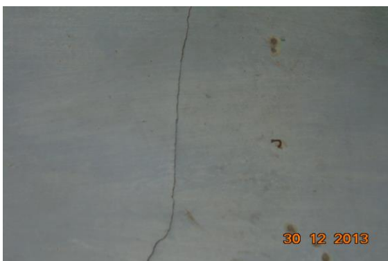
Photo 5 Inclined Crack on Wall No. 2 of Room No. 1, House No. 44 E/20, Second Floor Approx. Width = 1mm, Approx. Length = 1m. Distance from Wall 4 = 1m, Height from Floor = 1.65m.
