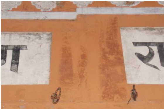
Photo 3 Inclined Crack on of External Col, Shop No. 296, Ground Floor Approx. Width = 1mm, Approx. Length = 0.8m. Height from Floor = 3m.
