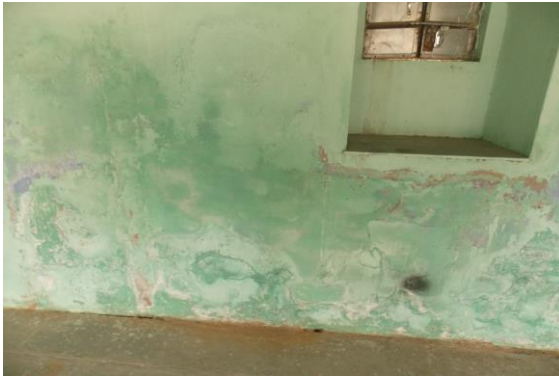
Photo 107 Dampness/Seepage on Wall No. 4 of Gallery of Ground Floor
