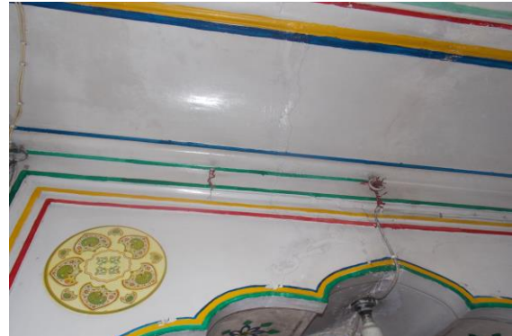
Photo 4 Inclined Crack on Wall No. 3 & Roof of Varanda 2, Part A, House No. 2414, First Floor Approx. Width = 0.3mm, Approx. Length = 1.8m. Distance from Wall No.1 = 1.5m, Height from Floor = 2.4m.
