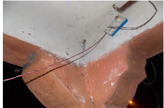
Photo 14 Horizontal Crack on L/s External Column of Varanda of Shop no.314, G/F Approx. Width = 0.8mm, Approx. Length = 0.6m.
