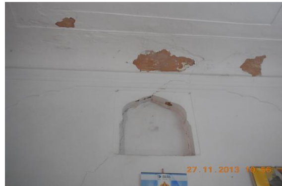
Photo 70 Dampness/Seepage on Roof of Office 1 of First Floor
