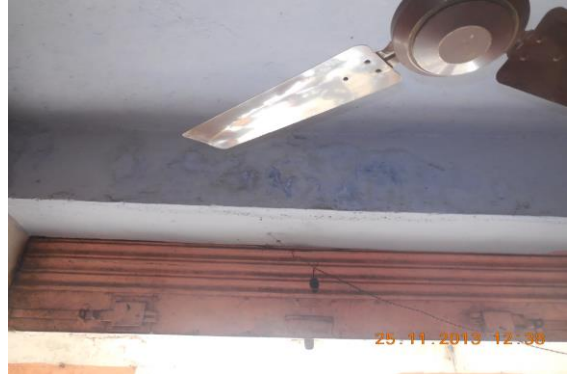
Photo 100 Dampness/Seepage on Wall No. 3 of Shop No.366 of Ground Floor
