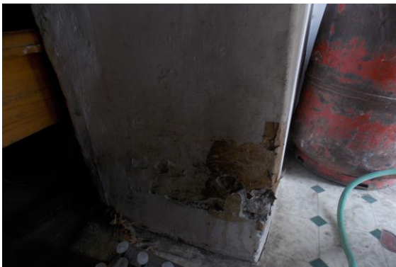
Photo 9 Peeling of Plaster on Wall No. 2 of Hall No. 1 of House No. 2414 First Floor
