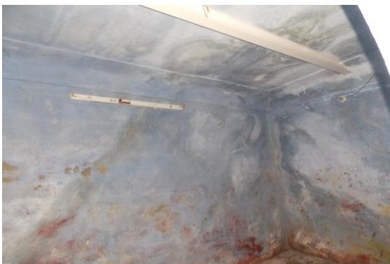
Photo 57 Dampness/Seepage on All Walls & Roof of Room No. 2 of Ground Floor
