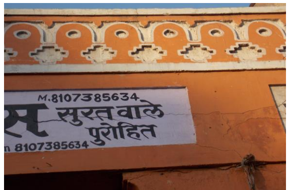
Photo 12 Inclined Crack on External Beam of Varanda of Shop No.286, Ground Floor Approx. Width = 2.5mm, Approx. Length = 3m. Heiht from Floor = 3.5m.
