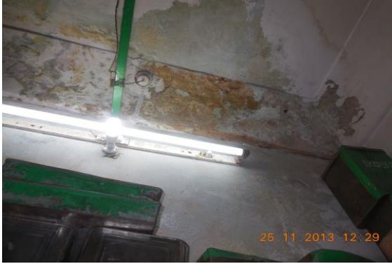
Photo 97 Peeling of Plaster on Roof of Room No. 2 of Ground Floor
