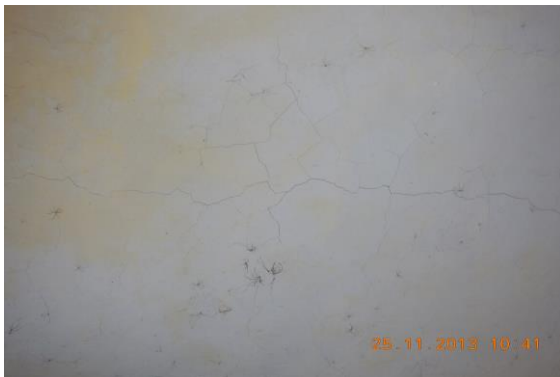
Photo 27 Horizontal Crack on Roof of Shop No.376, Ground Floor Approx. Width = 0.8mm, Approx. Length = 2m. Distance from Wall No.3 = 0m, Height from Floor = 3m.
