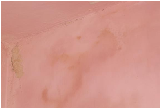
Photo 35 Dampness/Seepage on Wall No. 4 of Kitchen of House No. 1908 Second Floor
