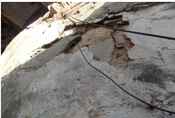
Photo 58 Peeling of Plaster on Wall No. 2 of Staircase Ground Floor to First Floor
