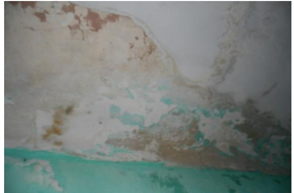
Photo 98 Dampness/Seepage on Roof of Toilet No. 10 of House No. 2198, First Floor
