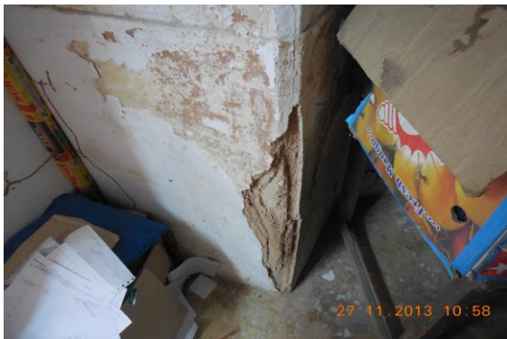
Photo 71 Peeling of Plaster on Wall No. 4 of Store 1 of First Floor
