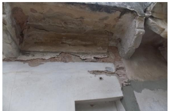
Photo 101 Peeling of Plaster on Wall No. 4 of Open Sky 1 of House No. 2198, First Floor
