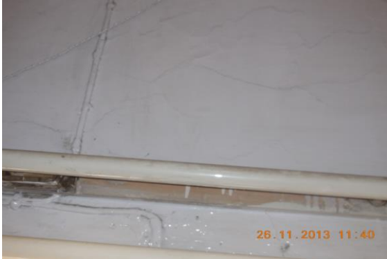
Photo 47 Peeling of Plaster on Wall No. 3 of Part A of Shop No.350 of Ground Floor
