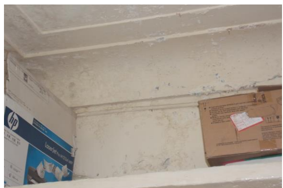
Photo 136 Dampness/Seepage on Wall No. 2 of First Floor
