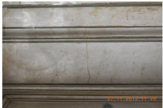
Photo 90 Plaster Crack on Wall No. 1, 4 & Roof of Varanda of First Floor
