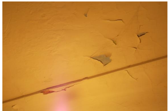
Photo 140 Peeling of Plaster on Roof of Toilet No. 1 of First Floor
