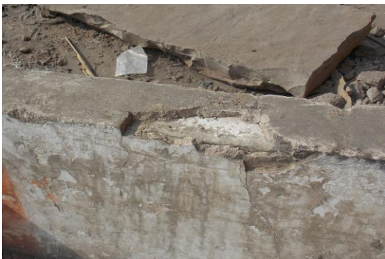
Photo 22 Peeling of Plaster on Wall No. 2 of Varnadah of First Floor
