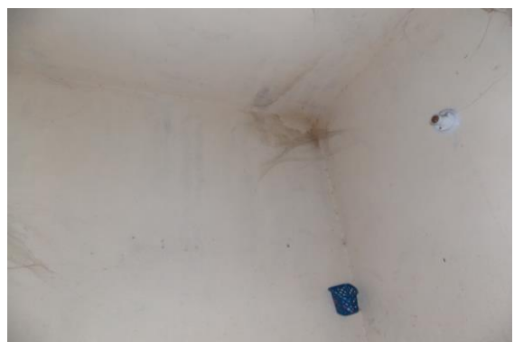
Photo 112 Dampness/Seepage on Wall No. 4 & Roof of Bathroom of Ground Floor
