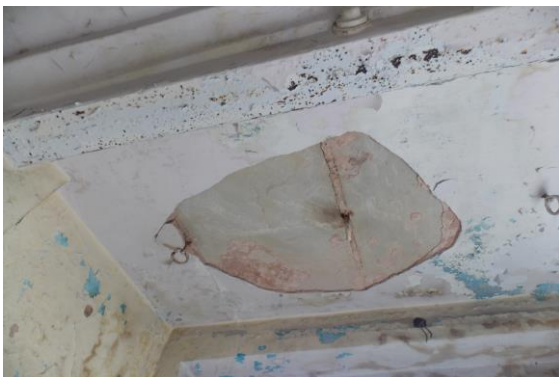
Photo 28 Peeling of Plaster on Roof of Room No. 2 of Second Floor
