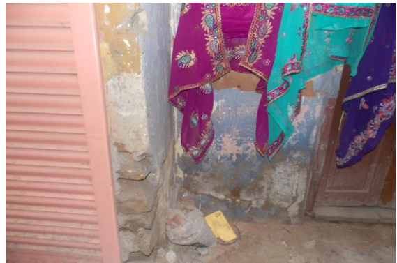
Photo 38 Peeling of Plaster on Front Wall of Ground Floor
