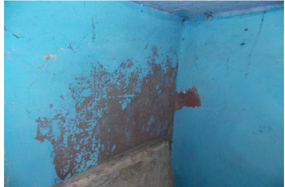
Photo 12 Peeling of Plaster on Wall No. 1 & 3 of Part B of Shop No.297 of Ground Floor
