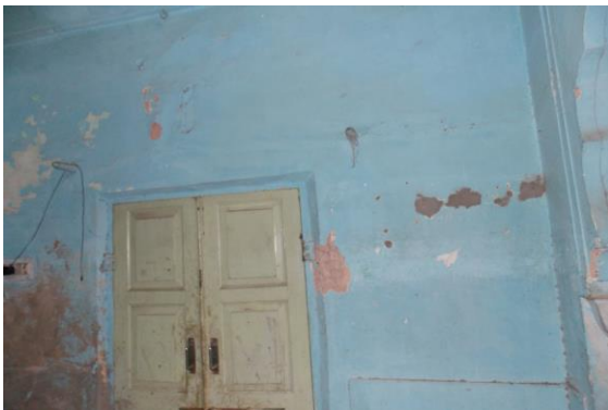
Photo 115 Peeling of Plaster on Wall No. 2 of Hall No. 1 of Ground Floor
