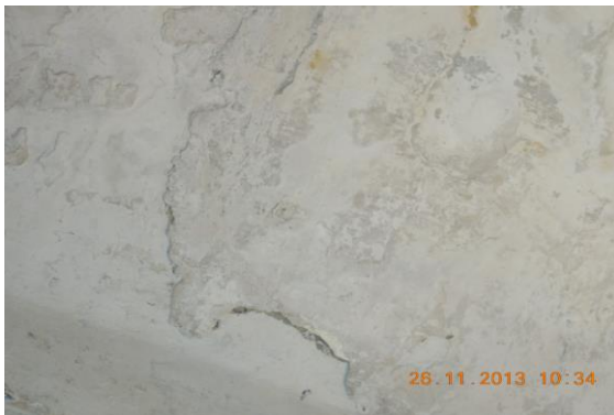
Photo 25 Peeling of Plaster on Beam of Varanda of Shop No.358 of Ground Floor
