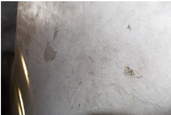
Photo 26 Peeling of Plaster on Wall No. 2 of First Floor
