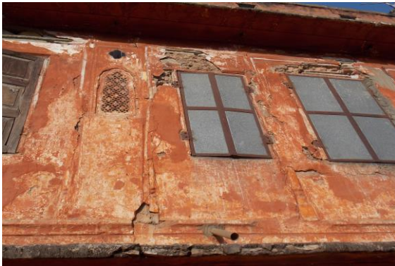
Photo 54 Peeling of Plaster on Frontside Wall of Second Floor
