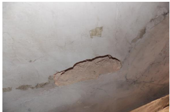
Photo 17 Peeling of Plaster on Wall No. 2 of Stair GF to FF
