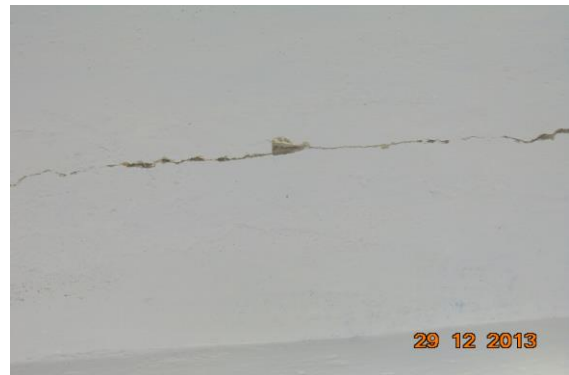
Photo 10 Horizontal Crack on Roof of House No. 2405 to 2408, First Floor Approx. Width = 0.5mm, Approx. Length = 2m. Distance from Wall No. 3 = 0.2m, Height from Floor = 2.5m.
