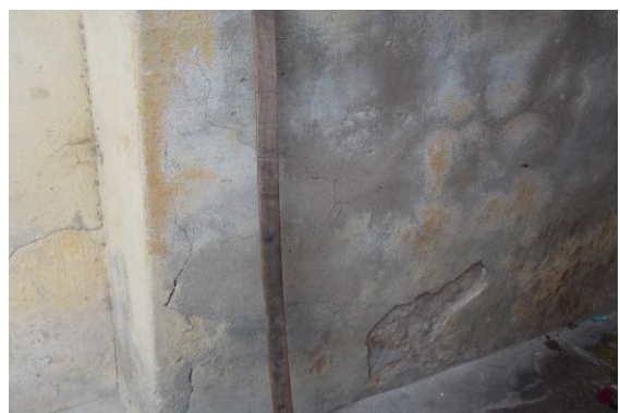
Photo 118 Peeling of Plaster on Wall No. 4 of Open Sky No.2 of Ground Floor
