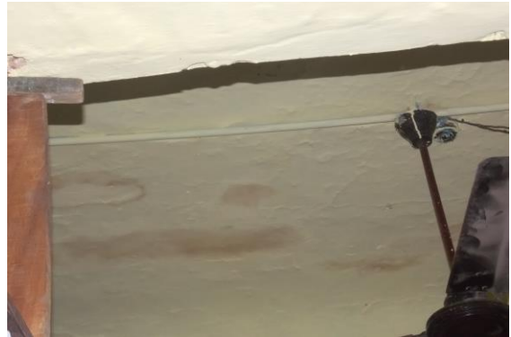
Photo 26 Dampness/Seepage on Roof of Shop Aggarwal Chai Bhandar of Ground Floor
