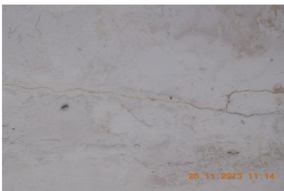
Photo 11 Inclined Crack on Rightside External Column of Shop No.354, Ground Floor Approx.Width = 0.5mm, Approx.Length = 3m.Distance from Rightside External Column = ,Heightom Floor= 3m.
