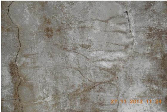
Photo 99 Plaster Crack on Wall No. 1, 4 & Roof of Varanda of First Floor
