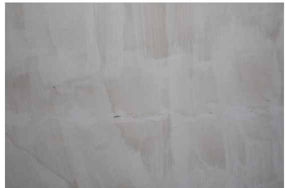
Photo 16 Horizontal Crack on Roof of Varanda of shop No.313, Ground Floor Approx. Width = 0.35mm, Approx. Length = 2m. Distance from Leftside External Column = 0.4m, Height from Floor = 3.5m.
