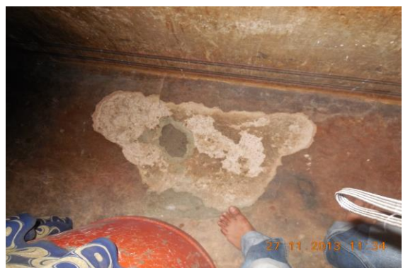
Photo 104 Peeling of Plaster on Floor of Passage 1 of First Floor
