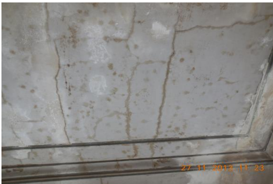
Photo 95 Plaster Crack on Wall No. 1, 4 & Roof of Varanda of First Floor
