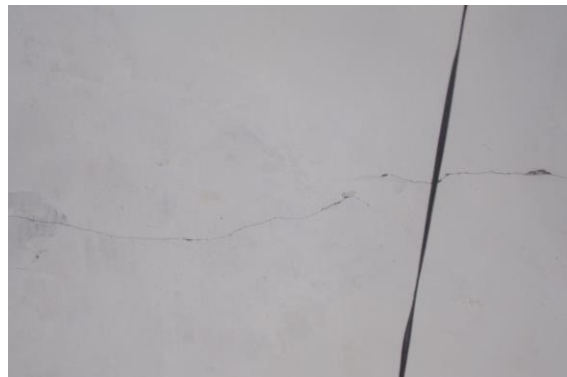
Photo 10 Horizontal Crack on Roof of Varanda of Shop No.329, Ground Floor Approx. Width = 0.35mm, Approx. Length = 2m. Distance from = Backside of L.S. ext col, Height from Floor = 3.5m.
