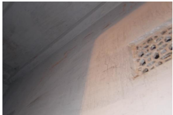
Photo 46 Peeling of Plaster on Wall No. 2 of Passage No.2 of Ground Floor
