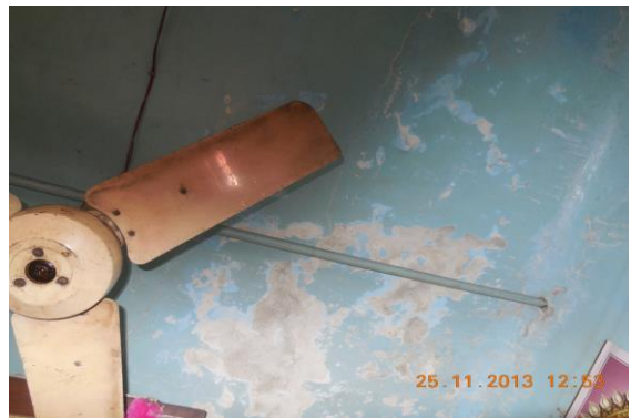
Photo 102 Dampness/Seepage on Roof & 4 of Shop No.363 of Ground Floor
