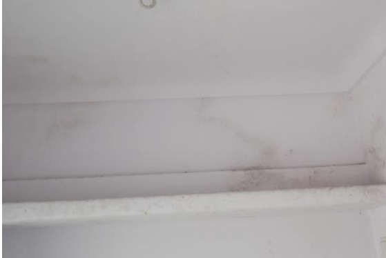
Photo 85 Dampness/Seepage on Wall No. 2, 4 & Roof of Room No. 4 of Second Floor
