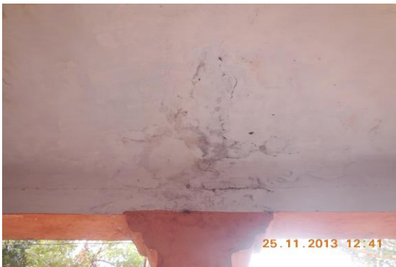
Photo 101 Dampness/Seepage on Roof of Varanda of Shop No.366 of Ground Floor
