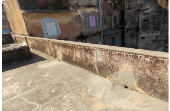
Photo 132 Peeling of Plaster on Wall No. 2 of Room No. 1 of House No. 2144, Second Floor
