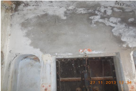
Photo 153 Peeling of Plaster on Wall No. 1 of Varanda 2 of Ground Floor
