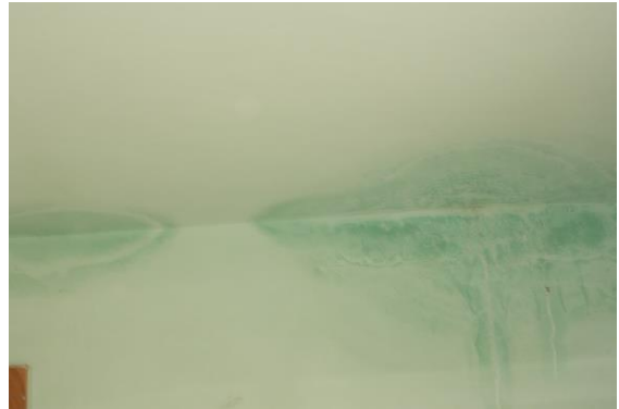
Photo 108 Dampness/Seepage on Wall No. 2 & Roof of Gallery of Ground Floor
