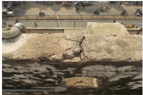
Photo 39 Peeling of Plaster on Parapet Wall 3 of Terrace
