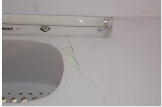
Photo 84 Peeling of Plaster on Wall No. 3 of Hall No. 3 of Second Floor
