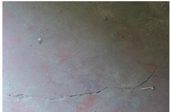
Photo 21 Peeling of Plaster on Floor of Room No. 1 of First Floor
