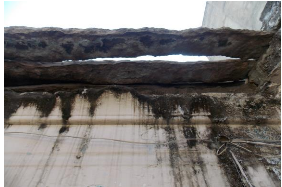
Photo 25 Peeling of Plaster on Wall No. 2 of Open Sky of Second Floor
