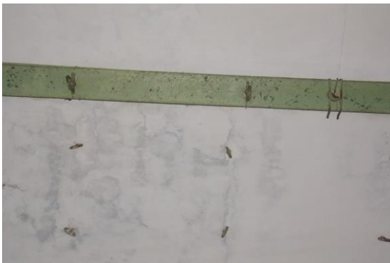
Photo 103 Dampness/Seepage on Roof of Hall No. 1 of Second Floor
