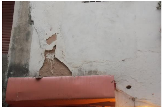
Photo 36 Peeling of Plaster on House No. 1908 Second Floor
