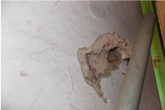
Photo 18 Peeling of Plaster on Wall No. 1 of First Floor
