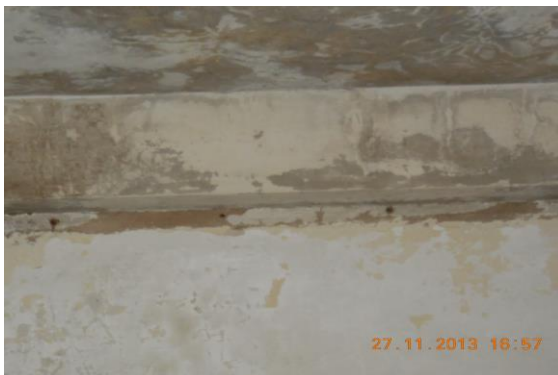
Photo 86 Dampness/Seepage on Wall No. 2 of Passage 1 of Munshi Shopping Complex, Second Floor
