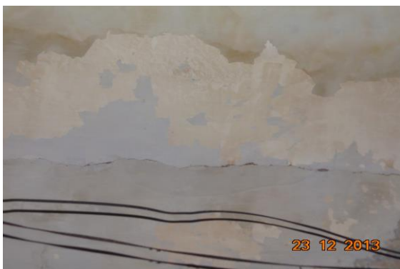
Photo 5 Horizontal Crack on Roof of Varanda of Shop No.299, Ground Floor Approx. Width = 1mm, Approx. Length = 2.8m. Distance from Leftside External Column = 0m, Height from Floor = 2.5m.
