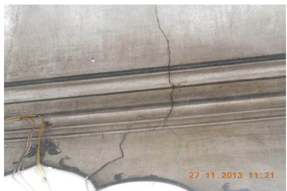
Photo 92 Plaster Crack on Wall No. 1, 4 & Roof of Varanda of First Floor
