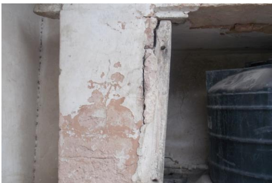
Photo 101 Peeling of Plaster on Wall No. 4 of Open Sky 1 of House No. 2198, First Floor
