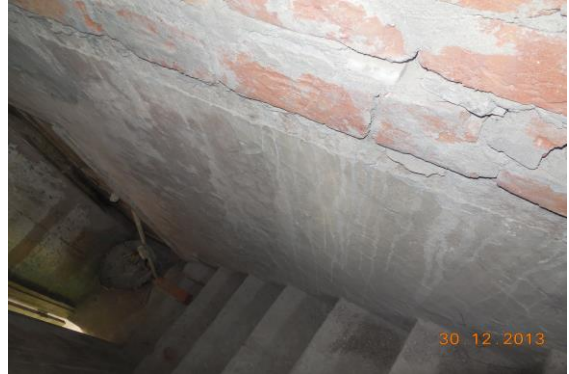
Photo 34 Peeling of Plaster on Wall No. 1 of Staircase Second Floor to Third Floor of House No. 2465, Second Floor
