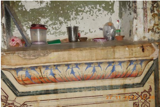
Photo 149 Peeling of Plaster on Wall No. 1 of Room No. 1 of Ground Floor
