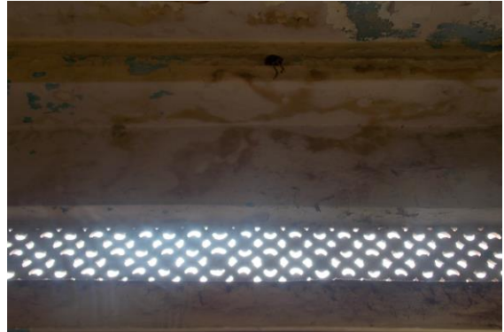
Photo 31 Dampness/Seepage on Wall No. 2 of Second Floor
