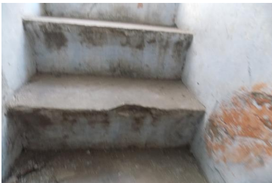
Photo 28 Peeling of Plaster on Wall No. Steps of Staircase Second Floor To Third Floor
