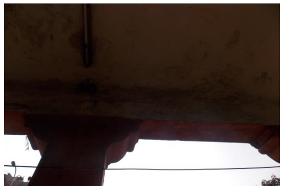
Photo 118 Dampness/Seepage on Varanda Roof of Shop No. 332, Ground Floor
