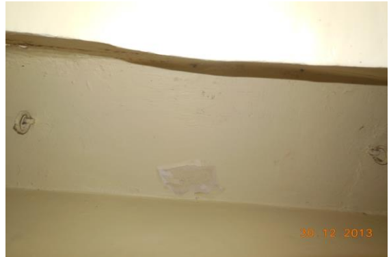
Photo 2 Peeling of Plaster on Roof of Varanda 1 of House No. 2463, First Floor
