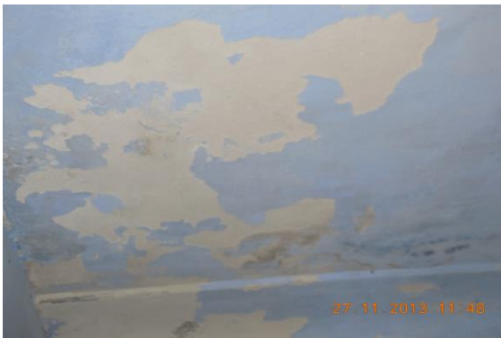
Photo 119 Peeling of Plaster on Roof of Bathroom 1 of First Floor
