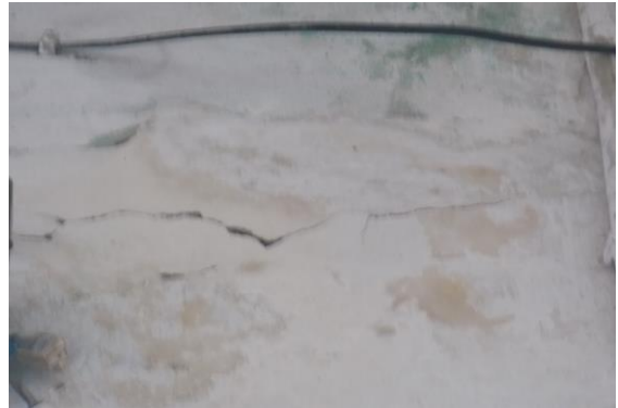
Photo 40 Horizontal Crack on Beam of Varanda of shop no.324, Ground Floor Approx. Width = 0.5mm, Approx. Length = 1.3m. Distance Backside of Leftside external column = 0m, Height Floor = 3.3m.
