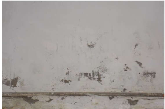
Photo 138 Peeling of Plaster on Wall No. 4 of First Floor
