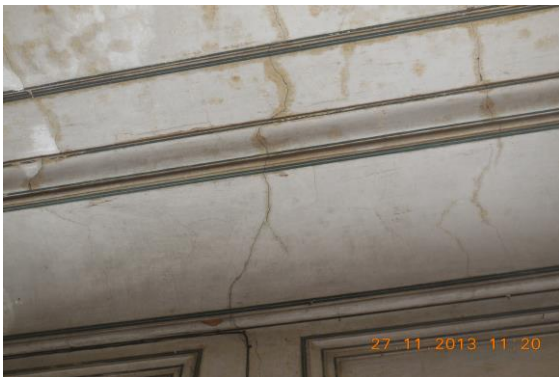
Photo 89 Plaster Crack on Wall No. 1, 4 & Roof of Varanda of First Floor
