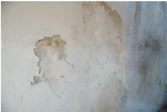
Photo 26 Peeling of Plaster on Wall No. 1 of Staircase Second Floor To Third Floor
