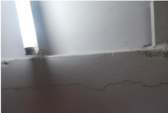
Photo 21 Peeling of Plaster on Roof of Part B of Shop No. 4, Ground Floor
