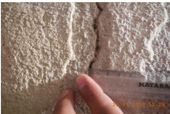
Photo 9A Inclined Crack on Wall No. 3 of Room No. 2, Shop Kailash Chand Sharma, Ground Floor Approx. Width = 0.5mm, Approx. Length = 1.5m. Distance from Wall No.1 = 1m, Height from Floor = 0m.
