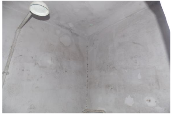
Photo 114 Dampness/Seepage on Room No. 3 of Fourth Floor
