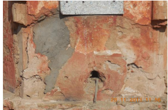
Photo 191 Peeling of Plaster on of Side B of External Façade
