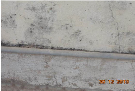
Photo 12 Plaster Crack on Wall No. 2 of Open Sky of House No. 2469, Terrace
