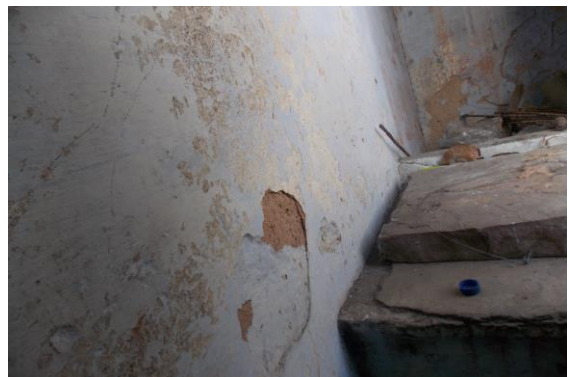
Photo 29 Peeling of Plaster on Wall No. 1 of Staircase Second Floor To Third Floor
