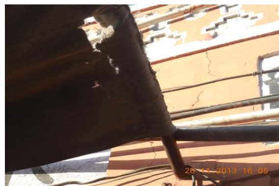
Photo 12 Inclined Crack on R/s External Column of Varanda of Shop No.343, G/F Approx. Width = 0.6mm, Approx. Length = 1.15m. Distance from R/s External Column = 0m, Height from Floor = 3m.
