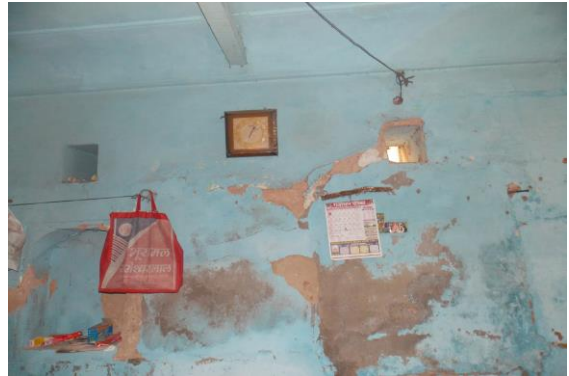
Photo 114 Peeling of Plaster on Wall No. 4 of Hall No. 1 of Ground Floor
