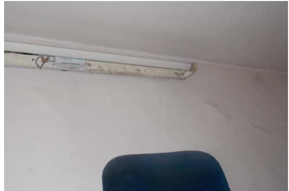
Photo 8 Peeling of Plaster on Wall No. 1 of Hall No. 1 of House No. 2414 First Floor
