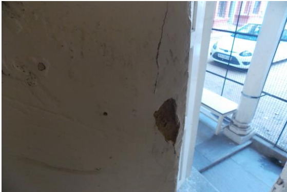
Photo 133 Peeling of Plaster on Wall No. 2 of First Floor
