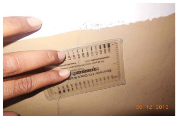
Photo 5A Inclined Crack on Wall No. 4 of Toilet No. 1, House No. 2462 First Floor Approx. Width = 0.4mm, Approx. Length = 2.6m. Distance from Wall No.2 = 0.4m, Height from Floor = 0m.
