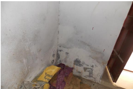
Photo 109 Dampness/Seepage on Wall No. 4 & 5 of Passage of Ground Floor
