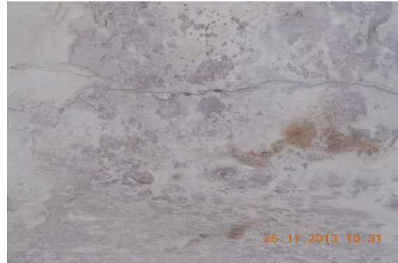
Photo 26 Horizontal Crack on of Varanda of Shop No.381, Ground Floor Approx. Width = 0.2mm, Approx. Length = 2m. Distance from Leftside Wall = Backsidem, Height from Floor = 3m.
