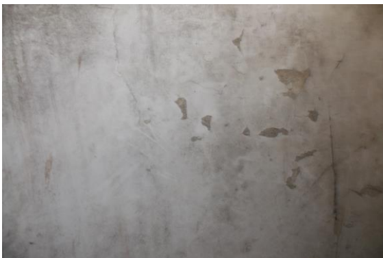
Photo 34 Peeling of Plaster on Wall No. 4 of Second Floor
