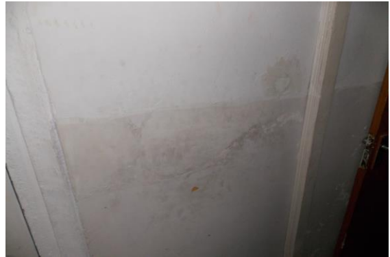
Photo 102 Dampness/Seepage on Wall No. 2 of Hall No. 3 of Second Floor
