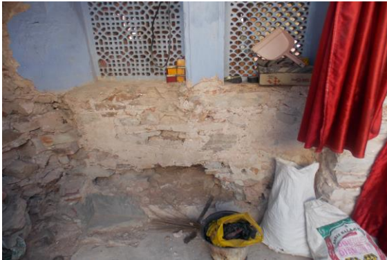
Photo 17 Peeling of Plaster on Open Sky Wall 3, Part A of House No. 2414, First Floor
