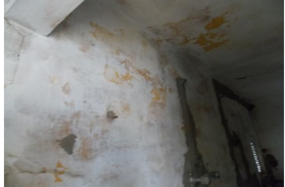
Photo 86 Dampness/Seepage on Wall No. 4 & Roof of Toilet No. Toilet & Bathroom No.3 of Second Floor
