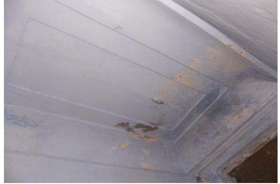
Photo 96 Dampness/Seepage on Wall No. 4 & Roof of Toilet No. 1 of Second Floor
