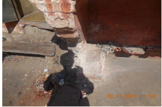
Photo 197 Peeling of Plaster on Side B of External Façade
