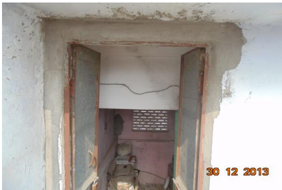
Photo 14 Peeling of Plaster on Wall No. 3 of Open Sky of House No. 2469, Terrace
