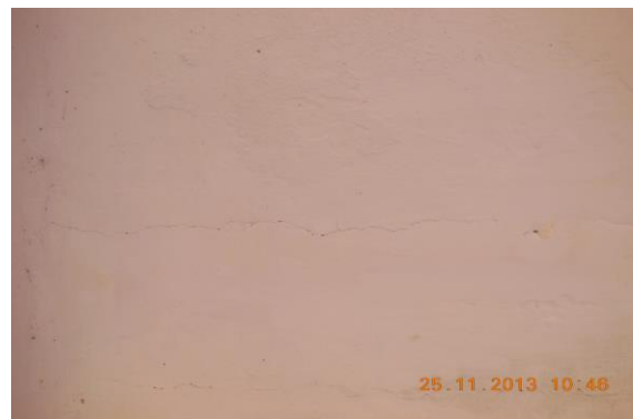
Photo 30 Horizontal Crack on Roof of Varanda of Shop No.376, Ground Floor. Approx. Width = 2mm, Approx. Length = 1.7m. Distance from Leftside External Column = Backsidem, Height from Floor = 2.8m.
