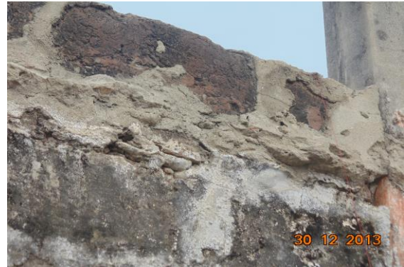
Photo 13 Peeling of Plaster on Wall No. 3 of Open Sky of House No. 2469, Terrace
