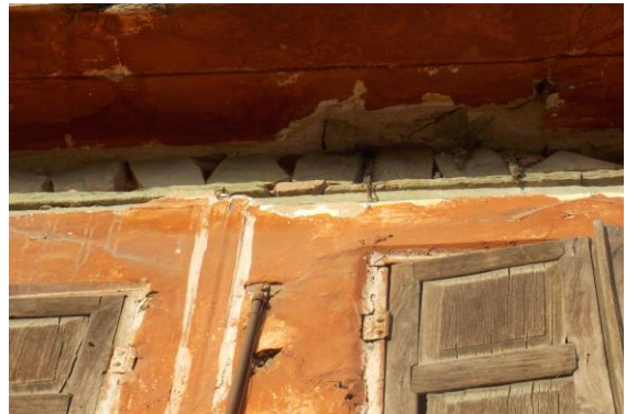
Photo 55 Peeling of Plaster on Frontside Wall of Second Floor
