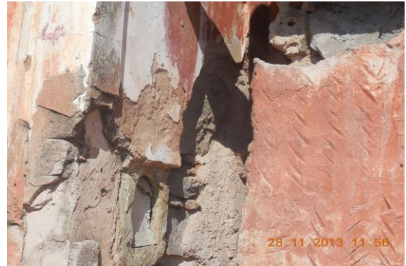
Photo 193 Peeling of Plaster on of Side B of External Façade
