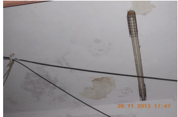
Photo 2 Dampness/Seepage on Roof of Varanda of Shop No.335 of Ground Floor
