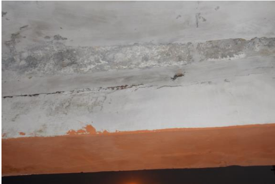
Photo 12 Exposed Reinforcement on Beam of Shop No. 294 of Ground Floor
