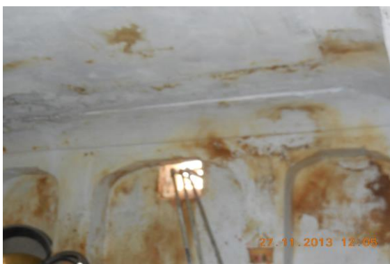
Photo 139 Dampness/Seepage on Wall No. 1 & Roof of Room No. 2 of Second Floor
