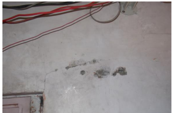
Photo 10 Peeling of Plaster on Wall No. 1 of Hall No. 2 of House No. 2414 First Floor
