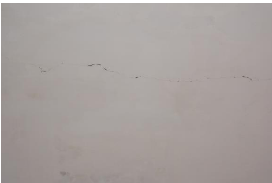
Photo 41 Horizontal Crack on Roof of Varanda of Shop No.321, Ground Floor Approx. Width = 0.35mm, Approx. Length = 2m. Distance from Leftside External column = 0.8m, Height from Floor = 3.5m.
