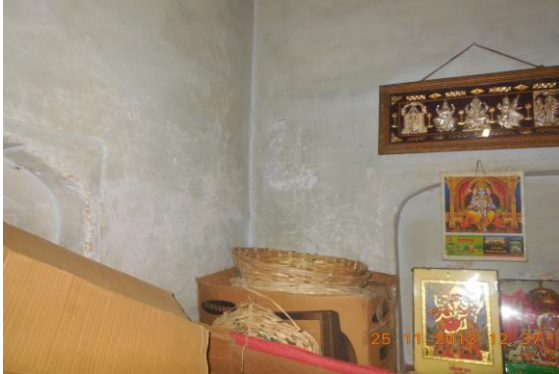
Photo 99 Dampness/Seepage on Wall No. 4 & 1 of Room No. 1 of Ground Floor
