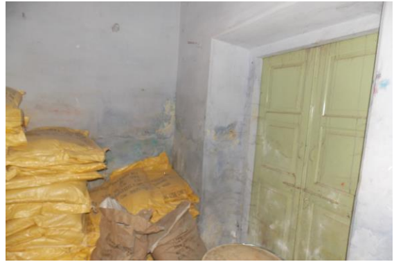
Photo 54 Dampness/Seepage on Wall No. 2 & 3 of Hall No. 1 of Ground Floor
