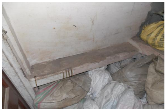
Photo 106 Peeling of Plaster on Wall No. 1 of Store No.1 of Second Floor
