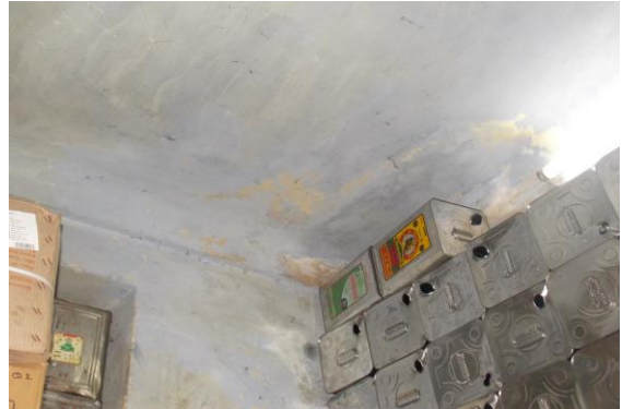
Photo 13 Peeling of Plaster on Wall No. 2, 4 & Roof of Shop No. 295 of Ground Floor
