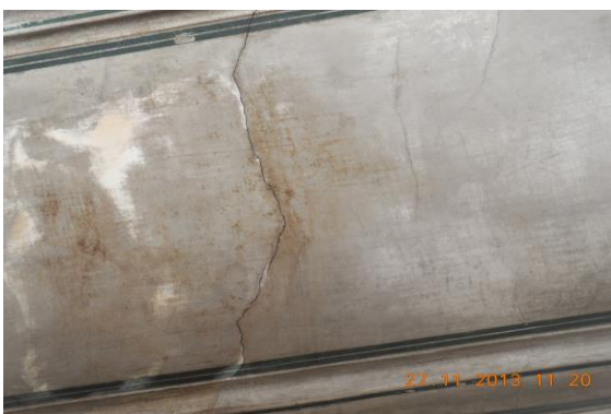
Photo 91 Plaster Crack on Wall No. 1, 4 & Roof of Varanda of First Floor
