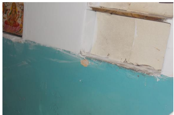
Photo 12 Peeling of Plaster on Wall No. 1 of Room No. 1 of House No. 2414 First Floor
