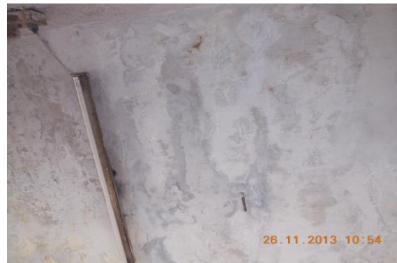
Photo 26 Dampness/Seepage on Varanda of Shop No.357 of Ground Floor
