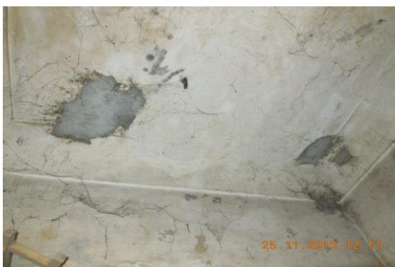
Photo 89 Peeling of Plaster on Roof of Room No. 2 of Ground Floor
