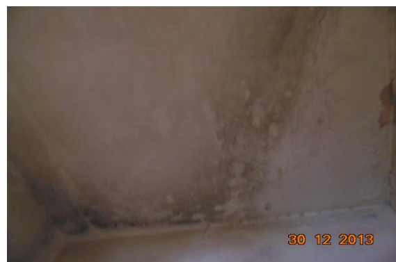
Photo 17 Dampness/Seepage on Roof of Stair Third Floor to Terrace of House No. 2469, Terrace
