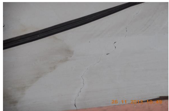
Photo 10 Inclined Crack on Outer Wall of Shop No.360, Ground Floor Approx. Width = 0.2mm, Approx. Length = 3m. Distance from Internal Leftside Beam = 0.7m, Height from Floor = 3m.
