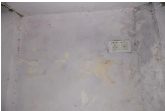
Photo 23 Peeling of Plaster on Wall No. 2 of Basement of Shop No. 4, Basement
