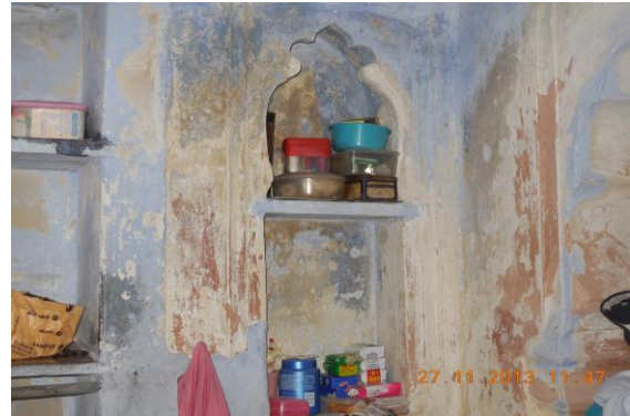
Photo 118 Dampness/Seepage on Wall No. 2 & 4 of Bathroom 1 of First Floor
