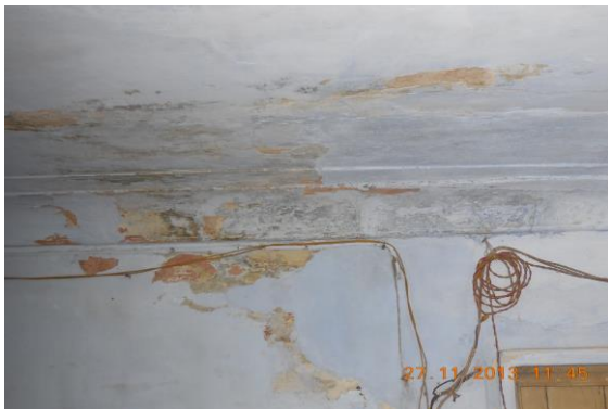
Photo 113 Peeling of Plaster on Wall No. 1 of Room No. 2 of First Floor
