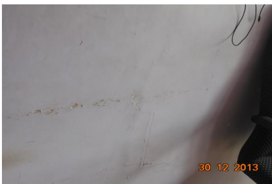
Photo 4 Peeling of Plaster on Wall No. 1 of Room No. 1 of House No. 2469, Third Floor
