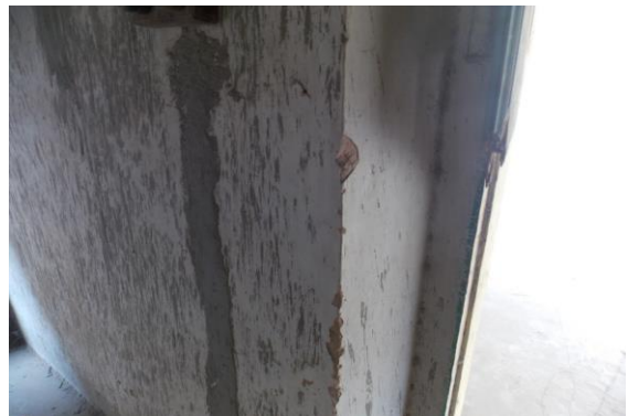
Photo 88 Peeling of Plaster on Wall No. 3 of Room No. 3 of Second Floor
