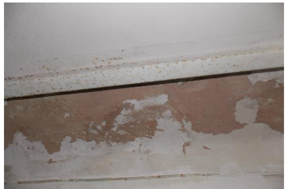
Photo 128 Peeling of Plaster on Roof of First Floor
