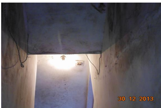
Photo 16 Dampness/Seepage on Wall No. 1, 2, 3 & Roof of Stair Third Floor to Terrace of House No. 2469, Terrace
