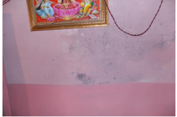
Photo 16 Peeling of Plaster on Wall No. 4 of Shop No.284 of Ground Floor
