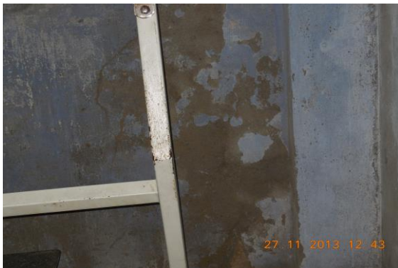
Photo 173 Dampness/Seepage on Wall No. 1 of Hall No. 1 of Ground Floor
