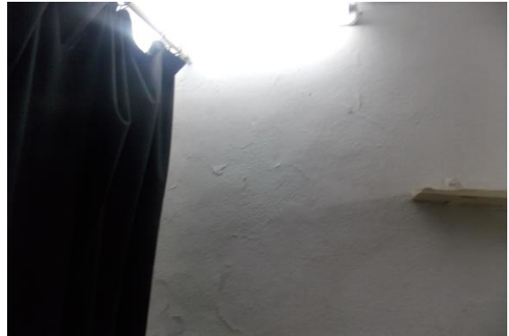
Photo 126 Peeling of Plaster on Wall No. 4 of Room No. 2 of First Floor
