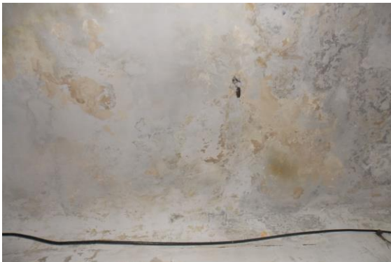
Photo 14 Peeling of Plaster on Roof of Varandah of Shop No. 295, Ground Floor
