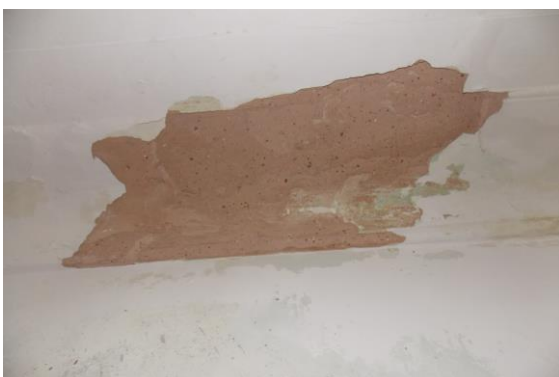
Photo 129 Peeling of Plaster on Roof & 3 of Room No. 5 of First Floor
