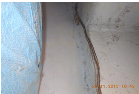
Photo 29 Vertical Crack on Wall No. 2 of Shop No.376, Ground Floor. Approx. Width = 0.8mm, Approx. Length = 3m. Distance from Wall No.2 = 0m, Height from Floor = 0m.
