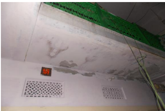
Photo 99 Dampness/Seepage on Wall No. 4 & Sunshade of open area of Second Floor
