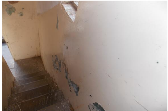
Photo 132 Peeling of Plaster on Wall No. 1 of First Floor
