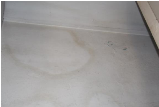
Photo 32 Dampness/Seepage on Wall No. 1 of Second Floor
