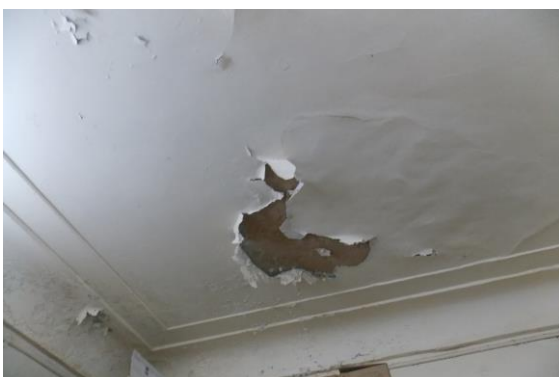
Photo 135 Peeling of Plaster on Roof of Hall No. 1 of First Floor
