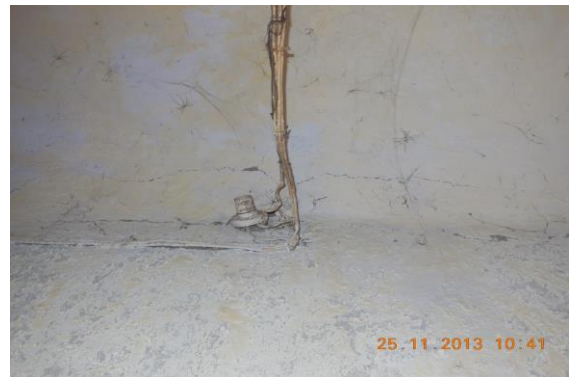
Photo 28 Horizontal Crack on Wall No. 3 of Shop No.376, Ground Floor Approx. Width = 0.4mm, Approx. Length = 1.5m. Distance from Wall No.2 = 0m, Height from Floor = 2.8m.
