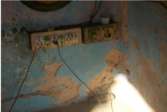
Photo 11 Peeling of Plaster on Wall No. 2 & 4 of Part A of Shop No.297 of Ground Floor
