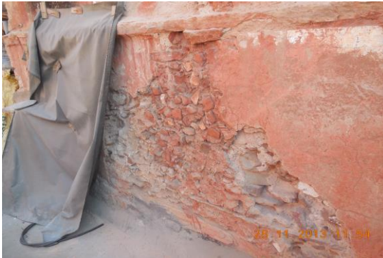
Photo 184 Peeling of Plaster on Front Side of External Façade
