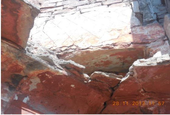
Photo 196 Peeling of Plaster on Side B of External Façade
