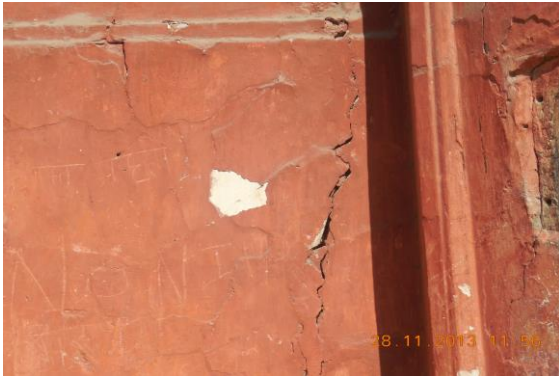
Photo 190 Peeling of Plaster on of Side B of External Façade
