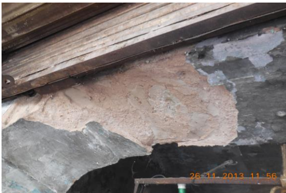
Photo 49 Peeling of Plaster on Entry Gate Roof of Part A of Shop No.351 of Ground Floor
