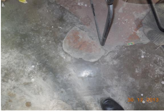
Photo 31 Peeling of Plaster on Floor of House No. 2465, Second Floor
