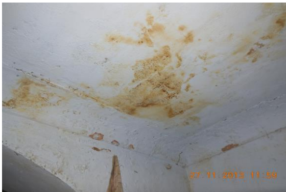
Photo 137 Peeling of Plaster on Floor of Room No. 1 of Second Floor
