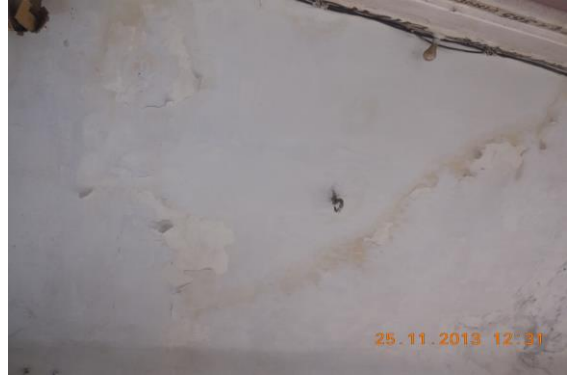
Photo 98 Dampness/Seepage on Roof of Varanda of Shop No.365 of Ground Floor
