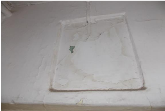
Photo 125 Peeling of Plaster on Wall No. 4 of First Floor
