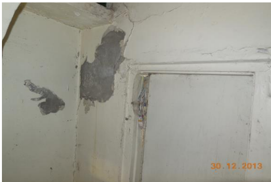
Photo 3 Peeling of Plaster on Wall No. 1 & 4 of Varanda No.1 of House No. 2463, First Floor
