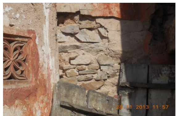
Photo 195 Peeling of Plaster on of Side B of External Façade
