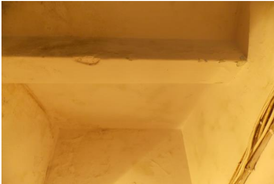
Photo 131 Dampness/Seepage on Roof & 4 of Stair GF to FF
