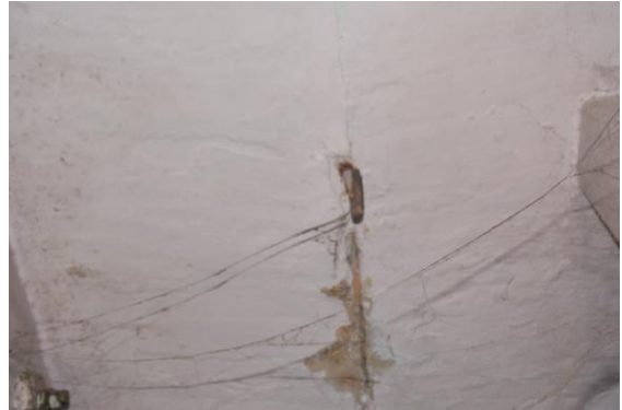
Photo 19 Peeling of Plaster on Roof of Lobby of First Floor
