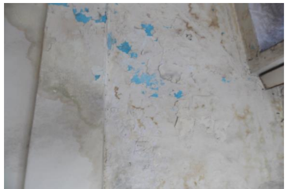
Photo 29 Dampness/Seepage on Wall No. 4 of Second Floor
