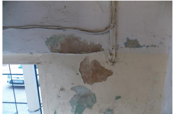
Photo 134 Peeling of Plaster on Wall No. 3 of First Floor
