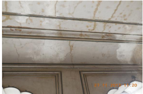
Photo 88 Plaster Crack on Wall No. 1, 4 & Roof of Varanda of First Floor
