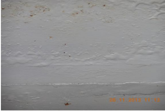
Photo 45 Peeling of Plaster on Roof of Shop No.354 of Ground Floor
