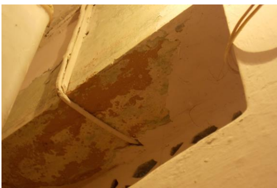
Photo 141 Peeling of Plaster on Wall No. 3 of Toilet No. 1 of First Floor
