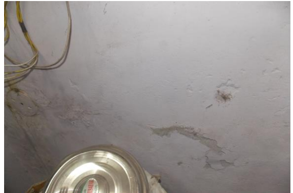
Photo 22 Peeling of Plaster on Wall No. 2 of Stair Gf To Basement of Shop No. 4, Ground Floor
