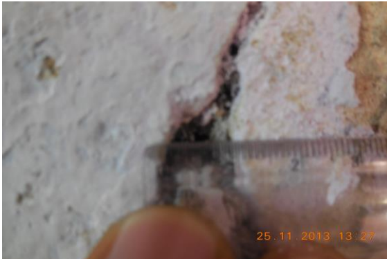
Photo 8A Horizontal Crack on Roof of Room No. 1, Shop Kailash Chand Sharma, Ground Floor Approx. Width = 10mm, Approx. Length = 2.3m. Distance from Wall No.2 = 0m, Height from Floor = 1.5m.
