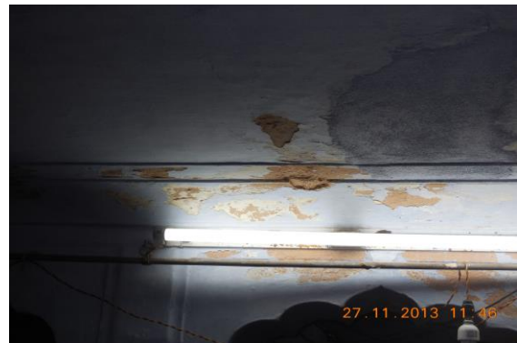
Photo 114 Peeling of Plaster on Wall No. 4 of Room No. 2 of First Floor
