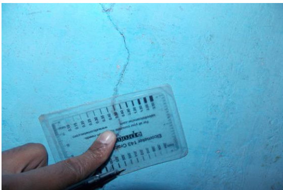
Photo 4A Inclined Crack on Wall No. 4 of Part B of Shop No.297, Ground Floor Approx. Width = 0.5mm, Approx. Length = 1.8m. Distance from Wall No.2 = 1.1m, Height from Floor = 0m.
