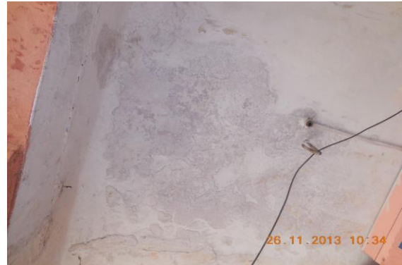
Photo 24 Dampness/Seepage on Roof of Varanda of Shop No.358 of Ground Floor
