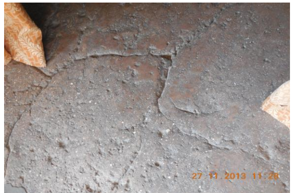
Photo 102 Peeling of Plaster on Floor of Room No. 1 of First Floor
