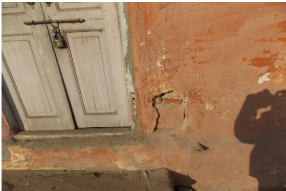
Photo 50 Peeling of Plaster on Frontside Wall of First Floor
