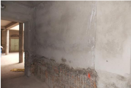
Photo 55 Peeling of Plaster on Wall No. 5 of Passage
