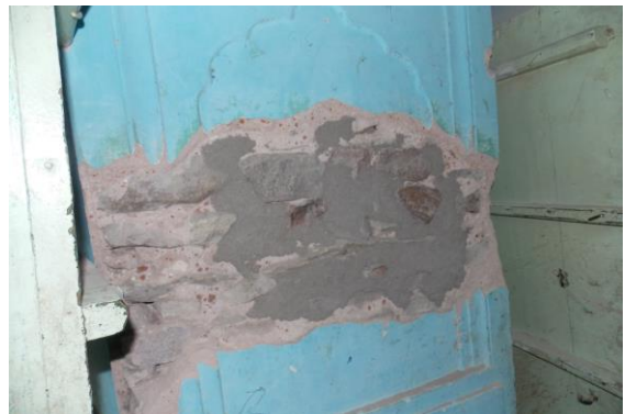
Photo 116 Peeling of Plaster on Wall No. 3 of Hall No. 1 of Ground Floor
