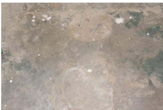
Photo 11 Peeling of Plaster on Wall No. 1 of Hall No. 1 of House No. 2405 to 2408, Ground Floor
