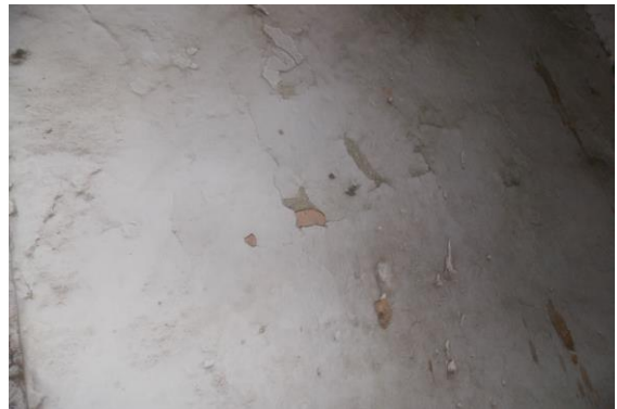
Photo 27 Peeling of Plaster on Wall No. 4 of First Floor
