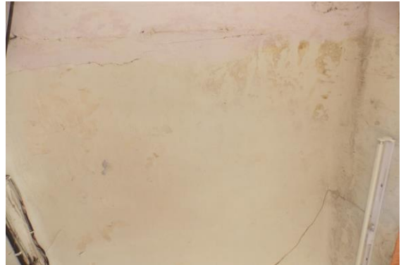
Photo 116 Dampness/Seepage on of Varandah Roof of Shop No. 332, Ground Floor
