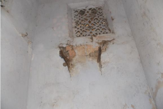
Photo 43 Peeling of Plaster on Wall No. 4 of Toilet No. 1 of Ground Floor
