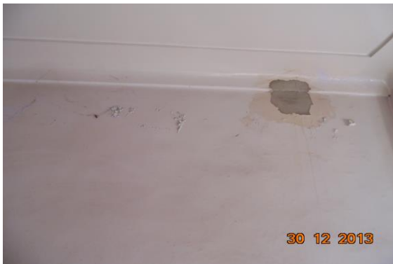
Photo 2 Peeling of Plaster on Wall No. 4 of Room No. 1 of House No. 2469, First Floor
