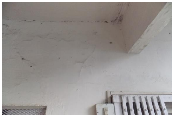
Photo 40 Peeling of Plaster on Wall No. 4 of Balcony of Shop No. SF 01 Second Floor
