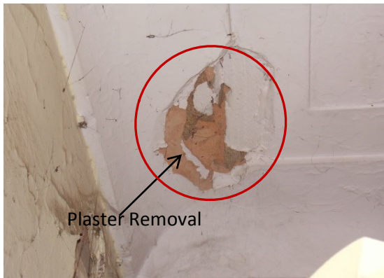
Photo 22A Plaster Removal on Roof of Gallery of House above Shop No.59, First floor
