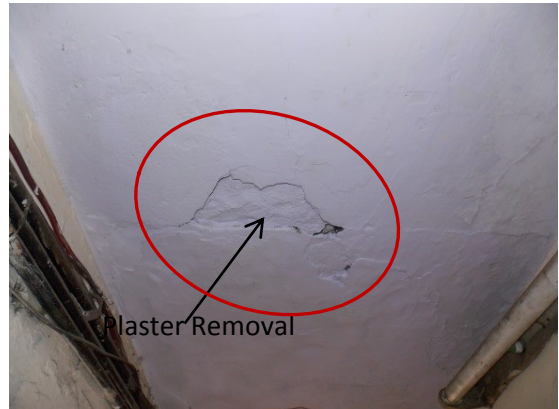
Photo 21 Plaster Removal on Roof of Stair of House above Shop No.59, First floor
