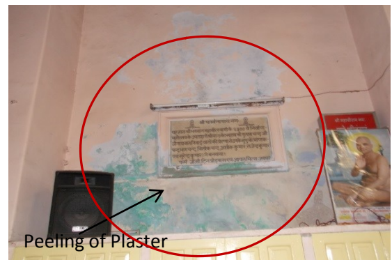
Photo 31 Peeling of Plaster on Wall No.4 of Hall No.2 of H.No.1144 Ground Floor
