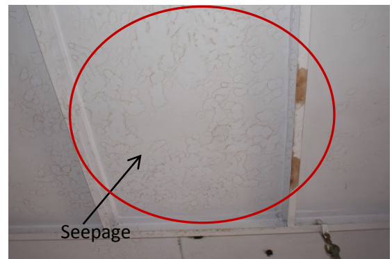
Photo 40 Seepage on Roof of Hall No.1 (Second Floor)
