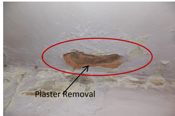
Photo 62 Plaster Removal on Roof of Lobby (4th Floor)
