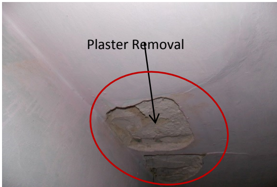
Photo 31 Plaster Removal on Roof of Passage of above Shop No.59, Second floor
