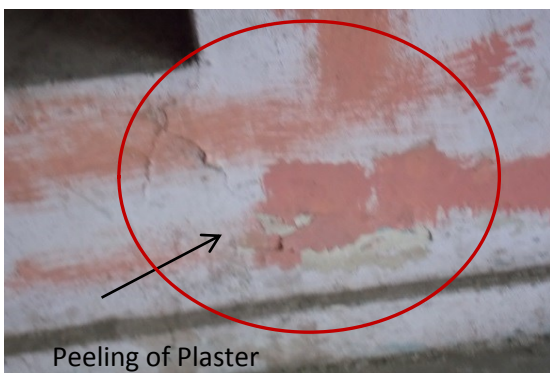
Photo 41 Peeling of Plaster on Wall No.4 of Hall No.1 (Second Floor)
