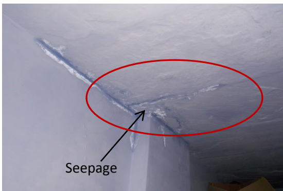
Photo 42 Seepage on Roof of Room No.1 of H.No.1144 First Floor
