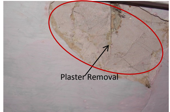
Photo 30 Plaster Removal on Roof of Staircase of above Shop No.59, First floor
