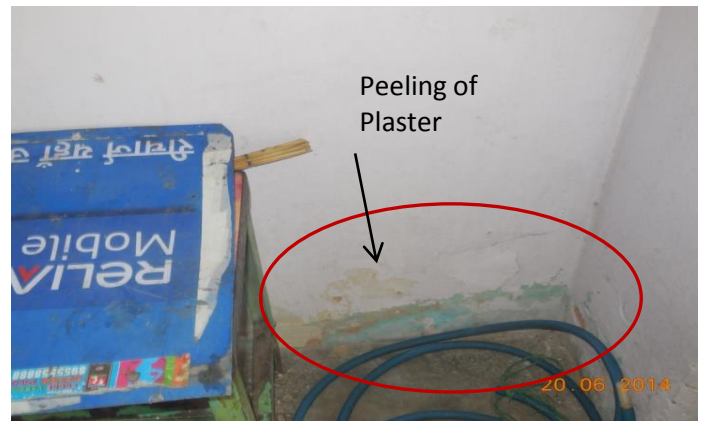
Photo 4 Peeling of plaster from wall no.2, shop no.4, Ground Floor
