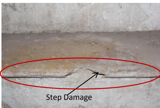
Photo 27 Step Damage of Stair Case of House above Shop No.59, Part A, First floor
