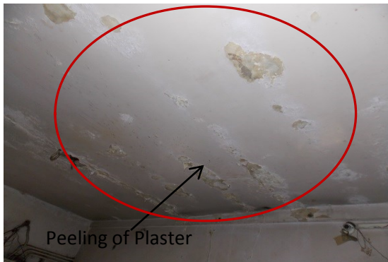
Photo 49 Peeling of Plaster on Roof of Kitchen No.1 (Third Floor)
