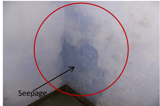
Photo 47 Seepage on Wall No.2 of Room No.9 of H.No.1144 First Floor
