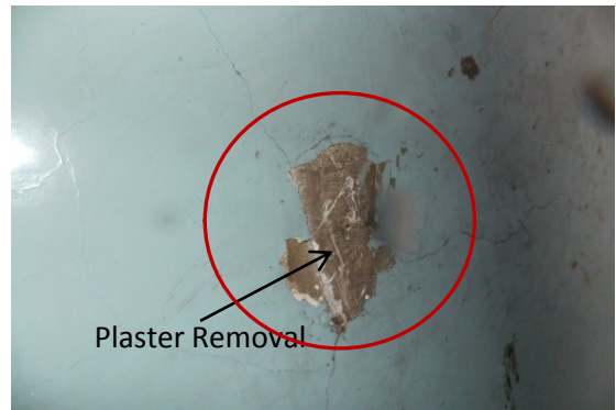
Photo 58 Plaster Removal on Wall No.4 of Stair T.F. to 4th F. (4th Floor)
