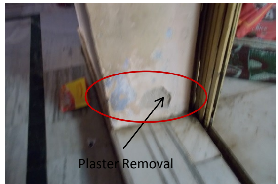
Photo 33 Plaster Removal on Wall No.1 of Gate No.1 of Hall No.2 Ground Floor
