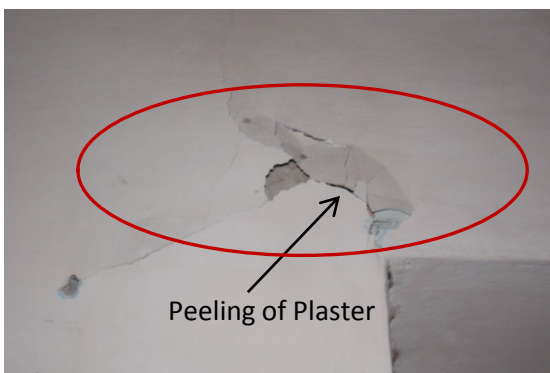
Photo 38 Peeling of Plaster on Wall No.3 of Hall No.1 of H.No.1144, First Floor
