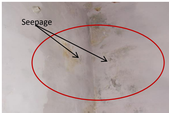
Photo 3 Seepage on Wall No.1 & 4 of Part-C of Shop No.72 Ground Floor
