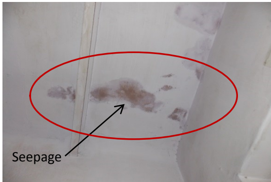
Photo 37 Seepage on Roof of Hall No.2, Second Floor
