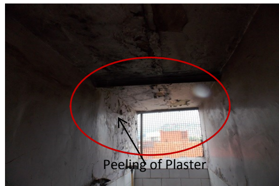
Photo 64 Peeling of Plaster on All Walls of Toilet No.1 (4th Floor)
