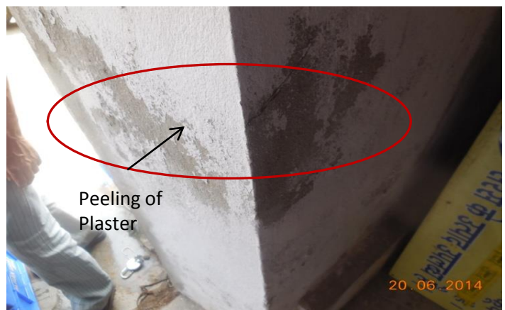
Photo 6 Peeling of plaster from wall no.3, shop no.1 Ground Floor
