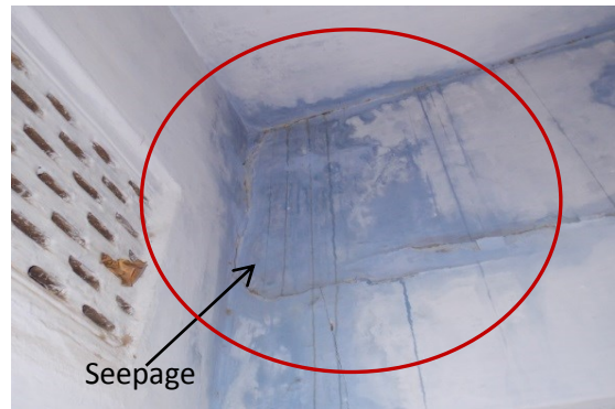
Photo 53 Seepage on Wall No.2 of Open Sky of H.No.1144 First Floor
