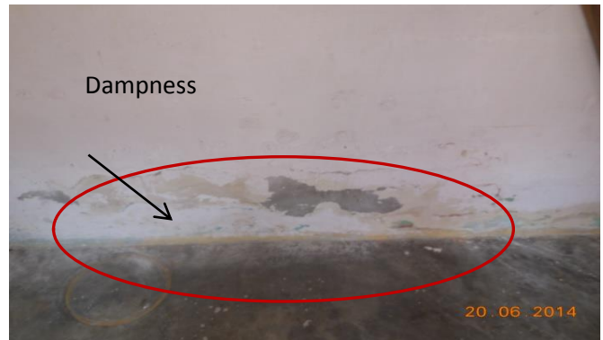
Photo 2 Dampness on Wall No. 4 of Shop No. 4, Ground Floor
