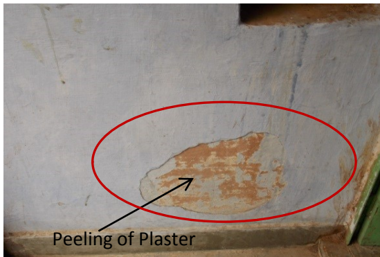
Photo 52 Peeling of Plaster on Wall No.2 of Open Sky of H.No.1144 First Floor
