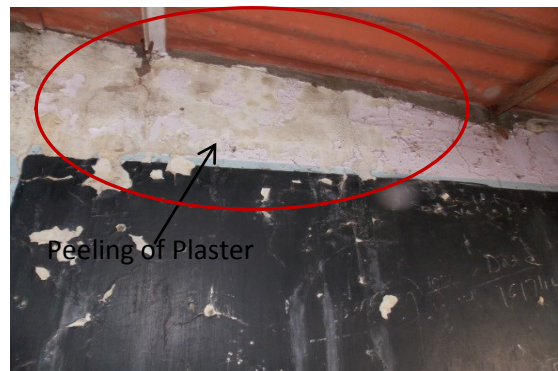
Photo 66 Peeling of Plaster on Wall No.3 of Tinshade Room (4th Floor)
