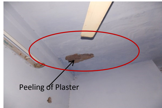
Photo 49 Peeling of Plaster on Roof of Room No.9 of H.No.1144 First Floor
