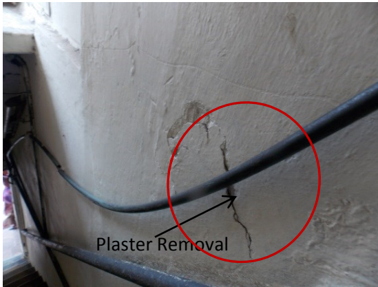
Photo 20 Plaster Removal on Wall No.1 of Stair of H.above Shop No.59, First floor
