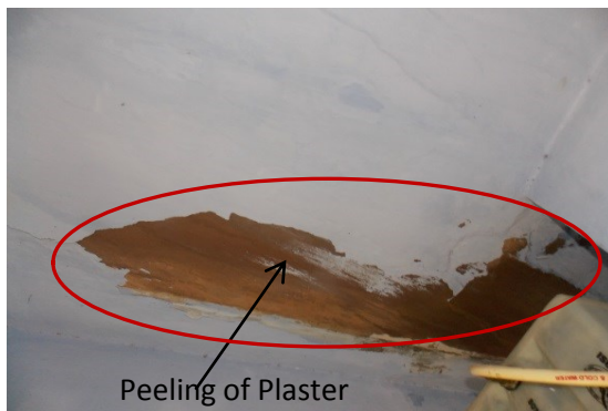
Photo 56 Peeling of Plaster on Roof of Washroom of H.No.1144 First Floor
