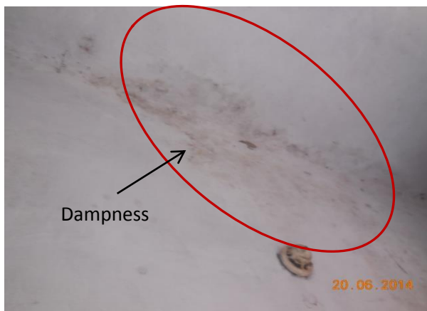
Photo 5 Dampness on roof, shop no.1, Ground Floor
