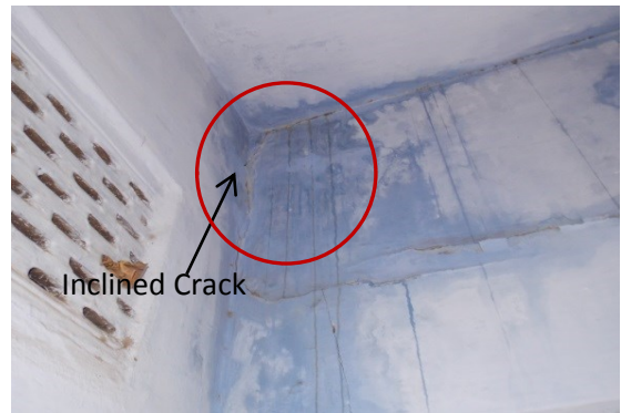
Photo 23 Inclined Crack on Wall No.2 to Roof of Opensky of H.No.1144(F.F.) Approx. Width = 1.0mm, Approx. Length = 1.50m. Distance from Wall No.4= 0m, Height from Floor = 2.20m.
