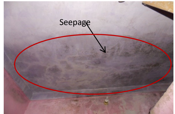
Photo 32 Seepage on Roof of Lobby of House above Shop No.59, Second floor
