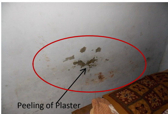
Photo 48 Peeling of Plaster on Wall No.1 of Room No.9 of H.No.1144 First Floor
