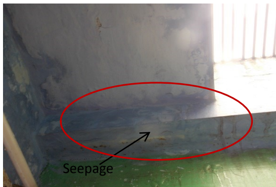
Photo 54 Seepage on Roof of Open Sky of H.No.1144 First Floor
