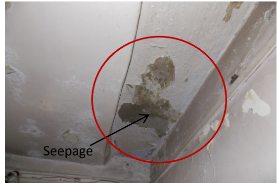
Photo 50 Seepage on Roof of Kitchen No.1 (Third Floor)
