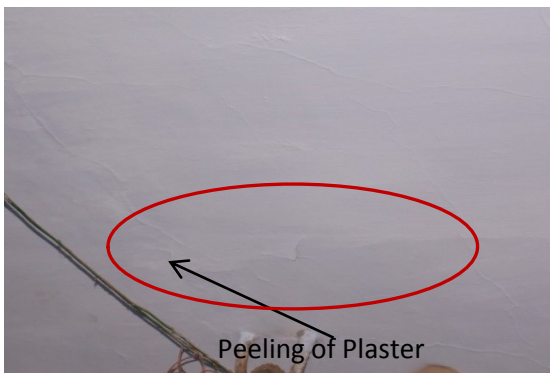
Photo 36 Peeling of Plaster on Roof of Room No.3 of H.No.1144, First Floor
