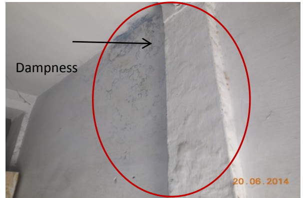
Photo 1 Dampness/Seepage on Wall No. 2 of Shop No. 325, Ground Floor
