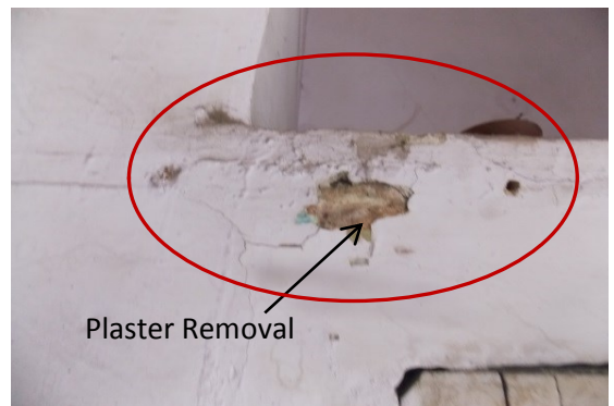
Photo 42 Plaster Removal on Wall No.4 of Hall No.1 (Second Floor)
