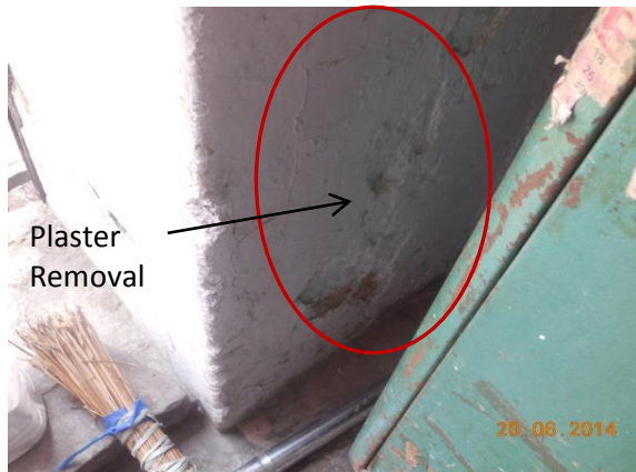
Photo 3 Plaster Removal of wall no.3, shop no.4, Ground Floor
