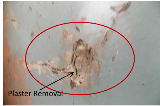
Photo 56 Plaster Removal on Wall No.4 of Stair T.F. to 4th F. (4th Floor)
