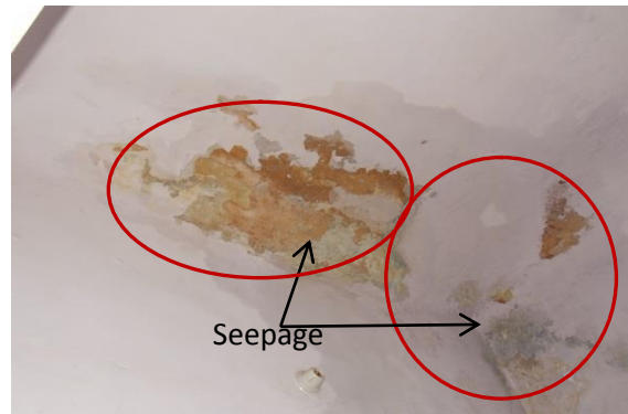
Photo 2 Seepage on Roof of Part-C of Shop No.72 Ground Floor
