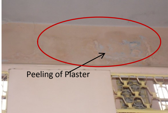
Photo 58 Peeling of Plaster on Wall No.1 of Balcony of H.No.1144 First Floor
