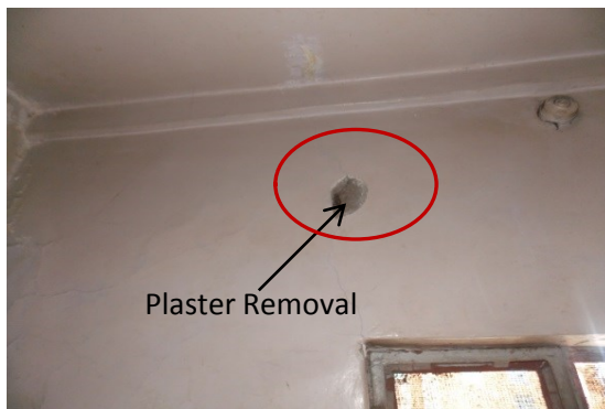
Photo 53 Plaster Removal on Wall No.4 of Kitchen No.1 (Third Floor)
