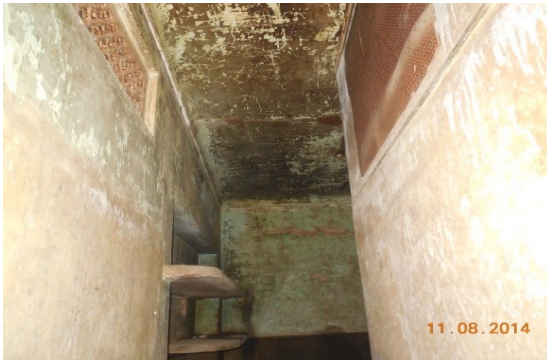
Photo 102 Seepage on All Walls & Roof of Toilet & Bath of Room No.7, Second Floor
