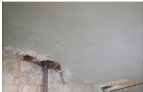
Photo 115 Plaster Crack on Roof of Varanda No. 2 of Hind Hotel, Third Floor
