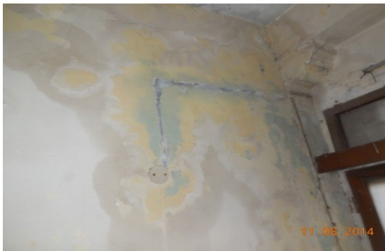
Photo 106 Seepage on Wall No. 3 & 5 of Room No. 13 of Hind Hotel, Second Floor
