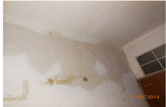
Photo 103 Seepage on Wall No. 2 & Roof of Room No. 12 of Hind Hotel, Second Floor
