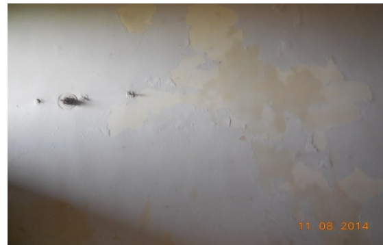
Photo 107 Peeling of Plaster on Wall No. 2 of Room No. 13 of Hind Hotel, Second Floor
