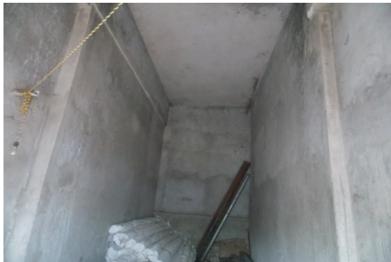
Photo 3 Repairing Work on All Walls of Shop No. E62, Ground Floor
