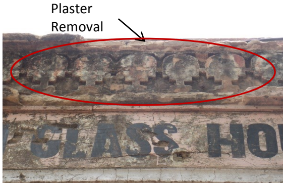
Photo 1 Plaster Removal of Outer Wall of Shop No. E62, Ground Floor
