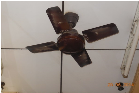
Photo 3 Covered with Wooden Ceiling, Roof of Shop No. 92A, Ground Floor
