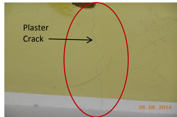
Photo 6 Plaster Crack on Wall No. 4 of Vandah of Temple, Ground Floor
