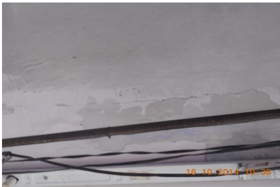
Photo 53 Horizontal Crack on Roof of Verandah of S.No.274,(G.F.) Approx. Width = 0.25mm, Approx.Length = 2.0m. Distance from L.Ext.Col. =0m, Height from Floor =2.8m.
