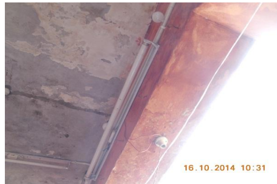
Photo 42 Dampness/Seepage on Ext. Beam & Roof of Verandah of S.No.270,G. Floor
