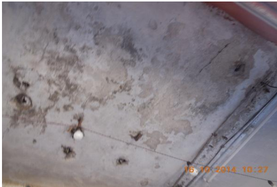
Photo 37 Dampness/Seepage on Roof of Verandah of S.No.268, Ground Floor
