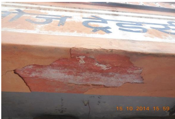
Photo 33 Peeling of Plaster on Ext. Beam of Verandah of S.No.241, Ground Floor
