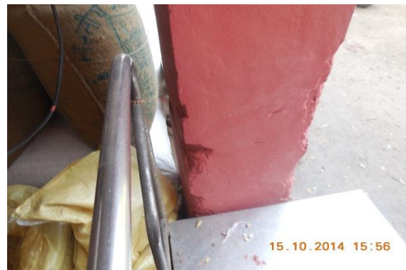
Photo 28 Plaster Removal on Right Ext. Col. of Verandah of Shop No.238
