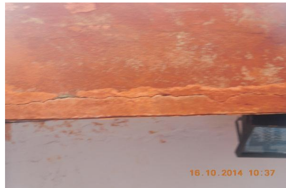
Photo 54 Horizontal Crack on Ext.Beam of Verandah of S.No.274,(G.F.) Approx. Width = 0.80mm, Approx.Length = 1.50m. Distance from R.Ext.Col. =0.40m, Height from Floor =2.0m.
