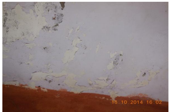
Photo 34 Peeling of Plaster on Roof of Verandah of S.No.241,Ground Floor
