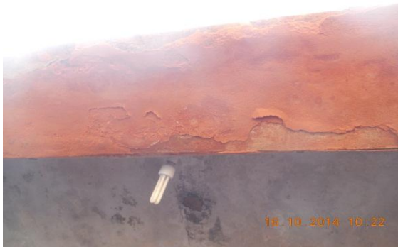
Photo 31 Dampness/Seepage on Beam Roof of Verandah of S.No.266, Ground Floor
