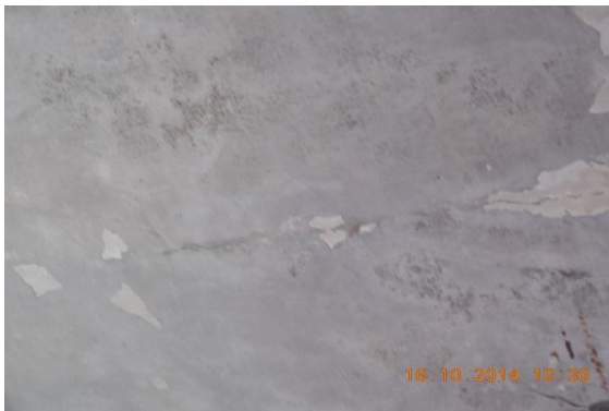
Photo 41 Horizontal Crack on Roof of Verandah of S.No.270,(G. Floor) Approx. Width = 0.15mm, Approx.Length = 2.0m. Distance from L.Ext.Col. =1.10m, Height from Floor =2.80m.
