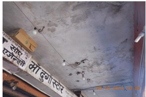
Photo 34 Dampness/Seepage on Roof of Verandah of S.No.267, Ground Floor
