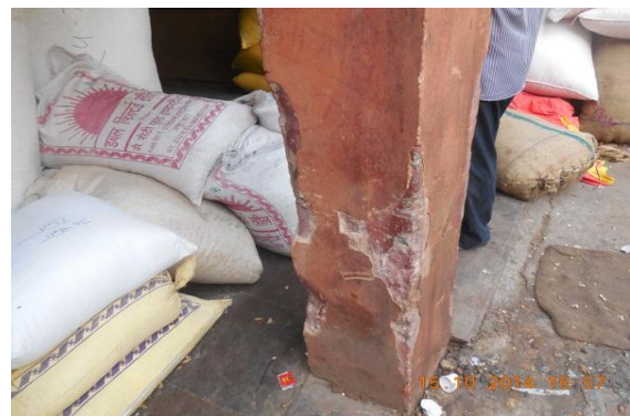
Photo 30 Plaster Removal on Right Ext. Col. of Verandah of Shop No.239
