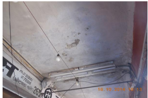
Photo 18 Dampness/Seepage on Roof of Verandah of S.No.263, Ground Floor
