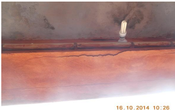
Photo 35 Peeling of Plaster on Ext. Beam Roof of Verandah of S.No.267, Ground Floor
