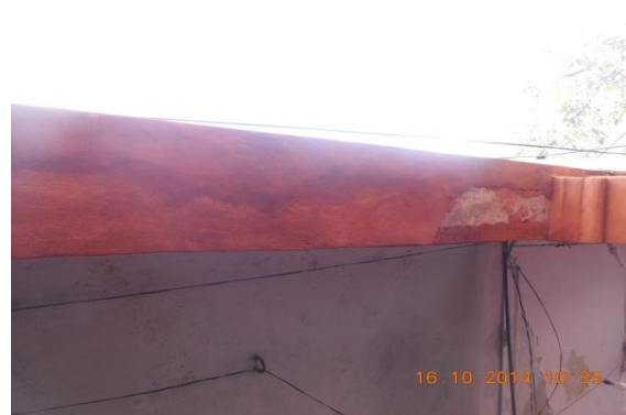
Photo 52 Dampness/Seepage on Ext.Beam of Verandah of S.No.273,, Ground Floor
