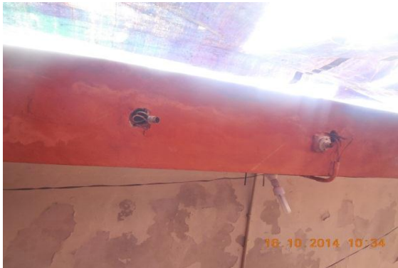
Photo 49 Dampness/Seepage on Ext. Beam of Verandah of S.No.272, Ground Floor
