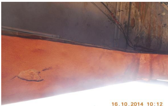
Photo 120 Dampness/Seepage on Ext.Beam & Col. of Verandah of S.No.262, Ground Floor
