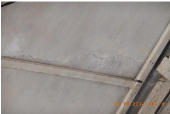
Photo 17 Horizontal Crack on Roof of Varanda of Shop No.263,(G. Floor) Approx. Width = 0.25mm, Approx.Length = 2.0m. Distance from R.Int.Col. =1.80m, Height from Floor =2.80m.
