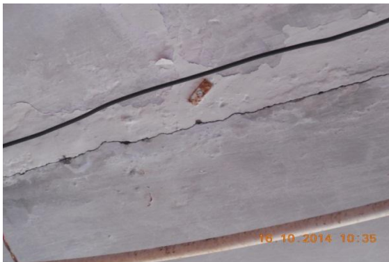
Photo 51 Horizontal Crack on Roof of Verandah of S.No.273,(G.F.) Approx. Width = 1.0mm, Approx.Length = 2.0m. Distance from L.Ext.Col. =0m, Height from Floor =2.8m.
