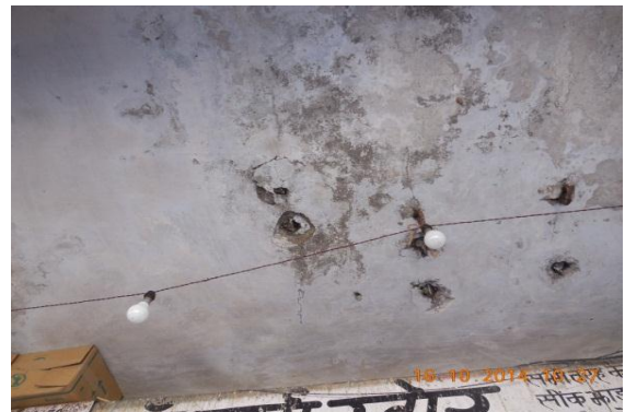
Photo 36 Plaster Removal on Roof of Verandah of S.No.268, Ground Floor
