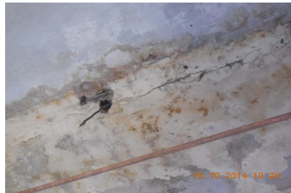
Photo 40 Horizontal Crack on Roof of Verandah of S.No.270,(G. Floor) Approx. Width = 0.25mm, Approx.Length = 2.0m. Distance from L.Ext.Col. =0m, Height from Floor =2.80m.
