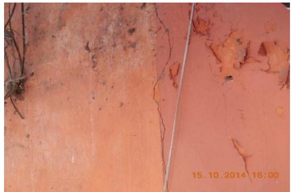
Photo 36 Inclined Crack on Wall No.4 of Varanda of Shop No.241,(G. Floor) Approx. Width = 1.0mm, Approx.Length = 1.30m. Distance from Entry Gate =1.10m, Height from Floor =1.50m.
