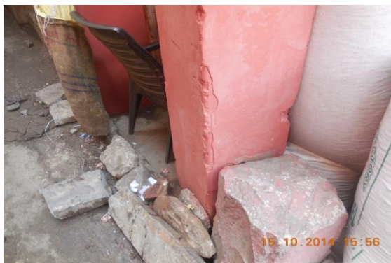
Photo 29 Plaster Removal on Left Ext. Col. of Verandah of Shop No.238
