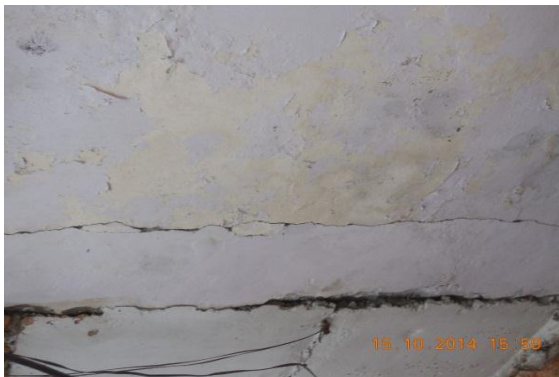
Photo 35 Horizontal Crack on Roof of Varanda of Shop No.241,(G. Floor) Approx. Width = 1.0mm, Approx.Length = 2.0m. Distance from L.Ext.Col. =0.0m, Height from Floor =2.50m.
