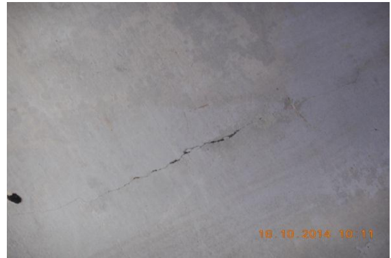
Photo 119 Plaster Crack on Roof of Verandah of S.No.262, Ground Floor
