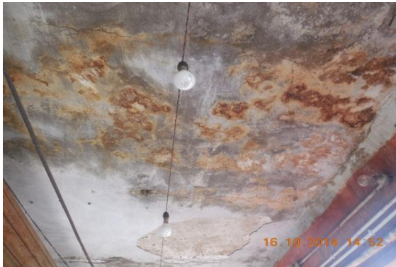
Photo 41 Dampness/Seepage on Roof of Verandah of S.No.213, Ground Floor
