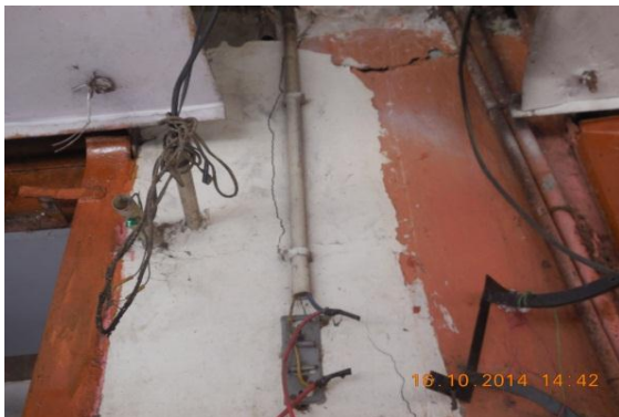
Photo 21B Inclined Crack on Roof & Right.Int.Col.of Verandah of S.No.208,GF Approx. Width = 0.80mm, Approx.Length = 0.80m. Distance from Right Ext.Col.=0.0m, Height from Floor =2.0m.
