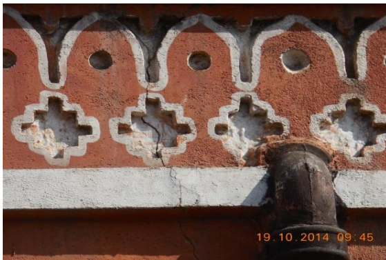
Photo 16B Inclined Crack on Outer L.Ext.Col. of Verandah of S.No.207(G.F) Approx. Width = 1.50mm, Approx.Length = 1.0m. Distance from L.Ext.Col. = 0m, Height from Floor = 2.70m.
