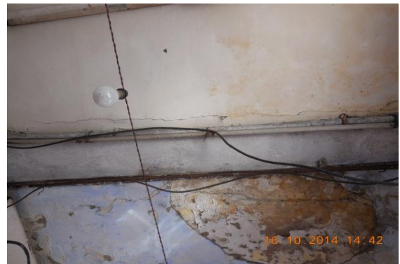
Photo 21A Inclined Crack on Roof & Right.Int.Col.of Verandah of S.No.208,GF Approx. Width = 0.80mm, Approx.Length = 0.80m. Distance from Right Ext.Col.=0.0m, Height from Floor =2.0m.
