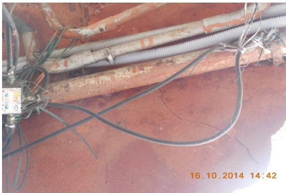
Photo 20 Inclined Crack on RHS Col.& Verandah Beam of S.No.208,(G.F.) Approx. Width = 0.80mm, Approx.Length = 0.80m. Distance from Right Ext.Col.=0.0m, Height from Floor =2.0m.
