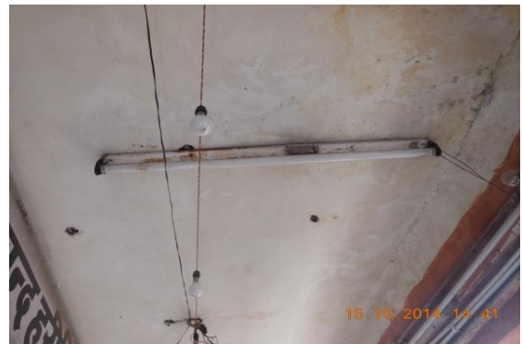
Photo 22 Dampness/Seepage on Roof of Verandah of S.No.208, Ground Floor
