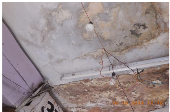
Photo 29 Horizontal Crack on Roof of Verandah of S.No.194,(G.F.), Approx. Width = 0.25mm, Approx.Length = 2.10m. Distance from R.Ext.Col. =0m, Height from Floor =2.80m.
