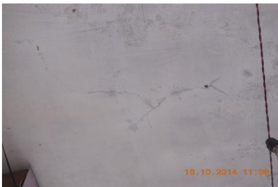
Photo 28 Plaster Crack on Roof of Verandah of S.No.193, Ground Floor
