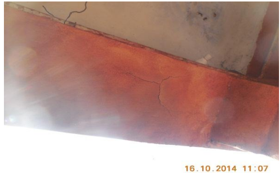
Photo 25 Dampness/Seepage on Ext.Beam of Verandah of S.No.192, Ground Floor
