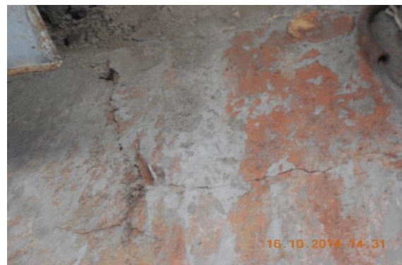
Photo 6 Inclined Crack on Left Int. Col. of Verandah of S.No.204,(G.F.) Approx. Width = 0.60mm, Approx.Length = 0.70m. Distance from L.Side Wall =0m, Height from Floor =2.20m.
