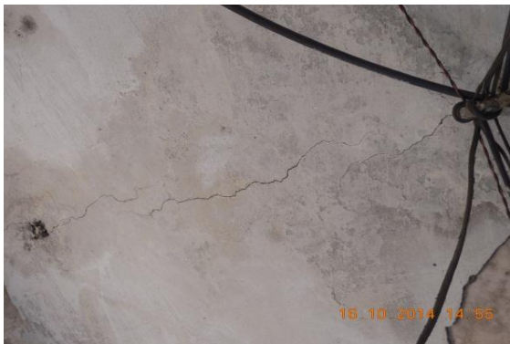
Photo 45 Horizontal Crack on Roof of Verandah of S.No.214,(G.F.), Approx. Width = 1.0mm, Approx.Length = 2.0m. Distance from Right Ext.Col. =1.30m, Height from Floor =2.80m.
