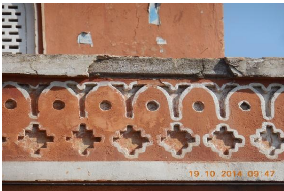
Photo 43 Plaster Removal on Outer Ext.Beam of Verandah of S.No.213, Ground Floor
