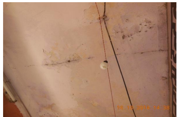
Photo 12 Horizontal Crack on Roof of Verandah of S.No.206,(G. Floor) Approx. Width = 0.35mm, Approx.Length = 2.0m. Distance from Right Ext. Col. =1.80m, Height from Floor =2.80m.
