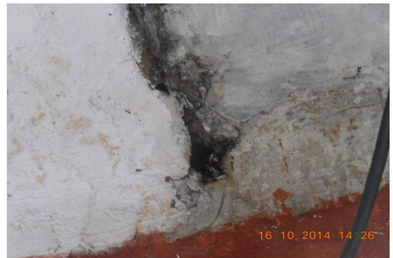
Photo 6 Plaster Removal on Roof of Verandah of S.No.201, Ground Floor
