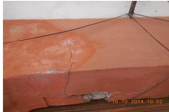
Photo 8 Horizontal Crack on Int. Beam of Verandah of S.No.189,(G. Floor) Approx. Width = 2.0mm, Approx.Length = 1.4m. Distance from L.Int.Col. =0.50m, Height from Floor =2.10m.
