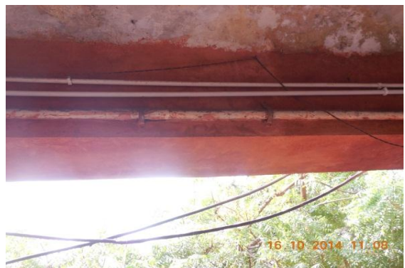
Photo 27 Dampness/Seepage on Ext. Beam of Verandah of S.No.193, Ground Floor
