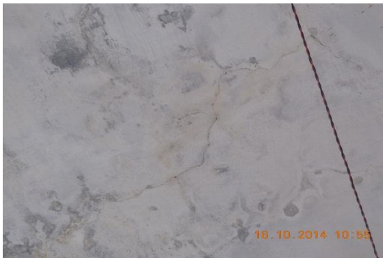
Photo 9 Horizontal Crack on Roof of Verandah of S.No.189,(G. Floor) Approx. Width = 0.15mm, Approx.Length = 1.5m. Distance from Wall No.3 =0m, Height from Floor =2.50m.
