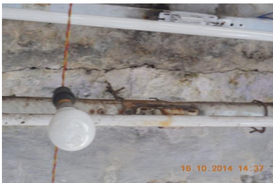
Photo 11 Horizontal Crack on Roof of Verandah of S.No.206,(G. Floor) Approx. Width = 0.60mm, Approx.Length = 2.0m. Distance from Left Ext. Col. =0m, Height from Floor =2.80m.
