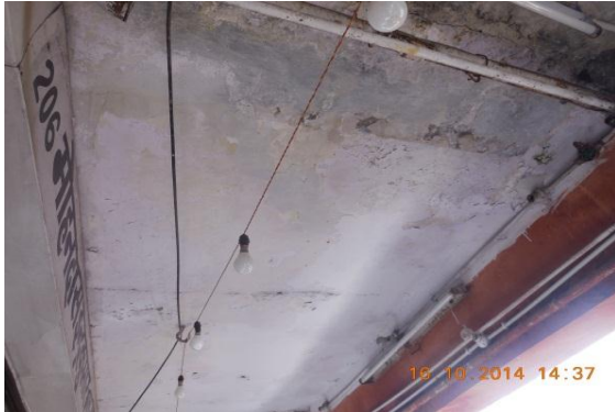
Photo 13 Dampness/Seepage on Ext.Beam of Verandah of S.No.206, Ground Floor
