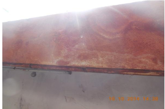
Photo 14 Dampness/Seepage on Roof of Verandah of S.No.206, Ground Floor
