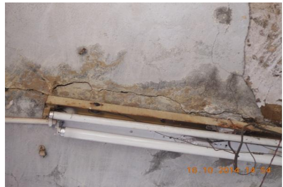
Photo 44 Horizontal Crack on Roof of Verandah of S.No.214,(G.F.), Approx. Width = 2.0mm, Approx.Length = 2.0m. Distance from Left Ext.Col. =0m, Height from Floor =2.80m.
