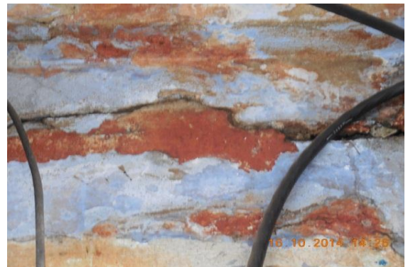
Photo 4 Inclined Crack on L.Int.Col. of Verandah of S.No.201, (G. Floor) Approx. Width = 0.50mm, Approx.Length = 0.80m. Distance from L.Int.Col. = 0m, Height from Floor = 2.50m.
