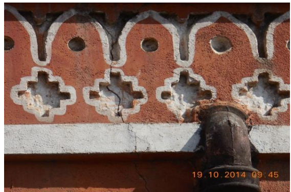
Photo 16A Inclined Crack on Outer L.Ext.Col. of Verandah of S.No.207(G.F) Approx. Width = 1.50mm, Approx.Length = 1.0m. Distance from L.Ext.Col. = 0m, Height from Floor = 2.70m.
