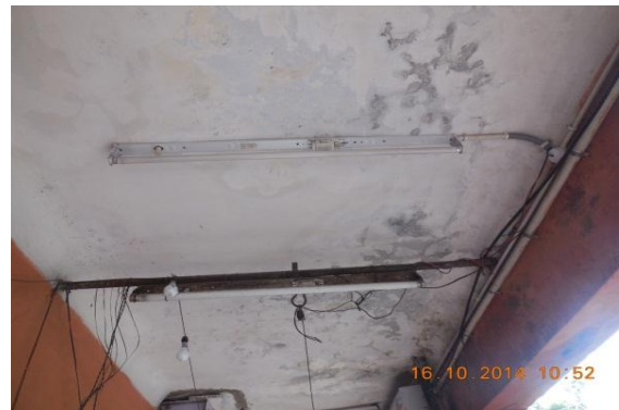
Photo 10 Dampness/Seepage on Roof of Verandah of S.No.189, Ground Floor
