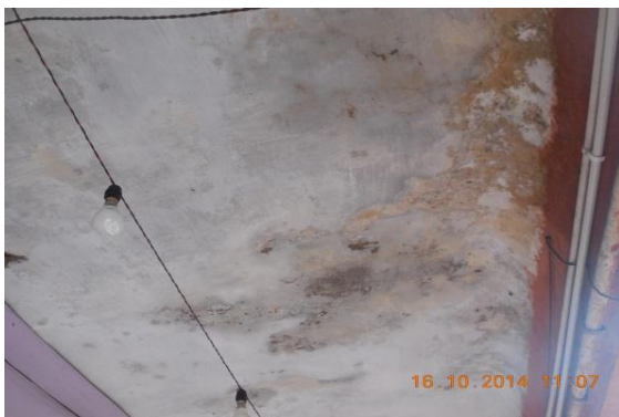
Photo 26 Dampness/Seepage on Roof of Verandah of S.No.193, Ground Floor
