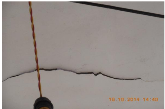
Photo 17 Peeling of Plaster on Roof of Verandah of S.No.207, Ground Floor
