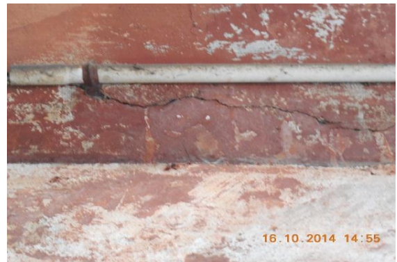
Photo 46 Horizontal Crack on Roof of Verandah of S.No.214,(G.F.), Approx. Width = 1.0mm, Approx.Length = 2.0m. Distance from Right Ext.Col. =0m, Height from Floor =2.80m.
