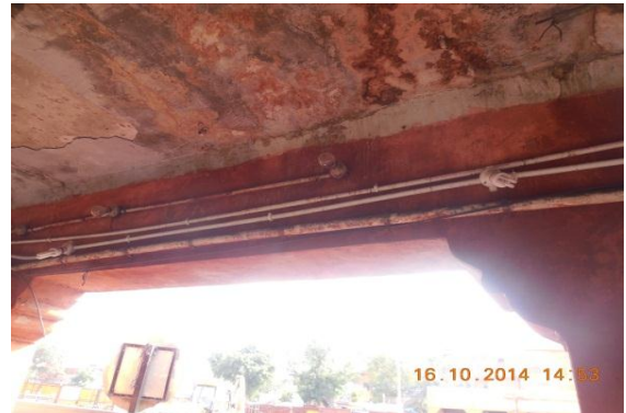
Photo 42 Dampness/Seepage on Ext.Beam of Verandah of S.No.213, Ground Floor
