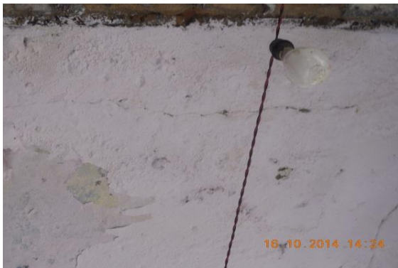
Photo 3 Horizontal Crack on Roof of Verandah of S.No.201, (G. Floor) Approx. Width = 0.15mm, Approx.Length = 2.0m. Distance from L.Ext.Col. = 0m, Height from Floor = 2.80m.
