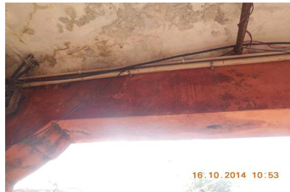
Photo 12 Dampness/Seepage on Ext. Beam of Verandah of S.No.189, Ground Floor
