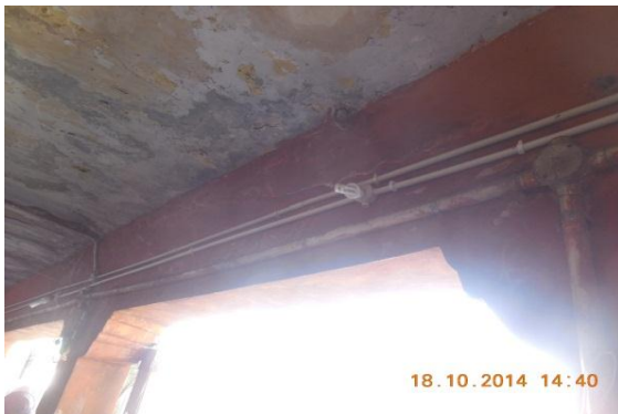
Photo 11 Dampness/Seepage on Ext.Beam of Verandah of S.No.364A & 364B, Ground Floor
