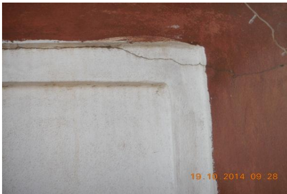
Photo 3A Horizontal Crack on Outer Ext.Beam of Verandah of S.No.353,GF Approx. Width = 0.50mm, Approx.Length = 3.0m. Distance from Left Ext.Col. = 0m, Height from Floor = 2.50m.
