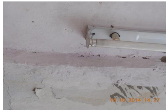
Photo 4 Horizontal Crack on Roof of Verandah of S.No.354, (G. Floor) Approx. Width = 0.80mm, Approx.Length = 2.50m. Distance from Right Ext.Col. = 0m, Height from Floor = 2.80m.
