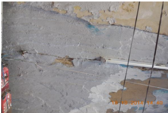
Photo 9 Horizontal Crack on Roof of Verandah of S.No.364A & 364B, GF Approx. Width = 2.0mm, Approx.Length = 2.50m. Distance from L.Ext.Col. = 0m, Height from Floor = 2.80m.
