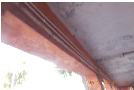
Photo 11 Dampness/Seepage on Ext.Beam of Verandah of S.No.357, Ground Floor
