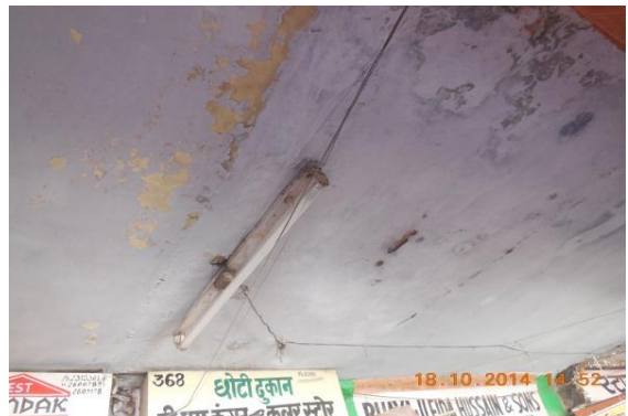
Photo 24 Dampness/ Seepage on Roof of Verandah of S.No.368, Ground Floor
