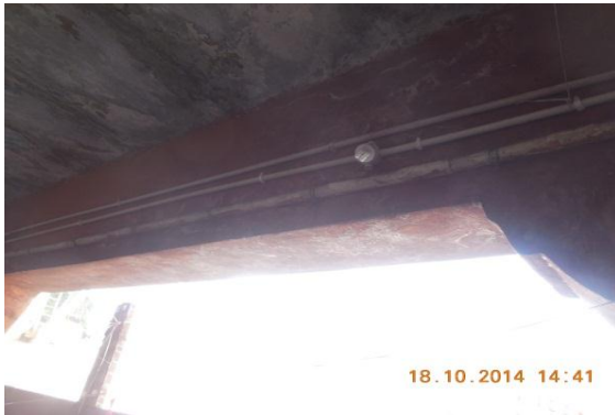
Photo 13 Dampness/Seepage on Ext.Beam of Verandah of S.No.365, Ground Floor
