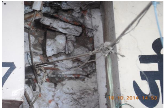
Photo 26 Plaster Removal on Left Int.Col. of Verandah of S.No.368, Ground Floor
