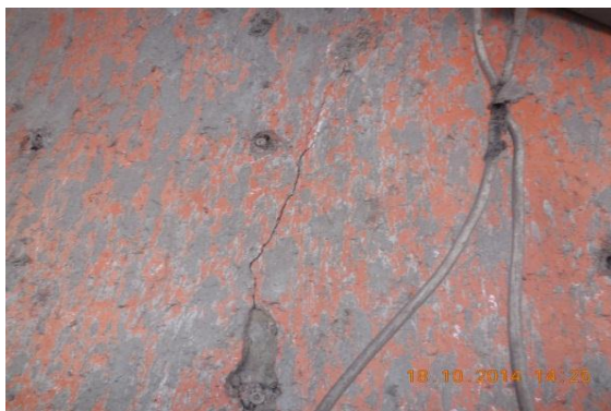
Photo 3A Inclined Crack on Right Int. Col. of Verandah of S.No.352,GF Approx. Width = 1.0mm, Approx.Length = 1.0m. Distance from Right Int.Col. =0m, Height from Floor =1.60m.
