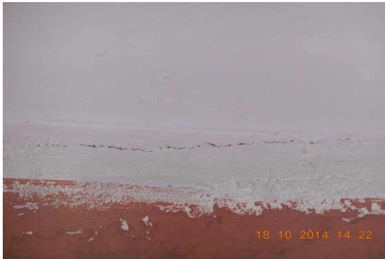
Photo 7 Plaster Crack on Ext.Beam of Verandah of S.No.350, Ground Floor
