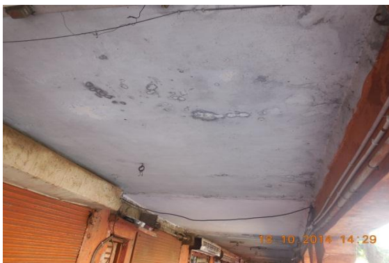
Photo 9 Dampness/Seepage on Roof of Verandah of S.No.357, Ground Floor
