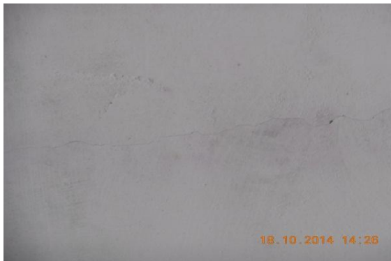
Photo 5 Plaster Crack on Roof of Verandah of S.No.354, Ground Floor
