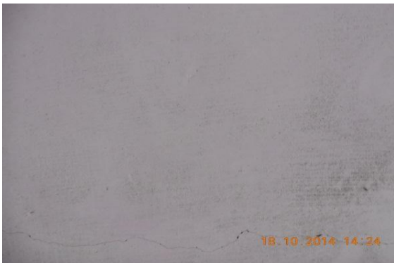
Photo 4 Plaster Crack on Roof of Verandah of S.No.353, Ground Floor
