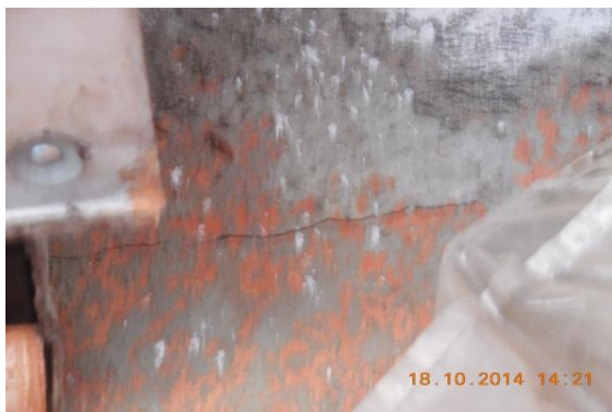
Photo 5 Plaster Crack on Right Int.Col. of Verandah of S.No.350, Ground Floor
