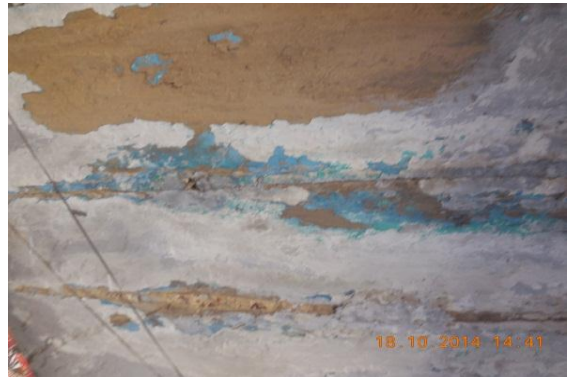
Photo 14 Stone Gap on Roof of Verandah of S.No.365, Ground Floor
