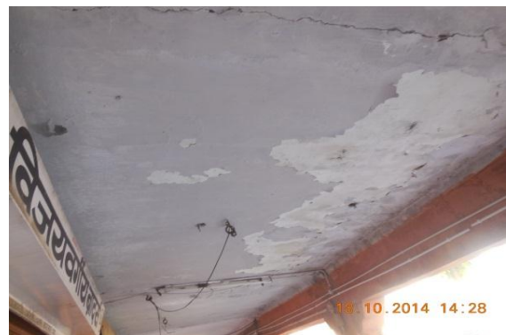
Photo 6 Dampness/Seepage on Roof of Verandah of S.No.356, Ground Floor
