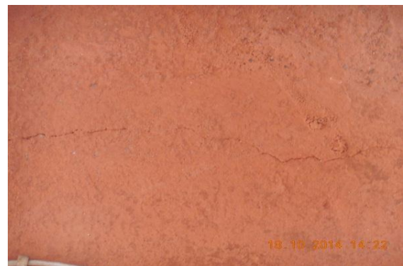
Photo 6 Plaster Crack on Left Ext.Beam of Verandah of S.No.350, Ground Floor
