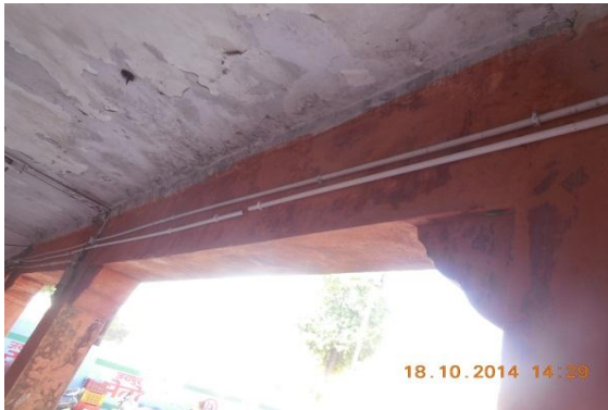
Photo 7 Dampness/Seepage on Ext.Beam of Verandah of S.No.356, Ground Floor
