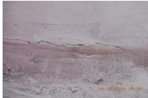
Photo 8 Horizontal Crack on Roof of Verandah of S.No.357, (G. Floor) Approx. Width = 1.0mm, Approx.Length = 2.50m. Distance from Right Ext.Col. = 0m, Height from Floor = 2.80m.
