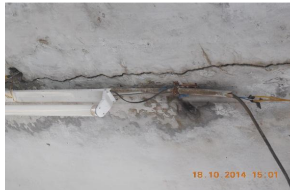
Photo 12 Horizontal Crack on Roof of Verandah of S.No.372,GF Approx. Width =15.0mm, Approx.Length = 2.50m. Distance from R.Ext.Col. = 0m, Height from Floor =2.80m.
