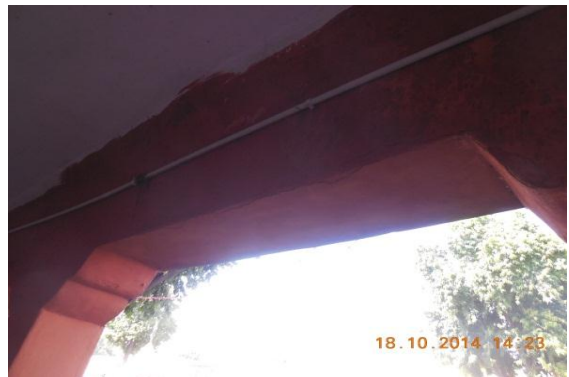
Photo 10 Peeling of Plaster on Ext.Beam of Verandah of S.No.351, Ground Floor
