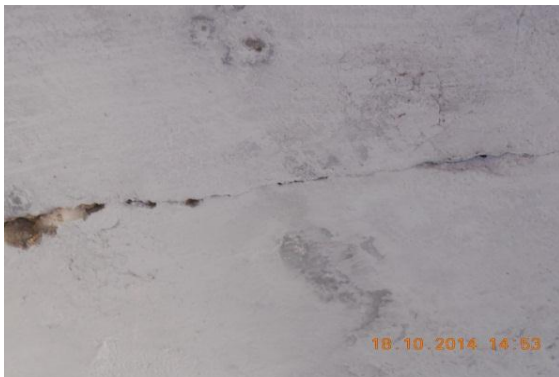
Photo 23 Horizontal Crack on Roof of Verandah of S.No.368,GF Approx. Width =0.50mm, Approx.Length = 2.50m. Distance from R.Ext.Col. = 0m, Height from Floor =2.80m.
