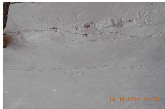
Photo 10 Plaster Crack on Roof of Verandah of S.No.357, Ground Floor
