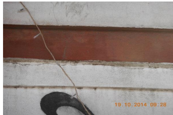
Photo 3B Horizontal Crack on Outer Ext.Beam of Verandah of S.No.353,GF Approx. Width = 0.50mm, Approx.Length = 3.0m. Distance from Left Ext.Col. = 0m, Height from Floor = 2.50m.
