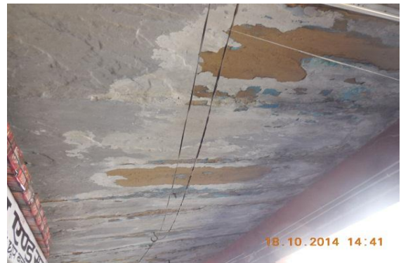
Photo 12 Dampness/Seepage on Roof of Verandah of S.No.365, Ground Floor
