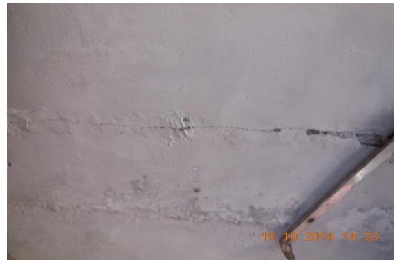
Photo 4 Horizontal Crack on Roof of Verandah of S.No.359, (G. Floor) Approx. Width = 2.0mm, Approx.Length = 2.50m. Distance from Right Ext.Col. = 0m, Height from Floor = 2.80m.
