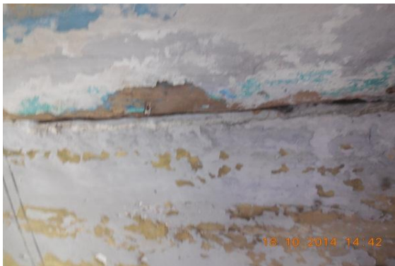
Photo 15 Joint Open on Roof of Verandah of S.No.365, Ground Floor
