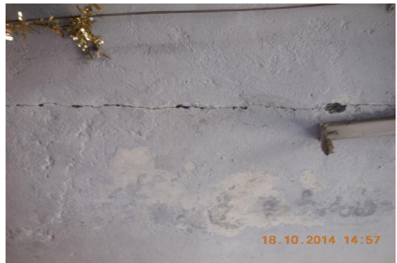
Photo 30 Horizontal Crack on Roof of Verandah of S.No.370&370A,GF Approx. Width = 3.0mm, Approx.Length = 2.50m. Distance from L.Ext.Col. = 0m, Height from Floor = 2.80m.
