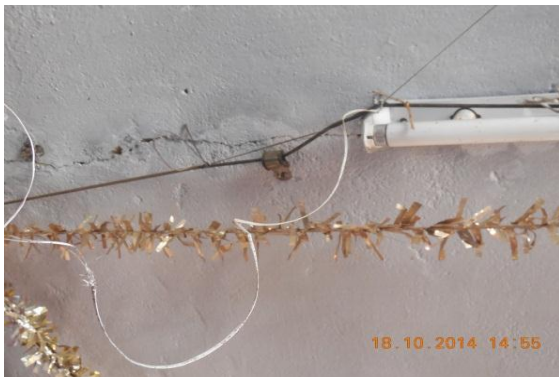
Photo 27 Horizontal Crack on Roof of Verandah of S.No.369,GF Approx. Width = 0.80mm, Approx.Length = 2.50m. Distance from R.Ext.Col. = 0m, Height from Floor = 2.80m.
