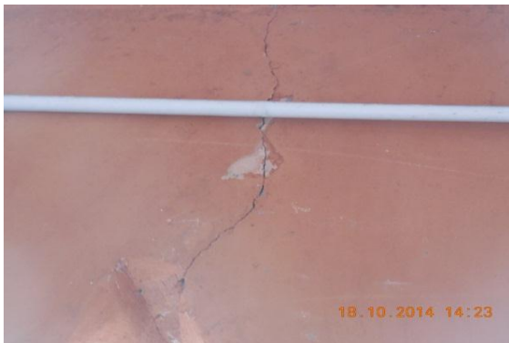
Photo 9 Inclined Crack on Left Ext.Col. of Verandah of S.No.351,GF Approx. Width = 0.80mm, Approx.Length = 0.80m. Distance from Right Ext.Col. = 0m, Height from Floor = 2.50m.
