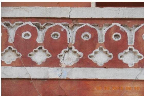
Photo 5 Inclined Crack on Outer Left Ext.Col. of Verandah of S.No.356, G.F. Approx. Width = 1.50mm, Approx.Length = 0.60m. Distance from Left Ext.Col. = 0m, Height from Floor = 2.30m.
