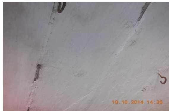
Photo 6 Joint Gap on Roof of Verandah of S.No.362, Ground Floor
