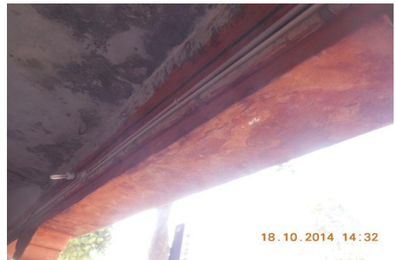
Photo 6 Dampness/Seepage on Ext.Beam of Verandah of S.No.359, Ground Floor
