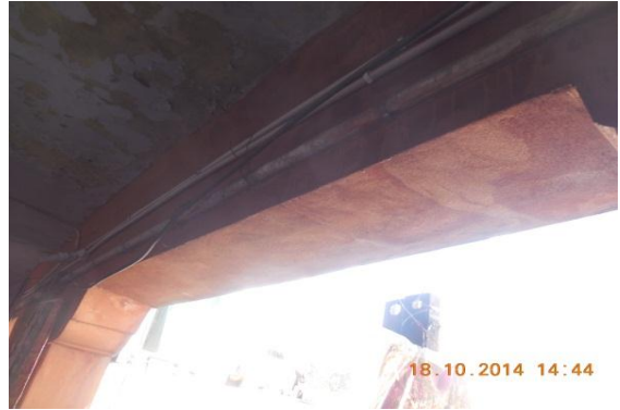
Photo 20 Dampness/Seepage on Ext.Beam of Verandah of S.No.366, Ground Floor
