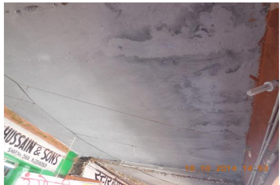
Photo 28 Dampness/Seepage on Roof of Verandah of S.No.369, Ground Floor
