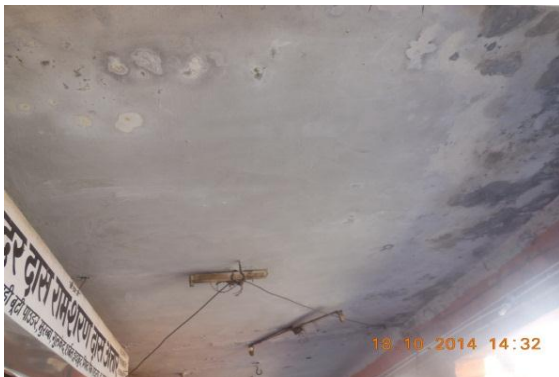
Photo 5 Dampness/Seepage on Roof of Verandah of S.No.359, Ground Floor
