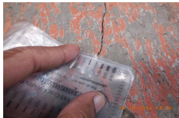
Photo 3B Inclined Crack on Right Int. Col. of Verandah of S.No.352,GF Approx. Width = 1.0mm, Approx.Length = 1.0m. Distance from Right Int.Col. =0m, Height from Floor =1.60m.
