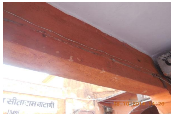
Photo 4 Dampness/Seepage on Left Ext.Beam of Verandah of S.No.350, Ground Floor
