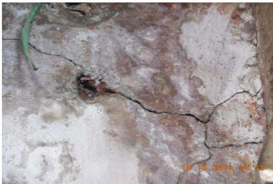
Photo 17 Plaster Crack on Int.Right Col.of Verandah of S.No.365, Ground Floor
