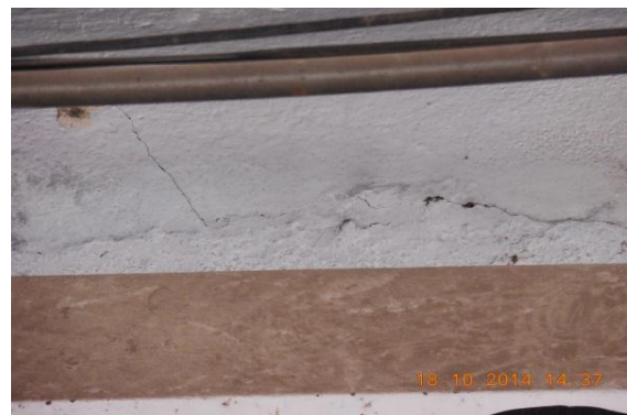
Photo 4 Horizontal Crack on Int.Beam of Verandah of S.No.362,(G. Floor) Approx. Width = 1.50mm, Approx.Length = 2.0m. Distance from Right Int.Beam =0m, Height from Floor =2.70m.
