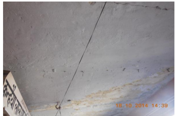
Photo 10 Dampness/Seepage on Roof of Verandah of S.No.364A & 364B, Ground Floor
