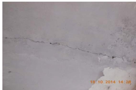
Photo 4 Horizontal Crack on Roof of Verandah of S.No.356, (G. Floor) Approx. Width = 1.50mm, Approx.Length = 2.50m. Distance from Left Ext.Col. = 0m, Height from Floor = 2.80m.
