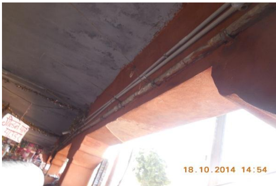
Photo 29 Dampness/Seepage on Ext.Beam of Verandah of S.No.369, Ground Floor
