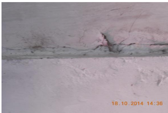
Photo 3 Horizontal Crack on Roof of Verandah of S.No.362,(G. Floor) Approx. Width = 0.60mm, Approx.Length = 2.50m. Distance from Left Ext.Col. =0m, Height from Floor =2.80m.
