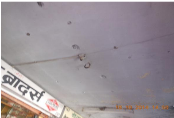
Photo 21 Dampness/Seepage on Roof of Verandah of S.No.367, Ground Floor
