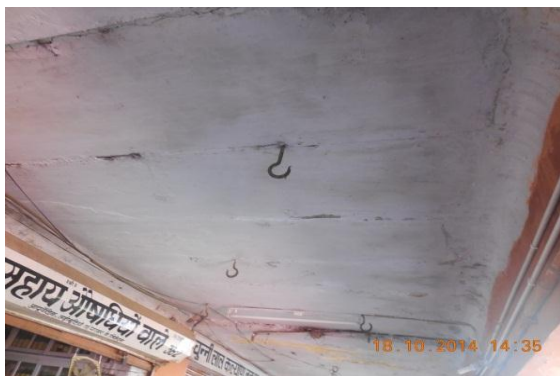
Photo 5 Dampness/Seepage on Roof of Verandah of S.No.362, Ground Floor
