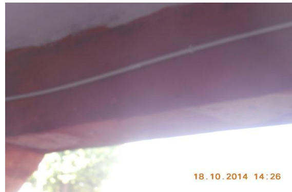
Photo 6 Dampness/Seepage on Ext.Beam of Verandah of S.No.354, Ground Floor
