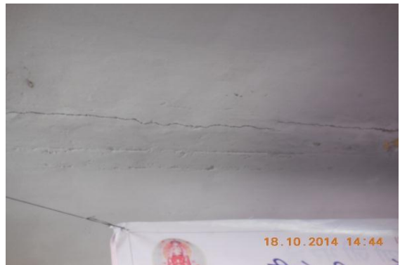
Photo 18 Horizontal Crack on Roof of Verandah of S.No.366,GF Approx. Width =2.50mm, Approx.Length = 2.50m. Distance from R.Ext.Col. = 0m, Height from Floor =2.80m.
