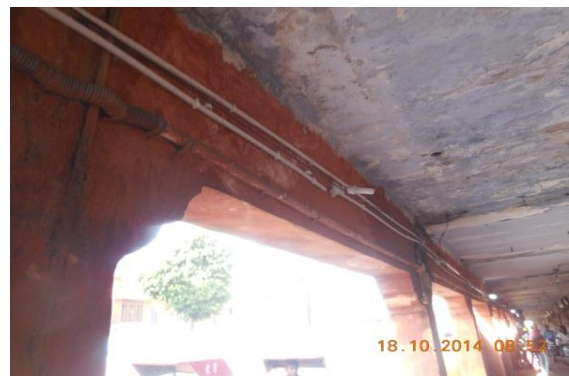
Photo 134 Dampness/Seepage on Ext.Beam of Verandah of S.No.26, Ground Floor
