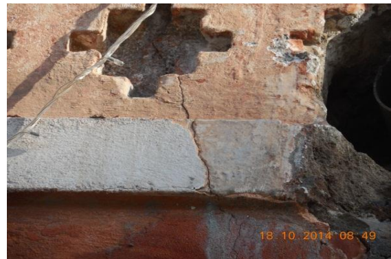
Photo 126 Inclined Crack on Outer L.Ext.Col. of Verandah of S.No.25, G.F. Approx. Width = 0.60mm, Approx.Length = 0.80m. Distance from L.Ext. Col. = 0m, Height from Floor = 3.10m.
