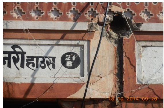
Photo 115 Plaster Removal on Outer Left Ext.Col. of Verandah of S.No.21B, Ground Floor
