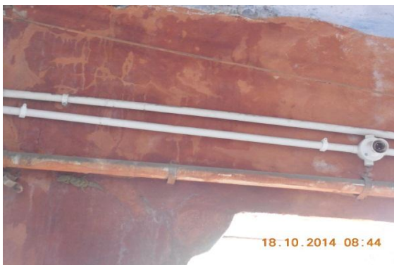
Photo 114 Dampness/Seepage on Ext.Beam & L.Ext.Col.of Verandah of S.No.21B, Ground Floor
