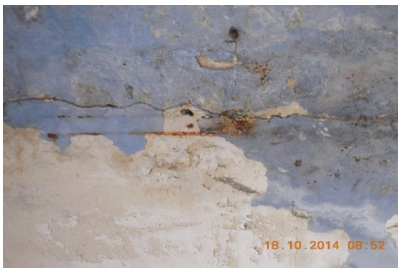
Photo 131 Horizontal Crack on Roof of Verandah of S.No.26, G.F. Approx. Width = 1.0mm, Approx.Length = 2.90m. Distance from L.Ext. Col. = 0m, Height from Floor = 2.80m.
