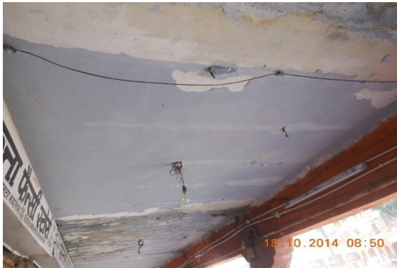
Photo 129 Dampness/Seepage on Roof of Verandah of S.No.25, Ground Floor
