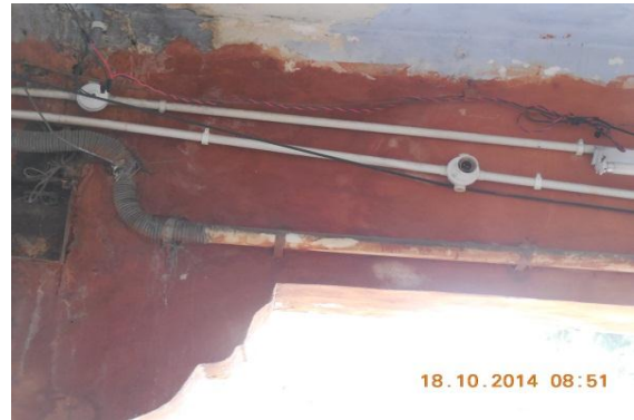
Photo 130 Dampness/Seepage on Ext.Beam of Verandah of S.No.25, Ground Floor
