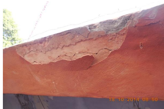
Photo 128 Plaster Removal on Ext. Beam of Verandah of S.No.25, Ground Floor
