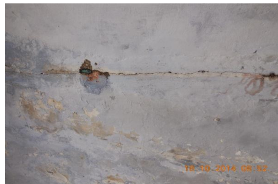
Photo 132 Horizontal Crack on Roof of Verandah of S.No.26, G.F. Approx. Width = 1.50mm, Approx.Length = 2.90m. Distance from R.Ext. Col. = 0m, Height from Floor = 2.80m.
