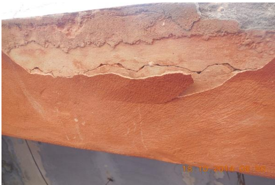
Photo 127 Horizontal Crack on Ext. Beam of Verandah of S.No.25, G.F. Approx. Width = 1.0mm, Approx.Length = 0.60m. Distance from L.Ext. Col. = 1.40m, Height from Floor = 2.30m.
