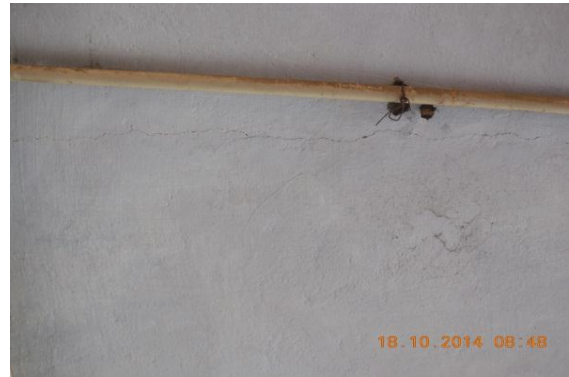
Photo 124 Plaster Crack on Roof of Verandah of S.No.24, Ground Floor
