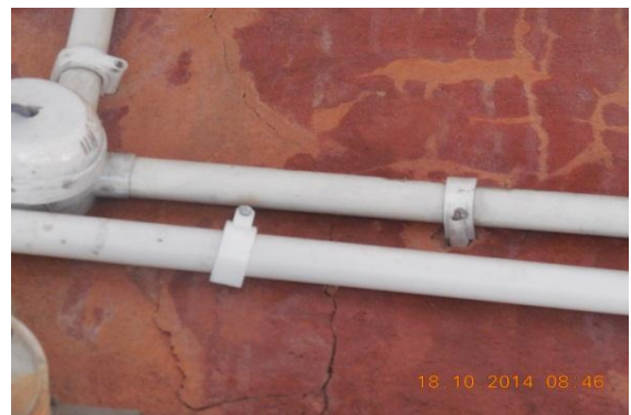
Photo 116B Horizontal Crack on Roof & L.Ext.Col.of Verandah of S.No.22,G.F. Approx. Width = 1.0mm, Approx.Length = 3.50m. Distance from L.Ext. Col. =0m, Height from Floor =2.80m.
