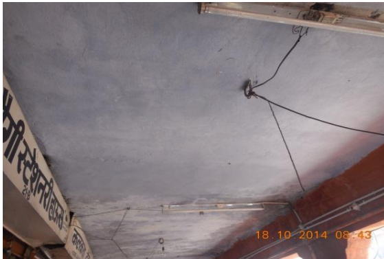
Photo 112 Dampness/Seepage on Roof of Verandah of S.No.21B, Ground Floor
