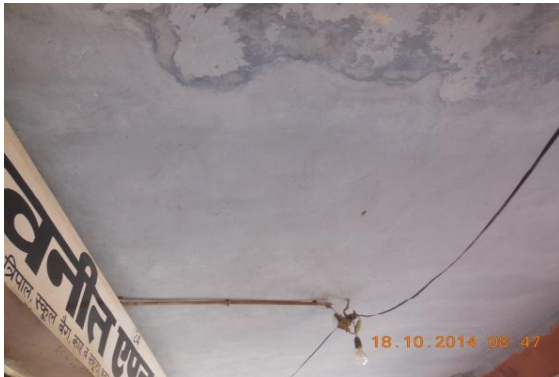
Photo 123 Dampness/Seepage on Roof of Verandah of S.No.24, Ground Floor
