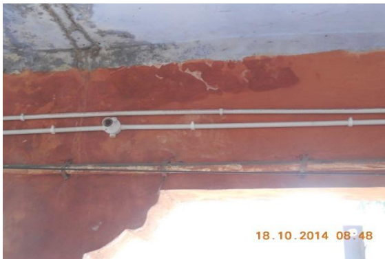
Photo 125 Dampness/Seepage on Ext. Beam of Verandah of S.No.24, Ground Floor
