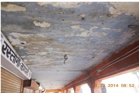
Photo 133 Dampness/Seepage on Roof of Verandah of S.No.26, Ground Floor
