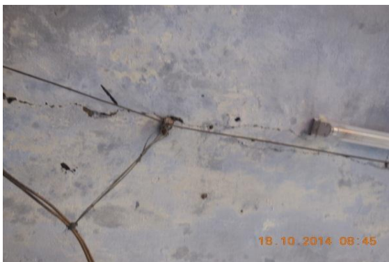
Photo 116A Horizontal Crack on Roof & L.Ext.Col.of Verandah of S.No.22,G.F. Approx. Width = 1.0mm, Approx.Length = 3.50m. Distance from L.Ext. Col. =0m, Height from Floor =2.80m.
