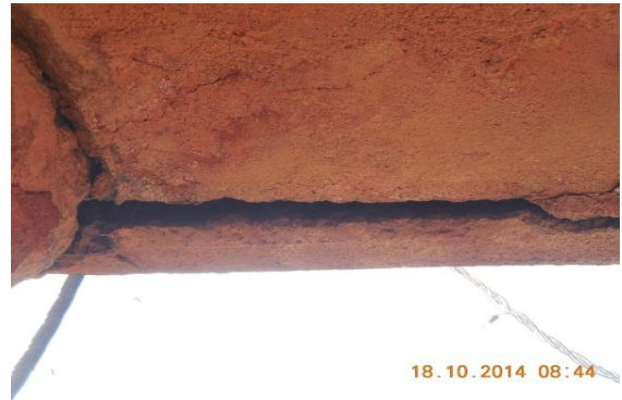
Photo 113 Plaster Removal on Ext.Beam of Verandah of S.No.21B, Ground Floor
