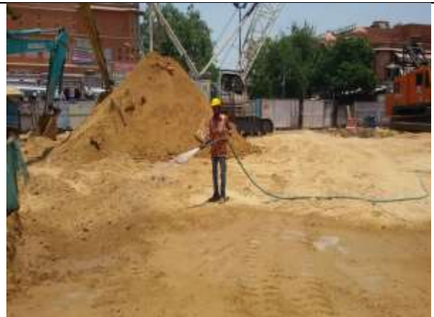
Water sprinkling for dust suppression at site
