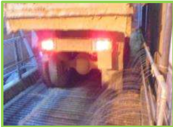
Cleaning the tyre of Loaded dumper before entering the public road.
