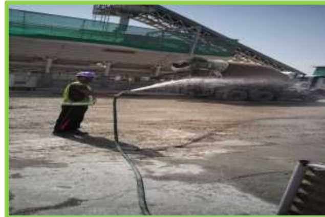
Water sprinkling for dust suppression at site
