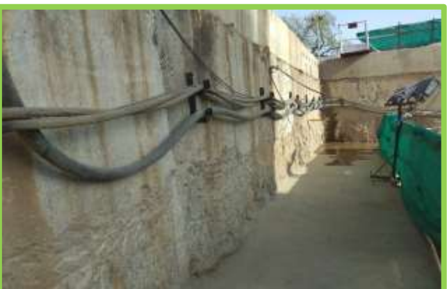
Proper Electrical cables route arrangement
