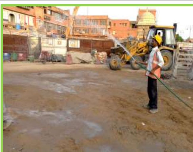
Water sprinkling for dust suppression at site
