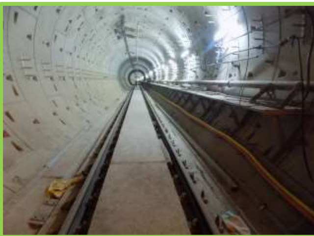
View of Track, Traction line and Utilities in the Down line track towards Badichouper
