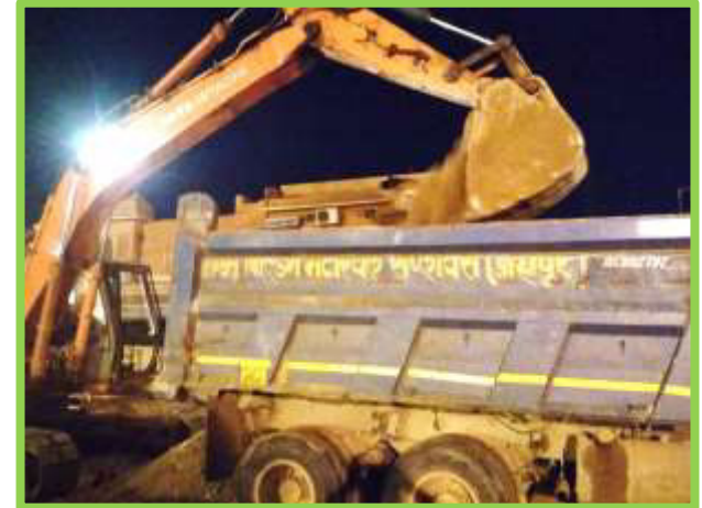
Muck loading into dumper by excavator
