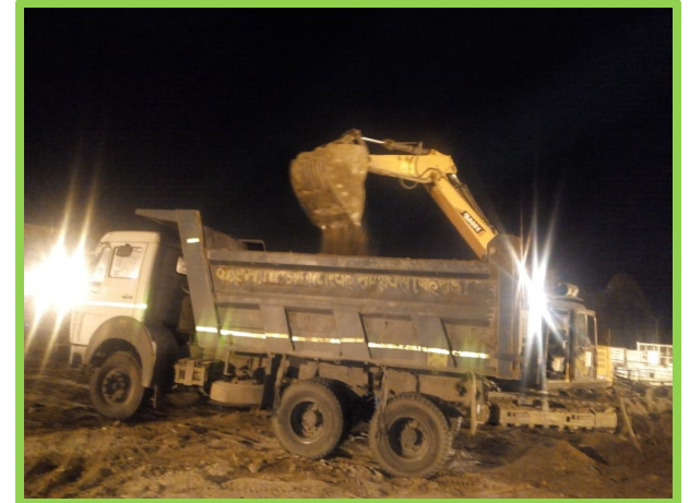
Muck loading into dumper by excavator
