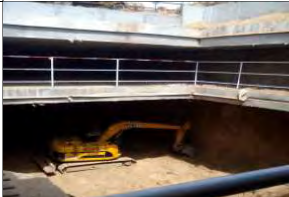
Soil Excavation for Top slab at Chhoti Chaupar
