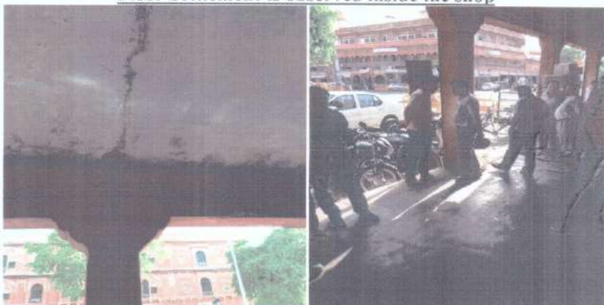
Crack is observed on verandah Slab, Floor settlement is observed at verandah
