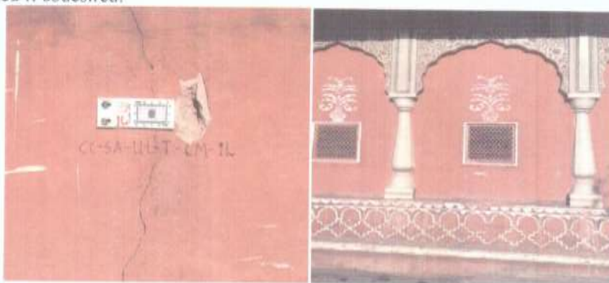
Damaged Crack Meters
