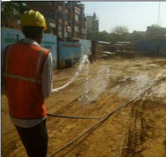
Manually Water sprinkling for Dust control on site access.
