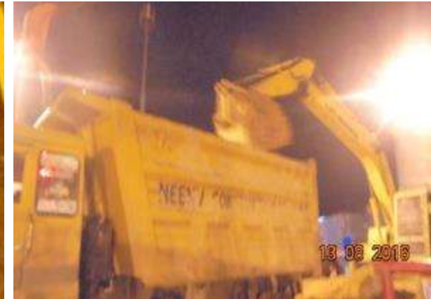
Muck loaded into dumper by L&T Komatsu long boom excavator from muck pit
