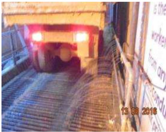
Cleaning the tyre of Loaded dumper before entering the public road.
