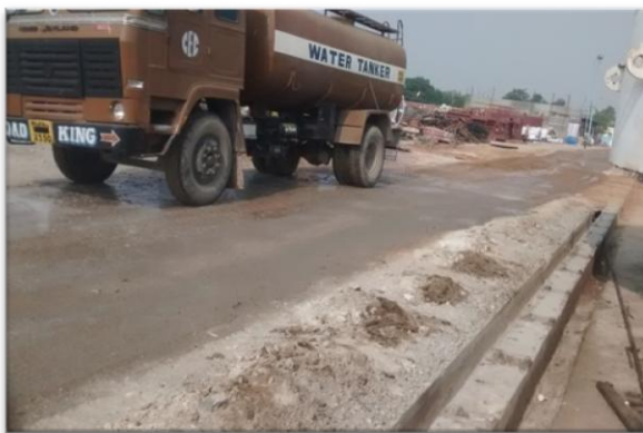
Water Sprinkling through Tank
