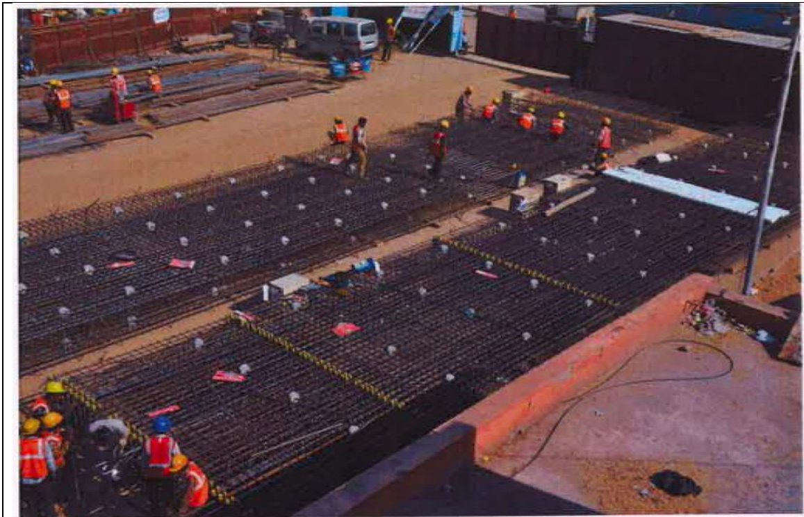
D-Wall Cage Febrication at Chhoti Chaupar
