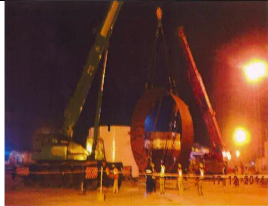
Tilting of TBM-1 Tail Shield
