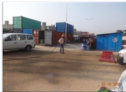
Manual Water Sprinkling at site
