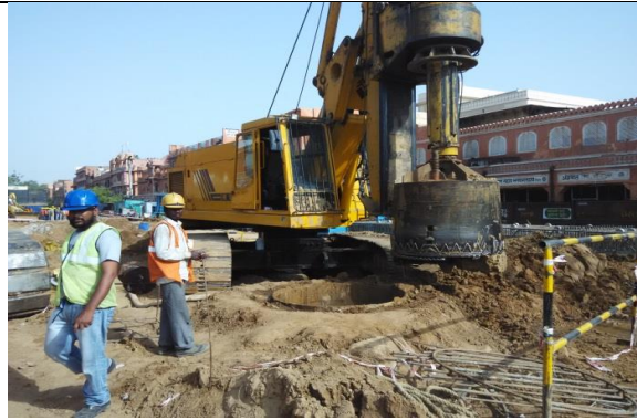
French Collum Excavation at Chhoti Chaupar
