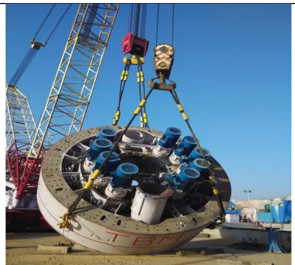
Tilting of TBM-2 at Chandpole Launching Shaft
