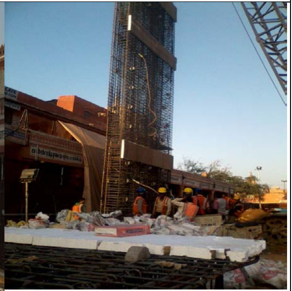
Roof Slab Febrication at Chhoti Chaupar
