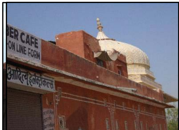
Damaged Parapet Wall, Cracks on below wall
