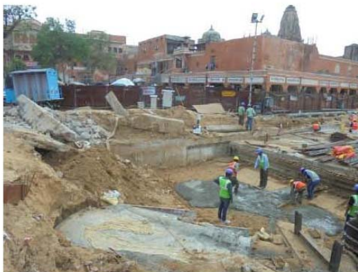
Right: Picture showing the construction of the D- Wall at Choti Chaupar
