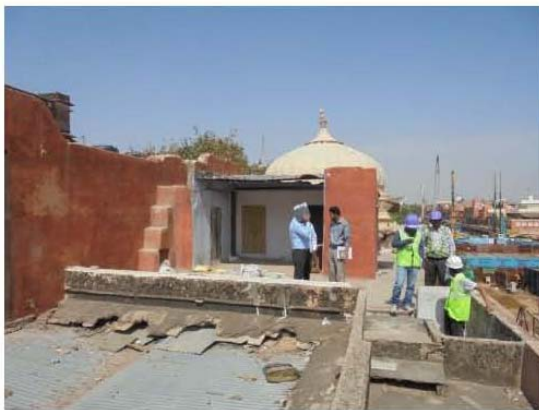
Photographs of damaged parapet wall above shops 374 - 376 next to Naval Kishor Temple
