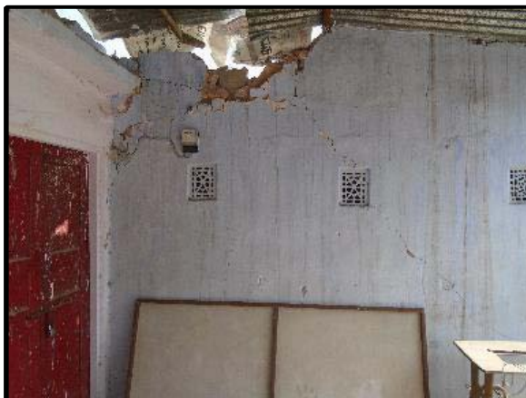
Damaged Parapet Wall, Cracks on below wall
