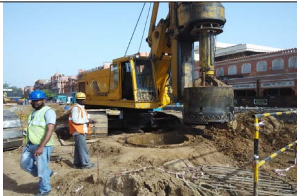
French Collum Excavation at Chhoti Chaupar
