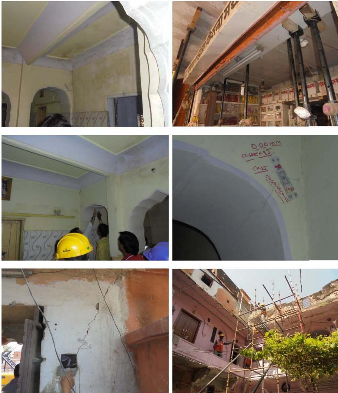
Photographs of monitoring of cracks; development of new cracks on the inner portion of the Naval Kishor Temple due to settlement or impact of crane boom over the masonry; repairs to the upper parapet been executed; propping of
