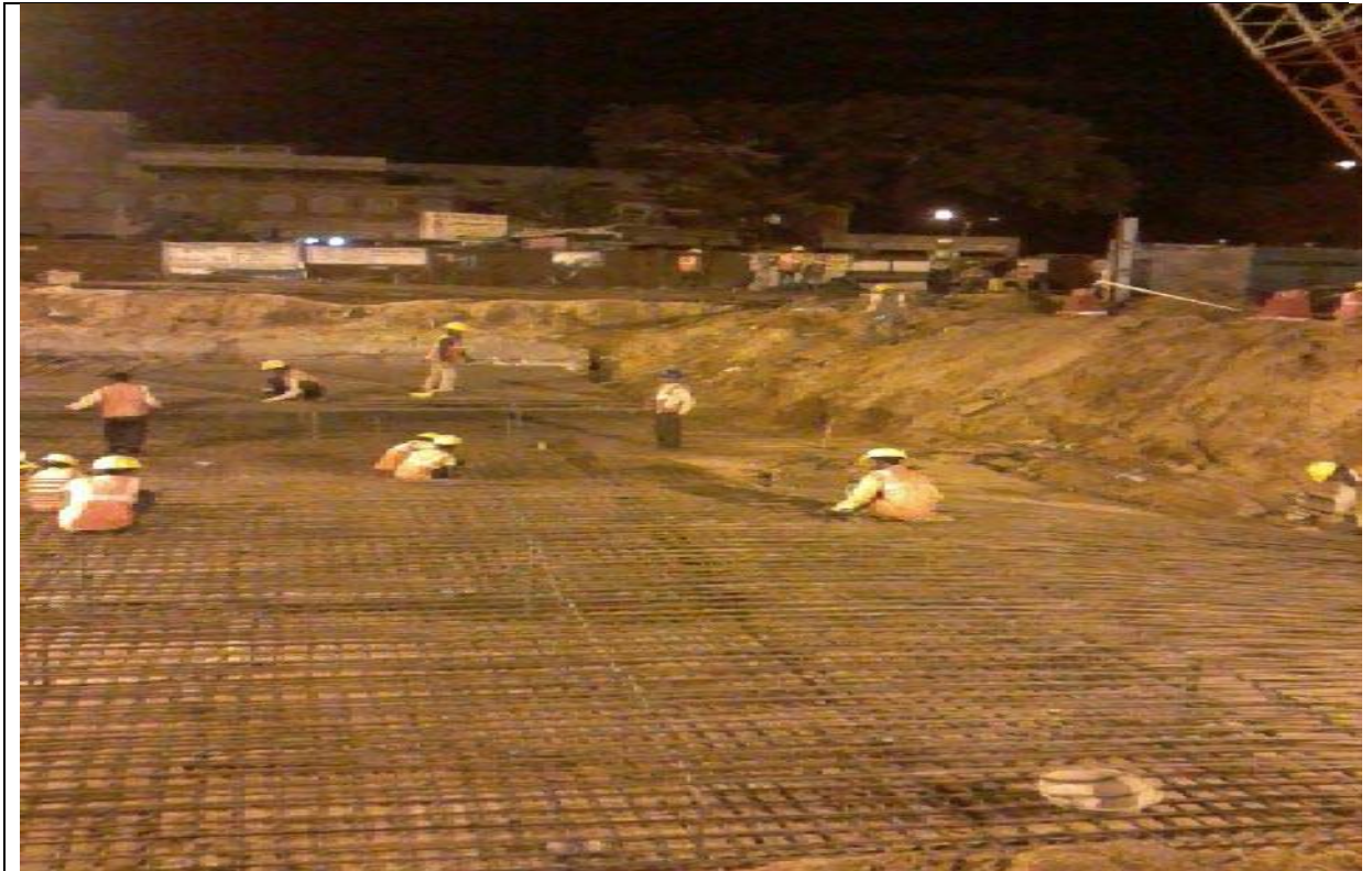
Roof Slab Febrication at Chhoti Chaupar
