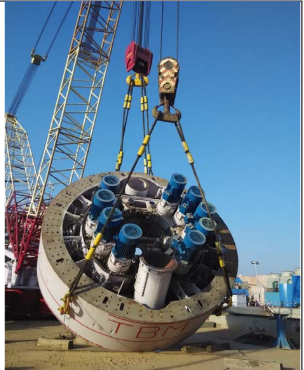
Tilting of TBM-2 at Chandpole Launching Shalft
