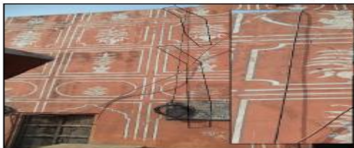
Vertical/ inclined crack is observed on wall.
