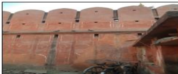
Wall Plaster damaged. Cavities are formed at wall-ground
