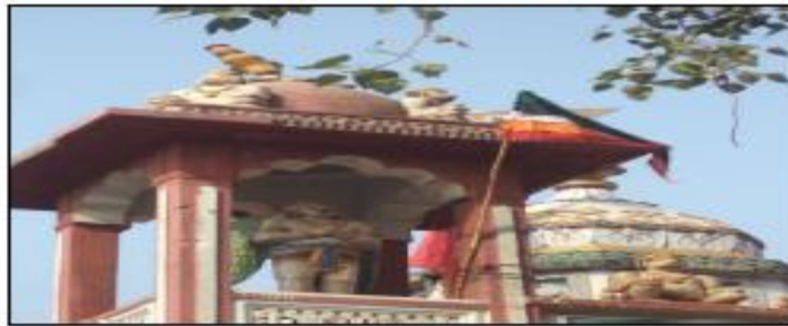
Minaret is damaged and dislocated (Hanumanji Ka Mandir)
