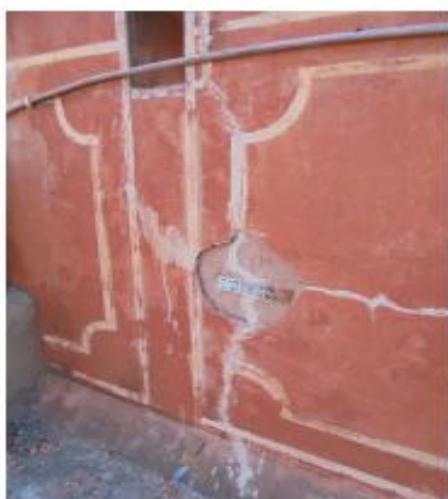
Older plaster cracks on the terrace walls already being monitored. Some of which have marginally expanded but all within permissible limit.
