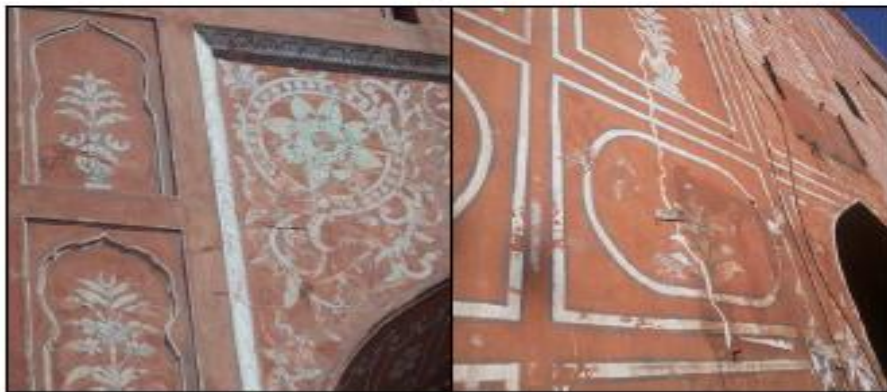
Plaster Crack observed above the arch (front side). Previous cracks which are being monitored with Crack meters
