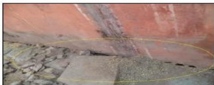
Cavities are formed at wall-ground joint.
