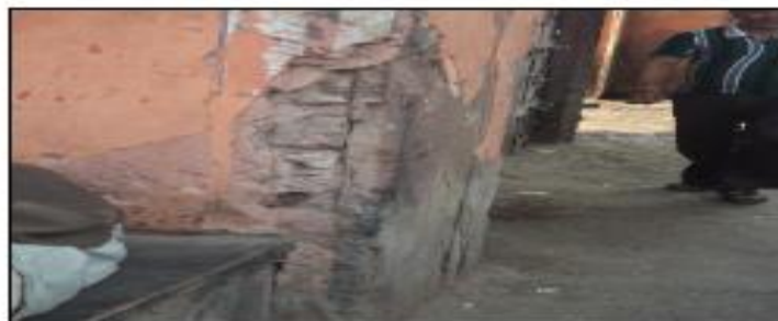
Plaster damaged and stones are exposed.
