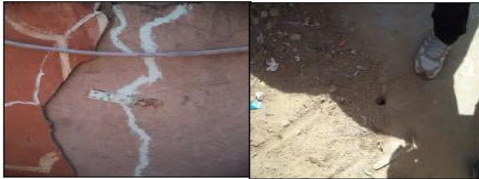
Plaster peeled off of walls on terrace of Gate Structure, Rat Holes are observed near Gate
