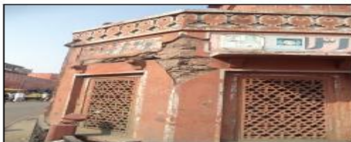
Wall Plaster damaged and stones are exposed.
