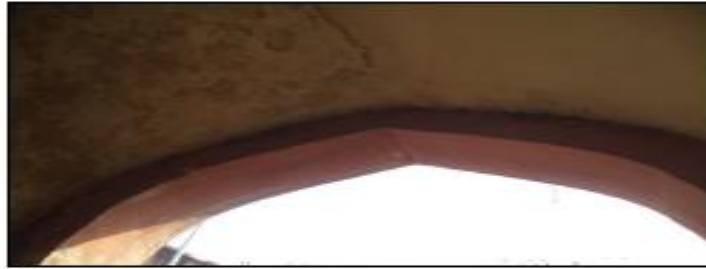
Seepage / Dampness is observed inside structure.
