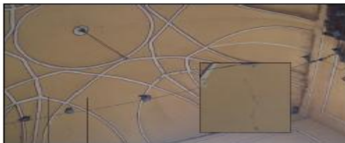
Crack is observed on the vault.
