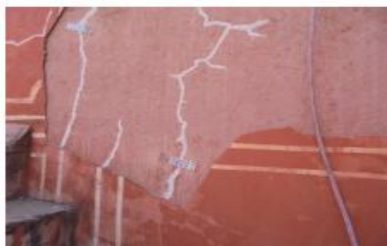
Older plaster cracks on the terrace walls already being monitored. Some of which have marginally expanded but all within permissible limit.
