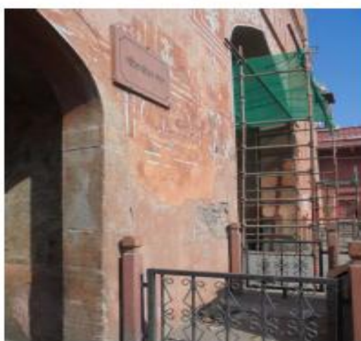
Older inherent problems with the plaster due to age which are unrelated with the TBM passing.
