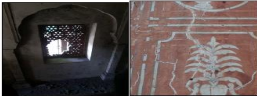
Broken RCC grill. Cracks are being monitored with glass strip to assess widening of cracks
