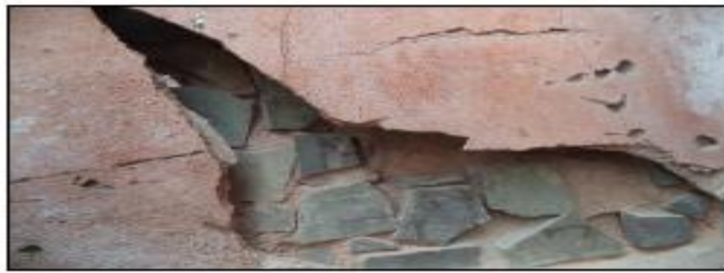
Wall plaster is observed and stones are exposed.
