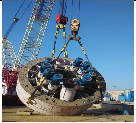
Tilting of TBM-2 at Chandpole Launching Shalft
