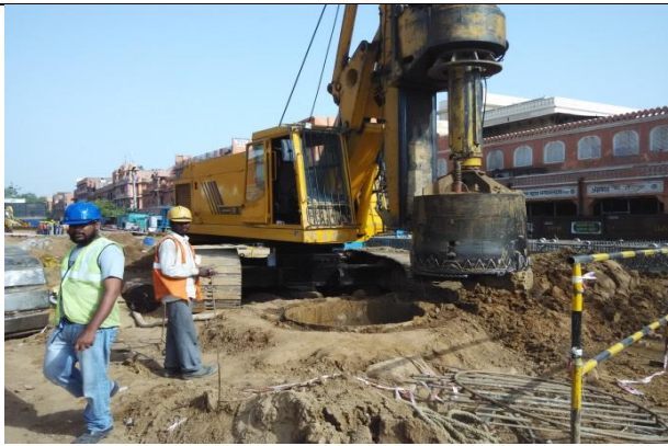
French Collum Excavation at Chhoti Chaupar
