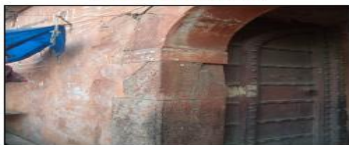
Column plaster damaged and gap is observed between stones
