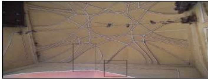
Crack is observed on the vault.
