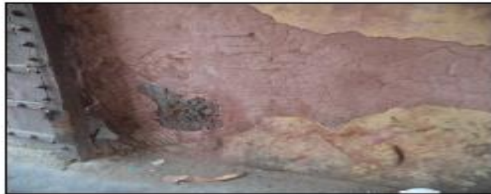
Wall plaster damaged and stones are exposed.
