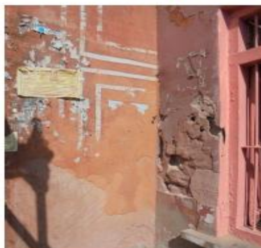
Older inherent problems with the plaster due to age which are unrelated with the TBM passing.
