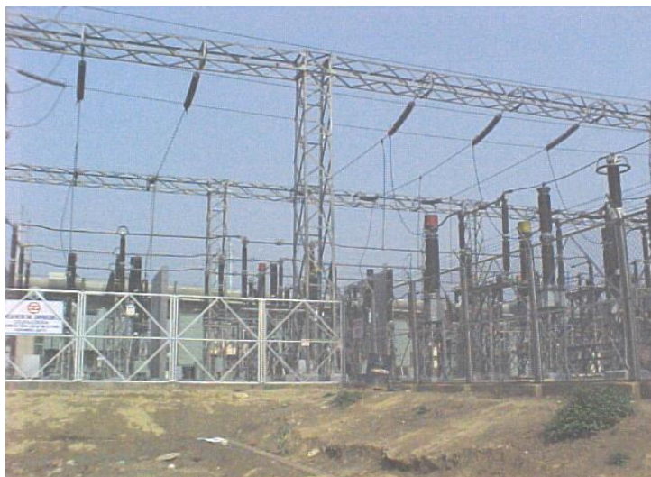
Typical High Voltage Receiving Sub-station
