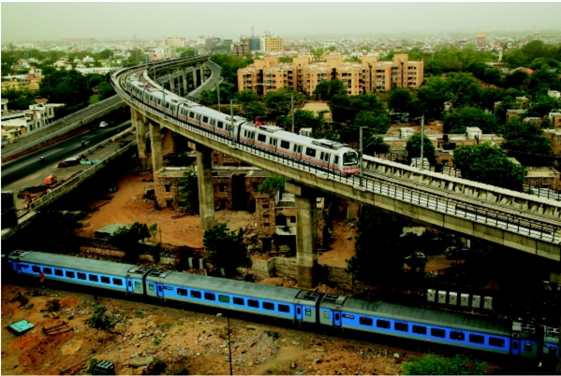
Railway track on the ground level, ROB & elevated road at First level and Metro track at Second level.
