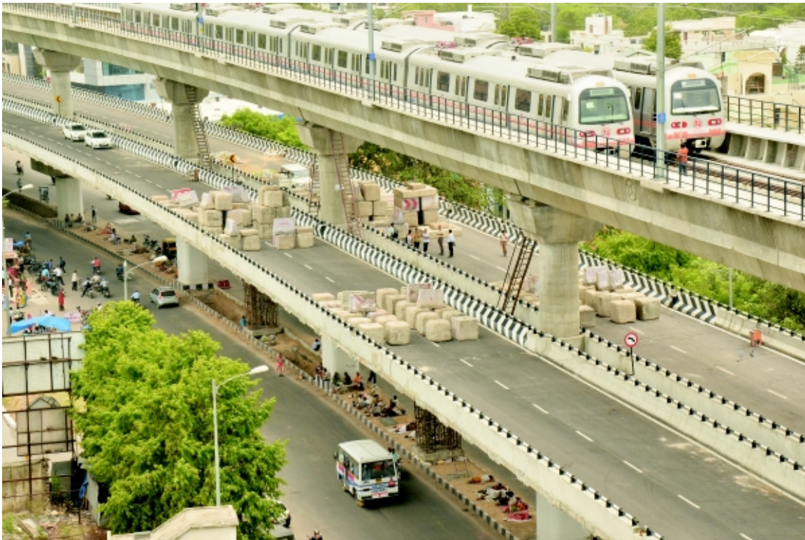
Load testing of double-decked Metro viaduct and elevated road structure on Ajmer Road.
