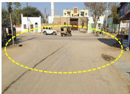
Absence of Road marking for junction
