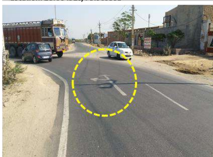
Arrow marking not as per IRC standard
