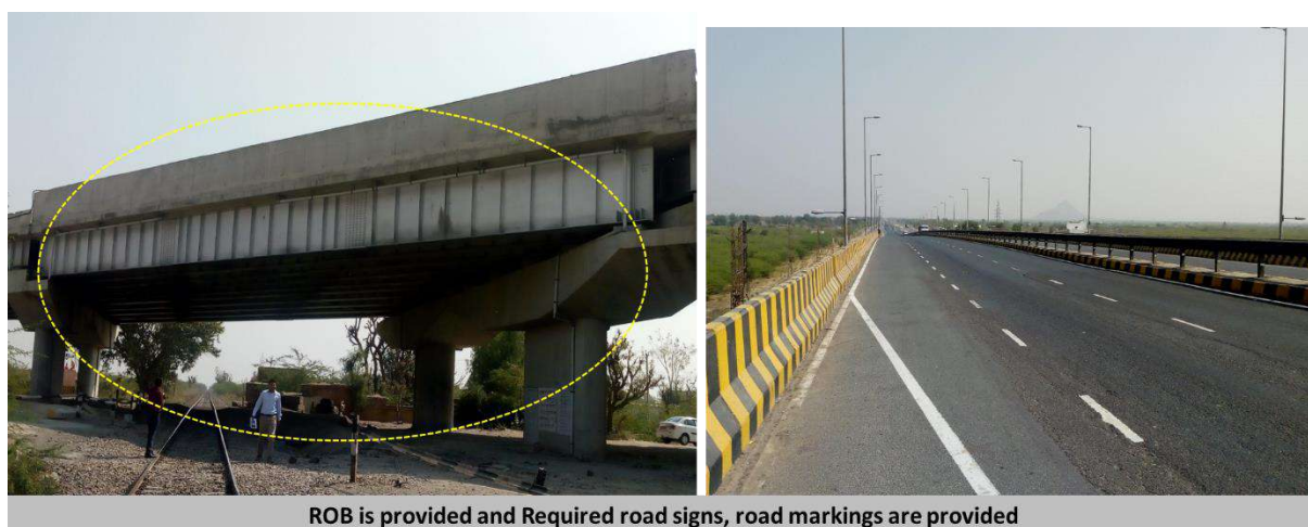
Exhibit 4-10: Visuals of rectification measures at Ch. 104+870 (NH 14)
