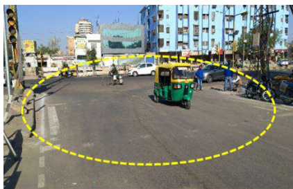
Stop line marking with zebra crossing not visible
