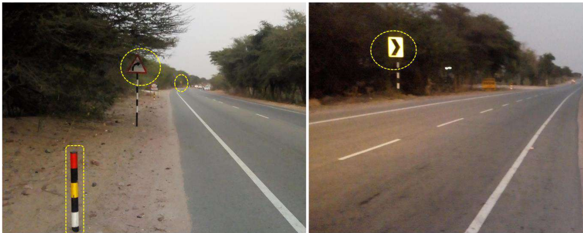
Provision of Road signs ( Cautionary signs) , Road markings , Road delineators ( Road studs, Roadway indicators)
