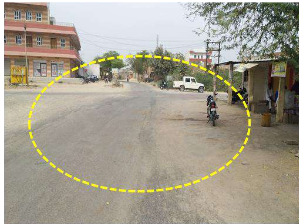
Absence of pavement marking for junction on MDR
