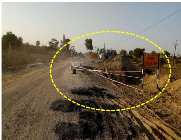
Absence of proper barricades to segregate the work zone from traffic
