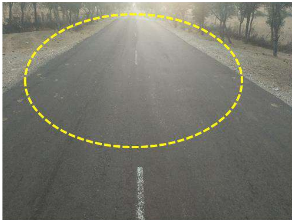
Absence of edge line marking on MDR
