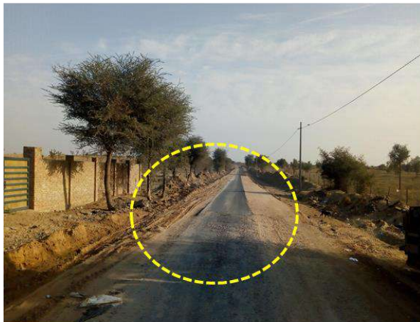
Absence of proper barricades and work zone signs on either side of carriageway
