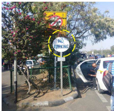
Regulatory Sign not as per IRC Standard
