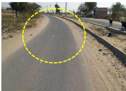
Pavement marking not visible
