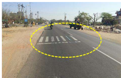
Edge line missing and pedestrian crossing not as per IRC standard
