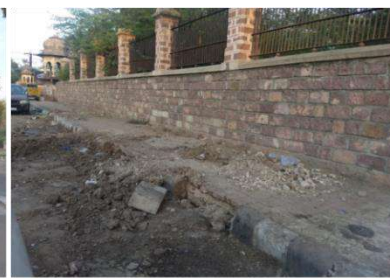
Footpath in poor condition due to improper maintenance
