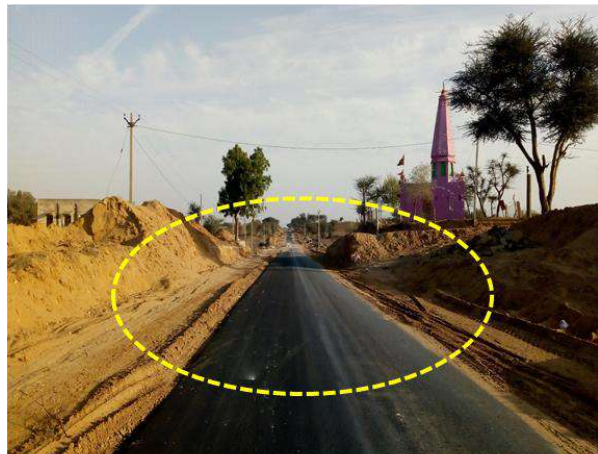
Absence of proper barricades and work zone signs on either side of carriageway
